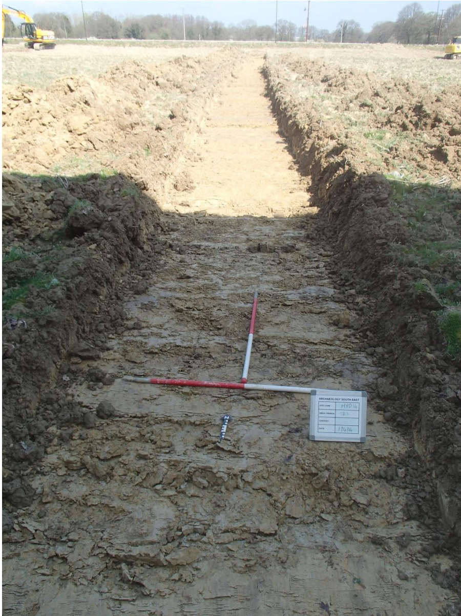
Southern end of Trench 1
