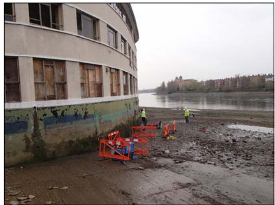
Test pits 7-9, under excavation
