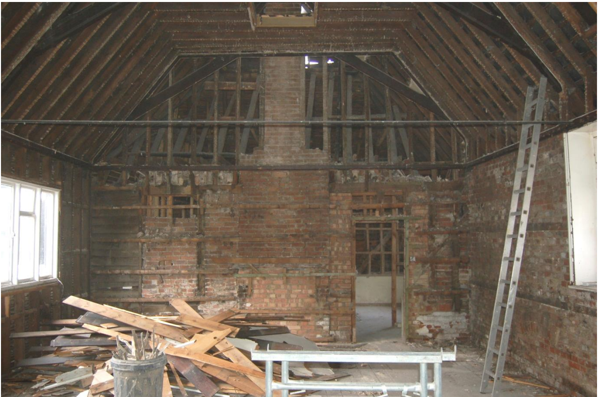
Plate 20 West wall of Room F2 after stripping-out
