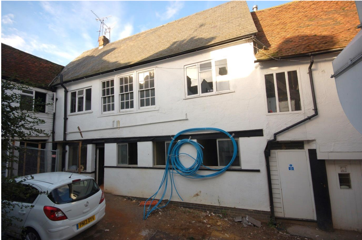
Plate 3 South elevation of Building 2
