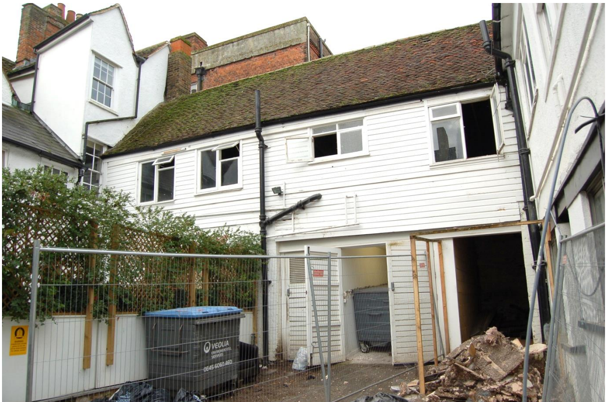
Plate 2 East elevation of Building 1 (east side)
