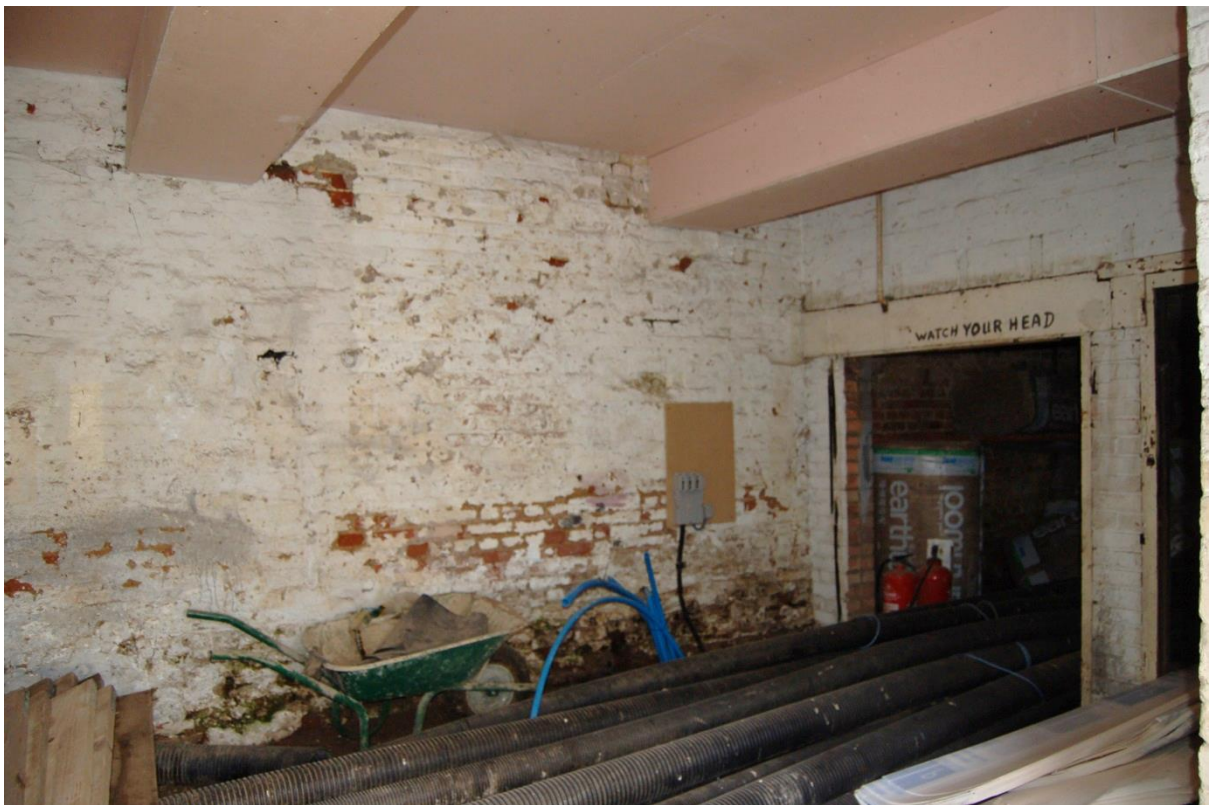
Plate 4 Room G1 and entrance to G2
