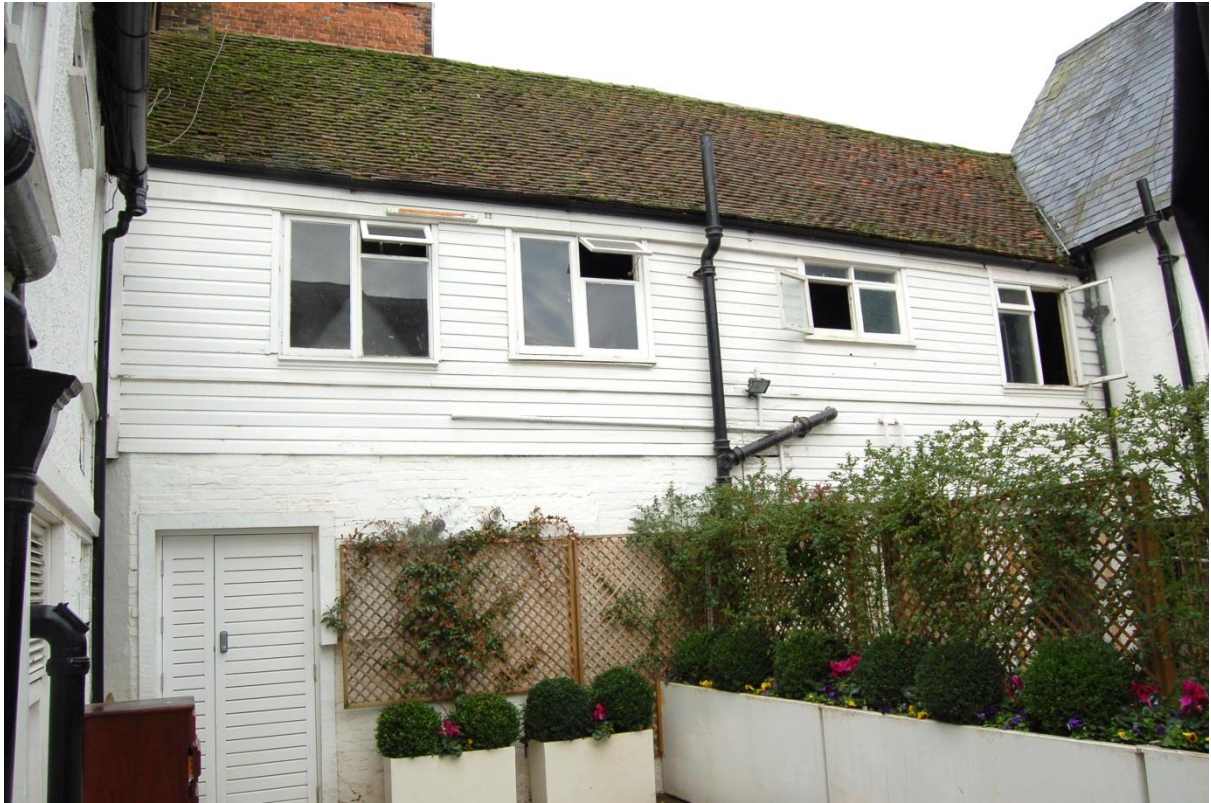
Plate 1 East elevation of Building 1 (west side)
