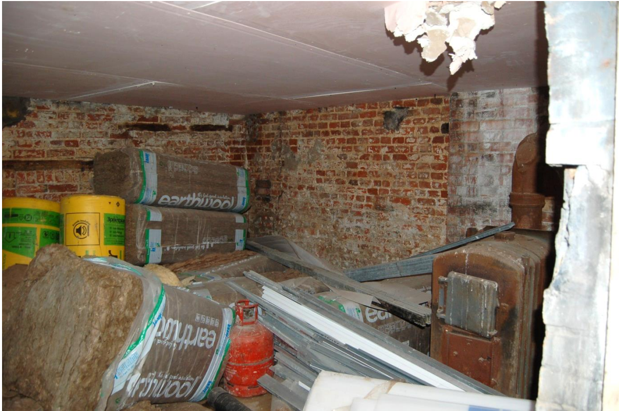
Plate 5 Room G2 viewed to north-west
