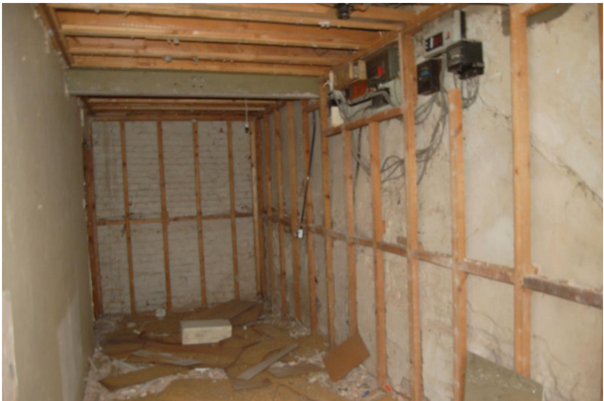
Plate 14 Remains of former stair in Room G5
