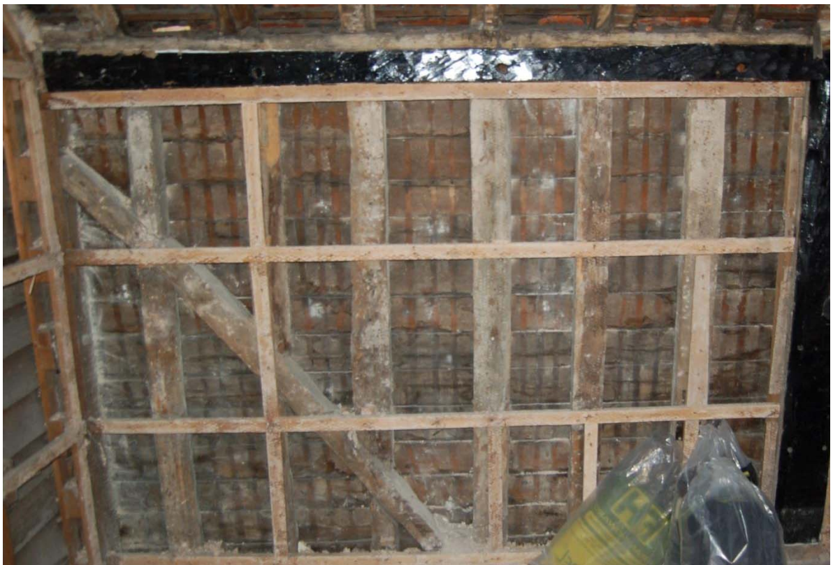
Plate 12 Peg-holes along wall plate in Room F1
