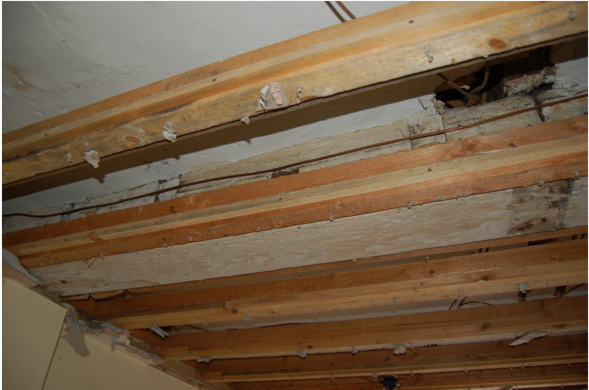
Plate 15 Main joist in Room G5
