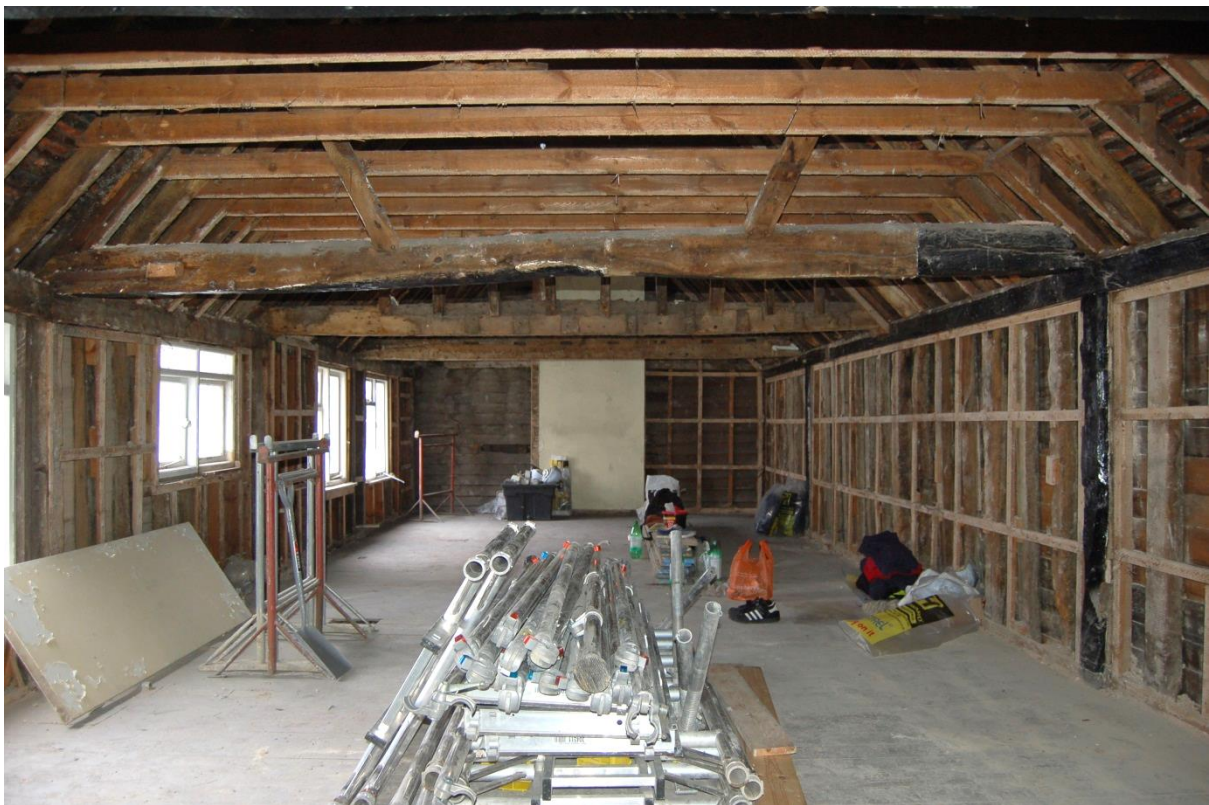
Plate 8 Room F1 viewed to south after stripping-out
