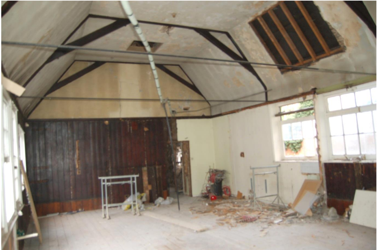
Plate 17 Room F2 viewed to north-west
