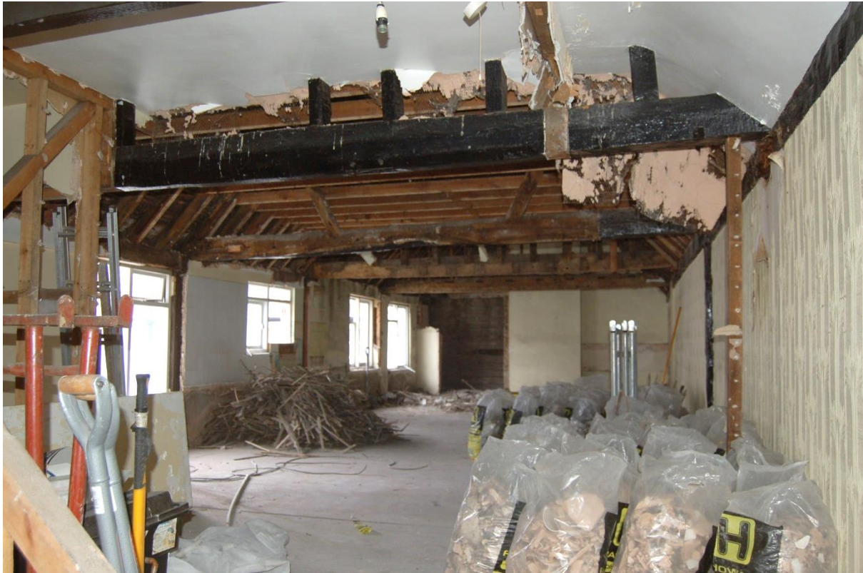
Plate 7 Room F1 viewed to south before stripping-out
