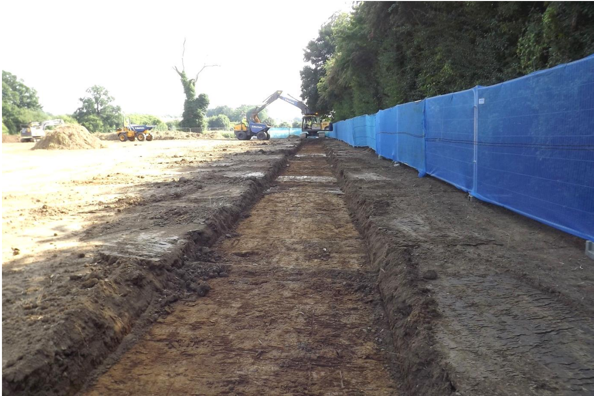
Figure 2: Excavation of access road, viewed to south
