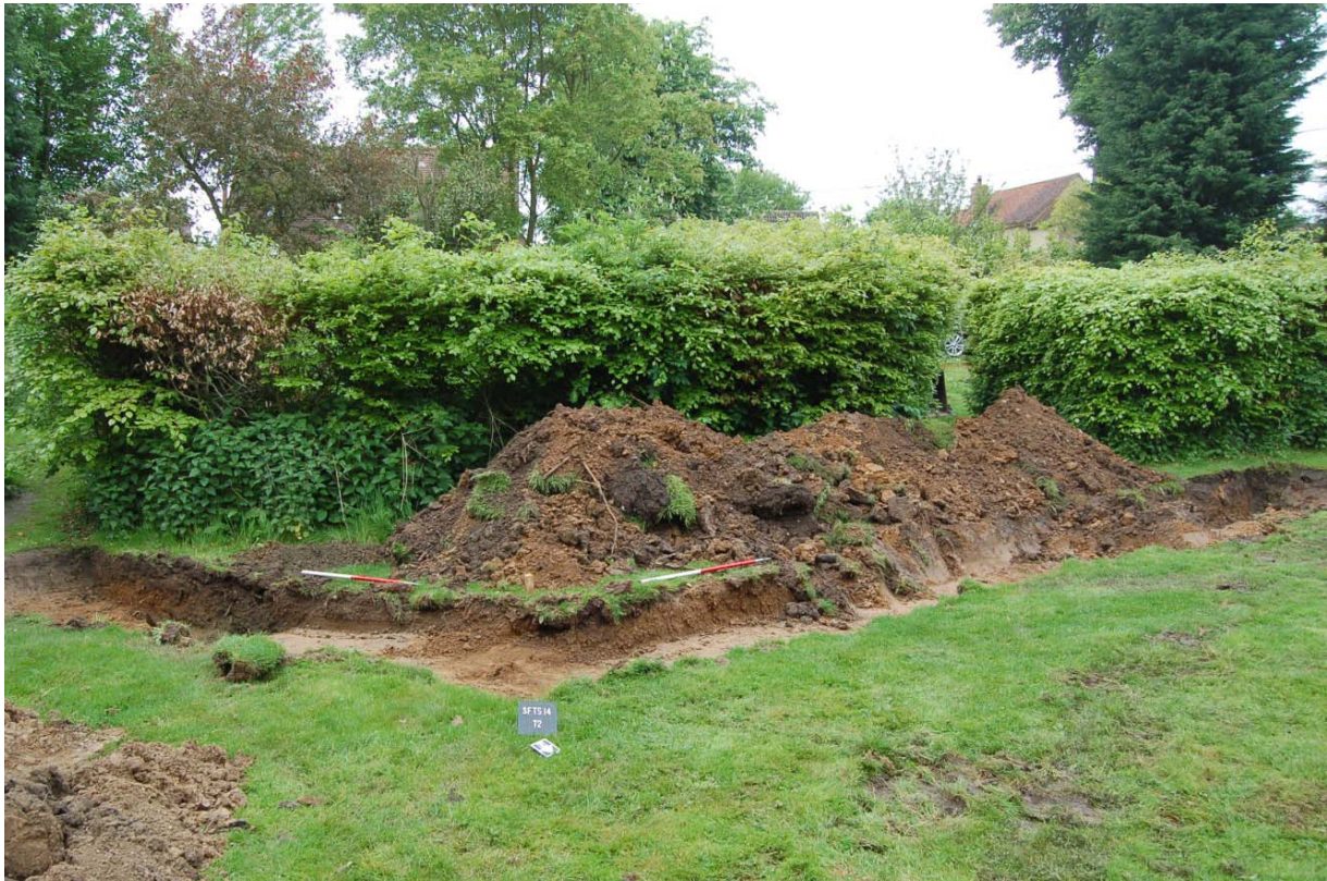
Figure 3 Trench 2 viewed to southwest
