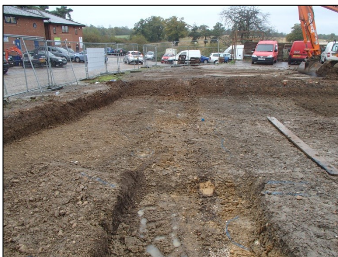
Figure 10: Site looking west, showing (G9) ditch [260] and reworked layers [48 / 240]
