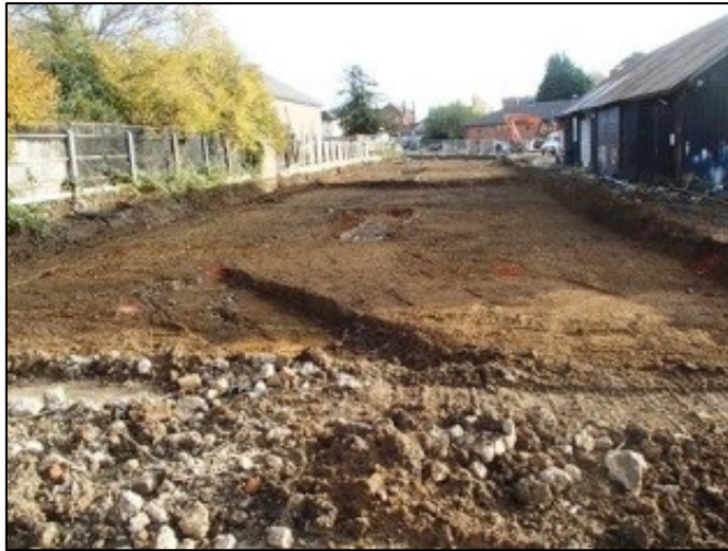
Figure 8: Site view, looking south
