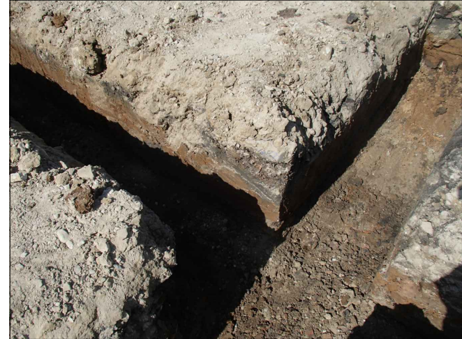
Footings across plots 1-4
