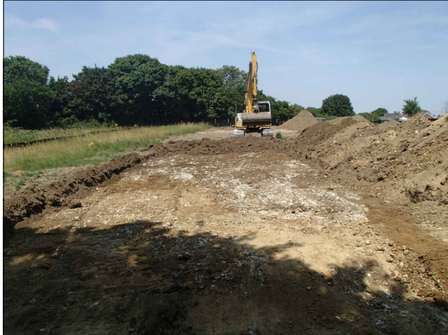
Subsoil strip across plot 8 looking south-west
