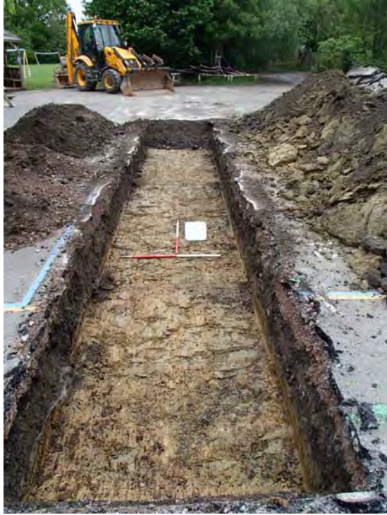
Trench 1 facing east
