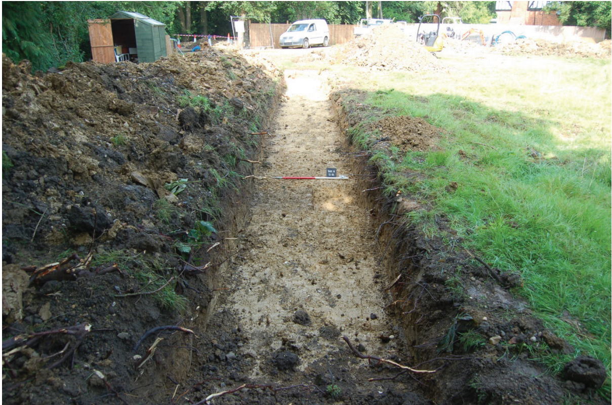
Figure 5: Trench 2 viewed to west (1m scale)
