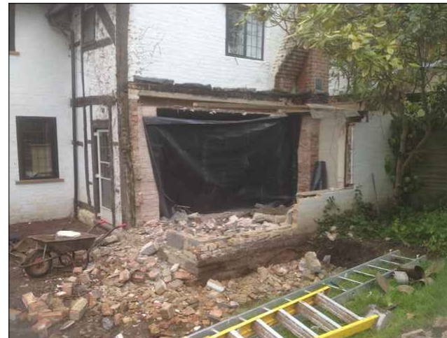
Extension during demolition, looking northeast (photo: client)
