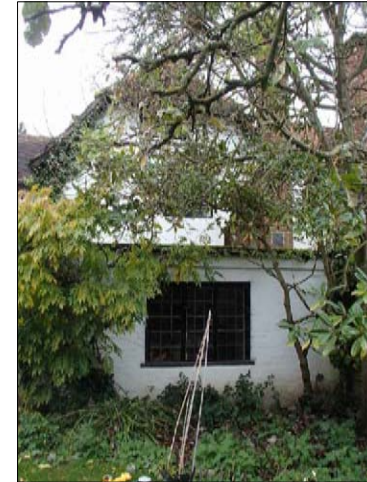
House and extension, looking north
