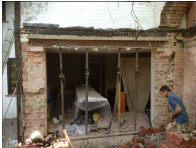
Extension during demolition, looking north (photo: client)
