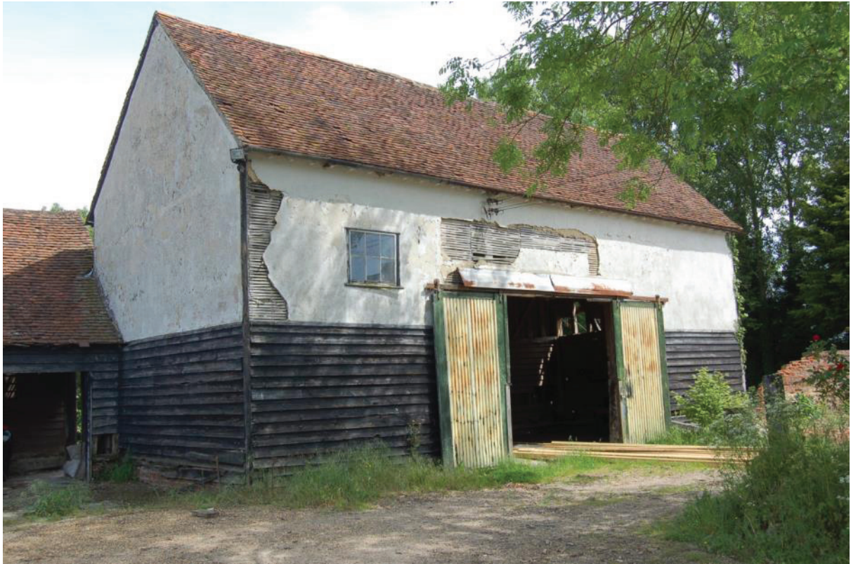
Plate 3 Barn viewed to north-east
