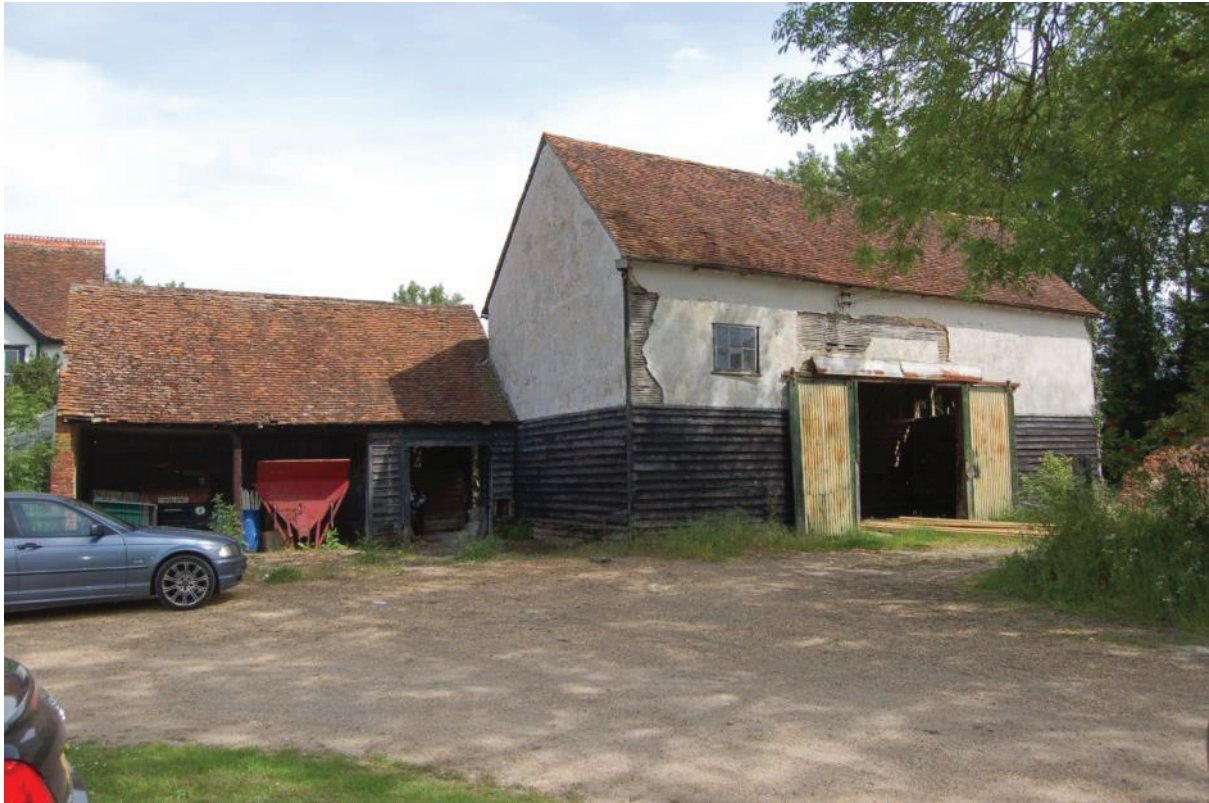
Plate 1 Barn and cart lodge viewed to north-east
