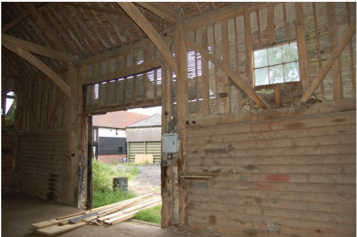
Plate 8 Internal south wall
