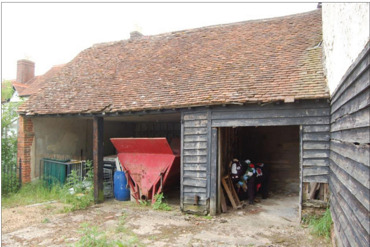
Plate 12 South elevation of cart lodge
