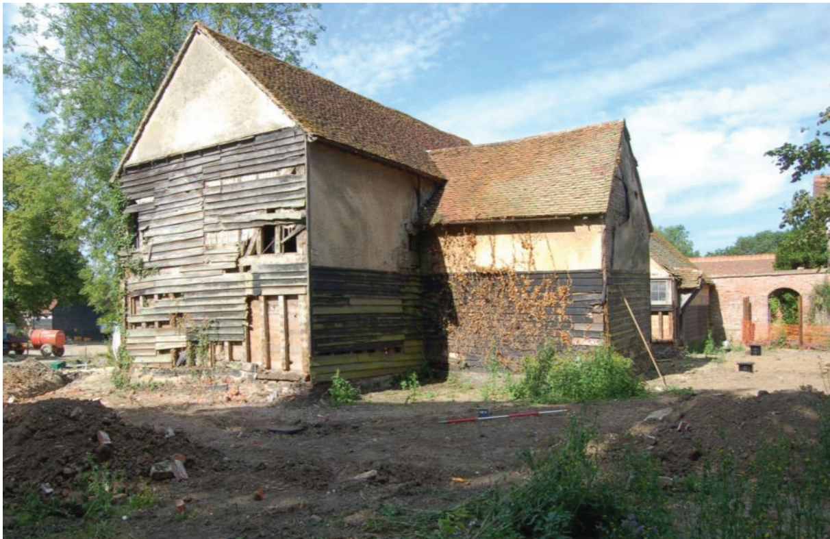
Plate 22 Location of pipe trench, viewed to south-west
