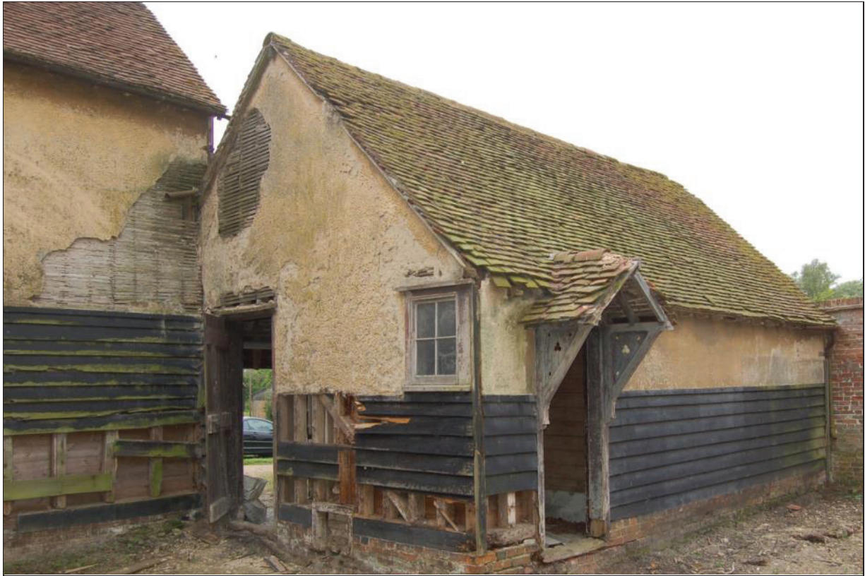
Plate 13 Rear of cart lodge viewed to south-west, showing blocked aperture at base of wall
