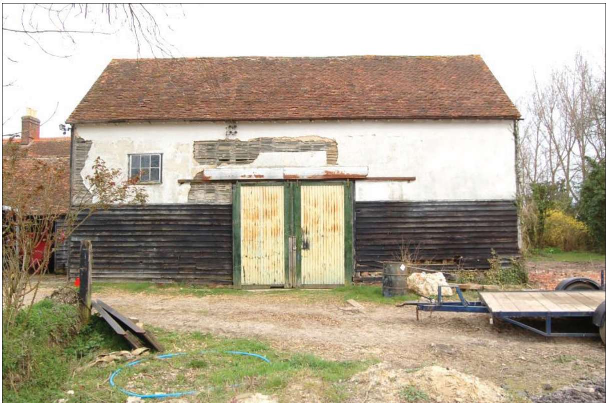
Plate 5 Barn viewed to north
