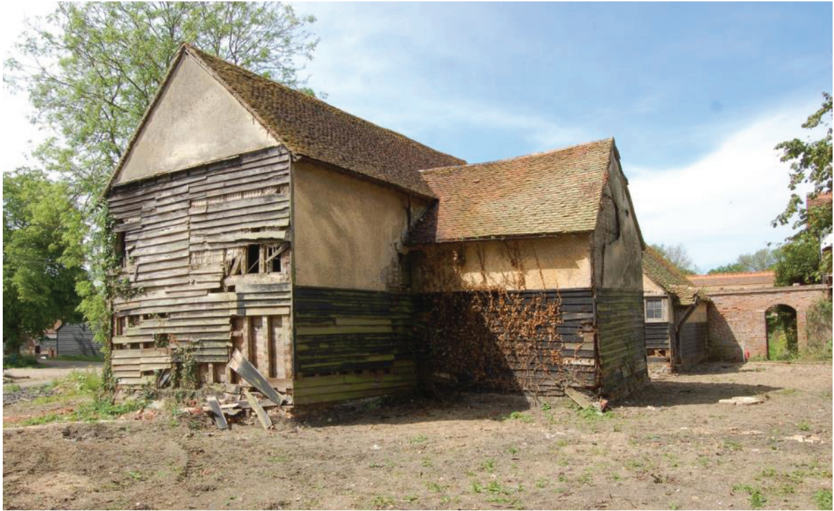
Plate 5 Barn viewed to south-west
