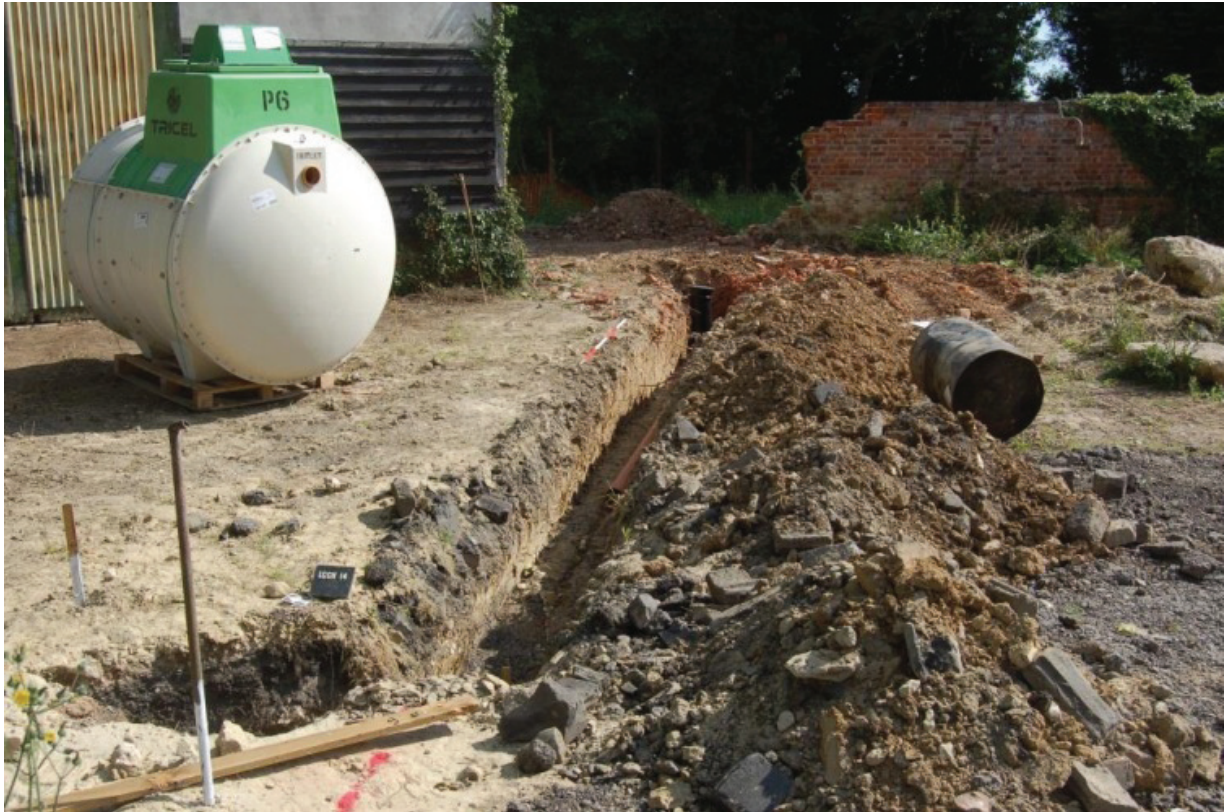
Plate 23 Pipe trench at front of barn, viewed to north-east
