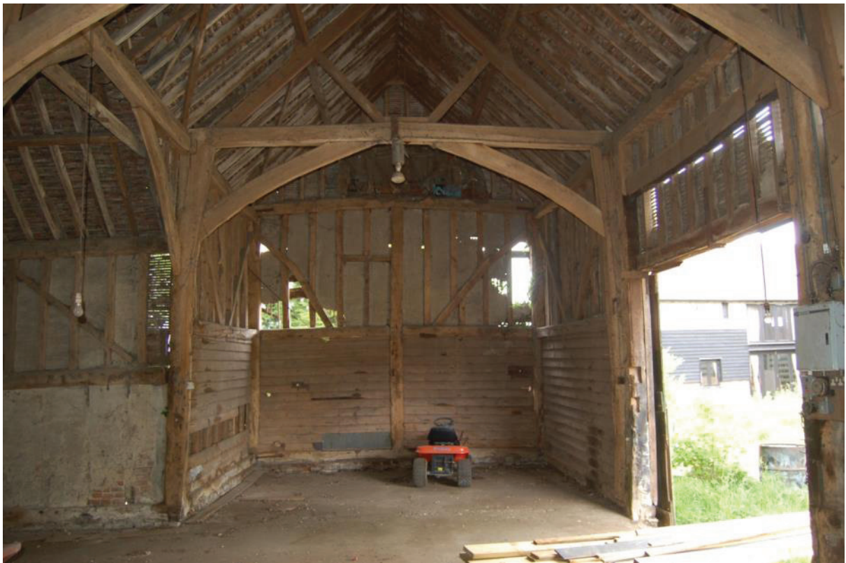
Plate 6 Interior of barn viewed to east
