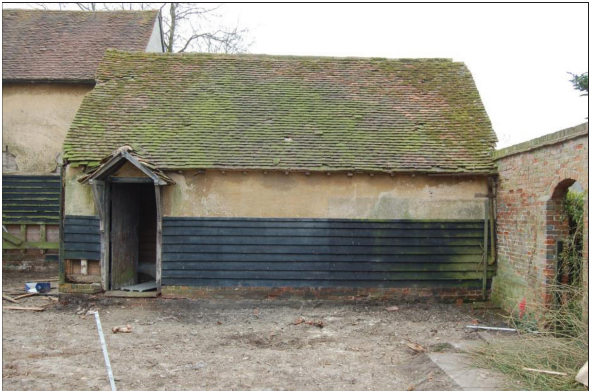
Plate 14 North elevation of cart lodge
