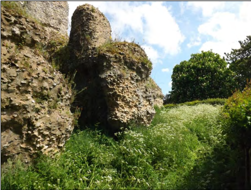
Figure 4: Keep forebuilding prior to investigation
