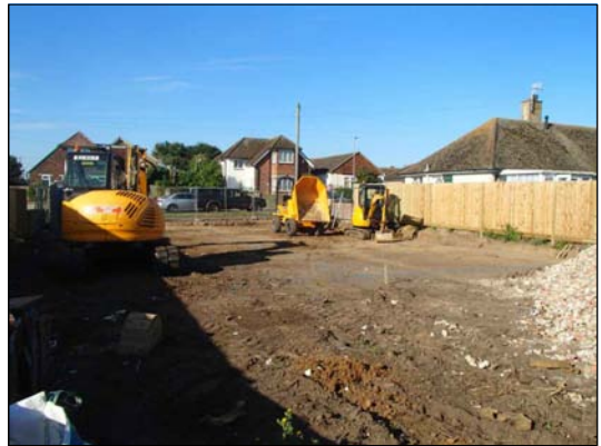
The site prior to construction work looking south
