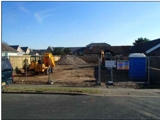
The site prior to construction work, looking north
