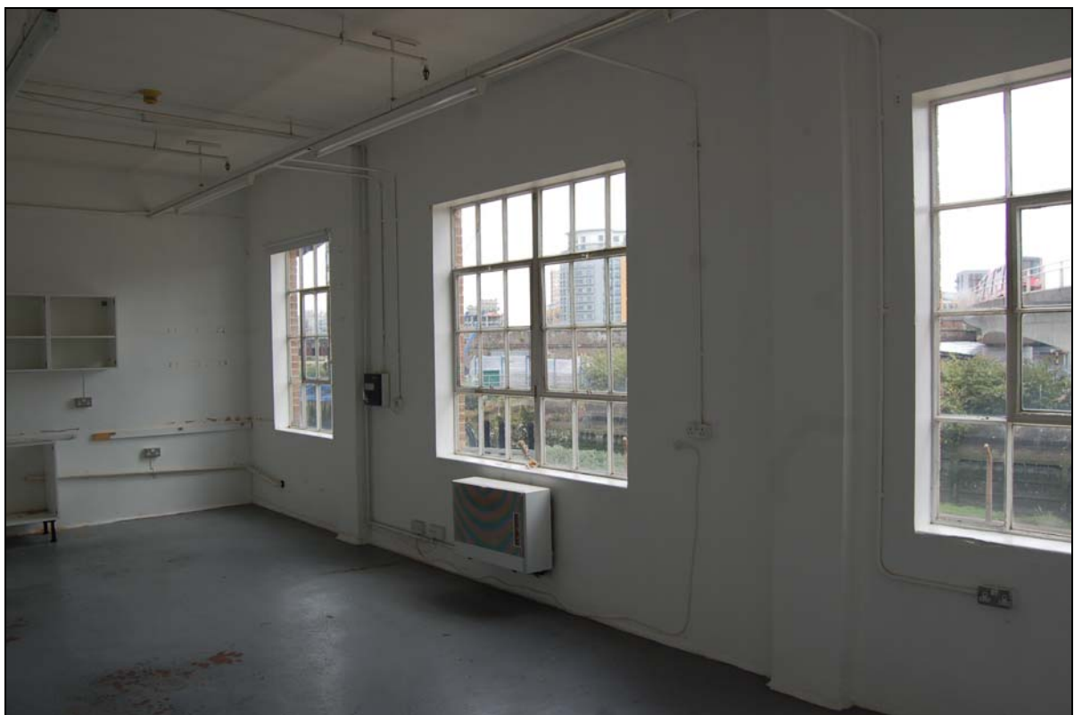
Plate 38. Building B, first floor, unit B108 (FCQ14-0118)
