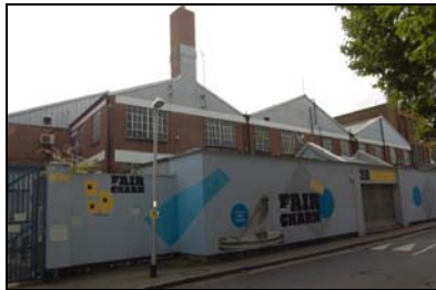
FCQ14-0004 Building A, Creekside elevation
