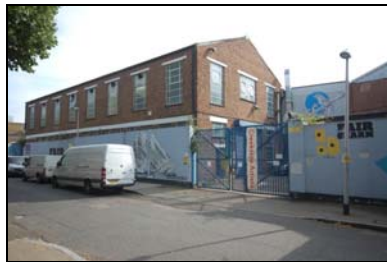
FCQ14-0164 Building C, oblique view, west and south elevations
