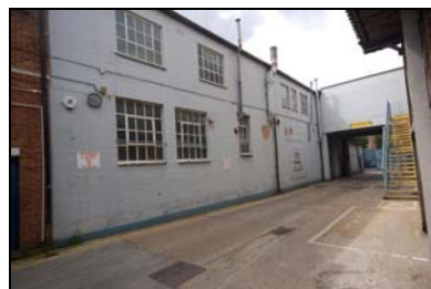
FCQ14-0011 Building A, north facing elevation
