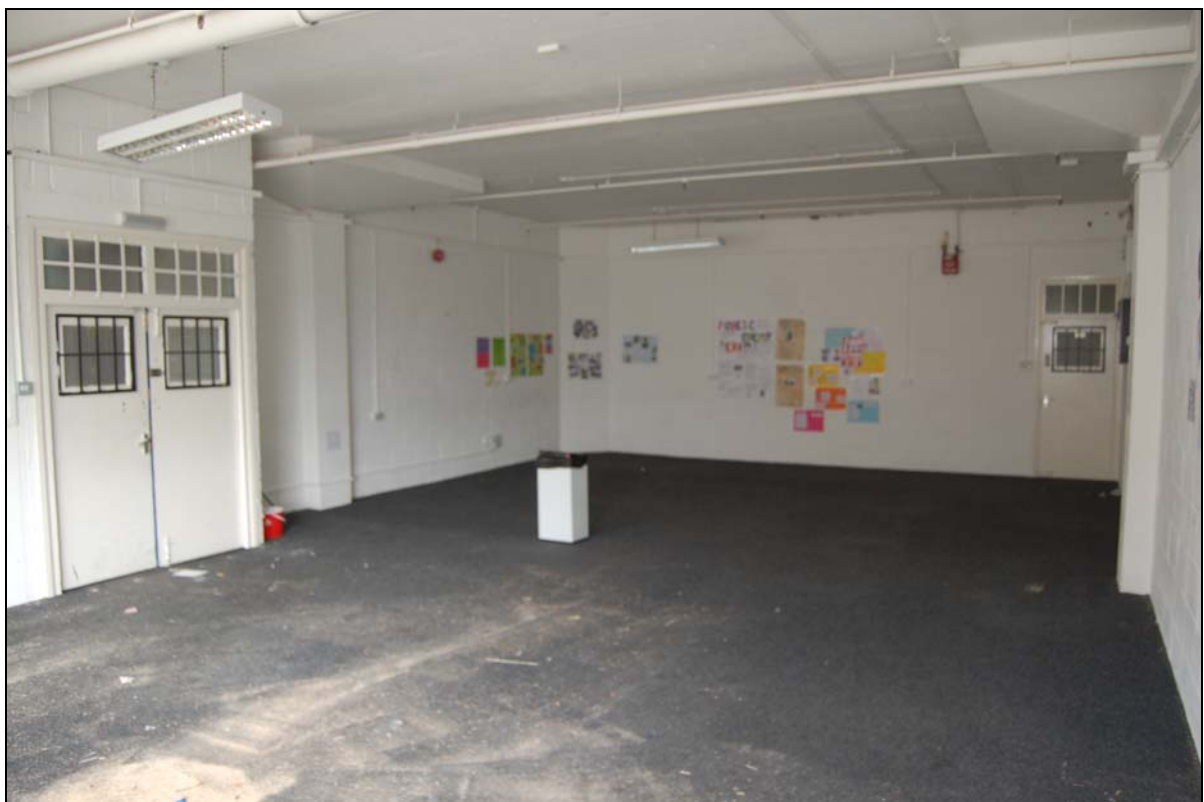
Plate 40. Building B, first floor, unit B114 (FCQ14-0109)
