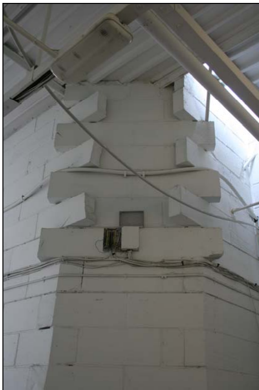
Plate 42. Building B, second floor, detail of chamfered breeze block wall (FCQ14-0142)
