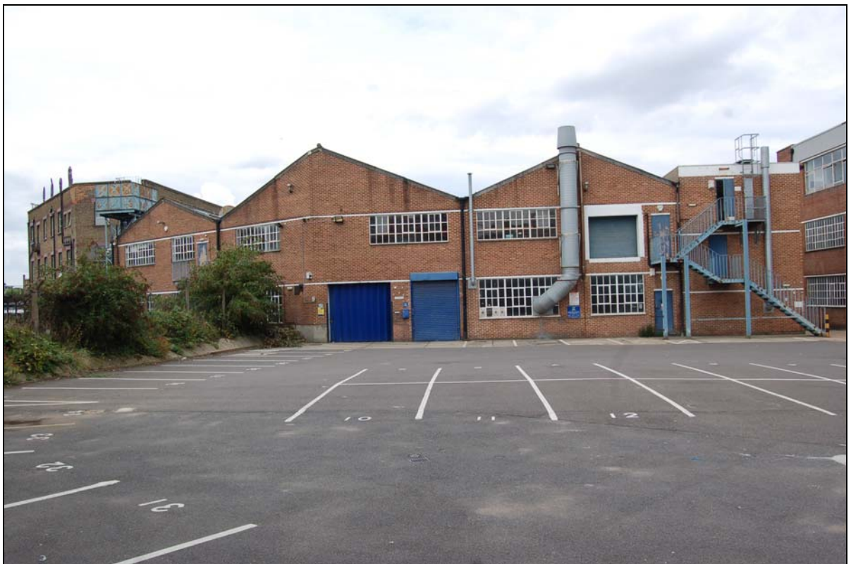
Plate 6. Building A, east facing (rear) elevation (FCQ14-0007)
