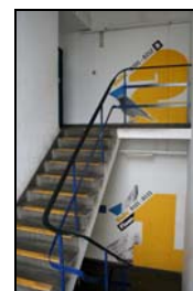
FCQ14-0120 Building B, first floor, stairs
