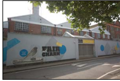
FCQ14-0002 Building A, Creekside elevation
