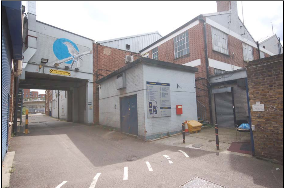
Plate 3. Building A, oblique view of north and west facing elevations (FCQ14-0012)
