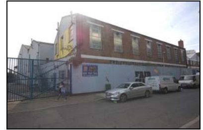
FCQ14-0162 Building C, west elevation
