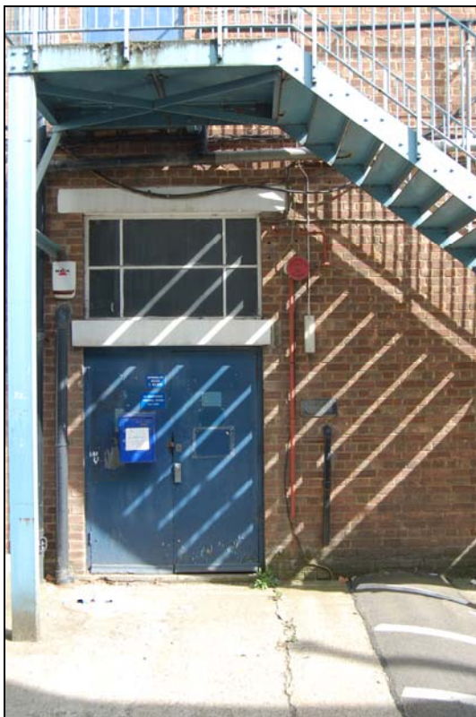
Plate 52. Building C, south elevation (FCQ14-0166)
