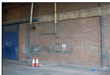
FCQ14-0167 Building C, east elevation
