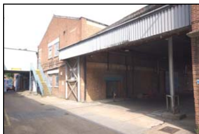
FCQ14-0155 Building C, oblique view, south and east elevations
