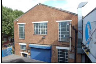
FCQ14-0145 Building C, south elevation
