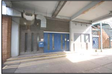
FCQ14-0160 Building C, south elevation
