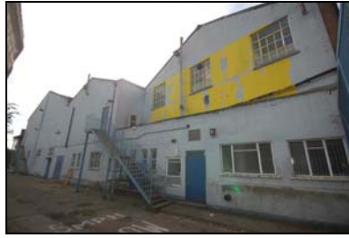
FCQ14-0158 Building C, north elevation
