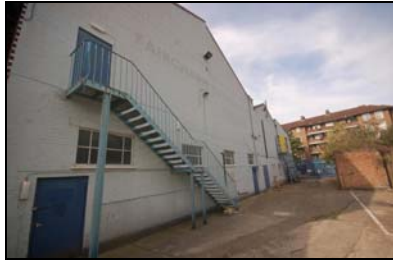
FCQ14-0157 Building C, north elevation
