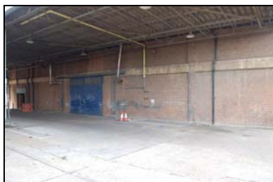
FCQ14-0154 Building C, east elevation
