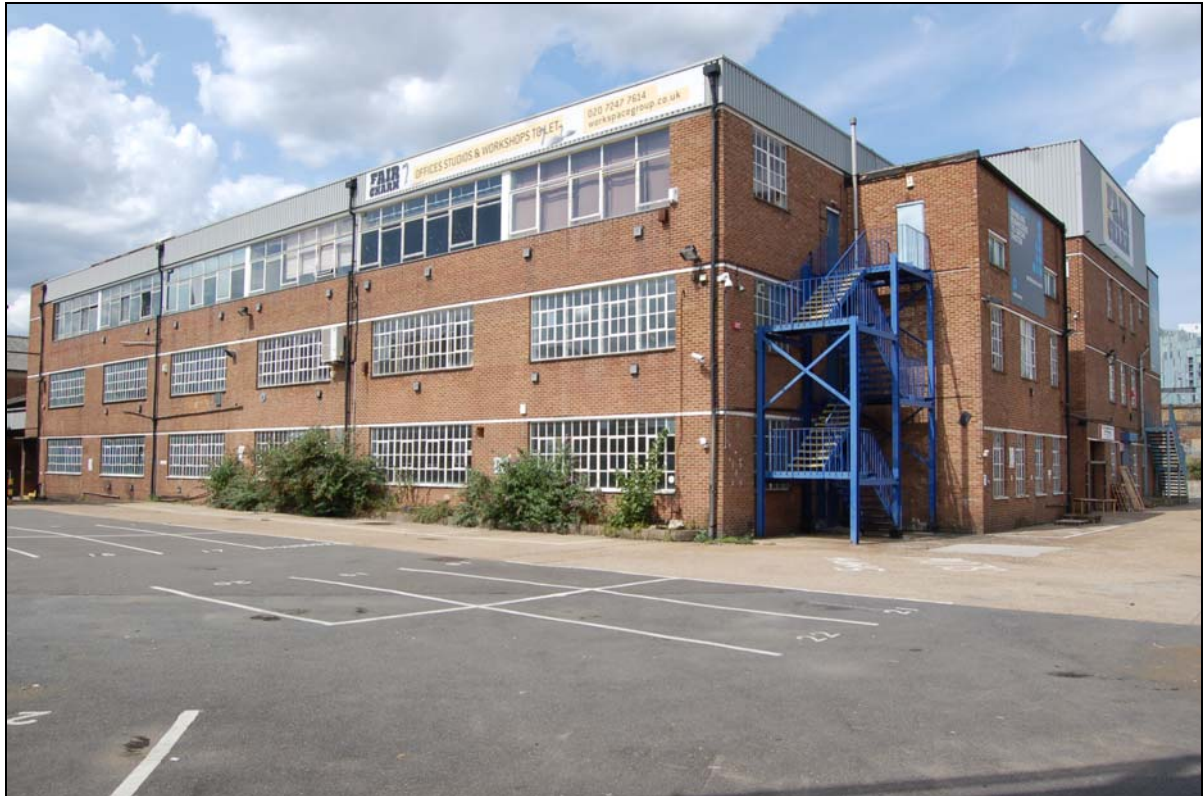
Plate 23. Building B, south elevation (FCQ14-0086)
