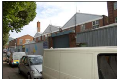
FCQ14-0005 Building A, Creekside elevation
