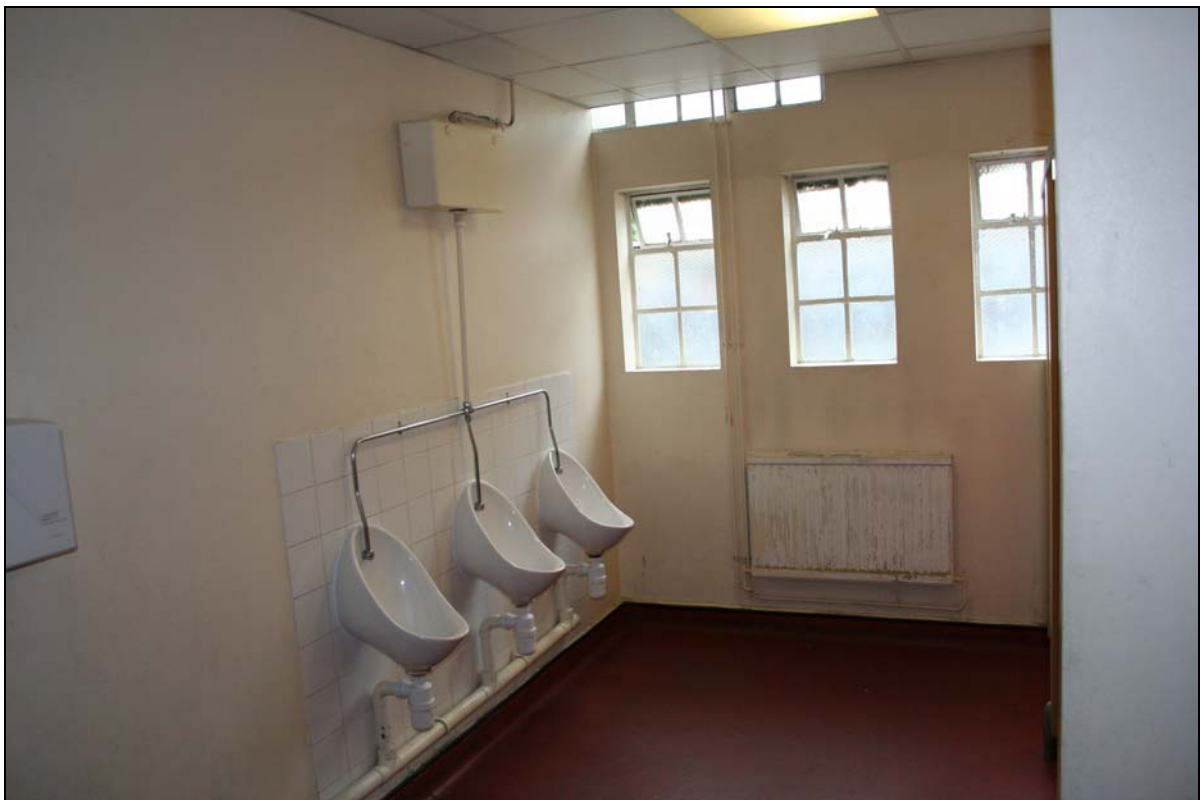
Plate 14. Building A, ground floor toilets (FCQ14-0049)
