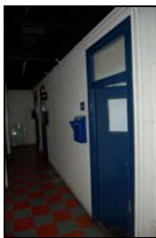
FCQ14-0115 Building B, first floor, corridor
