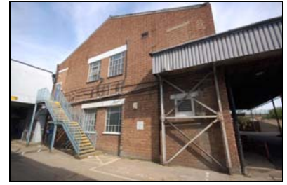
FCQ14-0159 Building C, south elevation
