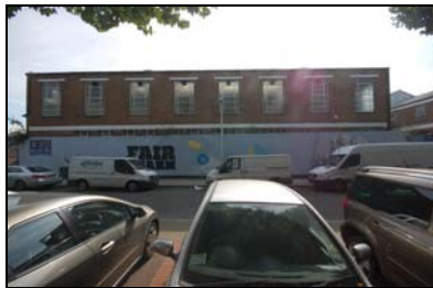
FCQ14-0163 Building C, west elevation
