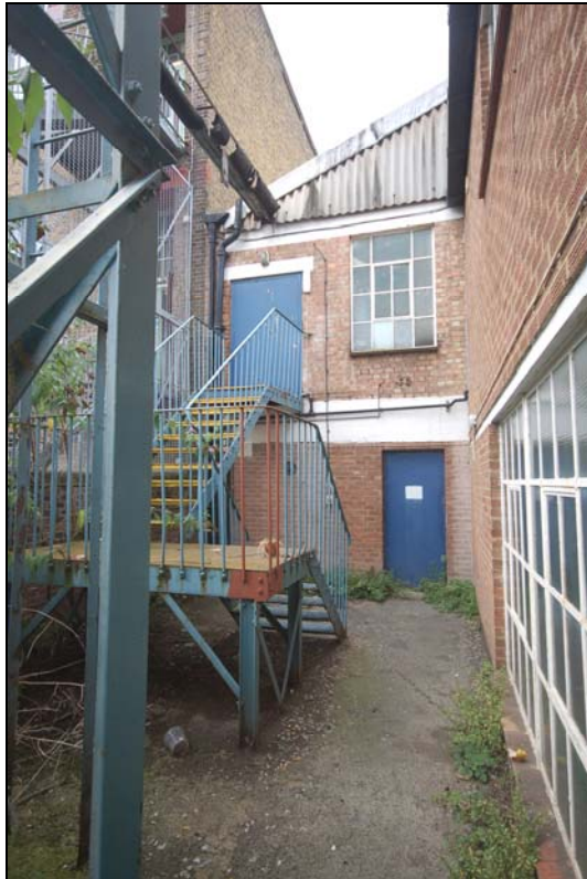
Plate 9. Building A, elevation to Deptford Creek (FCQ14-0018)
