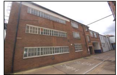
FCQ14-0009 Building A, north facing elevation
