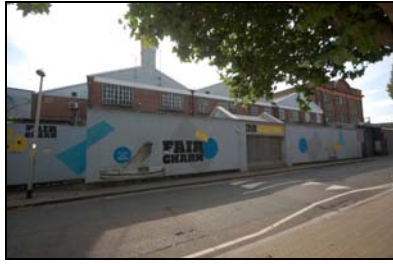
FCQ14-0001 Building A, Creekside elevation
