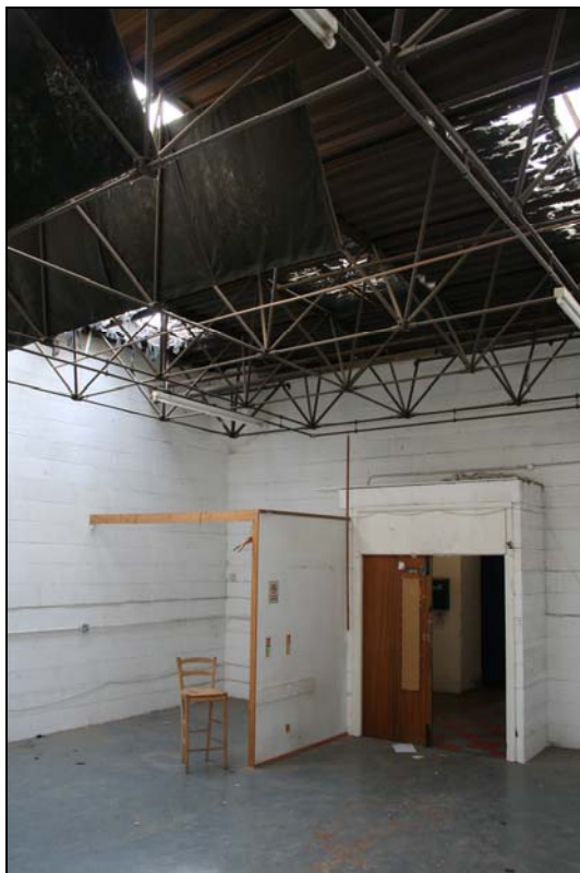
Plate 44. Building B, second floor, unit B205a (FCQ14-0130)
