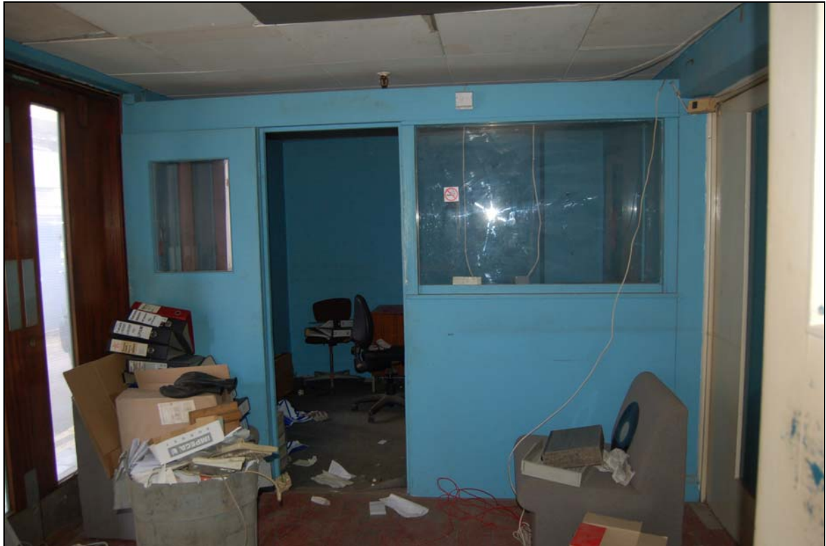
Plate 59. Building C, ground floor, office (FCQ14-0178)
