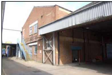
FCQ14-0151 Building C, oblique view, south and east elevations
