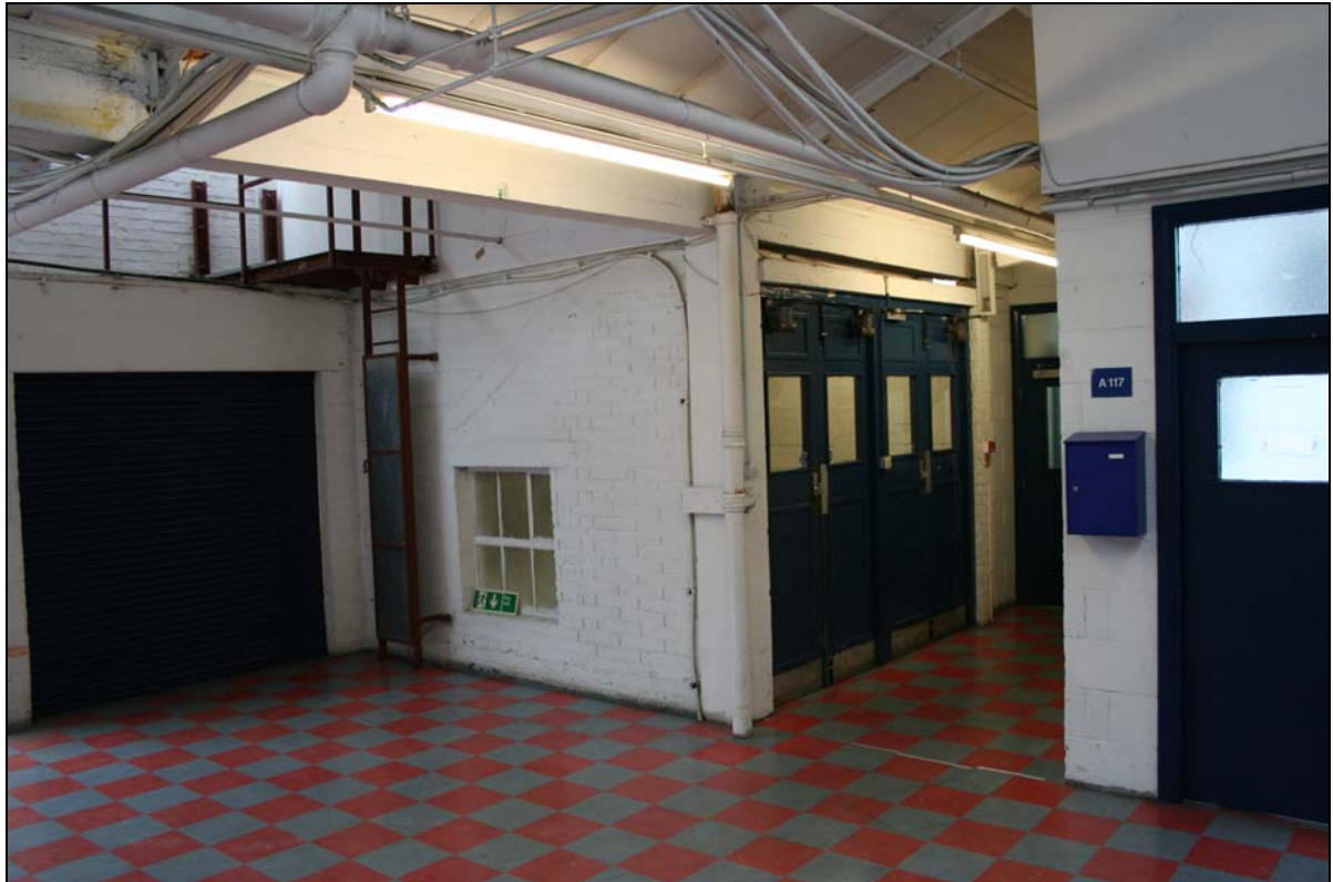
Plate 19. Building A, first floor, lift / stairs area (FCQ14-0064)
