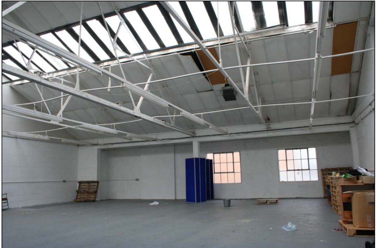
Plate 21. Building A, first floor, room A107/A109 (FCQ14-0073)
