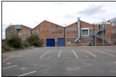
FCQ14-0007 Building A, east facing (rear) elevation
