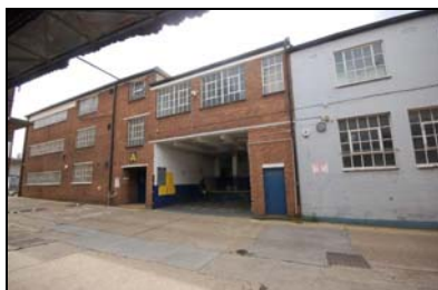
FCQ14-0010 Building A, north facing elevation
