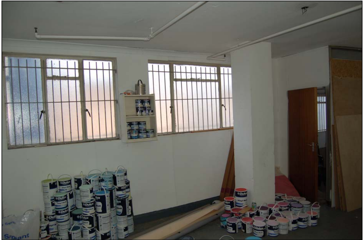
Plate 57. Building C, ground floor, unit 1 (FCQ14-0174)
