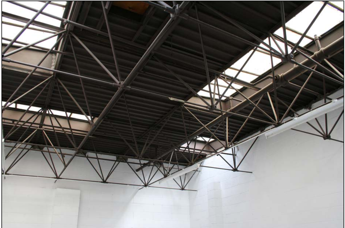
Plate 47. Building B, second floor, roof truss, unit B204 (FCQ14-0141)
