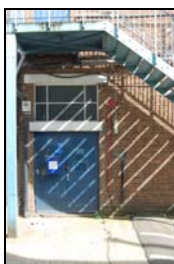
FCQ14-0166 Building C, south elevation
