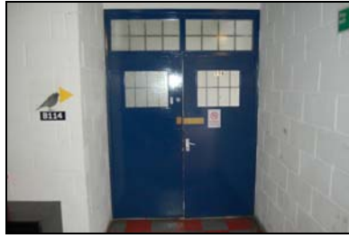
FCQ14-0110 Building B, first floor, double doors to unit B114
