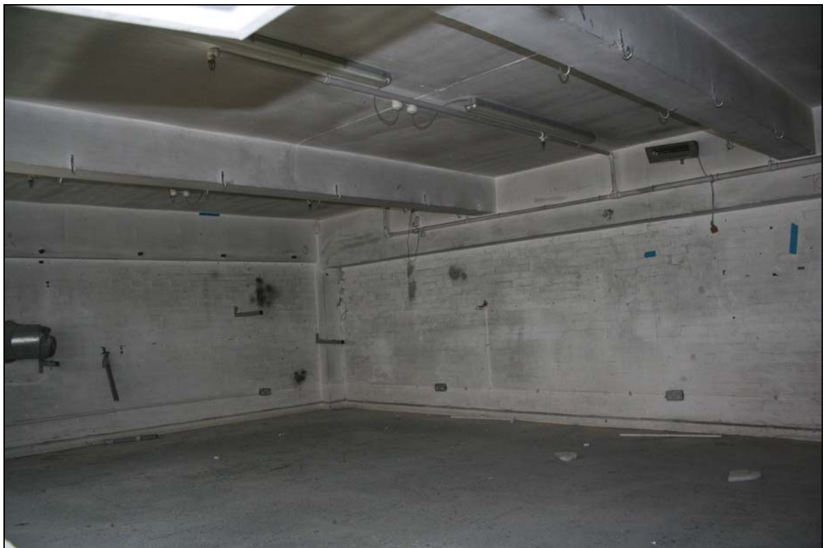
Plate 16. Building A, ground floor, store to north of room A3 (FCQ14-0056)
