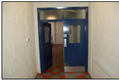
FCQ14-0112 Building B, first floor, double doors in corridor
