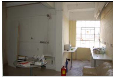
FCQ14-0113 Building B, first floor, unit B105
