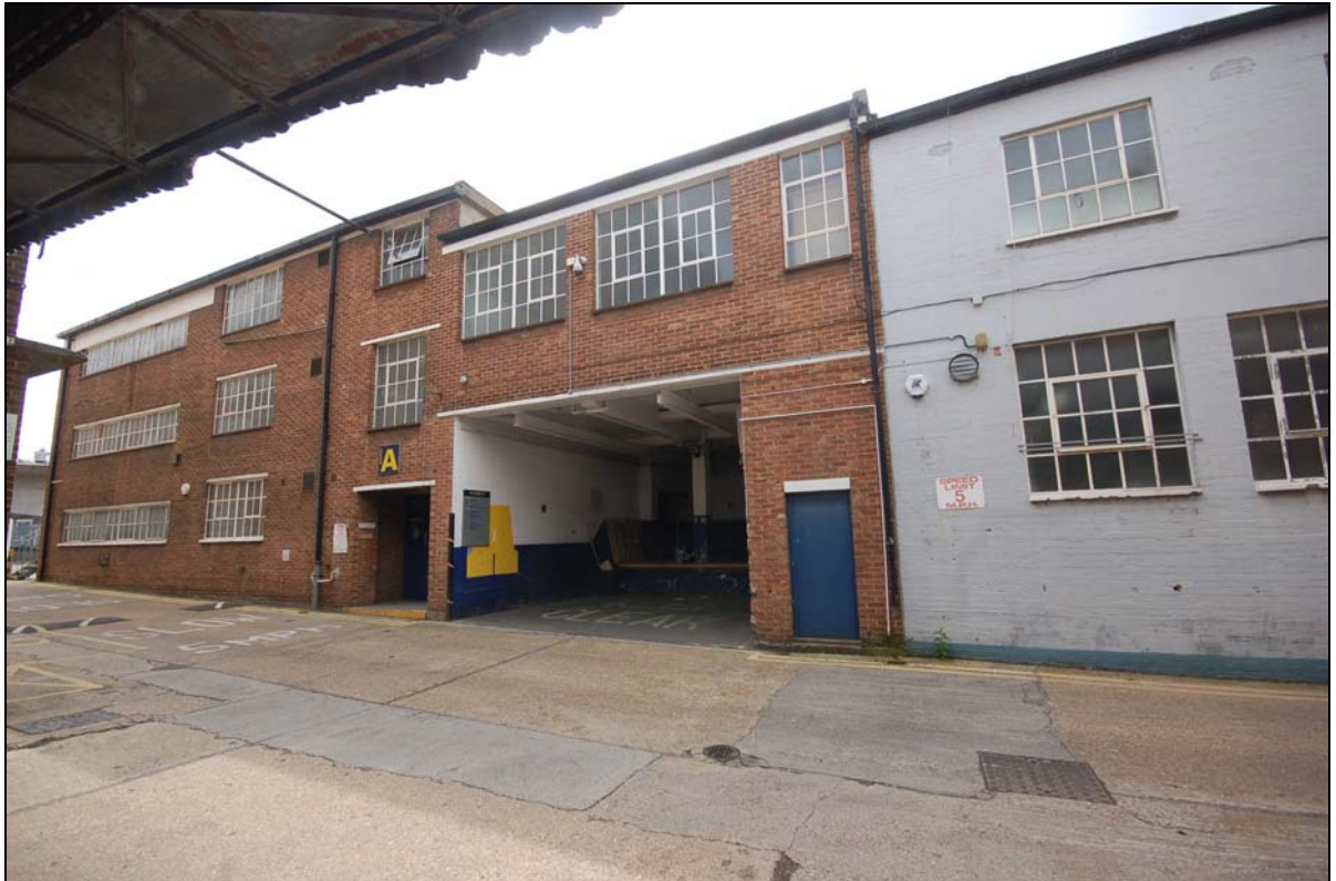
Plate 5. Building A, north facing elevation (FCQ14-0010)
