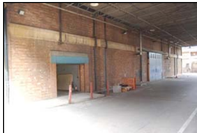
FCQ14-0152 Building C, east elevation
