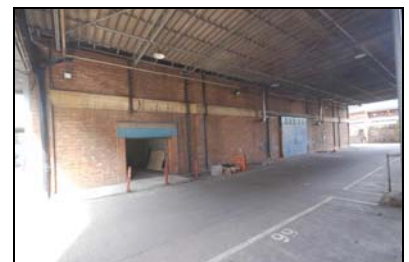
FCQ14-0156 Building C, east elevation
