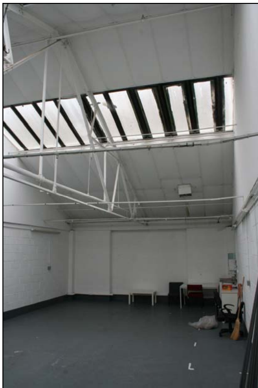
Plate 20. Building A, first floor, room A117 (FCQ14-0066)
