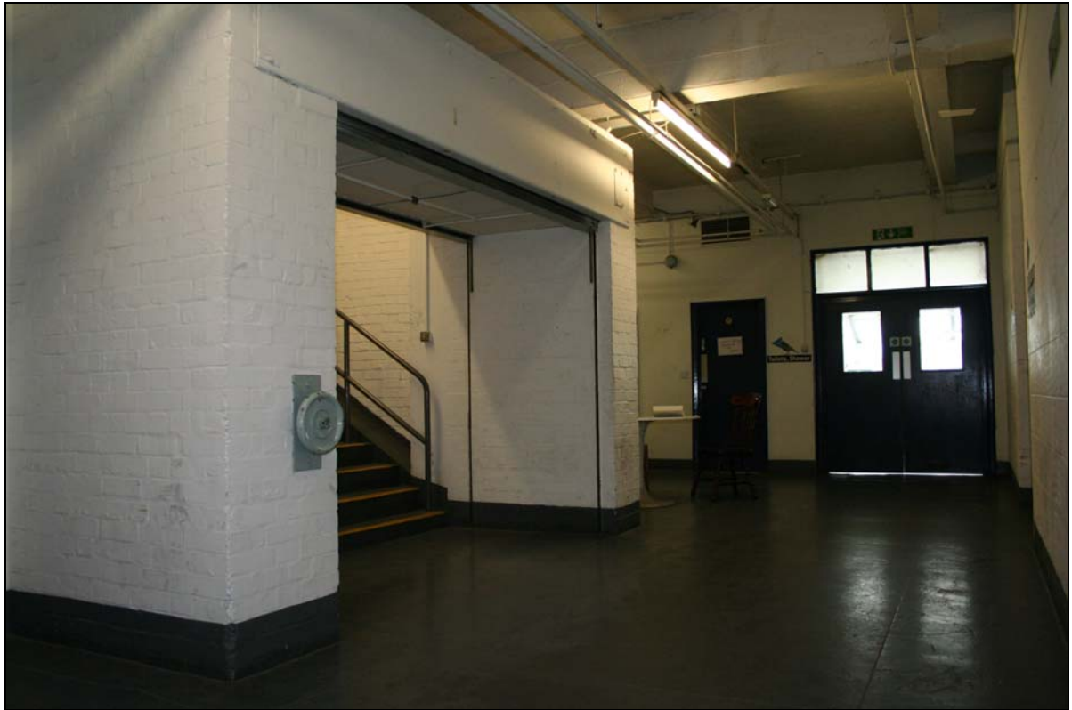
Plate 17. Building A, ground floor, main stairs to first floor (FCQ14-0042)
