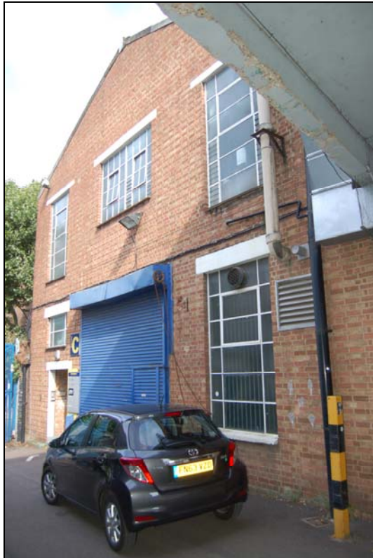
Plate 49. Building C, south elevation (FCQ14-0149)
