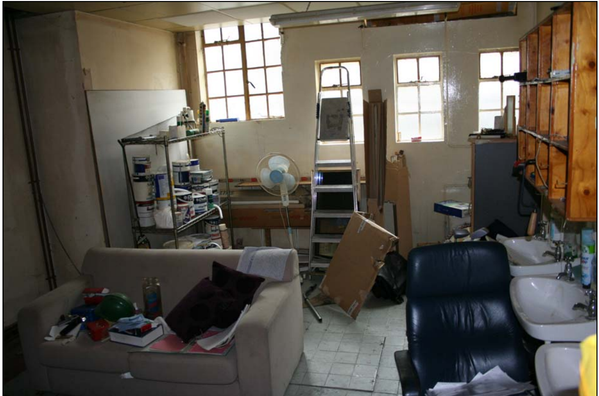
Plate 15. Building A, ground floor, disused toilets (FCQ14-0048)
