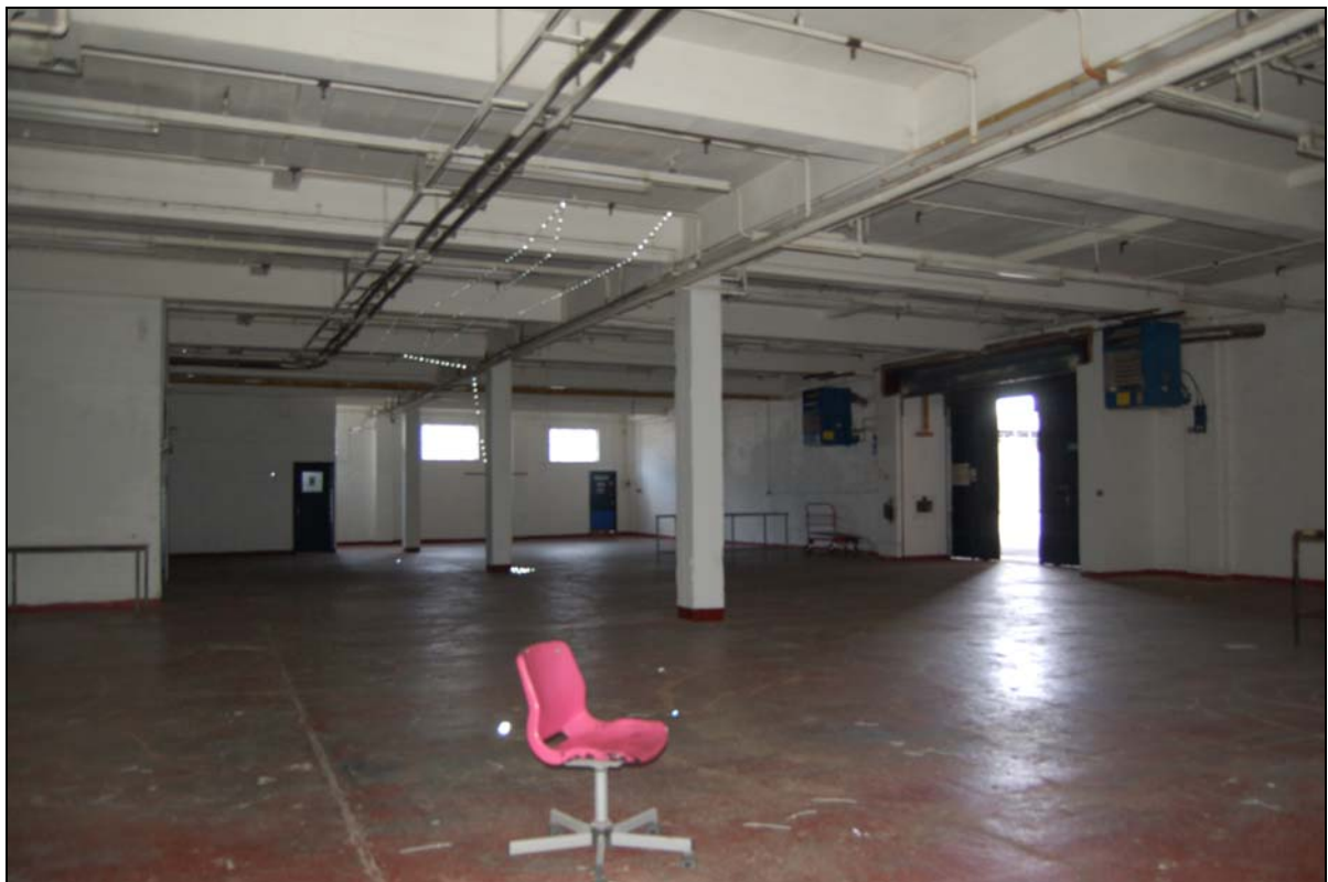
Plate 60. Building C, ground floor, unit 3 (FCQ14-0200)
