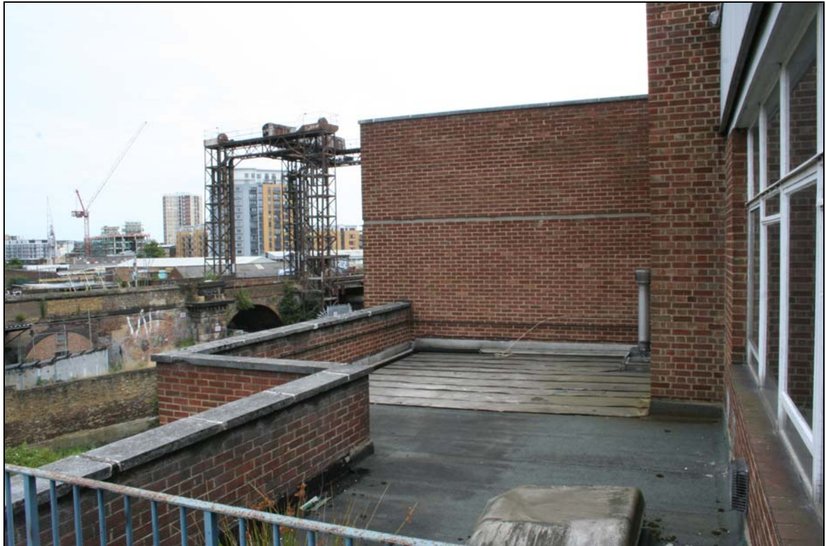
Plate 27. Building B, second floor, unit B204a (FCQ14-0140)
