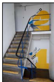
FCQ14-0119 Building B, first floor, stairs
