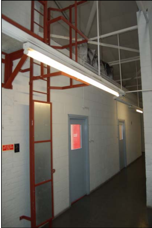
Plate 63. Building C, first floor, corridor, toilets to left (FCQ14-0198)
