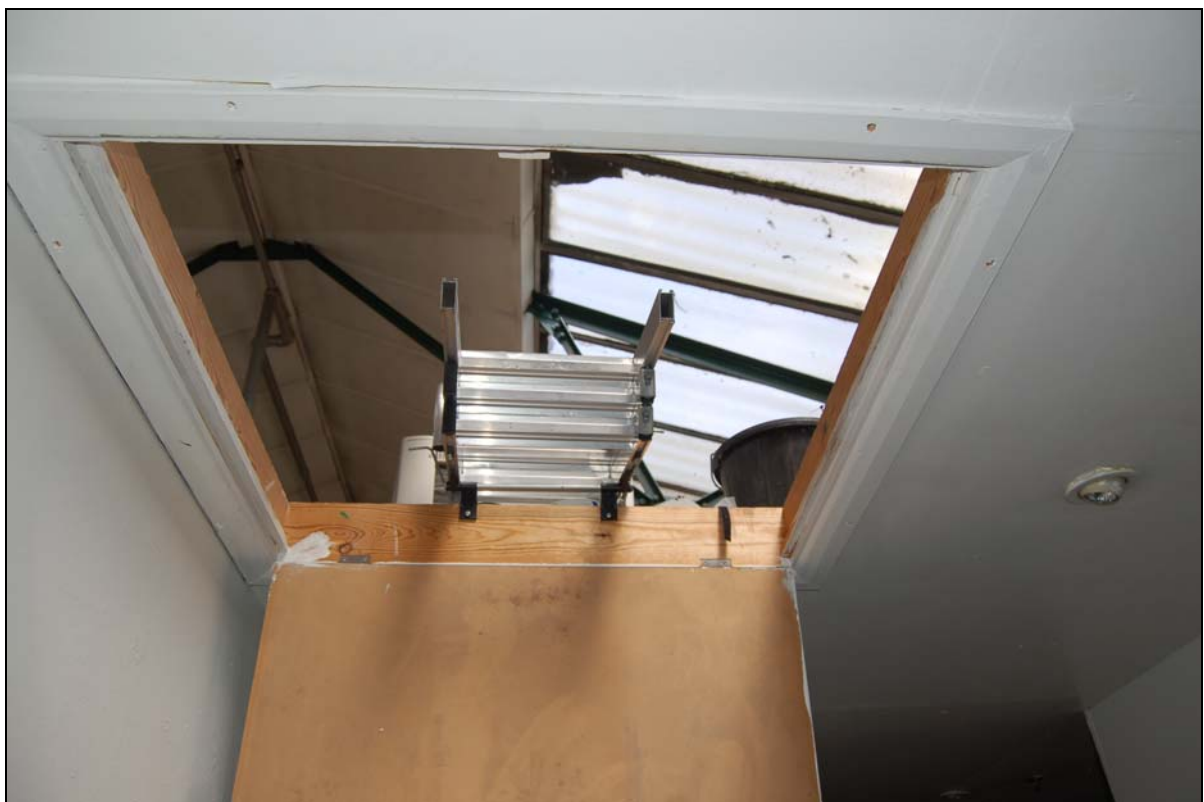
Plate 62. Building C, first floor, skylight over unit C102 (FCQ14-0194)
