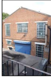
FCQ14-0146 Building C, south elevation
