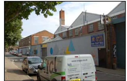
FCQ14-0006 Building A, Creekside elevation
