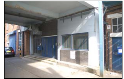
FCQ14-0150 Building C, south elevation
