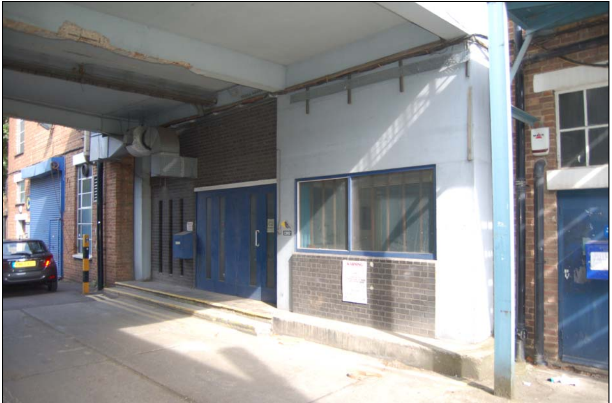
Plate 51. Building C, south elevation (FCQ14-0150)
