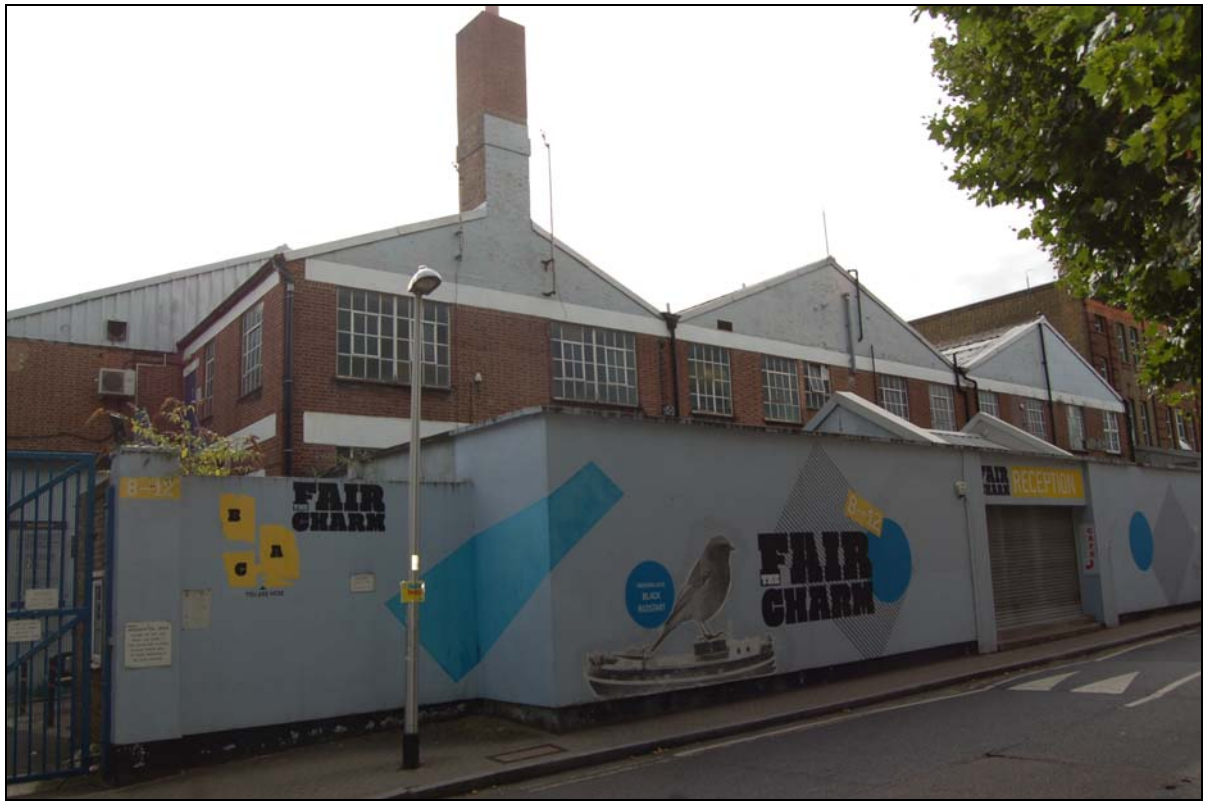
Plate 1. Building A, Creekside elevation (FCQ14-0004)
