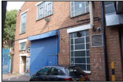
FCQ14-0148 Building C, south elevation
