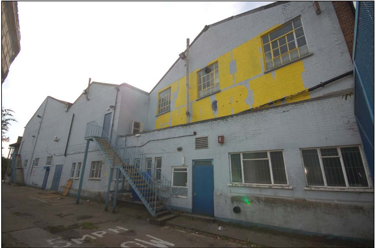
Plate 53. Building C, north elevation (FCQ14-0158)
