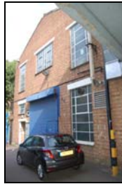
FCQ14-0149 Building C, south elevation
