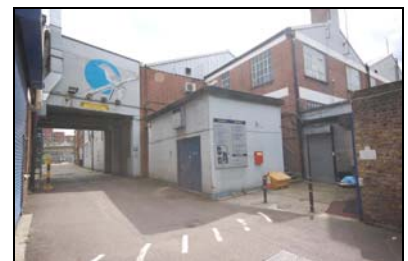
FCQ14-0012 Building A, oblique view of north and west facing elevations
