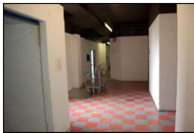
FCQ14-0116 Building B, first floor, eastern lift area
