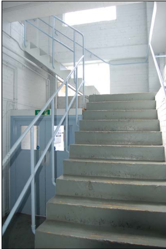
Plate 55. Building C, ground floor, stairs (FCQ14-0176)
