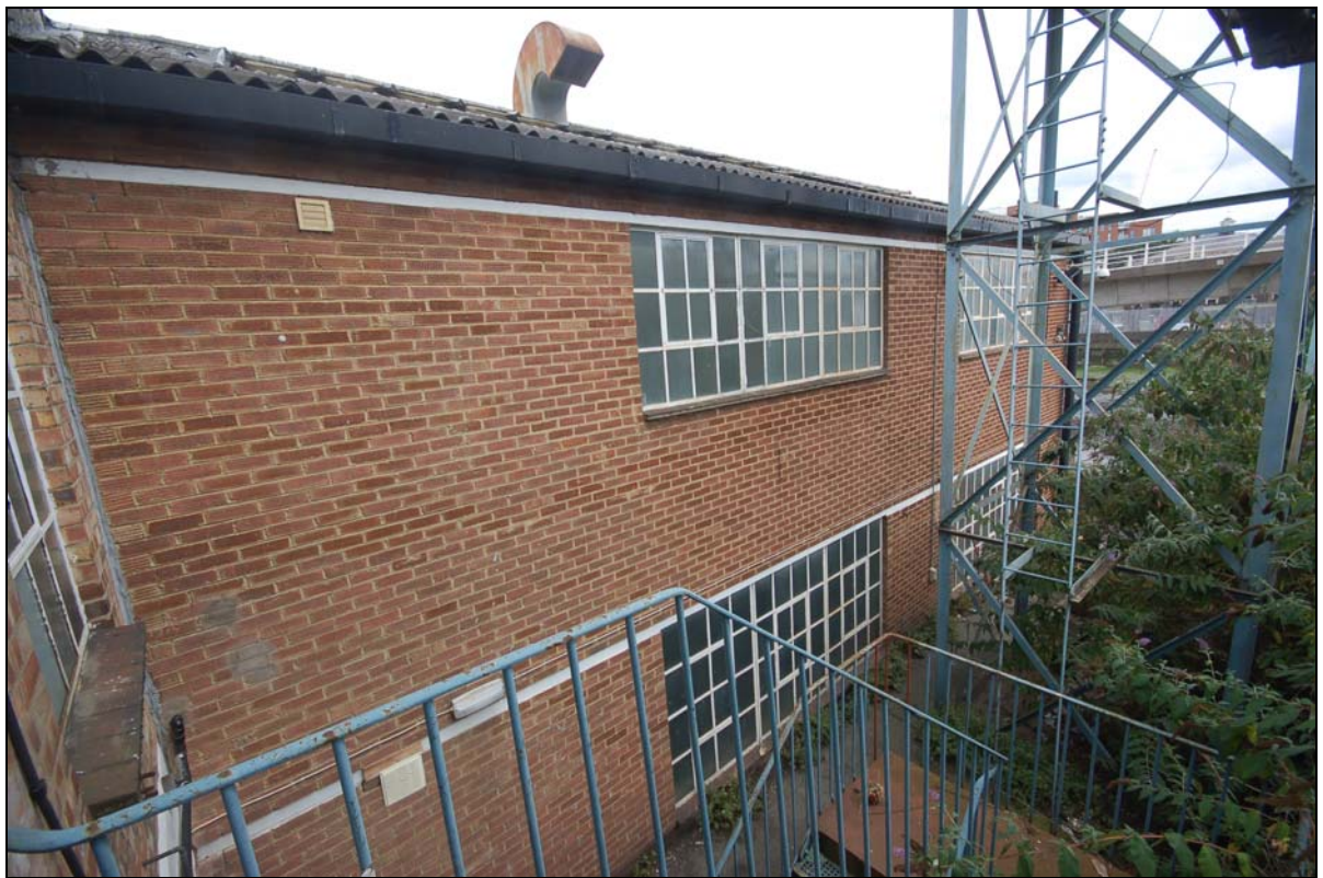
Plate 8. Building A, south facing elevation (FCQ14-0017)
