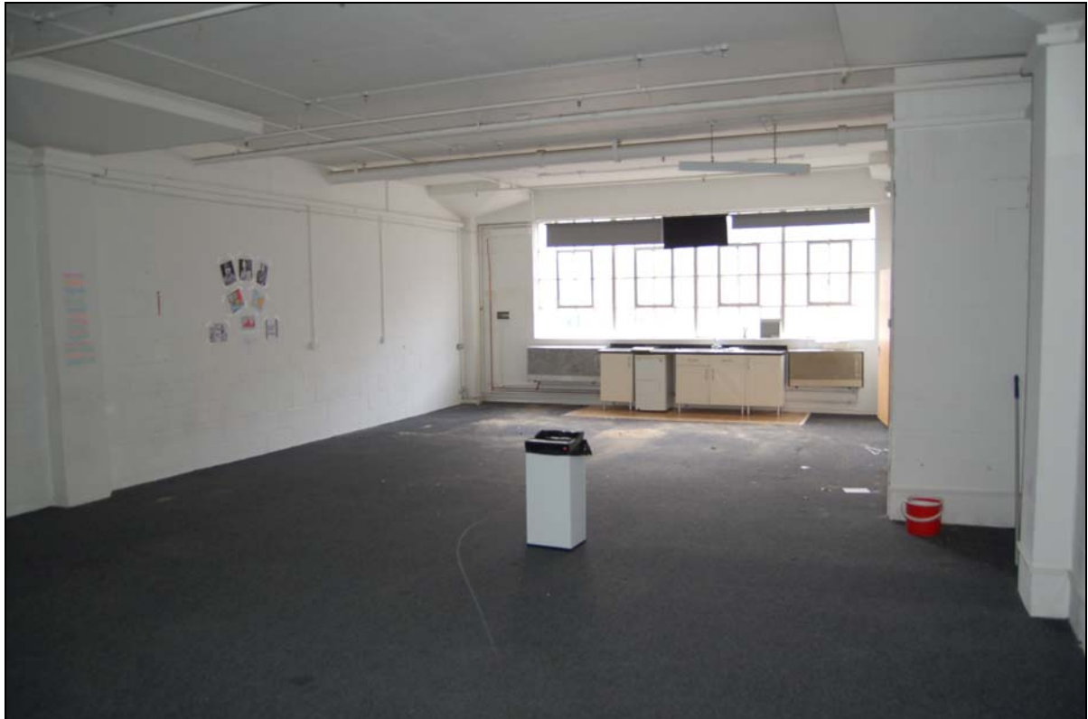
Plate 39. Building B, first floor, unit B114 (FCQ14-0108)
