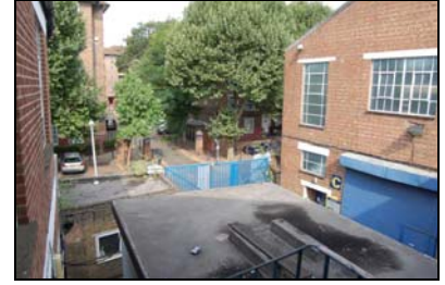
FCQ14-0147 Building C, south elevation
