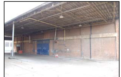
FCQ14-0153 Building C, east elevation
