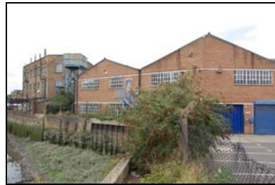
FCQ14-0008 Building A, southeast facing (rear) elevation along Deptford Creek
