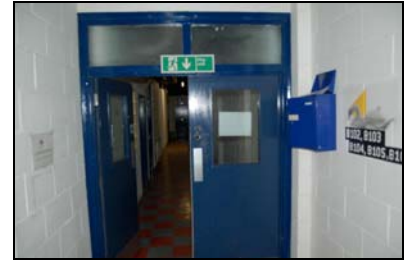
FCQ14-0111 Building B, first floor, double doors in corridor
