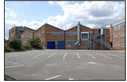
FCQ14-0003 Building A, east facing (rear) elevation
