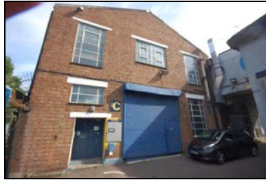
FCQ14-0161 Building C, south elevation
