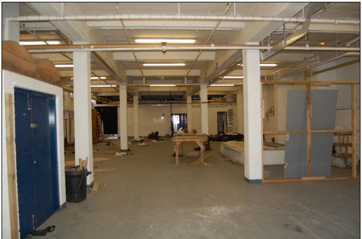
Plate 56. Building C, ground floor, unit 1 (FCQ14-0172)
