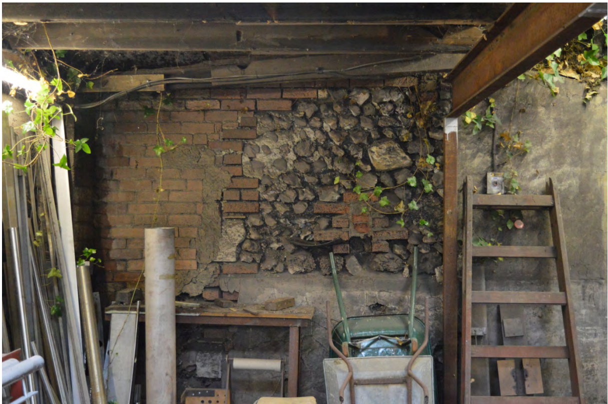
Plate 4: Flint wall on southern side of Building 3 (57)
