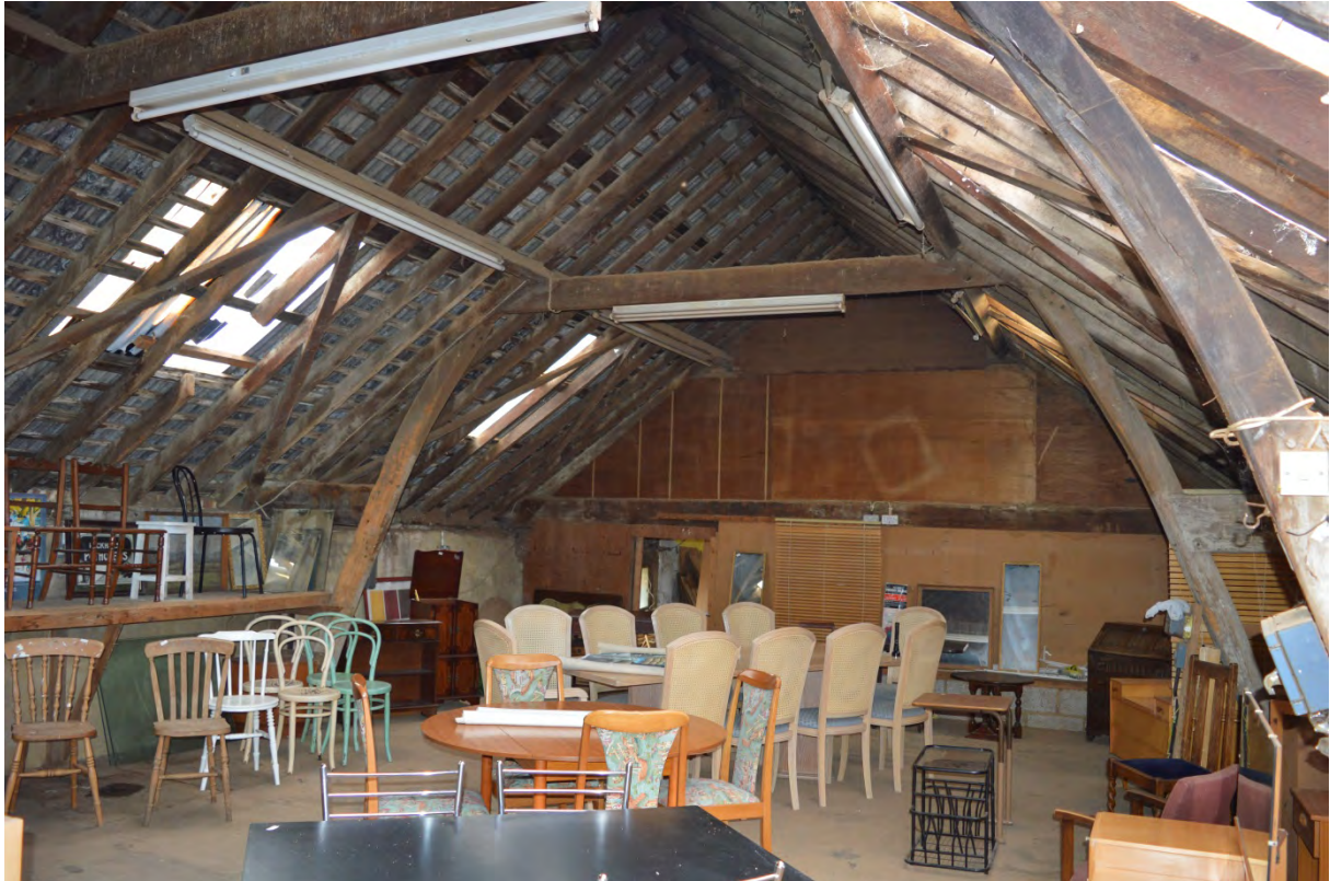
Plate 17: Trusses with interrupted tie beams and sling braces, in Building 13 (20)
