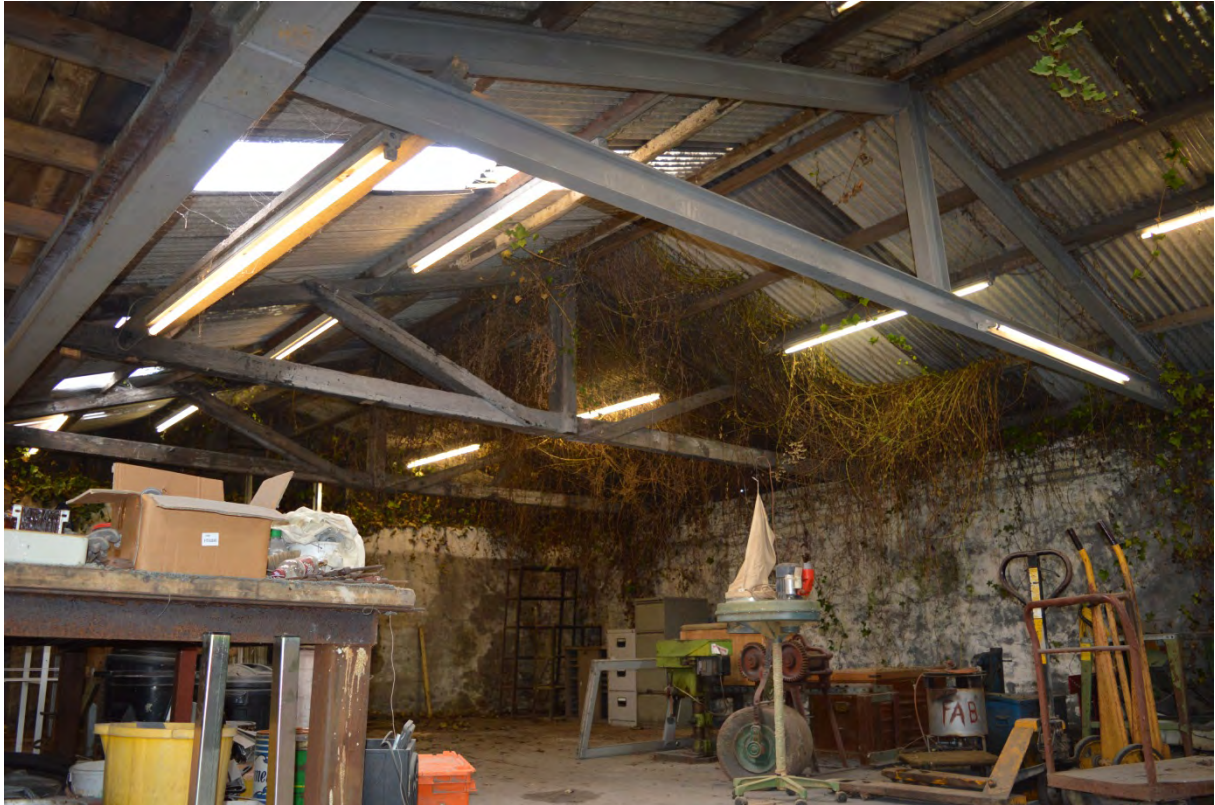
Plate 3: Interior of Building 3 (54)
