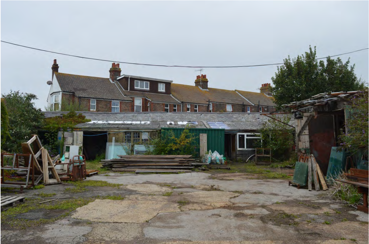
Plate 7: Buildings 7-11, looking north (31)
