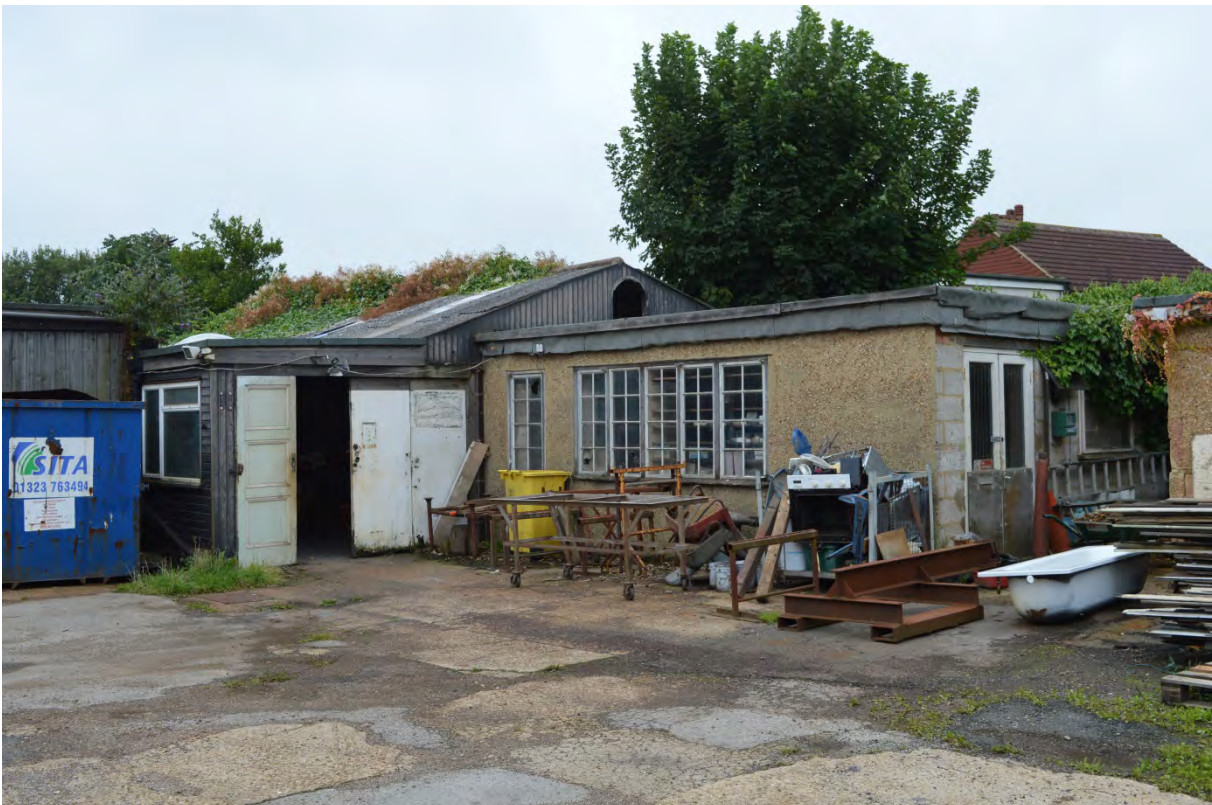
Plate 2: Buildings 3 & 4, looking south-west (51)
