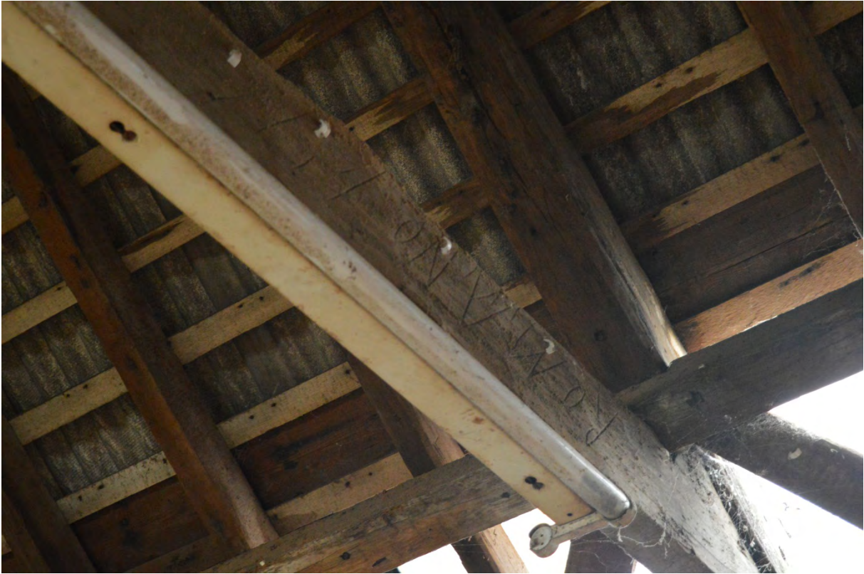
Plate 19: Collar in Building 12 with Baltic merchant's mark (22)
