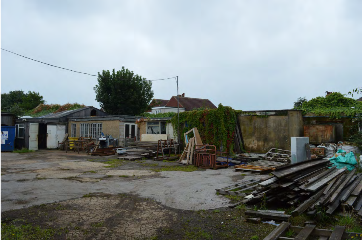
Plate 5: Buildings 3-6, looking south-west (49)
