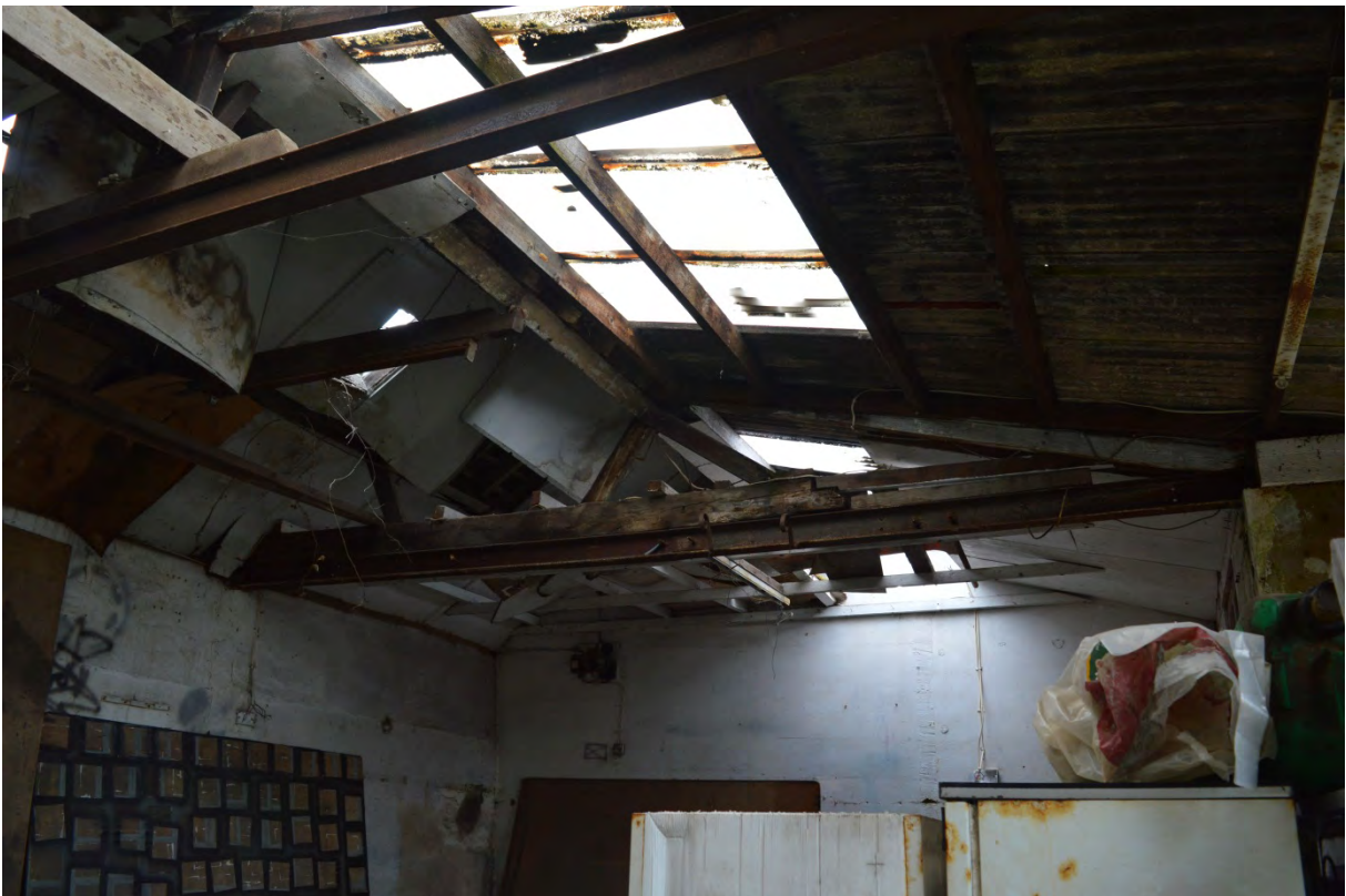
Plate 10: Roof structure of Buildings 7-11, viewed from Building 8 (42)
