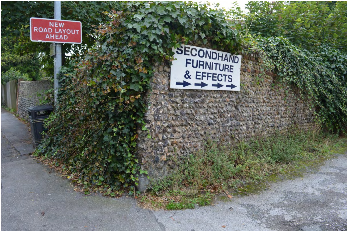
Plate 21: The eastern end of the southern boundary wall (63)
