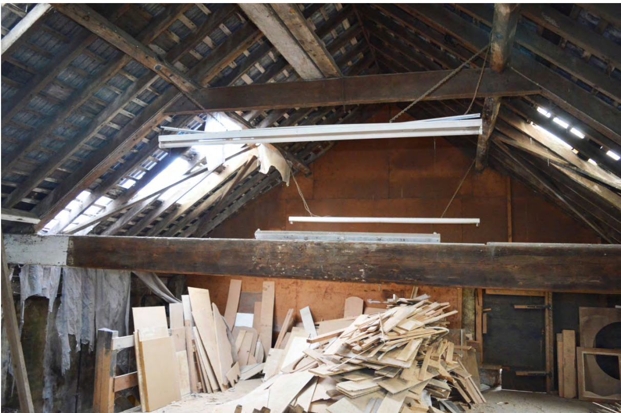
Plate 14: Roof structure over Building 12 (13)
