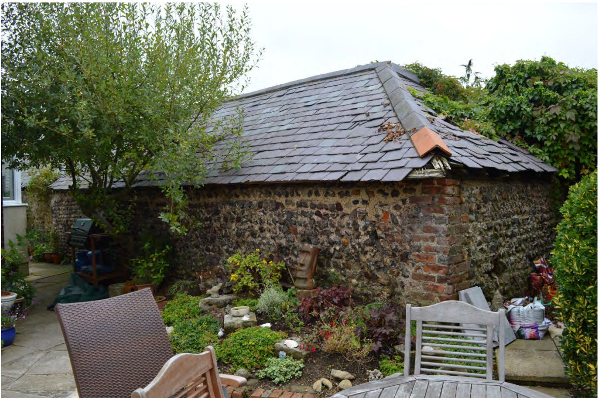
Plate 8: Buildings 7-8, from the north-west (46)
