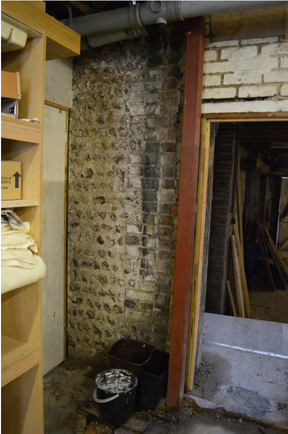
Plate 13: Visible area of flint wall construction in eastern wall of barn (9)
