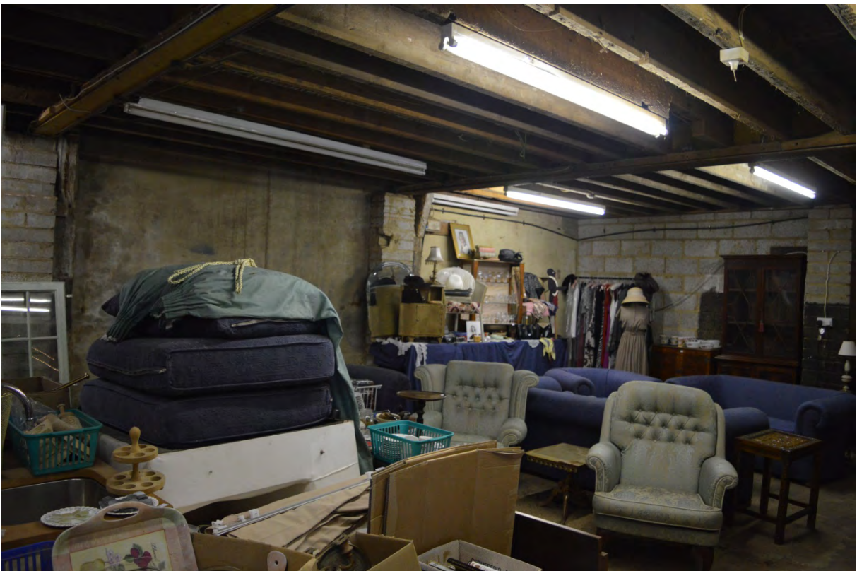
Plate 20: Inserted floor and partition in Building 13. The bottom half of the principal posts of the sling-braced trusses are visible to the centre and left of the photograph (26)
