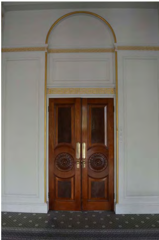
Plate 16: Doors between first floor rooms, 16-17 Park Crescent (7)
