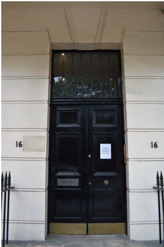
Plate 4: Doorway to 16 Park Crescent (113)
