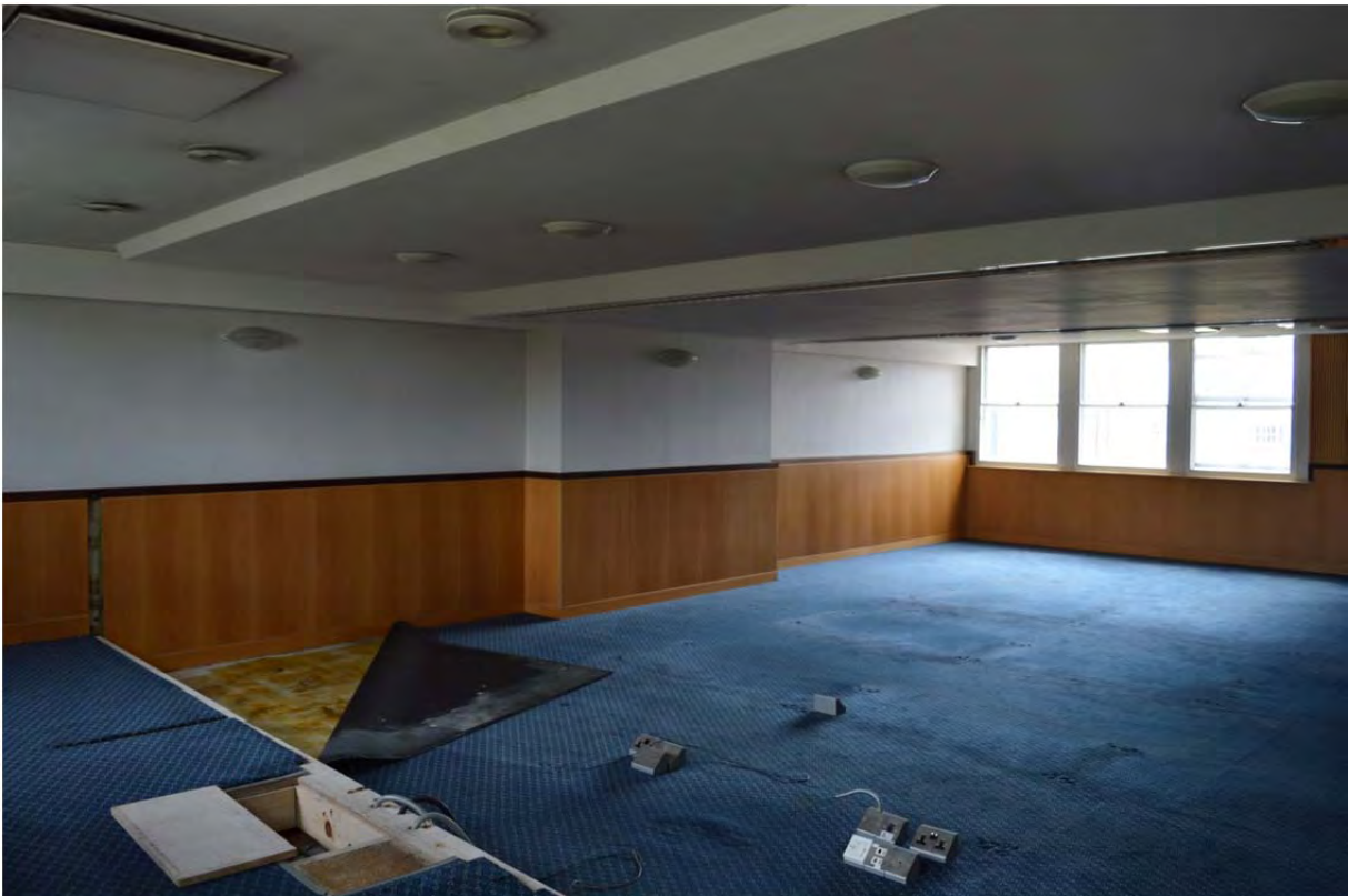
Plate 22: Possible chimney stack remnant at third floor level, 26 Park Crescent (48)
