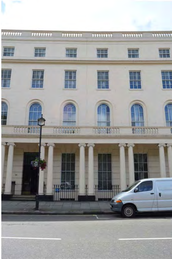
Plate 3: Example of expansion joint visible in stucco finish (14)
