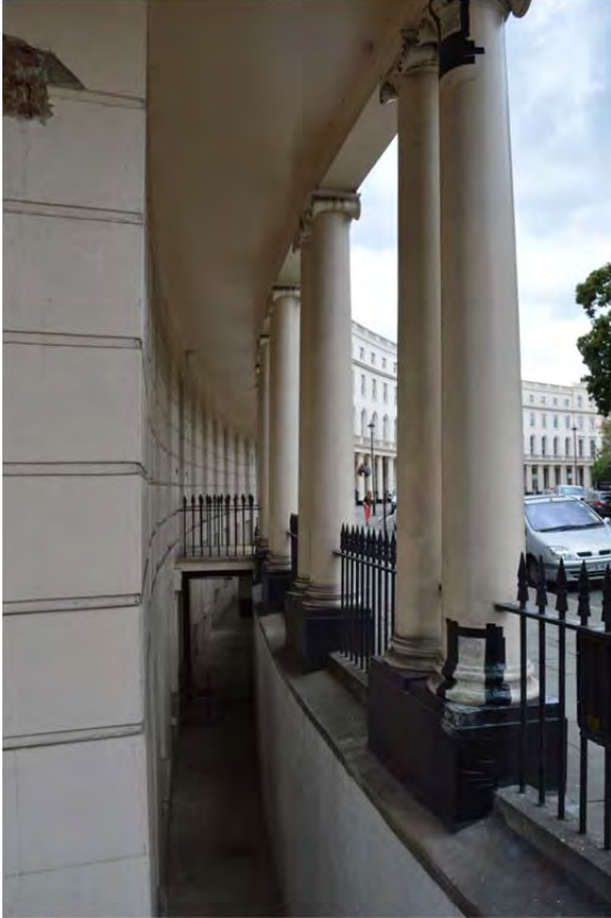
Plate 5: Basement lightwell, showing modern tiling (111)
