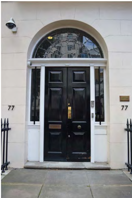
Plate 24: Door to 77 Portland Place (63)
