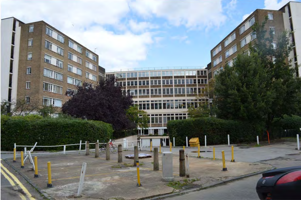
Plate 11: Typical character of rear elevation of 16-26 Park Crescent (54)
