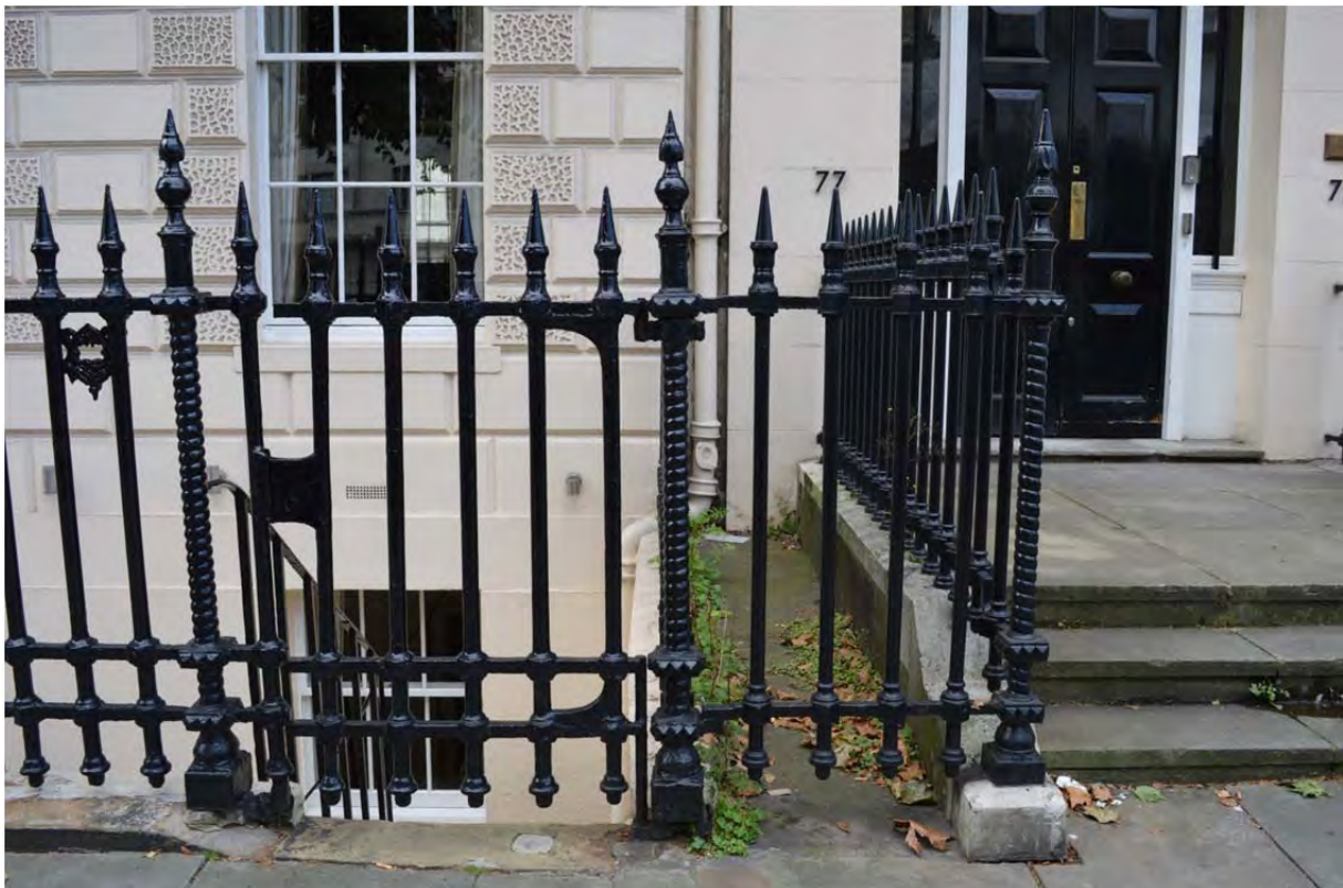
Plate 36: Historic railings (left) at No. 75 and modern railings (right) at No. 77 Portland Place (58)
