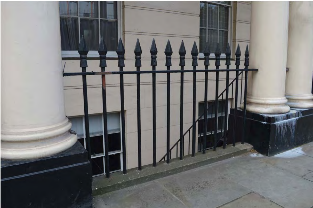
Plate 6: Railings outside 16 Park Crescent (66)
