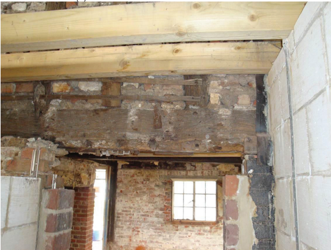
Plate 8: Redundant mortices for window jambs and mullions in south-east side girt (56)
