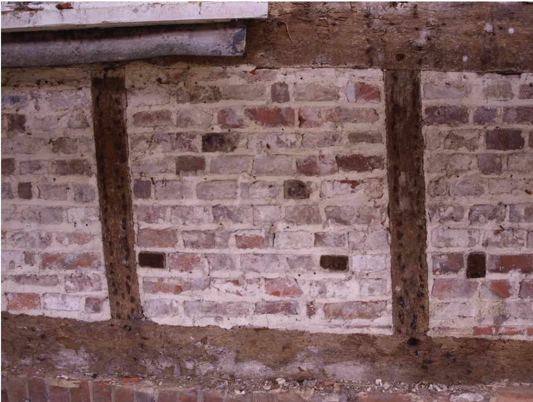
Plate 5: Brick infill to front elevation, showing small timber bearers (51)
