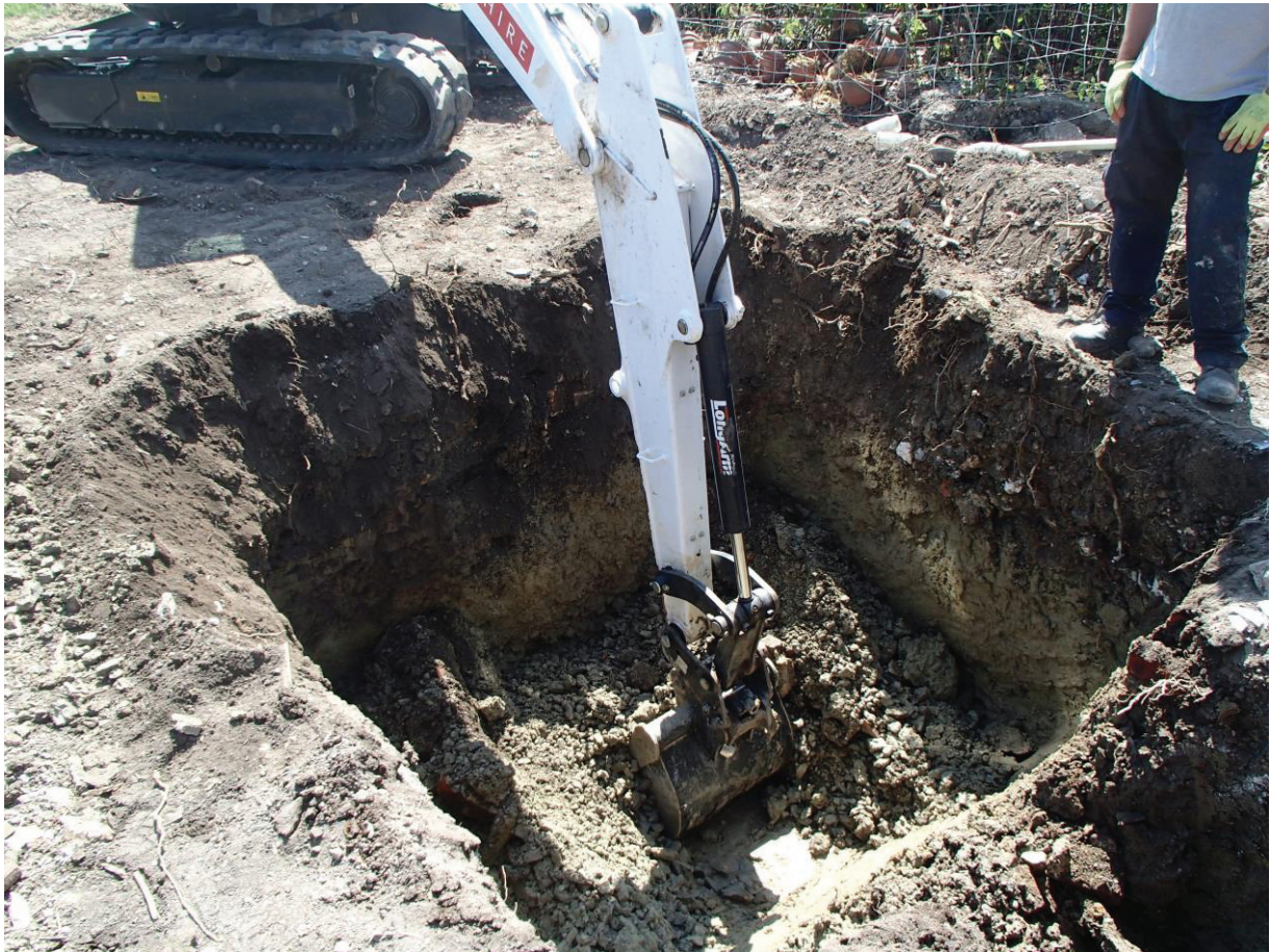
Plate 13: Excavations for the septic tank
