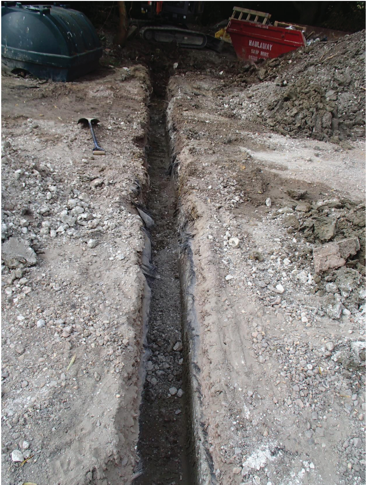
Plate 11: Oil trench looking SW in centre of site
