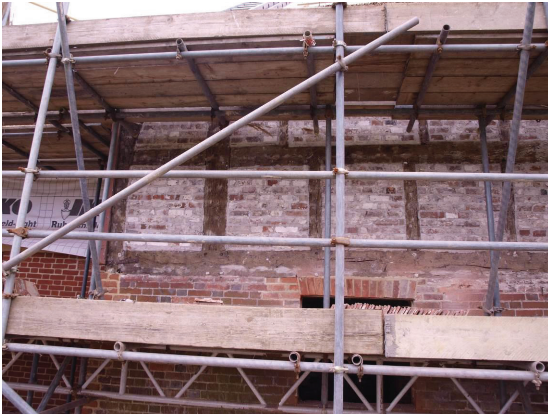
Plate 1: Small panel framing to the north-east elevation, showing substantial stud (44)
