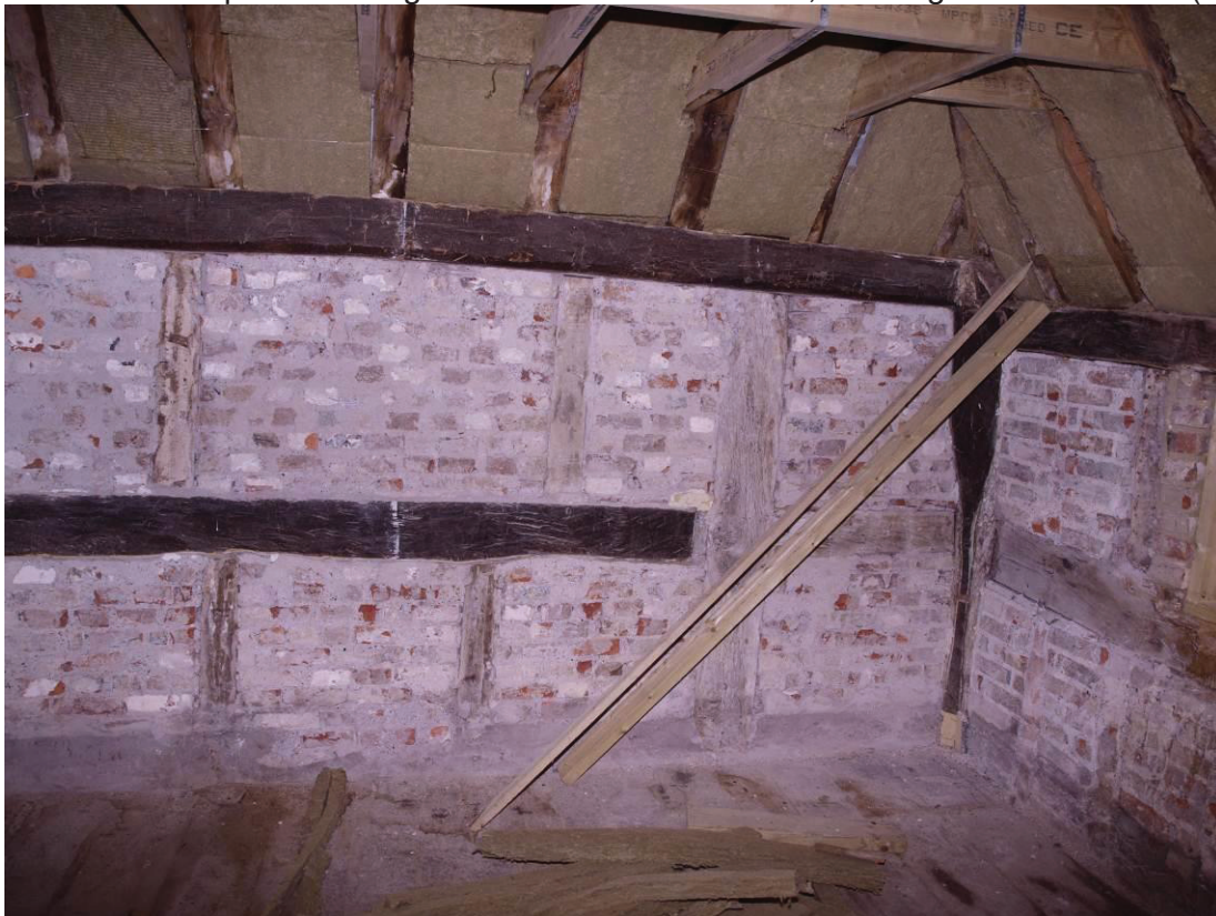
Plate 2: Interior view of first floor of the north-east wall (25)
