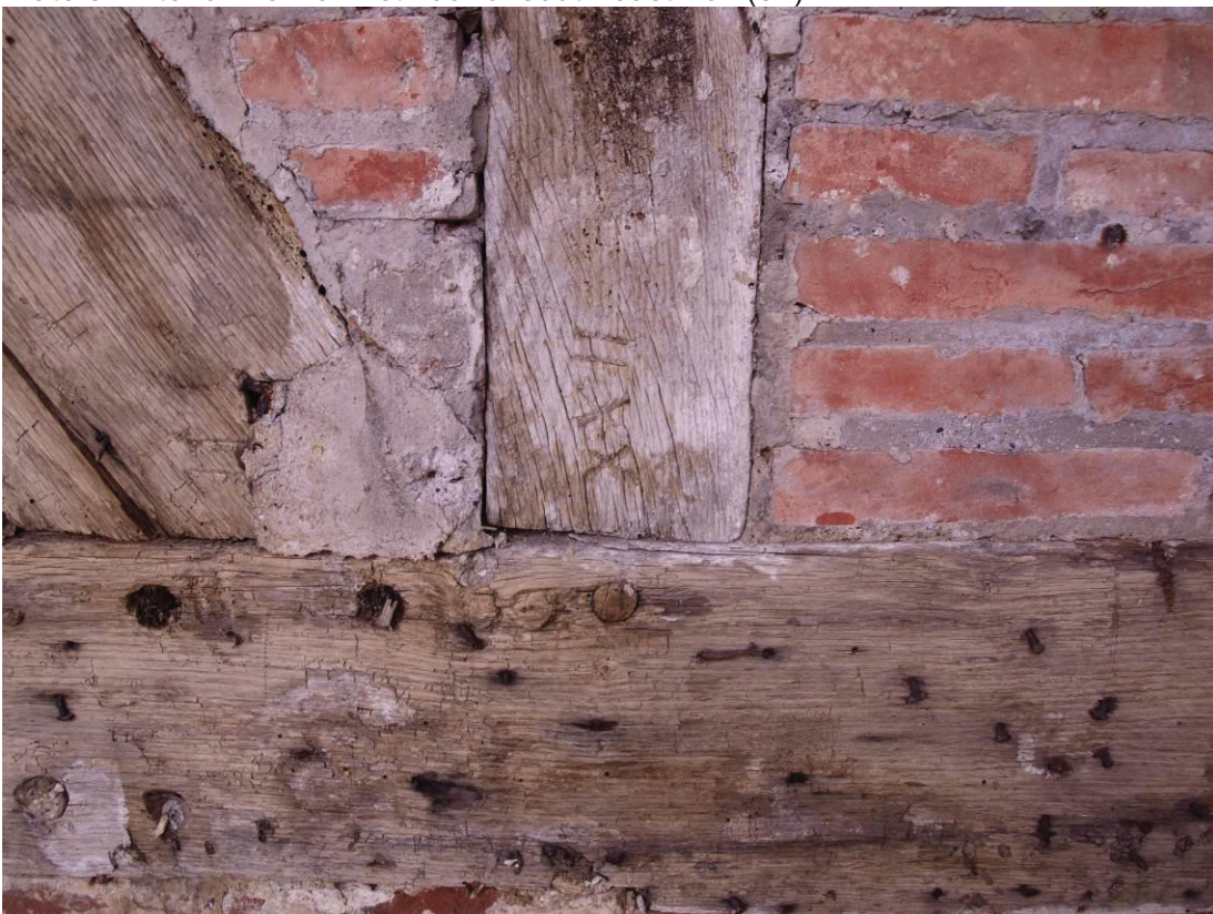
Plate 4: Carpentry mark on south-east elevation (49)
