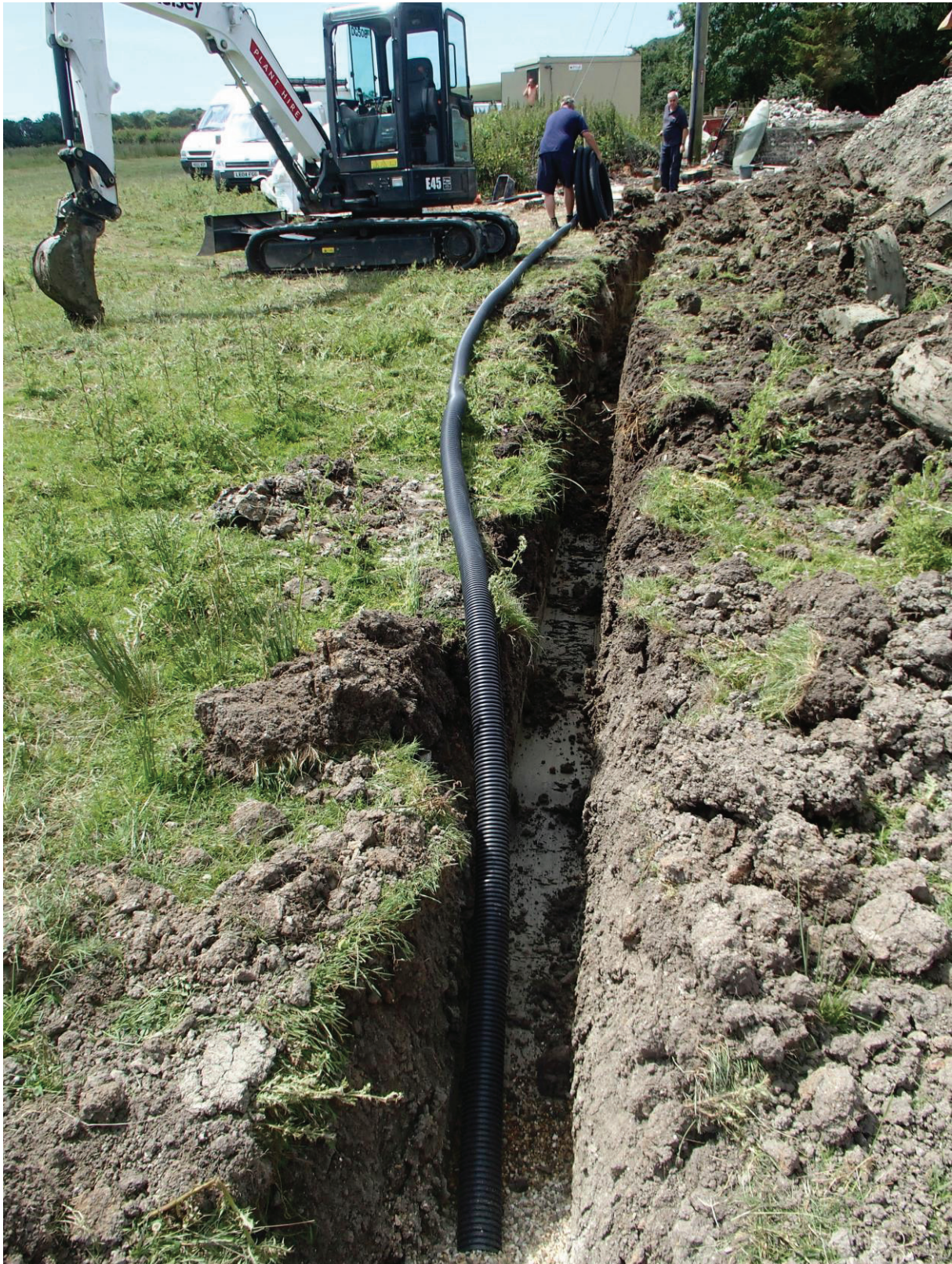
Plate 14: Outflow trench looking west
