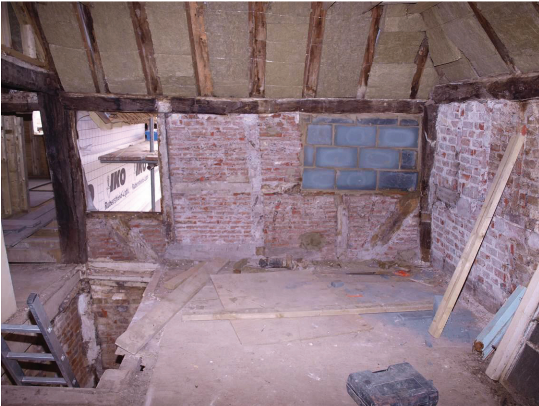
Plate 3: Interior view of first floor of south-east wall (34)
