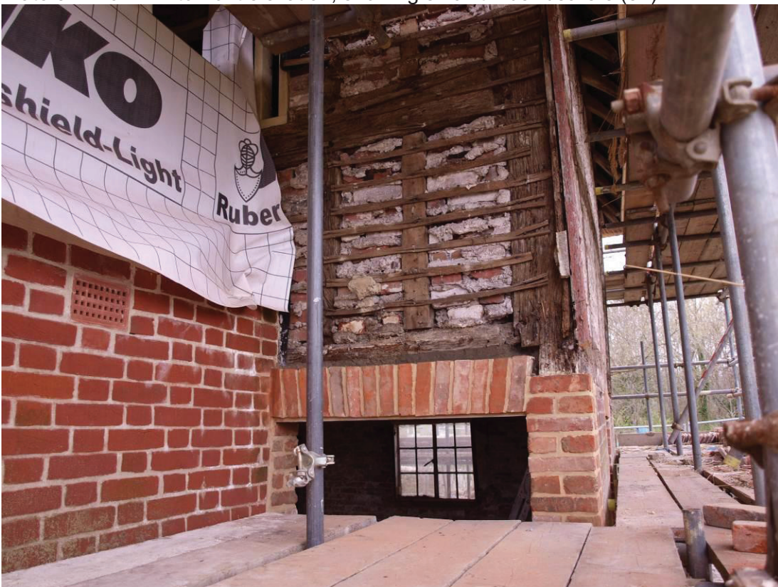
Plate 6: Intermediate stud and laths for tile-hanging (43)
