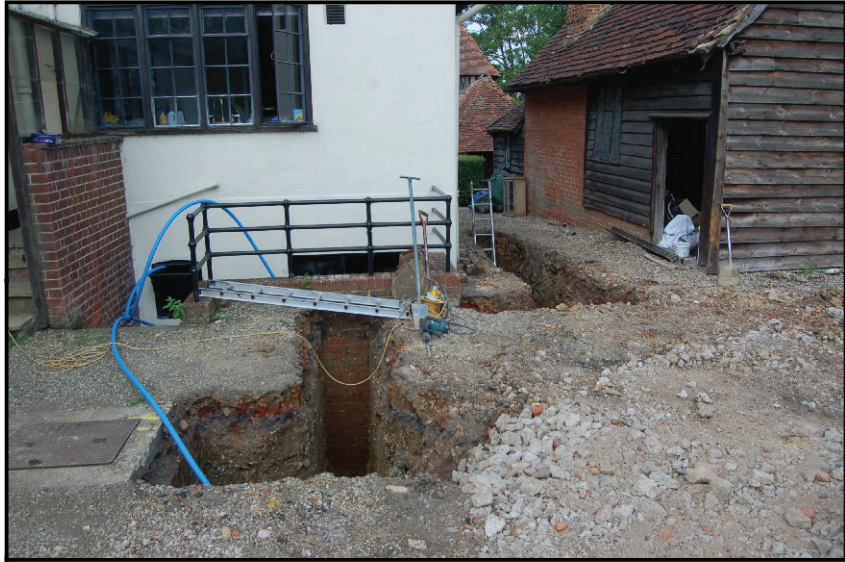
7.1 General view of the kitchen foundation trenches
