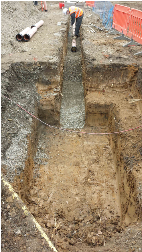
Service trenching adjacent to TP27
