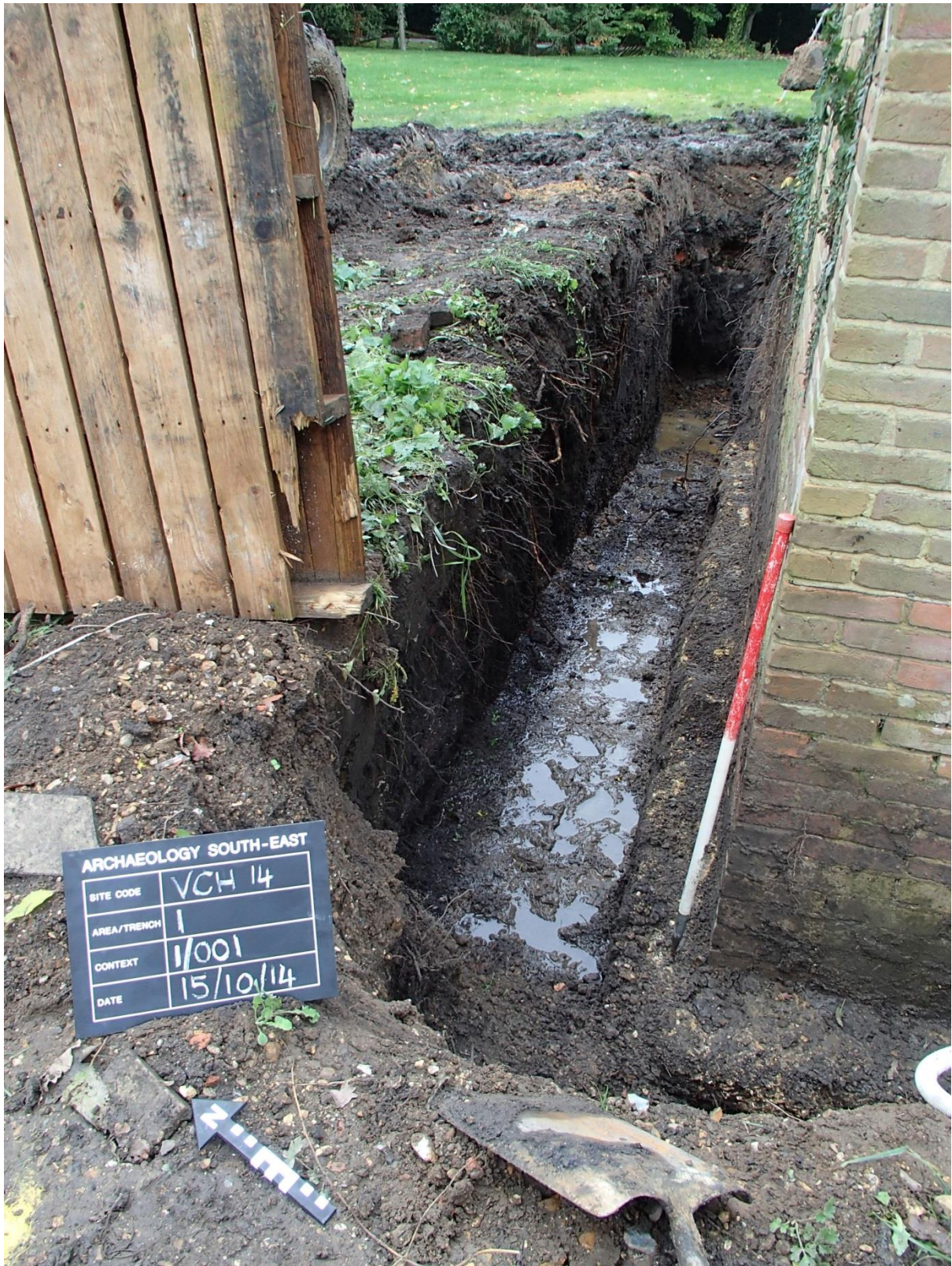
Figure 6: Disturbance from previous foundations, looking east
