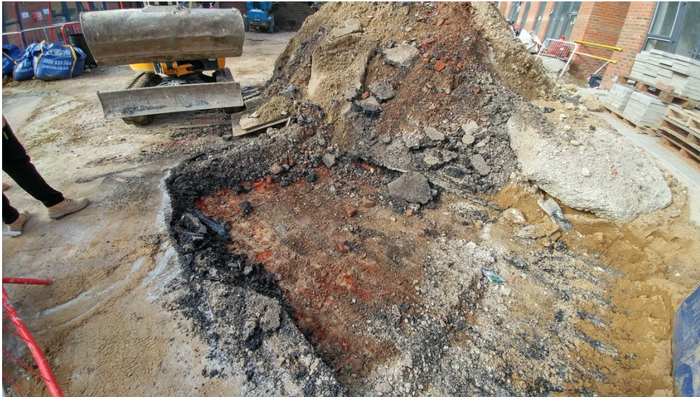
Plate 19: Made-ground underlying tarmac in the area of the predicted air-raid shelter, looking south. The new ground level will be level with the rear of the new-builds seen to the right.
