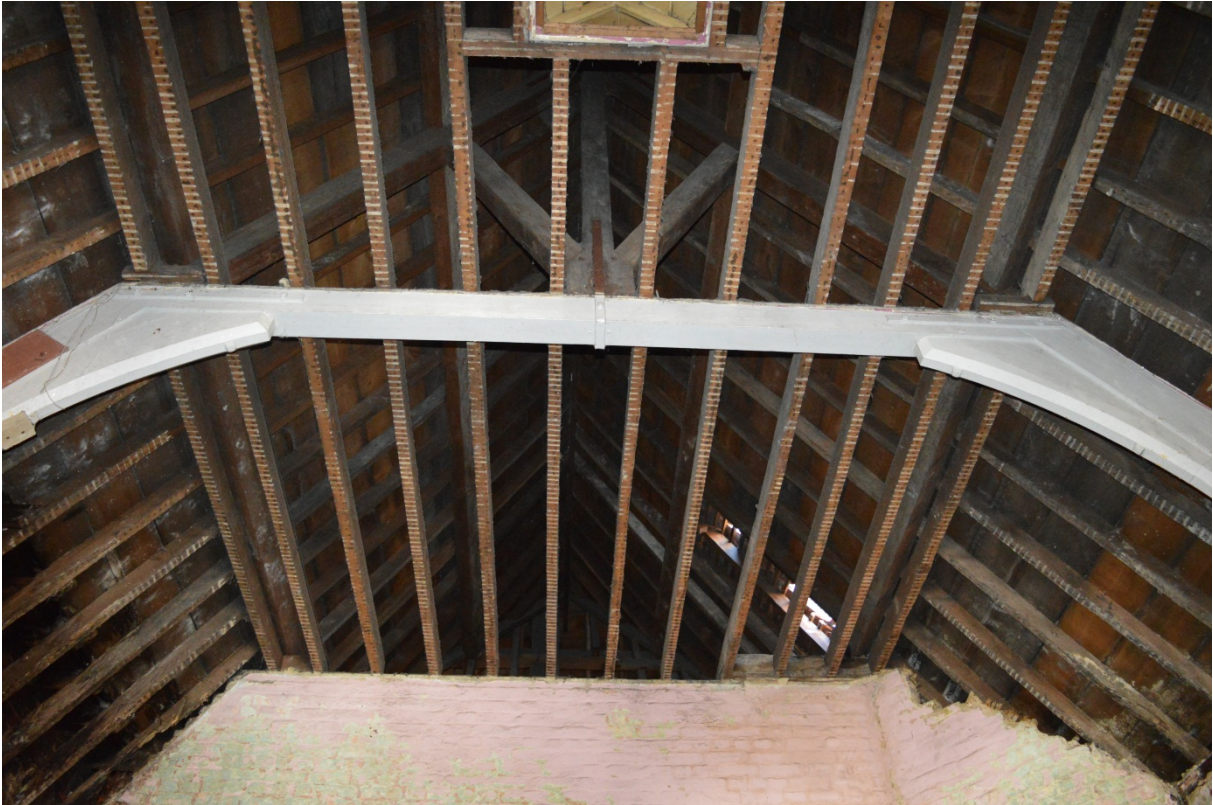
Plate 9: Central roof truss in Room 4 (63)
