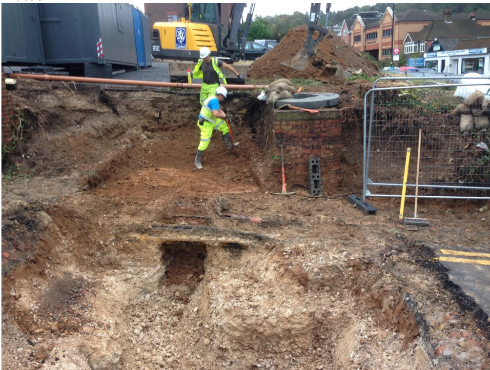
Plate 1: Monitoring the edge of the road service trench, looking south.
