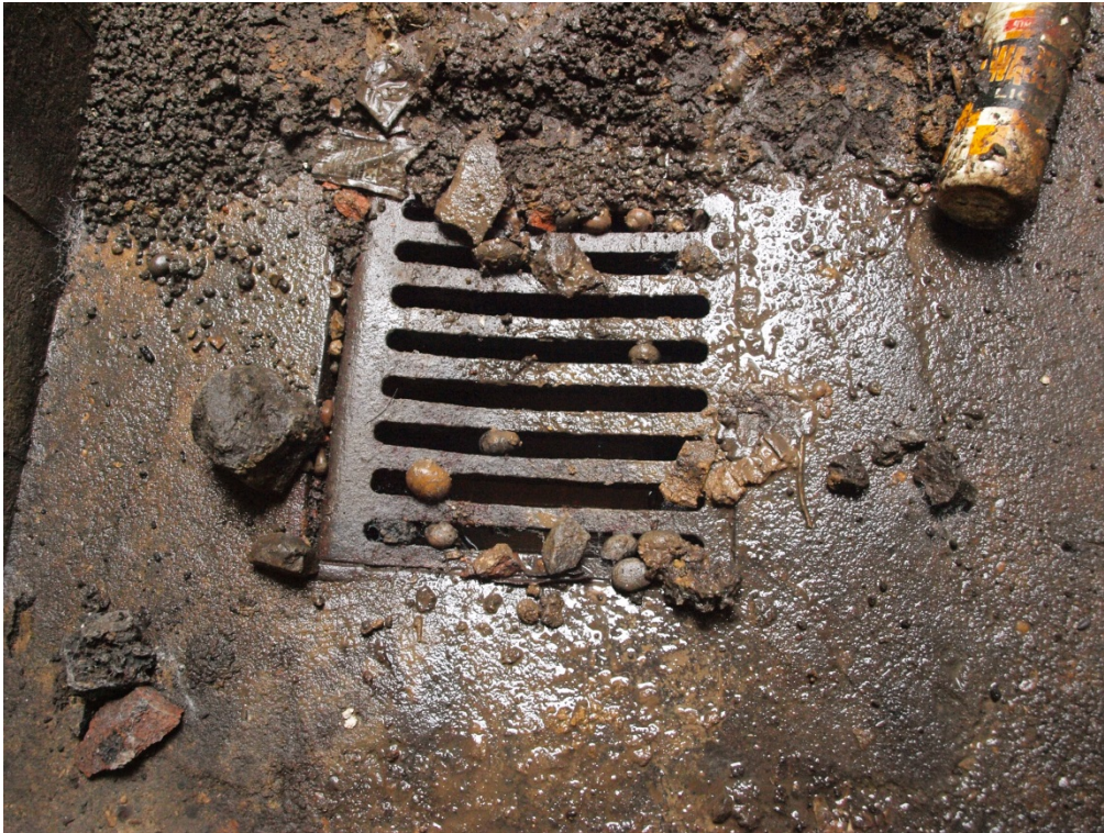
Plate 9: Drain in hallway, looking west.
