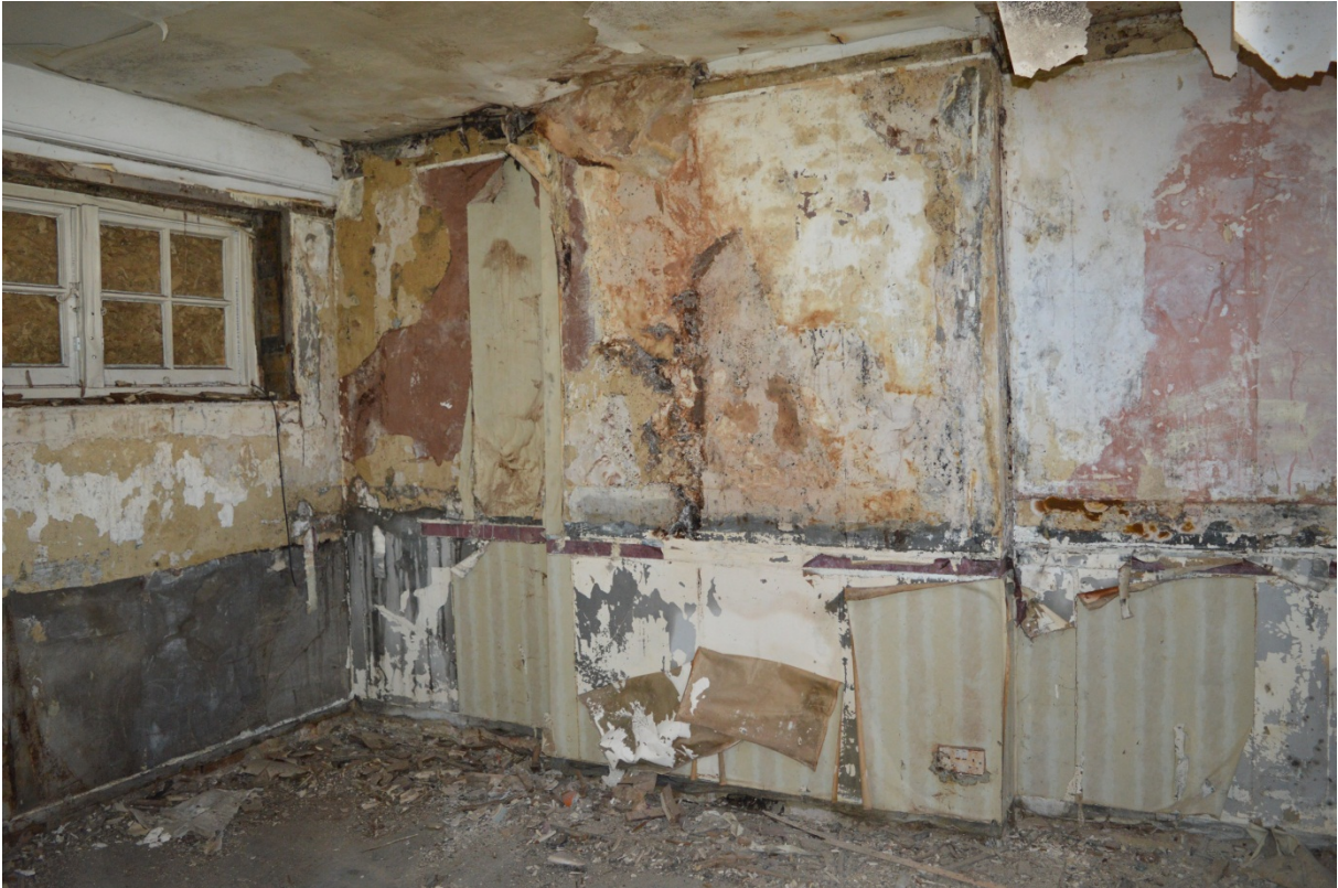
Plate 19: Room 11, looking south-west (114)
