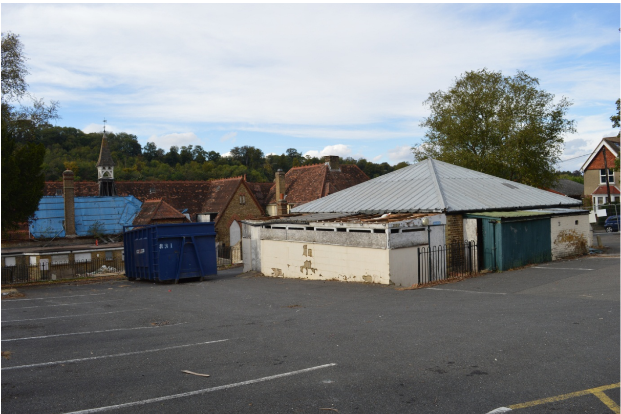
Plate 22: Building B, looking north-west (125)
