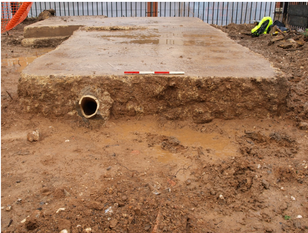
Plate 16: Ventilation pipe opening, east end of the shelter, looking west.
