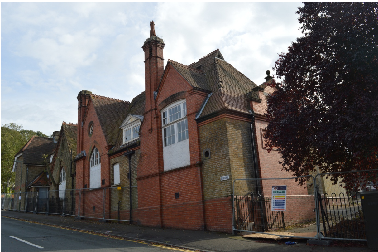
Plate 4: North elevation of north-east range, looking south-east (135)
