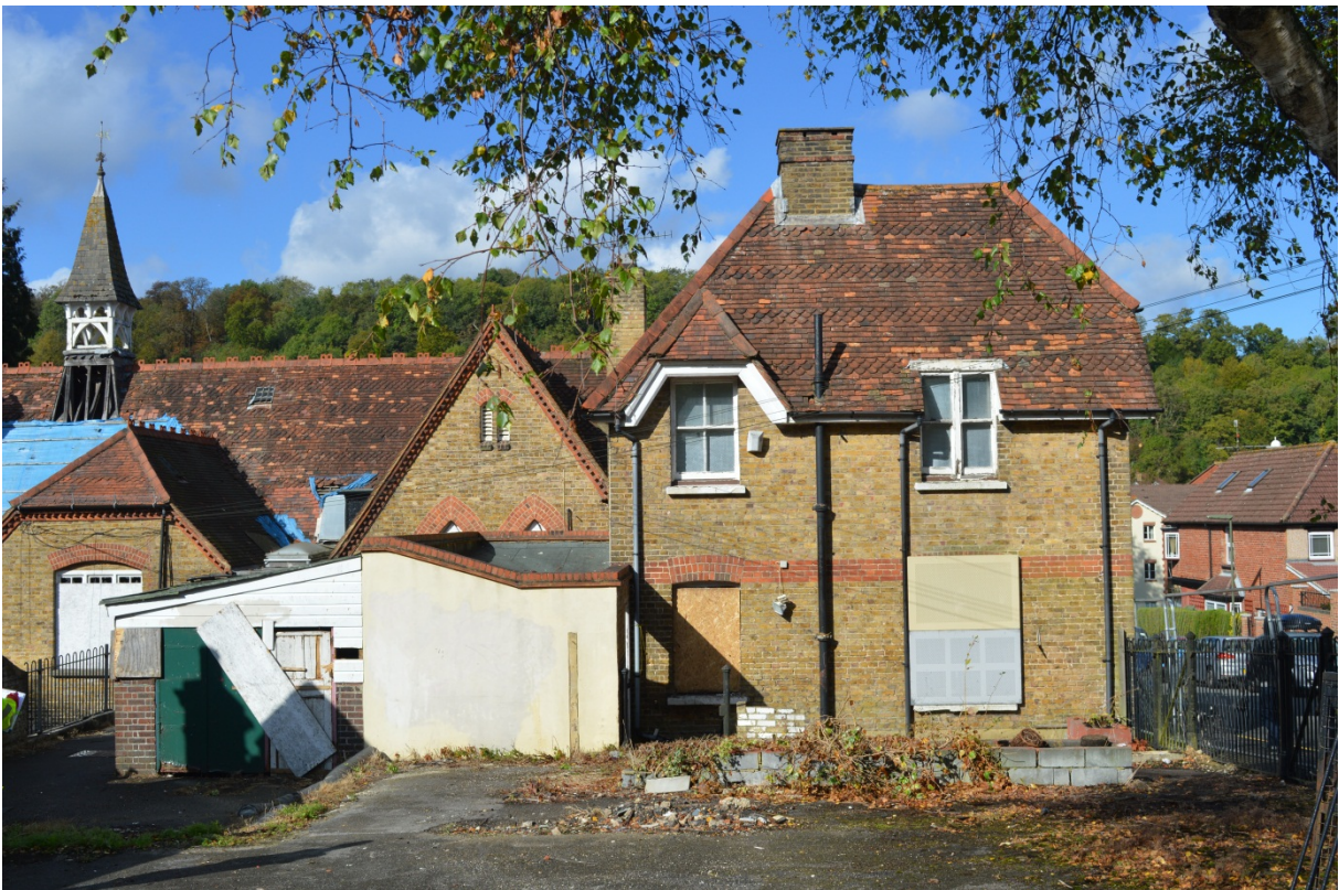
Plate 16: East elevation of teacher's house (16)
