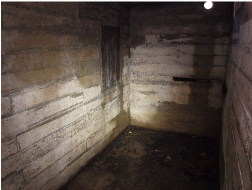
Plate 6: Interior of the shelter, looking East.
