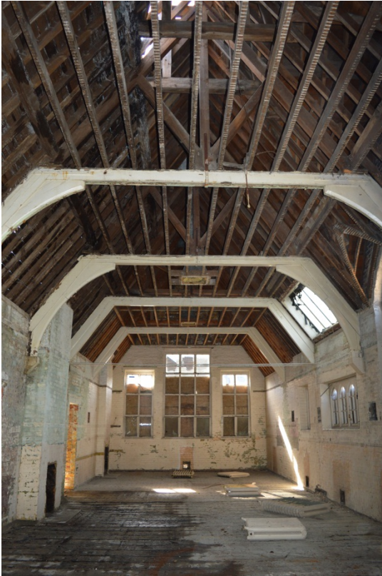
Plate 13: Room 8, looking south (85)
