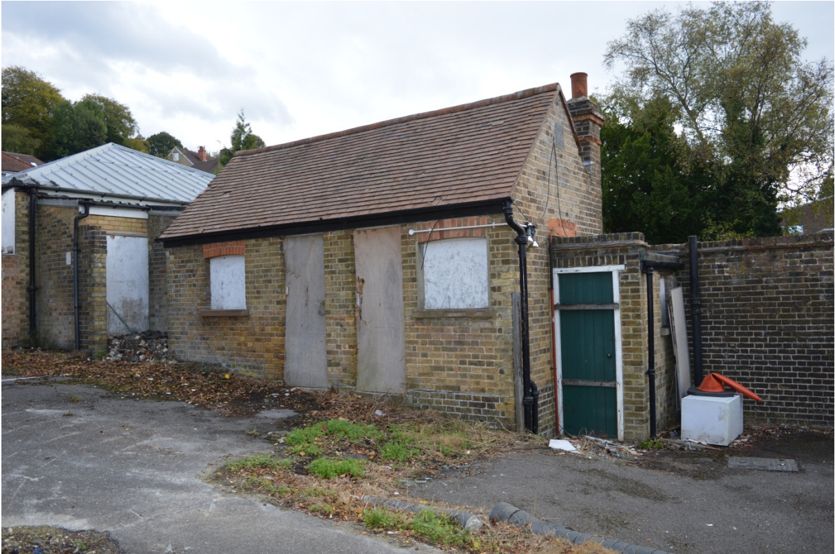
Plate 21: Building A, looking south-east (122)
