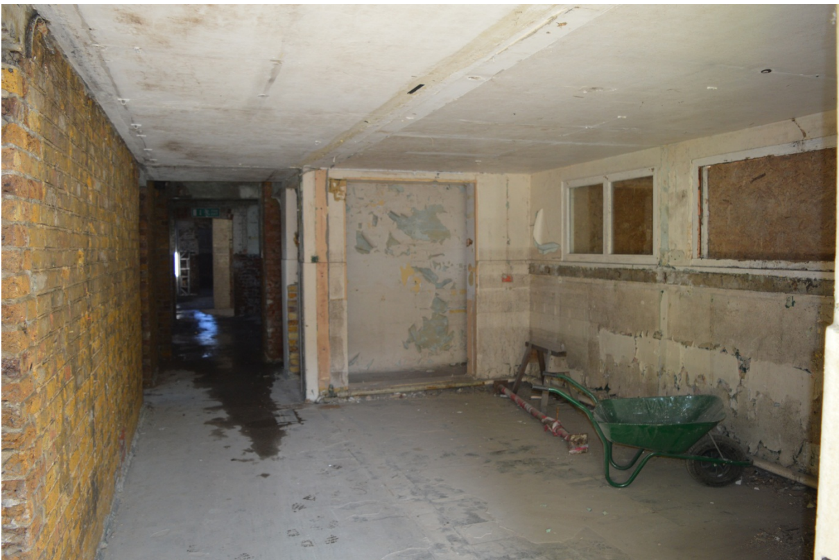
Plate 14: Room 9, looking north (97)
