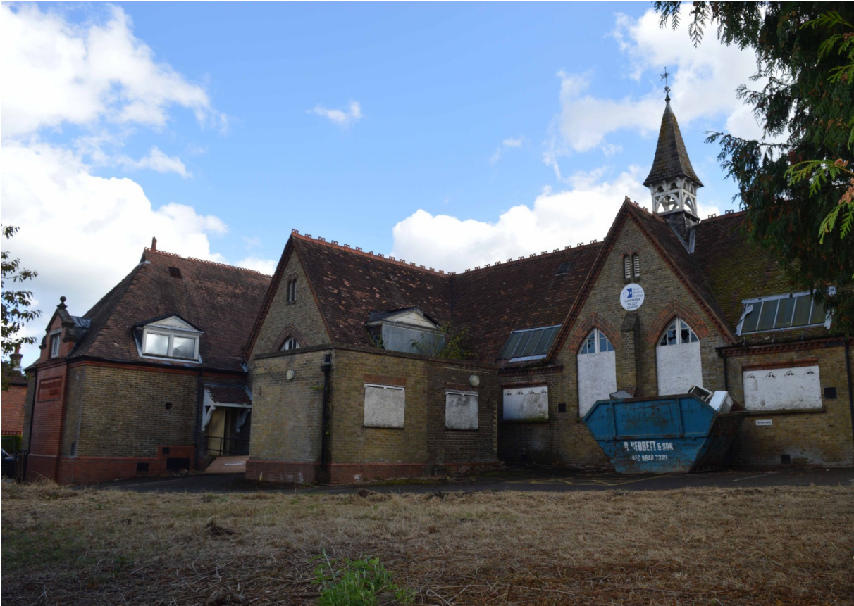
Plate 1: West elevation, looking north-west (42)
