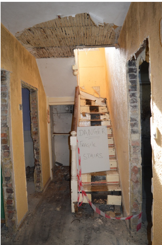
Plate 18: Entrance/stair hall in teacher's house (116)
