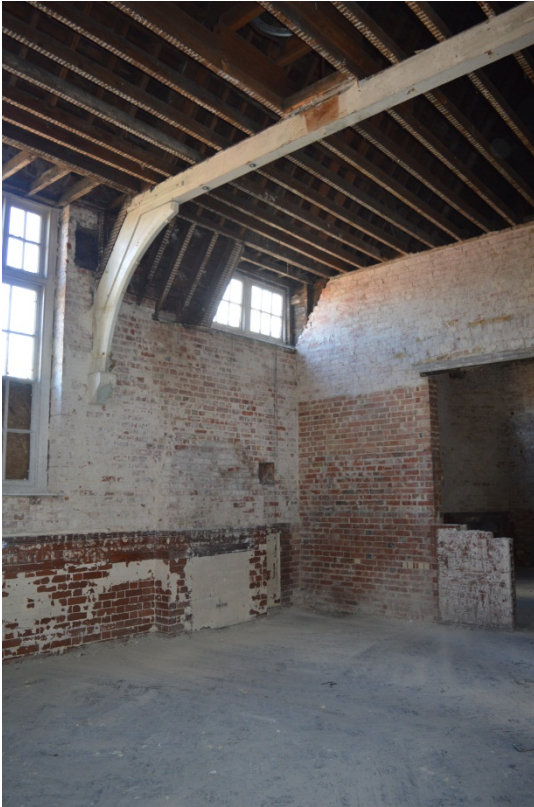
Plate 7: Room 1, looking north-east (44)
