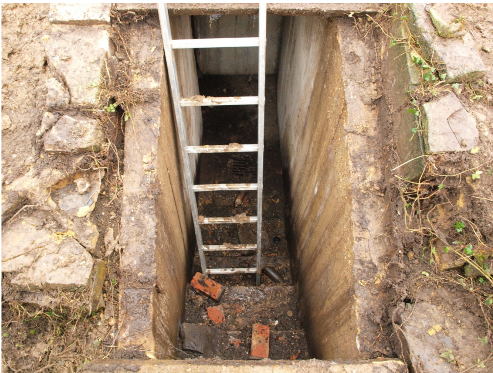
Plate 8: Steps down to the shelter, looking East.
