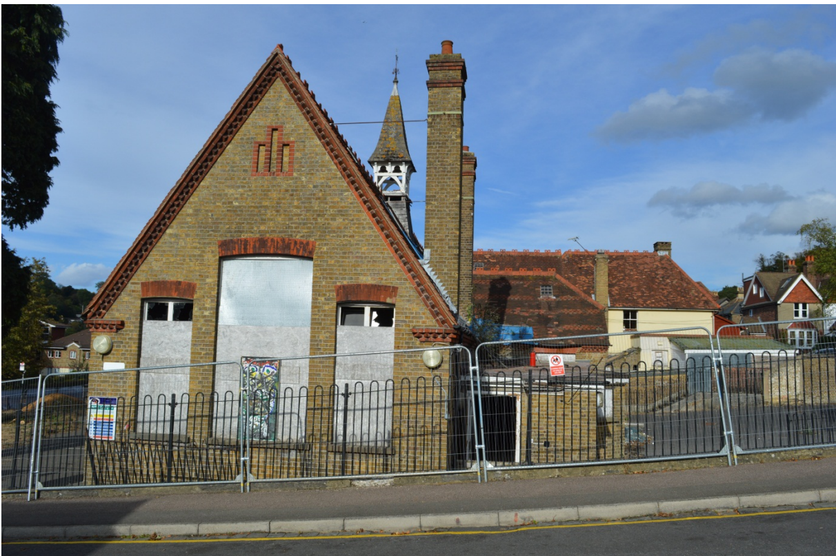
Plate 2: South elevation of south range (130)
