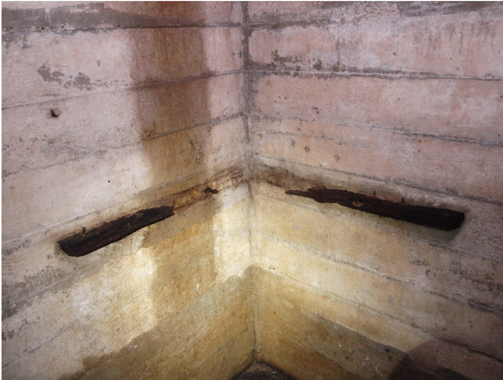
Plate 15: Remains of possible shelf in the south-east corner of the shelter.
