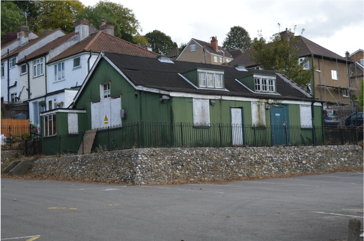
Plate 23: Building C, looking south-east (124)
