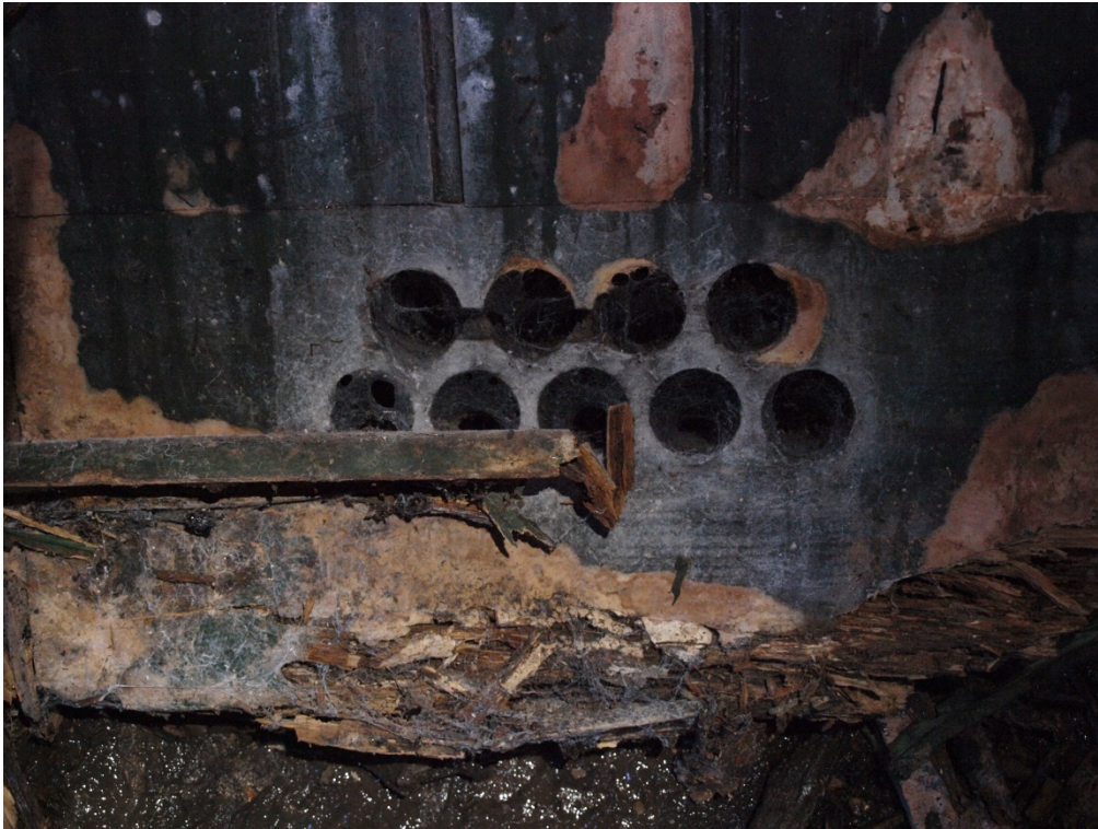
Plate 11: Closable vent on the door in the event of gas attacks.
