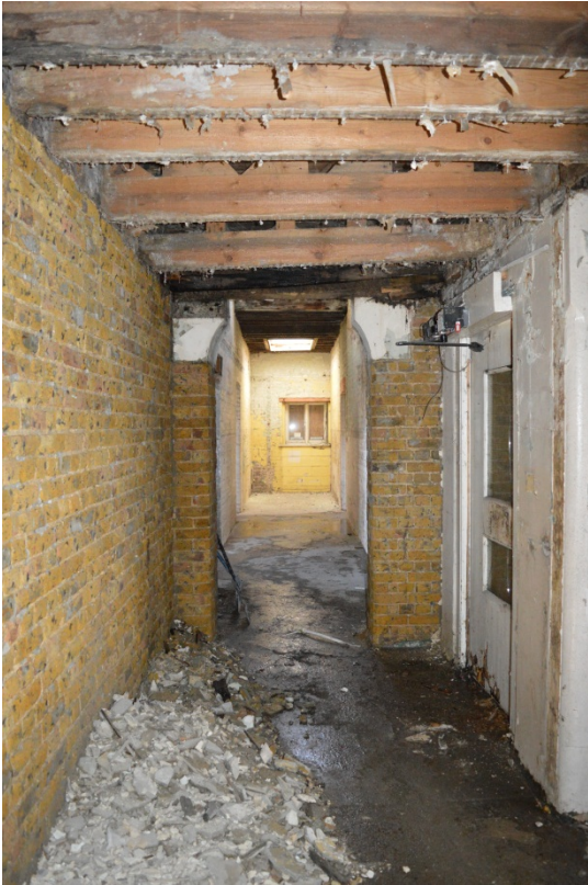
Plate 11: Probable original doorway to south range, now enclosed within Room 10 (106)
