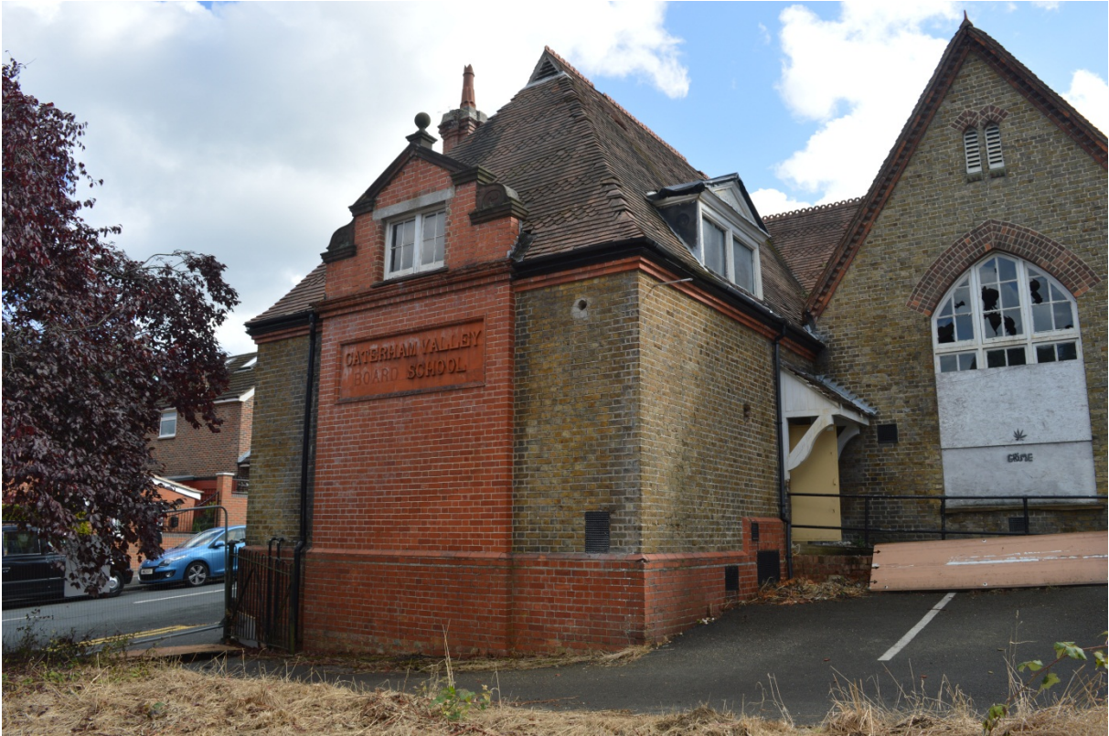
Plate 5: West elevation of the north-west range, looking north-east (35)
