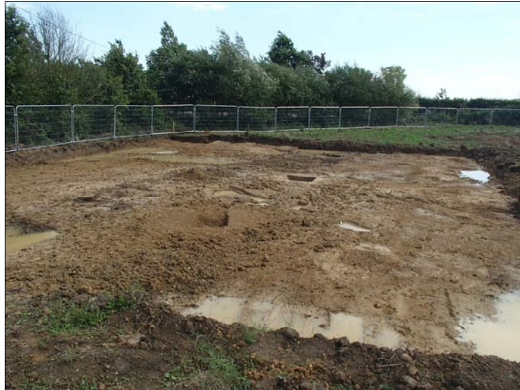
General view of excavation looking south
