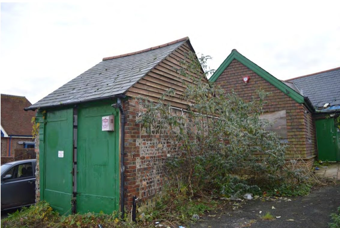
Plate 18: Building 2, view of north and west elevations, facing south-east (6969_0027)
