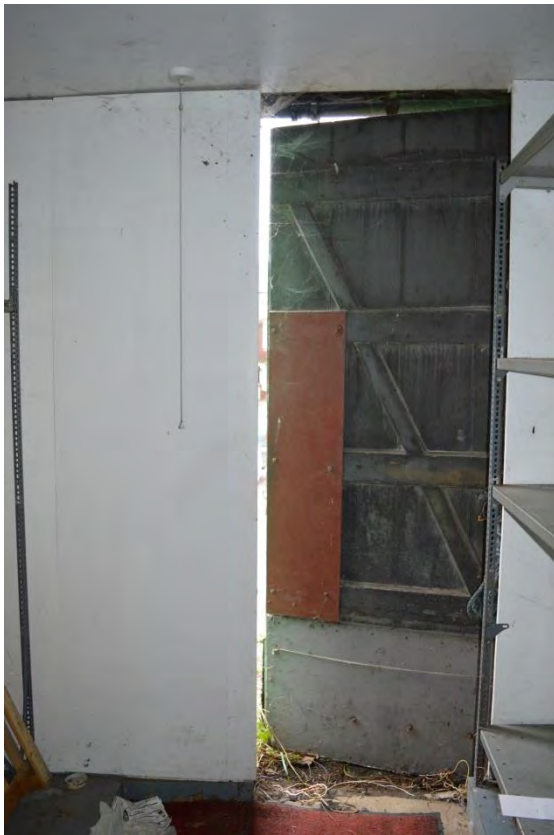
Plate 22: Building 2 interior, principal doorway, facing north (6969_0035)
