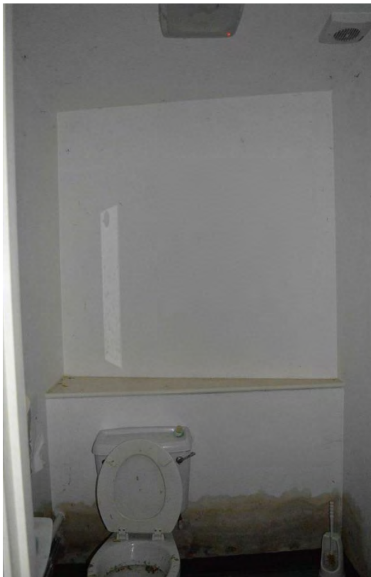
Plate 14: Building 1 interior, south-west room (WC facility), facing south (6969_0047)
