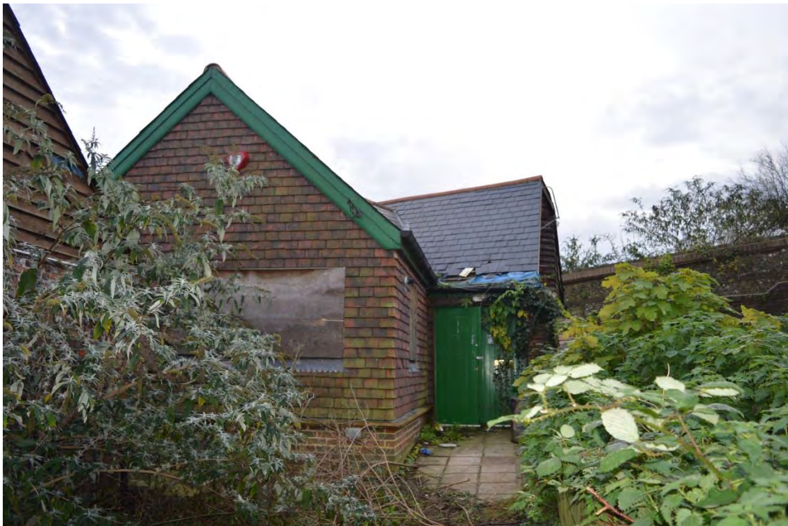
Plate 8: Building 1, view of modern north elevation and porch, facing south (6969_0025)
