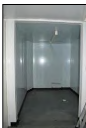
6969-0044 Building 1, interior, open-sided room to the east. Facing east
