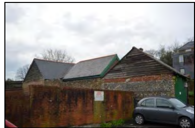
6969-0033 Overview of Buildings 1 & 2, view of east elevations. Facing southwest
