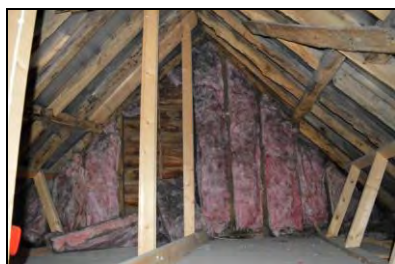
6969-0049 Building 1, interior, roof. Facing east
