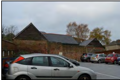
6969-0001 Buildings 1&2, east elevations & view of boundary wall. Facing west
