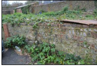
6969-0068 Retaining wall, Section 3. Facing southwest
