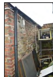
6969-0039 Building 2, view of south elevation. Facing east
