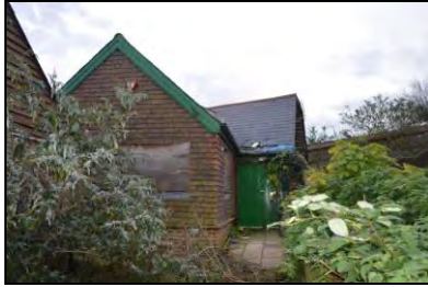
6969-0025 Building 1, view of modern north elevation and porch. Facing south
