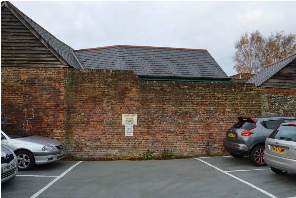
Plate 5: Building 1, view of boundary wall to the east, facing west (6969_0003)
