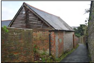
6969-0016 Building 1, view of south elevation fronting Brooman's Lane. Facing east
