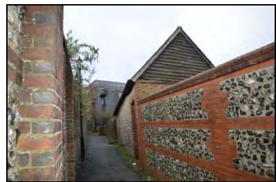
6969-0006 Building 1, view of south elevation along Brooman's Lane. Facing west
