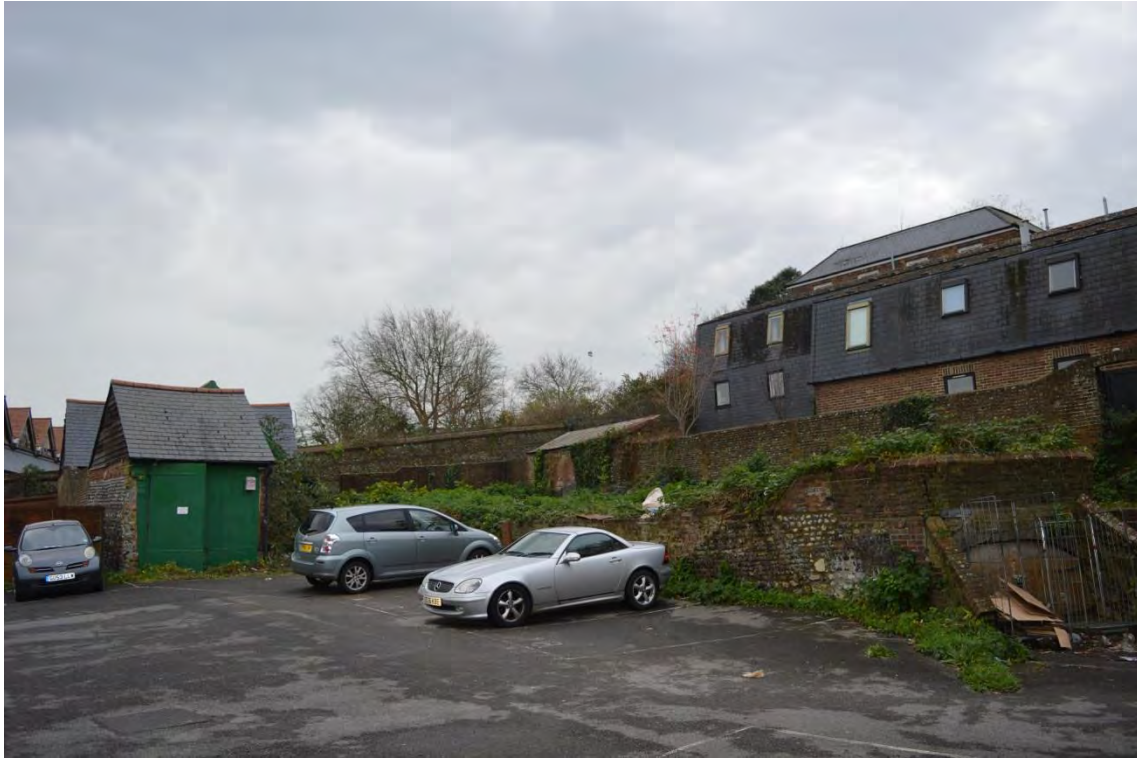
Plate 31: Overview of Building 2 and retaining wall, facing south-west (6969_0059)
