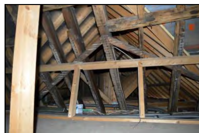
6969-0051 Building 1, interior, modern softwood roof over northern extension. Facing north
