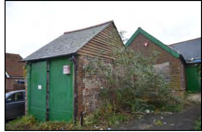
6969-0027 Building 2, view of north-west corner. Facing southeast
