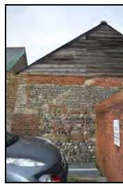
6969-0005 Building 2, view of south end of east elevation. Facing west
