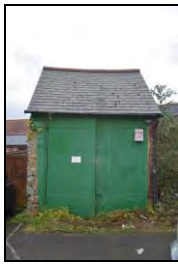
6969-0028 Building 2, view of north elevation. Facing south
