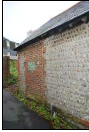
6969-0013 Building 1, view of south elevation and blocked original doorway. Facing northwest
