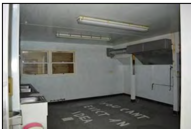
6969-0041 Building 1, interior, north-east corner of northern extension. Facing northeast
