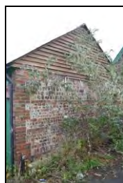
6969-0038 Building 2, view of west elevation. Facing southeast
