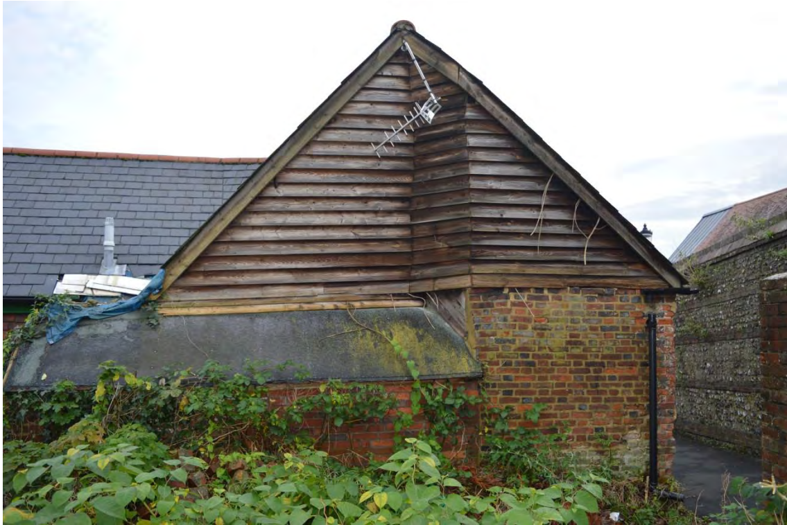
Plate 7: Building 1, view of west elevation of the southern range, facing east (6969_0018)
