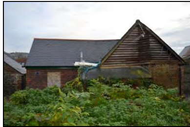
6969-0017 Building 1, view of west elevation. Facing east
