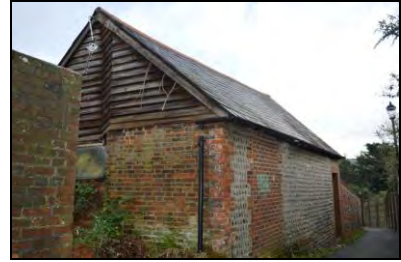
6969-0015 Building 1, view of south elevation fronting Brooman's Lane. Facing east
