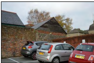
6969-0004 Building 2, view of east elevation. Facing northwest
