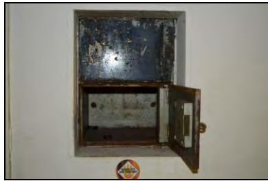
6969-0074 Building 1 interior, south-east room (office), safe detail (open). Facing south
