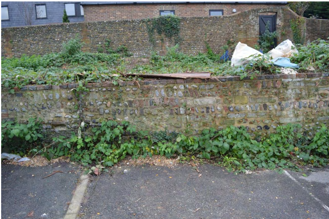
Plate 26: Retaining wall, Section 3, facing west (6969_0067)
