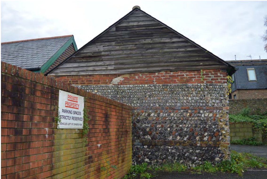
Plate 19: Building 2, view of east elevation, facing west (6969_0031)
