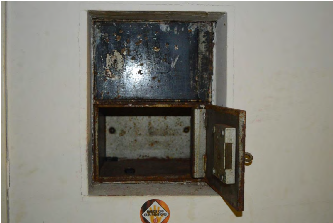
Plate 12: Building 1 interior, south-east room (office), safe detail, facing south (6969_0074)
