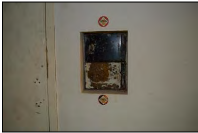
6969-0073 Building 1 interior, south-east room (office), safe detail (closed). Facing south
