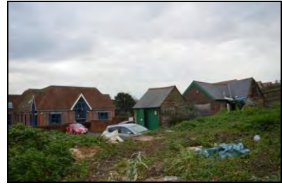
6969-0060 Overview of Buildings 1 & 2, taken from raised garden area (above vault). Facing southeast
