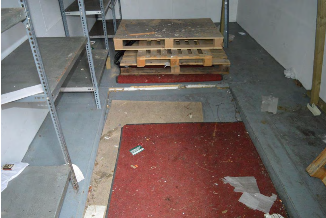
Plate 23: Building 2 interior, recessed floor level (vehicle inspection pit), facing south (6969_0037)
