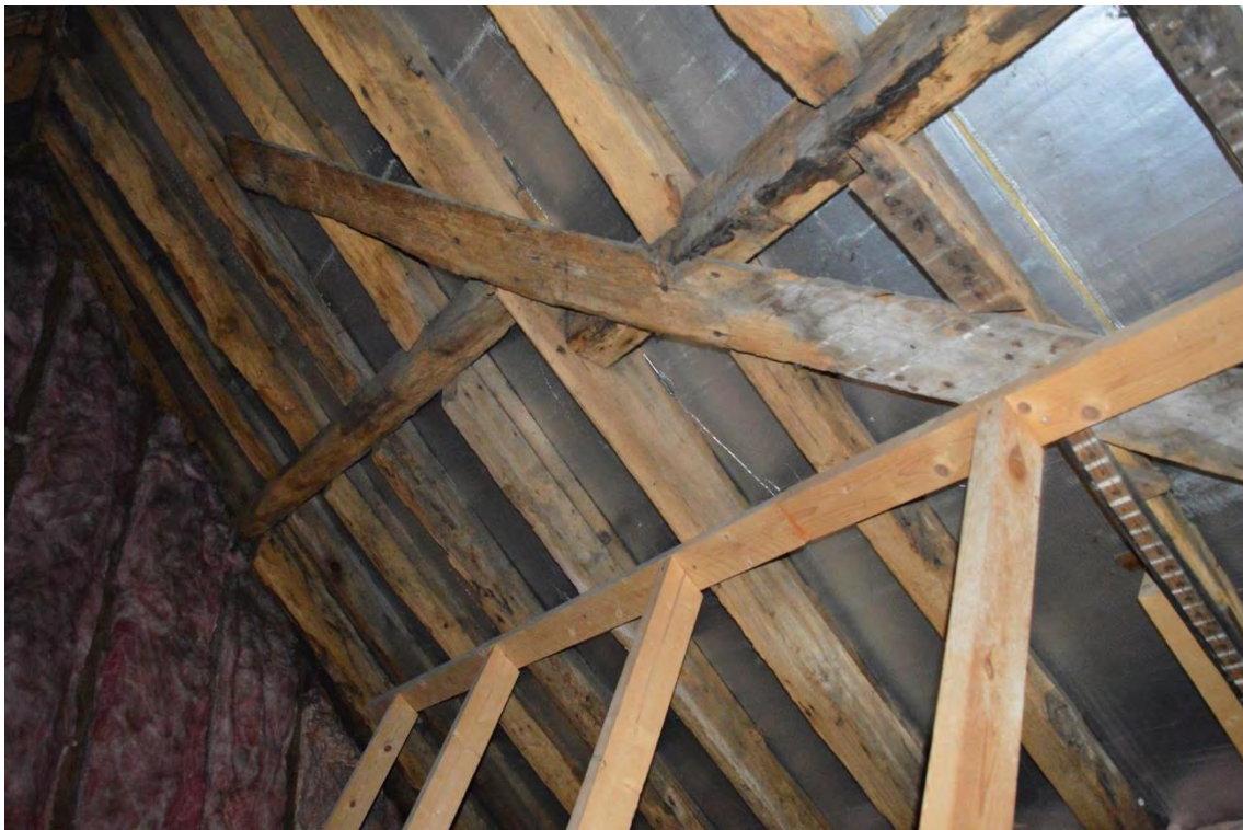
Plate 16: Building 1 roof interior, detail of rafter and purlin construction, facing south-east (6969_0055)
