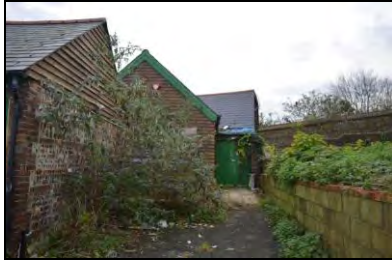
6969-0026 Building 2, west elevation & Building 1, view of north elevation and porch. Facing south
