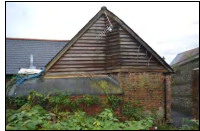
6969-0018 Building 1, view of west elevation of the southern range. Facing east
