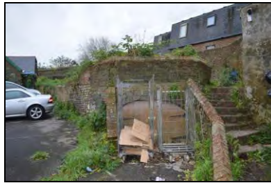
6969-0062 Retaining wall, showing entrance (Section 1) towards the northern end. Facing southwest
