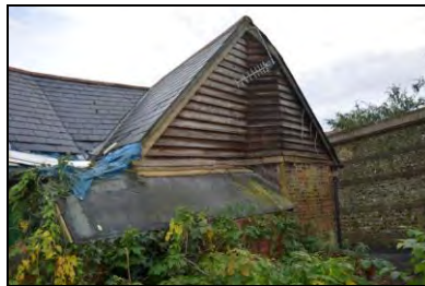
6969-0020 Building 1, view of west elevation of the southern range. Facing southeast
