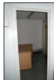
6969-0045 Building 1, interior, south-east room (office). Facing southeast
