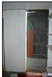
6969-0035 Building 2, interior, principal doorway. Facing north
