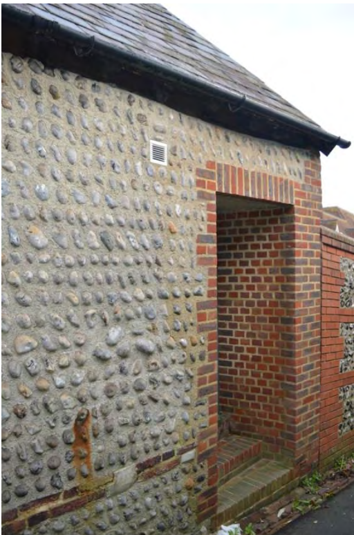
Plate 2: Building 1, view of south-east corner and modern doorway, facing east (6969_0010)
