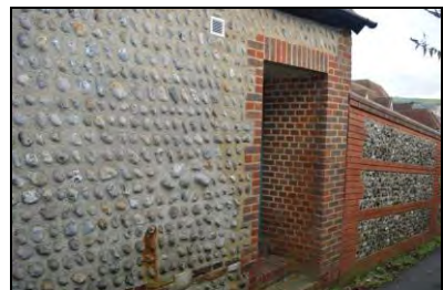
6969-0009 Building 1, view of south-east corner and modern doorway. Facing northeast
