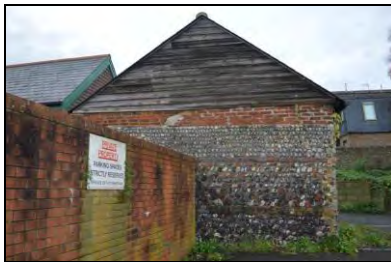
6969-0031 Building 2, view of east elevation. Facing west
