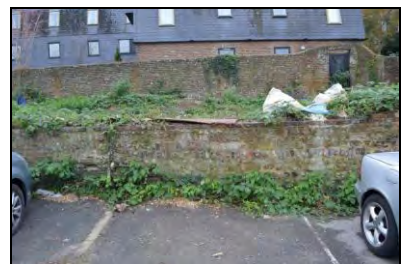
6969-0066 Retaining wall, Section 3. Facing west
