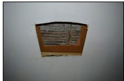
6969-0036 Building 2, interior, timber lathe ceiling. Facing south
