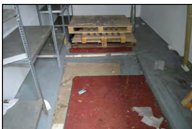
6969-0037 Building 2, interior, recessed floor level (vehicle inspection pit). Facing south
