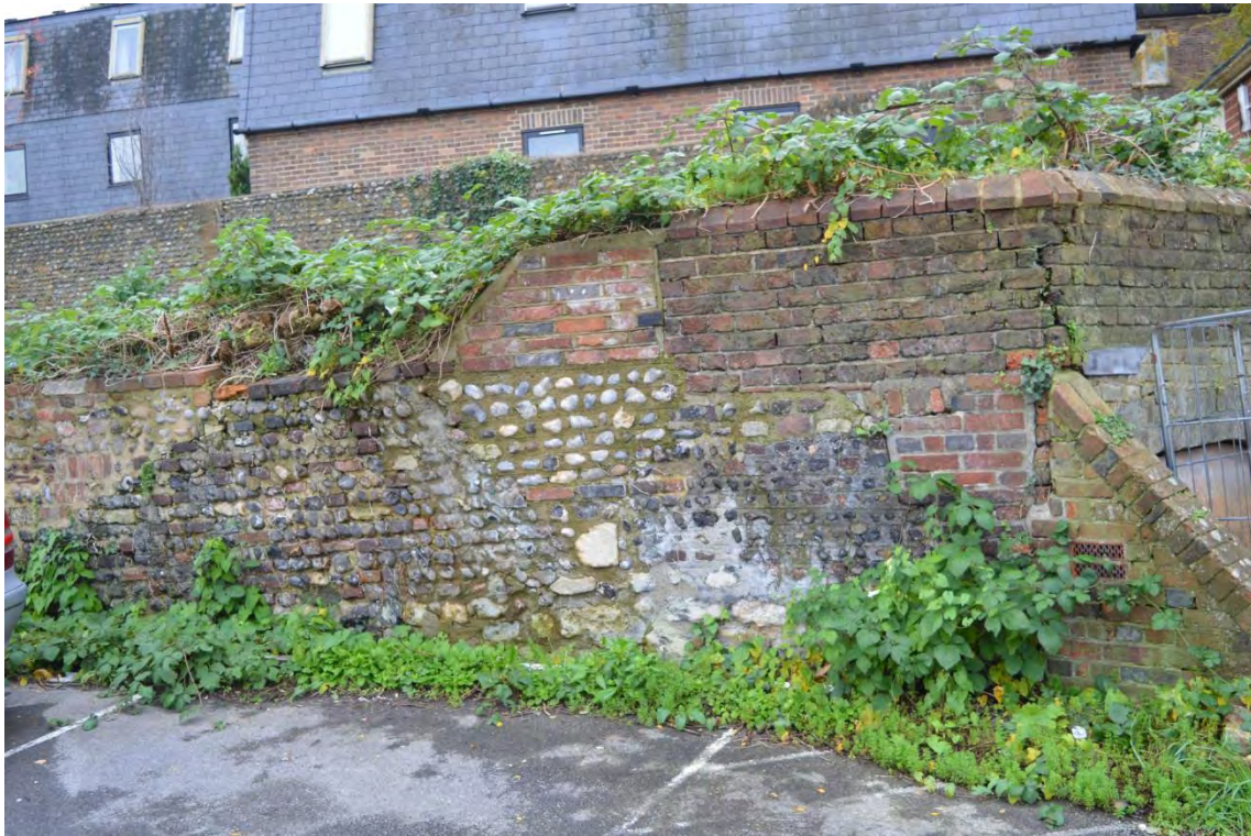
Plate 25: Retaining wall, Section 2, facing south-west (6969_0063)
