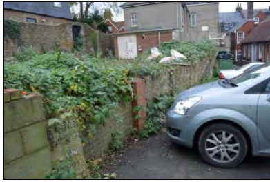
6969-0070 Retaining wall, Section 4, modern in-fill of suspected former access point. Facing northwest
