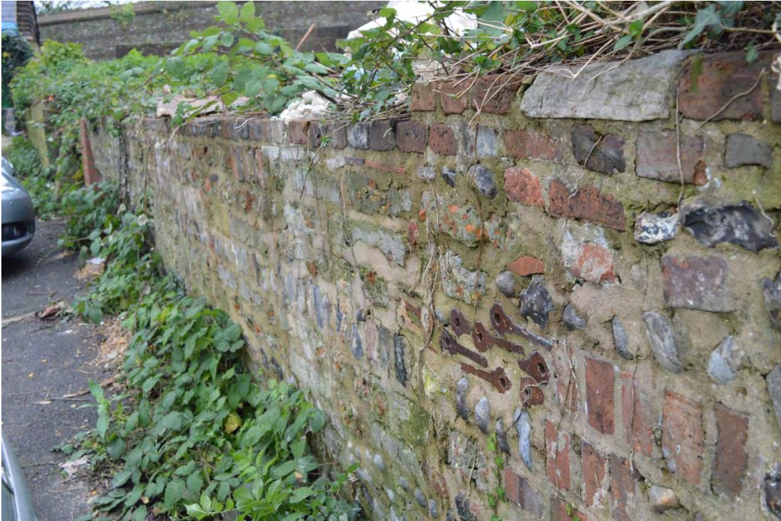
Plate 27: Retaining wall, Section 3, inlaid tile detail, facing south-west (6969_0065)
