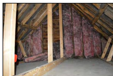
6969-0048 Building 1, interior, roof. Facing east
