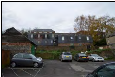
6969-0032 Overview of Building 2 & Retaining Wall. Facing west
