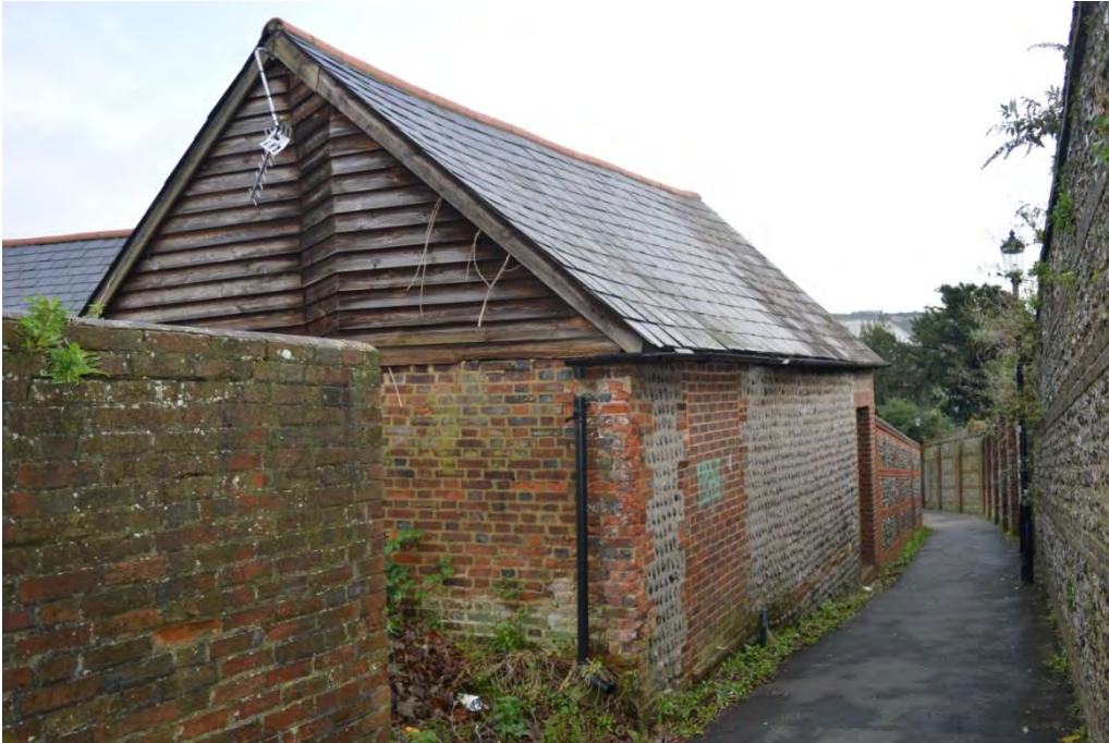
Plate 1: Building 1, view of south elevation fronting Brooman's Lane, facing east (6969_0016)
