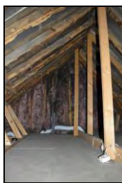
6969-0053 Building 1, interior, roof. Facing west
