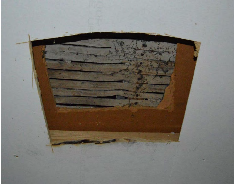
Plate 21: Building 2 interior, timber lathe ceiling, facing south (6969_0036)
