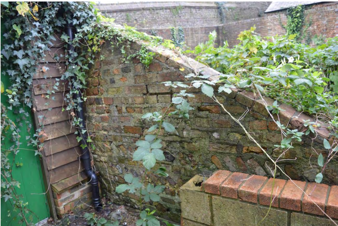
Plate 30: Retaining wall, Section 6, facing south-west (6969_0072)
