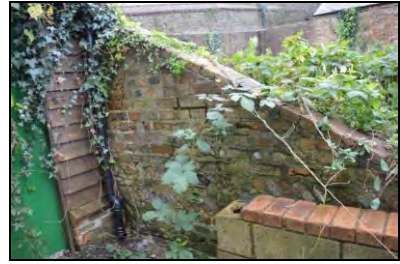
6969-0072 Retaining wall, Section 6. Facing southwest
