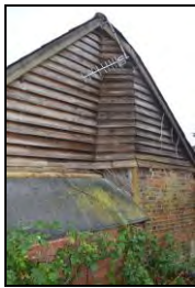
6969-0019 Building 1, view of west elevation of the southern range. Facing southeast
