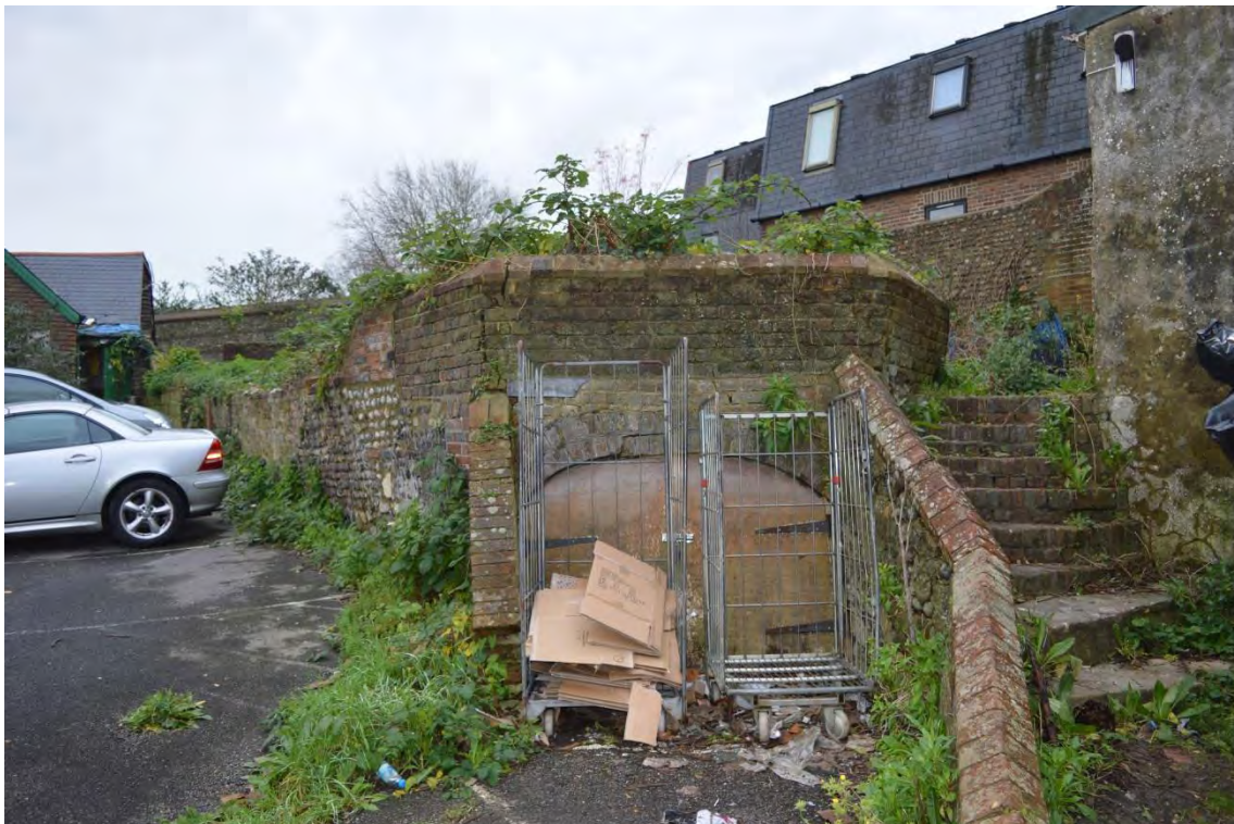
Plate 24: Retaining wall, showing entrance (Section 1) towards the northern end, facing south-west (6969_0062)
