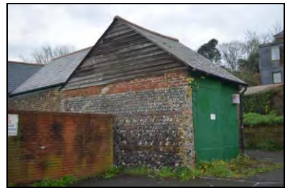
6969-0030 Building 2, view of north-east corner. Facing southwest
