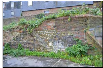
6969-0063 Retaining wall, Section 2. Facing southwest
