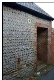
6969-0011 Building 1, view of south-east corner and modern doorway. Facing northeast
