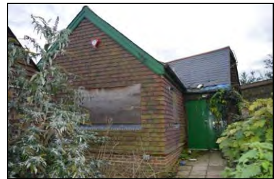
6969-0024 Building 1, view of modern north elevation and porch. Facing south
