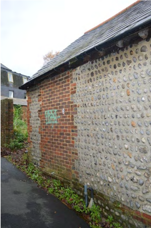
Plate 3: Building 1, view of south elevation and blocked original doorway, facing west (6969_0013)
