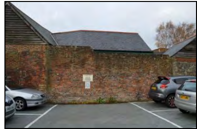
6969-0003 Building 1, view of boundary wall to the east. Facing west
