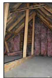
6969-0054 Building 1, interior, roof. Facing east
