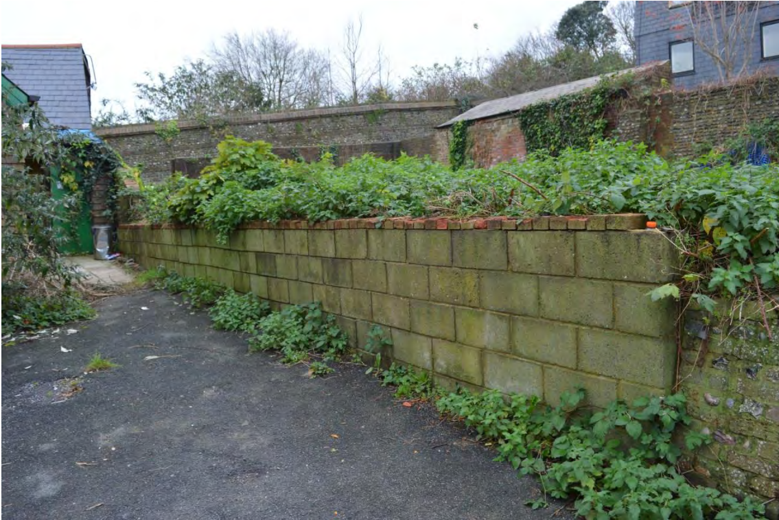
Plate 29: Retaining wall, Section 5, concrete block construction, facing south-west (6969_0071)
