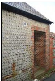
6969-0010 Building 1, view of south-east corner and modern doorway. Facing northeast
