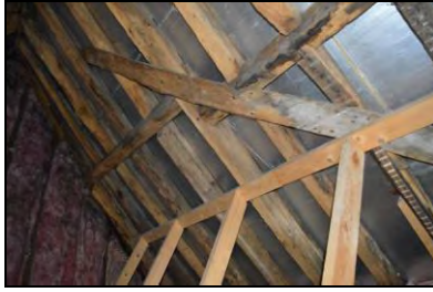
6969-0055 Building 1 roof interior, detail of rafter and purlin construction. Facing southeast
