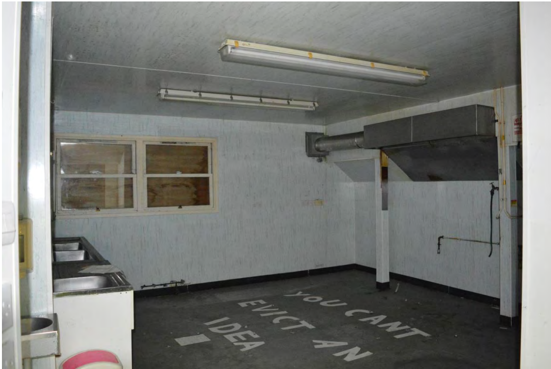
Plate 15: Building 1 interior, north-east corner of northern extension, facing north-east (6969_0041)
