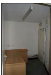
6969-0046 Building 1, interior, south-east room (office). Facing southeast
