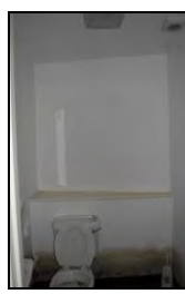
6969-0047 Building 1, interior, south-west room (WC facility). Facing south
