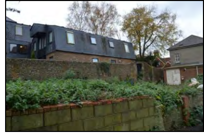
6969-0057 Overview of raised garden above vault. Facing northwest
