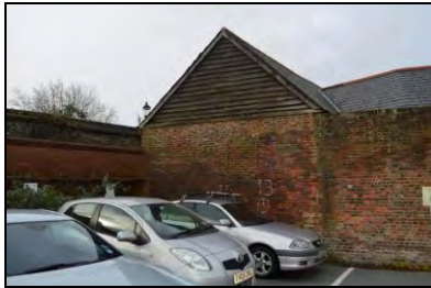
6969-0002 Building 1, view of east elevation. Facing southwest
