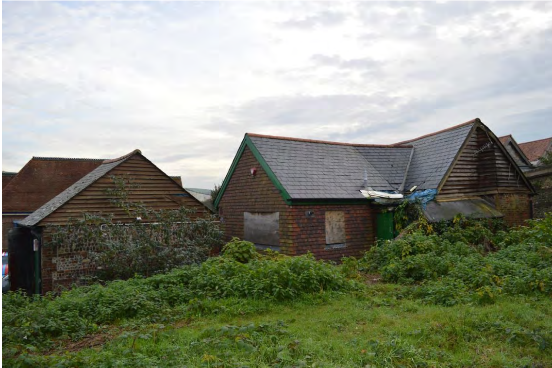
Plate 9: Overview of Buildings 1 & 2, north and west elevations, facing south-east (6969_0022)
