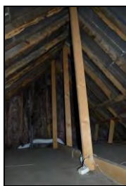
6969-0052 Building 1, interior, roof. Facing west
