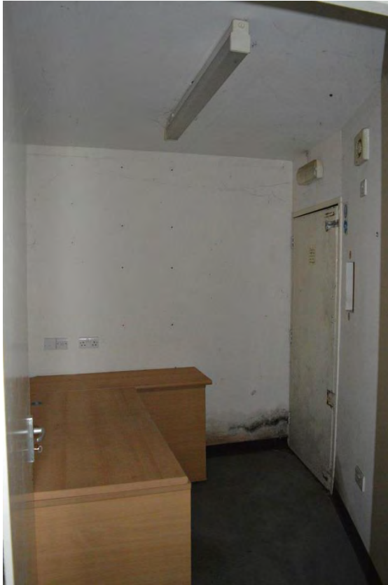
Plate 11: Building 1 interior, south-east room (office), facing east (6969_0046)
