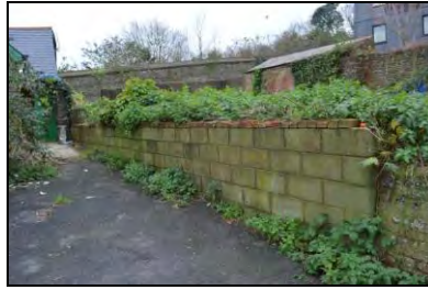
6969-0071 Retaining wall, Section 5, concrete block construction. Facing southwest
