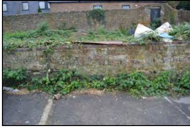
6969-0067 Retaining wall, Section 3. Facing west
