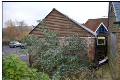
6969-0023 Building 2, view of west elevation. Facing east
