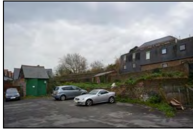
6969-0059 Overview of Building 2 and retaining wall. Facing southwest
