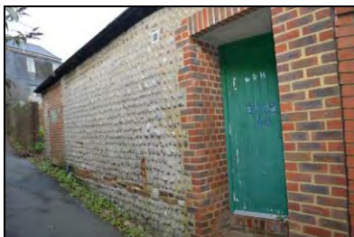
6969-0008 Building 1, view of south elevation. Facing northwest
