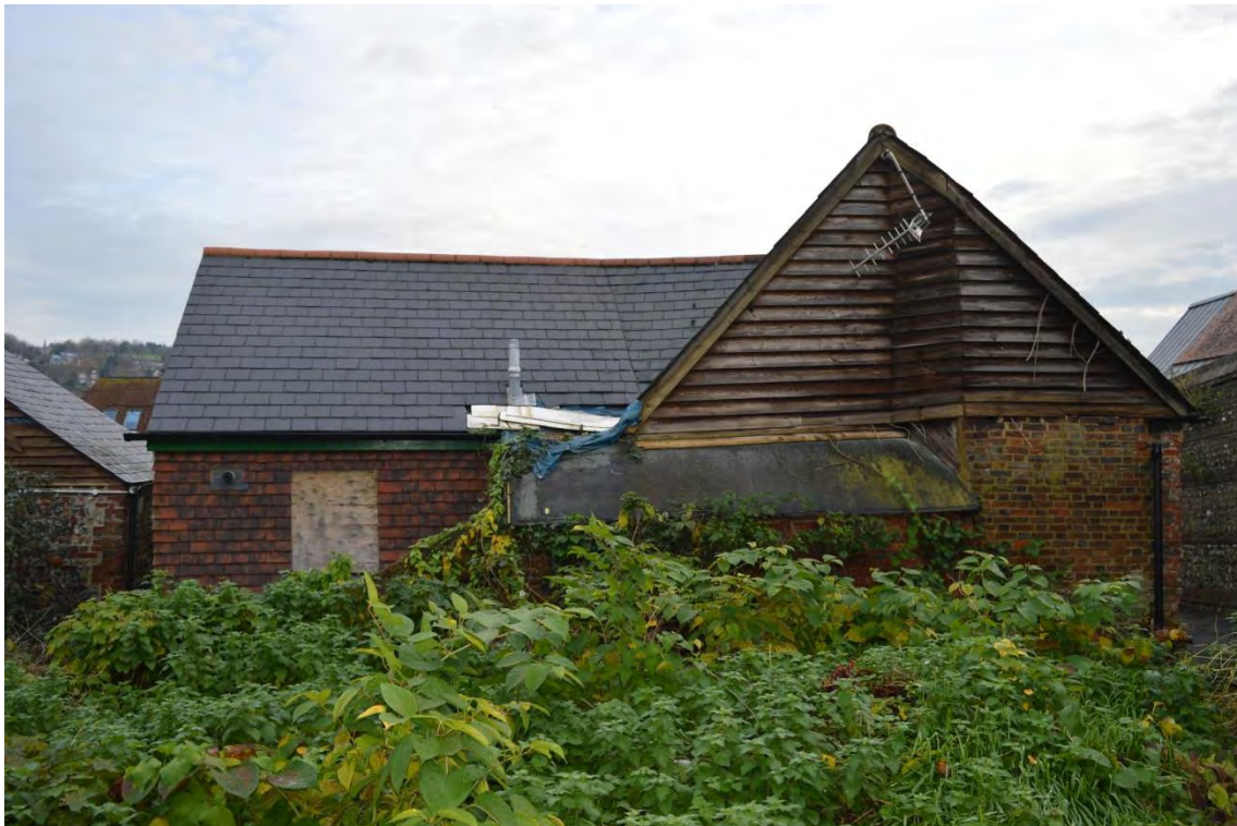
Plate 6: Building 1, view of west elevation, facing east (6969_0017)
