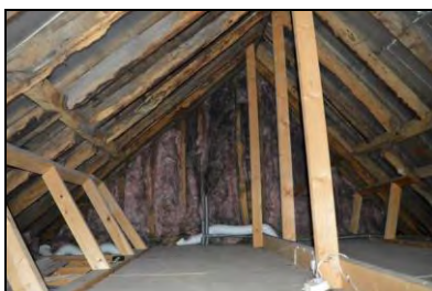
6969-0050 Building 1, interior, roof. Facing west
