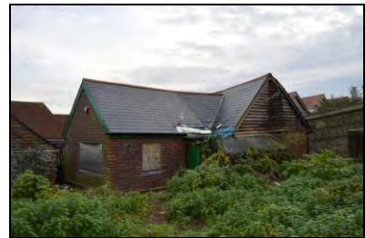
6969-0021 Building 1, view of north & west elevations. Facing southeast
