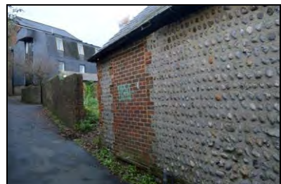
6969-0012 Building 1, view of south elevation and blocked original doorway. Facing northwest
