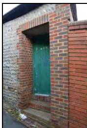
6969-0007 Building 1, view of south-east corner and modern doorway. Facing northwest
