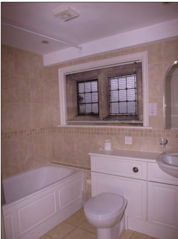
Photo 56: First floor, Room 1, bathroom, mock-Tudor window detail, facing north-east (7195-0056)
