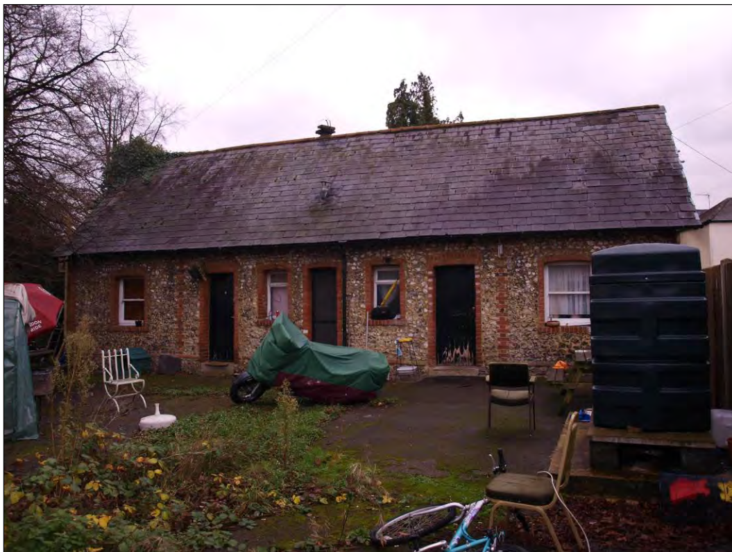
Photo 129: Outbuilding 2 (Elevation 12), facing south (7195-0129)
