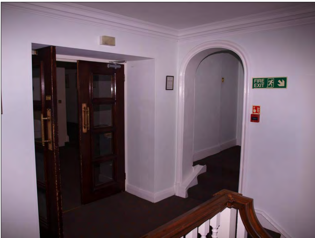
Photo 44: First floor, Landing 1, doorway to main circulation area, facing north-west (7195-0044)
