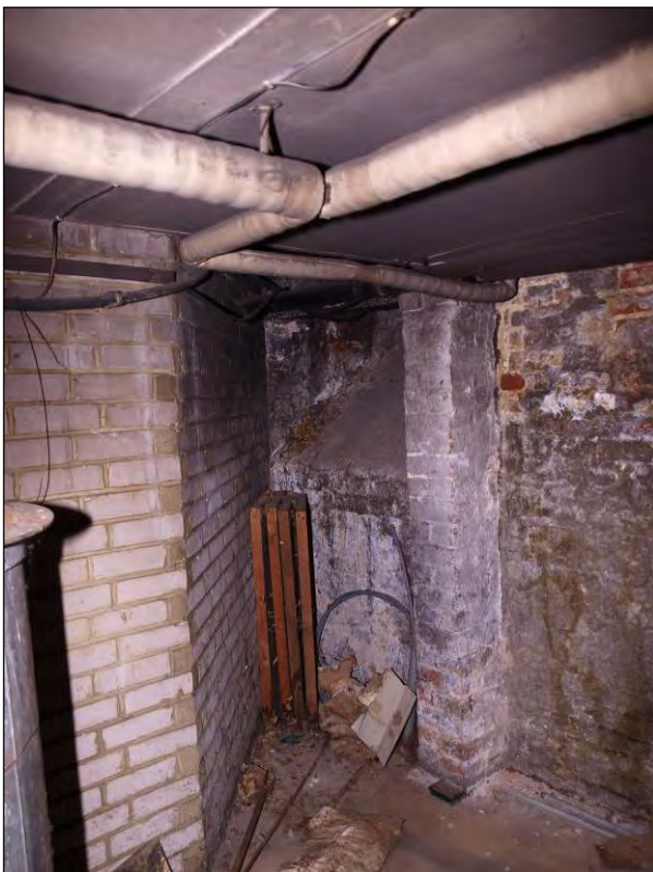
Photo 100: Basement, Boiler Room, coal chute, facing south-east (7195-0100)
