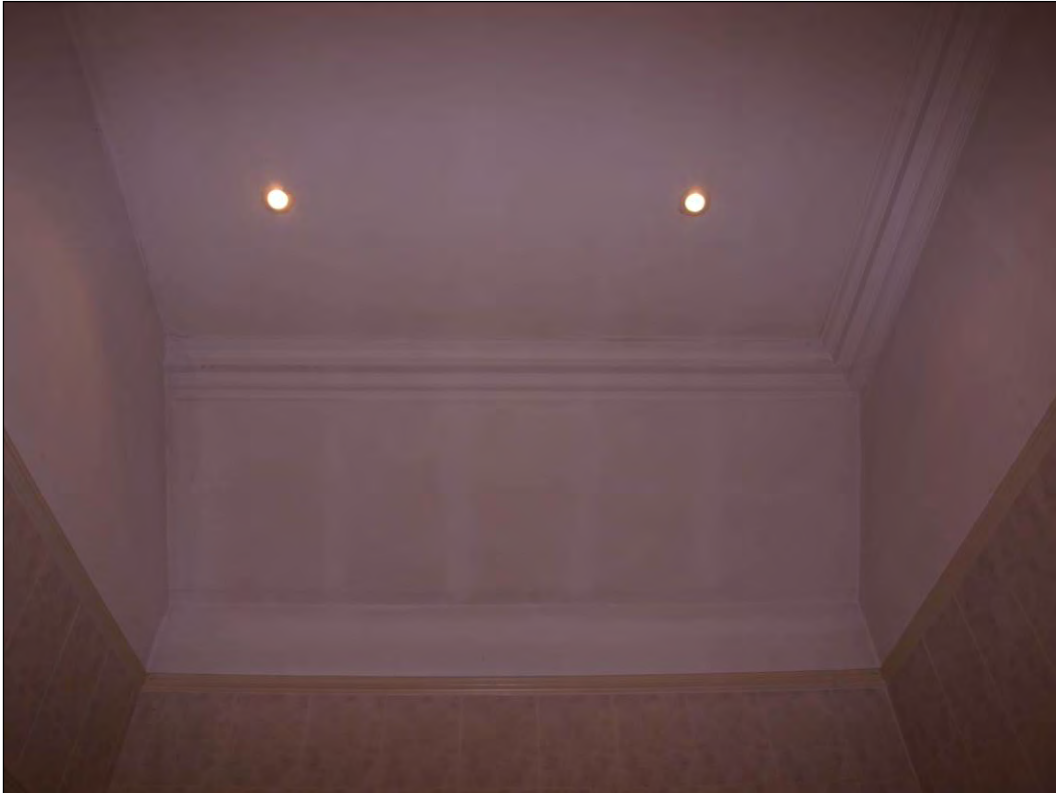
Photo 71: First floor, Room 3, bathroom, ceiling and cornice detail, facing west (7195-0071)
