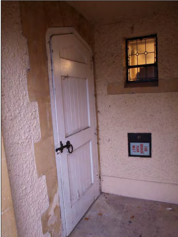
Photo 105: Door to garden, facing south-west (7195-0105)
