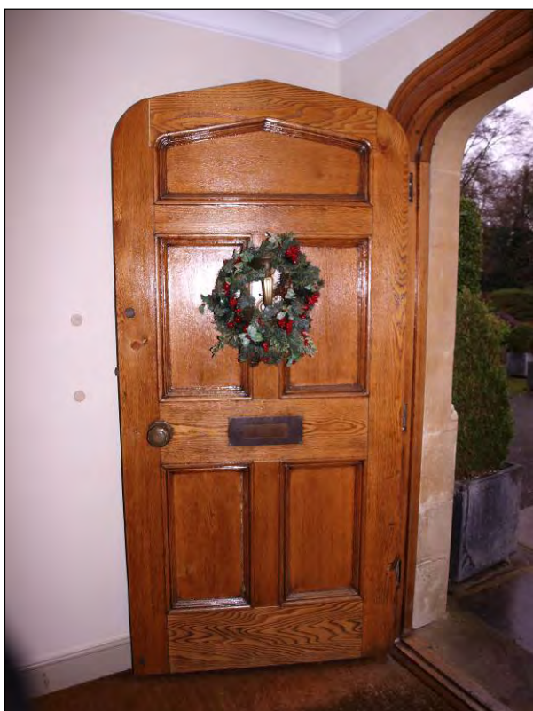
Photo 40: Ground floor, principal hotel entrance, facing north (7195-0040)
