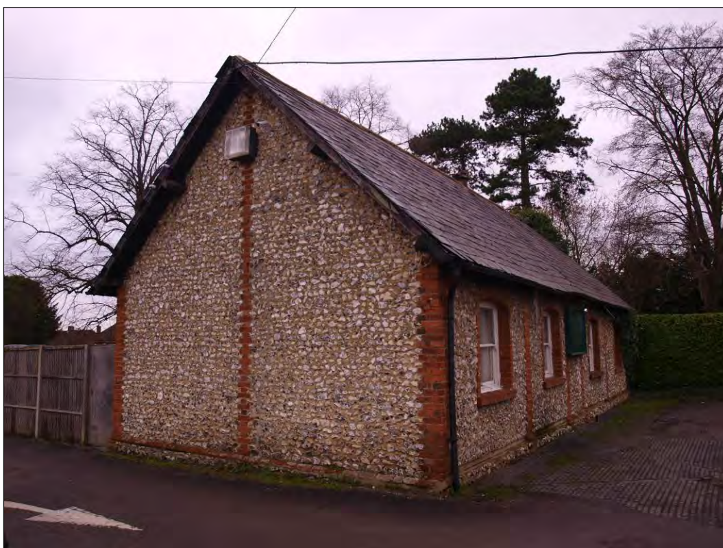
Photo 128: Outbuilding 2 (Elevation 11), facing north-east (7195-0128)
