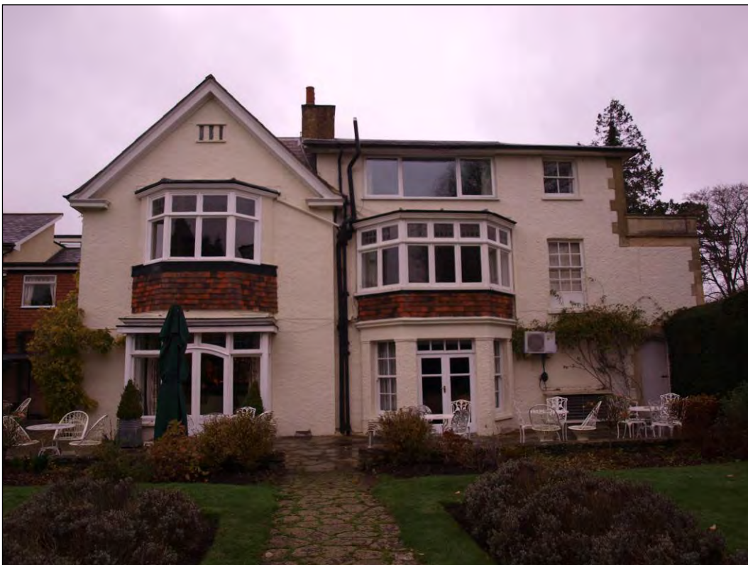
Photo 106: South elevation (Elevation 2), facing north (7195-0106)
