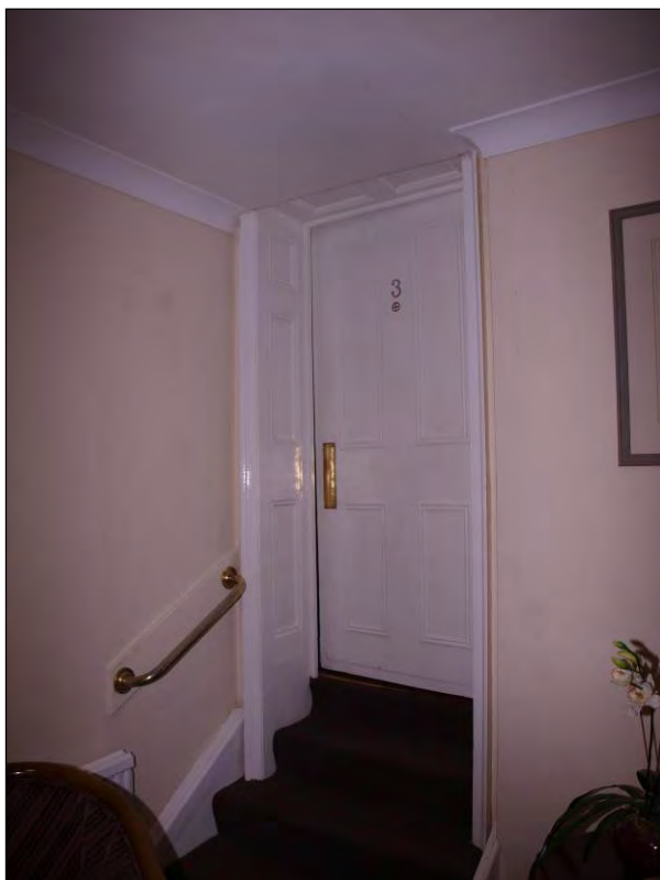
Photo 64: First floor, main circulation area leading from Landing 1, Room 3 access steps, facing south-west (7195-0064)
