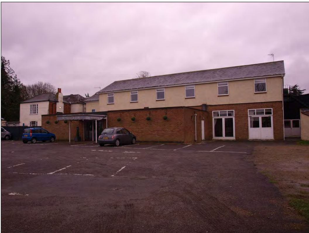
Photo 114: North elevation of Function Suite, facing south (7195-0114)
