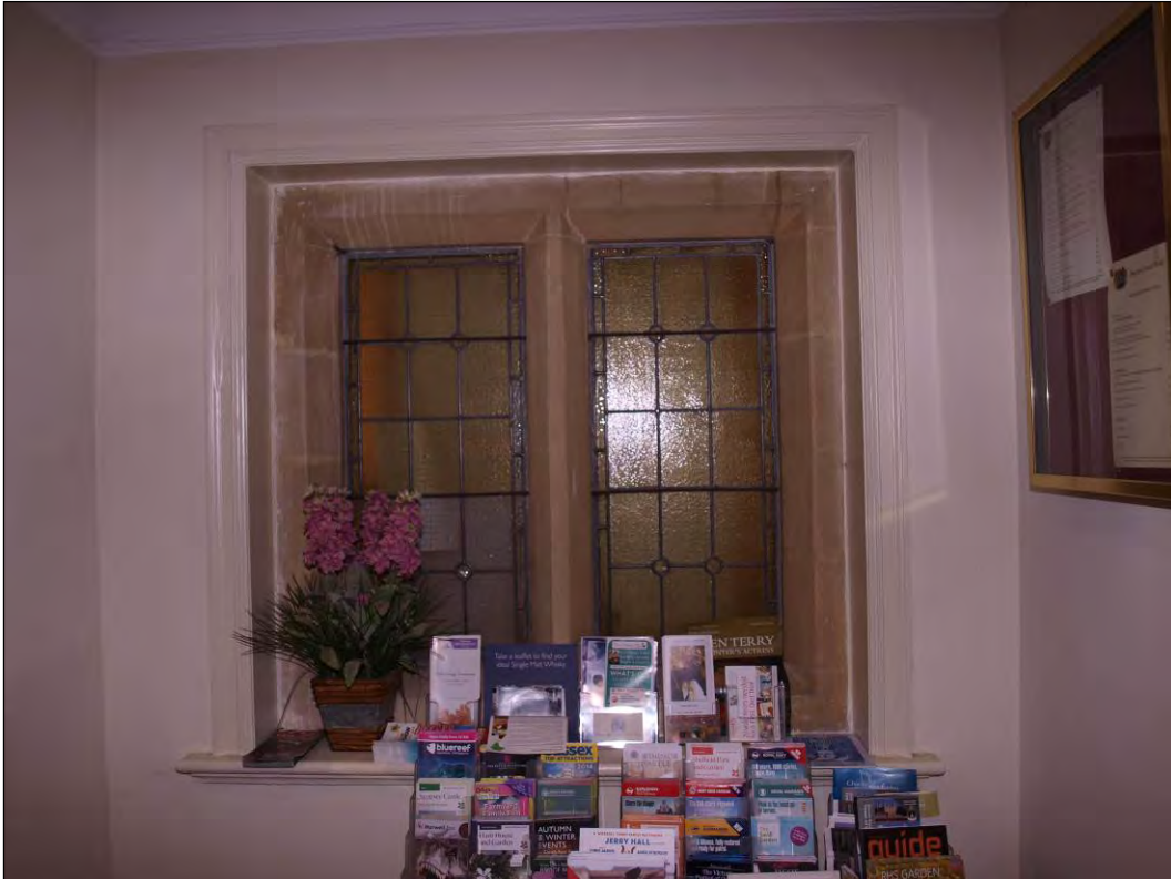
Photo 41: Ground floor, main entrance, mock-Tudor window detail, facing south (7195-0041)
