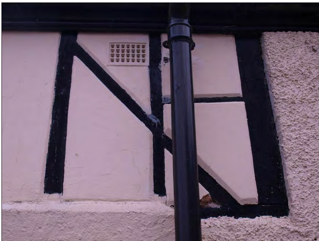
Photo 120: Outbuilding 1 (Elevation 6), detail of timber framework, facing east (7195-0120)
