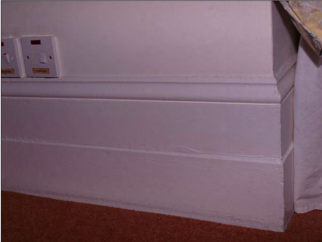
Photo 55: First floor, Room 1, skirting detail, facing east (7195-0055)
