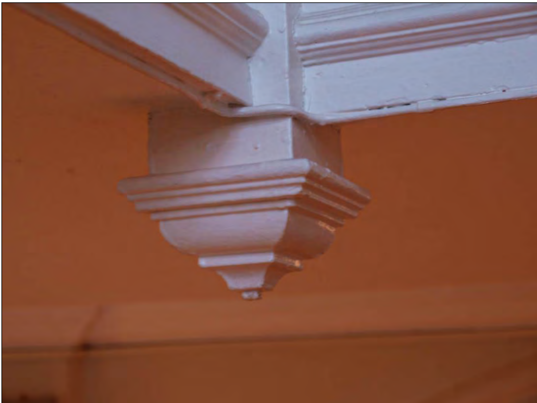
Photo 132: Hotel Entrance Lobby, ground floor, stair newel pendant detail, facing west (7195-0132)
