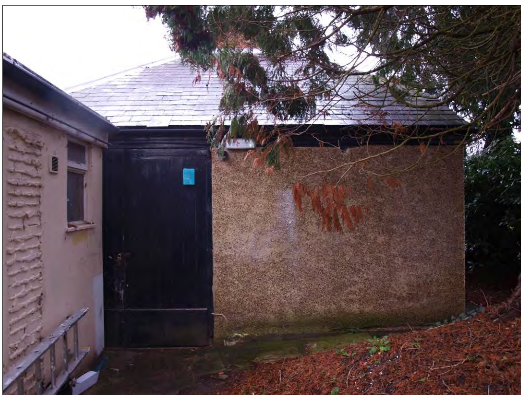
Photo 124: Outbuilding 1 (Elevation 9), facing north (7195-0124)
