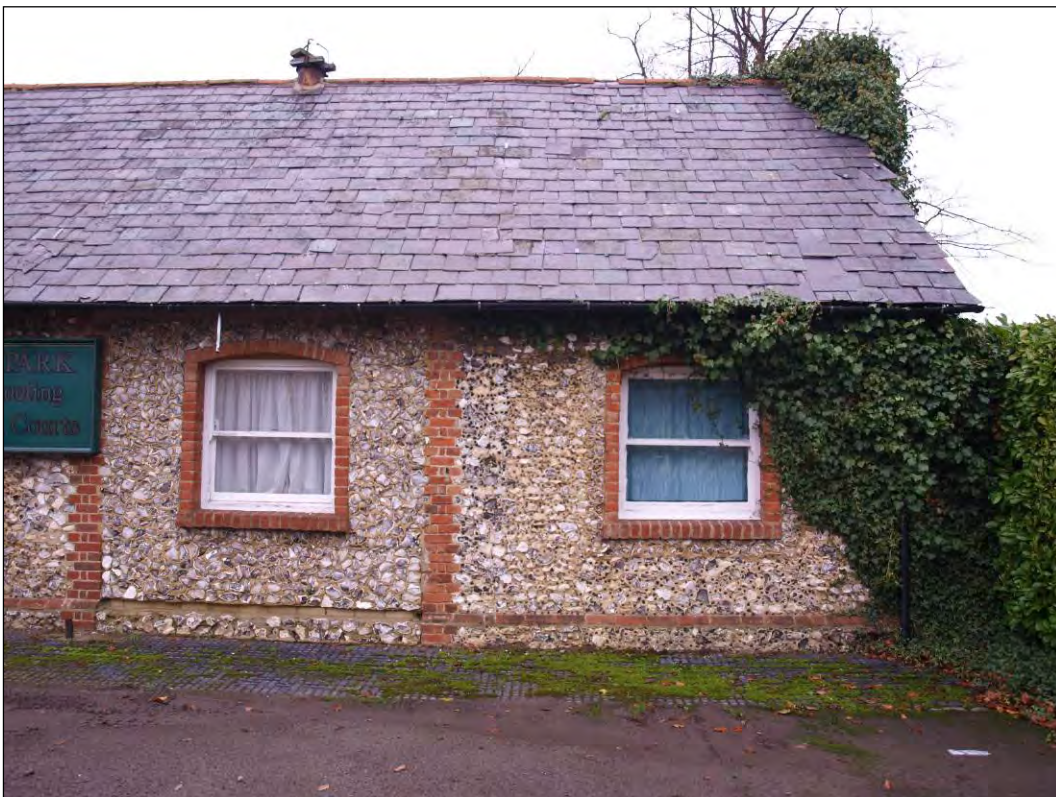
Photo 126: Outbuilding 2 (Elevation 10), facing north (7195-0126)
