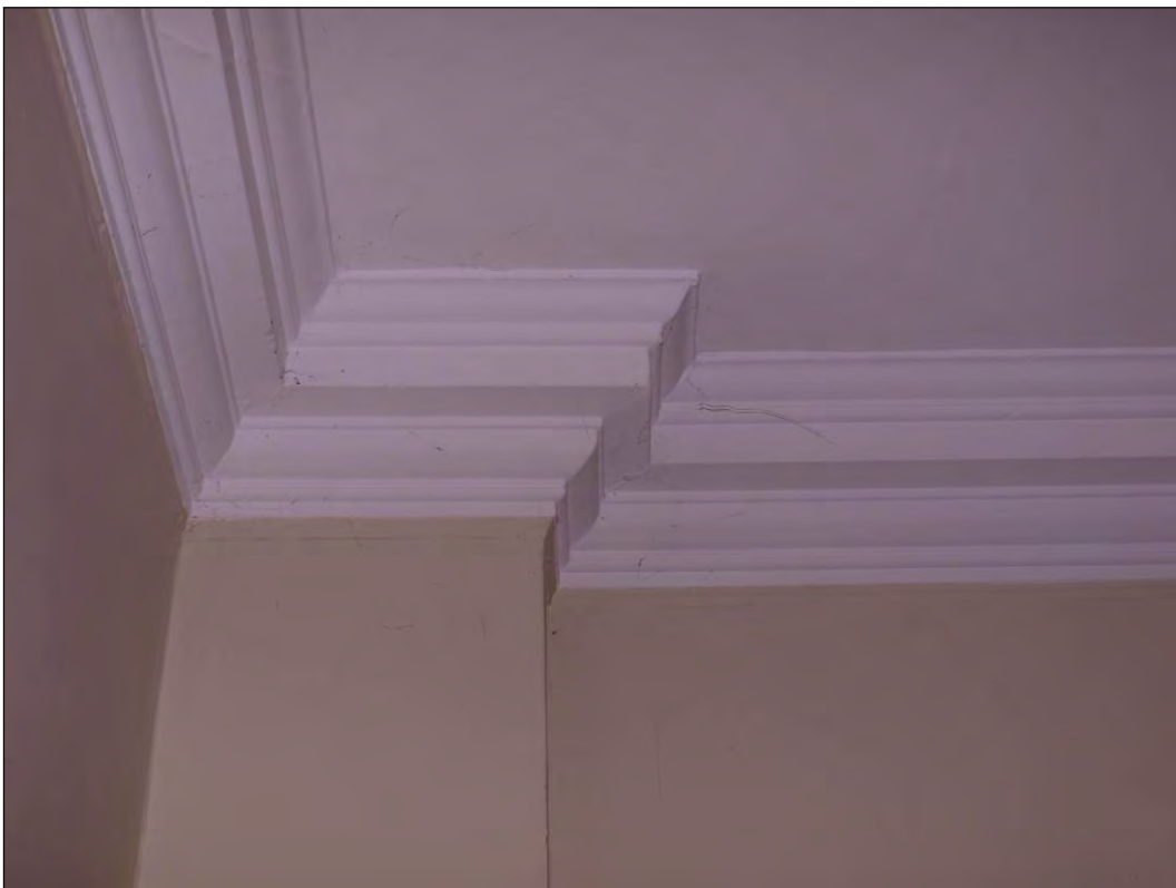
Photo 26: Ground floor, Lounge, cornice detail, north-east corner, facing east (7195-0026)
