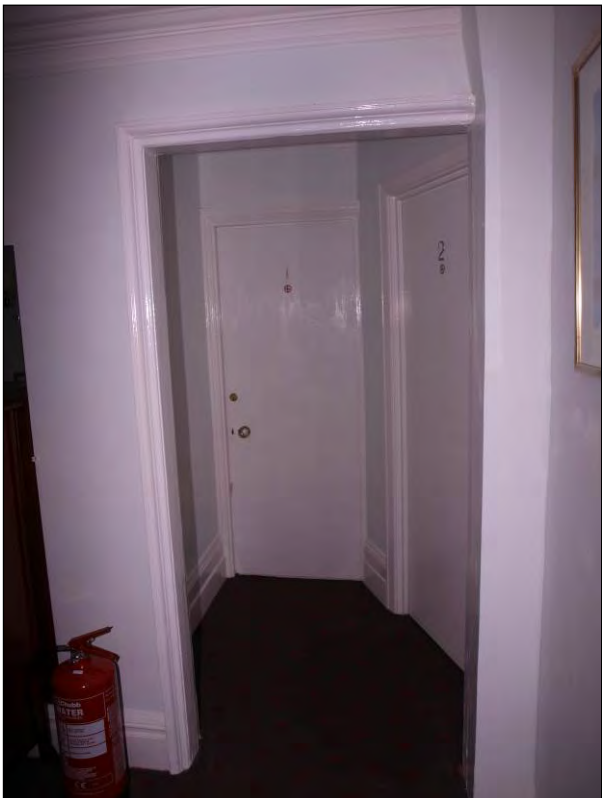
Photo 48: First floor, Landing 1, Rooms 1 & 2, facing south (7195-0048)
