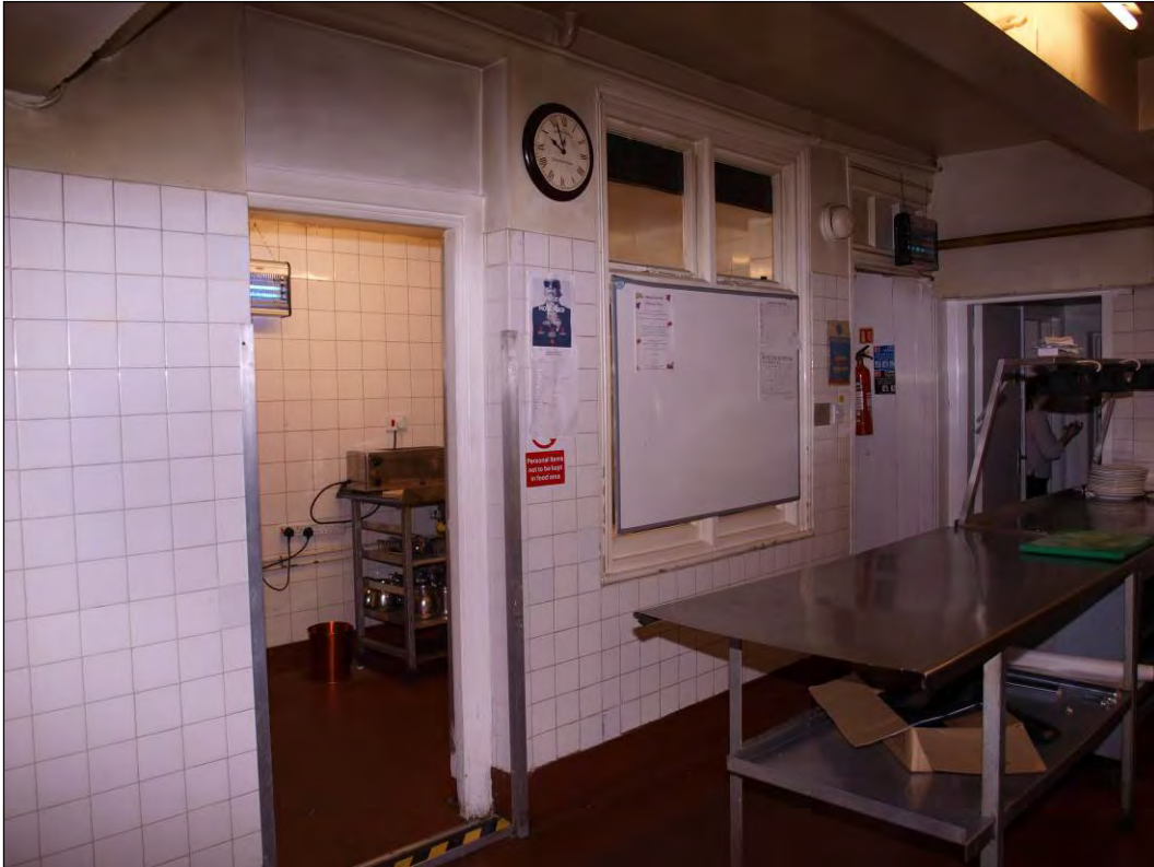
Photo 7: Ground floor, Kitchen Store entrance, facing south-east (7195-0007)
