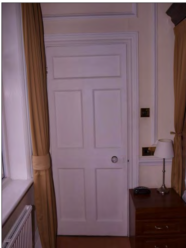
Photo 68: First floor, Room 3, bathroom door features, facing north (7195-0068)
