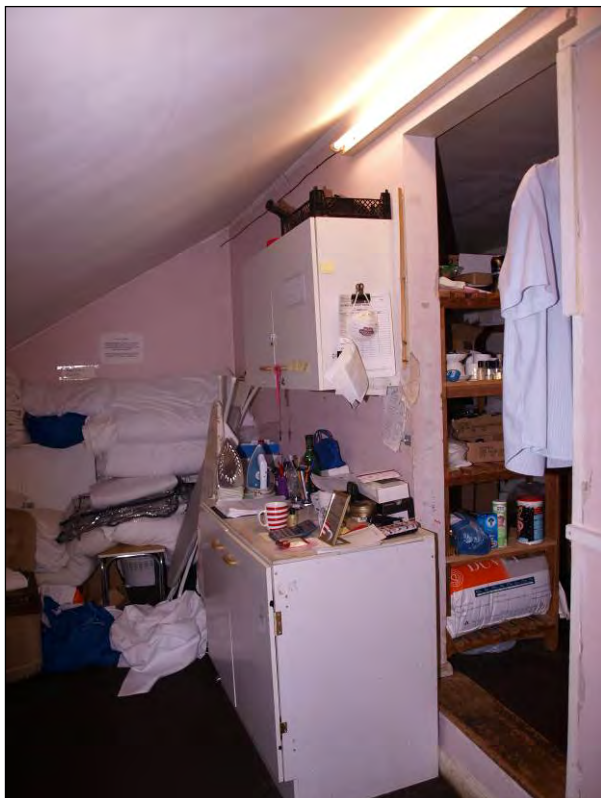
Photo 93: Second floor, Laundry Room & Store, overview, facing east (7195-0093)
