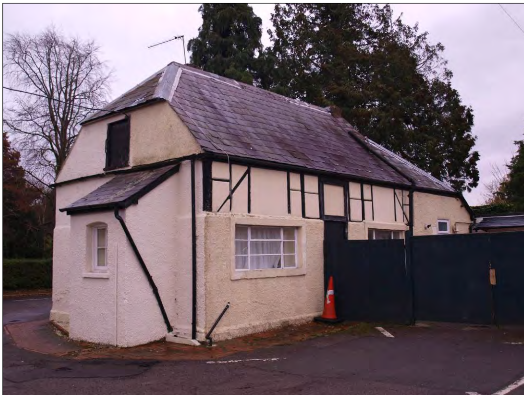
Photo 121: Outbuilding 1 (Elevations 6 & 7), facing south-east (7195-0121)
