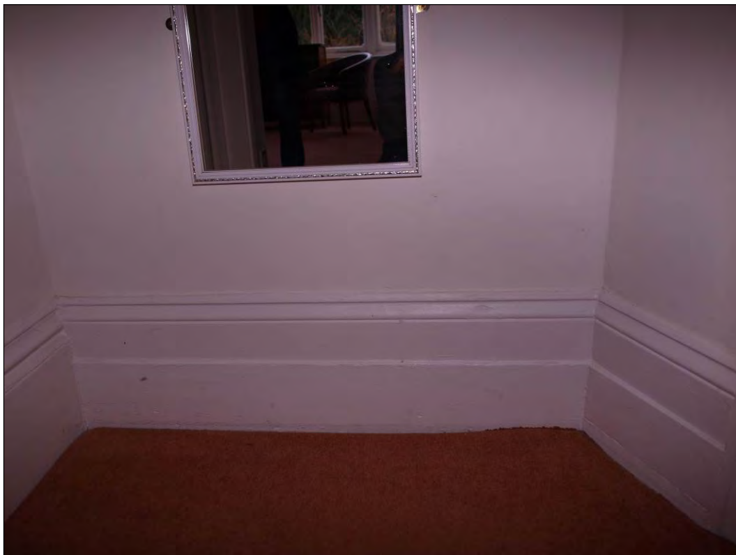
Photo 61: First floor, Room 2, skirting detail by door surround, facing north (7195-0061)
