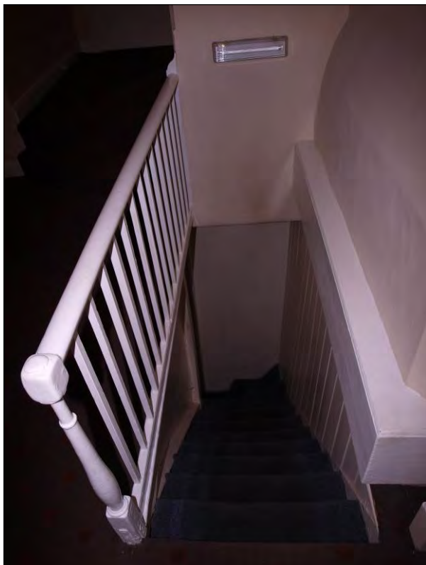
Photo 75: Second floor, northern stair, opening out onto Landing 2 (down), facing north (7195-0075)
