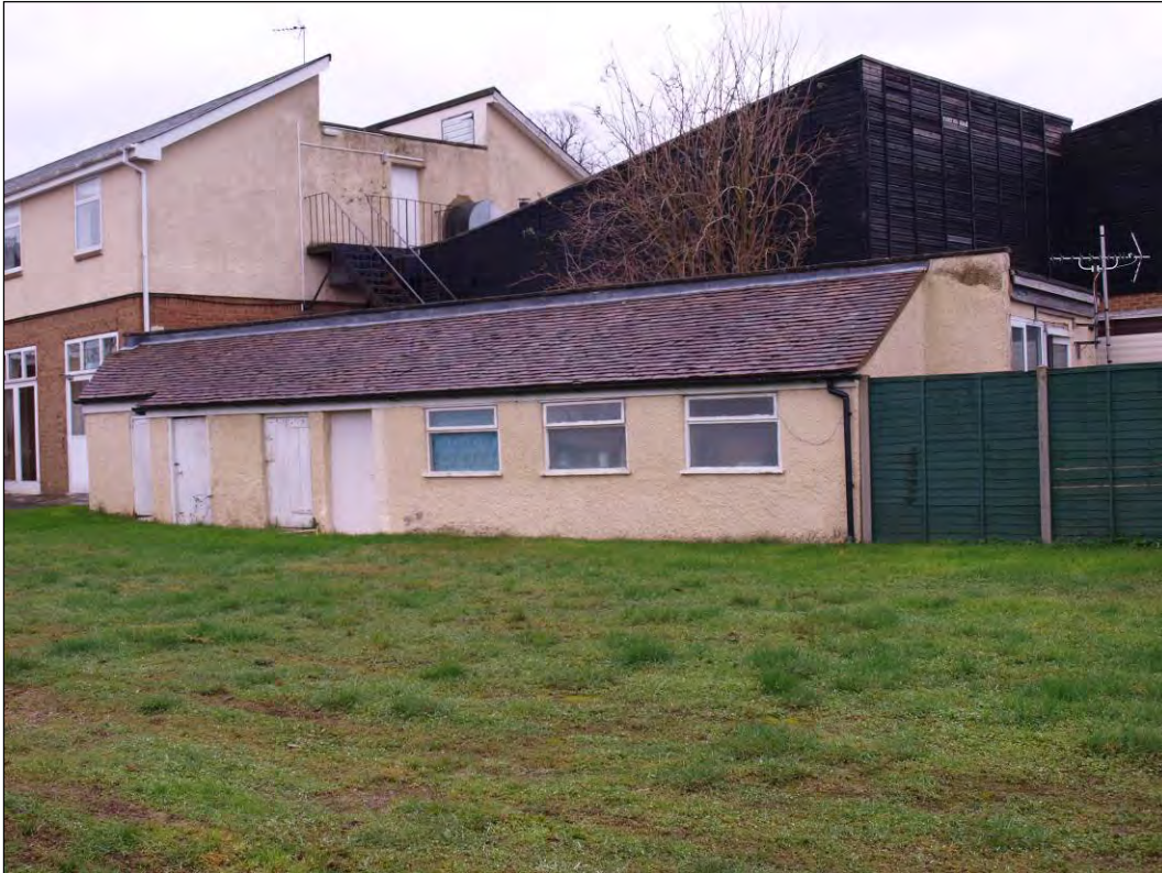
Photo 113: Outbuilding 3, facing south-east (7195-0113)
