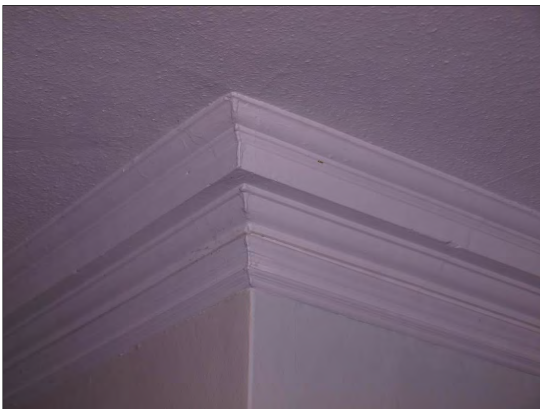
Photo 46: First floor, Landing 1, cornice detail above stairwell, facing south-east (7195-0046)
