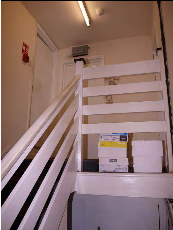
Photo 97: Upper first floor, western stair landing (no access to rooms on this level), facing west (7195-0097)
