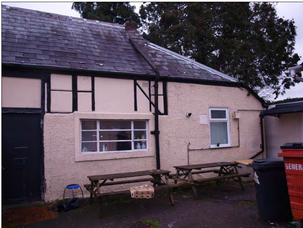
Photo 119: Outbuilding 1 (Elevation 6), southern end, facing south-east (7195-0119)
