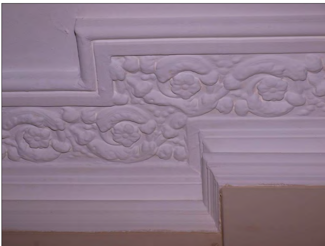
Photo 34: Ground floor, Meeting Room 2, plaster cornice & moulding detail, facing west (7195-0034)
