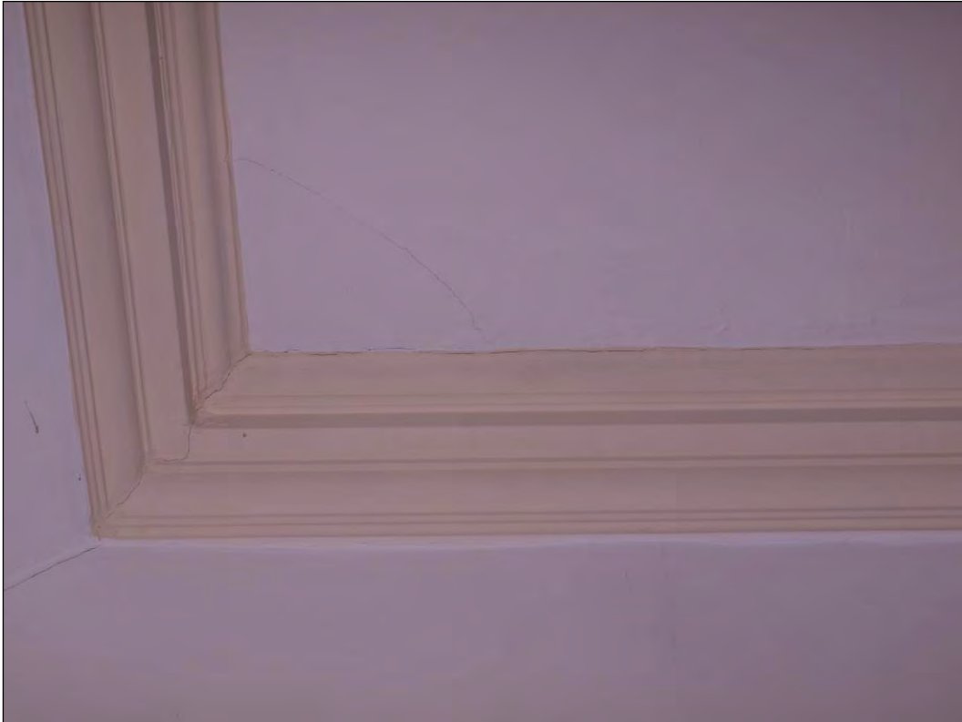
Photo 69: First floor, Room 3, cornice detail situated above bathroom door, facing north (7195-0069)
