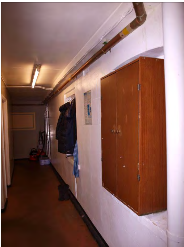
Photo 8: Ground floor, Kitchen 1 corridor access to Stores, facing east (7195-0008)
