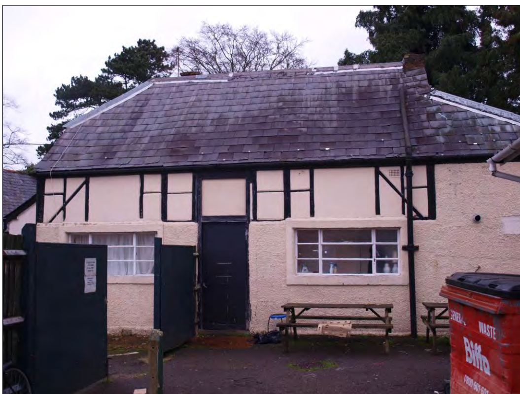
Photo 118: Outbuilding 1 (Elevation 6), facing east (7195-0118)
