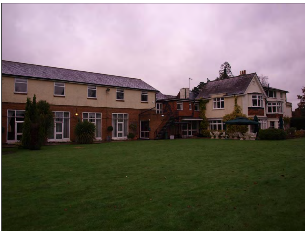
Photo 110: South elevation, facing north-east (7195-0110)
