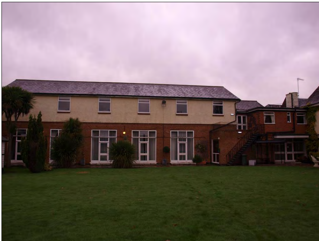
Photo 109: South elevation of Function Suite, facing north (7195-0109)
