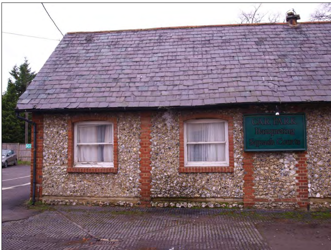
Photo 127: Outbuilding 2 (Elevation 10), facing north (7195-0127)
