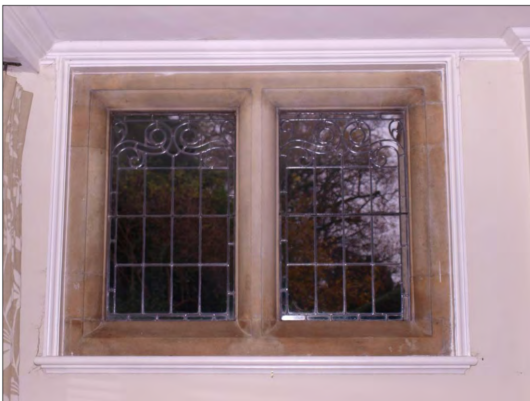
Photo 14: Ground floor, Dining Room, mock-Tudor window, facing south (7195-0014)
