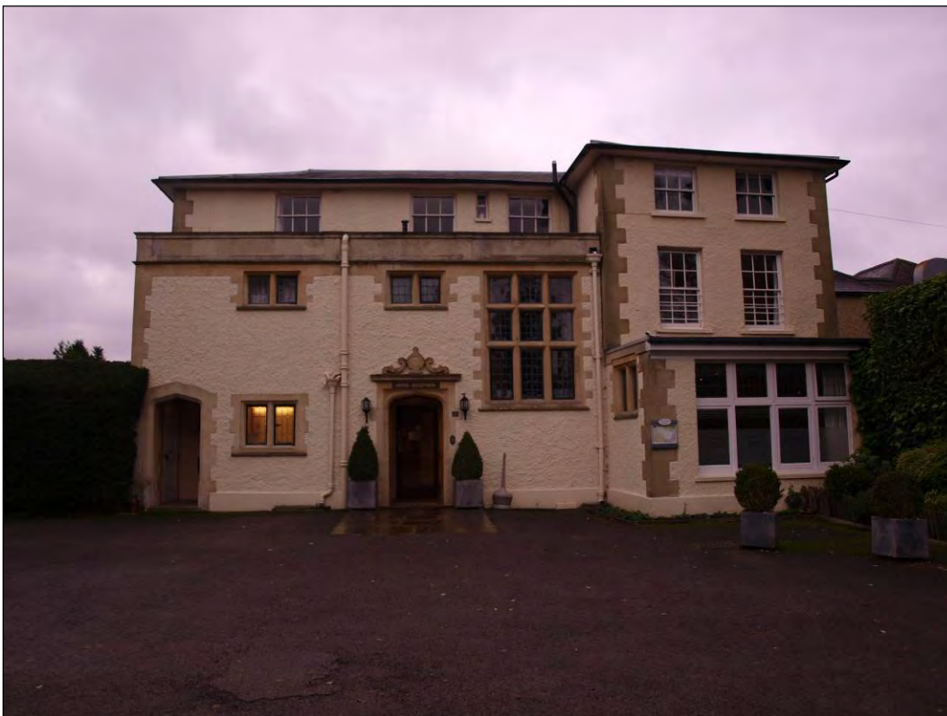
Photo 104: Principal elevation (Elevation 1), facing west (7195-0104)
