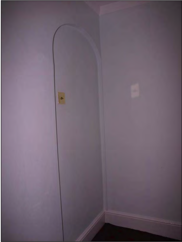
Photo 47: First floor, blocked opening opposite entrance to Room 4, facing north-west (7195-0047)
