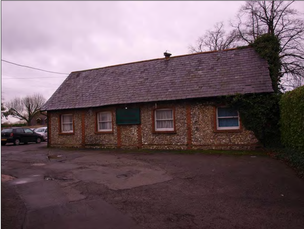
Photo 125: Outbuilding 2 (Elevation 10), facing north (7195-0125)
