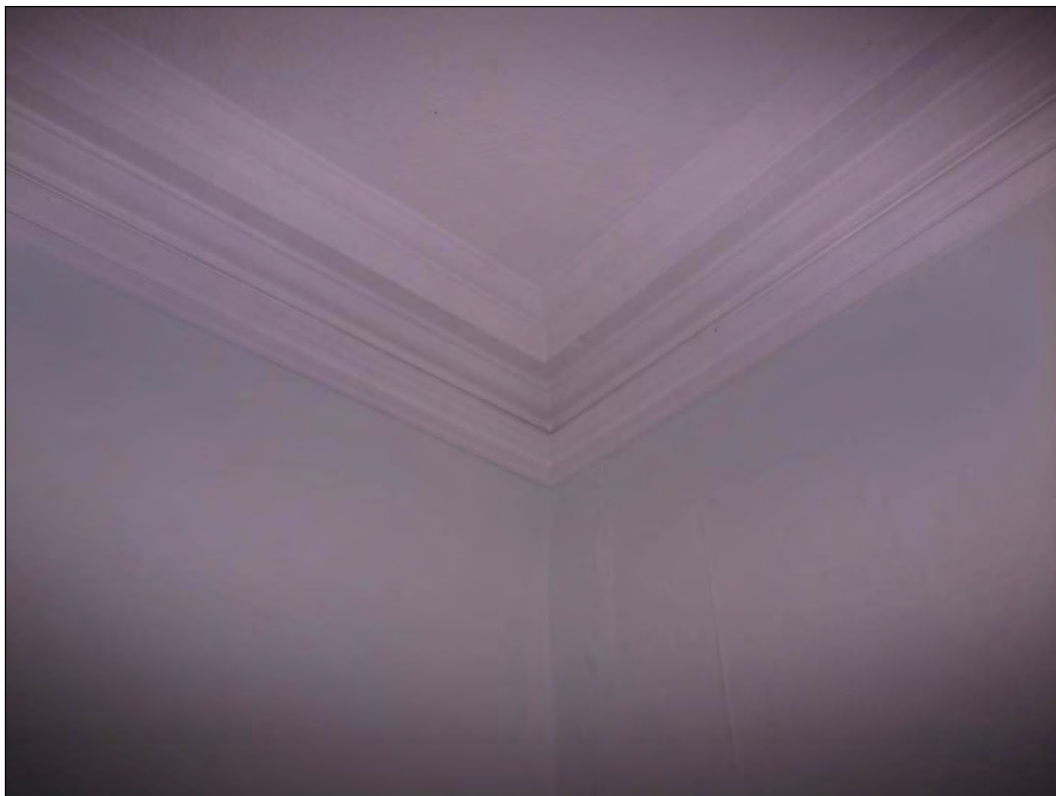
Photo 45: First floor, Landing 1, cornice detail, facing south-east (7195-0045)
