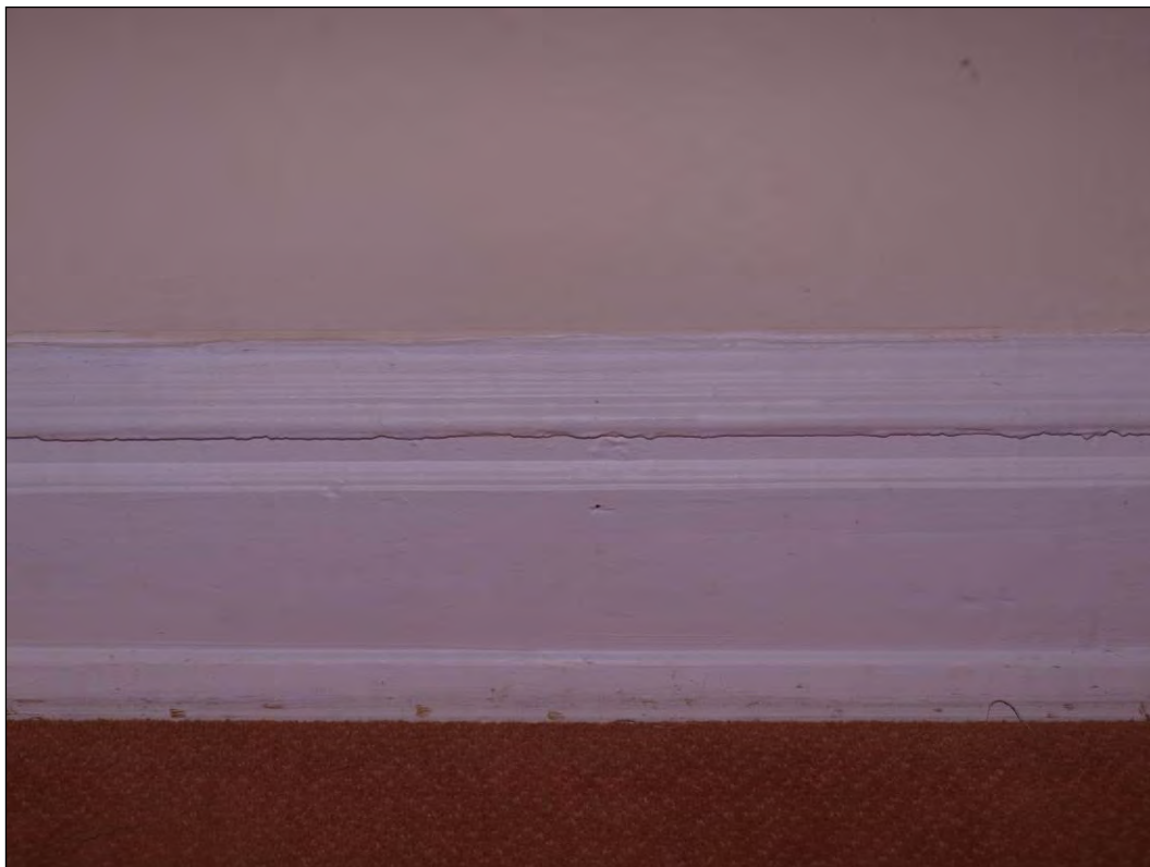
Photo 67: First floor, Room 3, skirting board detail, facing west (7195-0067)
