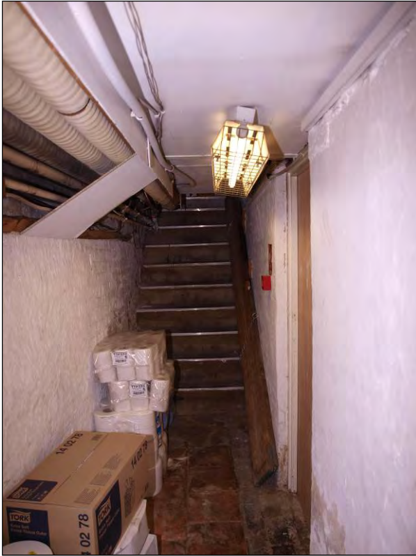
Photo 103: Basement, staircase leading to ground floor, facing north (7195-0103)
