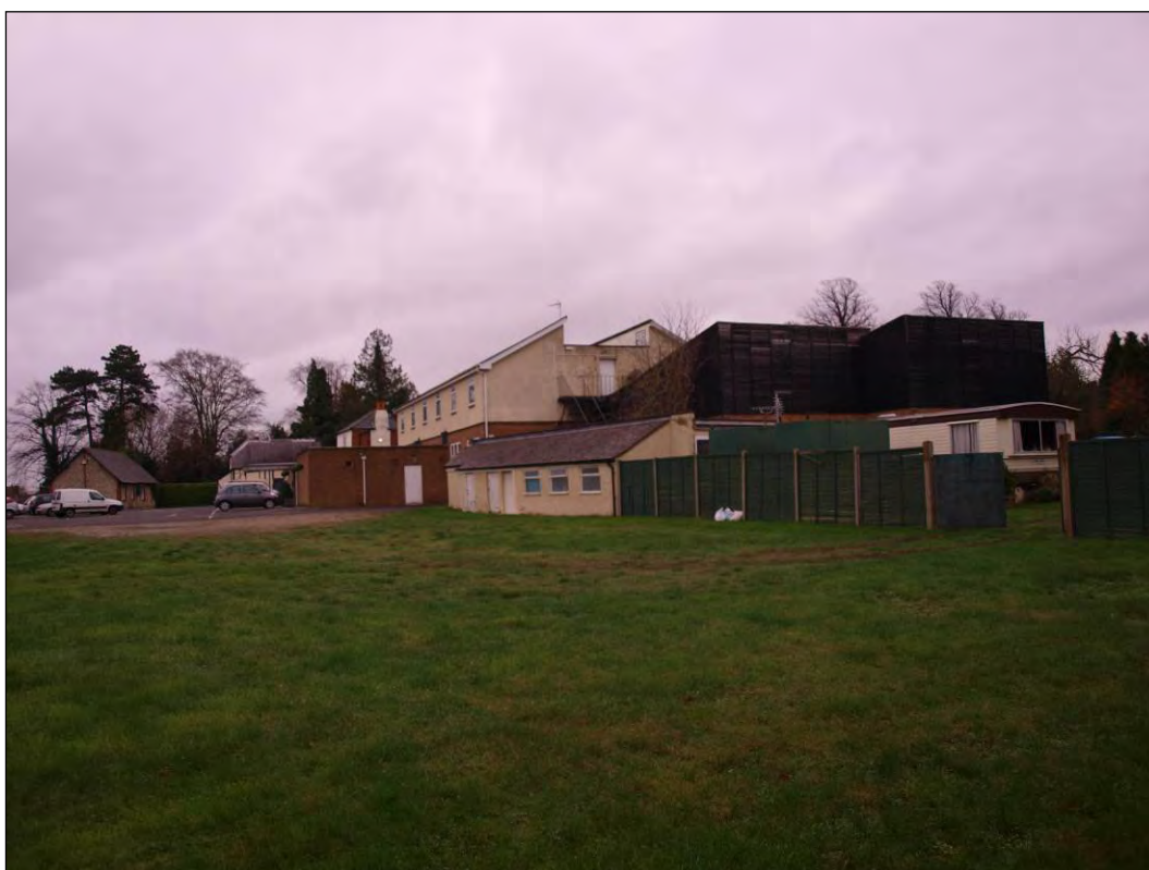
Photo 112: View of the hotel, facing south-east (7195-0112)
