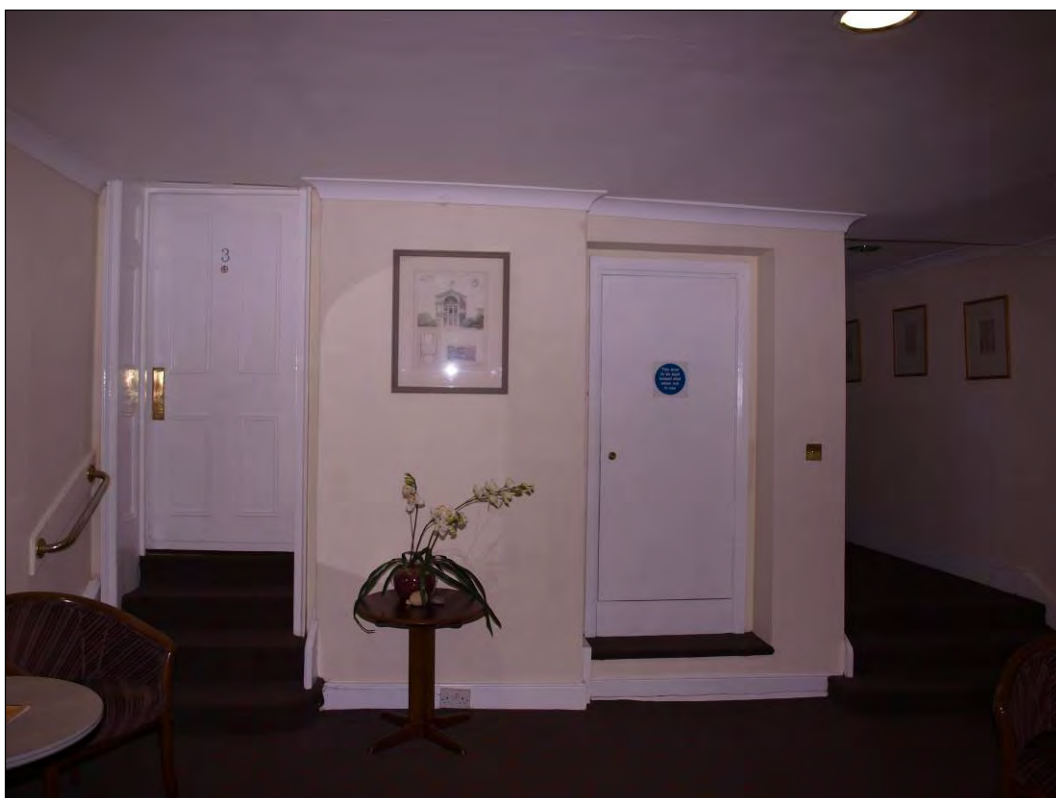
Photo 62: First floor, main circulation area leading from the landing, facing west (7195-0062)
