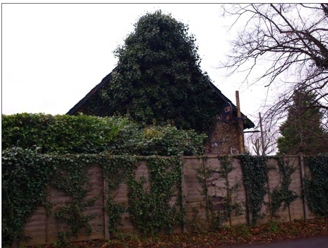
Photo 130: Outbuilding 2 (Elevation 13) view from Rectory Lane, facing west (7195-0130)
