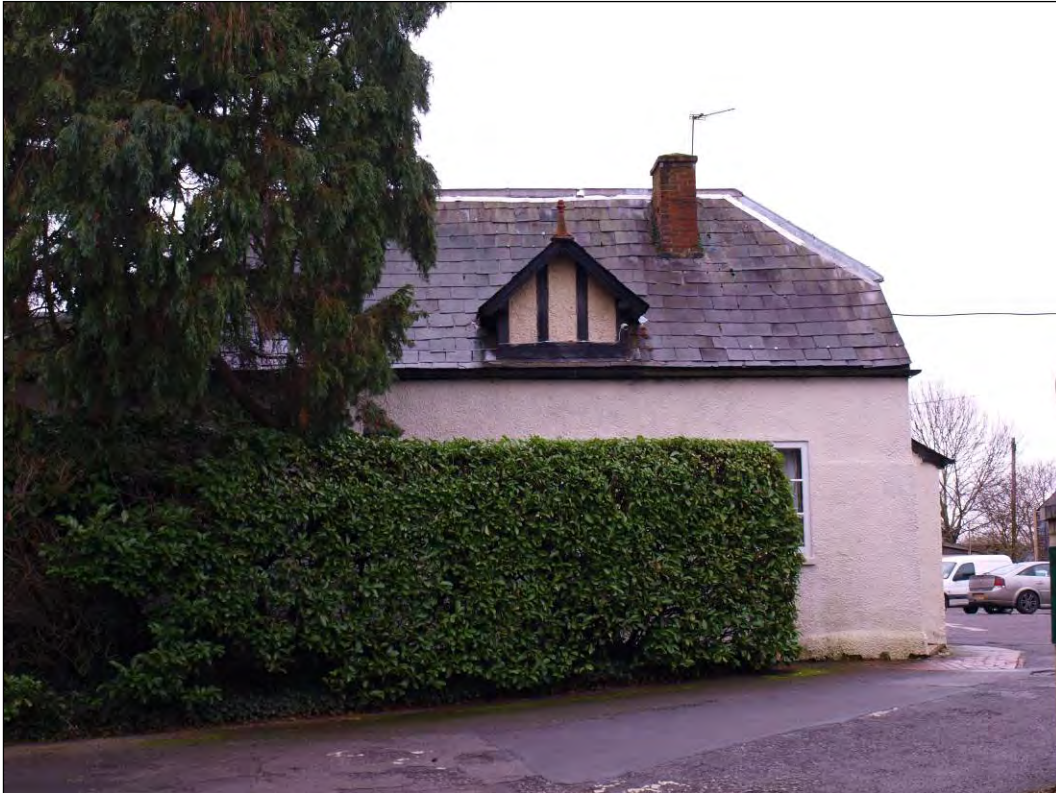
Photo 131: Outbuilding 1 (Elevation 8) view from Rectory Lane, facing west (7195-0131)
