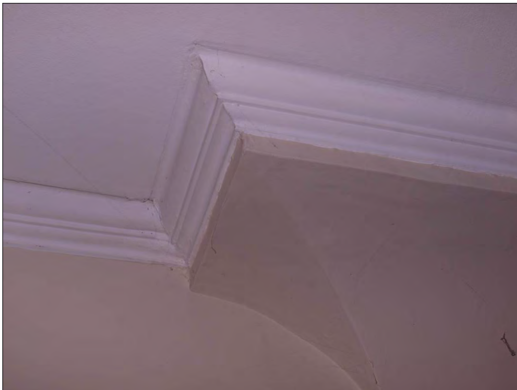
Photo 15: Ground floor, Dining Room, cornice detail, facing south-west (7195-0015)
