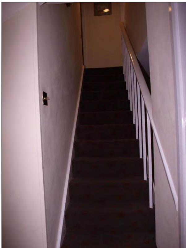
Photo 77: First floor, northern stair, taken from Landing 2 (up), facing south (7195-0077)
