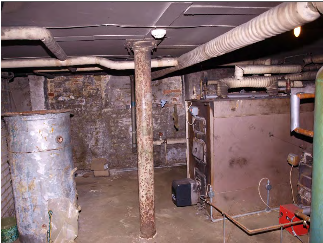
Photo 98: Basement, Boiler Room, facing south (7195-0098)
