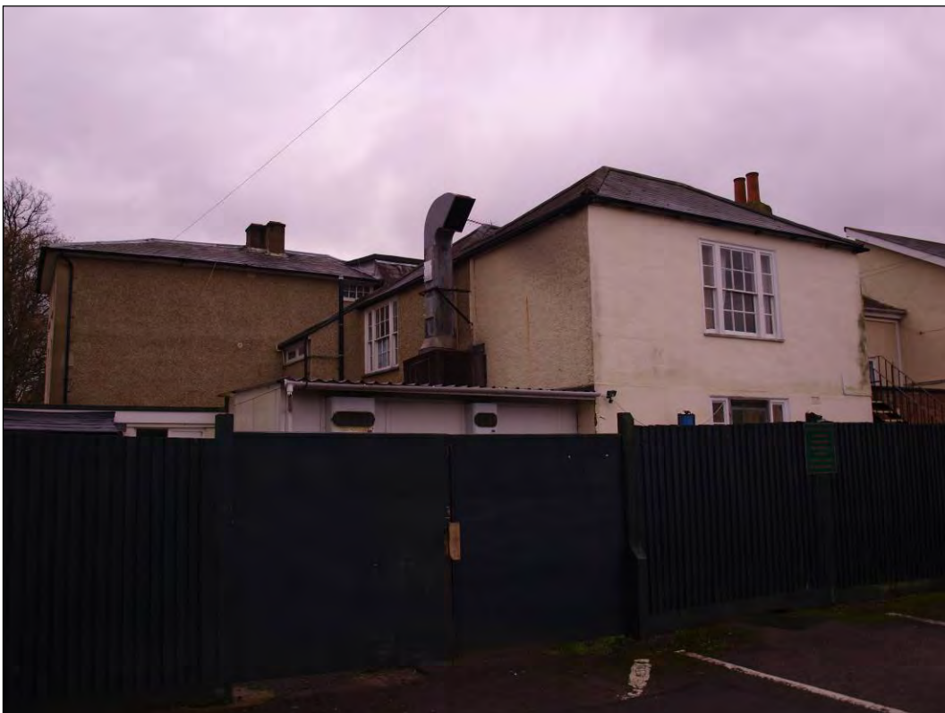
Photo 116: North elevation (Elevation 5), facing south-west (7195-0116)
