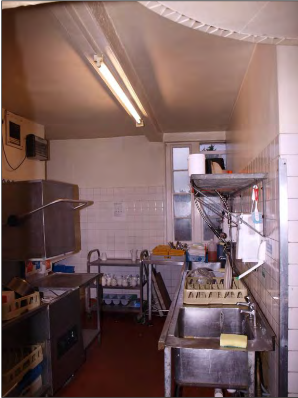
Photo 3: Ground floor, Kitchen 2, wash facilities, facing north (7195-0003)
