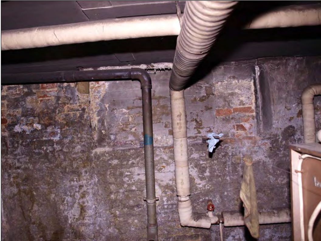
Photo 101: Basement, Boiler Room, brickwork detail, facing south (7195-0101)
