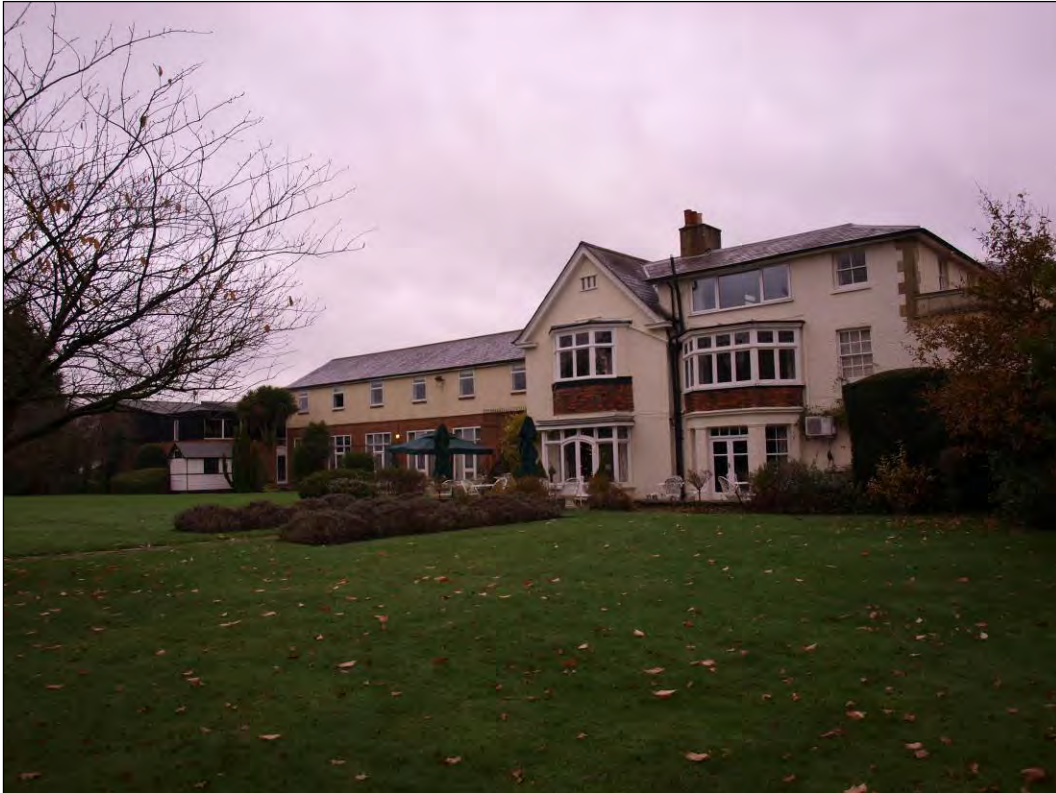
Photo 107: South elevation (Elevation 2), showing Function Suite, facing north-west (7195-0107)
