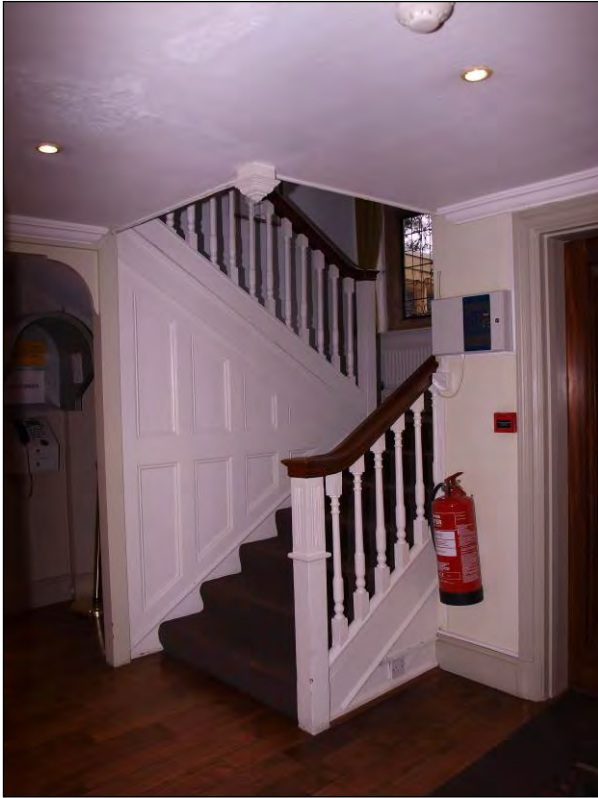
Photo 35: Ground floor, Entrance Lobby, staircase detail, facing north-east (7195-0035)
