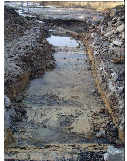
Trench 2, looking South West
