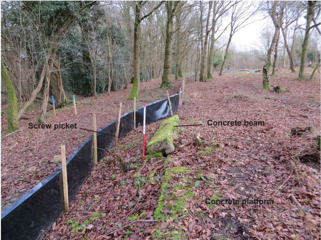
Site 22, concrete footing, concrete beam and screw picket, looking east
