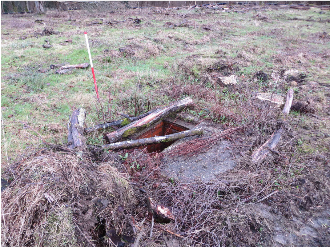
Site 16, inspection chamber at western end of hut platform
