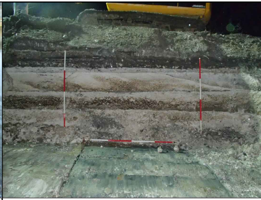
Completed stabilised riverbank
