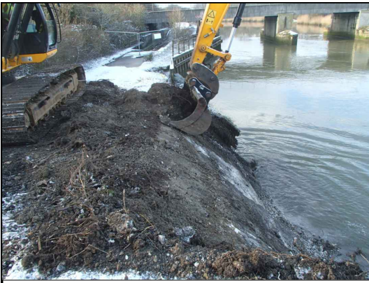
Machine excavation along riverbank
