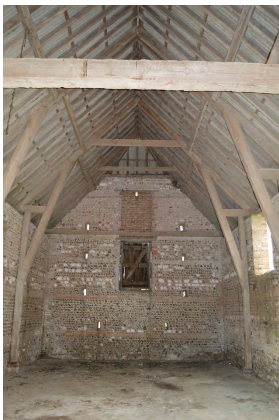
Plate 20: New Barn, interior view of roof construction, facing west (7251_0020)
