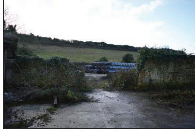
7251-0014 New Barn, external view of opening on southern yard wall. Facing south
