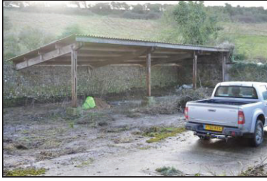
7251-0013 New Barn, external view of Shelter 2. Facing southeast
