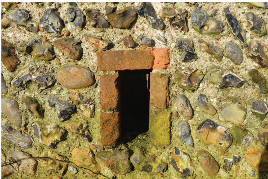
Plate 1: New Barn, detail of a ventilation hole on the east elevation, facing west (7251_0004)
