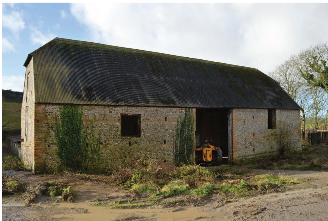
Plate 2: New Barn, view of north elevation, facing south-west (7251_0001)
