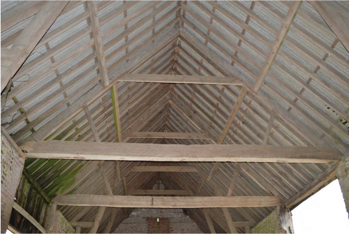
Plate 11: New Barn, interior view of midstrey bay construction (7251_0023)
