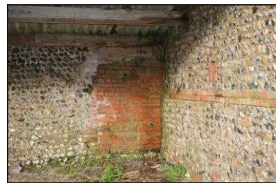
7251-0009 New Barn, detail of former doorway on west wall of southern yard. Facing west
