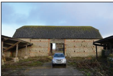
7251-0007 New Barn, external view of south elevation. Facing north
