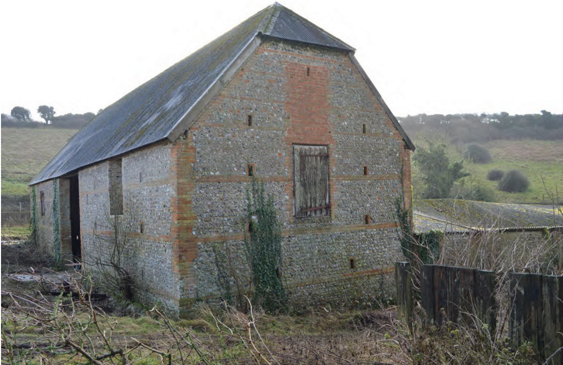
Plate 5: New Barn, view of west elevation, facing south-east (7251_0005)
