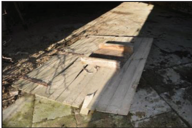
7251-0019 New Barn, detail of modern timber doorway (now detached). Facing west
