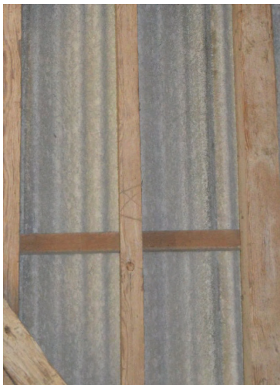
Plate 22: New Barn, detail of Baltic marks on rafters, facing south (7251_0043)
