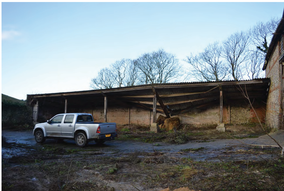
Plate 27: View of Shelter 1 within the main yard, facing west (7251_0012)
