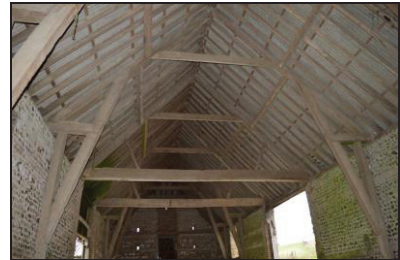
7251-0021 New Barn, interior detail of roof construction over midstreys. Facing west
