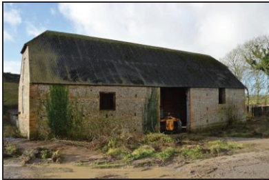
7251-0001 New Barn, external view of north elevation. Facing southwest
