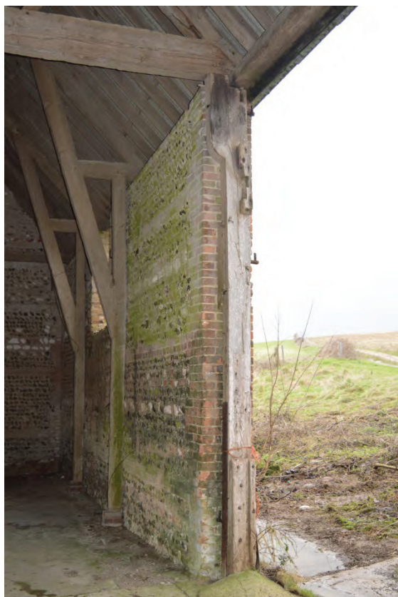
Plate 17: New Barn, detail of northern post of Truss 5, facing north-west (7251_0032)
