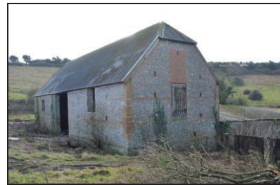
7251-0006 New Barn, external view of north-west corner. Facing southeast
