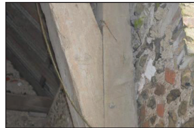
New Barn, detail of 'leap-board' on door post. Facing northwest
