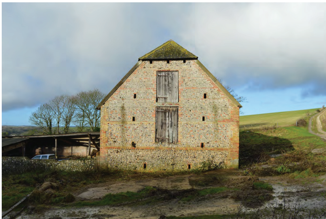
Plate 4: New Barn, view of east elevation, facing west (7251_0003)
