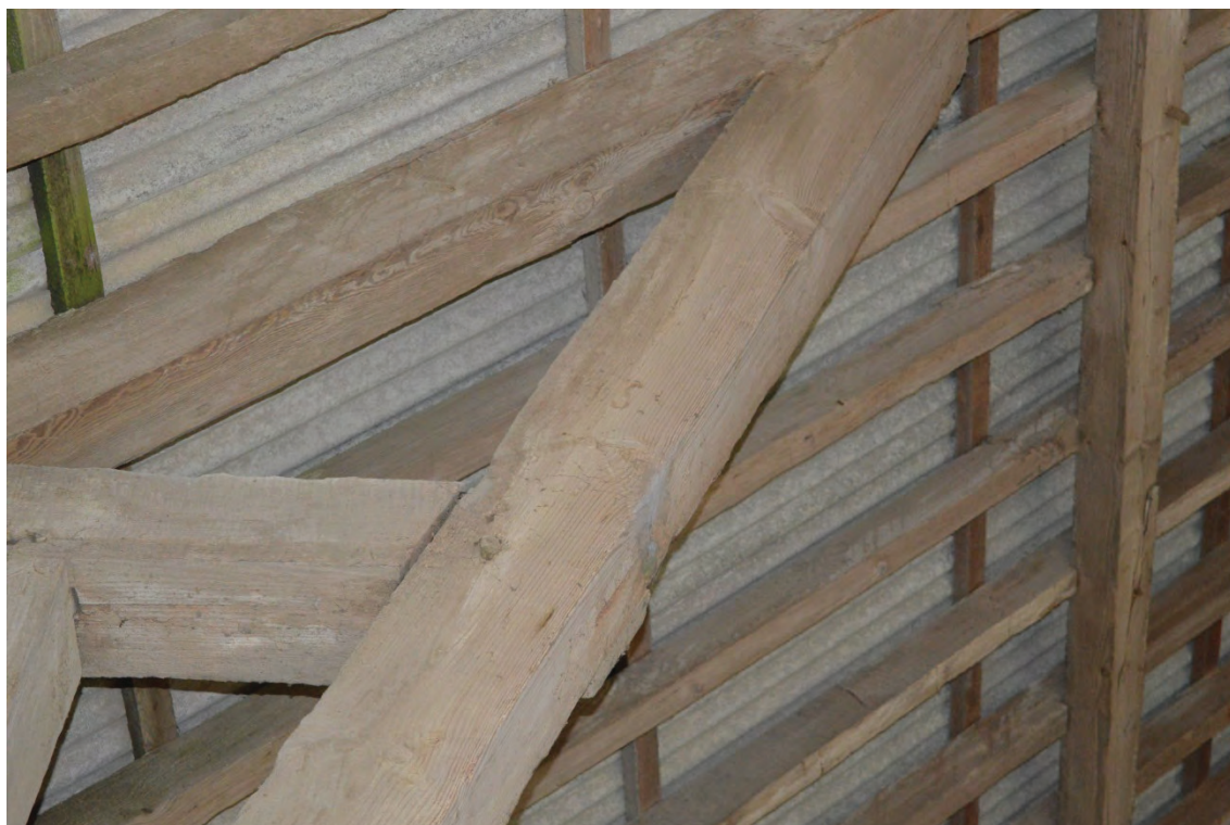
Plate 16: New Barn, detail of 'J.S.' inscription to south end of Truss 6, facing west (7251_0038)
