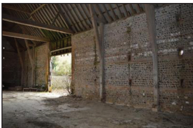
7251-0025 New Barn, interior view of south elevation. Facing southeast
