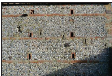
7251-0011 New Barn, detail of redundant sockets to the eastern side of southern elevation. Facing north
