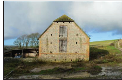
7251-0003 New Barn, external view of east elevation. Facing west
