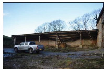
7251-0012 New Barn, external view of Shelter 1. Facing west
