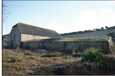
7251-0017 New Barn, external view of the sites western elevation. Facing northeast
