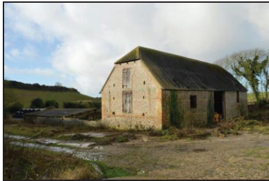
7251-0002 New Barn, external view of north-east corner. Facing southwest
