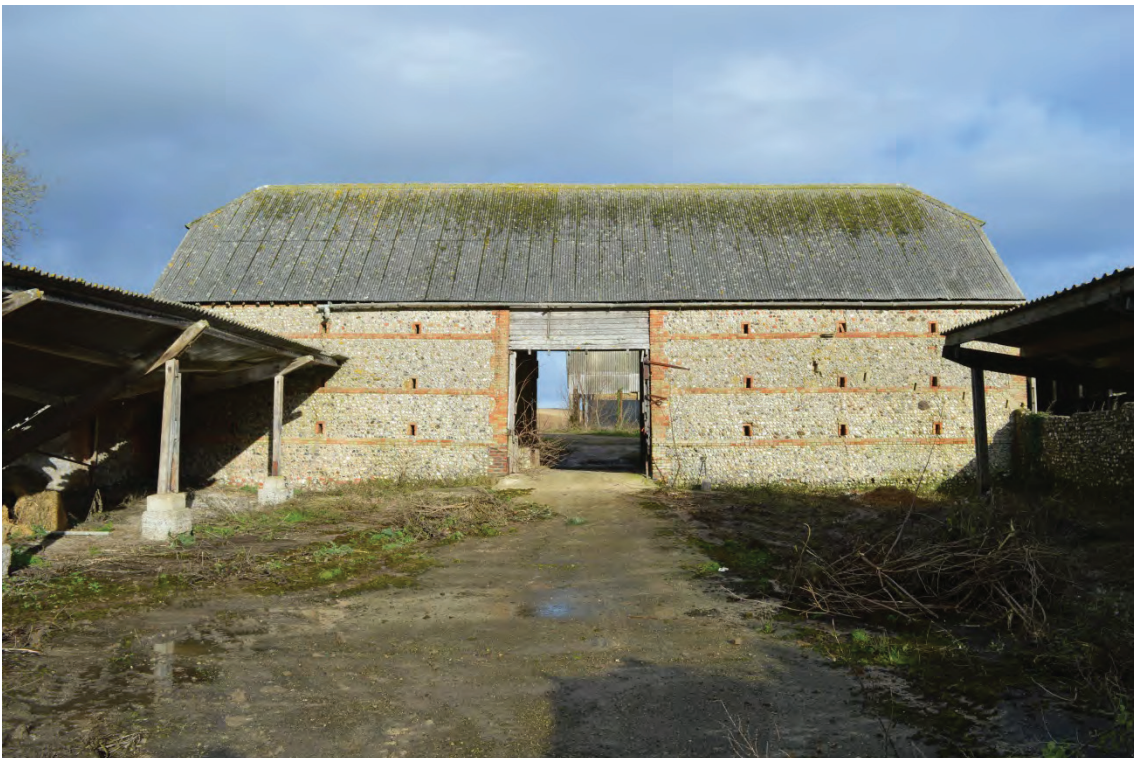
Plate 6: New Barn, view of south elevation, facing north (7251_0048)
