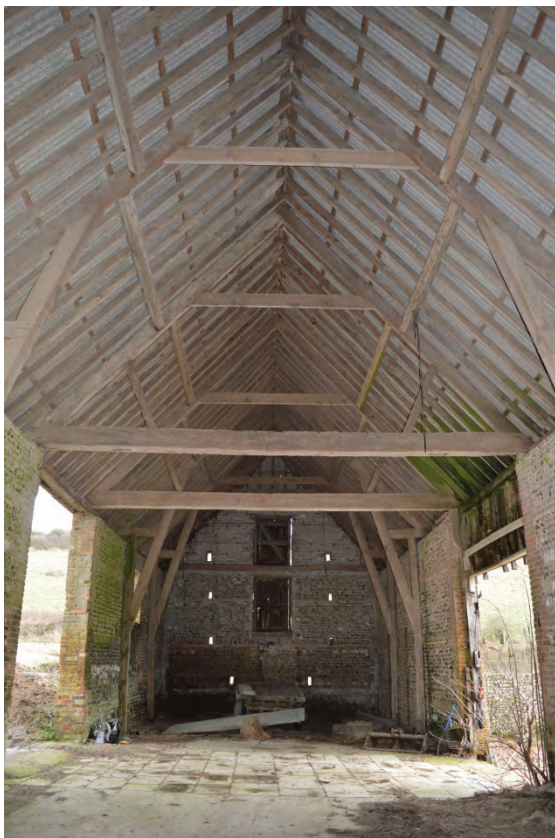
Plate 10: New Barn, view of internal timber frame construction, facing east (7251_0024)
