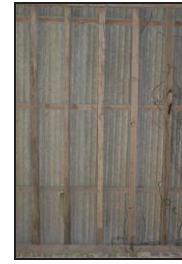
New Barn, detail of staining on rafters from former thatched roof. Facing north
