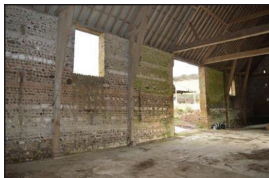
7251-0026 New Barn, interior view of north elevation. Facing northeast
