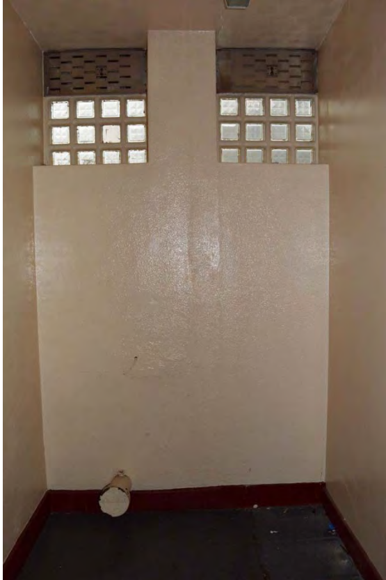
Plate 53: Magistrates court, view of Room B6 cell in western range (7338_173)
