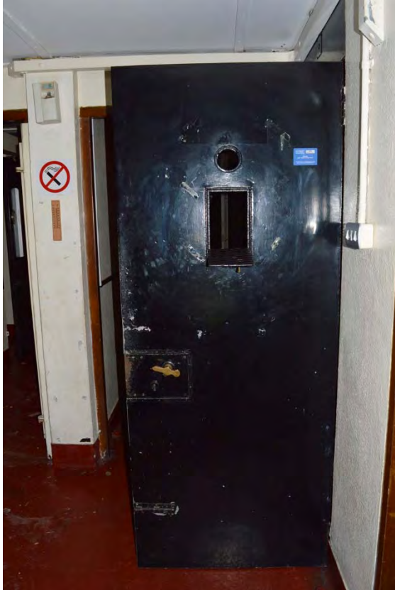
Plate 49: Magistrates court, detail of original cell door in western range (7338_171)
