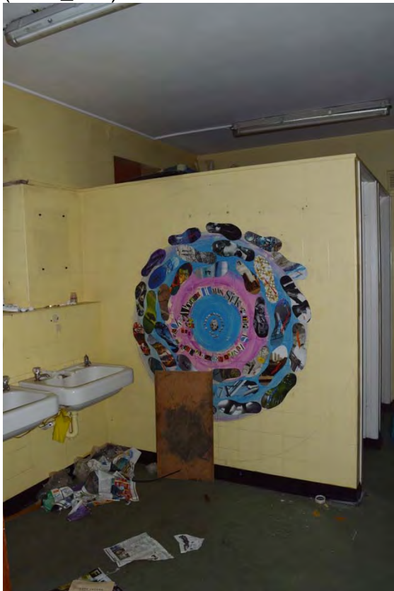
Plate 84: Police station, view of bathroom facilities at first floor level (7338_220)
