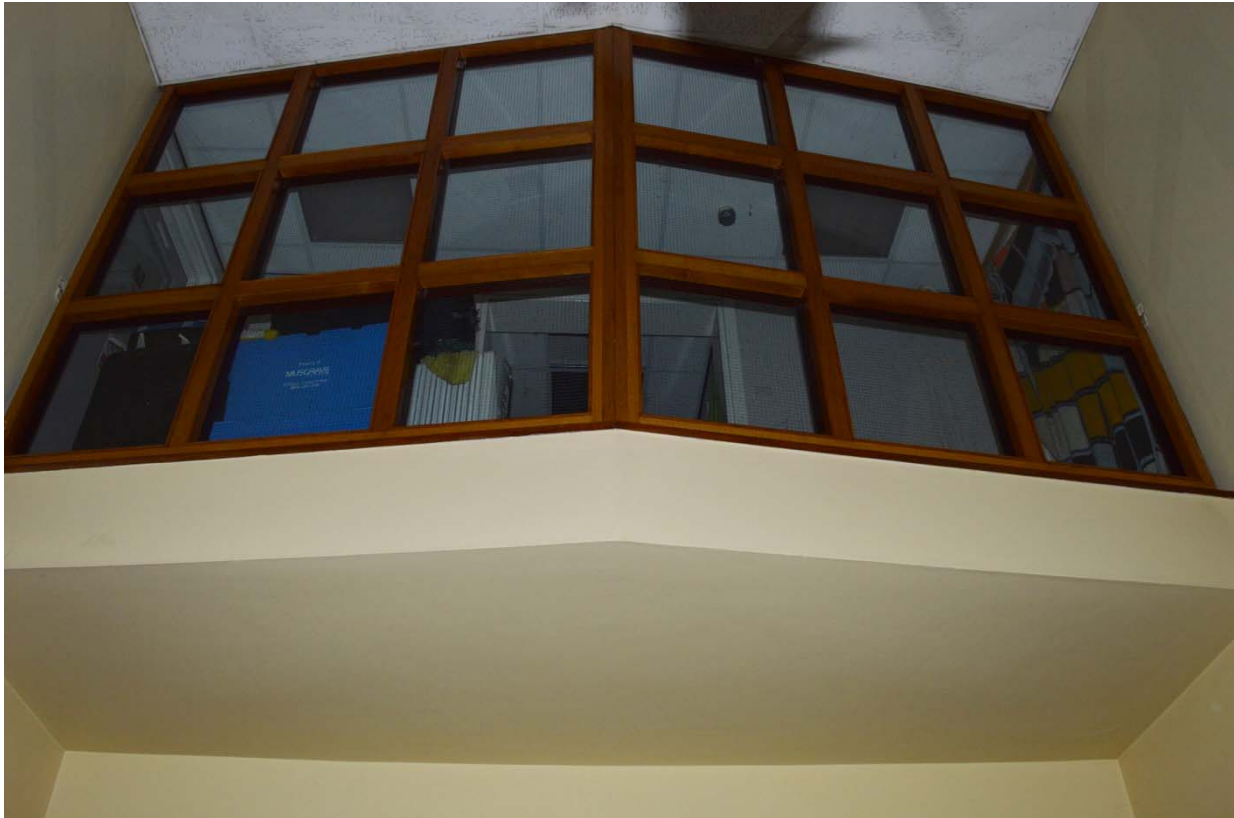
Plate 81: Police station, view of north lobby first floor mezzanine (7338_225)
