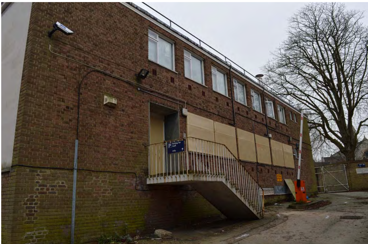
Plate 2: Magistrates court, external view of north elevation (7338_117)
