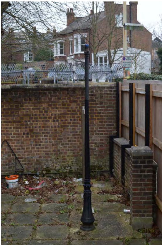
Plate 74: Police station, external view of police lamp-post to the north site boundary (7338_138)
