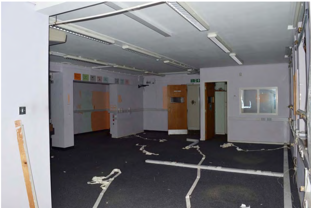
Plate 12: Magistrates court, view of northern office partition within the lobby (7338_084)
