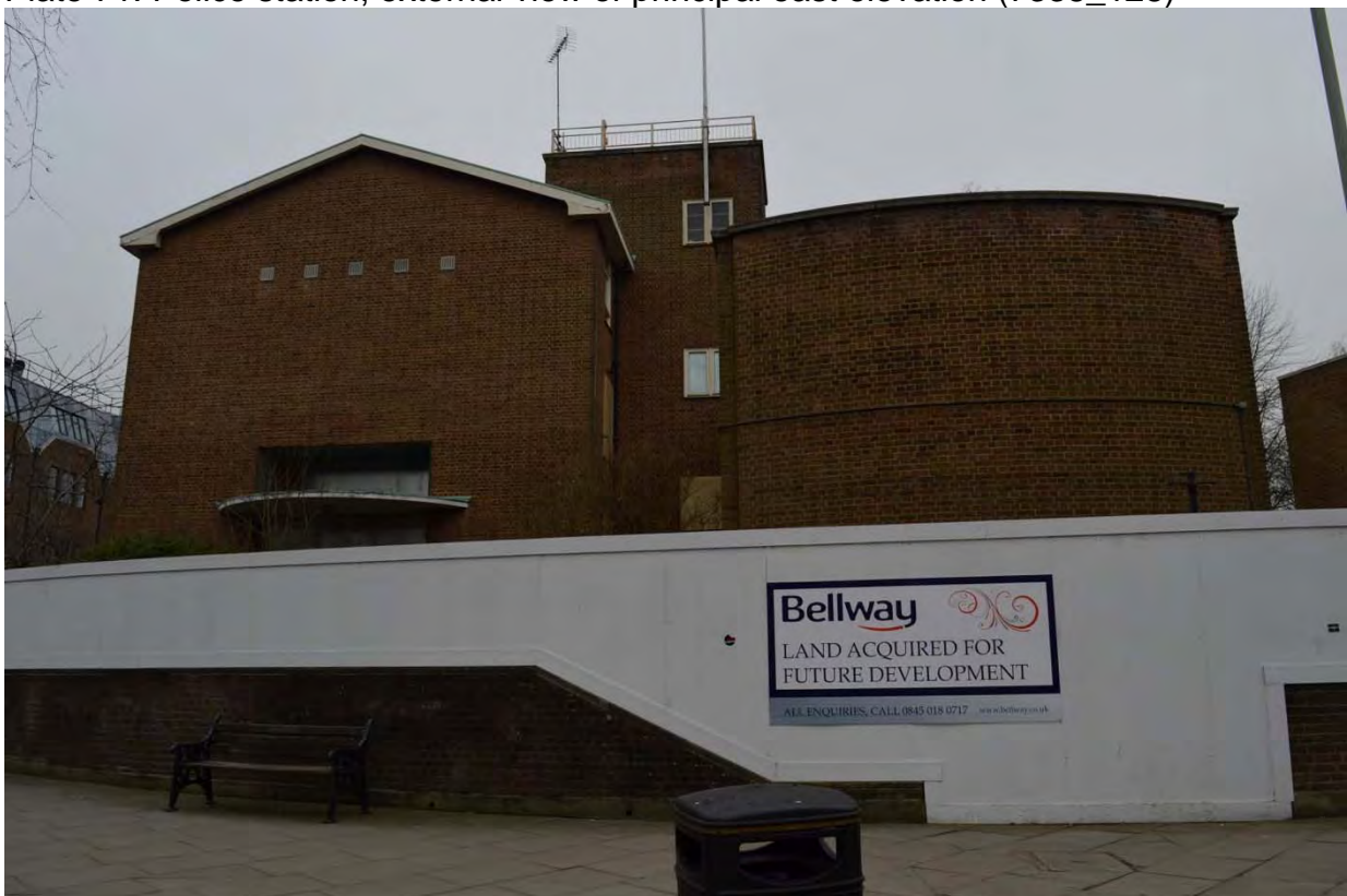
Plate 72: Police station, external view of north elevation (7338_129)
