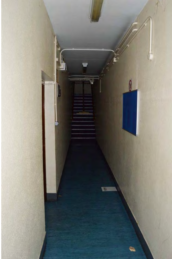
Plate 45: Magistrates court, view of basement passage (7338_161)
