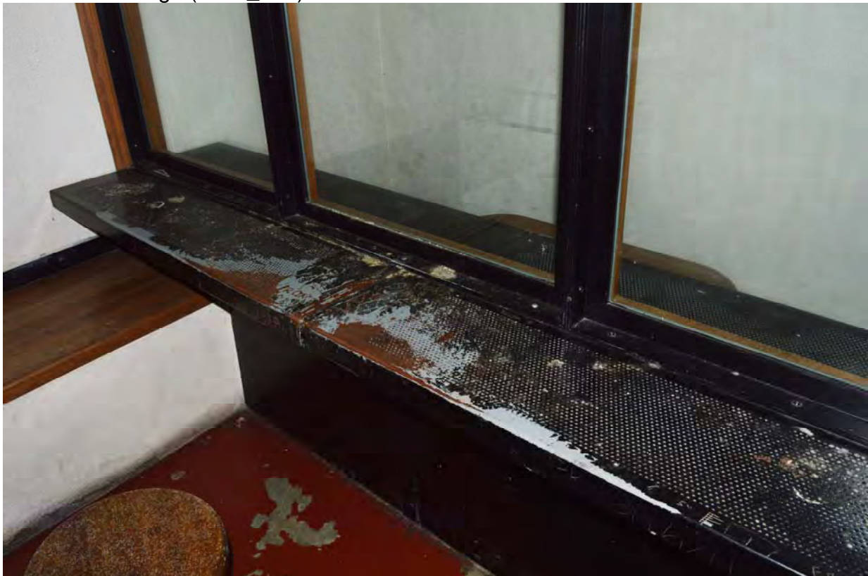
Plate 58: Magistrates court, detail of worn surfaces within the detainee side of the interview/consultation room of the western range (7338_190)
