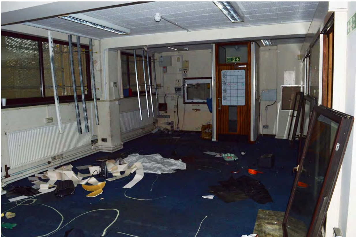
Plate 92: Telfer House, view of ground floor principal office (7338_017)
