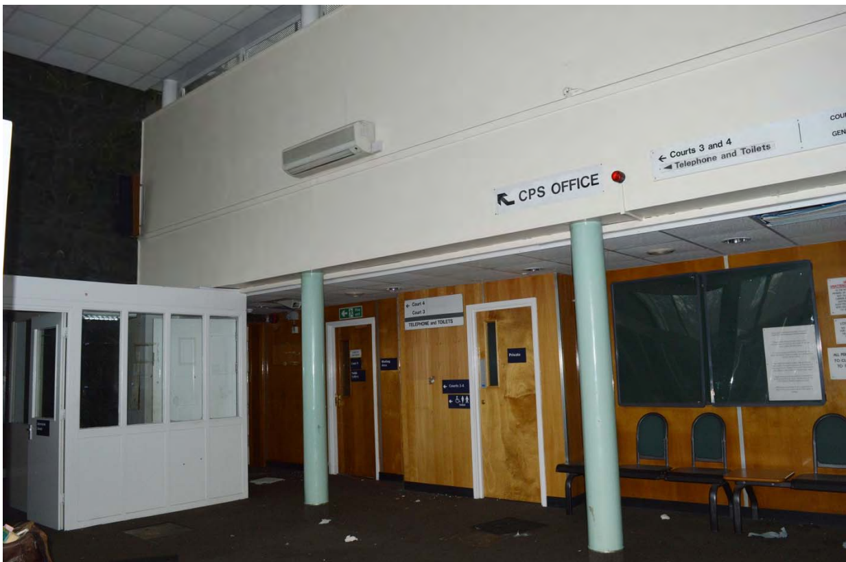
Plate 8: Magistrates court, view of portico to western side of lobby (7338_077)
