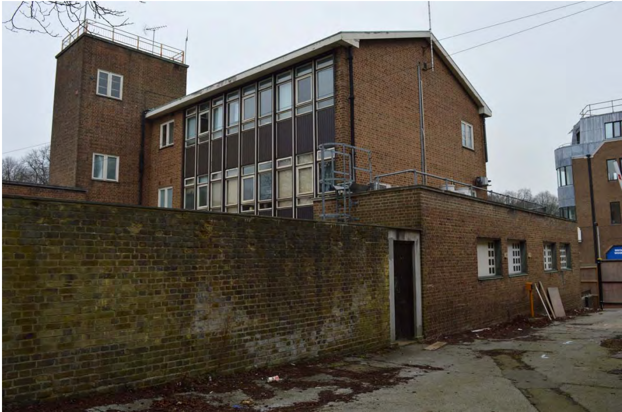
Plate 79: Police station, external view of south elevation (7338_126)
