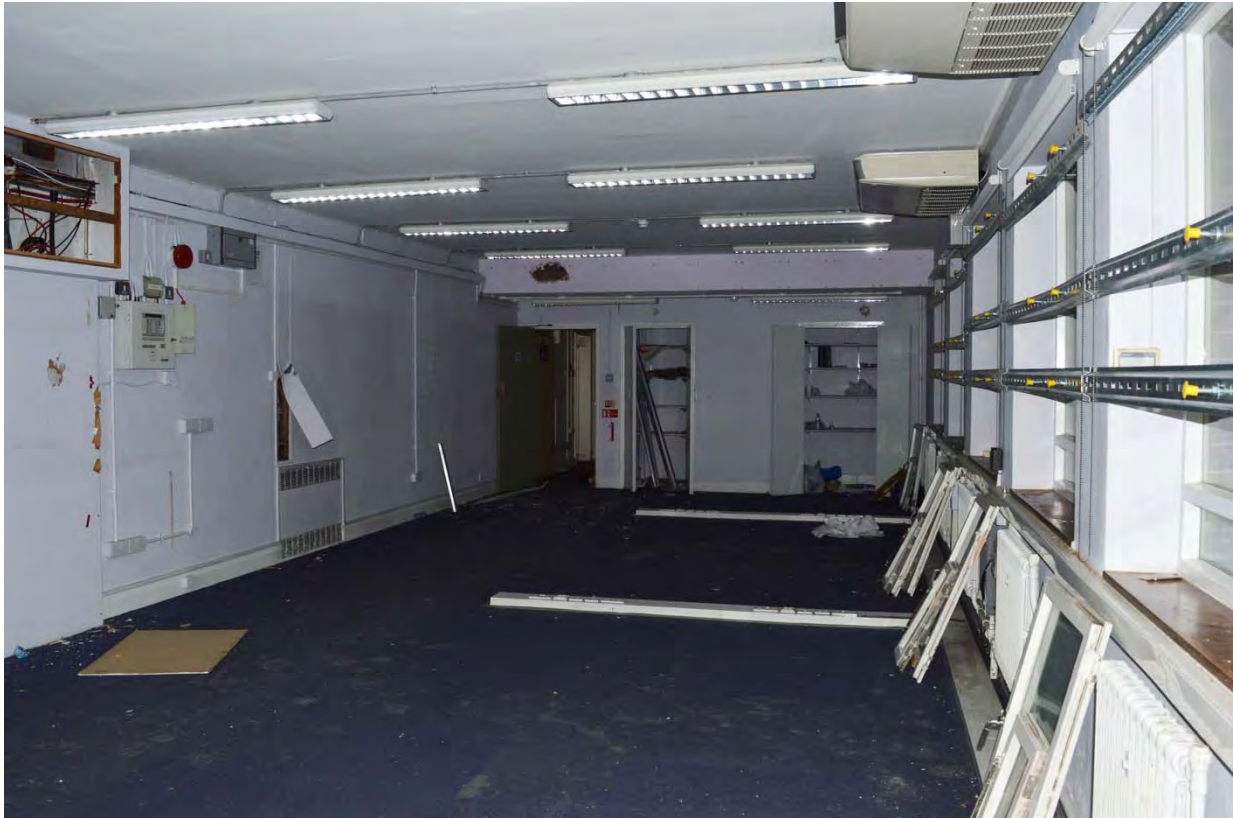
Plate 27: Magistrates court, view of southern range office at ground floor level (7338_032)
