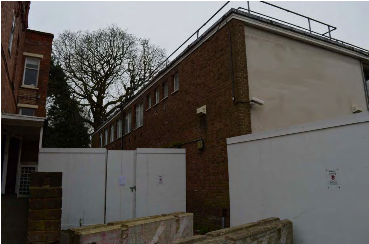
Plate 3: Magistrates court, external view of south elevation (7338_123)
