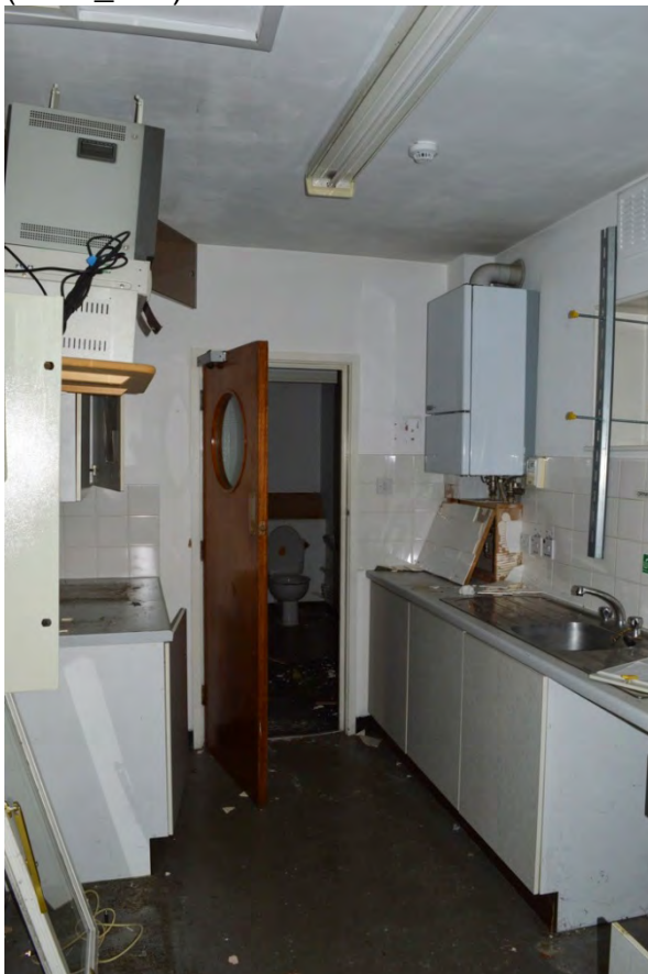
Plate 40: Magistrates court, view of kitchen in western range (7338_102)
