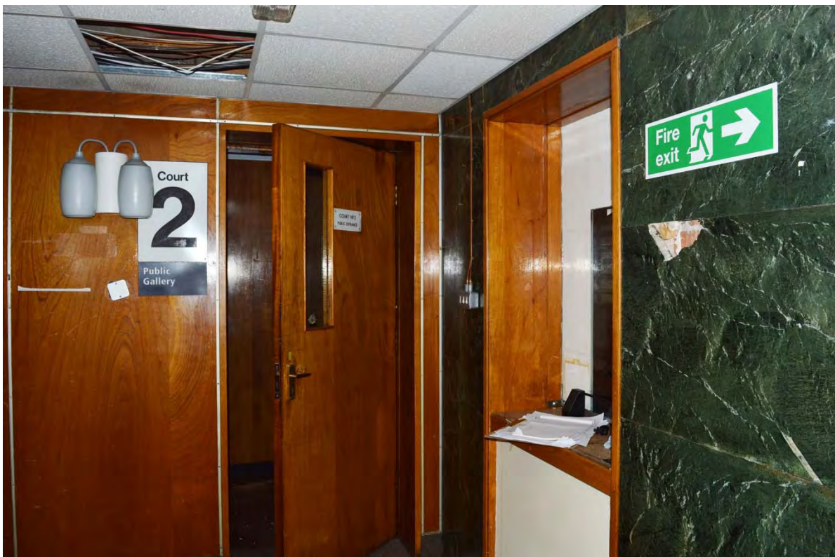
Plate 26: Magistrates court, view of public entrance to Courtroom 2 (7338_039)
