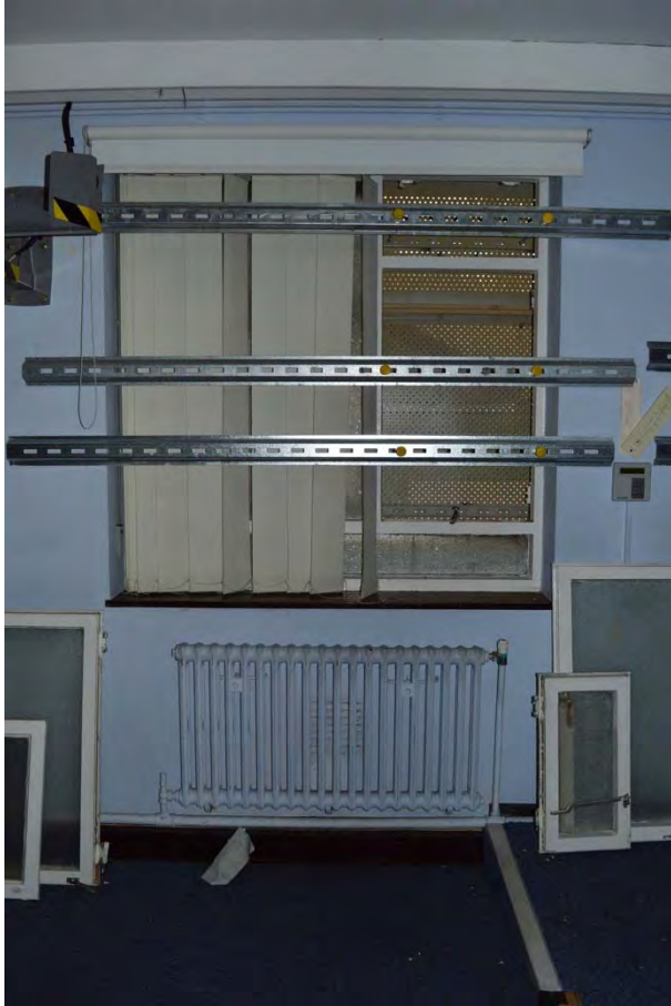
Plate 25: Magistrates court, detail of Courtroom 3 window and radiator (7338_066)
