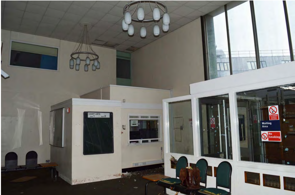
Plate 9: Magistrates court, view of office and reception addition to lobby (7338_074)
