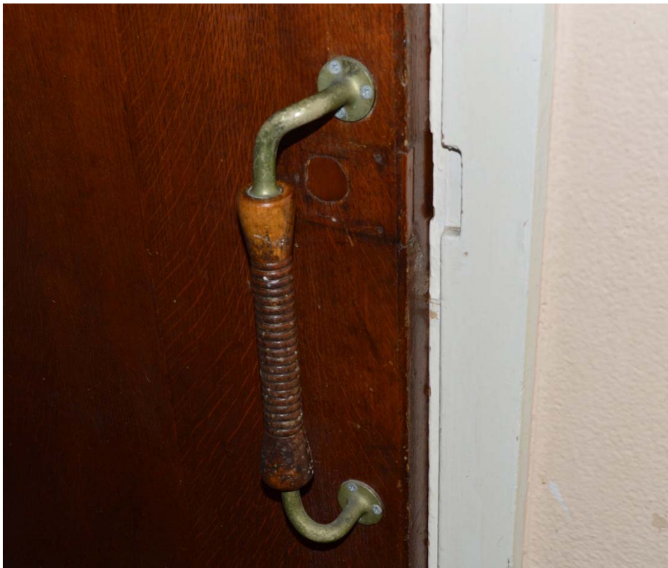
Plate 88: Police station, detail of early handle fitting (7338_228)
