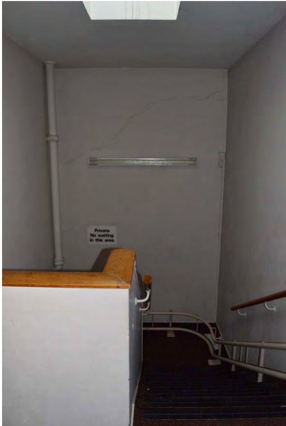
Plate 63: Magistrates court, detail of south-west stairwell at first floor level (7338_146)
