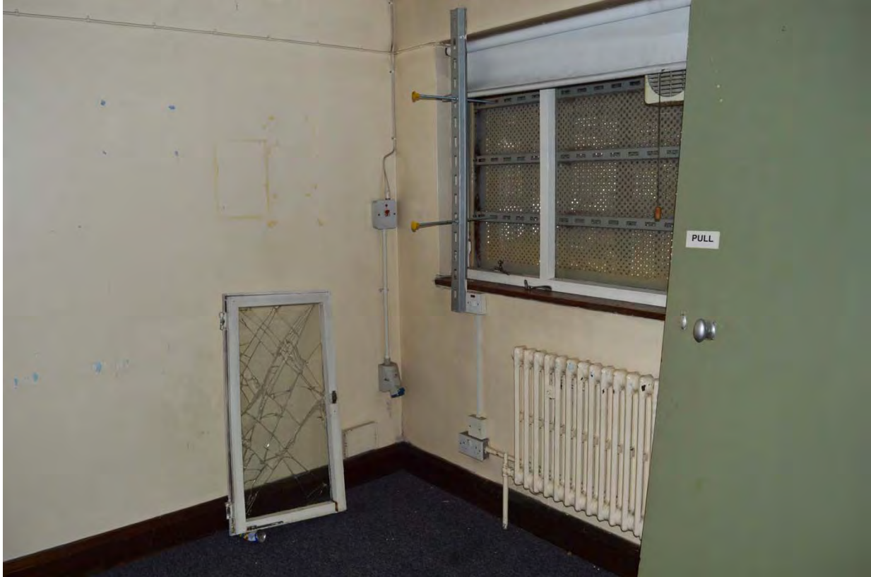
Plate 29: Magistrates court, view of security office (7338_036)
