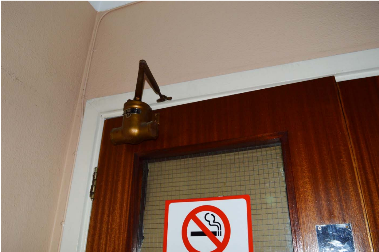
Plate 89: Police station, detail of early door closer fitting (7338_221)
