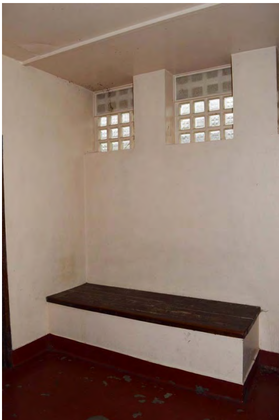
Plate 54: Magistrates court, view of Room B7 cell in western range (7338_177)
