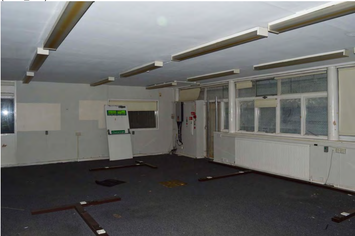
Plate 66: Magistrates court, view of northern first floor mezzanine office space (7338_151)
