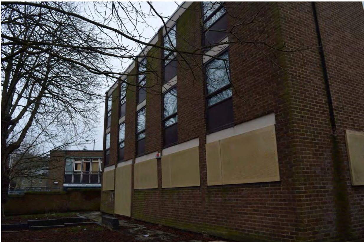
Plate 90: Telfer House, external view of principal north elevation (7338_029)
