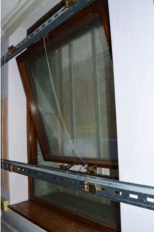
Plate 13: Magistrates court, view of window detail within lobby's east elevation (7338_087)
