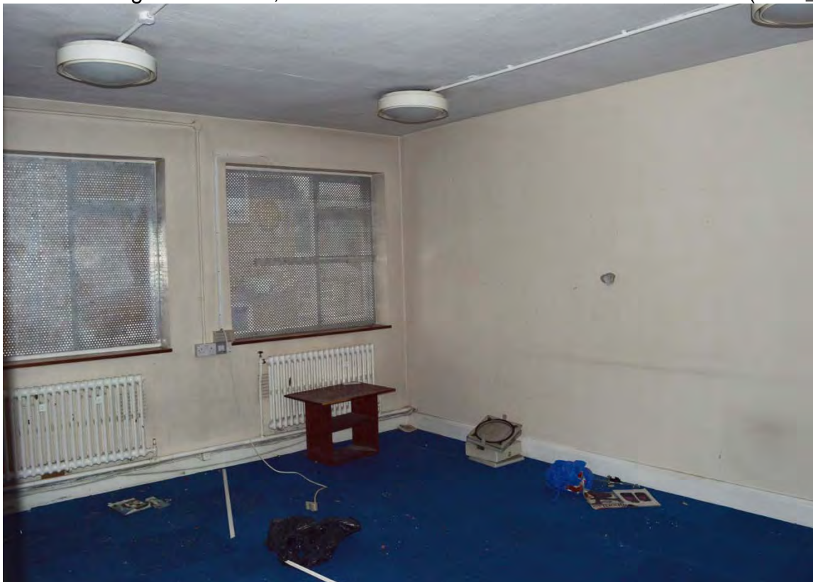
Plate 64: Magistrates court, view of northern range office on the first floor (7338_142)
