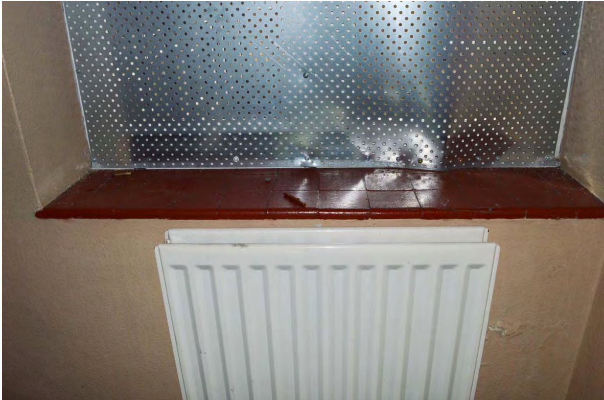
Plate 87: Police station, detail of early tile window sill within the first floor stairwell (7338_254)
