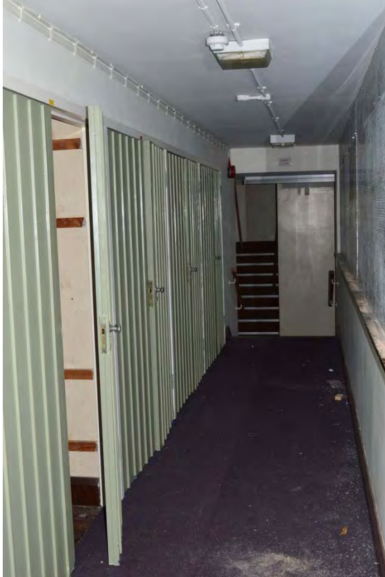
Plate 31: Magistrates court, view of corridor to the west of the courtrooms (7338_094)
