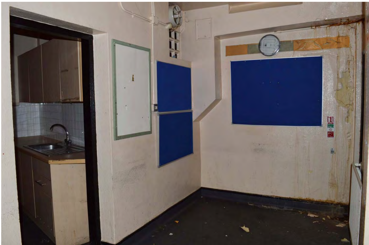
Plate 46: Magistrates court, view of Room B2 office in western range (7338_165)
