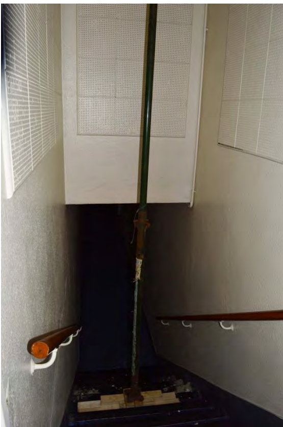
Plate 44: Magistrates court, view of basement stairwell to the rear of the custody dock in Courtroom 1 (7338_158)
