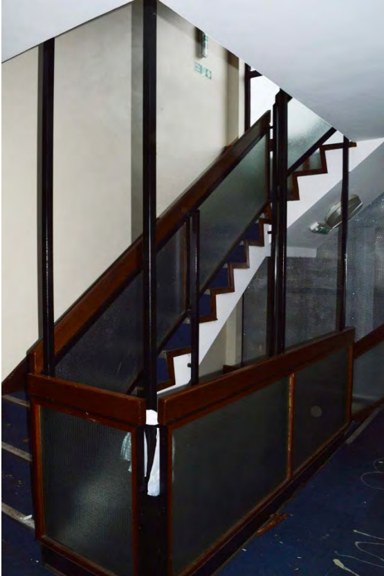
Plate 95: Telfer House, view of stairwell at first floor level (7338_008)
