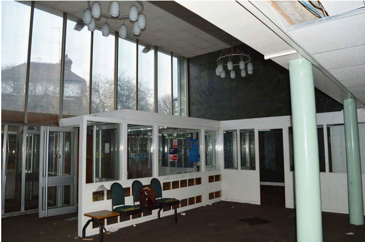
Plate 7 Magistrates court, view of principal public entrance within the lobby (7338_073)
