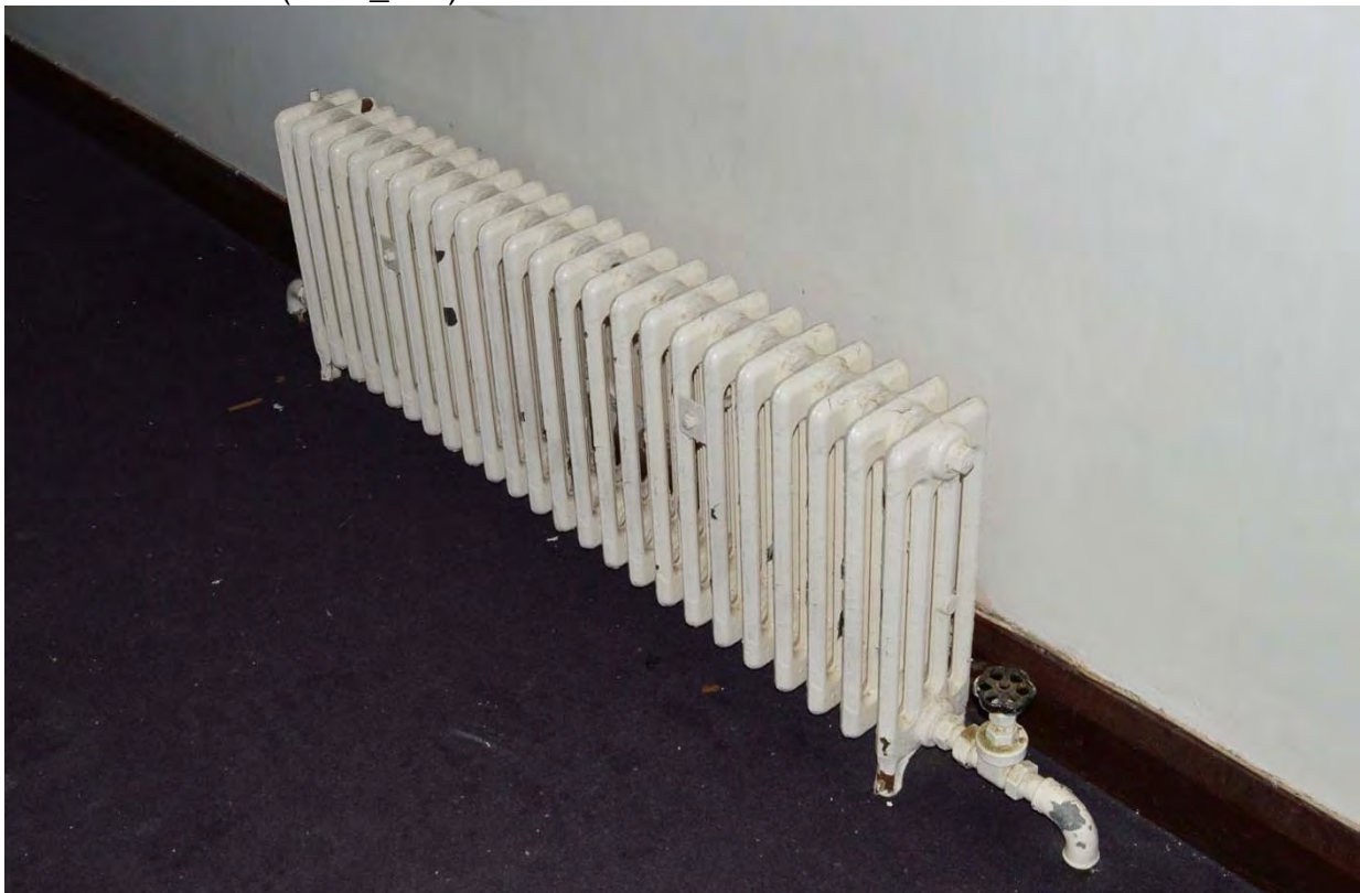
Plate 36: Magistrates court, detail of original radiator within the western range corridor (7338_097)
