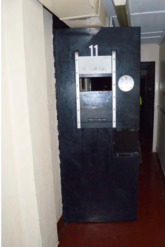
Plate 51: Magistrates court, detail of modern replacement cell door in western range (7338_183)
