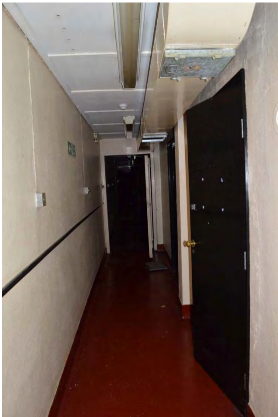
Plate 52: Magistrates court, view of northern corridor in western range (7338_172)
