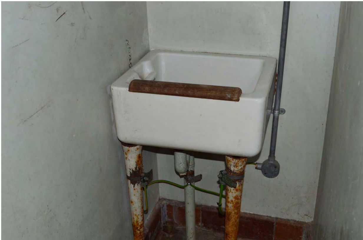
Plate 32: Magistrates court, detail of original sink within end corridor cupboard (7338_095)
