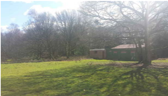
Fig. 7b Site shot facing south east. Buildings
