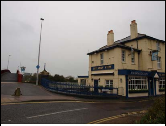
Reach 4, General Shot, looking north west
