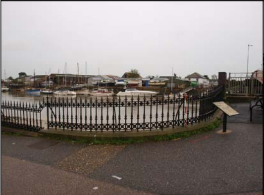
Reach 4, General Shot looking South east
