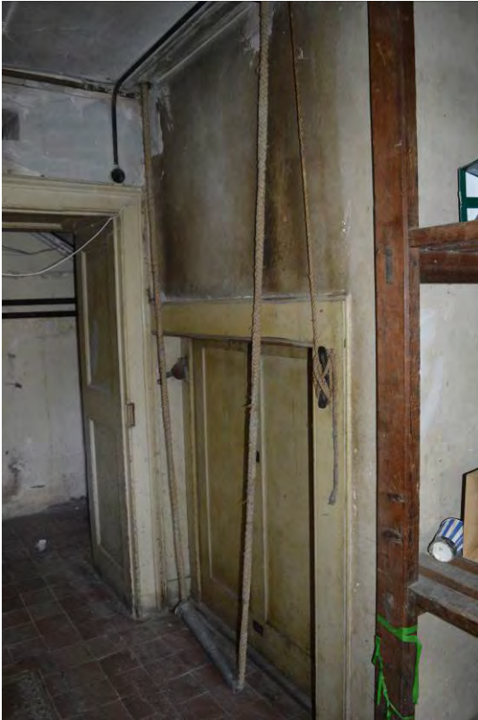
Plate 63: Dumb waiter, Room B7 (321)
