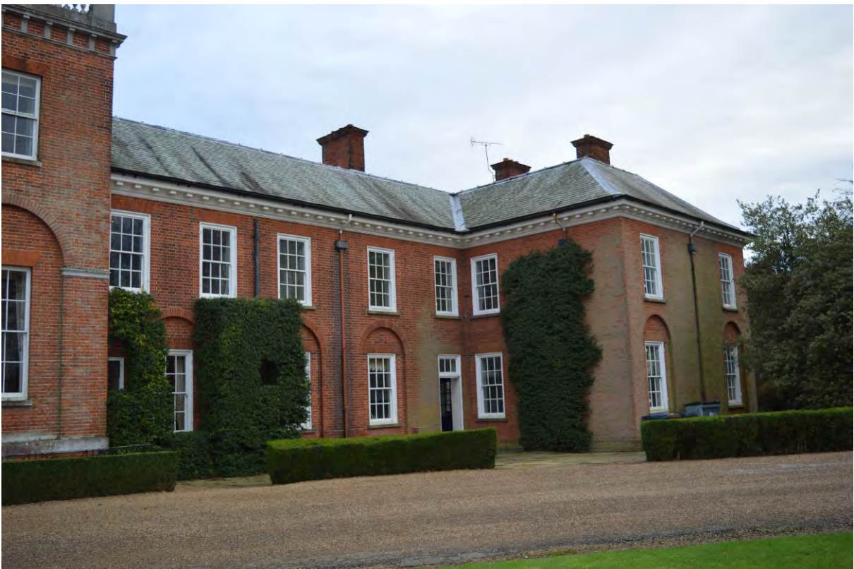
Plate 18: South range, west elevation, looking south-east (83)
