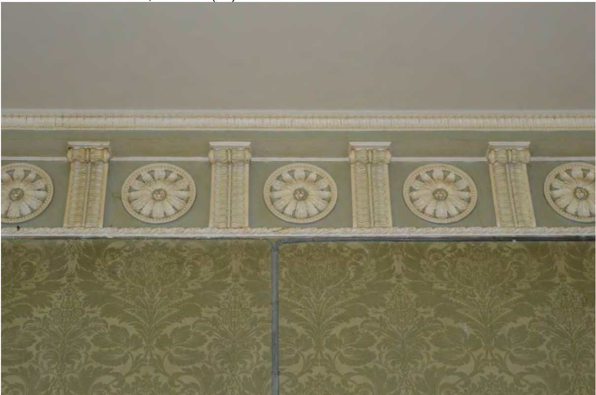
Plate 46: Detail of frieze and cornice, Room 6 (67)
