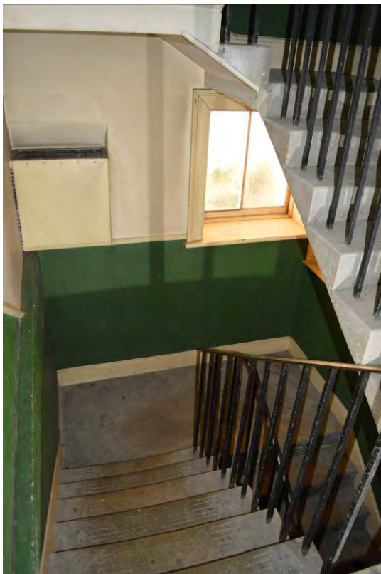
Plate 48: The service stair, and metal casing of unknown purpose (303)
