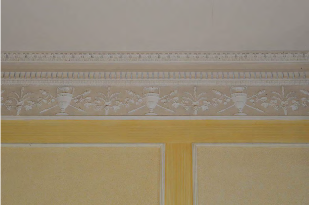
Plate 33: Detail of frieze and cornice, Room 3 (40)
