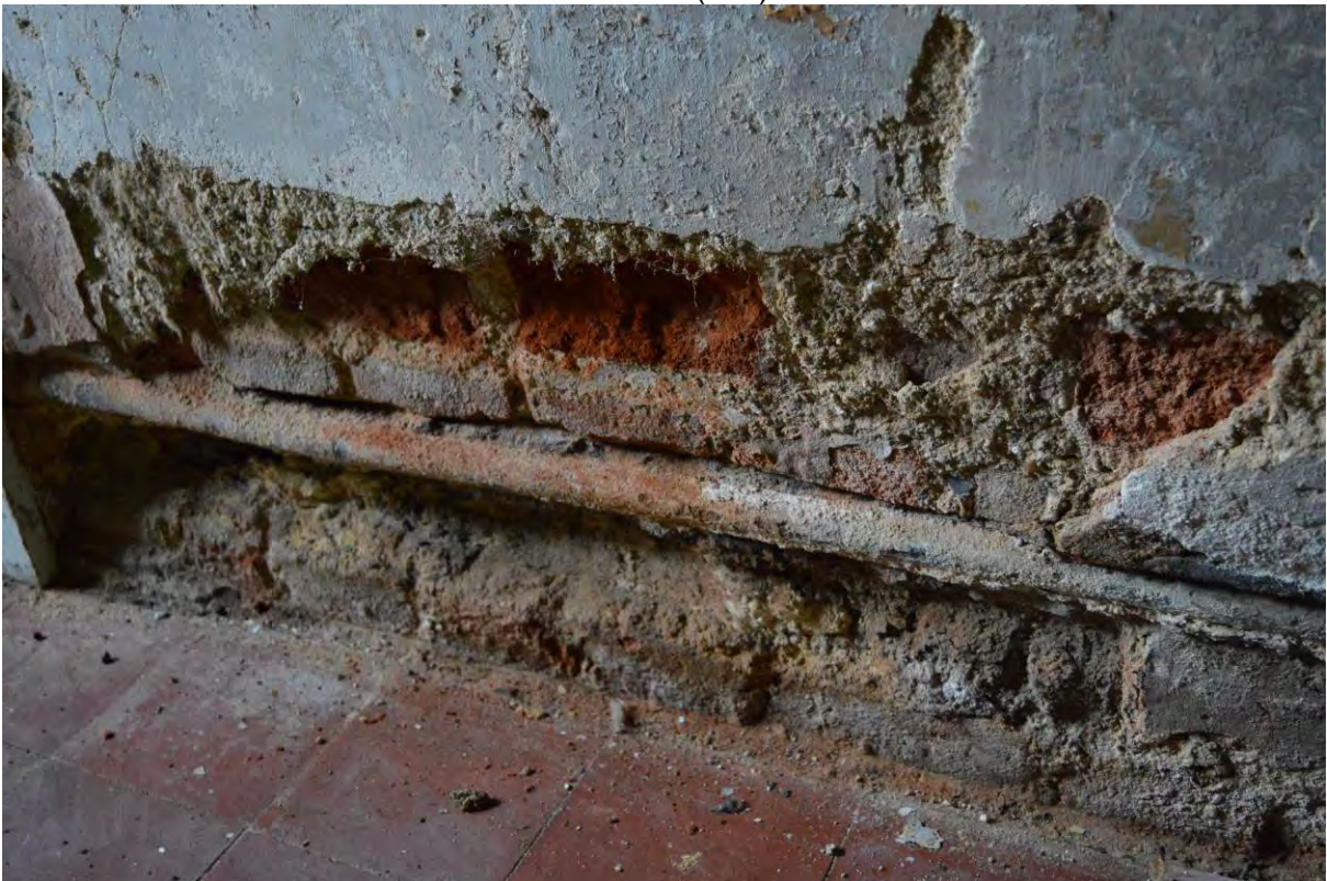
Plate 62: Construction of ovolo moulding to plaster skirting, Room B7 (320)
