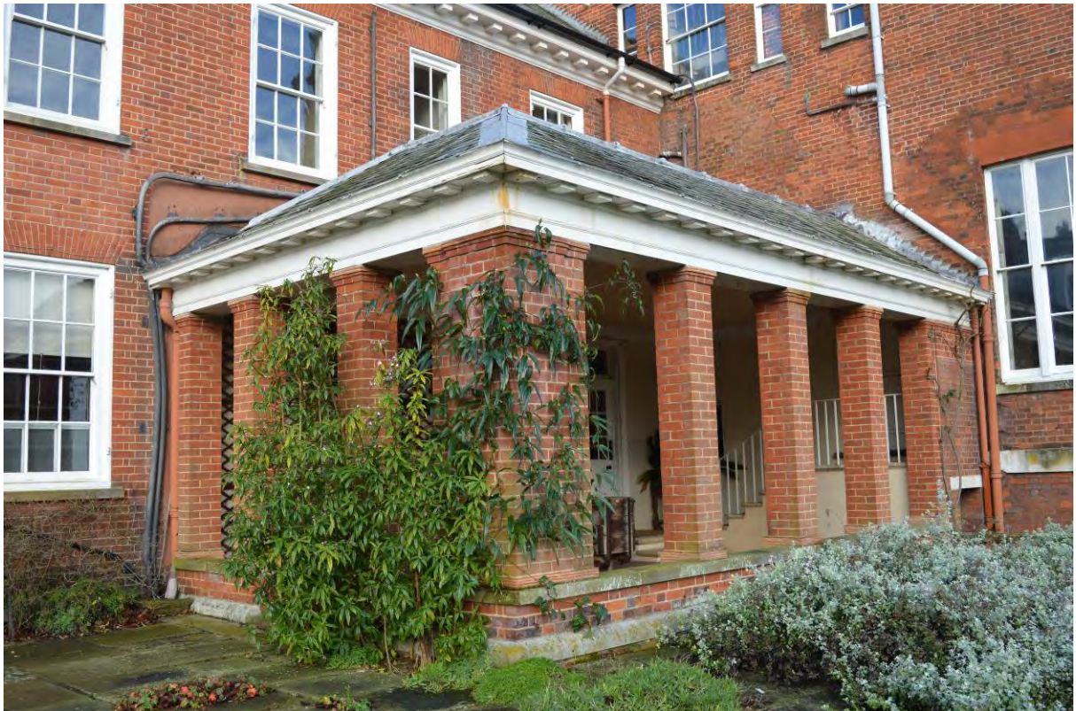
Plate 24: The loggia, showing scar to brickwork probably relating to earlier glasshouse (101)
