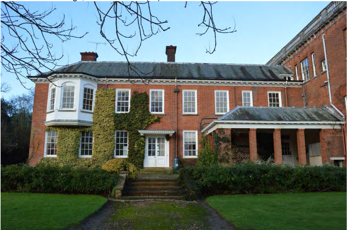
Plate 20: South range, east elevation (100)
