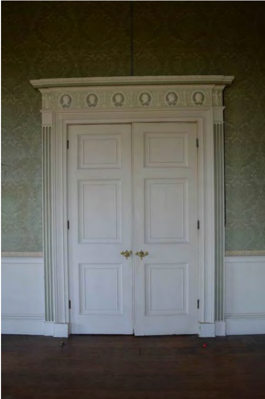
Plate 45: Detail of door, Room 6 (66)
