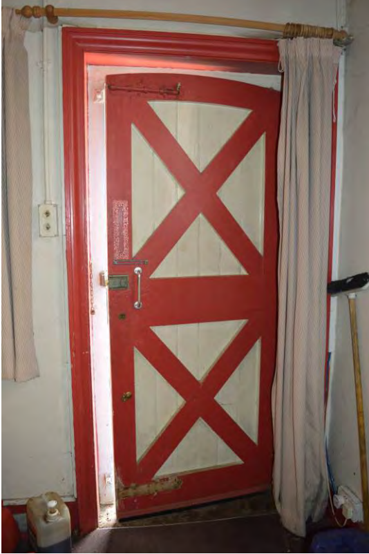
Plate 97: Interior face of external door, Room N4 (356)
