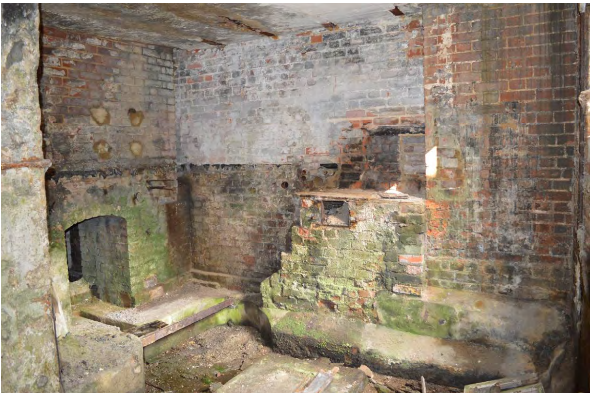
Plate 120: Former 'heating place' in northern chamber of external cellar (377)
