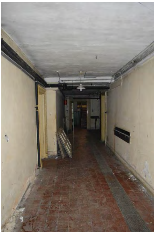
Plate 56: Room B2, looking south (309)
