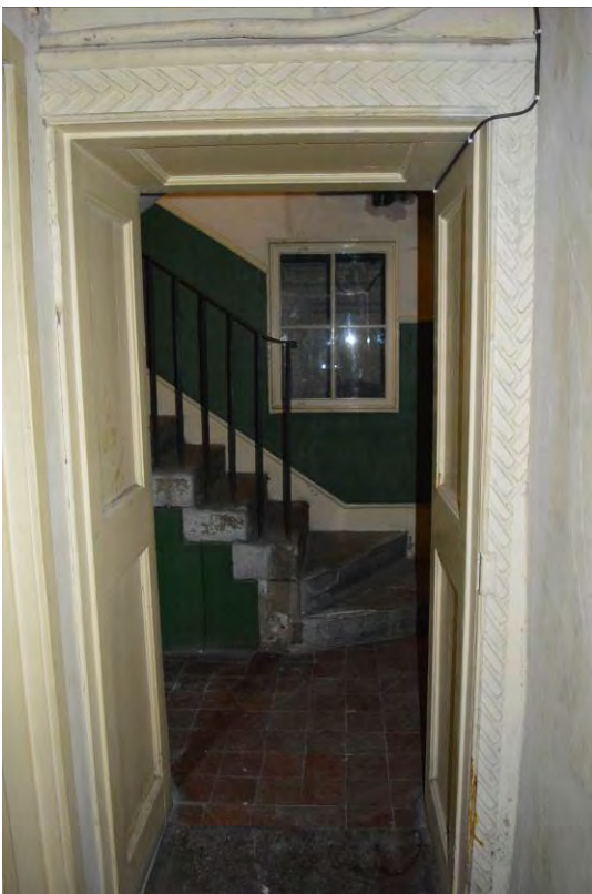
Plate 64: Lattice-style architrave on room side of doorway, Room B9 (327)
