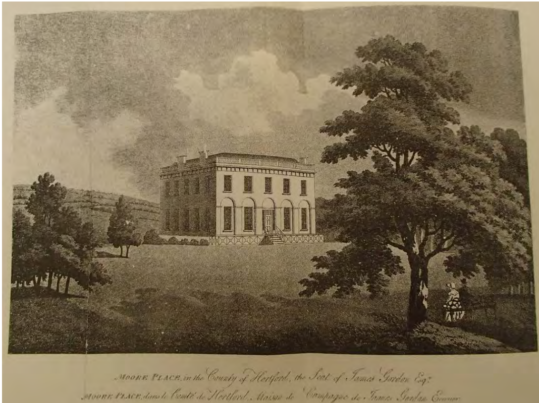
Plate 1: View of Moor Place (west façade) by Robert Mitchell, Architect, published 1801 (HALS ref DE/Gr/33/1/20)
