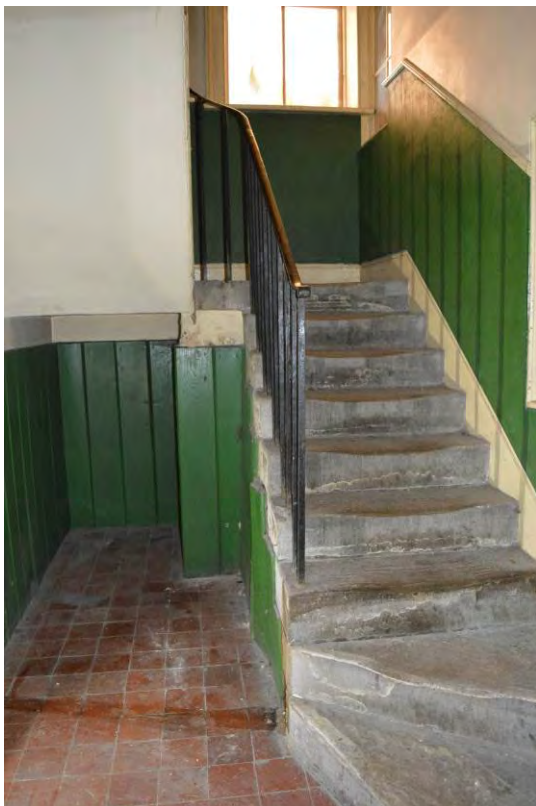
Plate 54: Stair lobby at bottom of service stair (305)
