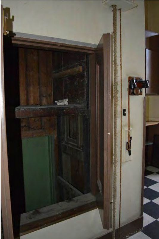
Plate 49: Dumb waiter and telephone in Room 8 (78)
