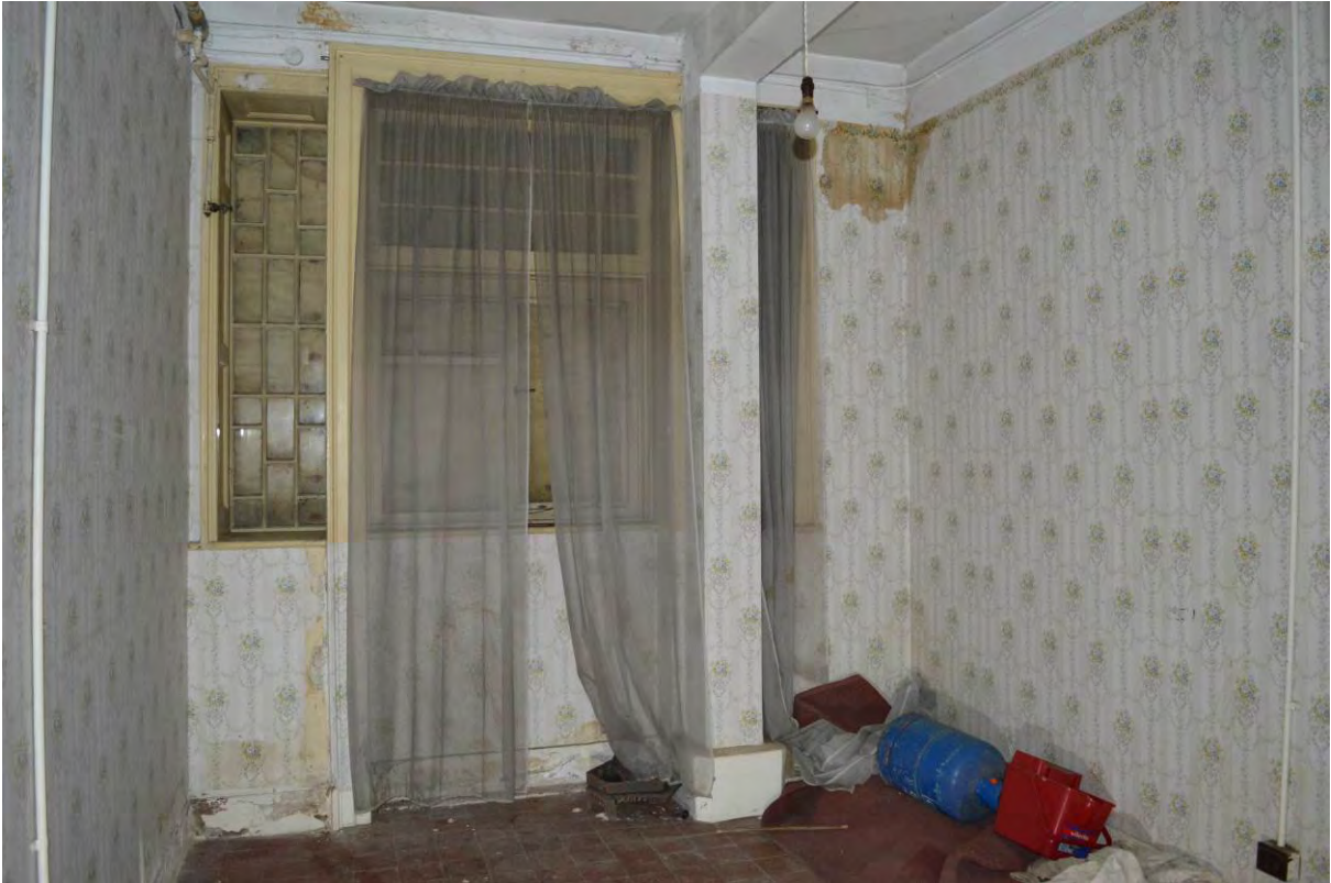
Plate 61: Former external entrance to basement (317)
