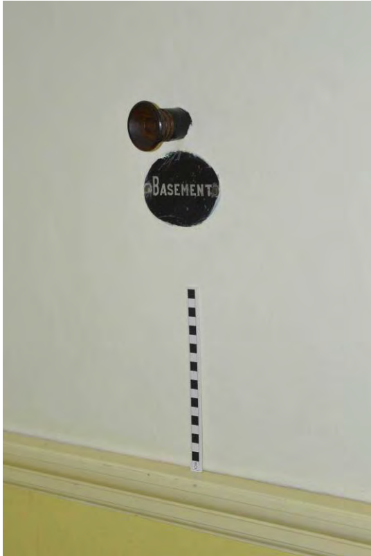
Plate 53: Mouthpiece for speaking tube (228)
