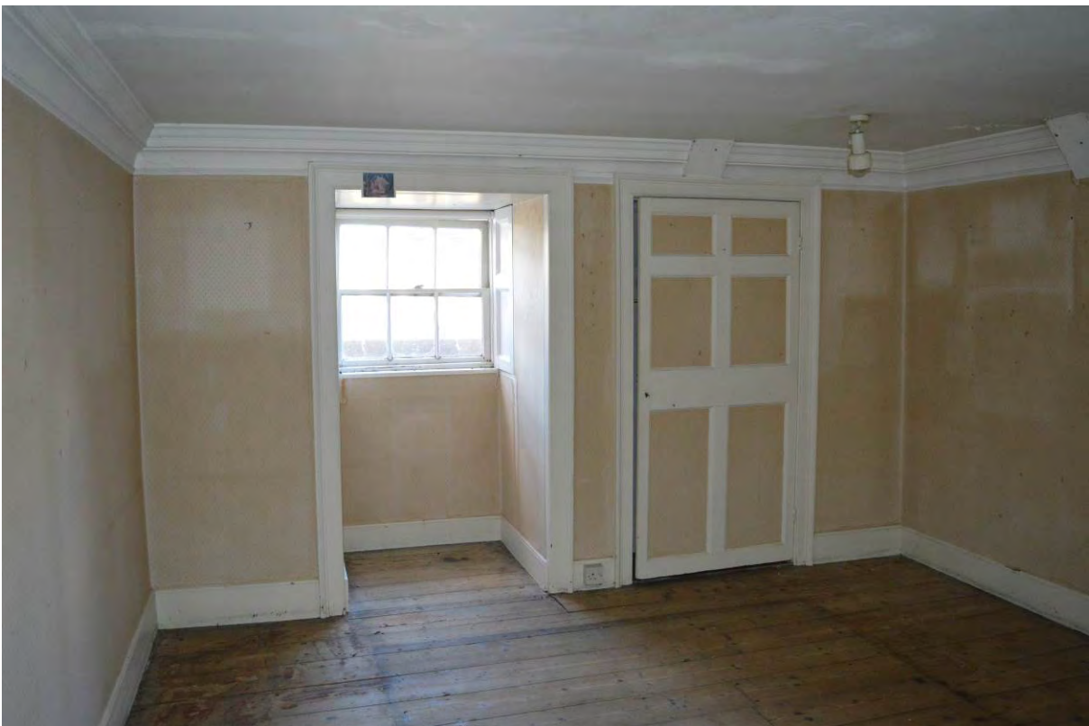
Plate 92: Room 30, looking north (210)
