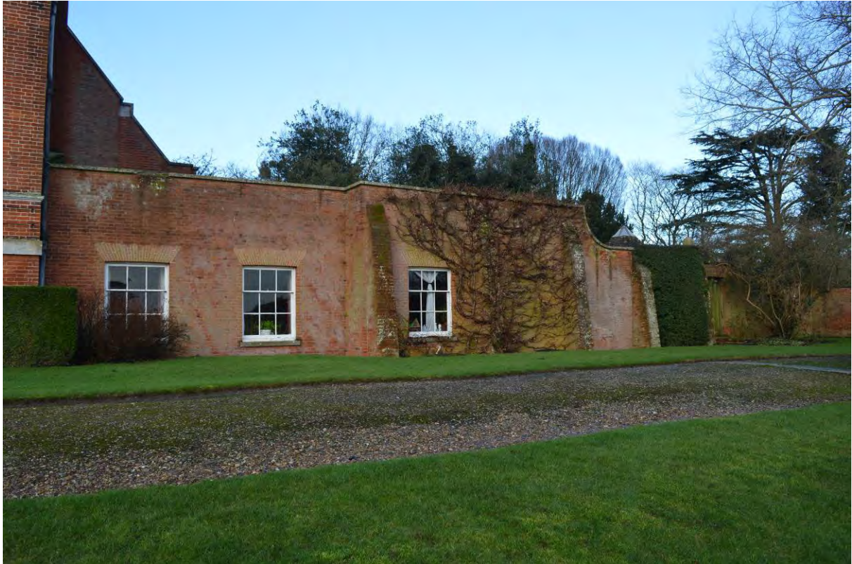
Plate 15: North range, east elevation (110)
