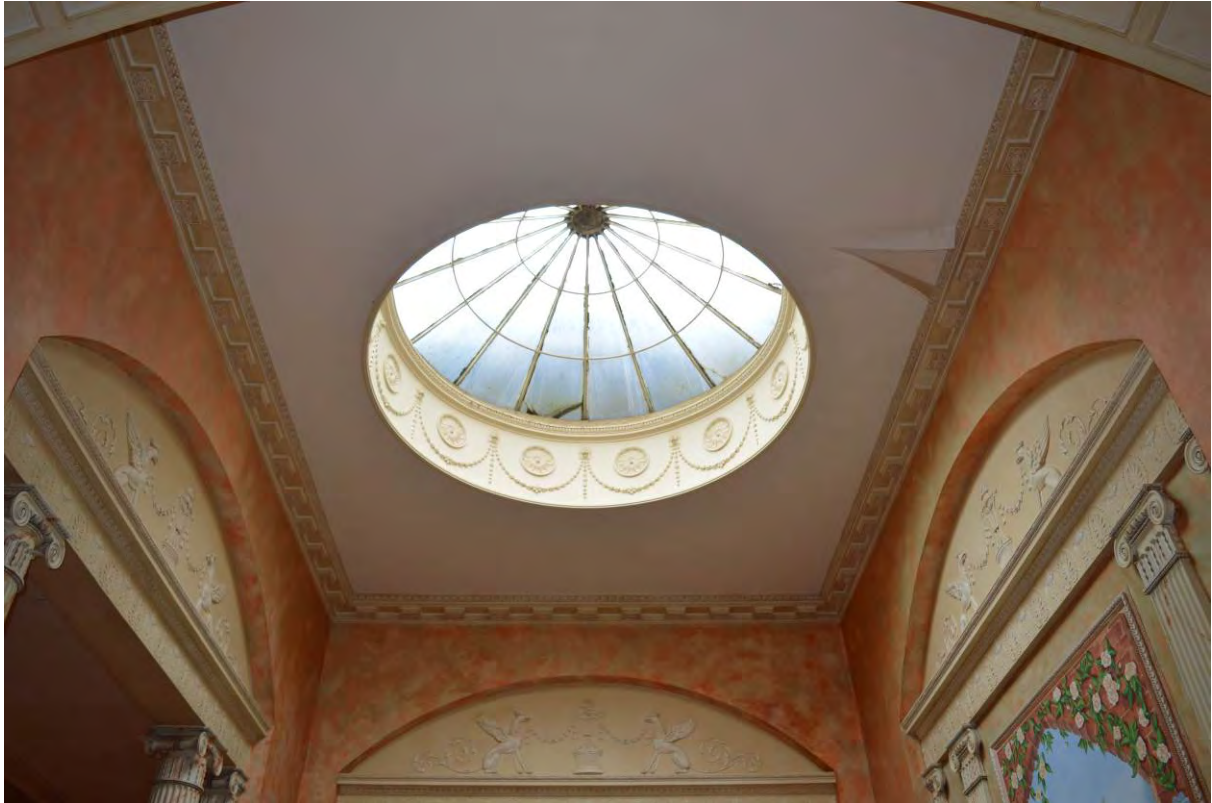
Plate 73: Glazed roof lantern lighting stair hall (28)
