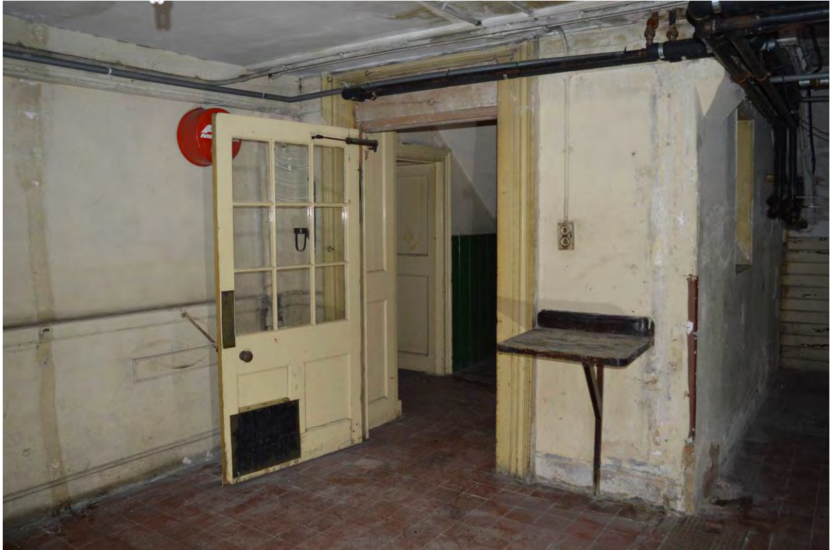
Plate 55: Room B2, looking towards stair lobby (307)
