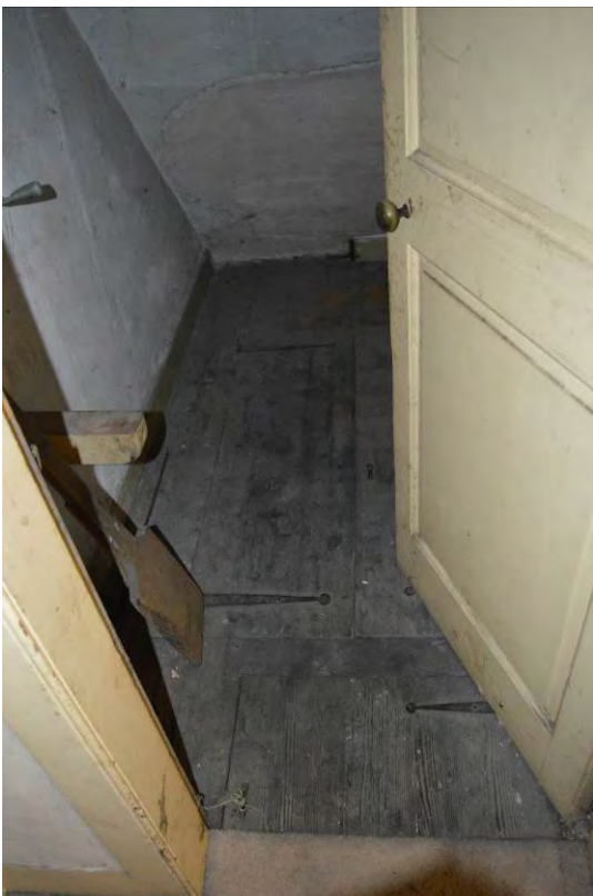
Plate 90: Trapdoors in floor of Room 27 (201)
