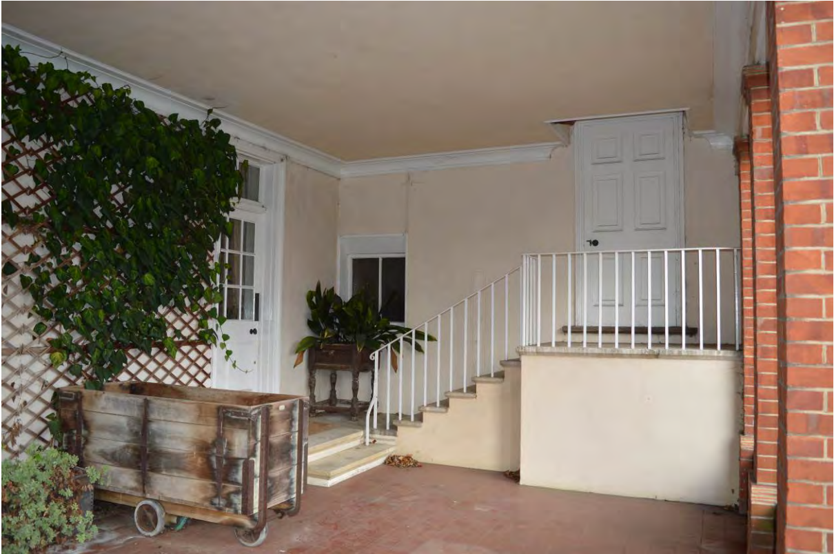
Plate 21: View of interior of loggia to east elevation of south range (103)
