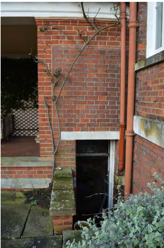
Plate 22: Steps and door to small basement room (104)
