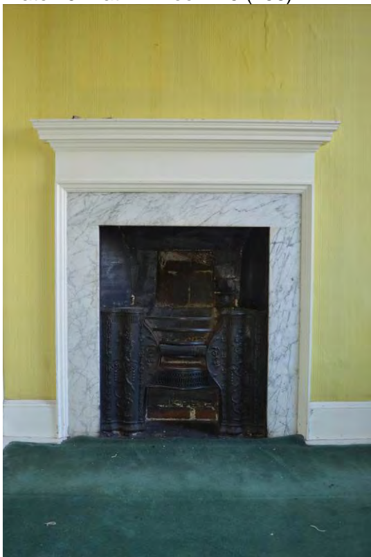
Plate 80: Fireplace in Room 17 (162)
