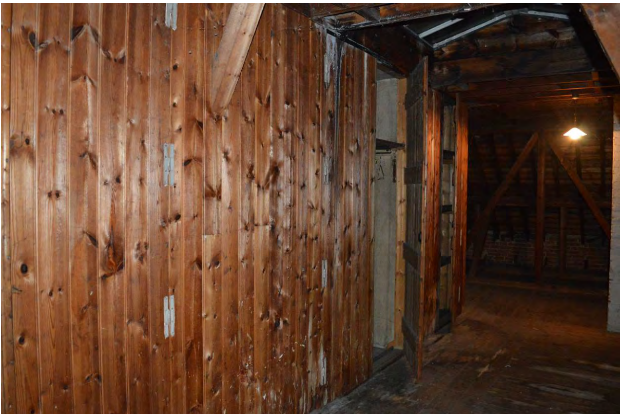
Plate 116: Storage cupboards in attic of south range (295)
