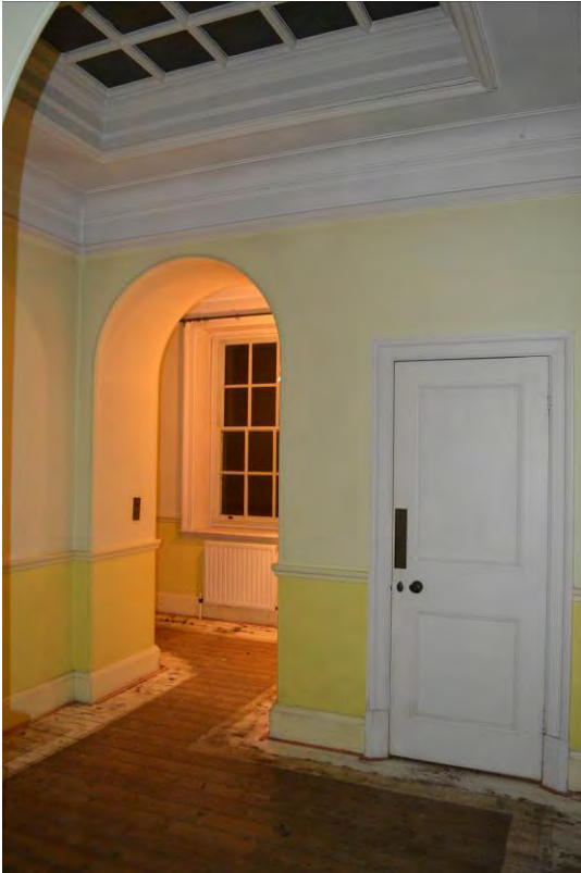
Plate 115: North lobby, looking north-west (284)
