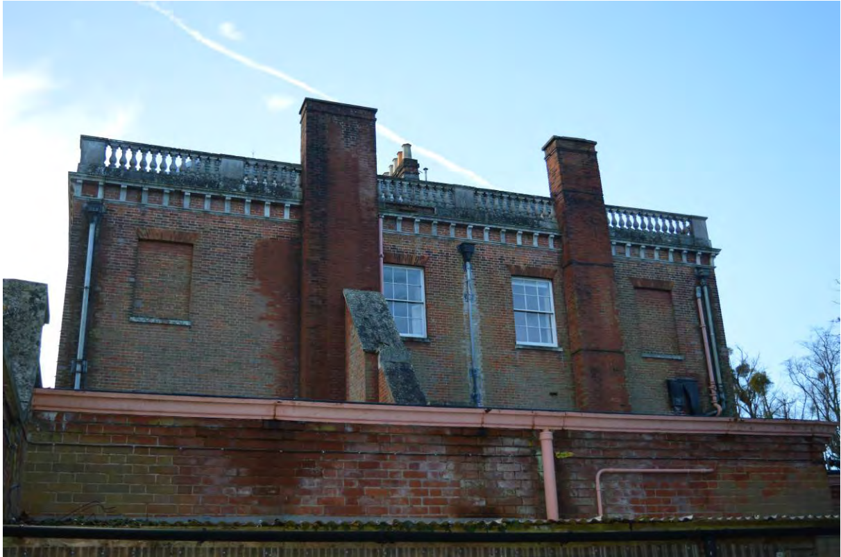
Plate 13: North elevation showing detail of first floor and parapet (112)
