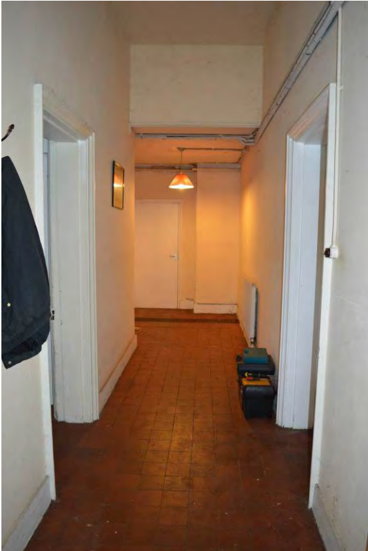
Plate 98: Corridor N6, looking south (357)
