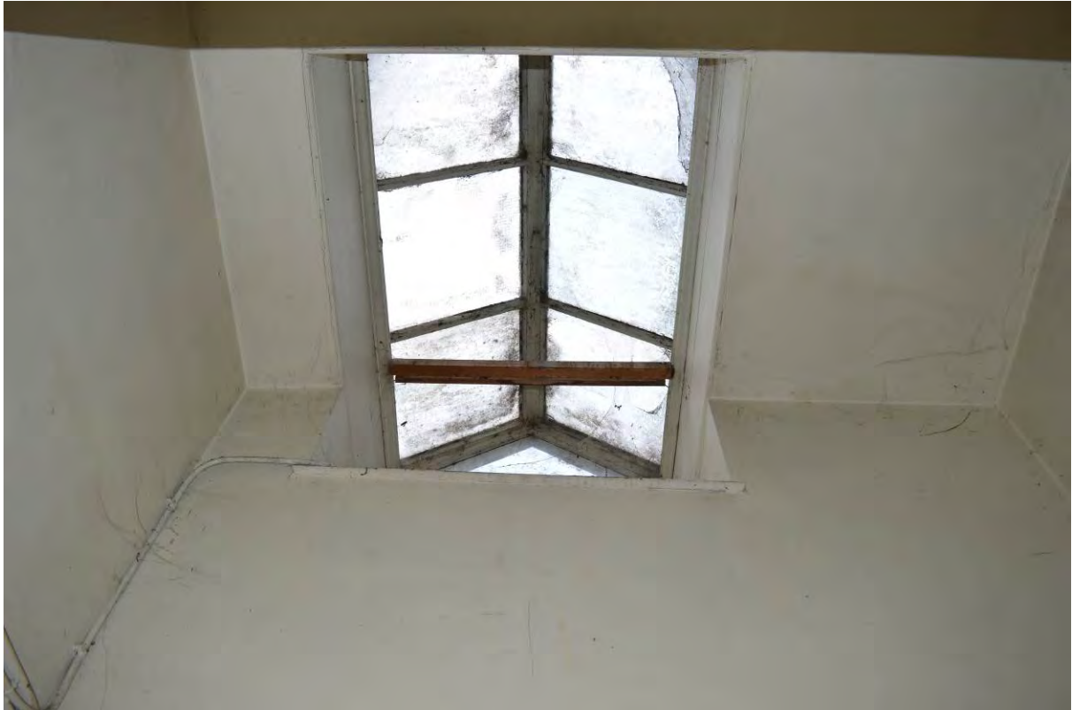
Plate 99: Roof lantern above Room N7, previously lighting corridors N6 and B2 (362)
