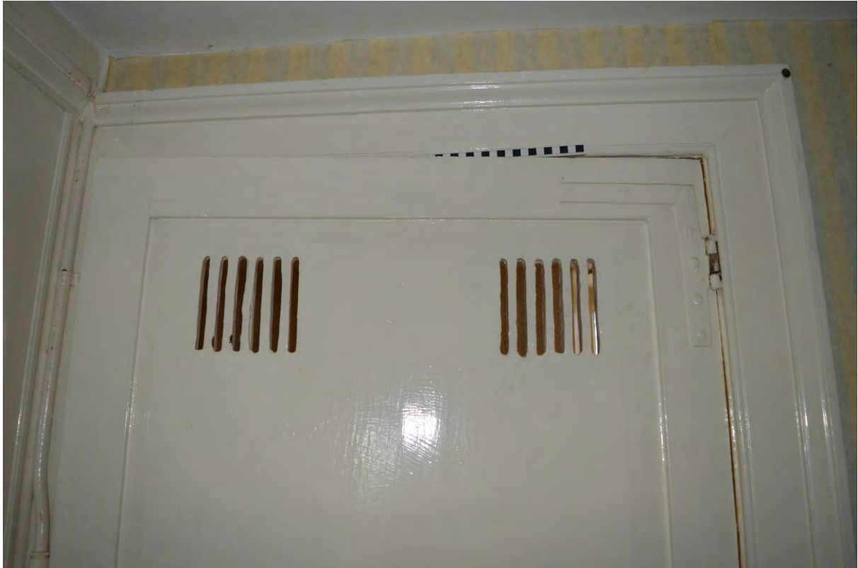
Plate 93: Detail of door, Room 31 (217)
