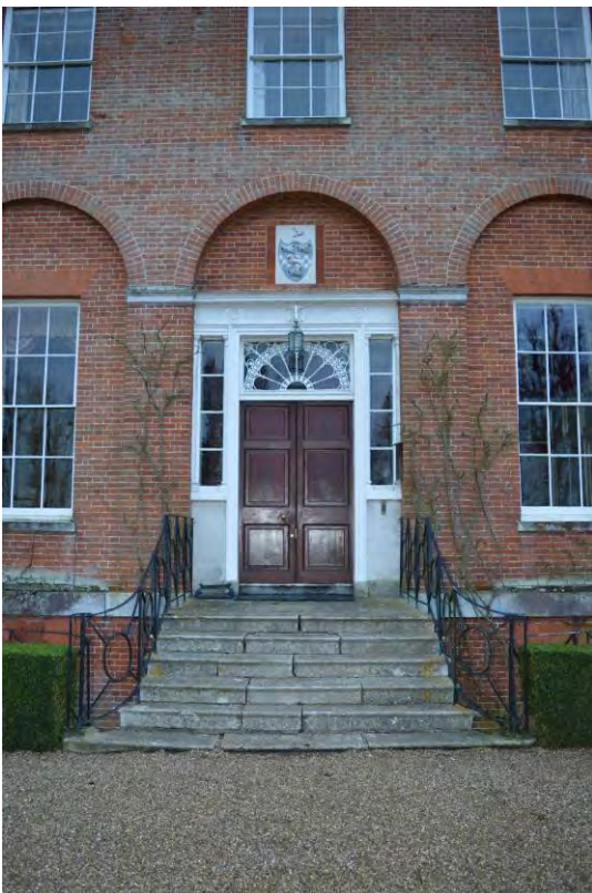
Plate 6: Principal entrance doorway (88)
