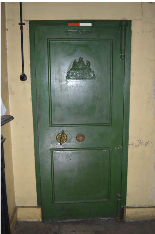
Plate 58: Door to safe, Room B3 (313)
