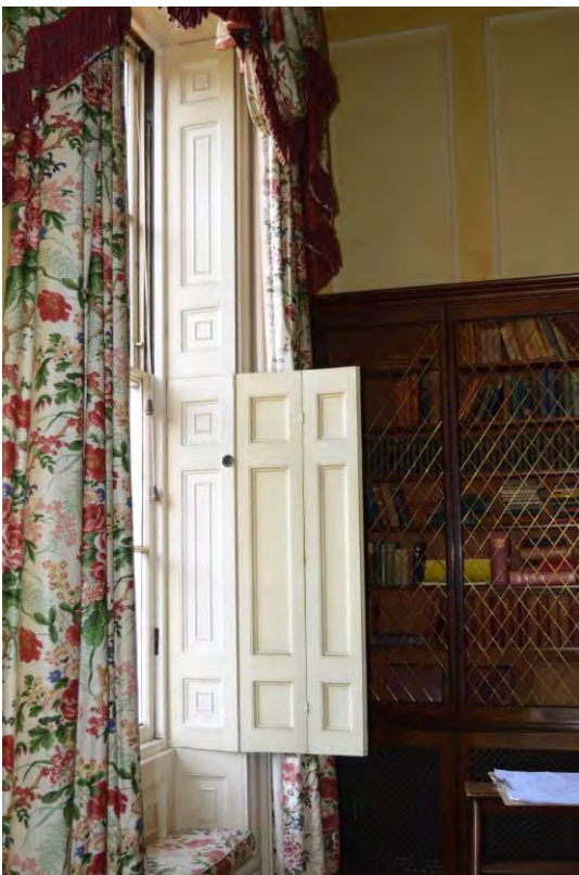
Plate 32: Type 2 shutters in Room 3 (43)
