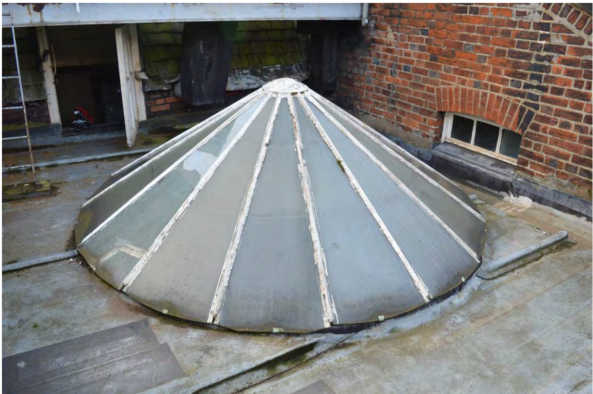
Plate 94: External detail of roof lantern (223)
