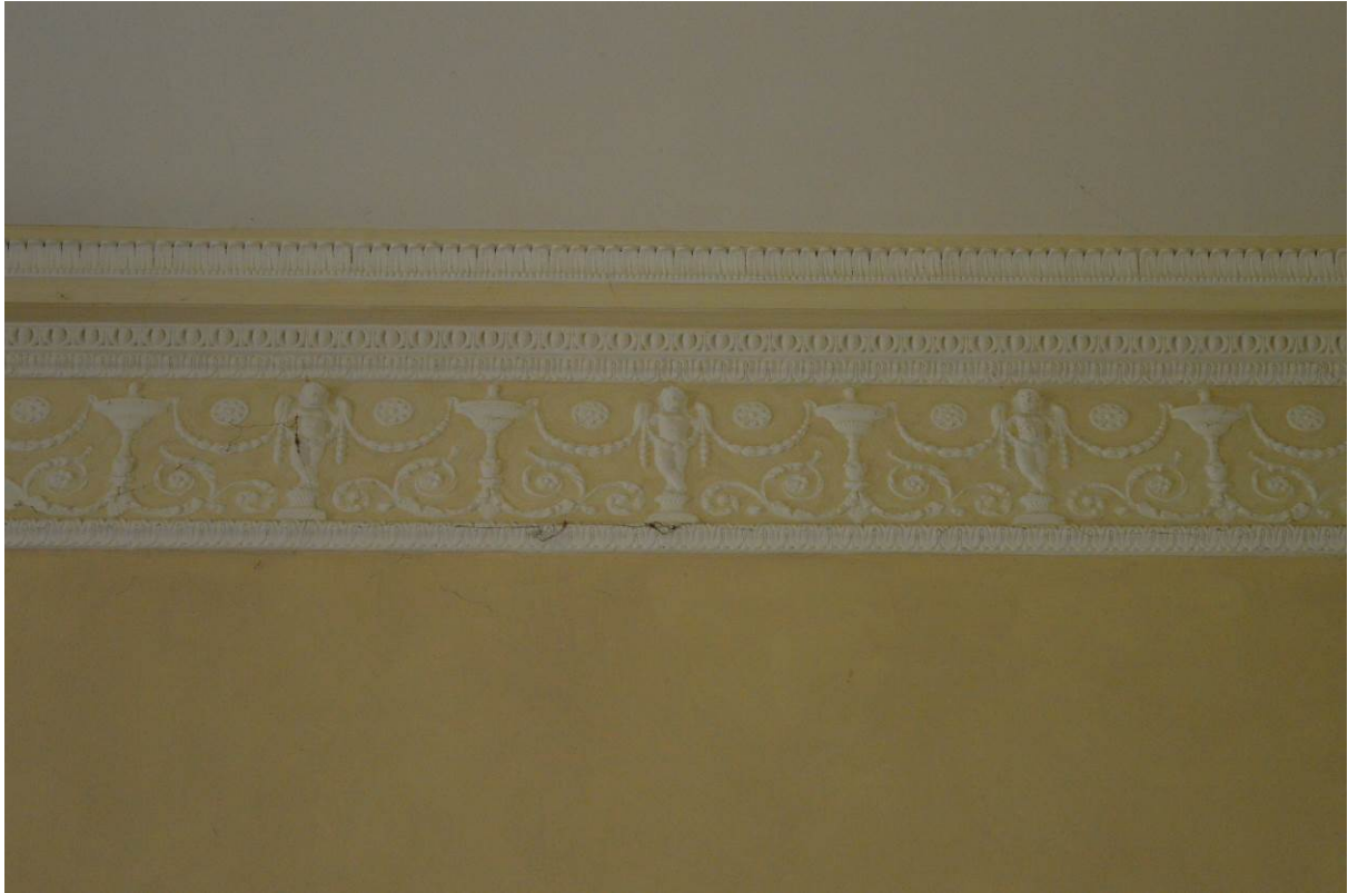
Plate 39: Detail of frieze and cornice, Room 4 (53)
