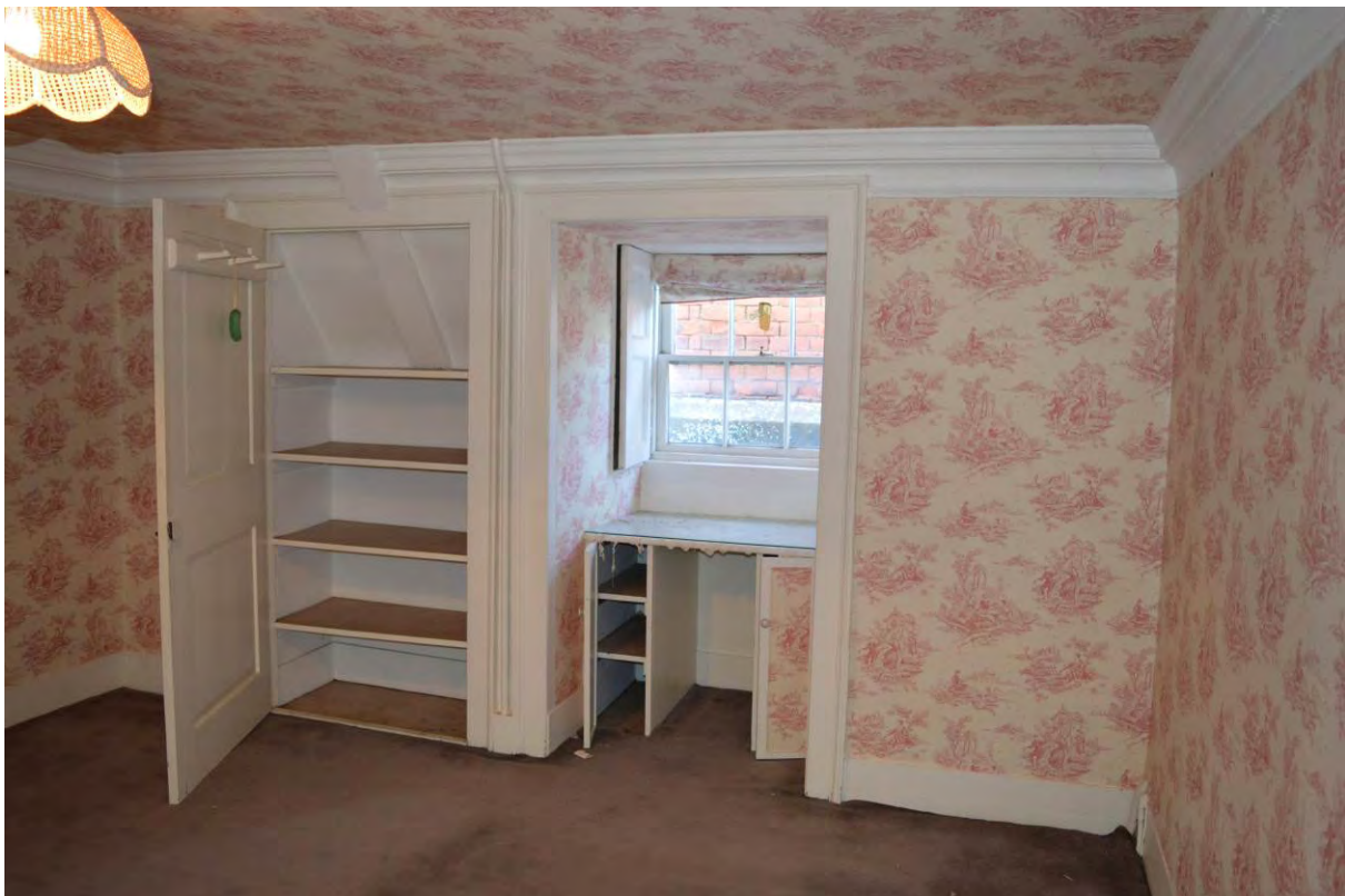
Plate 86: Room 23, looking north-west (186)
