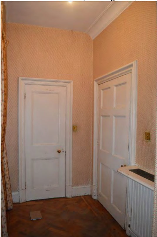
Plate 104: Corridor (S1) with inserted partition forming cupboard in south range (237)
