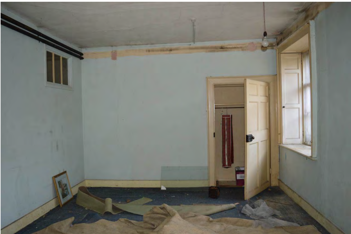
Plate 60: Room B5, looking south (319)
