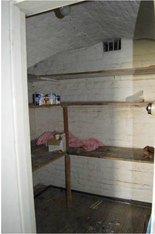
Plate 69: Interior of store cupboard in Room B11 (339)
