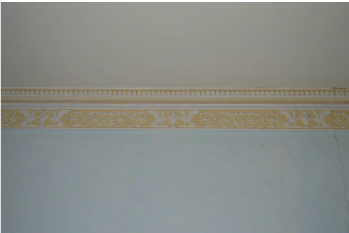
Plate 76: Room 10, detail of cornice (135)
