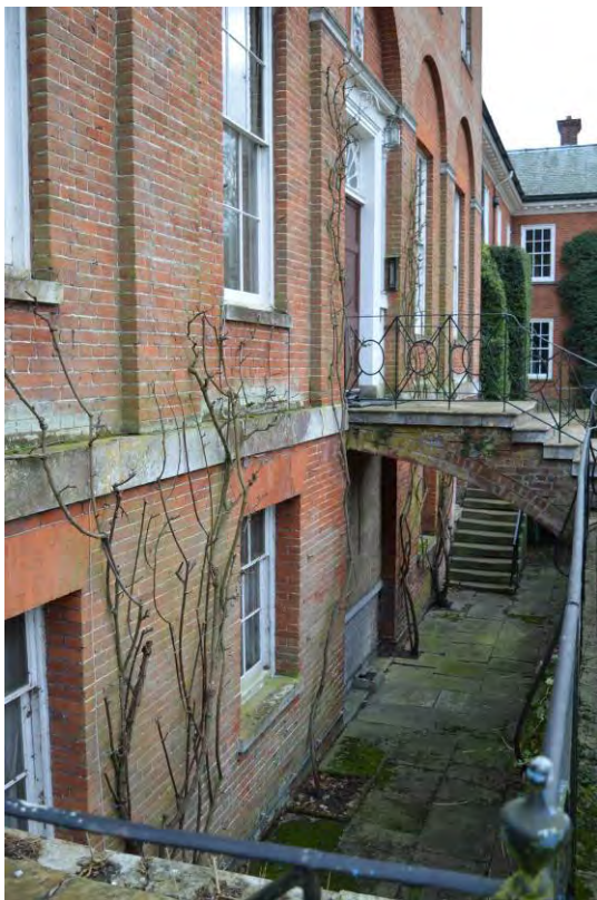
Plate 8: The basement lightwell (85)
