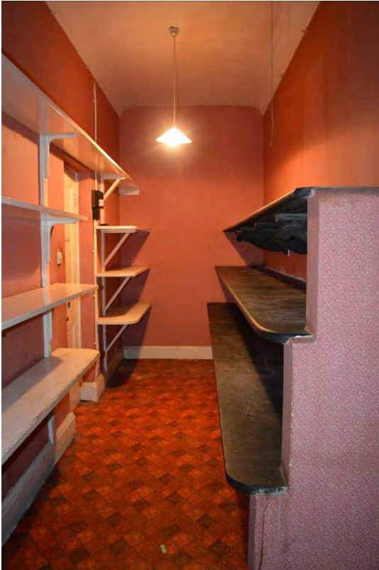
Plate 107: Former corridor (S4) looking north, showing pantry shelves (245)
