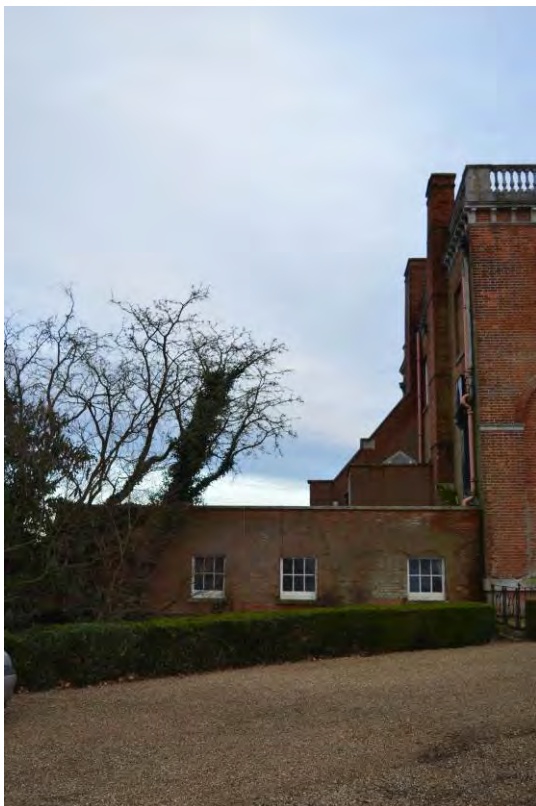
Plate 14: North range, west elevation (84)
