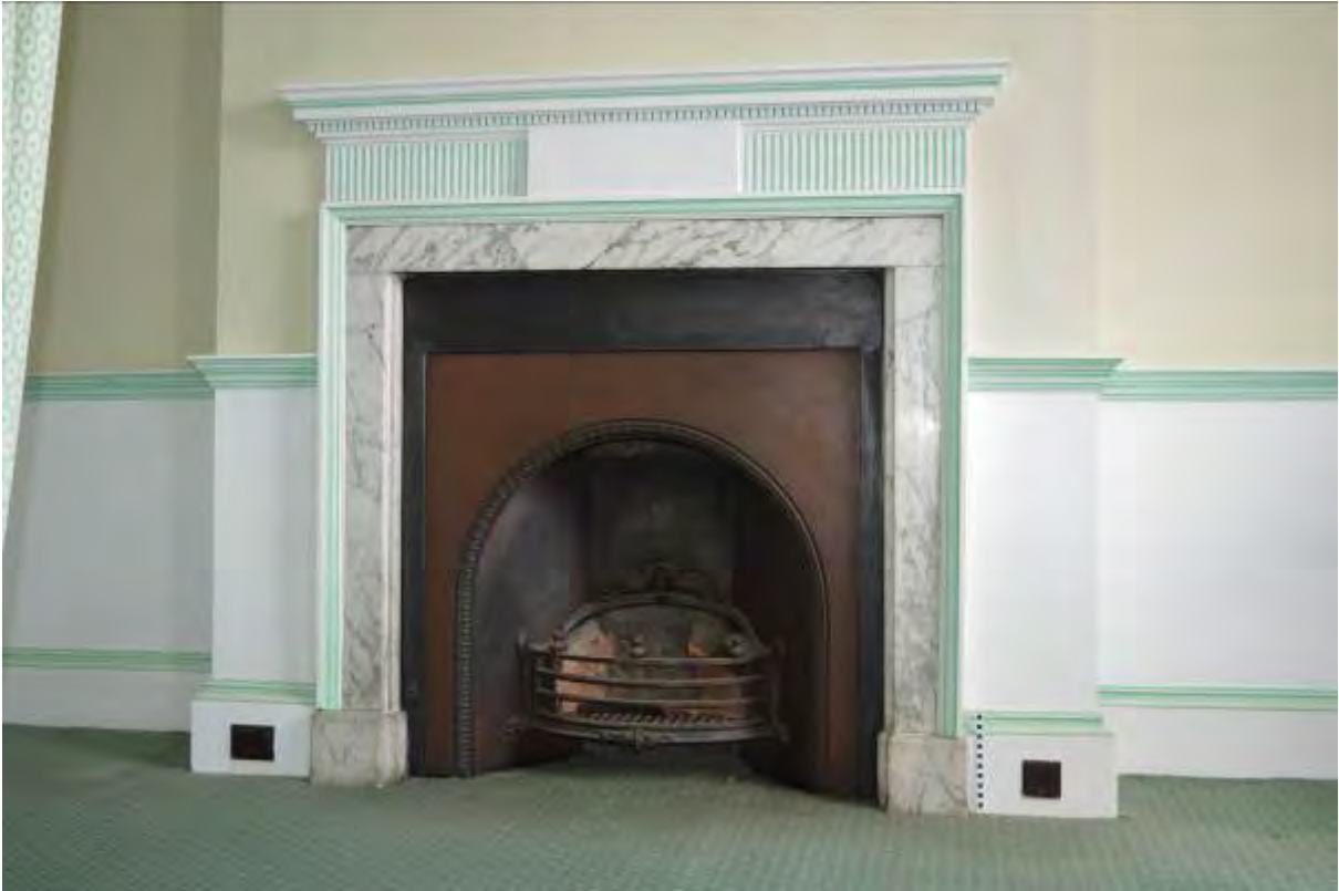
Plate 83: Detail of fireplace, Room 19 (171)
