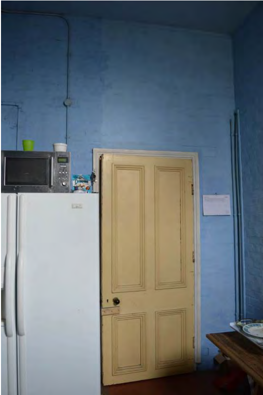
Plate 103: Room N10, looking east, showing brick relieving arch for wider door (371)
