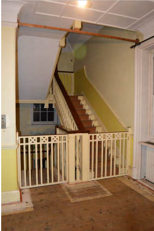
Plate 111: Dog-gates, first floor landing (S9) (262)
