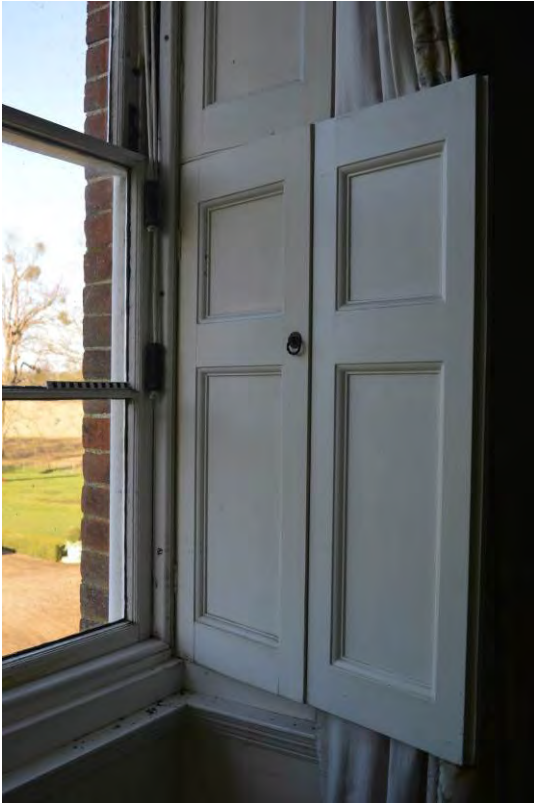
Plate 75: Room 10, detail of shutters (139)
