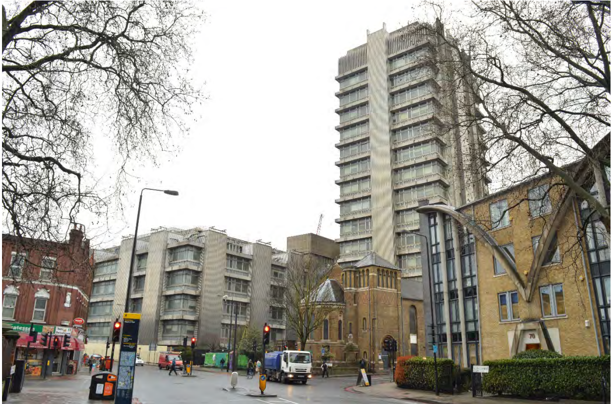
Plate 1: Keybridge House from the north-east (1)
