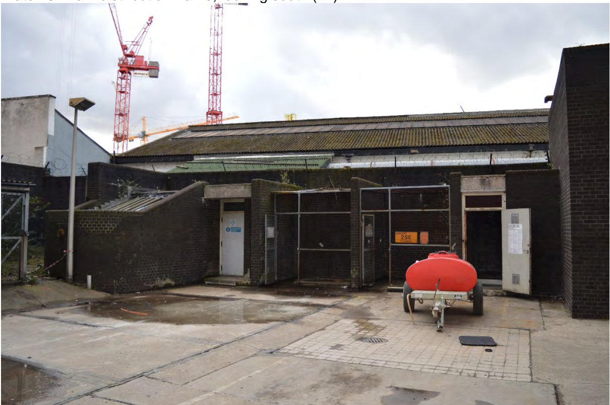
Plate 14: Brick external storage with exit stair to left (182)
