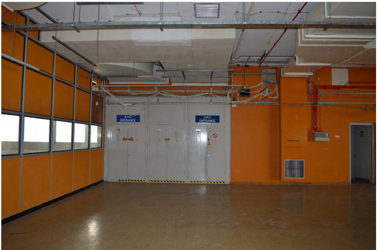
Plate 8: Access to AHU service duct, fourth floor of podium (33)
