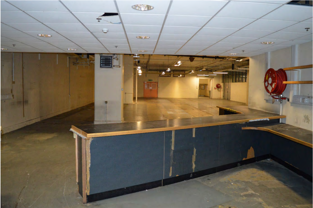
Plate 11: Stores for customer equipment and stock for engineers (64)
