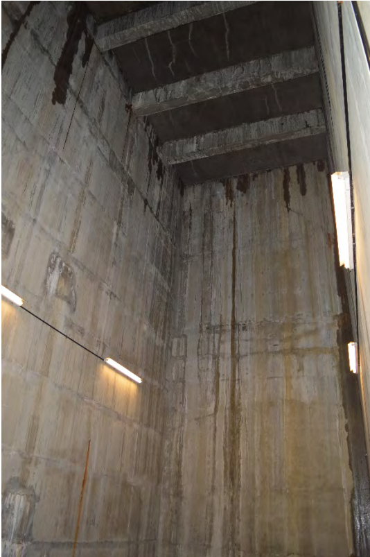
Plate 17: Void for engine access with removable concrete ceiling (58)
