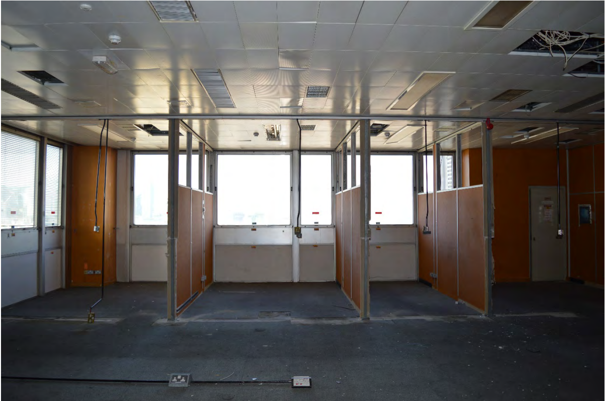
Plate 33: Office/workshop cubicles on tenth floor (97)
