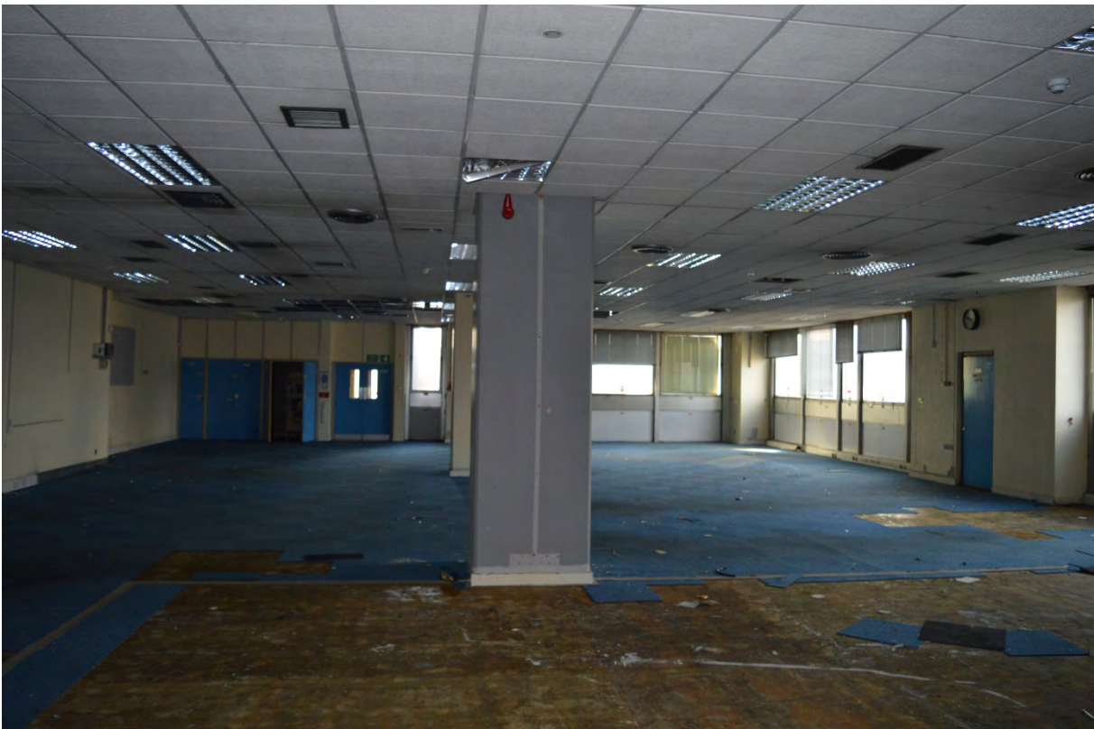
Plate 28: Office in first floor of tower (158)
