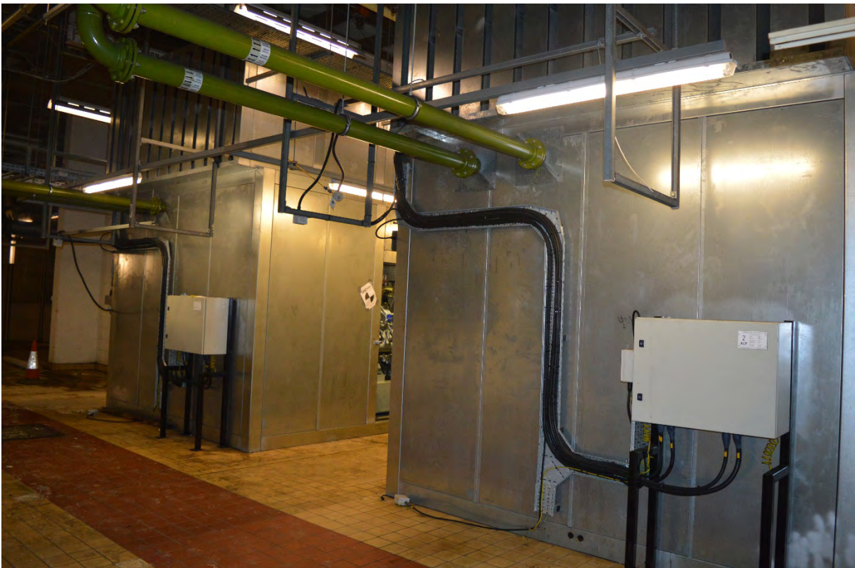
Plate 18: Soundproofed metal enclosures for DRUP engines (53)
