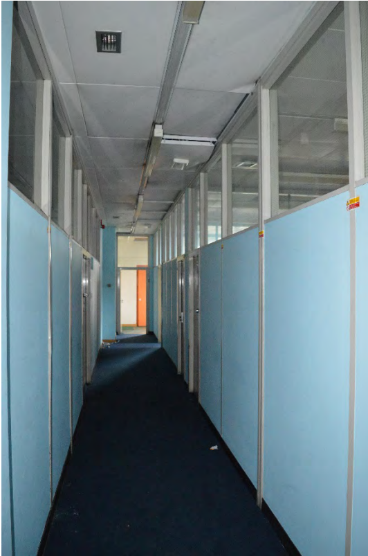
Plate 27: Lightweight partitions forming corridor in first floor of tower (157)
