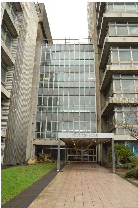
Plate 6: Principal entrance on east side of link building (13)
