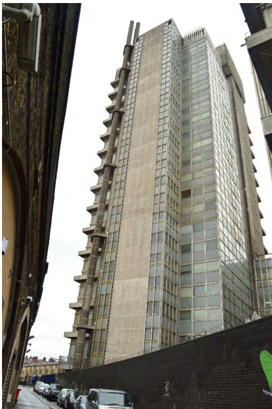
Plate 4: The tower from the south-west (6)
