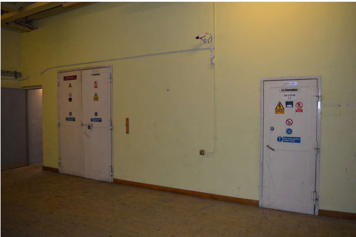
Plate 24: Entrance to first floor substation (159)
