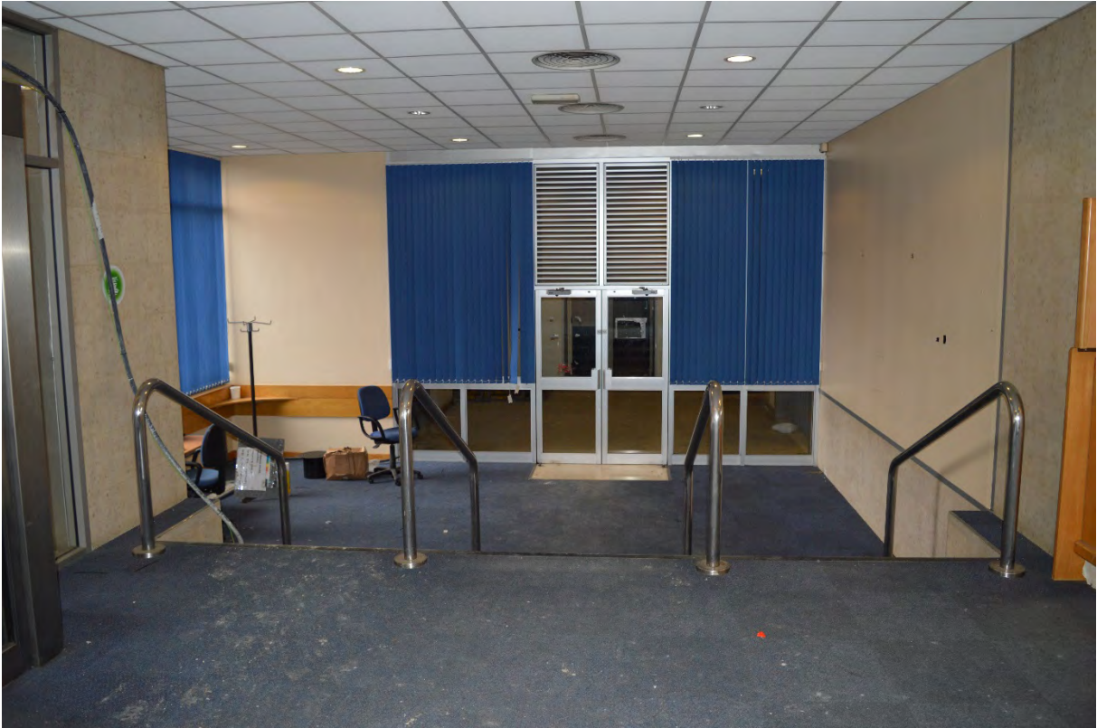
Plate 9: Entrance lobby, looking south towards podium (69)
