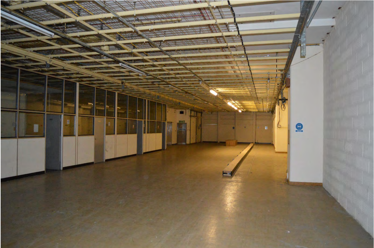
Plate 13: Main distribution frame, looking south (44)
