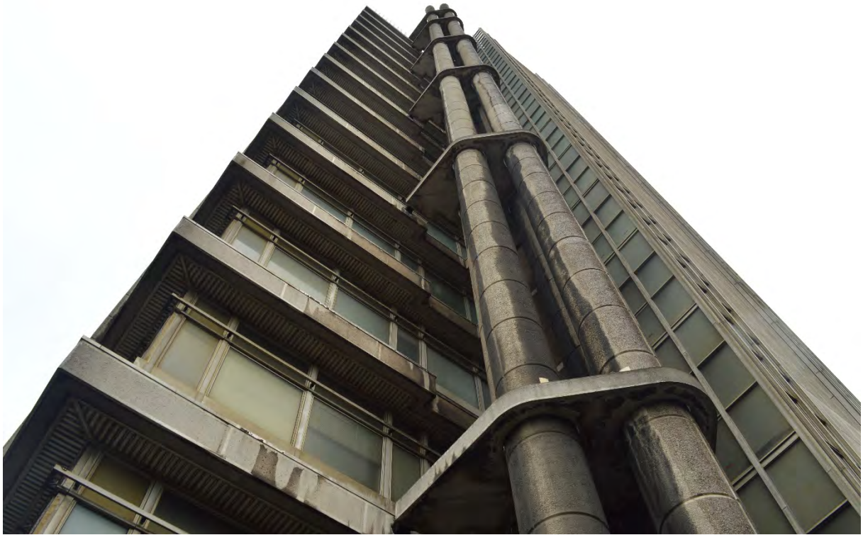
Plate 7: Detail of concrete flues on east side of tower (4)
