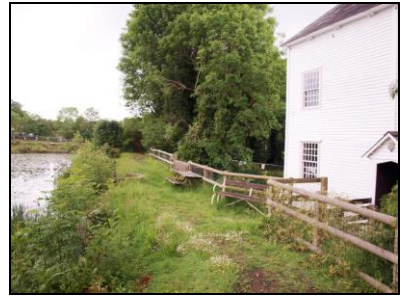
6621-0024 Dam and mill. Facing west
