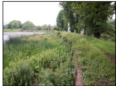
6621-0030 Dam face. Facing west
