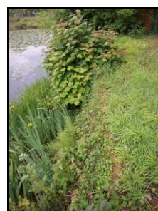
6621-0015 Dam face. Facing west
