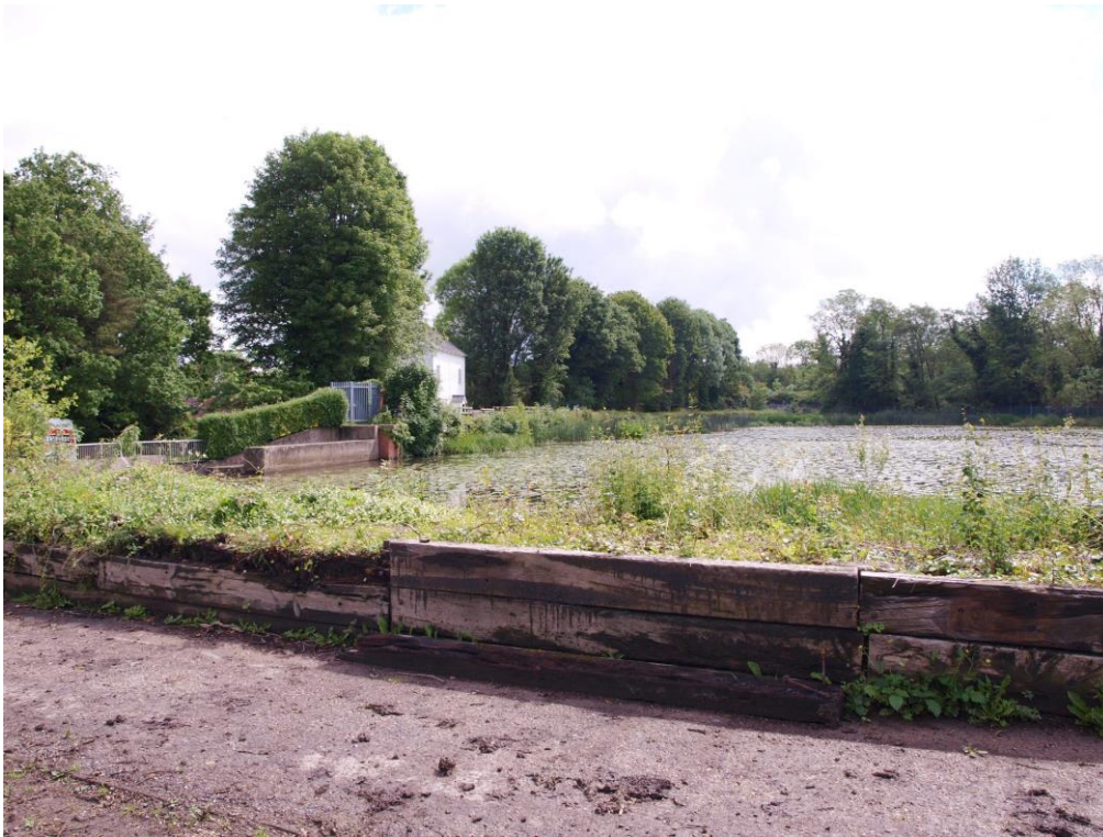
Plate 1 – General view of the Ifield Mill and dam, looking north-east
