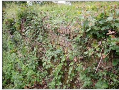
6621-0032 Dam face. Facing northwest
