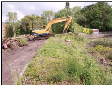
6621-0043 Pond bank. Facing north
