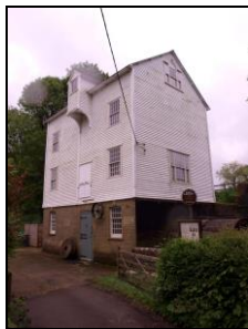
6621-0001 Ifield Mill. Facing southeast
