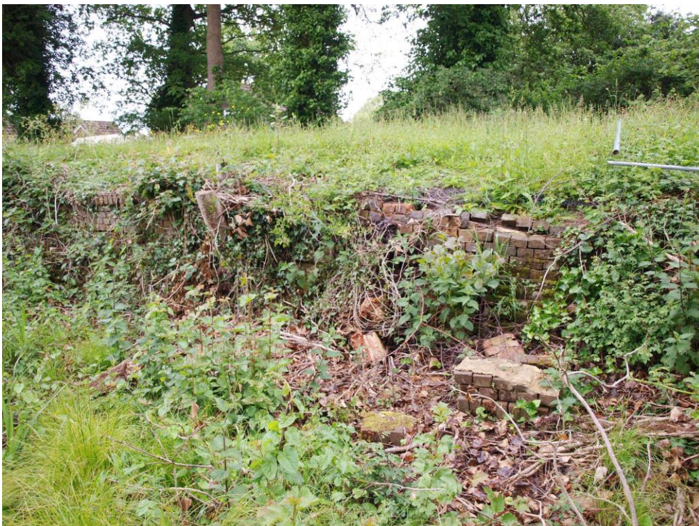
Plate 6 – Brick facing to eastern end of dam, looking north
