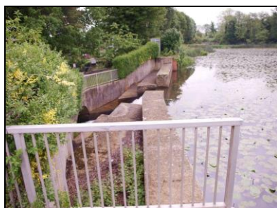
6621-0010 Spillway. Facing east
