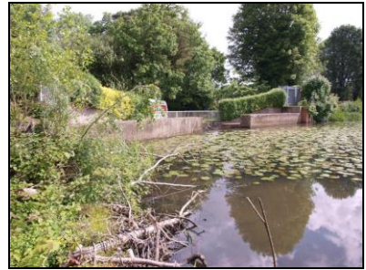
6621-0039 Spillway. Facing northeast
