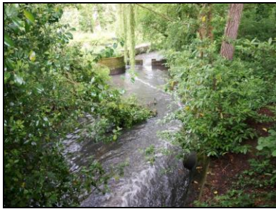
6621-0034 Spillway pond. Facing north
