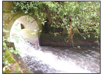
6621-0036 Spillway bridge. Facing southwest
