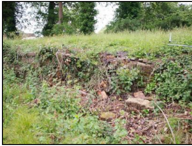
6621-0031 Dam face. Facing northwest
