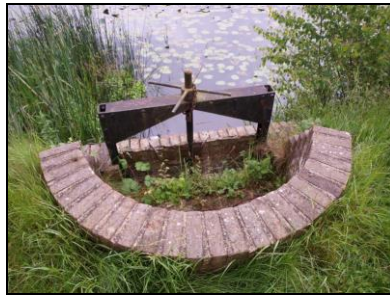
6621-0020 Penstock. Facing south
