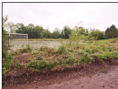
6621-0008 Dam rear. Facing south
