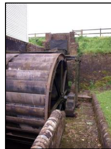
6621-0003 Ifield Mill wheel pit. Facing south
