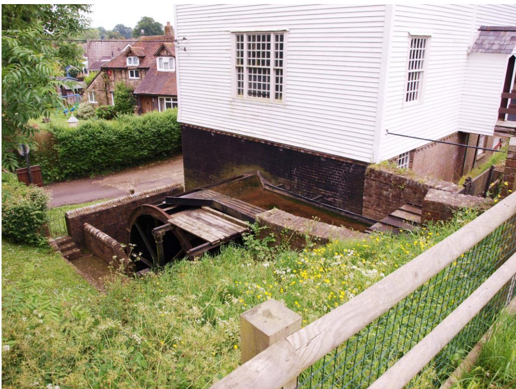
Plate 12 – General view of wheel pit and head race, looking north-east
