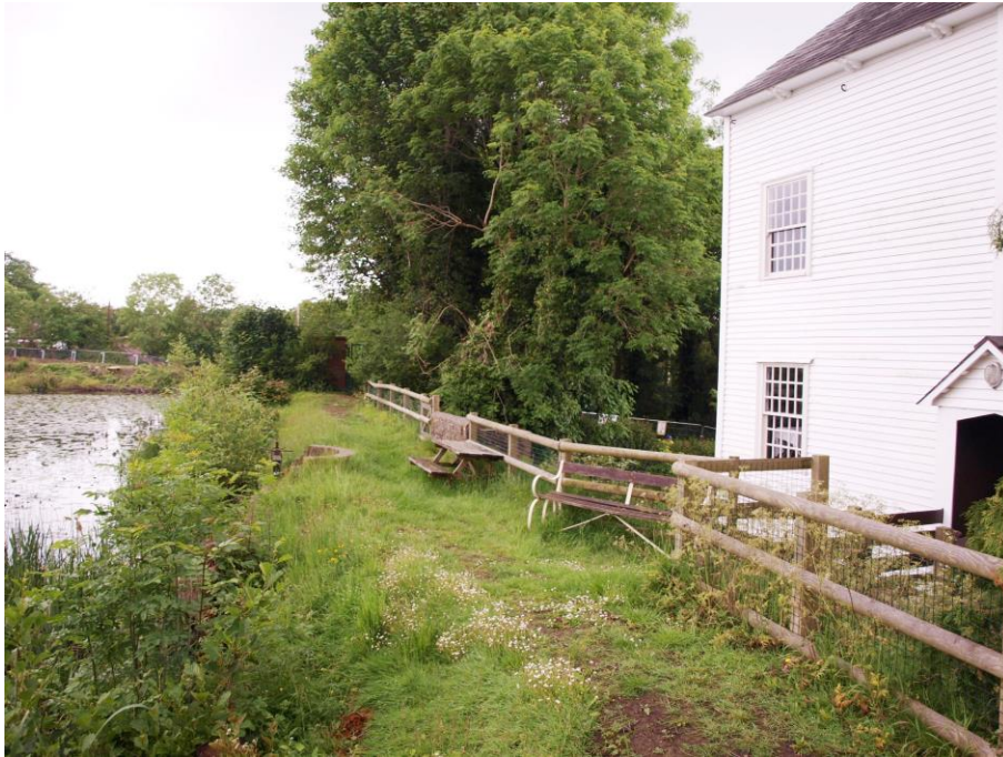
Plate 3 – The dam walkway, looking west from Ifield Mill
