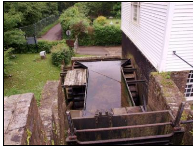
6621-0017 Mill race. Facing north
