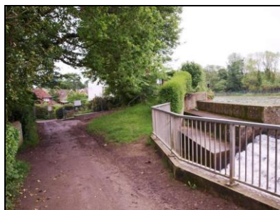
6621-0007 Spillway. Facing east
