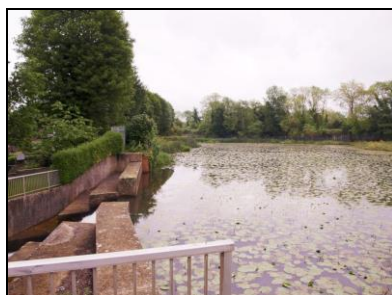
6621-0011 Dam and pond. Facing east
