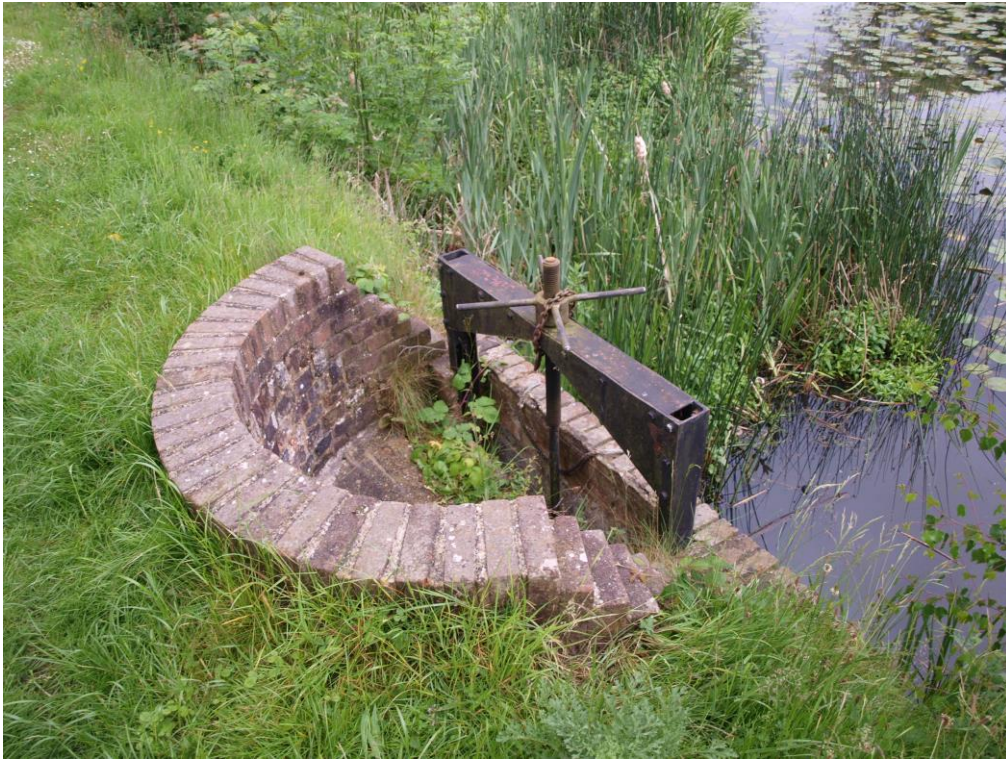
Plate 7 – Penstock and brick culvert to head race, looking south-east
