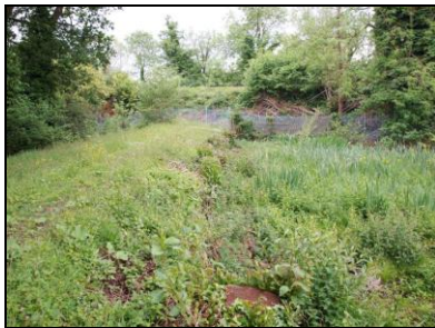
6621-0028 Dam and railway. Facing east
