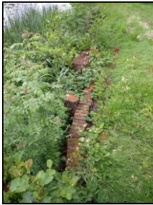
6621-0025 Dam face. Facing west
