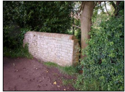
6621-0033 Spillway bridge. Facing northwest
