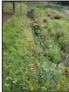
6621-0026 Dam face. Facing east
