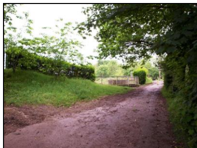
6621-0005 Dam rear. Facing southwest
