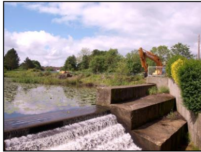
6621-0038 Spillway. Facing southwest
