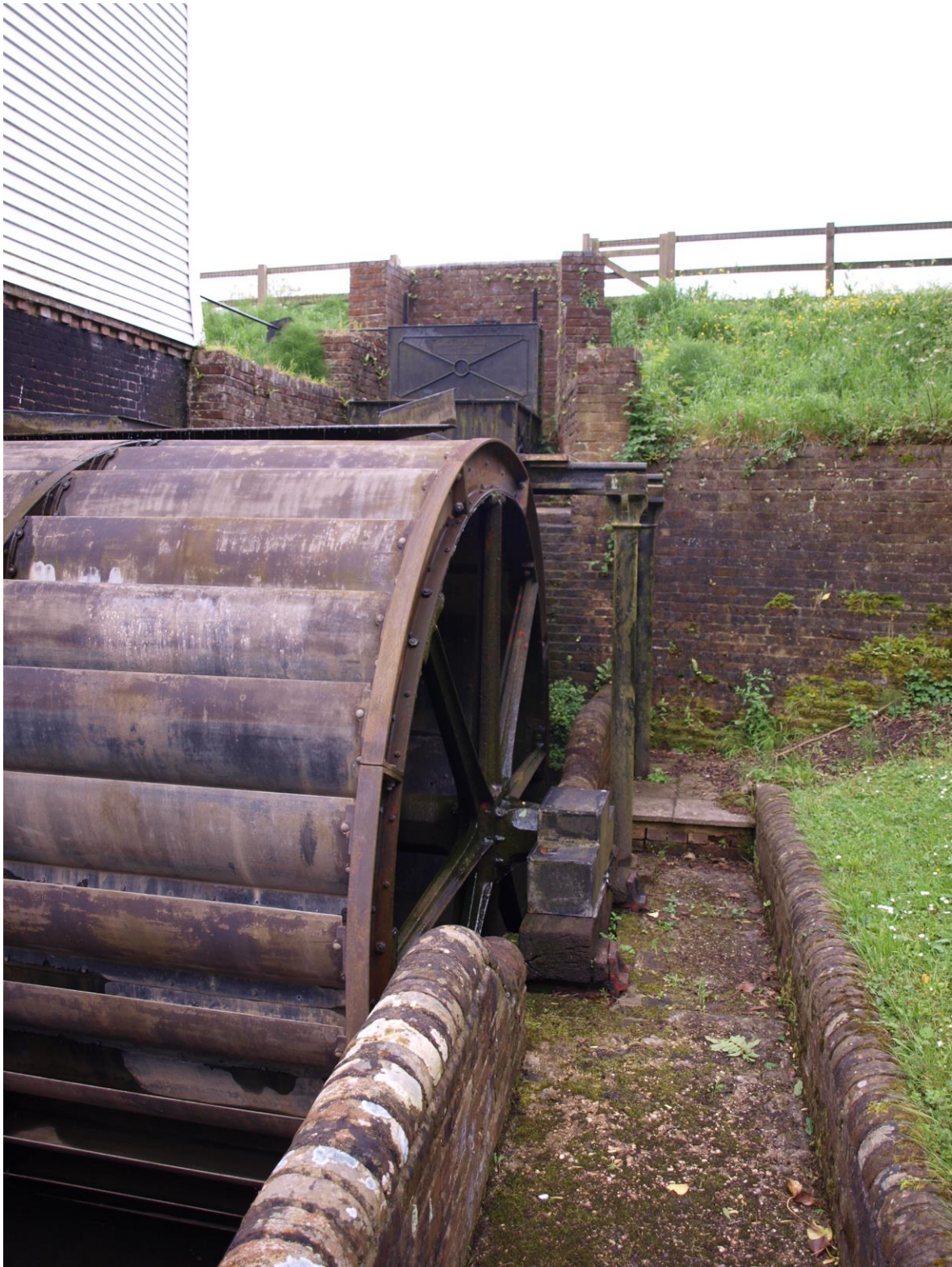
Plate 13 – General view of wheel pit and head race, looking south
