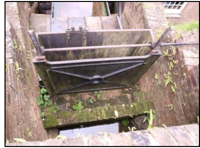
6621-0018 Mill race. Facing north
