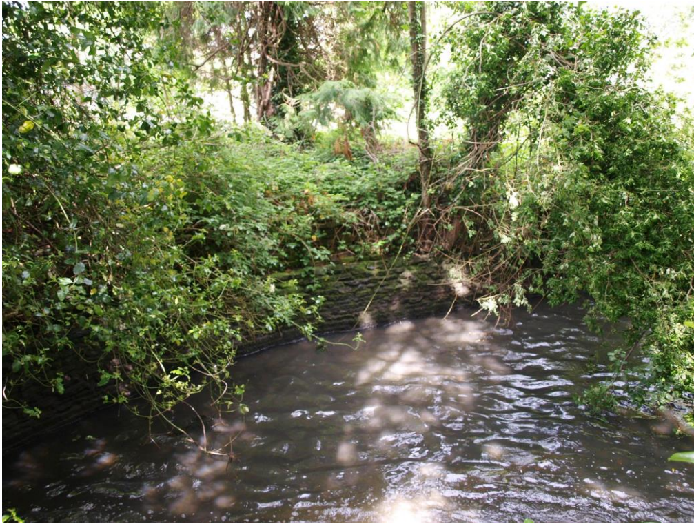
Plate 11 – Sandstone and brick pond beyond spillway, looking north-west
