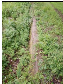
6621-0029 Dam face. Facing west
