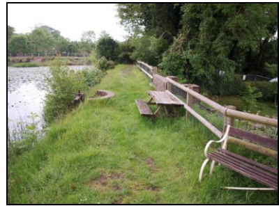
6621-0021 Dam walkway. Facing west
