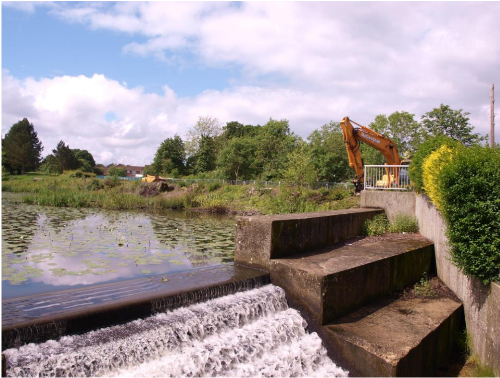
Plate 9 – Stepped weir and concrete spillway, looking south-west
