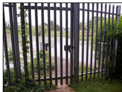
6621-0012 Spillway gate. Facing south
