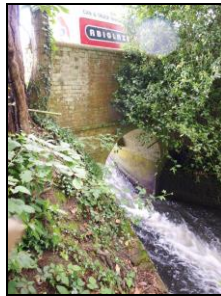
6621-0035 Spillway bridge. Facing southwest
