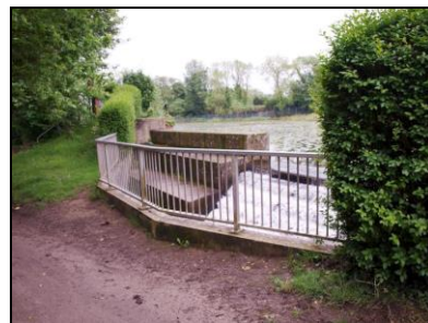
6621-0006 Spillway. Facing southeast
