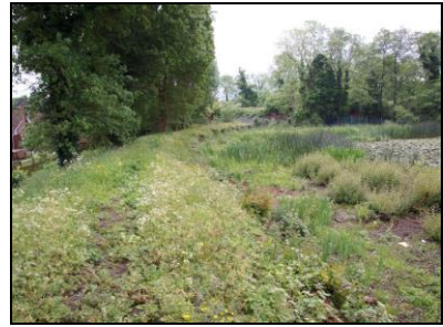
6621-0027 Dam. Facing east
