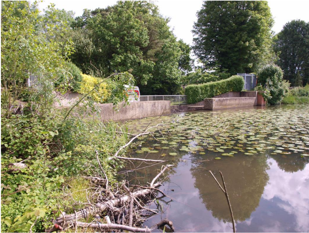
Plate 5 – Concrete spillway, looking north-east
