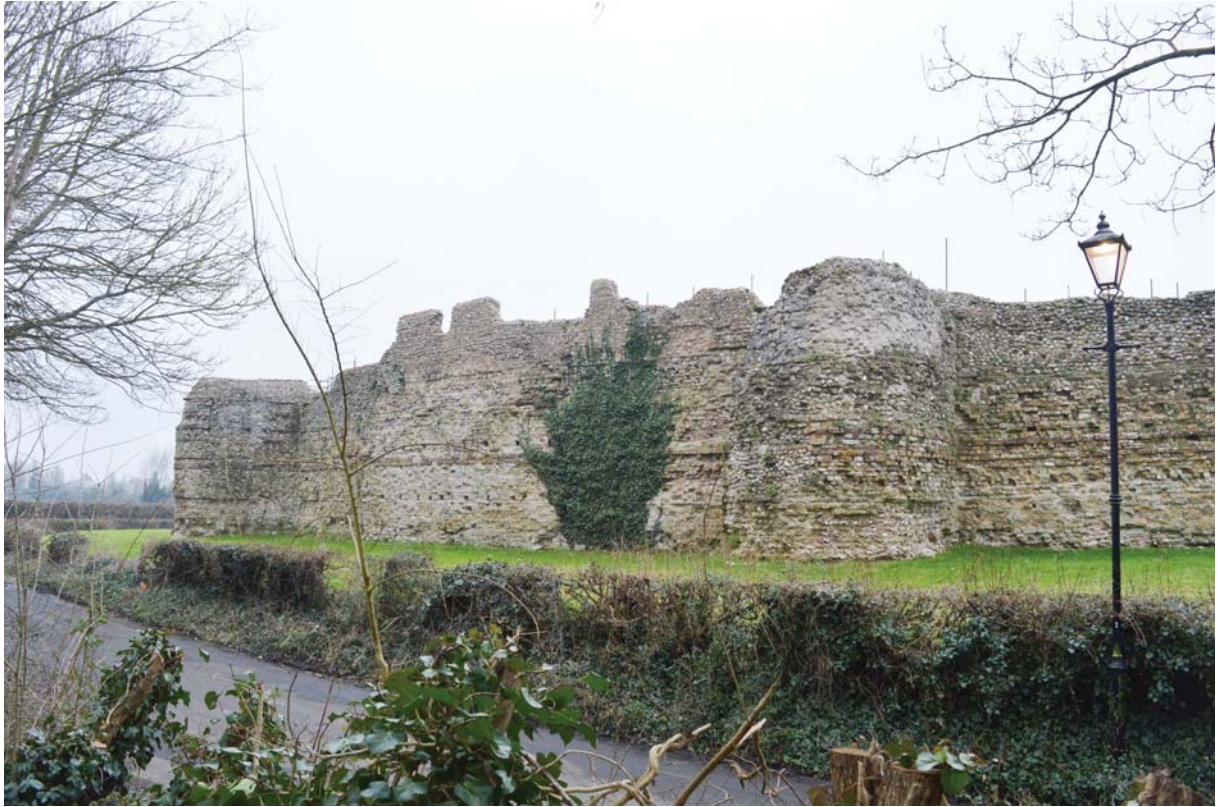
External view between bastions 4 & 5
