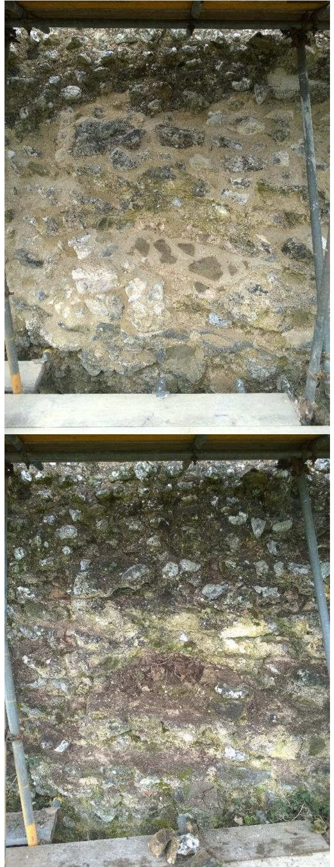
Bay 2 As Built (above) Before (below)
