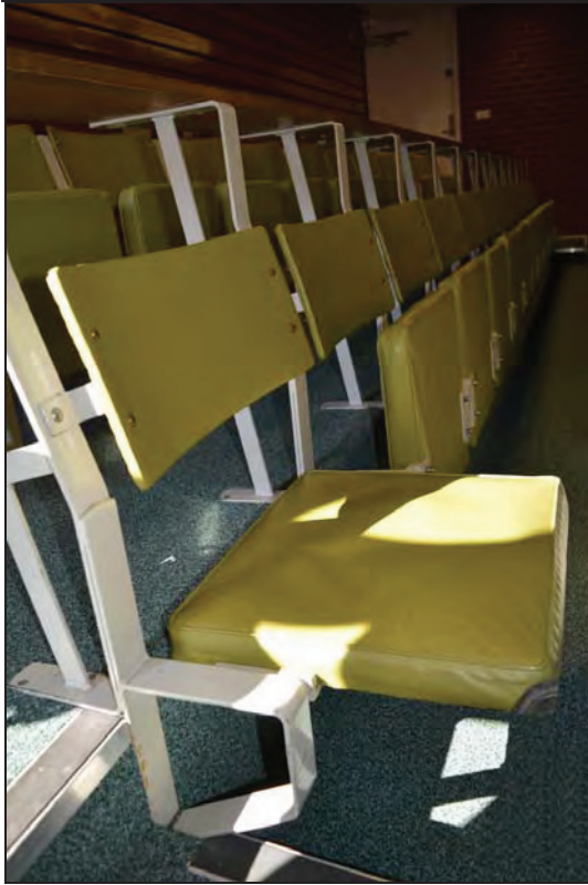
Plate 7. Shawcross Building, Lecture Theatre AS01, detail of tip-up seat in seating position, facing SE (7499-0007)
