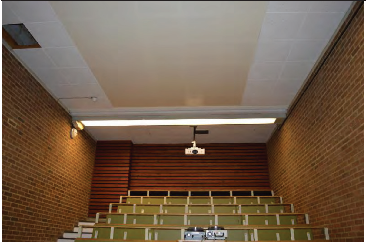
Plate 61. Arts A Building, Lecture Theatre A103, view of fibreboard ceiling panels and strip lighting, facing W (7499-0061)
