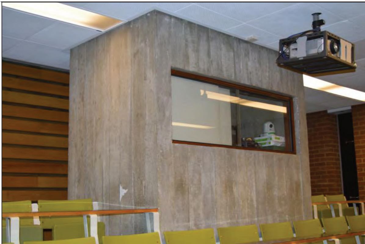
Plate 31. Shawcross Building, Lecture Theatre AS02, view of concrete projector control room, facing NW (7499-0031)
