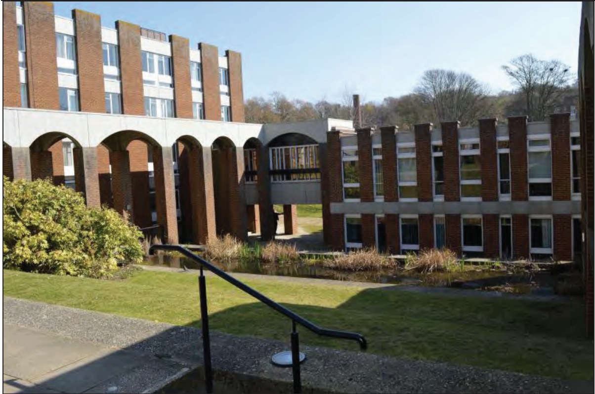
Plate 125. Arts A Building, external view of courtyard between Arts A and B Buildings, facing NE (7499-0125)
