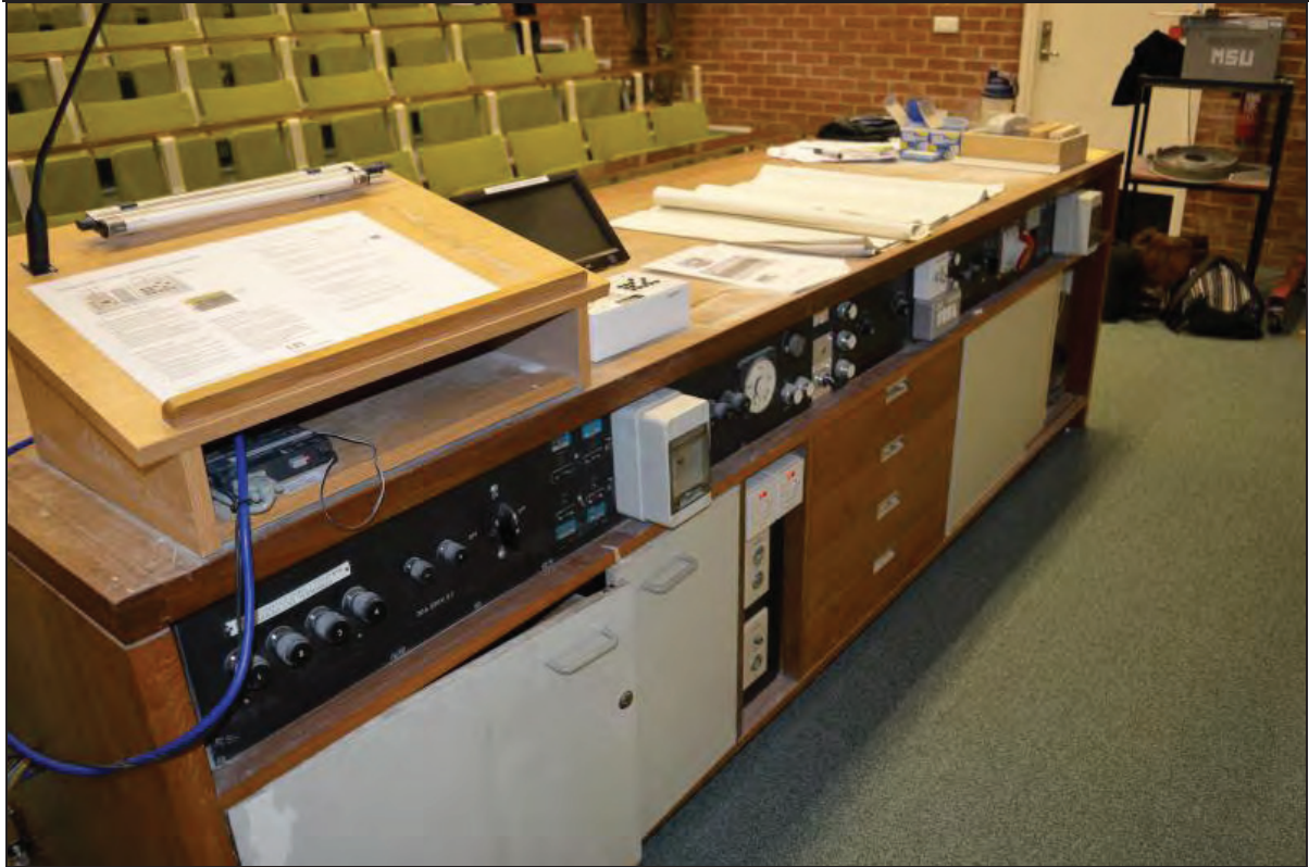
Plate 11. Shawcross Building, Lecture Theatre AS01, detail of lectern and lighting/sound equipment, facing SE (7499-0011)
