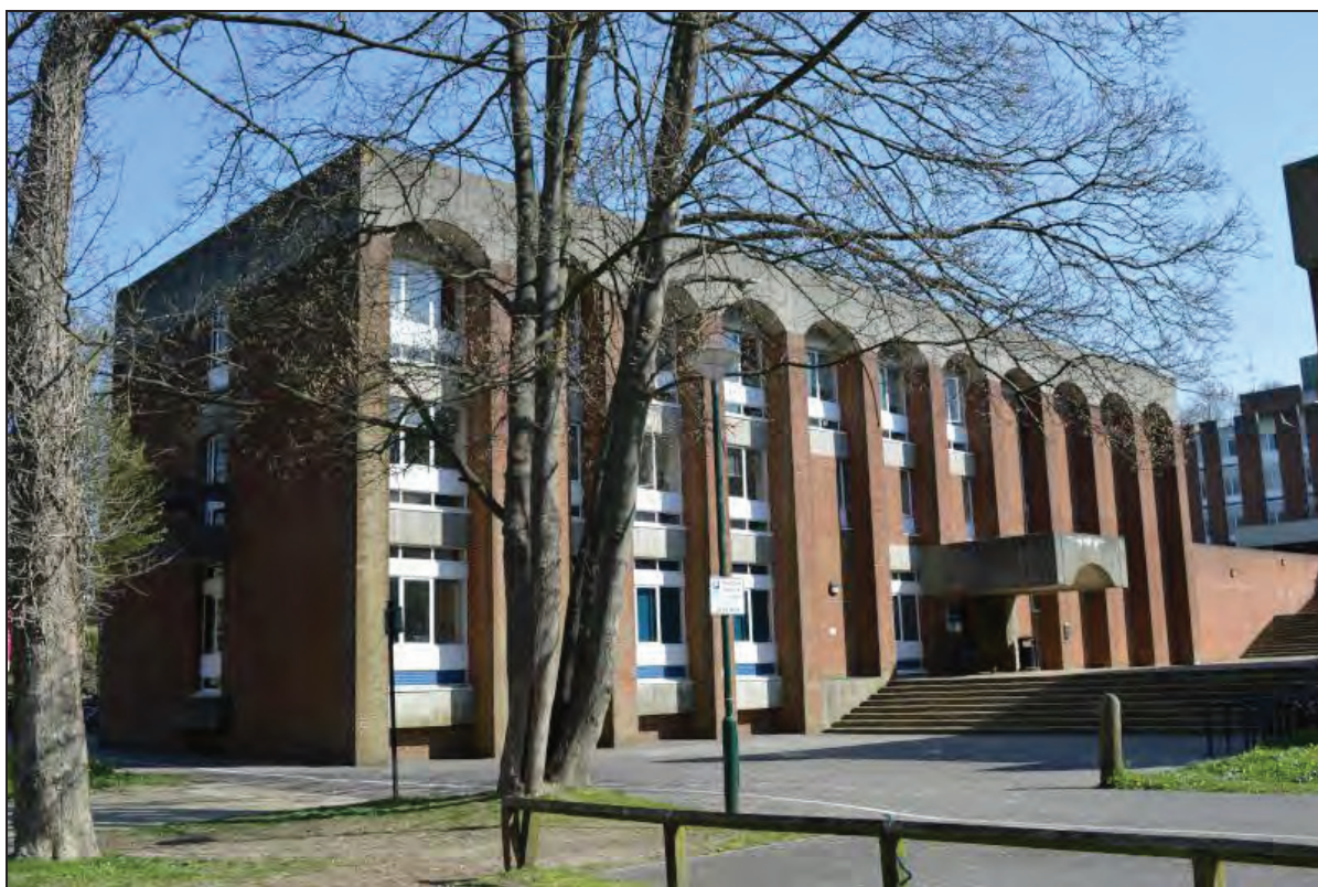
Plate 134. Shawcross Building, exterior view of arcaded southern elevation, facing NW (7499-0134)
