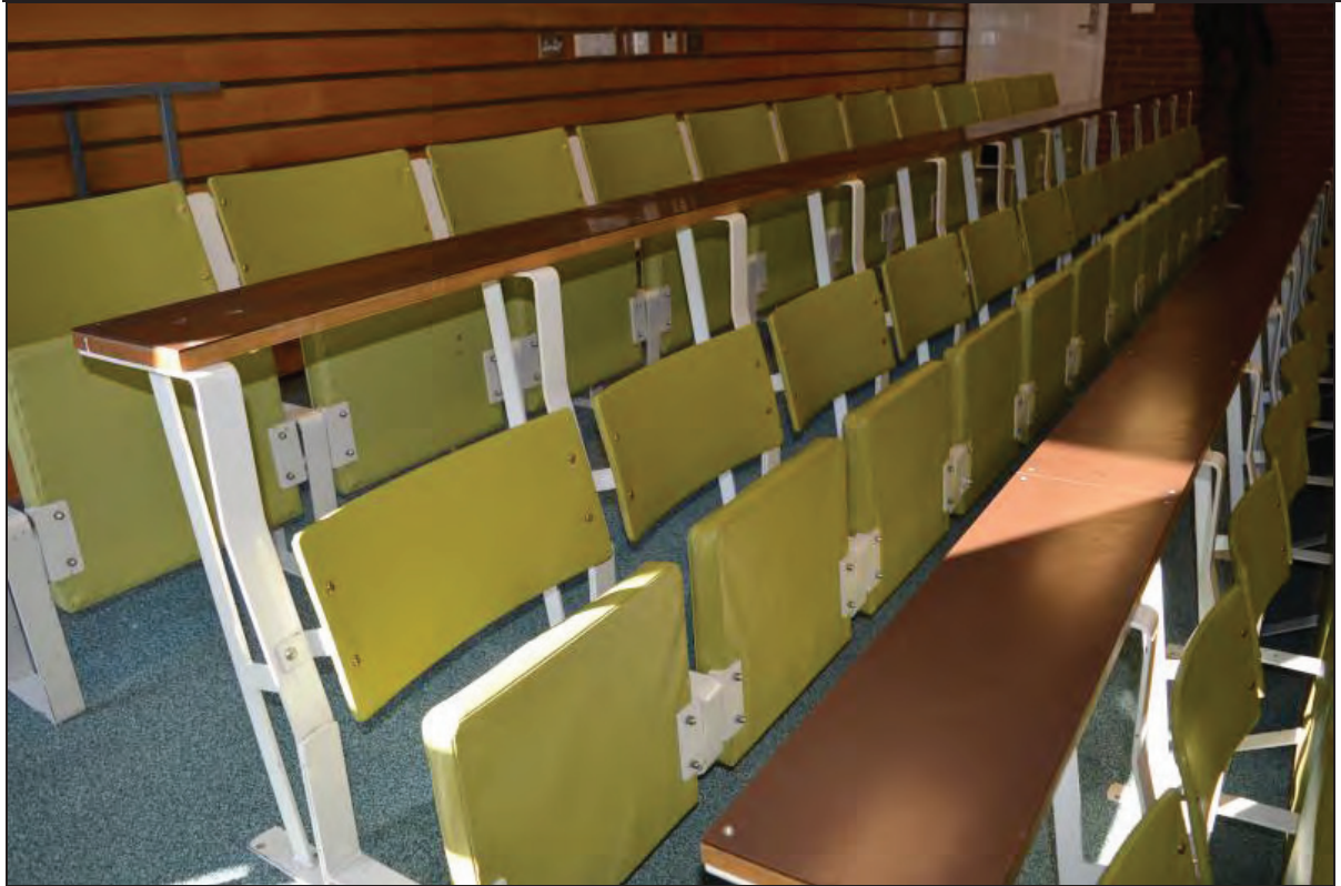
Plate 5. Shawcross Building, Lecture Theatre AS01, detail of tip-up seating and timber writing desks, facing SE (7499-0005)
