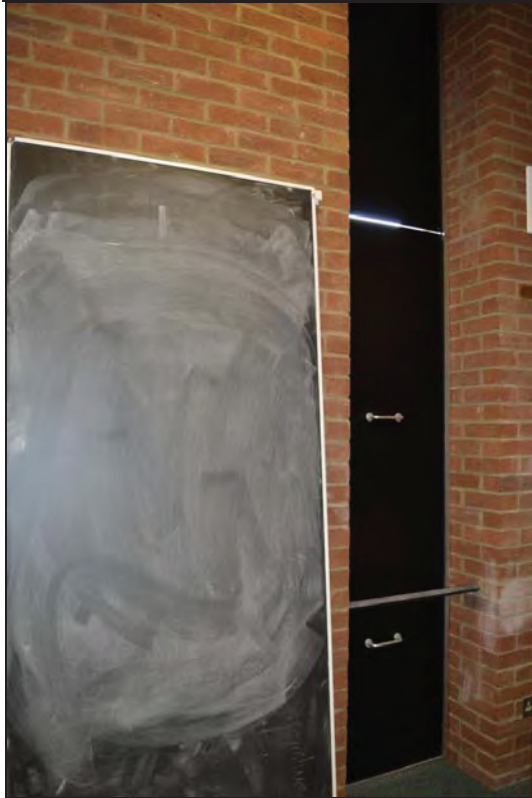
Plate 41. Shawcross Building, Lecture Theatre AS02, north-east external window (covered), facing NE (7499-0041)
