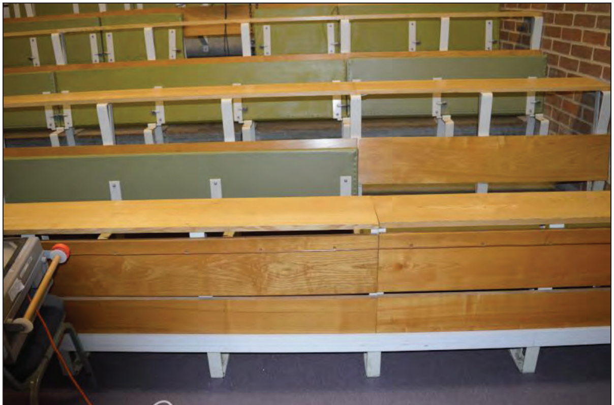
Plate 80. Arts A Building, Lecture Theatre A103, detail of timber modesty panel, facing W (7499-0080)
