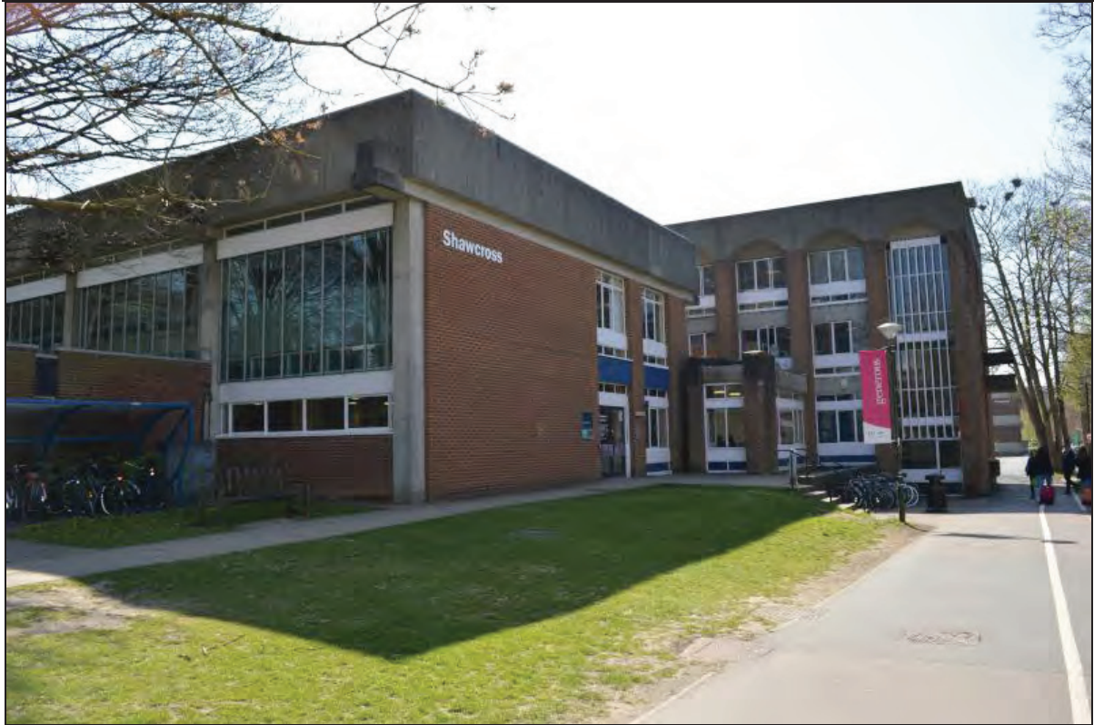
Plate 139. Shawcross Building, external view of southern elevation, facing NE (7499-0139)
