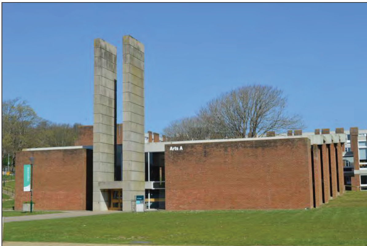
Plate 142. Arts A Building, main entrance, facing NW (7499-0142)
