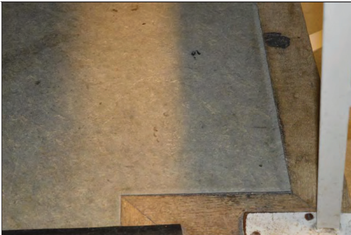
Plate 103. Arts A Building, Lecture Theatre A05, detail of timber edge of linoleum flooring under seating, facing N (7499-0103)
