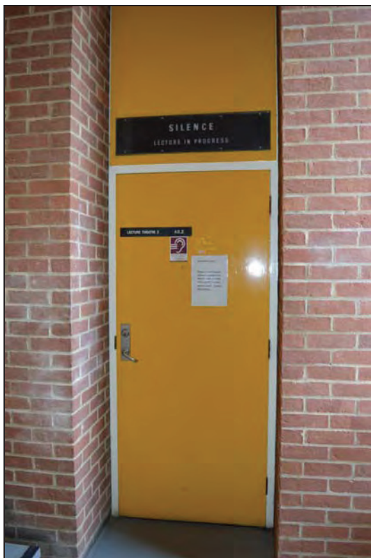
Plate 48. Shawcross Building, Lecture Theatre AS02, south-east access door, facing N (7499-0048)
