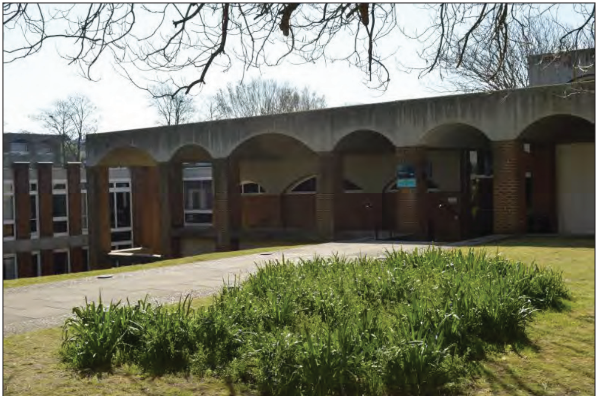
Plate 126. Arts A Building, external colonnaded walkway running to the building's northern elevation, facing SE (7499-0126)
