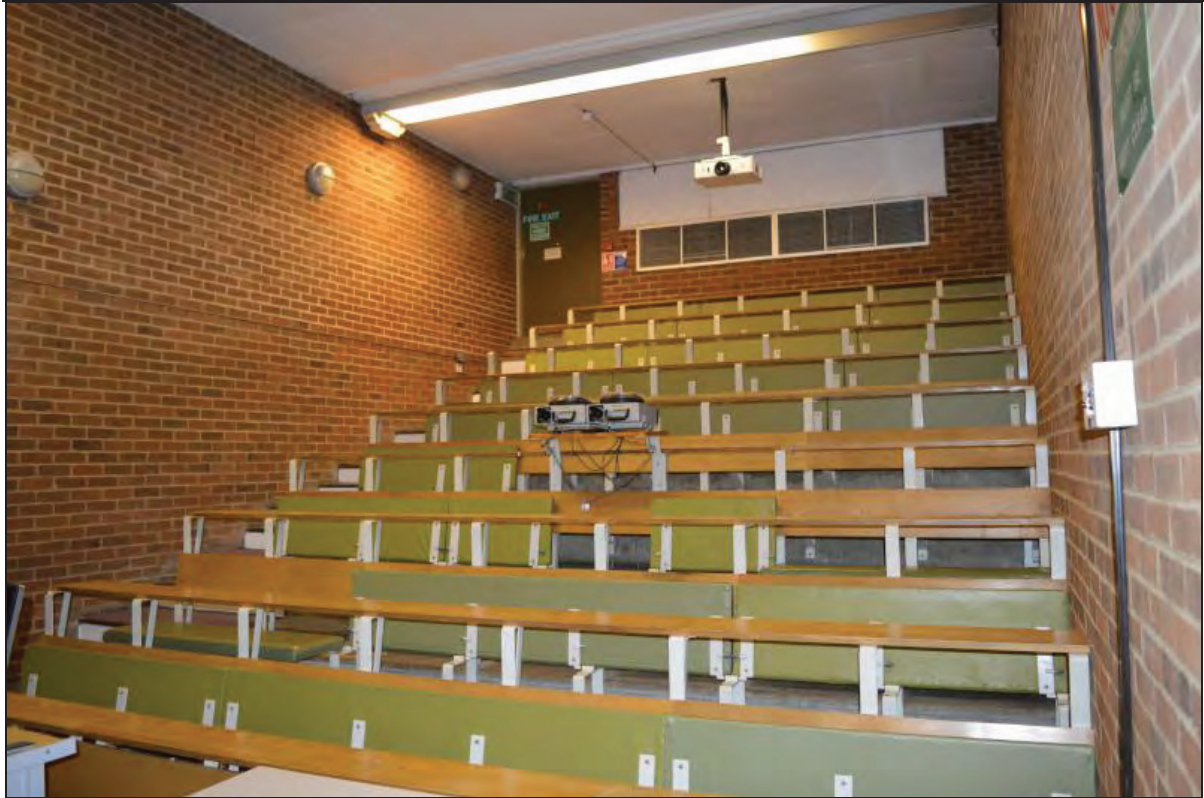
Plate 85. Arts A Building, Lecture Theatre A05, general view of theatre and rear fire exit, facing SW (7499-0085)
