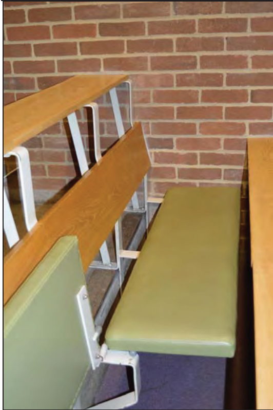
Plate 63. Arts A Building, Lecture Theatre A103, detail of tip-up bench in seating position, facing N (7499-0063)
