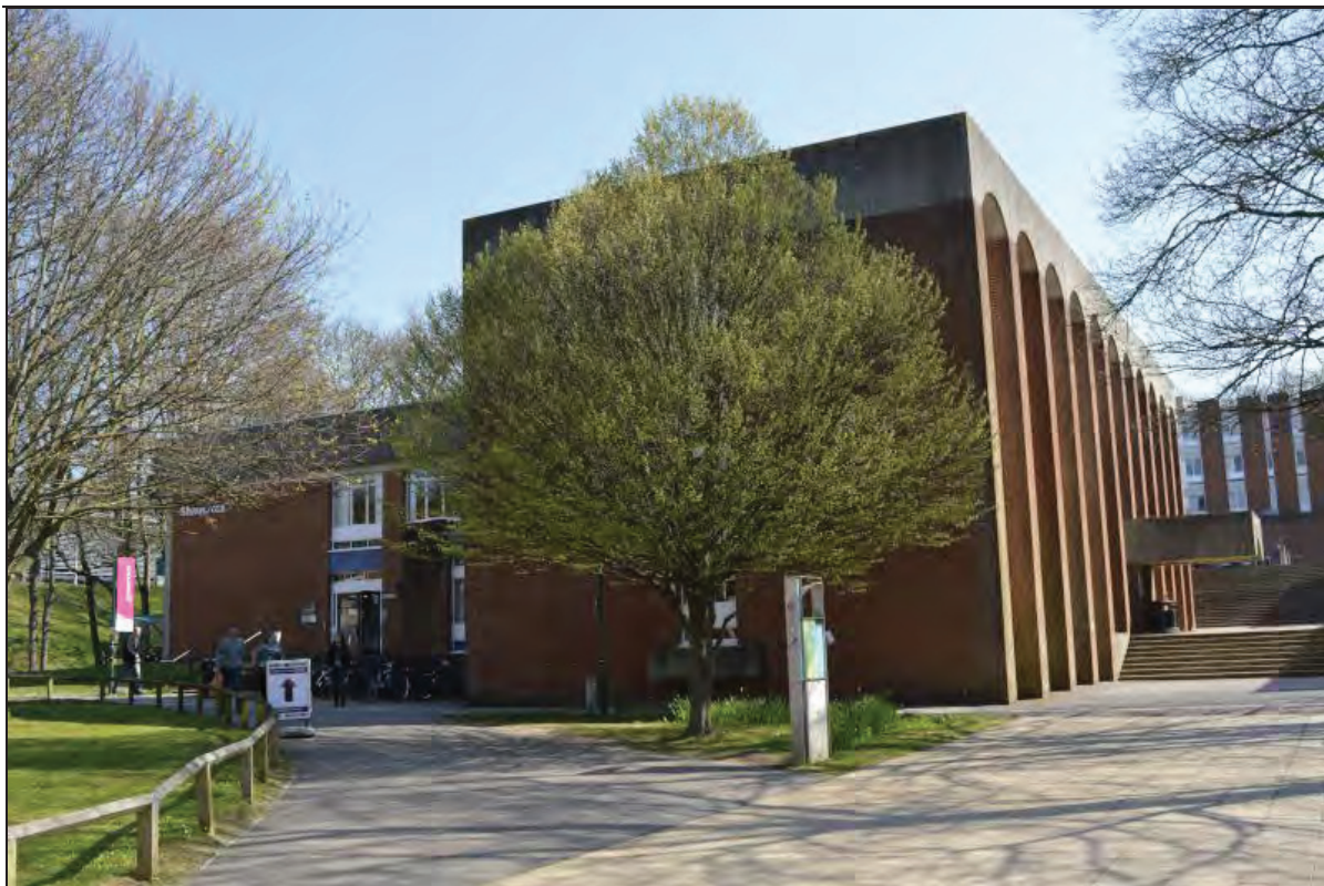
Plate 133. Shawcross Building, external view of southern elevation, facing NE (7499-0133)
