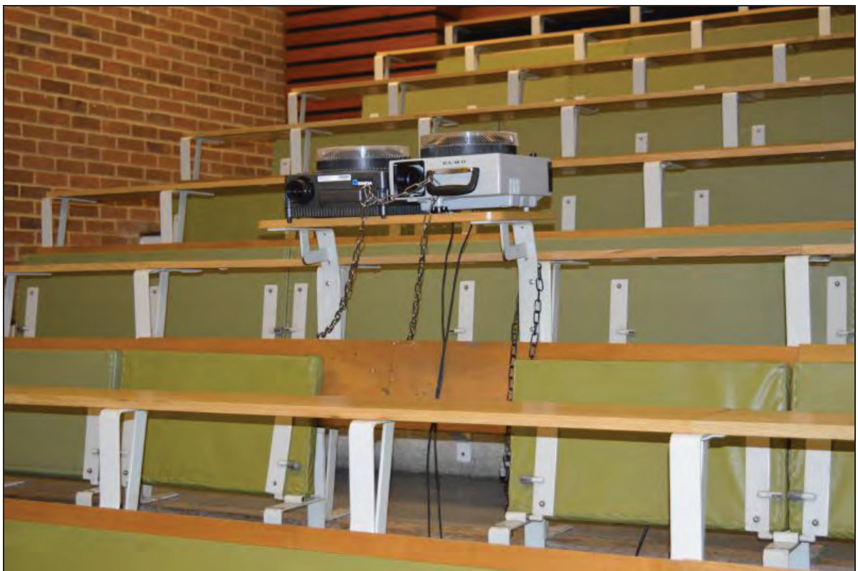
Plate 82. Arts A Building, Lecture Theatre A103, detail of desk mounted projector (note seat removal), facing SW (7499-0082)
