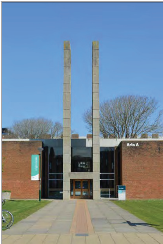
Plate 143. Arts A Building, Grade II* listed main entrance, facing N (7499-0143)
