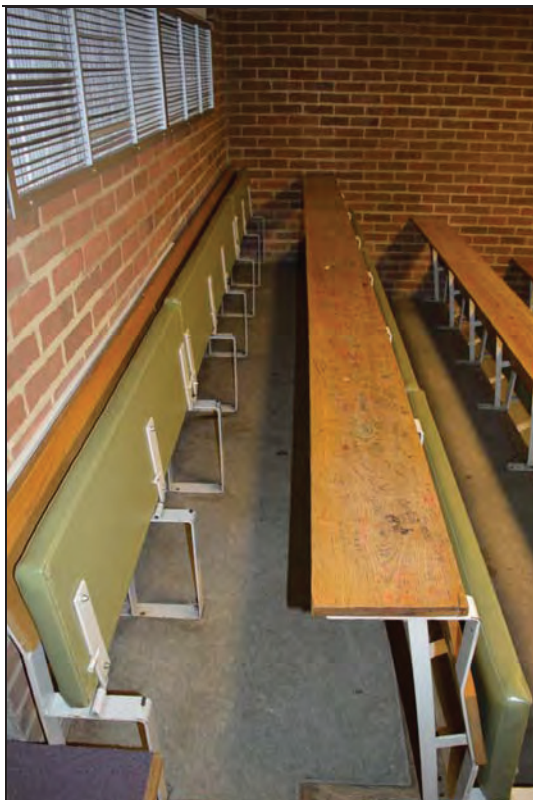
Plate 97. Arts A Building, Lecture Theatre A05, view of rear ventilation grille and graffitied timber writing desk, facing N (7499-0097)
