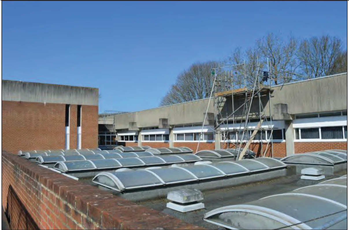
Plate 137. Shawcross Building, external view of two storey northern end, facing SW (7499-0137)
