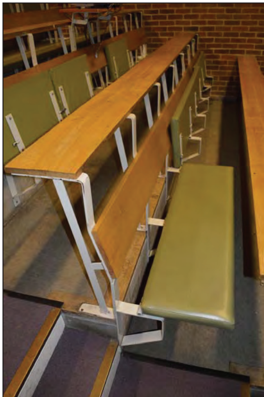
Plate 116. Arts A Building, Lecture Theatre A05, general view of seat back and bench detail in seating position, facing NW (7499-0116)
