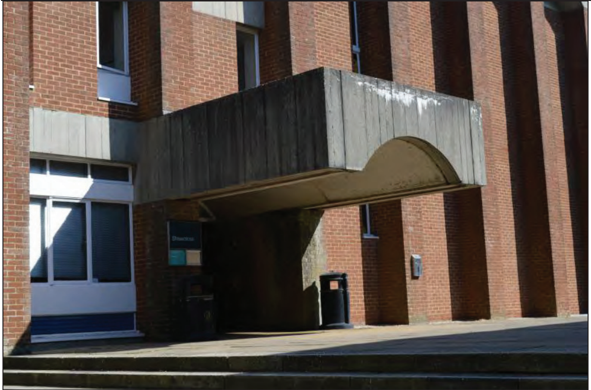
Plate 135. Shawcross Building, external southern entrance with bare-wood cast concrete porch, facing NW (7499-0135)
