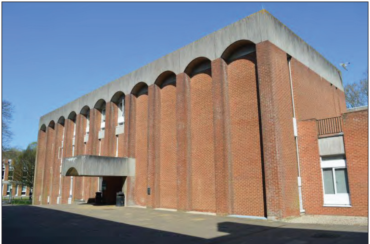
Plate 136. Shawcross Building, external view of southern elevation, facing SW (7499-0136)
