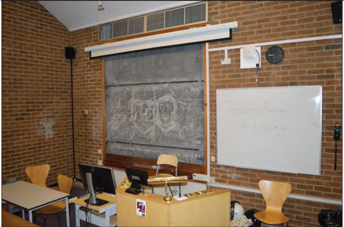
Plate 117. Arts A Building, Lecture Theatre A05, general view of theatre front, facing NE (7499-0117)
