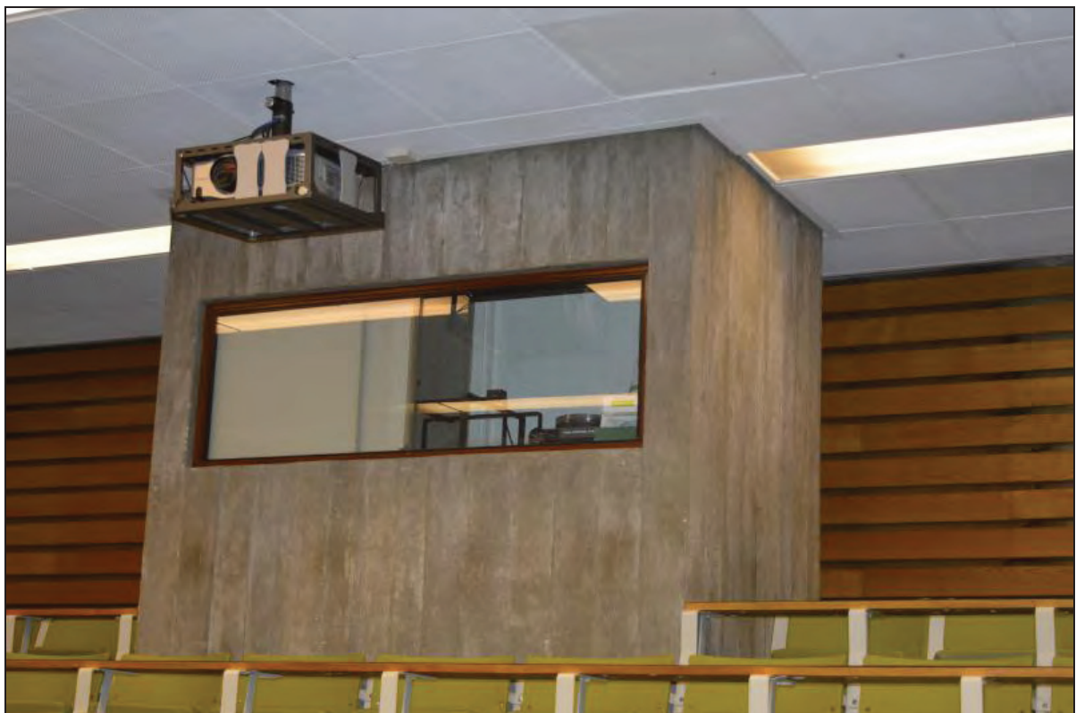
Plate 42. Shawcross Building, Lecture Theatre AS02, view of projector control room and ceiling projector fitting, facing SW (7499-0042)
