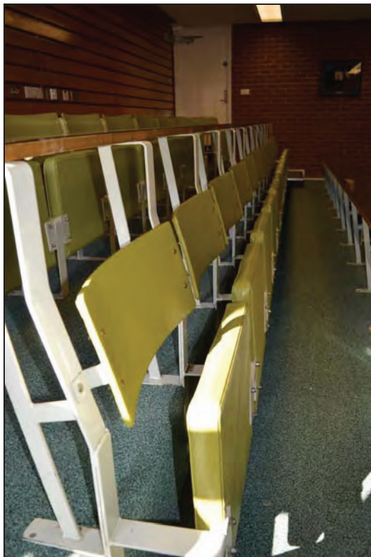
Plate 6. Shawcross Building, Lecture Theatre AS01, detailed view of tip-up seating and metal frame arrangement, facing SE (7499-0006)
