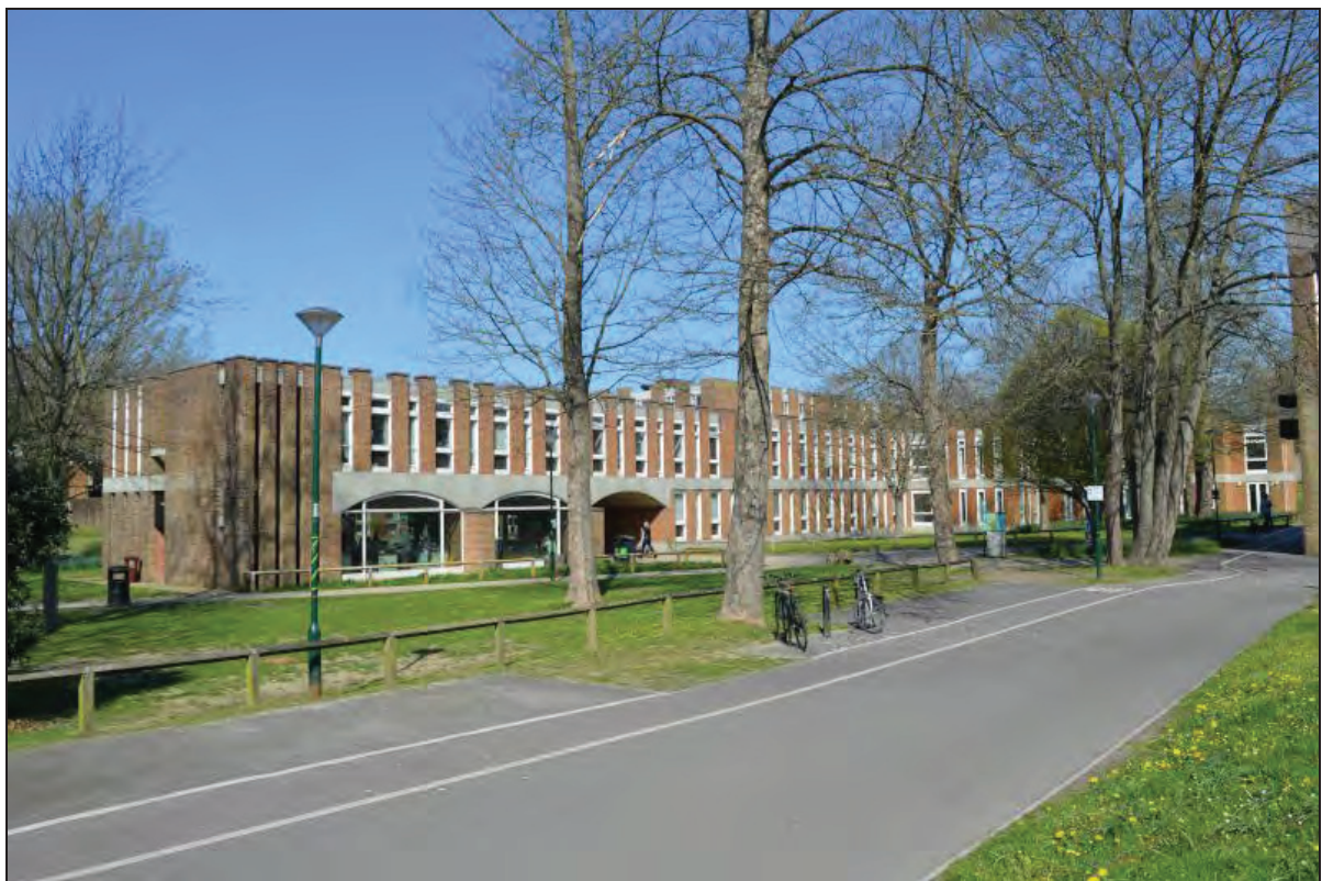
Plate 140. Arts A Building, general external view of eastern range, facing NW (7499-0140)
