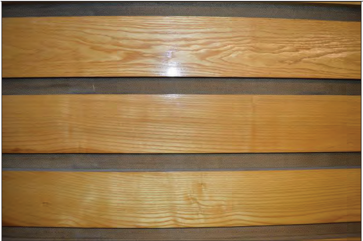
Plate 47. Shawcross Building, Lecture Theatre AS02, close-up detail of timber cladding cover to rear wall, facing W (7499-0047)
