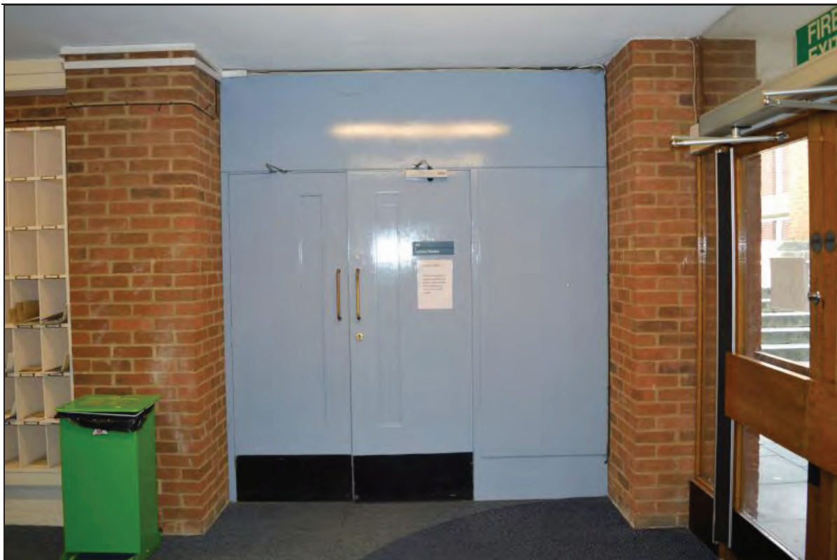
Plate 83. Arts A Building, Lecture Theatre A05, internal access door, facing N (7499-0083)
