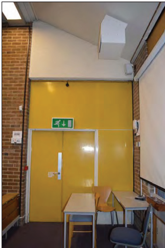
Plate 58. Arts A Building, Lecture Theatre A103, external access door, facing N (7499-0058)
