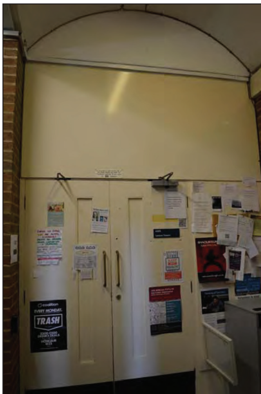
Plate 56. Arts A Building, Lecture Theatre A103, internal access door, facing N (7499-0056)
