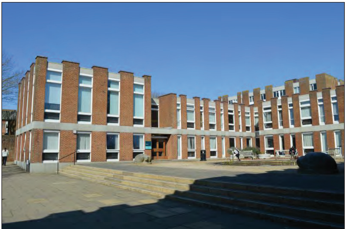
Plate 120. Arts A Building, external view of raised seating area around principal entrance, facing NW (7499-0120)
