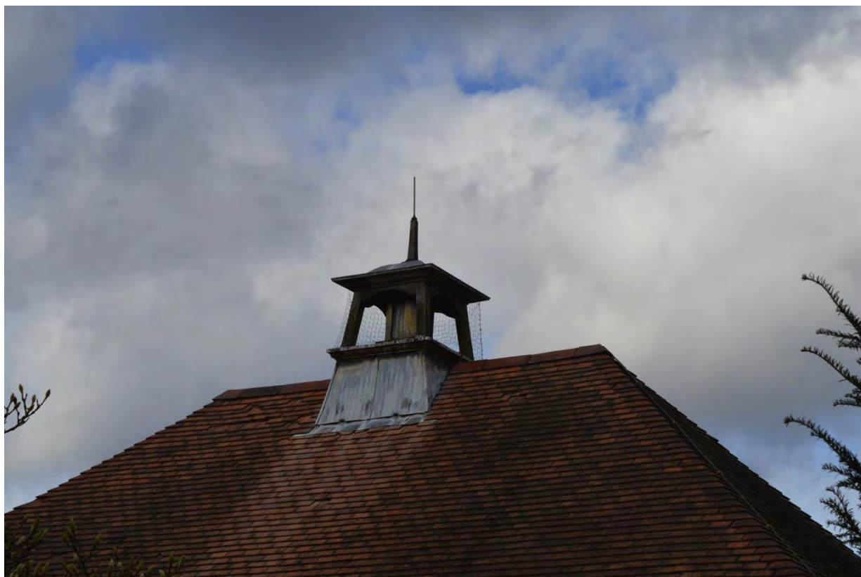
Plate 27: Building 7, detail of timber cupola with lead dressings, facing north-east (7335_0014)
