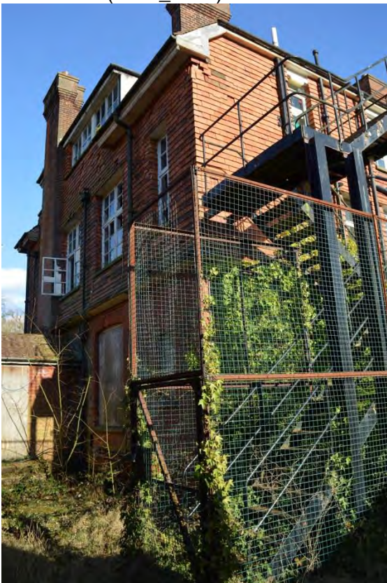
Plate 54: Building 10, view of north-west elevation, facing south-east (7335_0045)
