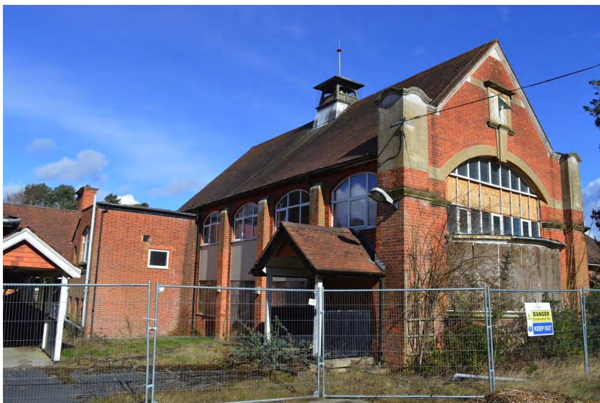
Plate 16: Building 6, view of south and west elevations, facing north-east (7335_0026)
