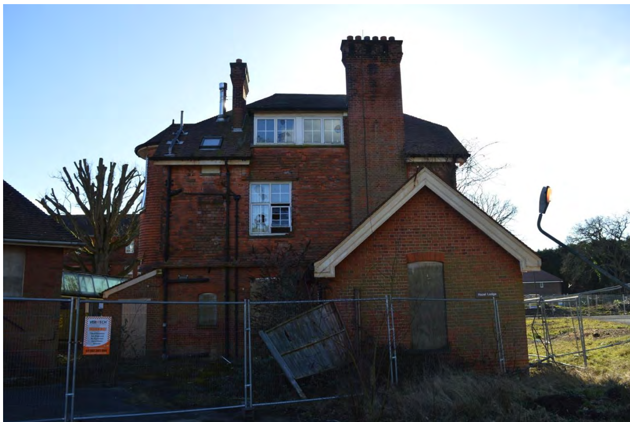
Plate 35: Building 9, view of the north-east elevation, facing south-west (7335_0039)
