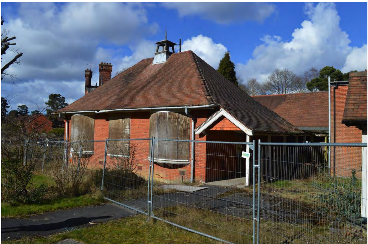
Plate 26: Building 8, view of south-east corner, facing north-west (7335_0029)
