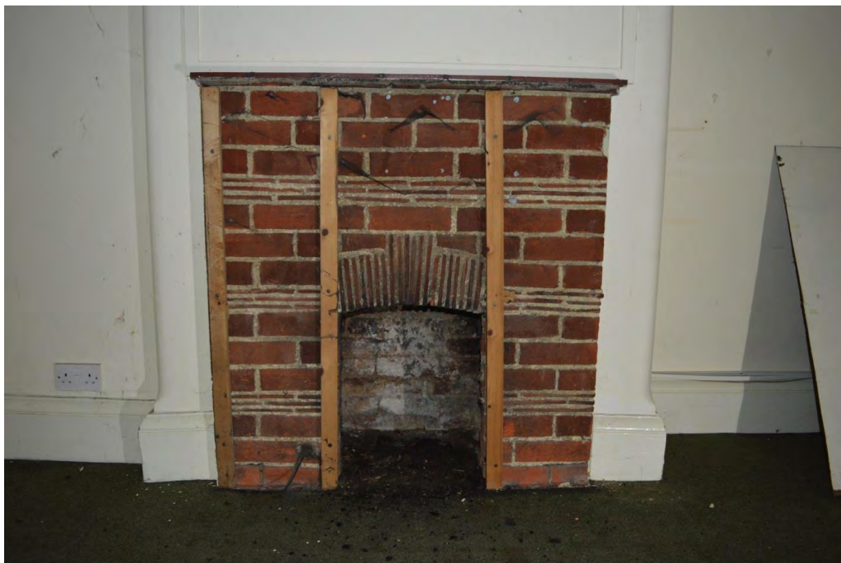
Plate 60: Building 10, ground floor, Room 5, fireplace detailing, facing south-west (7335_0062)
