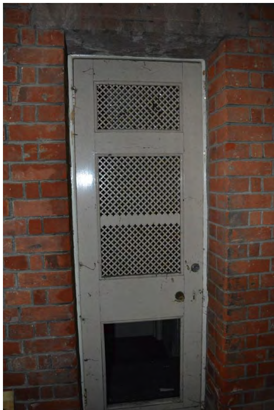
Plate 23: Building 6, detail of external basement entrance, facing south (7335_0132)
