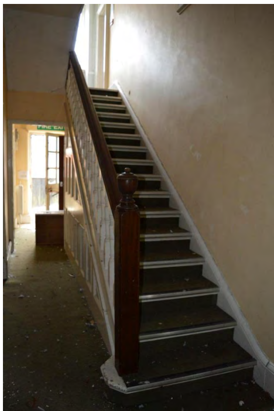
Plate 63: Building 10, ground floor, view of hallway and staircase, facing north-west (7335_0069)
