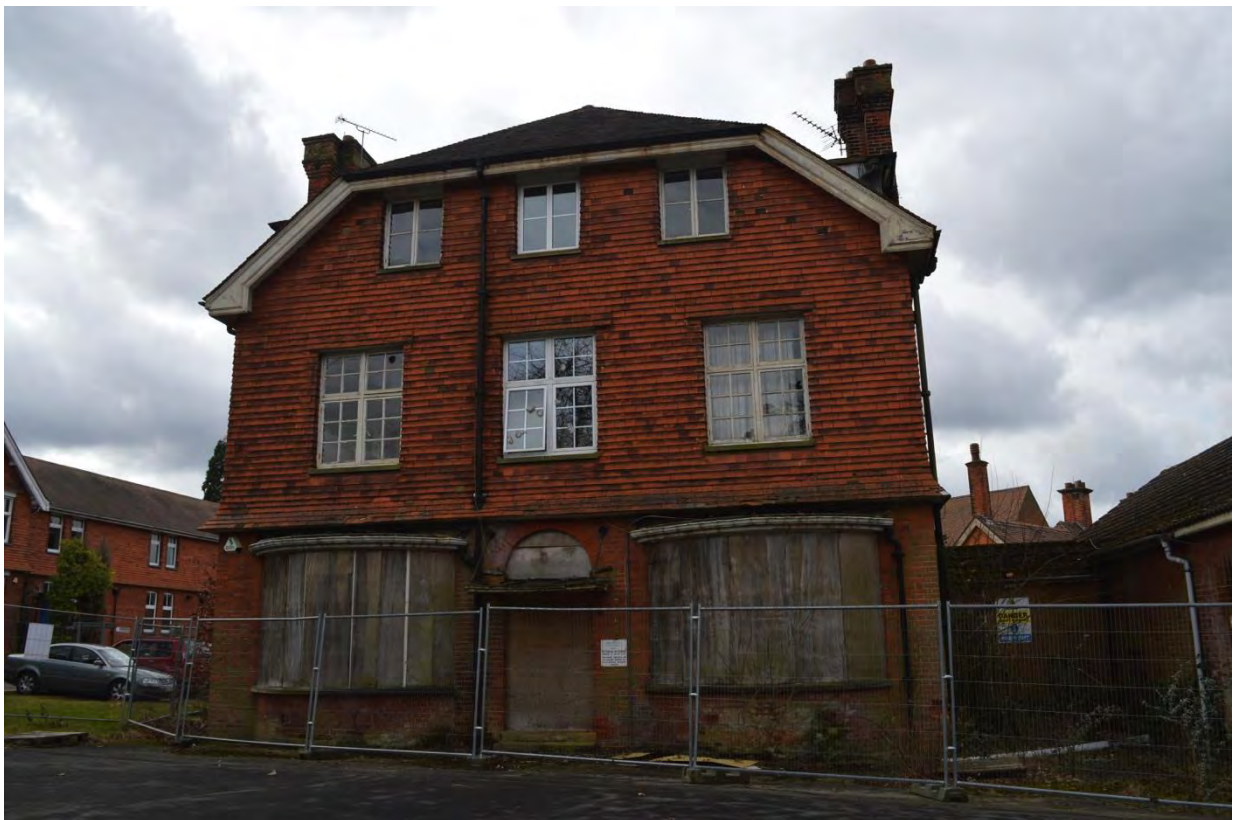
Plate 52: Building 10, view of principal north-east elevation, facing south-west (7335_0005)
