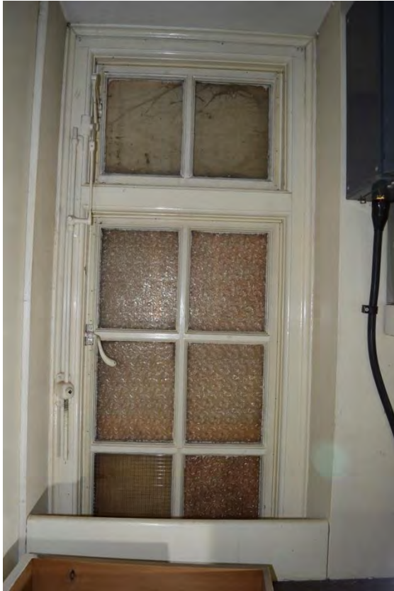
Plate 61: Building 10, ground floor, Room 6, original window detail, facing south-west (7335_0064)
