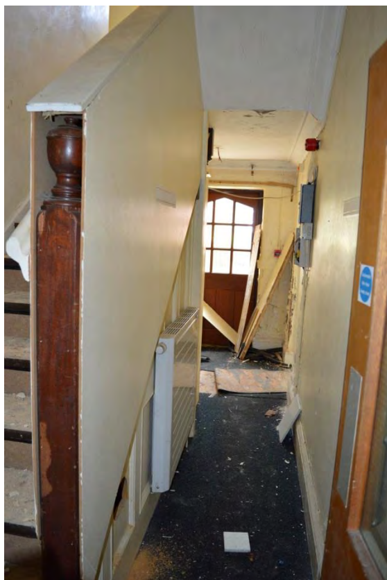
Plate 43: Building 9, ground floor, secondary hallway and stair detail, facing east (7335_0143)
