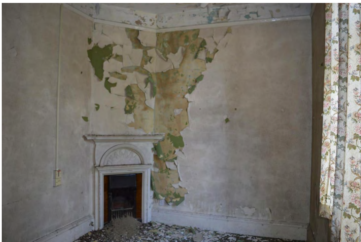
Plate 66: Building 10, first floor, Room 13 layout, facing north-west (7335_0077)
