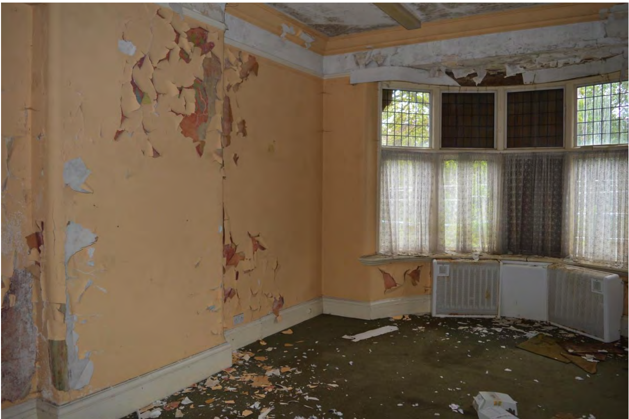
Plate 58: Building 10, ground floor, Room 2 arrangement, facing north-east (7335_0056)
