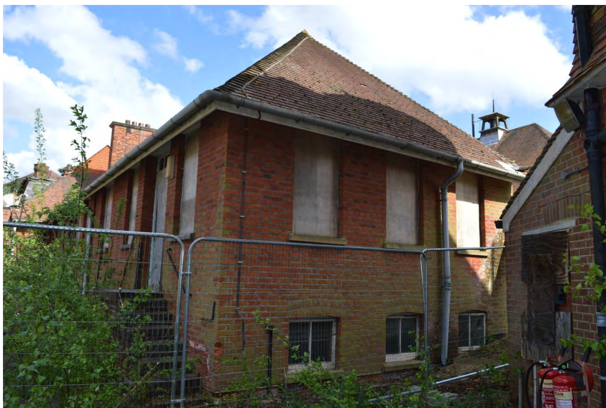
Plate 4: Building 5, arrangement of west elevation, facing south-east (7335_0174)
