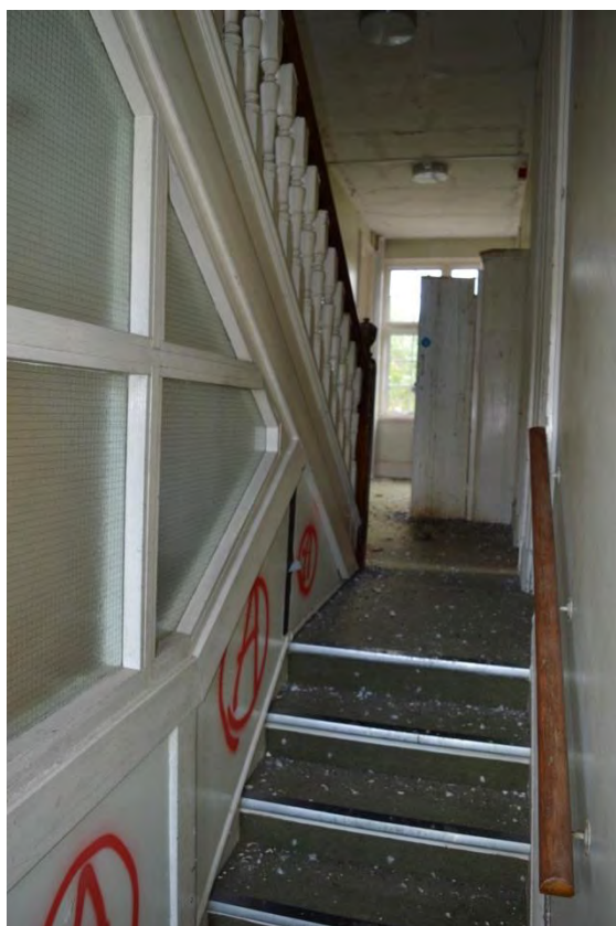
Plate 64: Building 10, first floor, upper landing arrangement, facing north-west (7335_0072)
