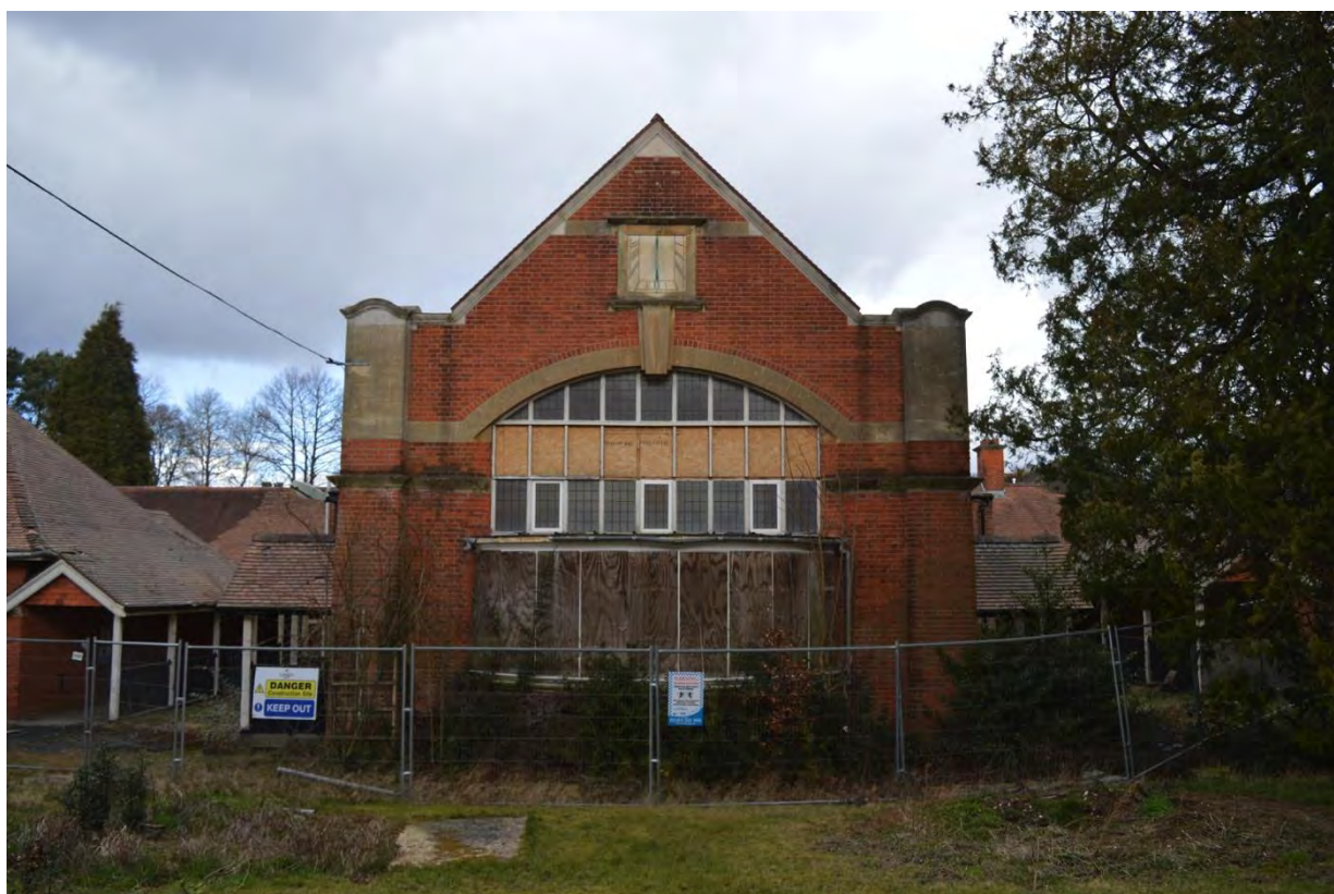
Plate 18: Building 6, view of principal south elevation, facing north (7335_0021)
