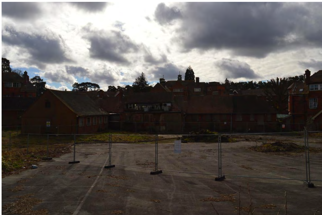
Plate 1: Building 5, arrangement of north elevation, facing south (7335_0002)
