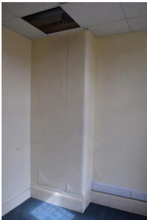
Plate 39: Building 9, ground floor, Room 1, truncated chimney stack, facing south-east (7335_0147)
