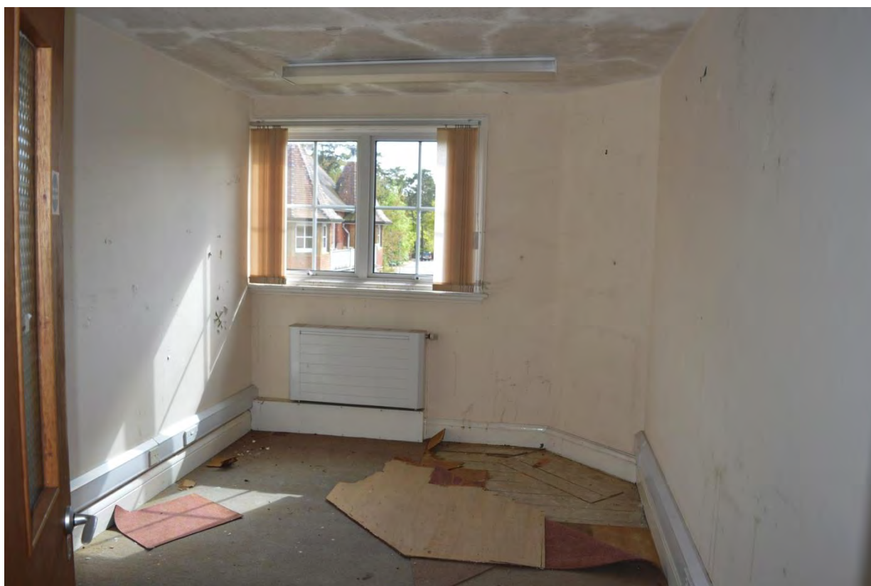
Plate 50: Building 9, attic, Room 22 arrangement, note the corner chimneystack, facing south (7335_0170)
