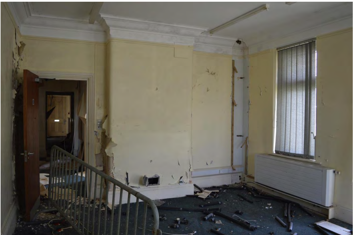
Plate 42: Building 9, ground floor, Room 7, north-west extension, facing south-west (7335_0154)
