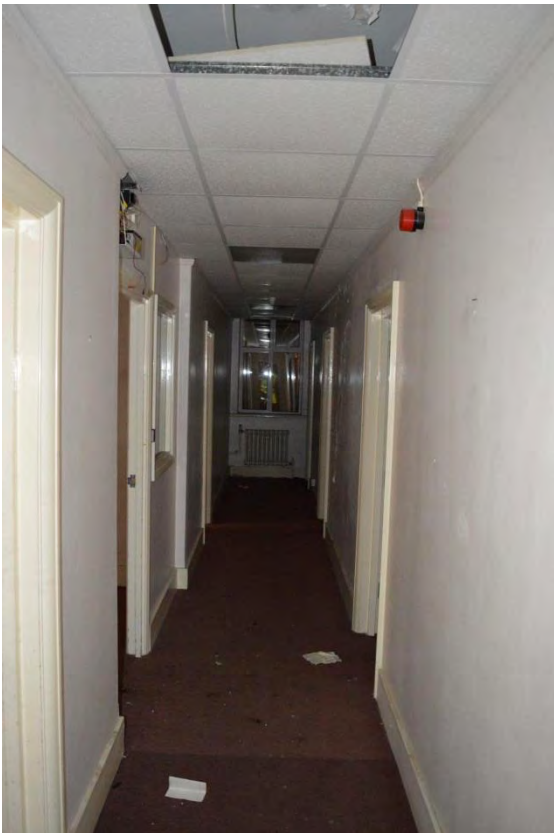
Plate 72: Building 11, ground floor, view of central access corridor, facing south-west (7335_0085)
