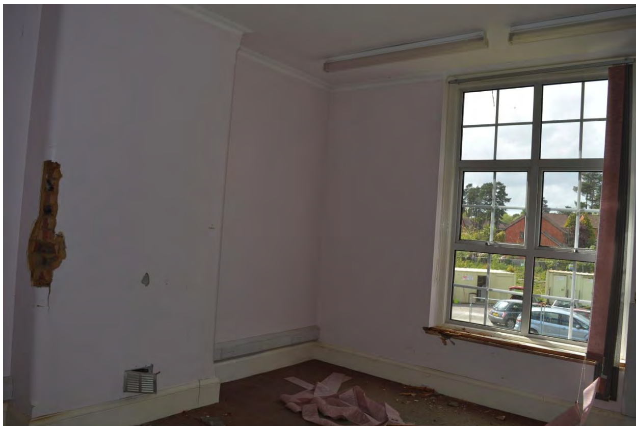
Plate 47: Building 9, first floor, Room 15 layout, facing south-west (7335_0159)
