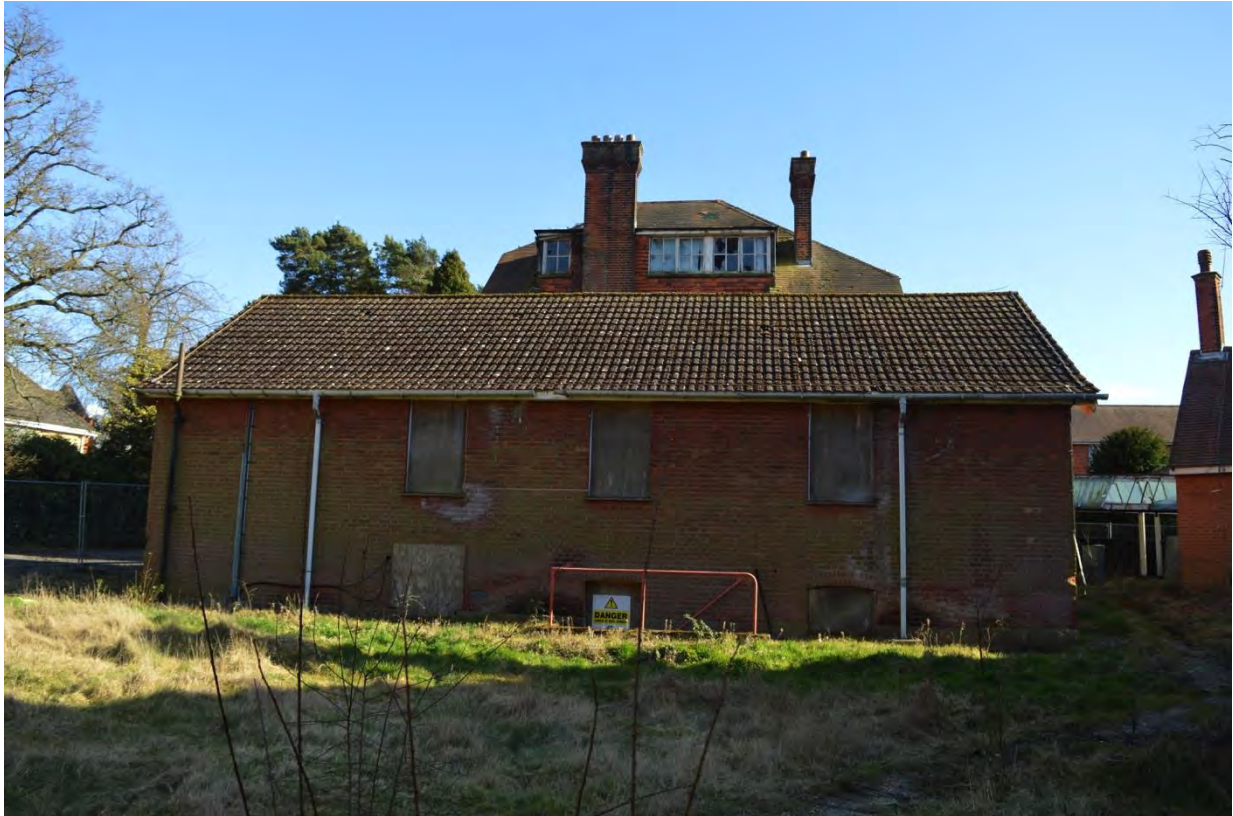
Plate 69: Building 11, view of north-west elevation, facing south-east (7335_0043)
