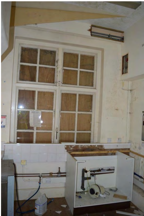
Plate 62: Building 10, ground floor, Room 7 layout, facing north-west (7335_0065)
