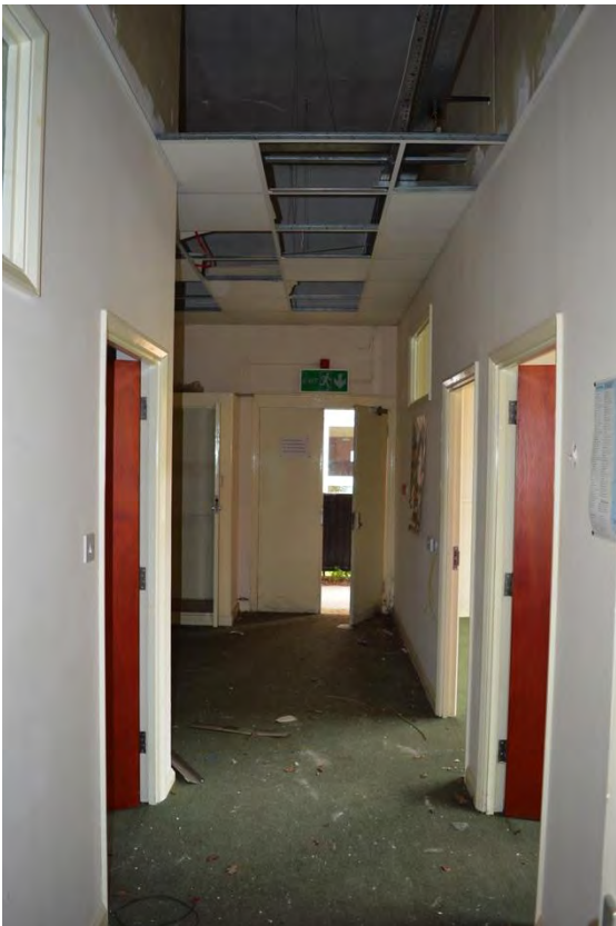
Plate 30: Building 8, ground floor, view of central corridor, facing east (7335_0116)
