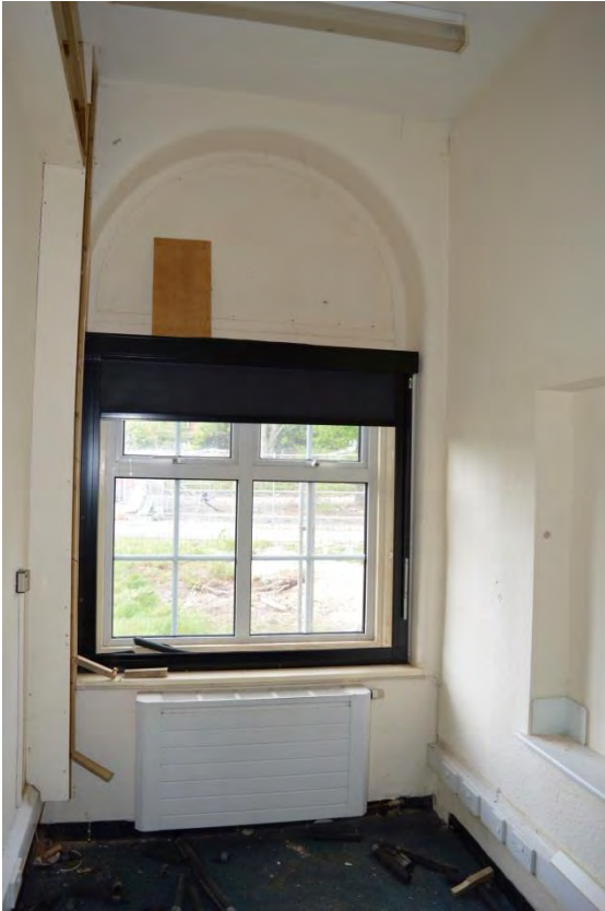
Plate 41: Building 9, ground floor, Room 4, original entrance, facing north-west (7335_0150)
