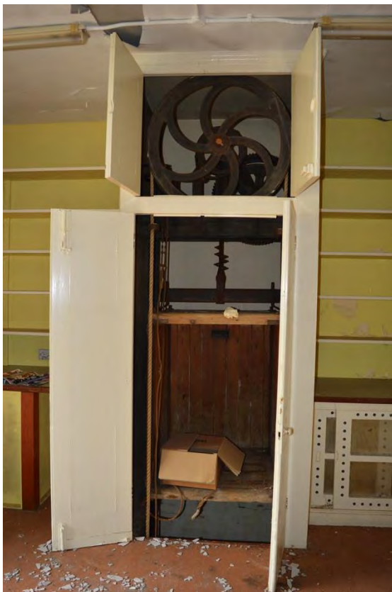
Plate 14: Building 5, ground floor, Room 13, detail of dumb-waiter mechanism, facing east (7335_0109)
