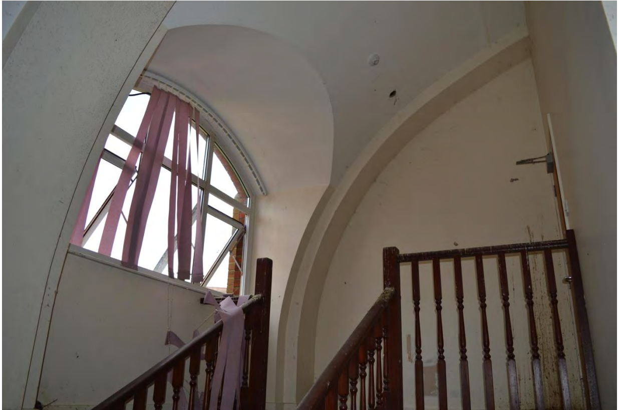
Plate 21: Building 6, first floor stairwell, detail of arched plaster ceiling obscured by later insertions, facing south-east (7335_0136)
