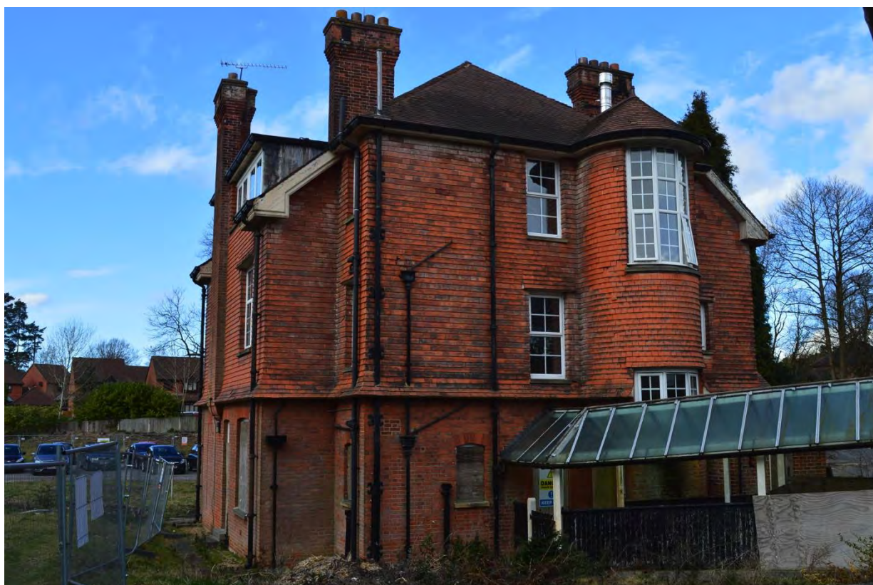
Plate 36: Building 9, view of the south-east elevation, facing north-west (7335_0038)
