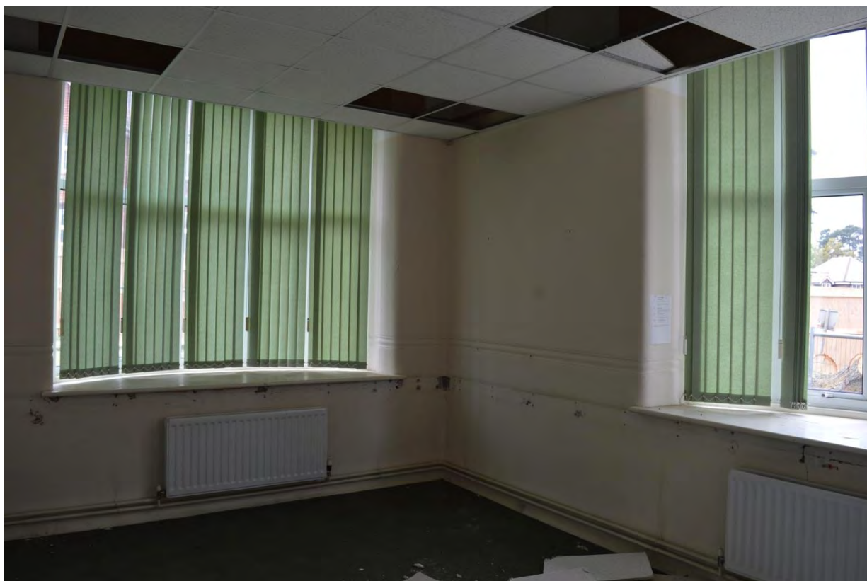
Plate 31: Building 8, ground floor, view of far western partition, facing south-west (7335_0117)
