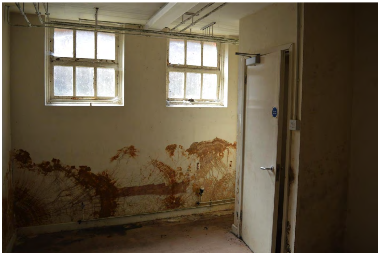
Plate 24: Building 6, basement, detail of far west room, facing west (7335_0138)
