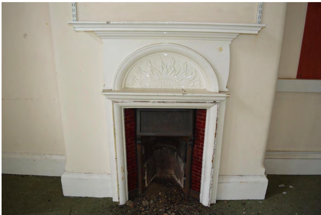
Plate 65: Building 10, first floor, Room 11, fireplace detailing, facing south-west (7335_0074)
