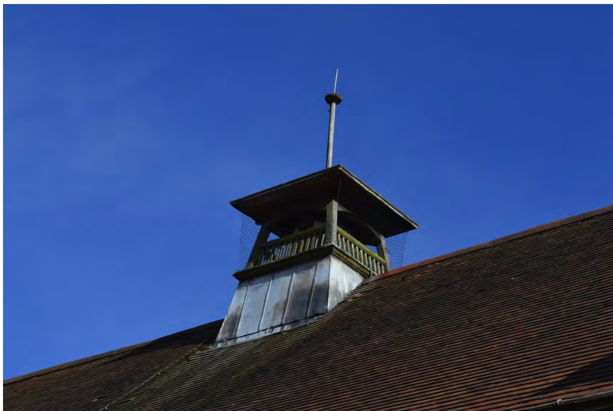
Plate 17: Building 6, detail of timber cupola with lead dressings, facing north-east (7335_0028)
