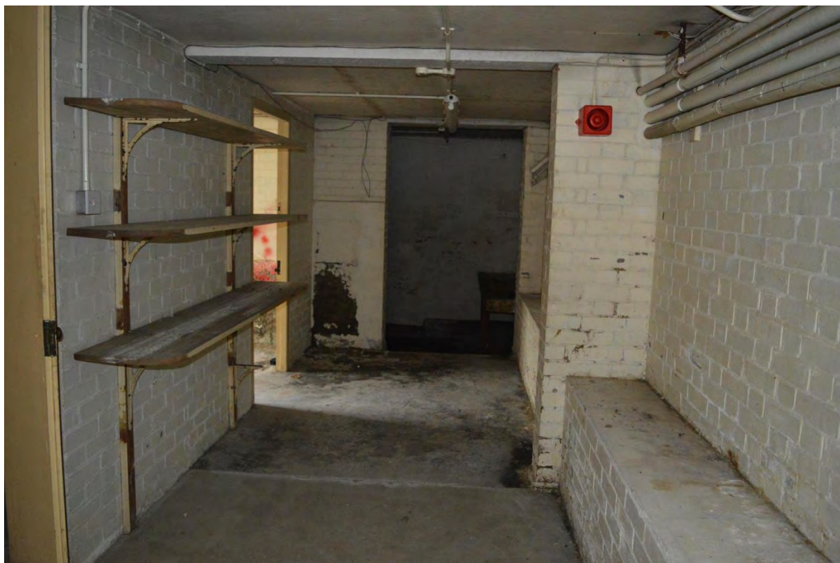
Plate 15: Building 5, basement, access corridor, facing east (7335_0113)
