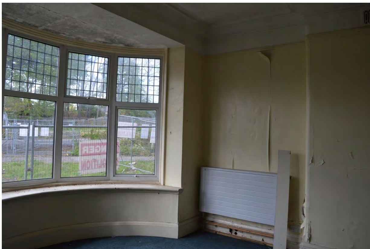
Plate 40: Building 9, ground floor, Room 5 layout, facing north-west (7335_0153)
