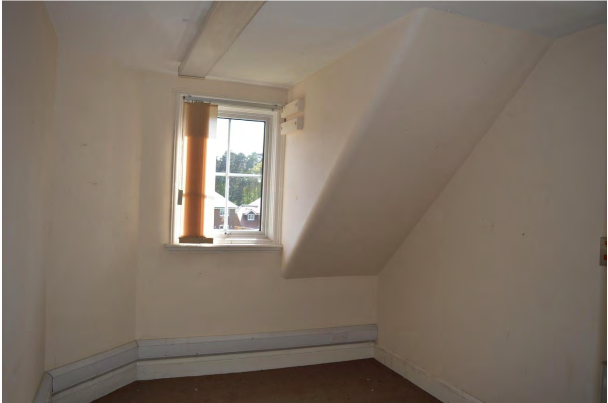
Plate 51: Building 9, attic, Room 24 arrangement, facing south-west (7335_0172)
