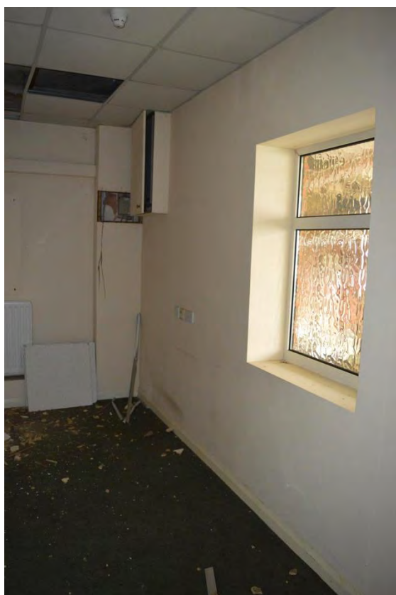
Plate 32: Building 8, ground floor, northern extension, facing north-east (7335_0119)
