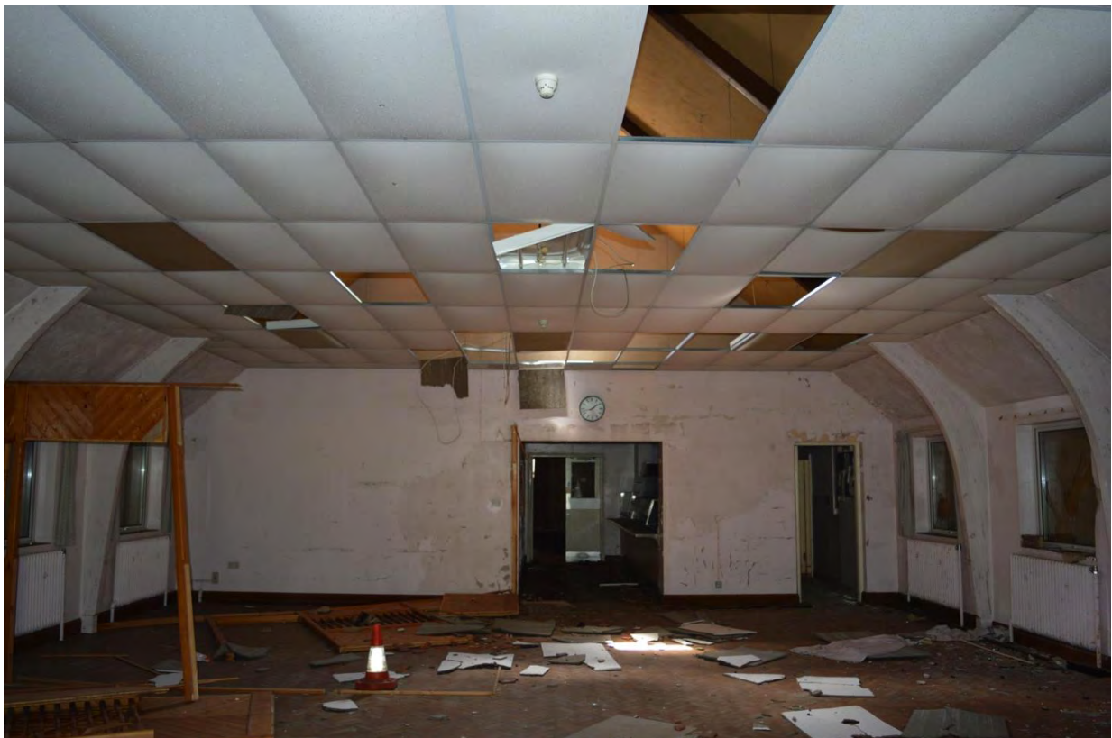
Plate 8: Building 5, ground floor, Room 7 layout, facing south (7335_0095)
