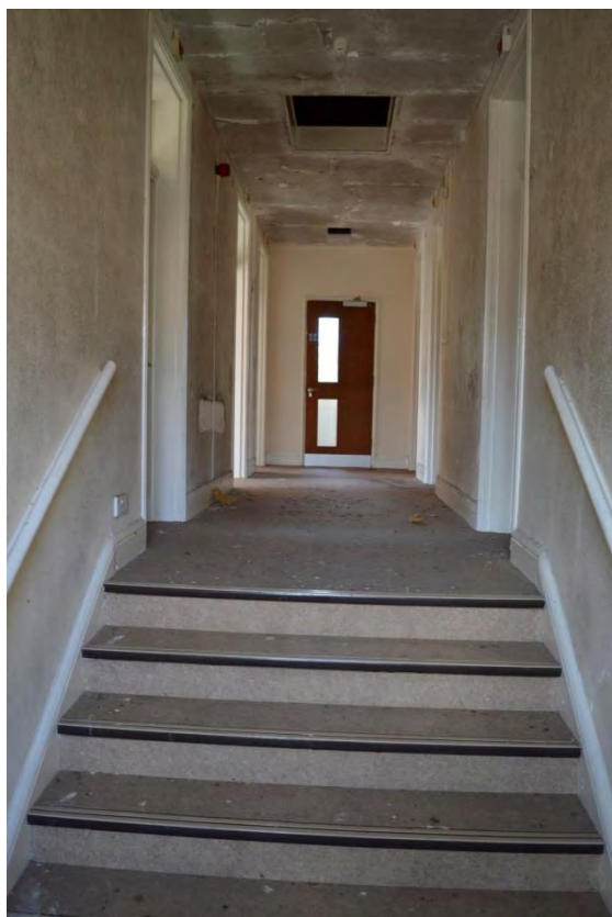
Plate 48: Building 9, attic, upper landing layout, facing south-west (7335_0168)
