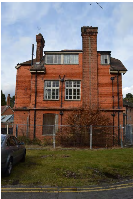
Plate 55: Building 10, view of south-east elevation, facing north-west (7335_0011)
