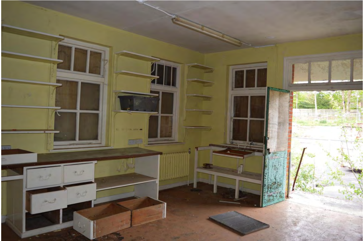
Plate 13: Building 5, ground floor, Room 13 arrangement, facing north-west (7335_0107)
