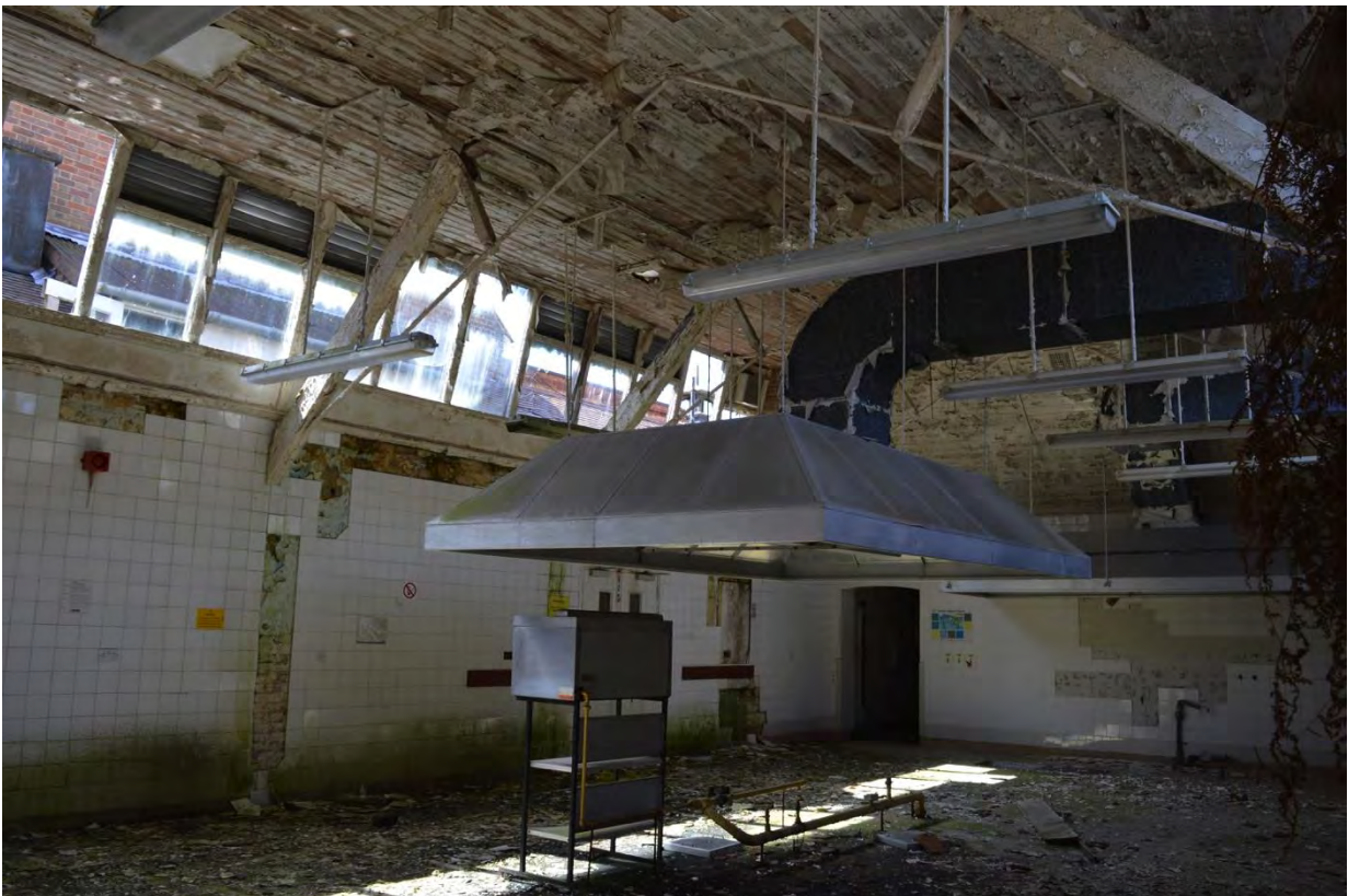
Plate 10: Building 5, ground floor, Room 8 layout, facing south-west (7335_0099)
