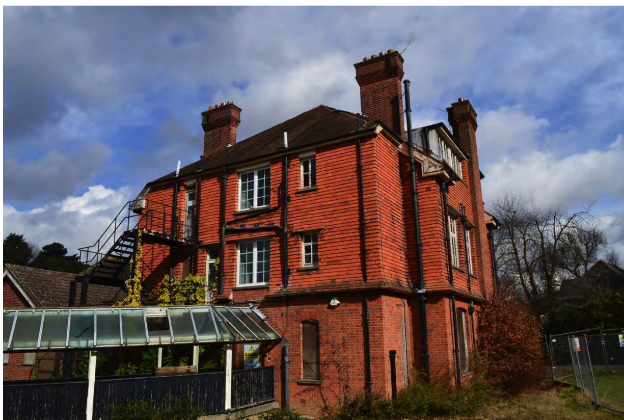
Plate 56: Building 10, view of south-west elevation, facing north-east (7335_0012)
