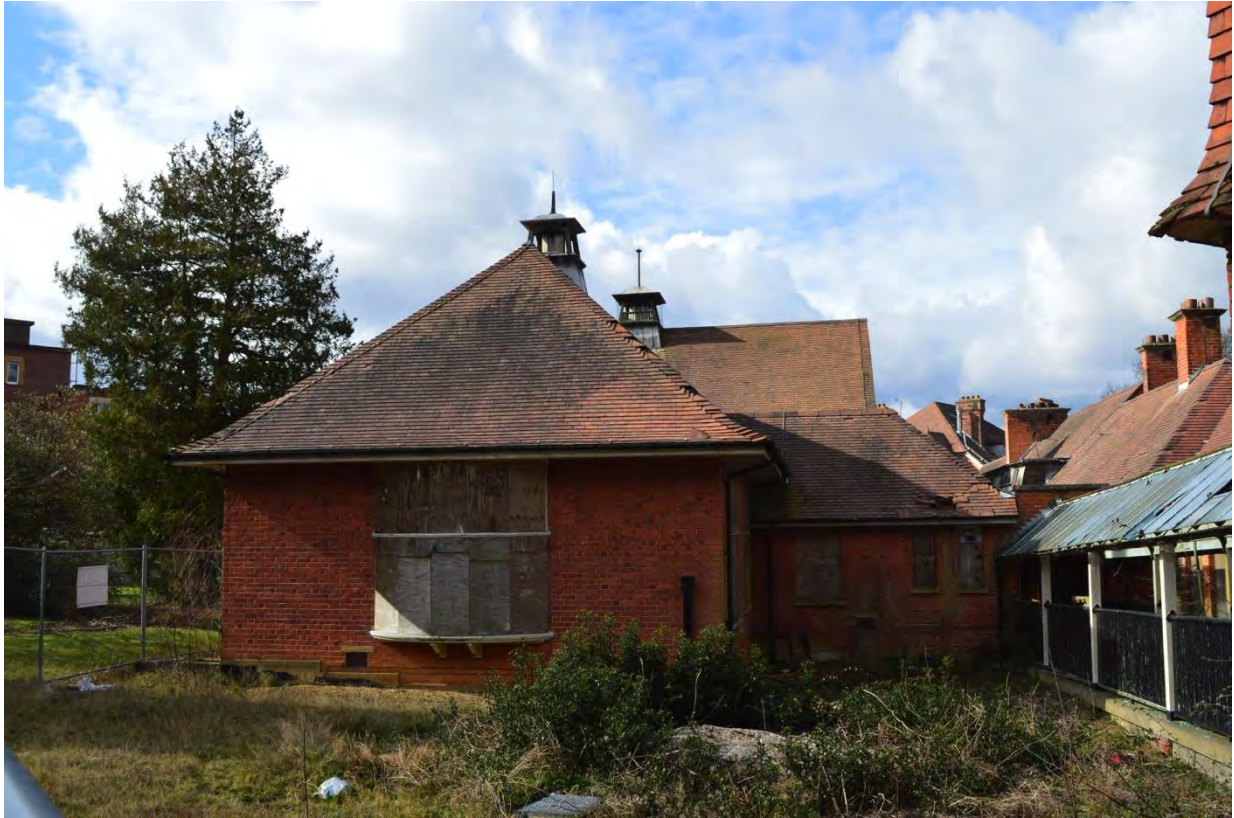
Plate 25: Building 7, view of east elevation, facing west (7335_0016)
