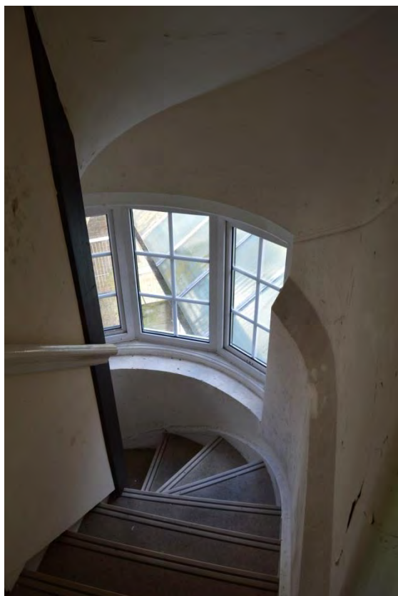
Plate 44: Building 9, first floor, secondary stair to the north-east elevation, facing north-east (7335_0165)
