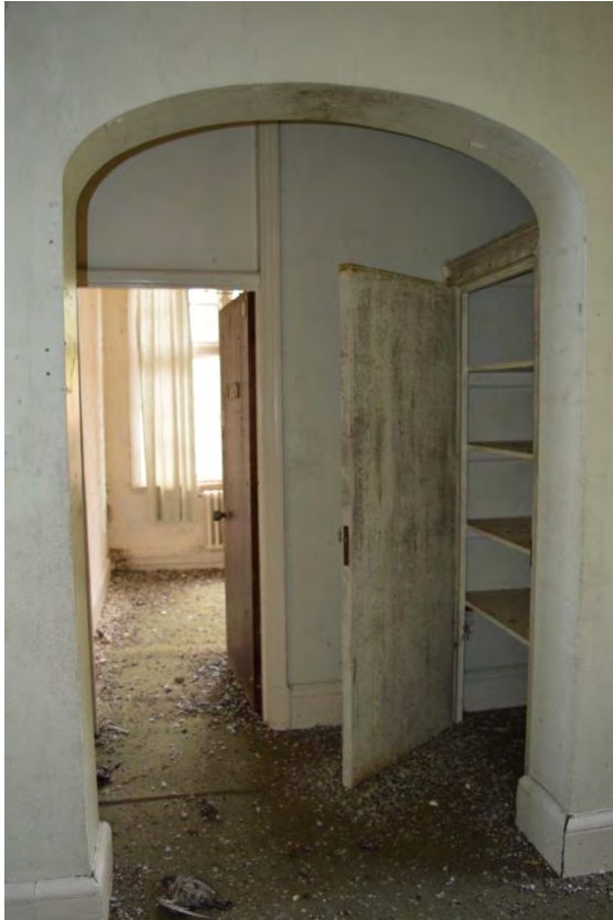
Plate 67: Building 10, first floor, Room 14 arched entrance, facing north (7335_0076)
