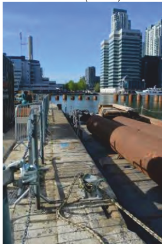
Plate 28: Mid Cut, looking south. (Photo#5)
