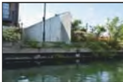
7525-0079 7525_West India Dock_Blackwall Basin_Timber Revetment. Facing south
