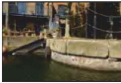
7525-0073 7525_West India Dock_Blackwall Basin_1878 Wall Within Graving Dock. Facing south-west
