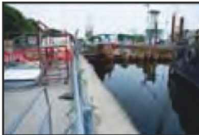
7525-0139 7525_West India Dock_South Dock_North Wall and Ongoing Construction. Facing east
