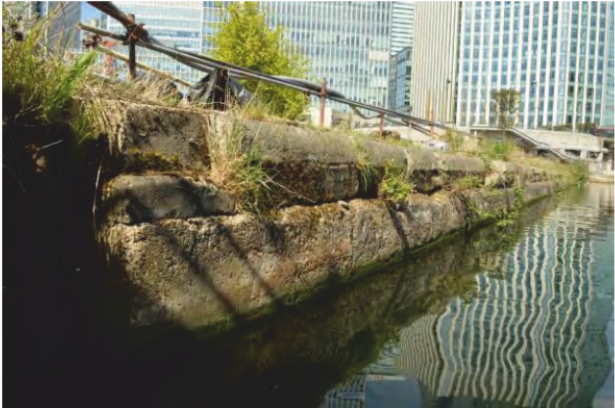
Plate 17: Concrete wall with granite coping [8], looking west. (Photo#97)
