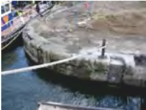
1. Wood Wharf 3 – WWS3 (2)
