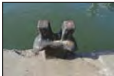
7525-0006 7525_West India Dock_South Dock_North Wall_Staghorn Mooring Bollard. Facing south
