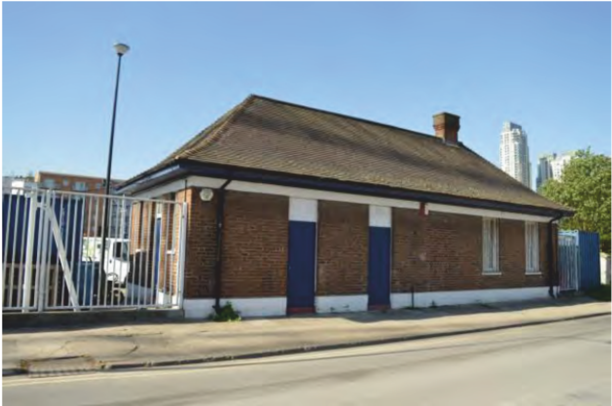
Plate 39: North elevation of the Canal and River Trust Building, looking southwest. (Photo#22)
