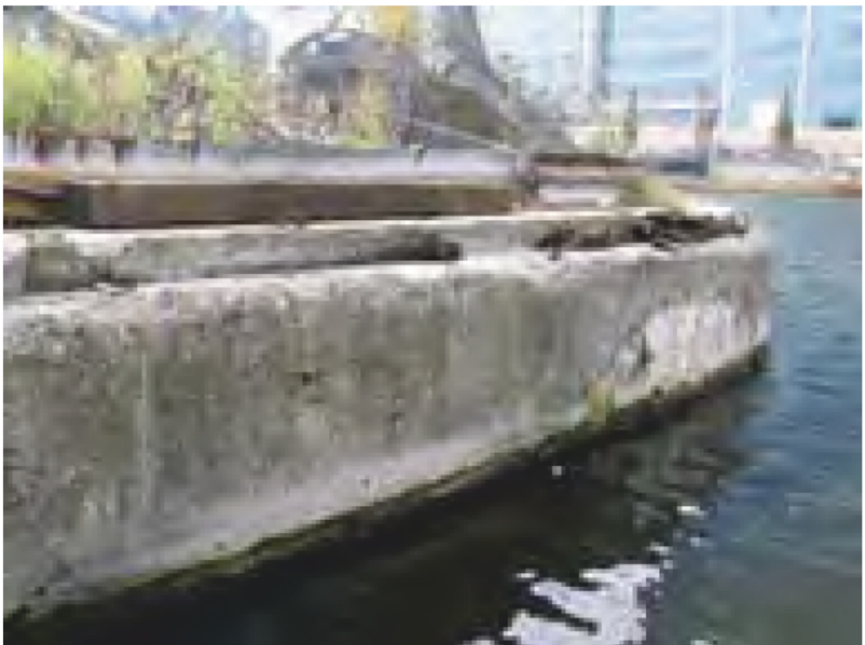
Plate 10: Concrete north eastern corner of the middle cut
