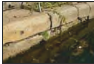
7525-0062 7525_West India Dock_Blackwall Basin_West Wall of the Basin. Facing north-west
