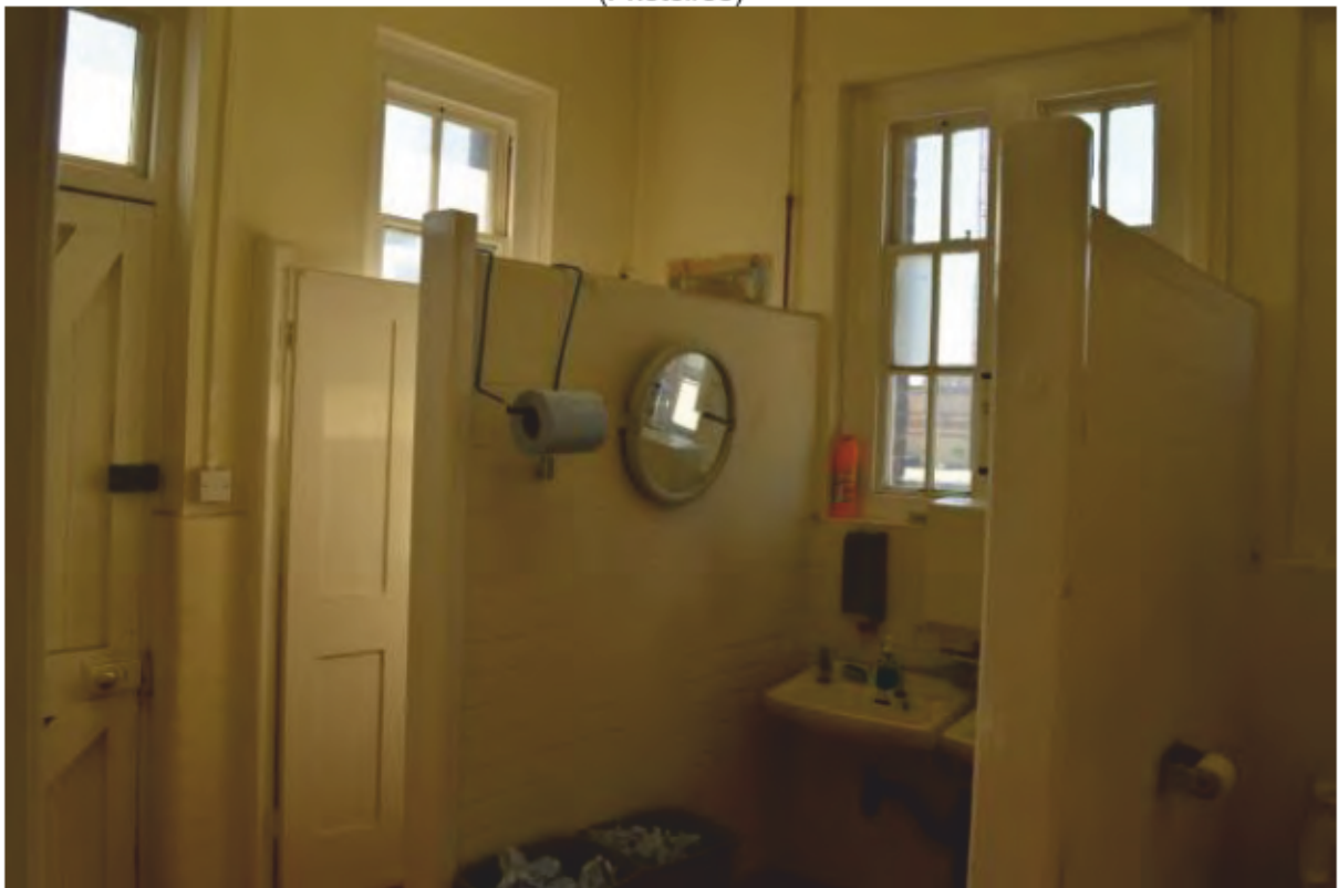
Plate 44: Overview of the toilet in the Canal and River Trust Building, looking southeast. (Photo#39)
