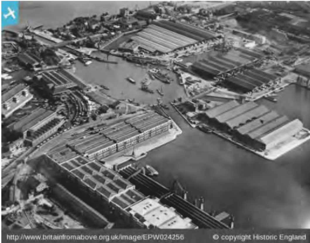
Plate 1: 1928 Aerial photograph showing Blackwall Basin and the construction of the new South Dock entrance lock
