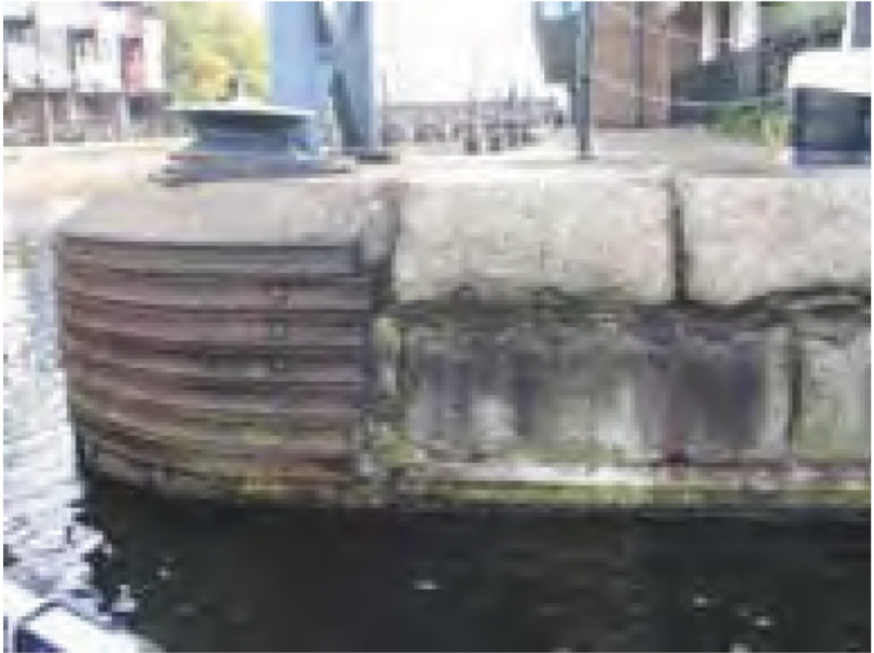
Plate 7: Knuckle at the inner end of the entrance lock
