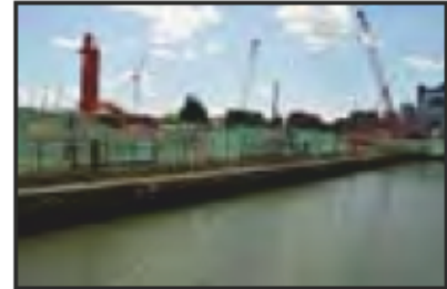
7525-0123 7525_West India Dock_Export Dock_East Wall. Facing south-east
