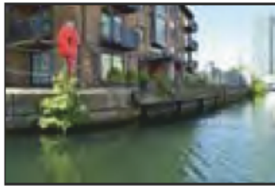
7525-0076 7525_West India Dock_Blackwall Basin_1878 Wall and Timber Revetted Wall. Facing south-west
