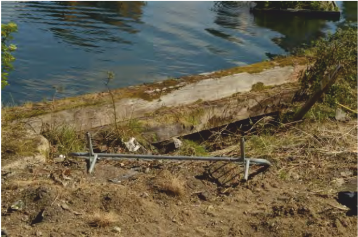
Plate 5: Excavated fill to the rear of the timber revetment [2]. (Photo#66)
