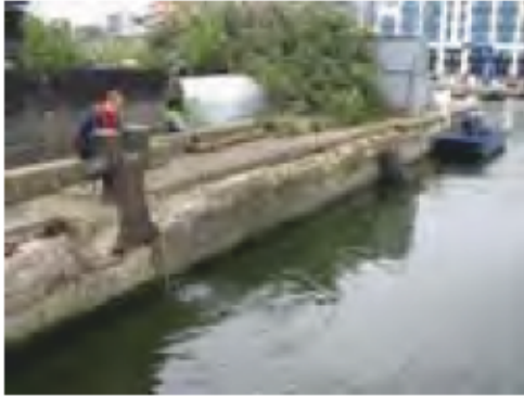
1. Wood Wharf 5 – WWS (4)
