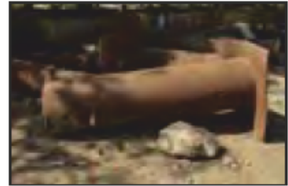
7525-0108 7525_West India Dock_Blackwall Basin_Removed Mooring Bollard. Facing south
