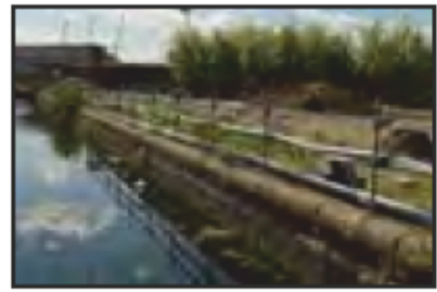
7525-0060 7525_West India Dock_Blackwall Basin_1926-9. Facing south-east
