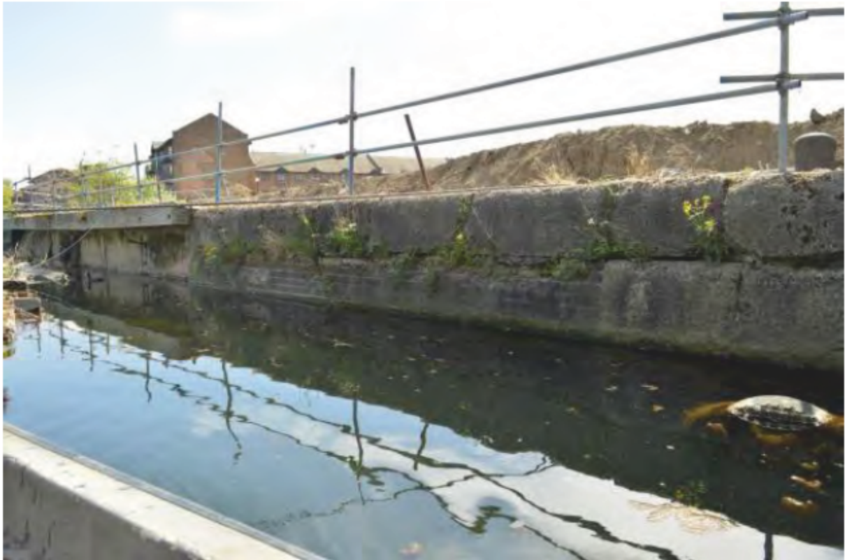
Plate 11: Engineering brick repair work [3] east section, looking east. (Photo#91)
