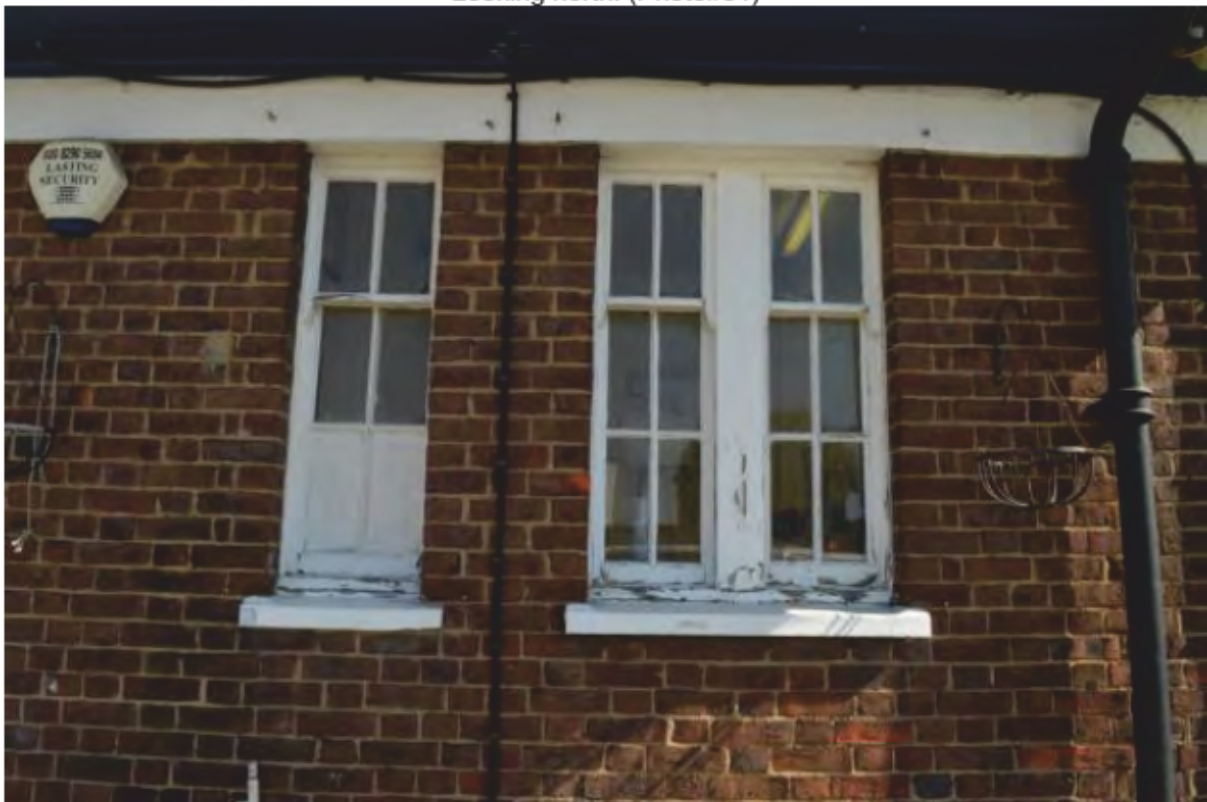
Plate 36: Narrow sash windows to the east of the principal elevation of the Canal and River Trust Building, looking north. (Photo#30)
