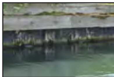
7525-0083 7525_West India Dock_Blackwall Basin_Timber Revetment. Facing south- west
