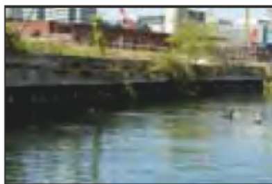
7525-0082 7525_West India Dock_Blackwall Basin_Timber Revetment. Facing south- west
