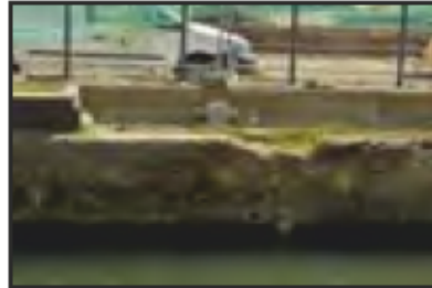
7525-0122 7525_West India Dock_Export Dock_East Wall. Facing east
