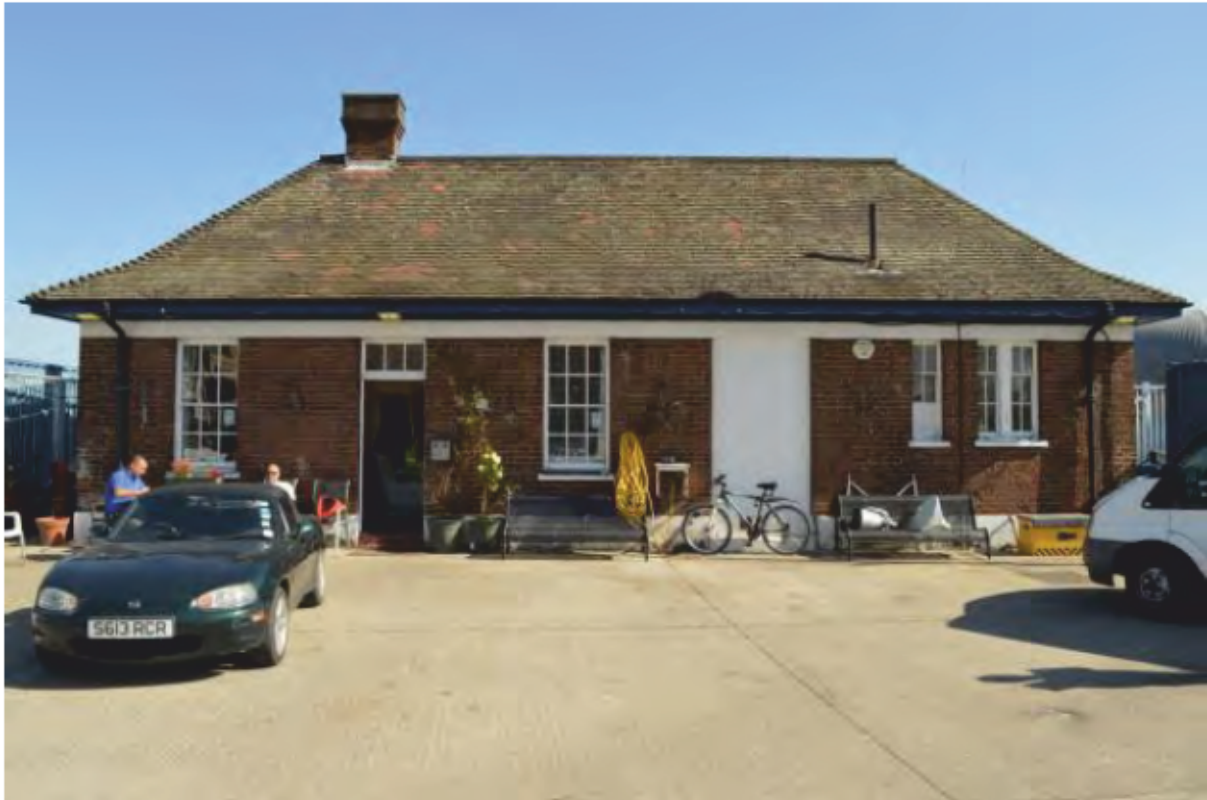
Plate 33: Principal elevation of the Canal and River Trust Building, looking north. (Photo#32)
