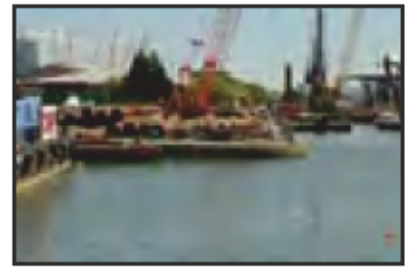
7525-0135 7525_West India Dock_Export Dock_Middle Cut. Facing east
