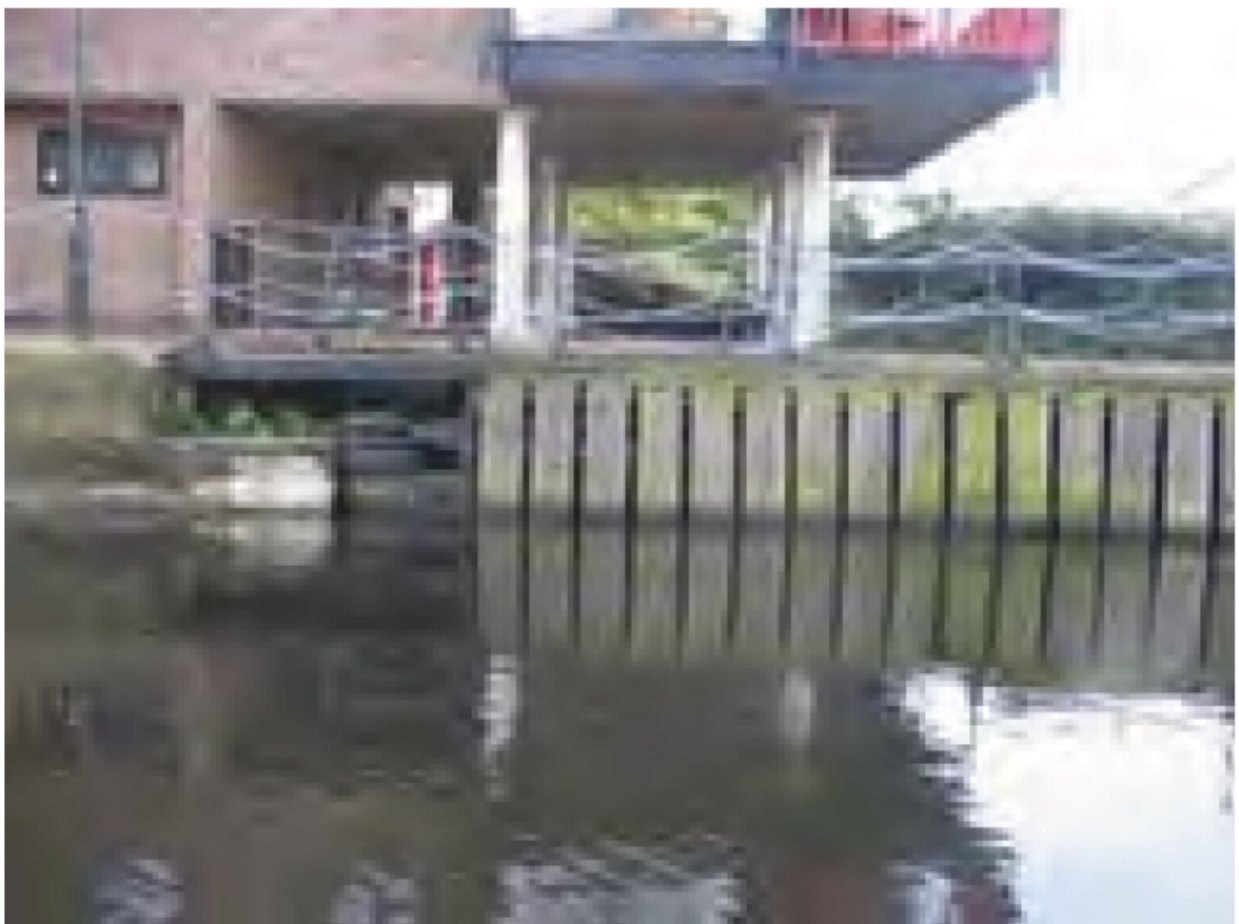
Plate 6: Surviving inner lock gates of the entrance lock to the basin
