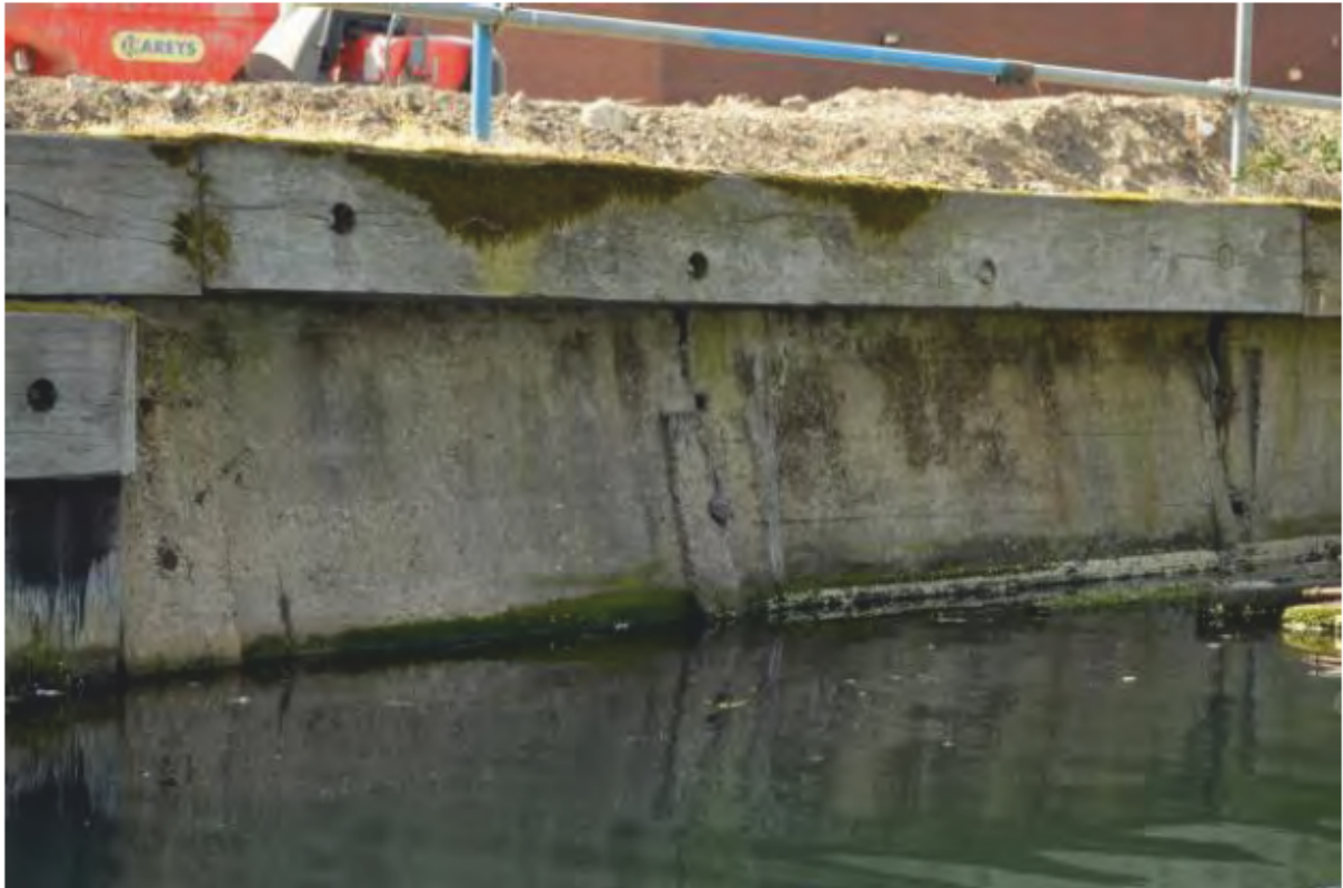
Plate 9: Exposed concrete with banked sides and bracketing [2]. (Photo#87)
