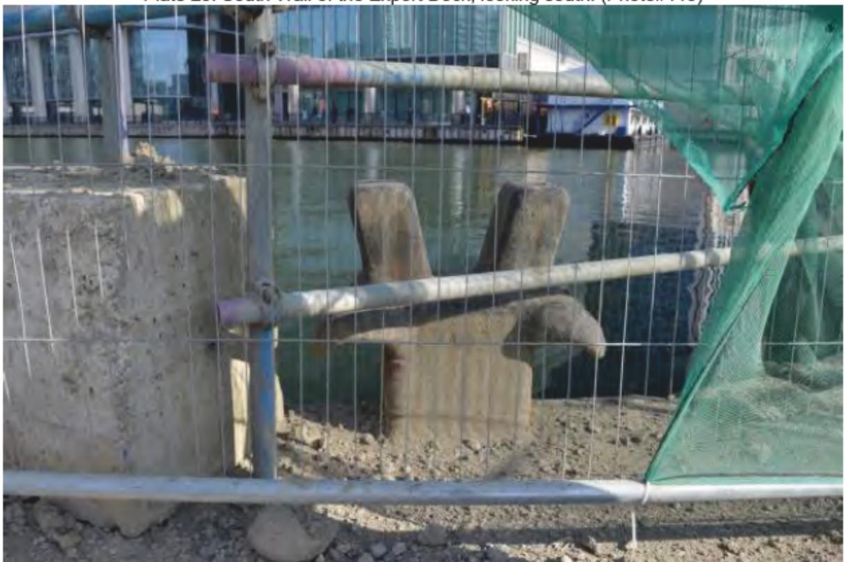
Plate 26: Staghorn mooring bollard at the east end of the South Wall of the Export Dock, looking northwest. (Photo#1)
