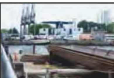
7525-0145 7525_West India Dock_South Dock_East Wall_North of Lock. Facing east
