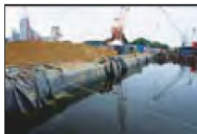
7525-0143 7525_West India Dock_South Dock_North Wall Covered During Development. Facing north-east
