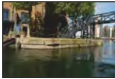
7525-0074 7525_West India Dock_Blackwall Basin_1878 Wall within Graving Dock. Facing west
