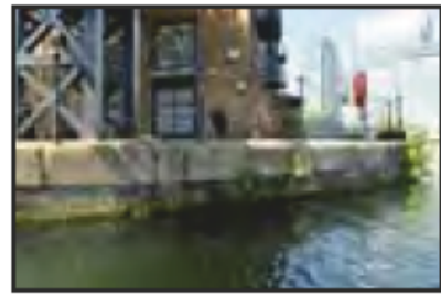
7525-0075 7525_West India Dock_Blackwall Basin_1878 Wall. Facing west
