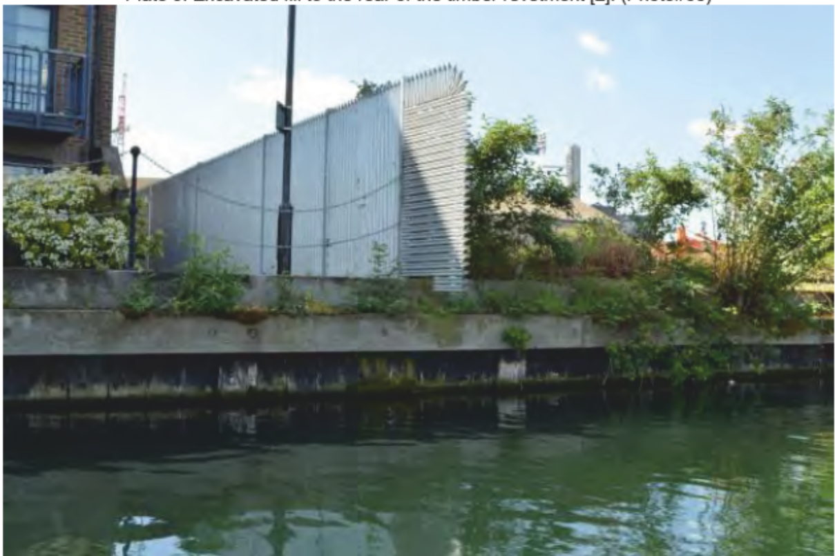
Plate 6: Timber revetment with king posts and capping beams [2]. Looking south. (Photo#79)
