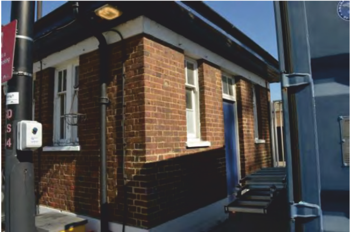
Plate 37: East elevation of the Canal and River Trust Building, looking northwest. (Photo#27)
