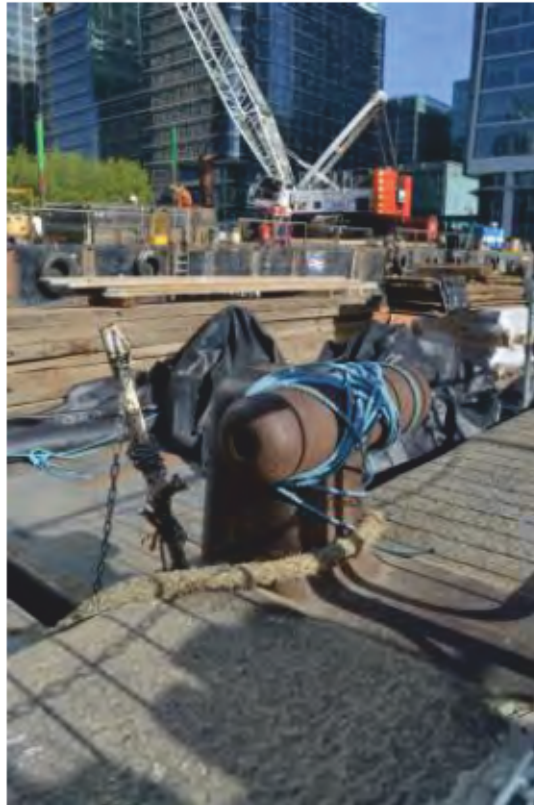
Plate 29: T-head mooring bollard on the Middle Cut, looking northwest. (Photo#8)
