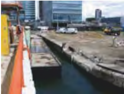
1. Wood Wharf 3 – WWS3 (5)
