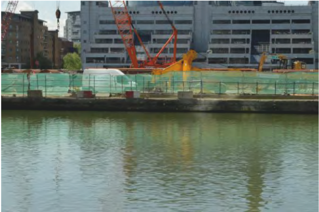
Plate 25: South Wall of the Export Dock, looking south. (Photo#115)
