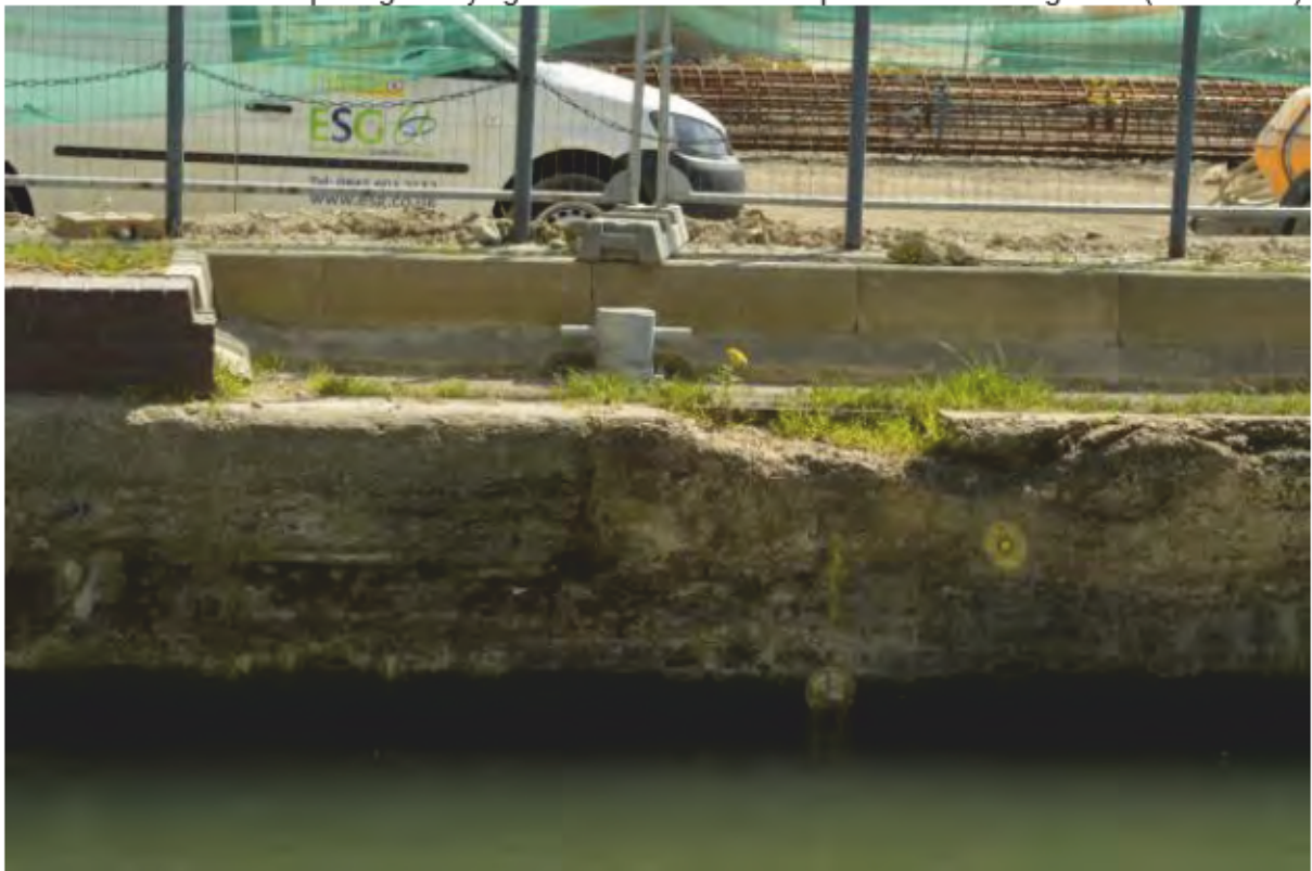
Plate 24: East Wall of the Export Dock single-bitt mooring bollard. (Photo#122)
