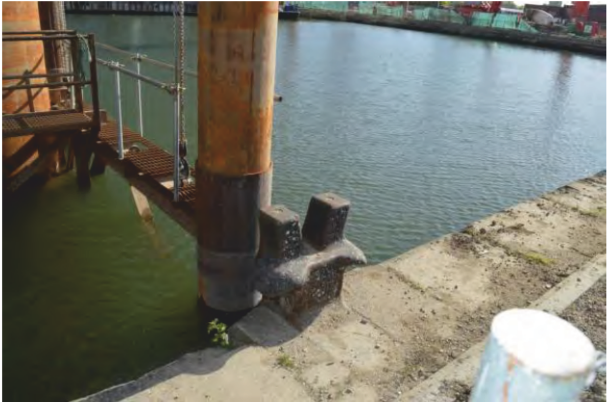
Plate 27: Staghorn mooring bollard at the west end of the South Wall of the Export Dock, looking northeast. (Photo#2)
