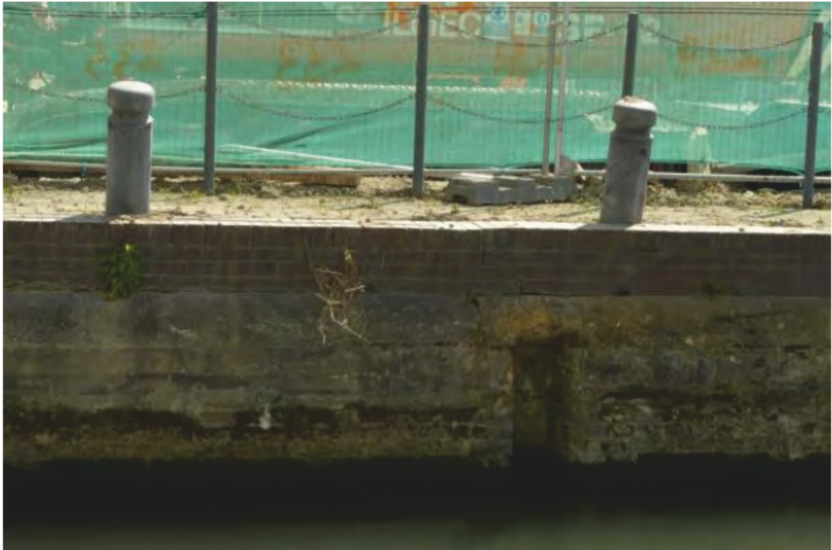
Plate 23: Modern brick paving overlying the East Wall of the Export Dock. Looking East. (Photo#121)
