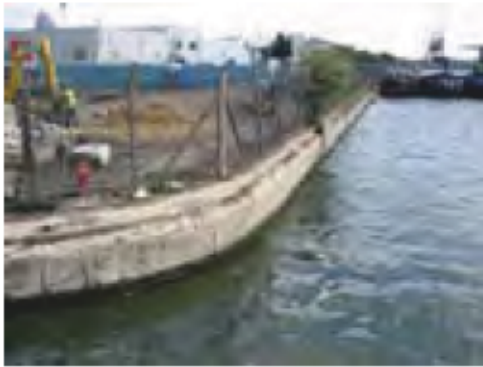
1. Wood Wharf 4 – WWS4 (1)
