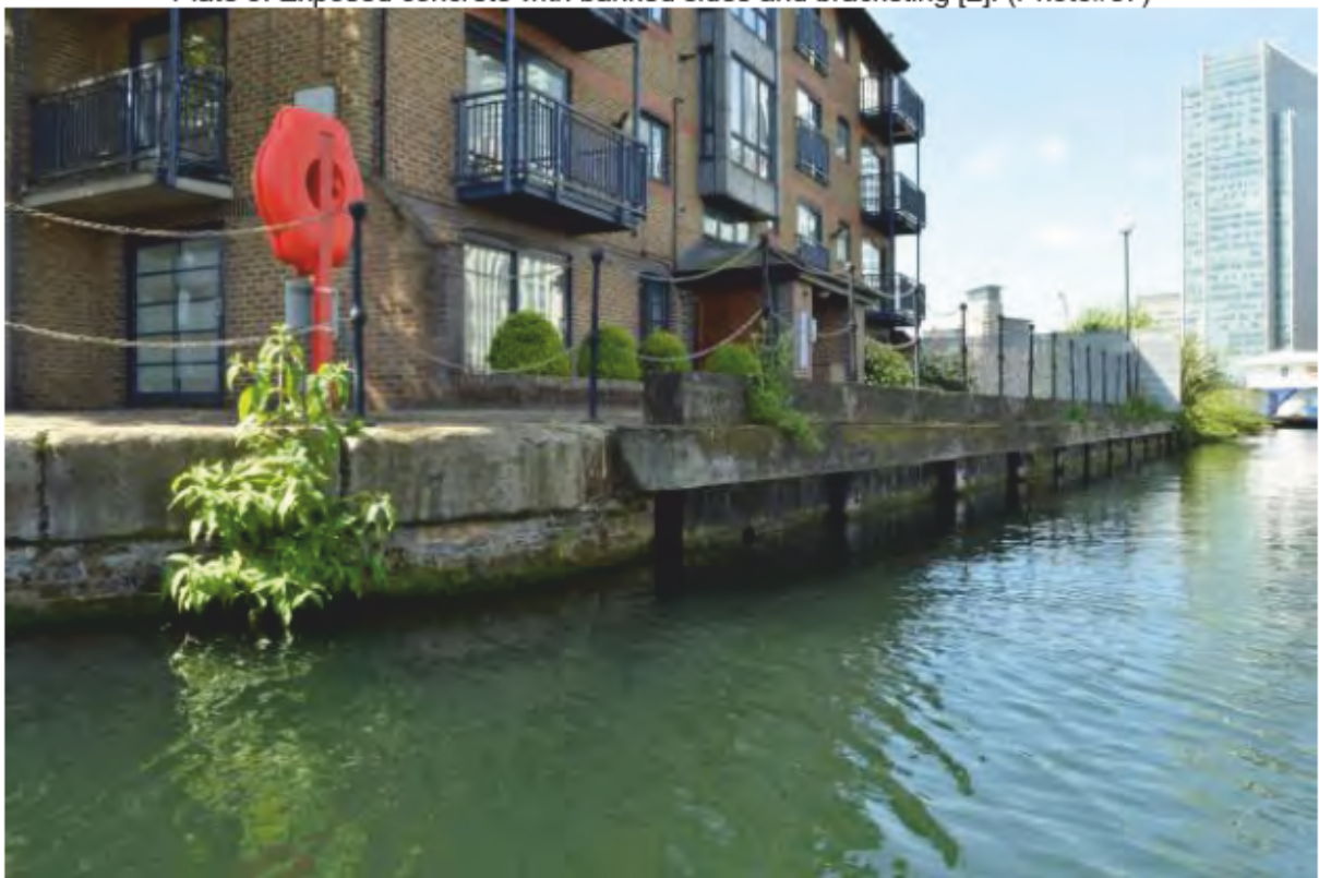
Plate 10: Timber revetted wall surmounted by bollards [2], looking west. (Photo#76)
