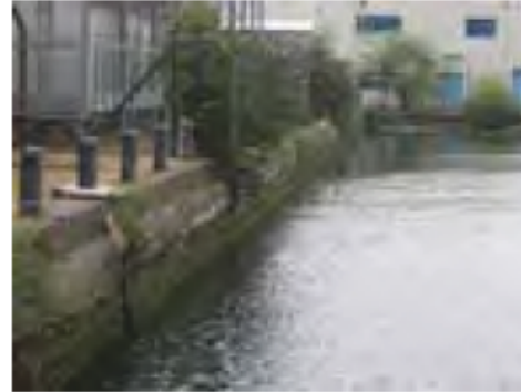
2. Detail Survey 13, Chainage 40 Wood Wharf 1 – WWS1 (11)
