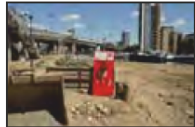
7525-0126 7525_West India Dock_Blackwall Basin_Mooring Bollard. Facing north
