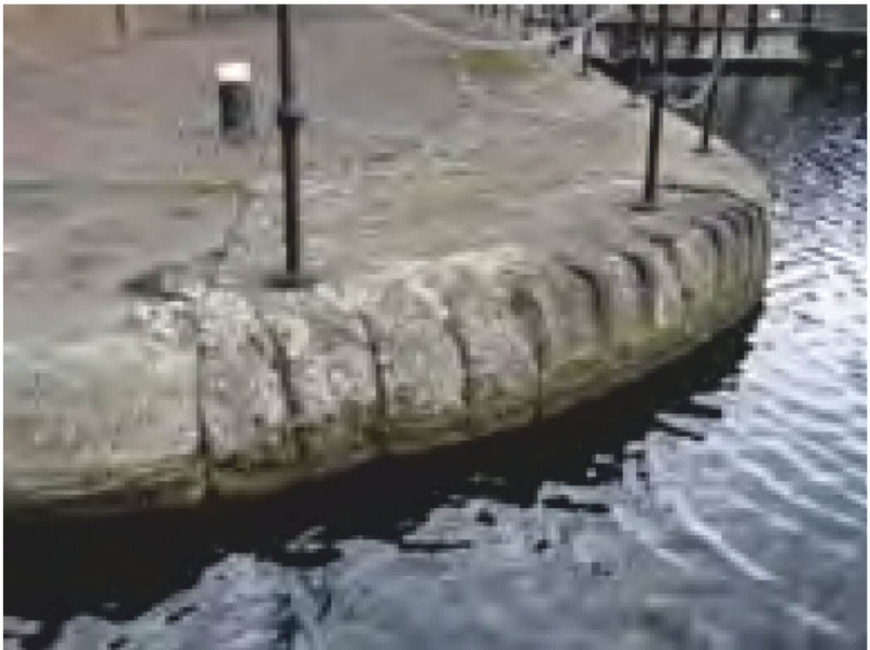
Plate 8: Steel reinforcing bars on the knuckle between the basin and the canal to poplar dock
