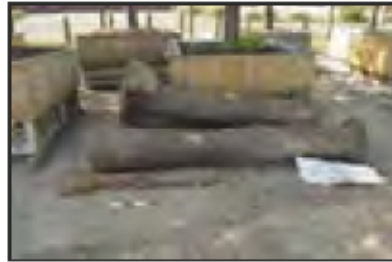
7525-0107 7525_West India Dock_Blackwall Basin_Removed Mooring Bollards. Facing south
