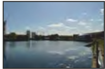
7525-0063 7525_West India Dock_Blackwall Basin_Overview. Facing east
