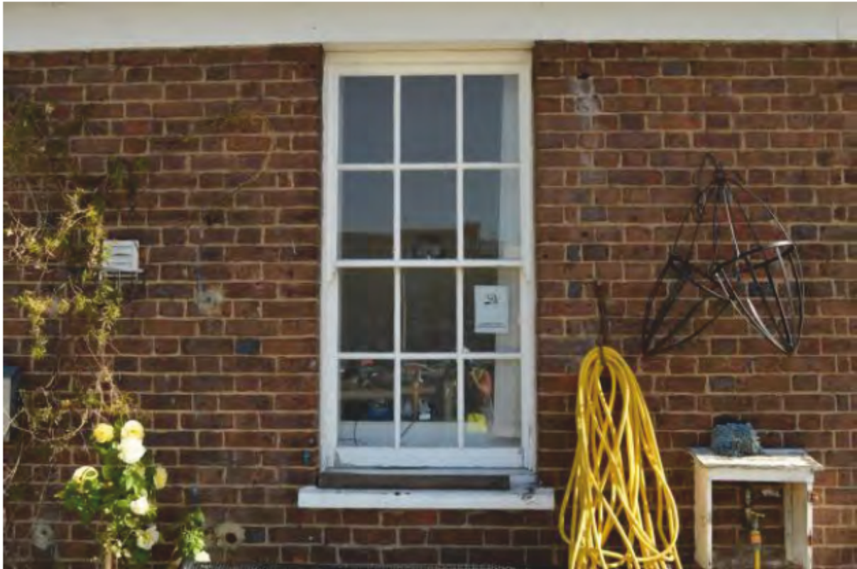
Plate 35: Horned-sash window on the principal elevation of the Canal and River Trust Building. Looking north. (Photo#31)
