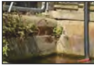
7525-0104 7525_West India Dock_Blackwall Basin_1926-9 Wall. Facing west
