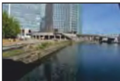
7525-0010 7525_West India Dock_Blackwall Basin_1926-9 Wall. Facing west
