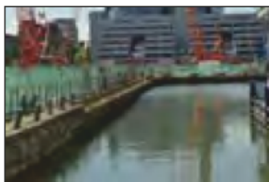
7525-0112 7525_West India Dock_Export Dock_East Wall. Facing south
