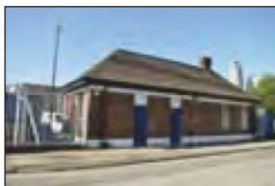
7525-0022 7525_West India Dock_Canal & River Trust Building_North Elevation. Facing south-west
