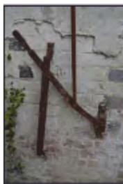
7494-0067 Combers Glasshouses - Building 1 - lever tackle. Facing north
