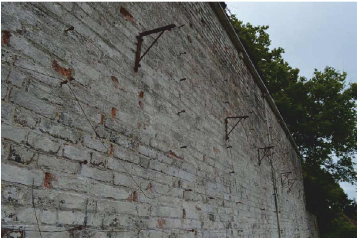
Plate 22: Building 2, pegs and wires in the back wall Bay 2, looking north-east (Photo #17)
