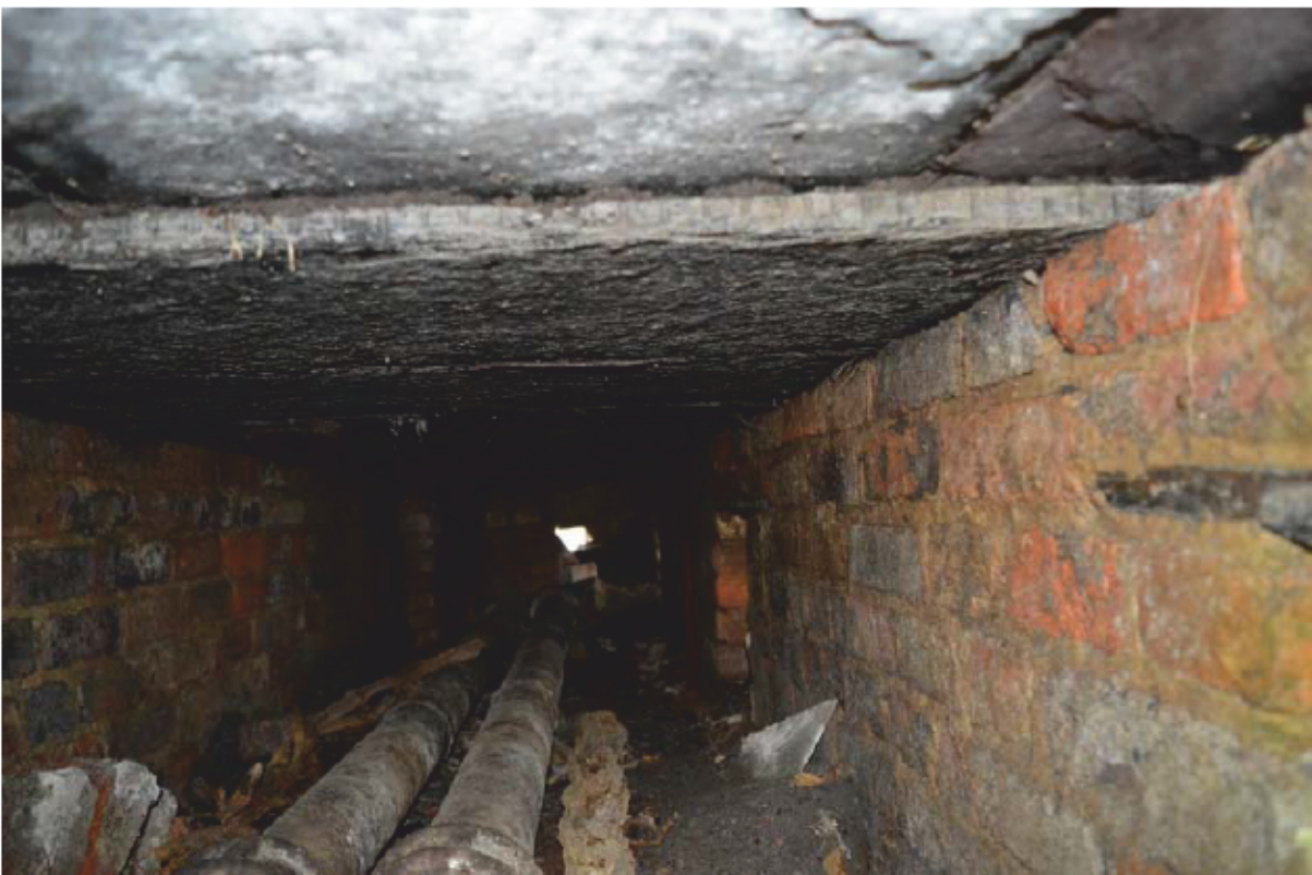
Plate 10: Southern lean-to, Building 1, void beneath the southern bed, looking west (Photo #74)
