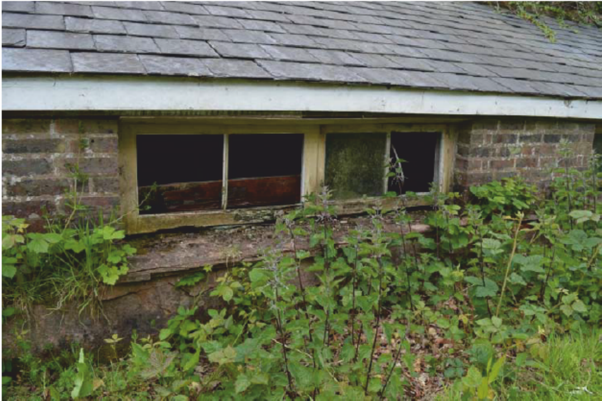
Plate 35: Building 4, windows in west end of building, looking south (Photo #42)
