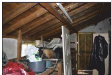
7494-0089 Combers Glasshouses - Building 5 - north room overview. Facing north
