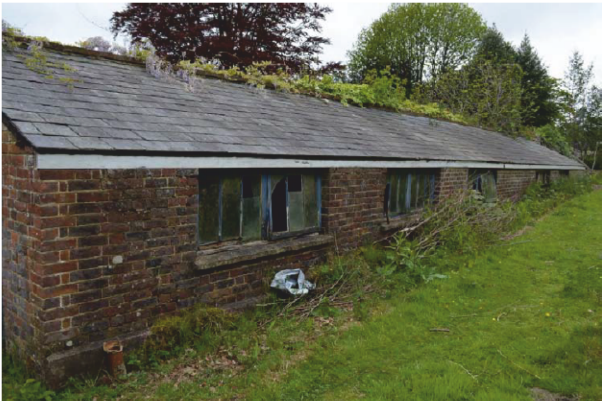
Plate 32: Building 4 overview, looking west (Photo #39)
