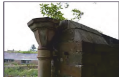
7494-0102 Combers Glasshouses - Building 2 - downpipe at east end. Facing south-west
