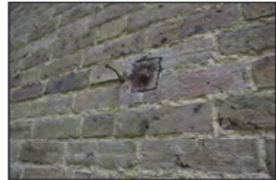
7494-0099 Combers Glasshouses - Building 2 - tie in north of back wall. Facing south
