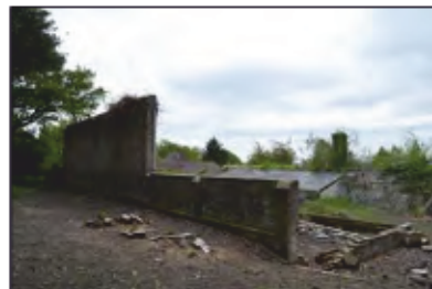
7494-0003 Combers Glasshouses - Building 2 - Overview. Facing east
