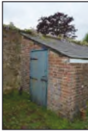
7494-0034 Combers Glasshouses - Building 4 - East elevation. Facing south-west
