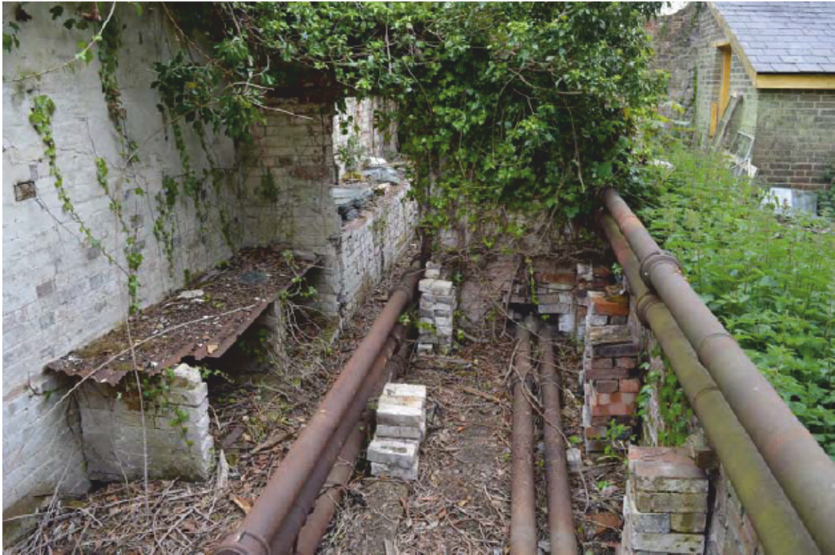
Plate 3: West side of the southern lean-to, Building 1, looking east (Photo #68)
