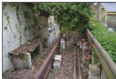
7494-0068 Combers Glasshouses - Building 1 - south lean-to overview. Facing east
