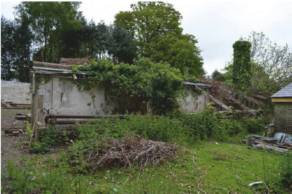
Plate 2: South elevation of Building 1, southern lean-to, looking north (Photo #62)
