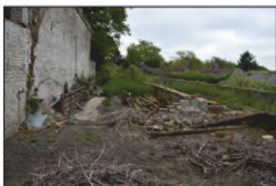
7494-0014 Combers Glasshouses - Building 2 - overview. Facing east
