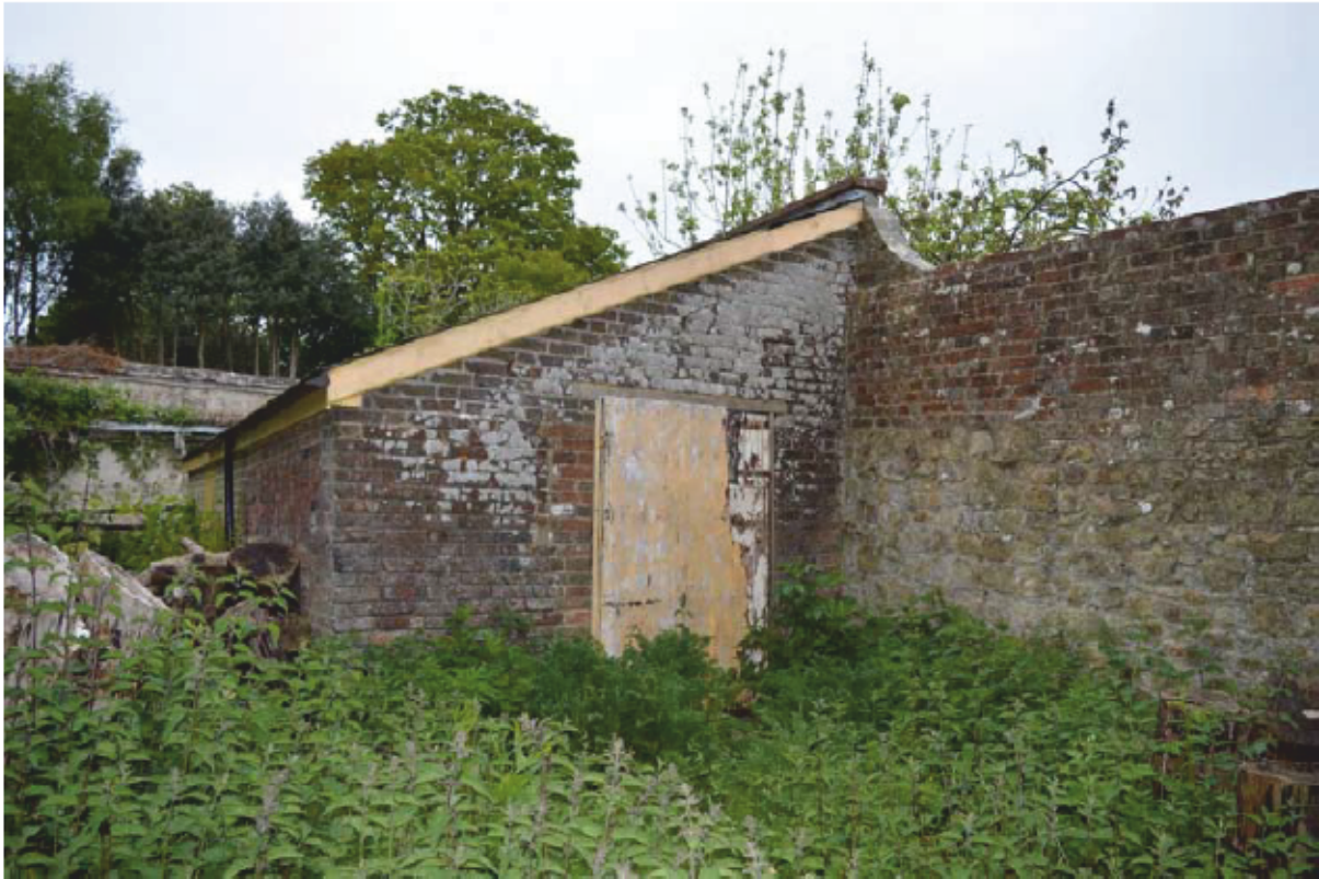
Plate 41: Building 5, blocked timber door in south elevation, looking north (Photo #81)
