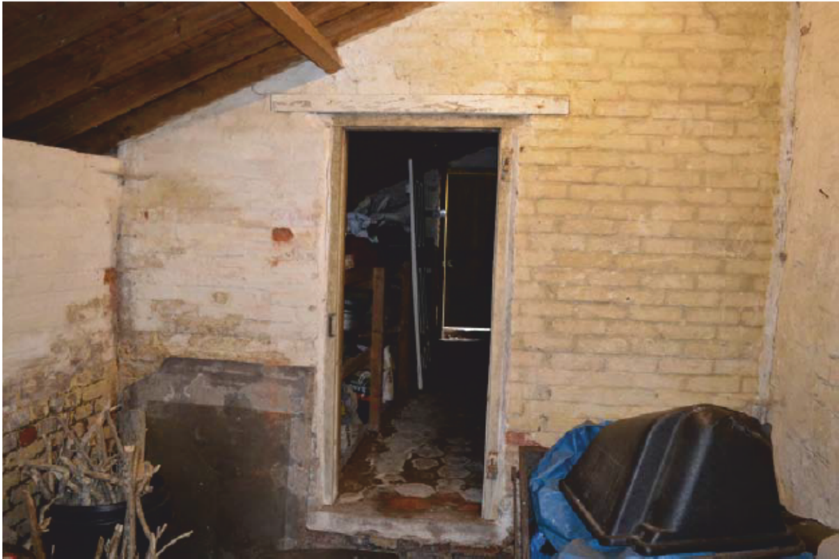
Plate 43: Building 5, south room, looking north (Photo #92)
