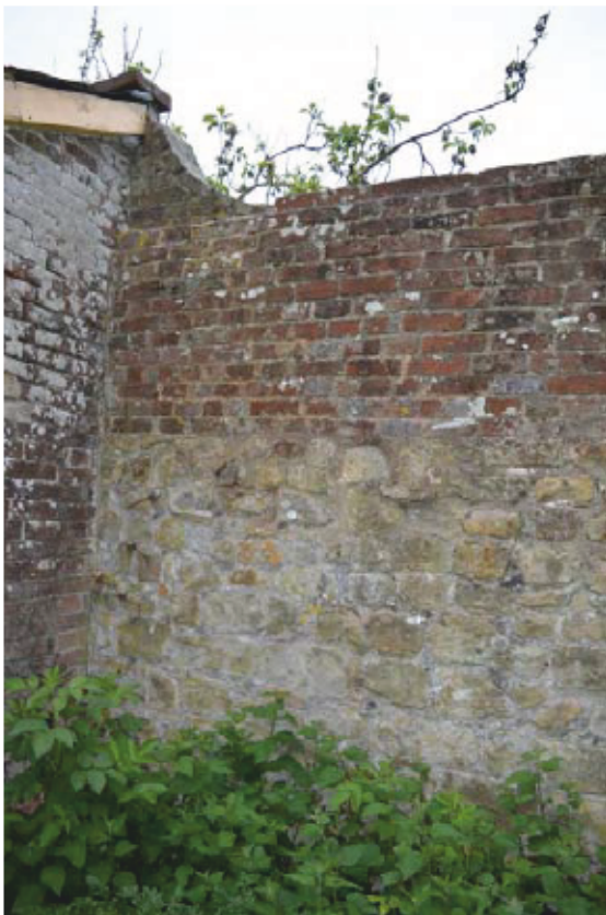
Plate 38: Building 5, kitchen garden wall, looking northeast (Photo #82)
