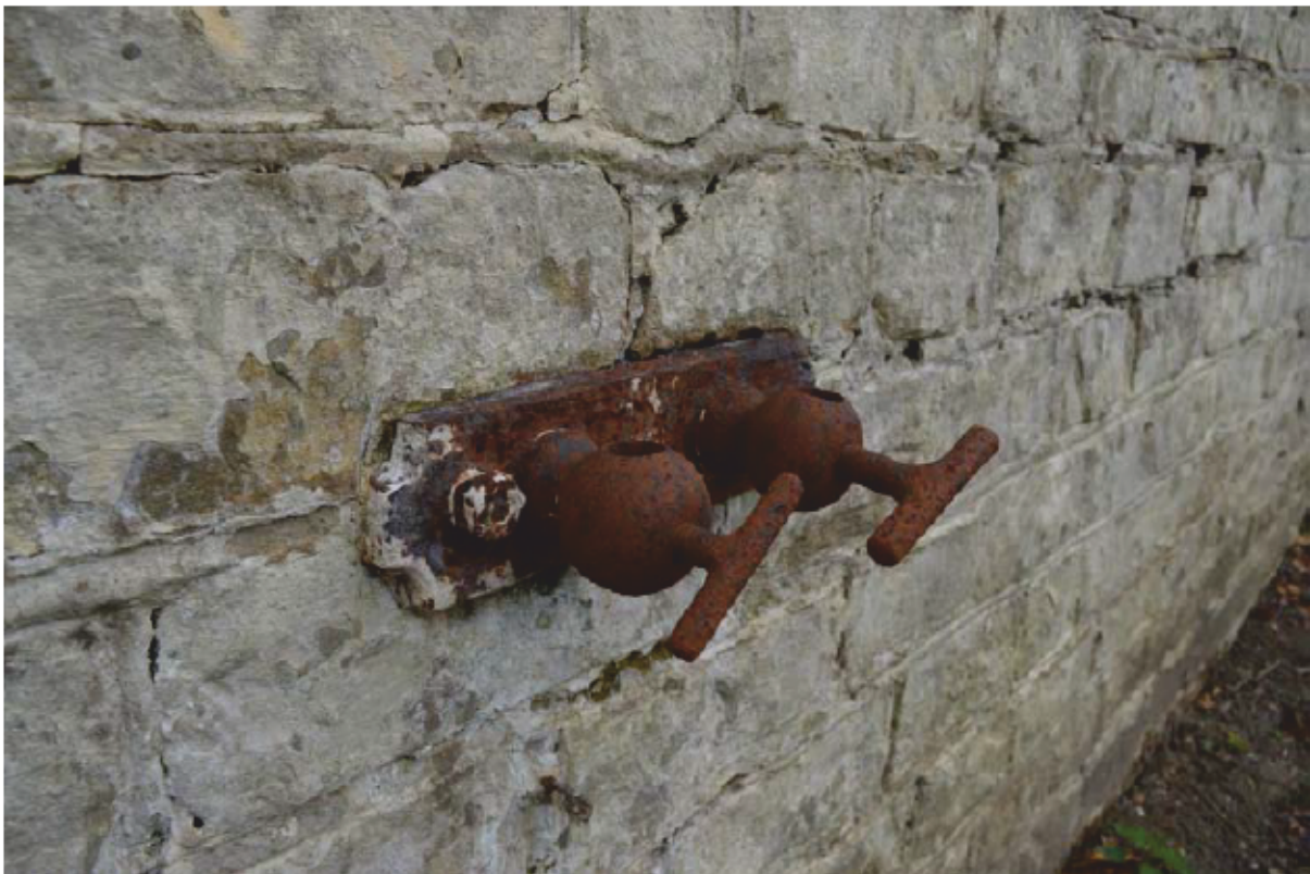
Plate 24: Building 2, screw operated window opening device, looking north-east (Photo #12)
