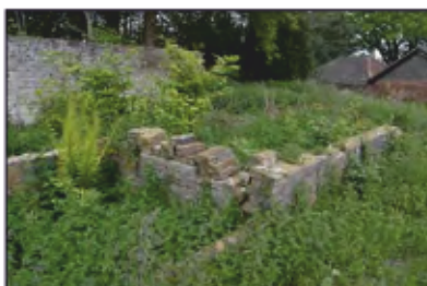
7494-0028 Combers Glasshouses - Building 2 - Bay 4 overview. Facing north-east
