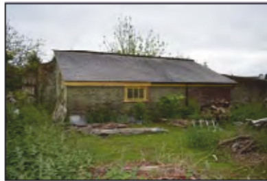
7494-0080 Combers Glasshouses - Building 5 - overview. Facing east
