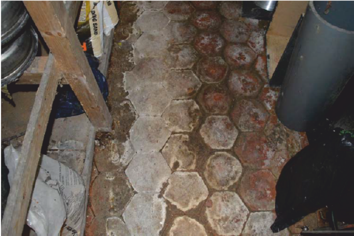
Plate 45: Building 5, tile floor in north room, looking south (Photo #90)
