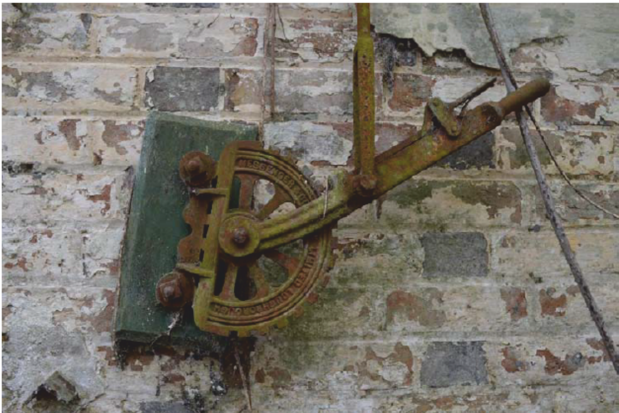
Plate 14: Northern lean-to, Building 1, lever tackle, looking south (Photo #53)
