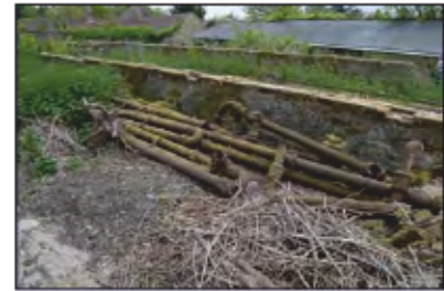
7494-0018 Combers Glasshouses - Building 2 - Bays 2 and 3, arches in brickwork. Facing south-east
