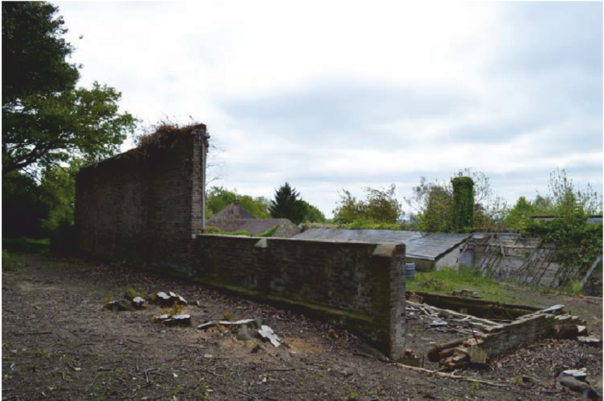
Plate 19: Building 2, view of the bracketing to the rear of the back wall, looking south-east (Photo #3)
