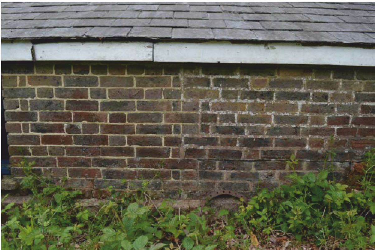
Plate 34: Building 4, joint in brickwork, looking south (Photo #41)
