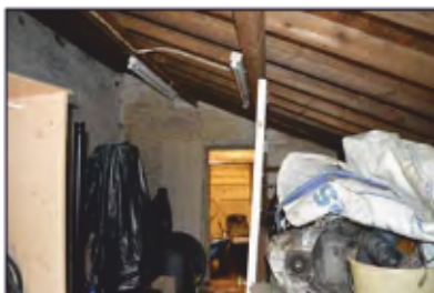
7494-0088 Combers Glasshouses - Building 5 - interior overview. Facing south
