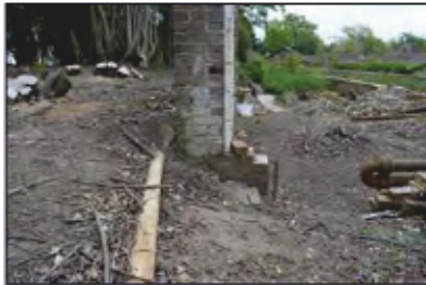
7494-0097 Combers Glasshouses - Building 2, west elevation and pipe. Facing east
