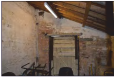
7494-0091 Combers Glasshouses - Building 5 - south room overview. Facing south
