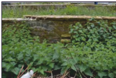
7494-0022 Combers Glasshouses - Building 2 - Bay 3, brick arches. Facing south
