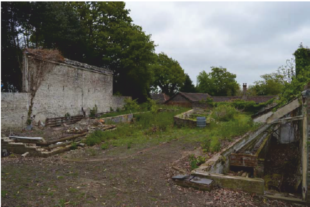
Plate 48: Brick-bordered pathway between glasshouses, looking east (Photo #96)
