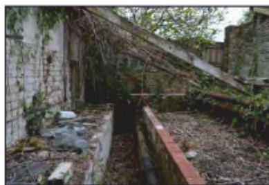
7494-0071 Combers Glasshouses - Building 1 - east end of south lean-to overview. Facing east
