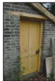
7494-0086 Combers Glasshouses - Building 5 - doorway in north elevation. Facing south
