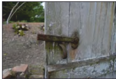
7494-0065 Combers Glasshouses - Building 1 - door hardware detail. Facing west
