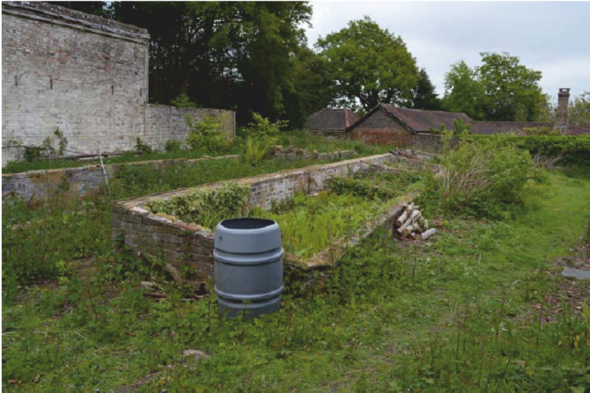
Plate 31: Building 3 overview, looking north-east (Photo #29)
