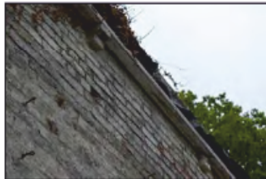
7494-0020 Combers Glasshouses - Building 2 - Bay 2, brick brackets. Facing north-east
