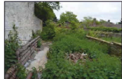
7494-0021 Combers Glasshouses - Building 2 - Bay 3 overview. Facing east
