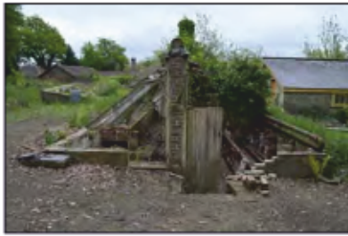
7494-0061 Combers Glasshouses - Building 1 - Overview. Facing east
