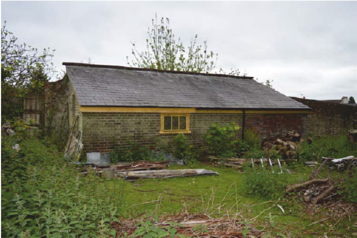
Plate 37: Building 5 overview, looking east (Photo #80)
