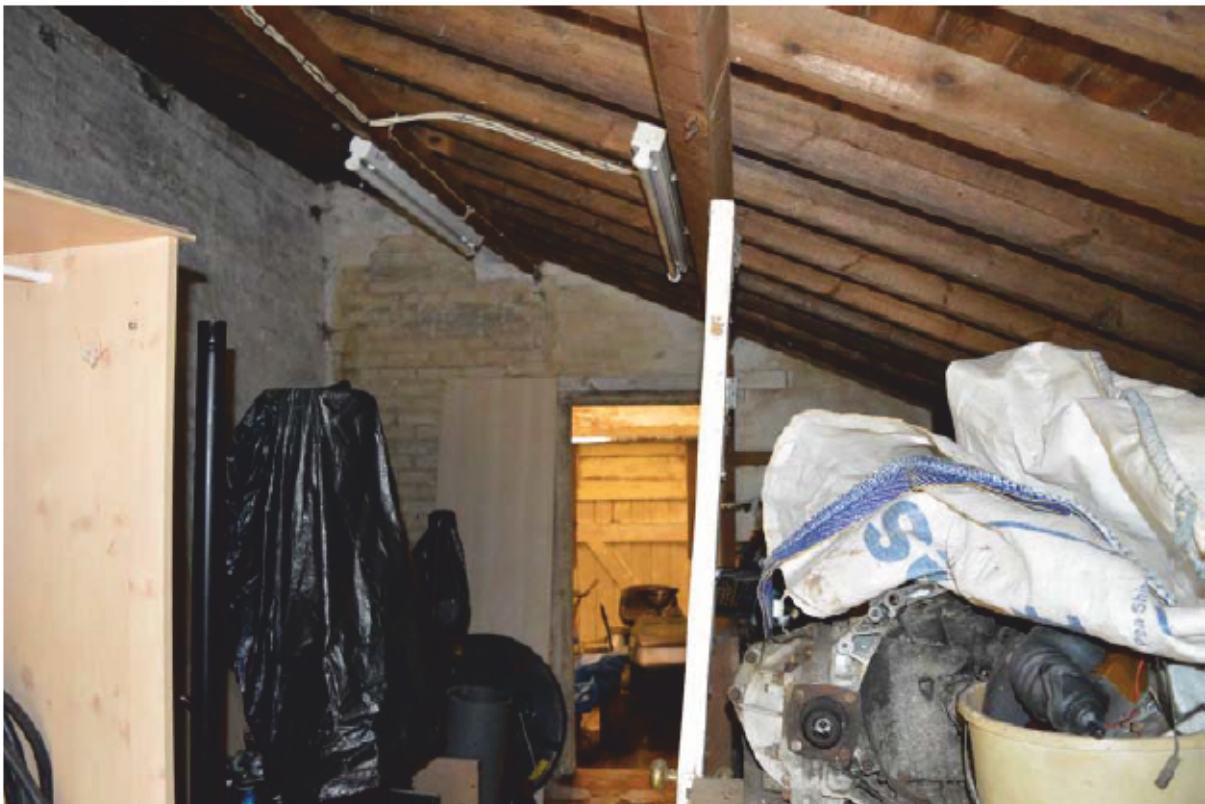
Plate 42: Building 5, north room, looking south (Photo #88)
