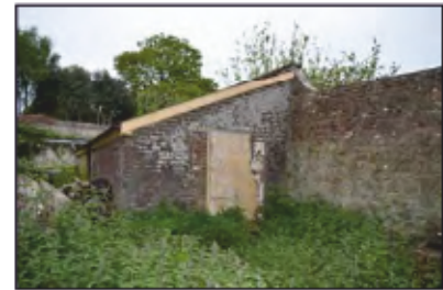
7494-0081 Combers Glasshouses - Building 5 - south elevation. Facing north
