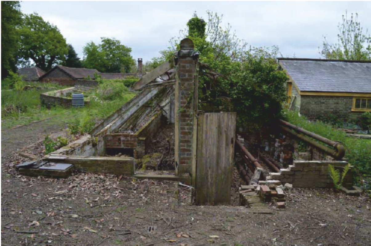
Plate 1: West elevation of Building 1, looking east (Photo #61)
