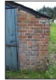
7494-0036 Combers Glasshouses - Building 4 - East elevation. Facing west
