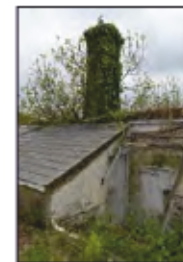
7494-0045 Combers Glasshouses - Building 4/Building 1 - Intersection and Chimney Stack. Facing south-east
