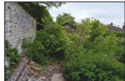
7494-0024 Combers Glasshouses - Building 2 - Bay 4, overview. Facing east
