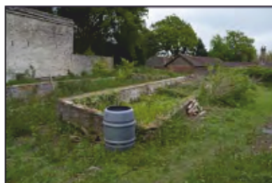
7494-0029 Combers Glasshouses - Building 3 - Overview. Facing north-east
