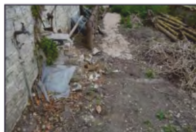
7494-0015 Combers Glasshouses - Building 2 - Bay 1/Bay 2 doorway. Facing east
