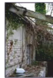
7494-0072 Combers Glasshouses - Building 1 - void mortise, east end, south lean-to. Facing east
