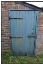
7494-0037 Combers Glasshouses - Building 4 - East elevation. Facing west
