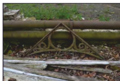
7494-0009 Combers Glasshouses - Building 2 - Bay 1, bracket spandrel. Facing south
