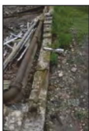
7494-0010 Combers Glasshouses - Building 2 - Bay 1. Facing east
