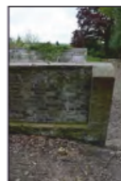
7494-0006 Combers Glasshouses - Building 2 - Bracket. Facing south
