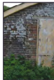
7494-0083 Combers Glasshouses - Building 5 - south elevation. Facing north
