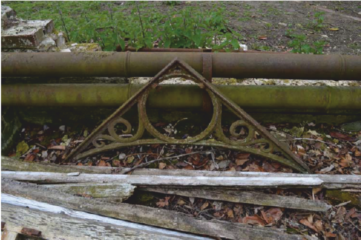
Plate 27: Building 2, spandrel in Bay 1, looking south (Photo #9)
