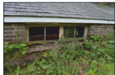
7494-0042 Combers Glasshouses - Building 4 - Window in north elevation. Facing south
