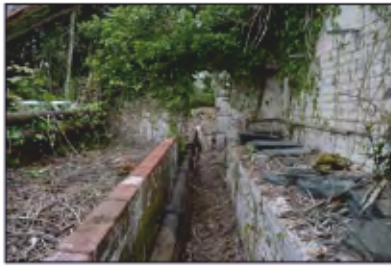
7494-0076 Combers Glasshouses - Building 1 - overview. Facing west
