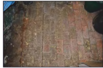
7494-0093 Combers Glasshouses - Building 5 - Brick floor in south room. Facing south
