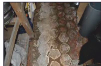
7494-0090 Combers Glasshouses - Building 5 - tile floor in north room. Facing south
