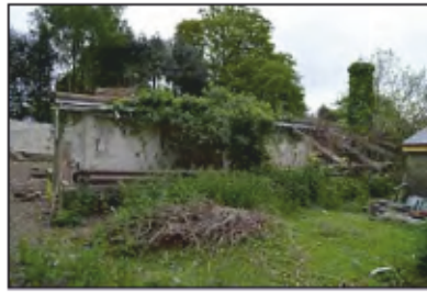
7494-0062 Combers Glasshouses - Building 1 - overview. Facing north
