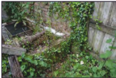
7494-0079 Combers Glasshouses - Building 1 - east end of south lean-to. Facing north-east
