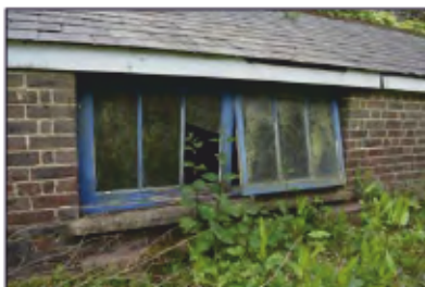
7494-0040 Combers Glasshouses - Building 4 - Window in north elevation. Facing south
