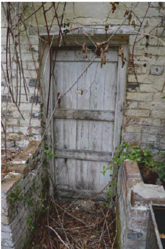
Plate 6: Southern lean-to, Building 1, door to northern lean-to, looking north (Photo #75)
