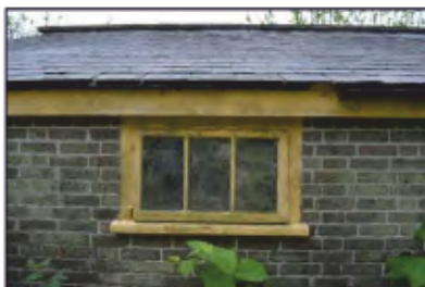
7494-0085 Combers Glasshouses - Building 5 - window in west elevation. Facing east
