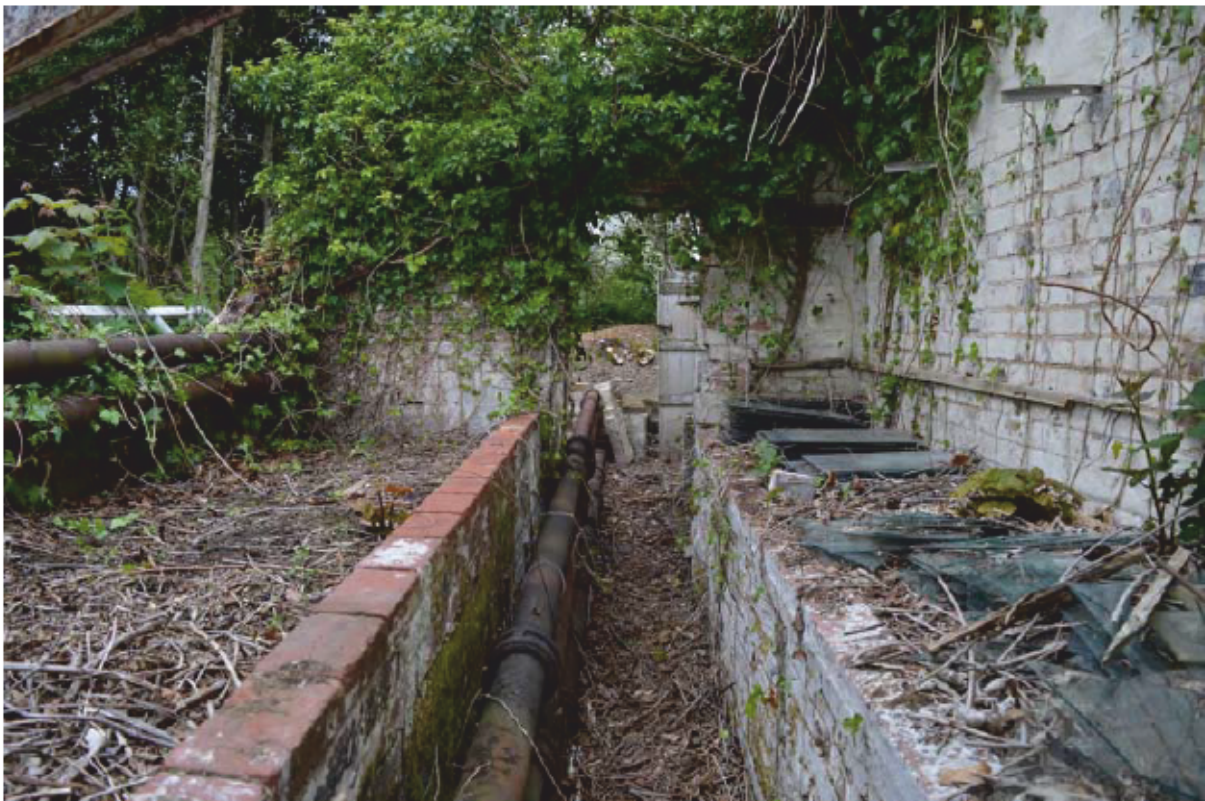
Plate 4: East side of the southern lean-to, Building 1, looking west (Photo #76)
