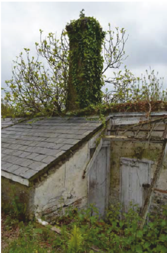
Plate 36: Building 4, chimney stack, looking south-east (Photo #39)
