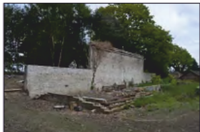
7494-0001 Combers Glasshouses - Building 2 - Overview. Facing north-east
