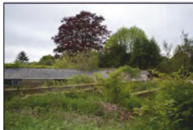
7494-0101 Combers Glasshouses - Context shot. Facing south-west
