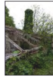
7494-0063 Combers Glasshouses - Building 1 - roof, south lean-to. Facing north-east
