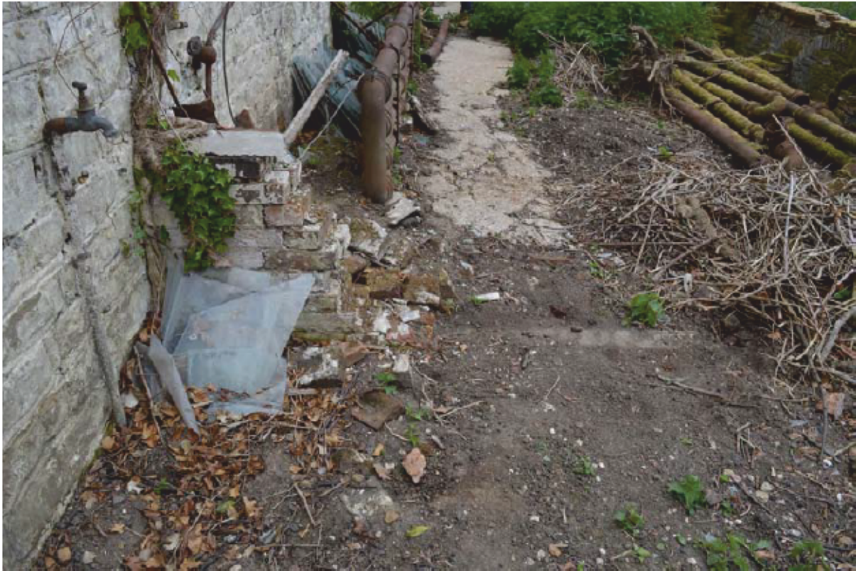
Plate 23: Building 2, tap in Bay 1 and doorway to Bay 2, looking east (Photo #15)
