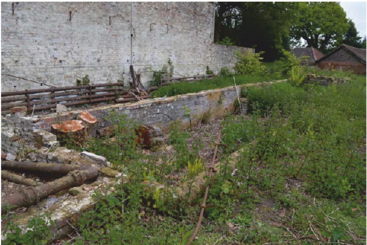
Plate 20: Building 2, plant bed, looking north-east (Photo #26)
