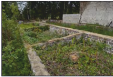
7494-0031 Combers Glasshouses - Building 3 - Overview. Facing west
