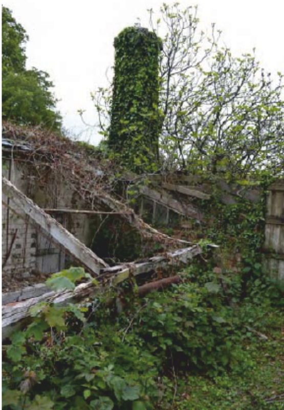
Plate 7: Southern lean-to, Building 1, roof construction, looking north-east (Photo #63)
