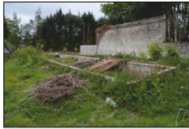
7494-0032 Combers Glasshouses - Building 3 - Overview. Facing north-west
