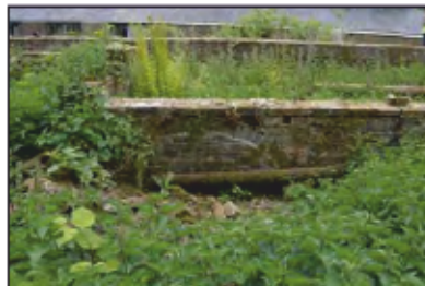
7494-0023 Combers Glasshouses - Building 2 - Bay 3 Brick Arches. Facing south
