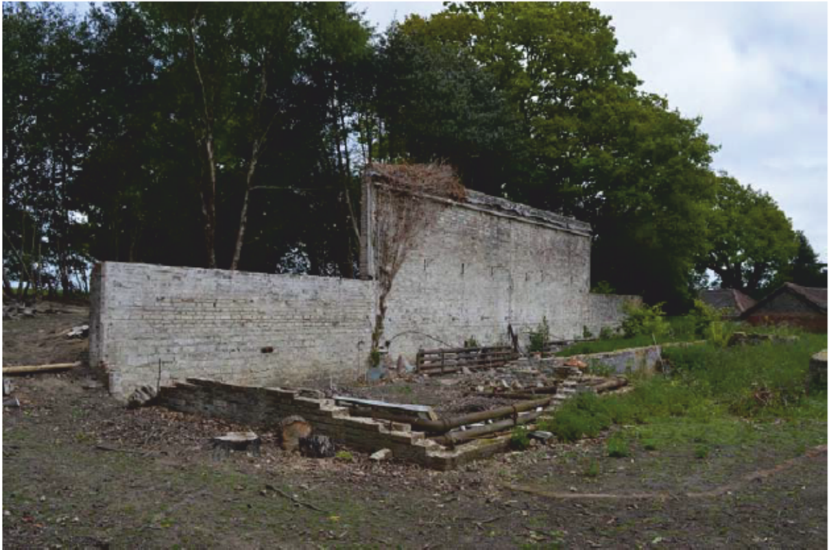
Plate 17: Building 2 overview, looking north-east (Photo #1)
