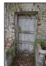
7494-0075 Combers Glasshouses - Building 1 - doorway north through spine wall. Facing north
