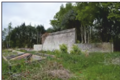
7494-0002 Combers Glasshouses - Building 2 - Overview. Facing north-west
