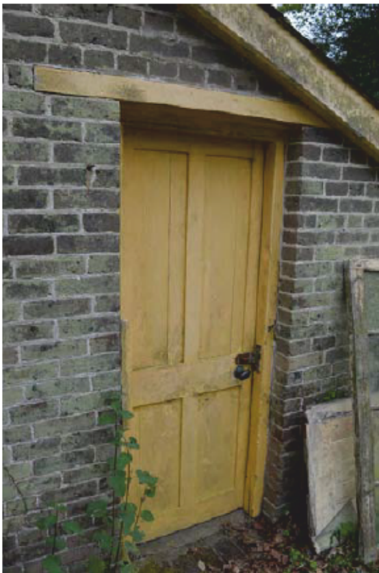
Plate 40: Building 5, panel door in north elevation, looking south (Photo #86)
