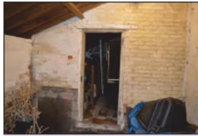
7494-0092 Combers Glasshouses - Building 5 - south room overview. Facing north
