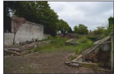
7494-0096 Combers Glasshouses - Context shot - brick-bordered path. Facing east
