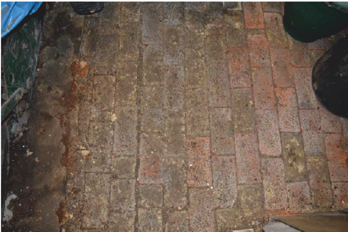
Plate 44: Building 5, brick floor in south room, looking north (Photo #93)
