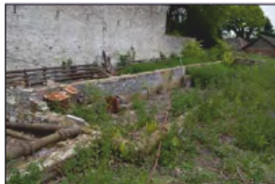
7494-0026 Combers Glasshouses - Building 2 - Bed to front of the building. Facing north-east
