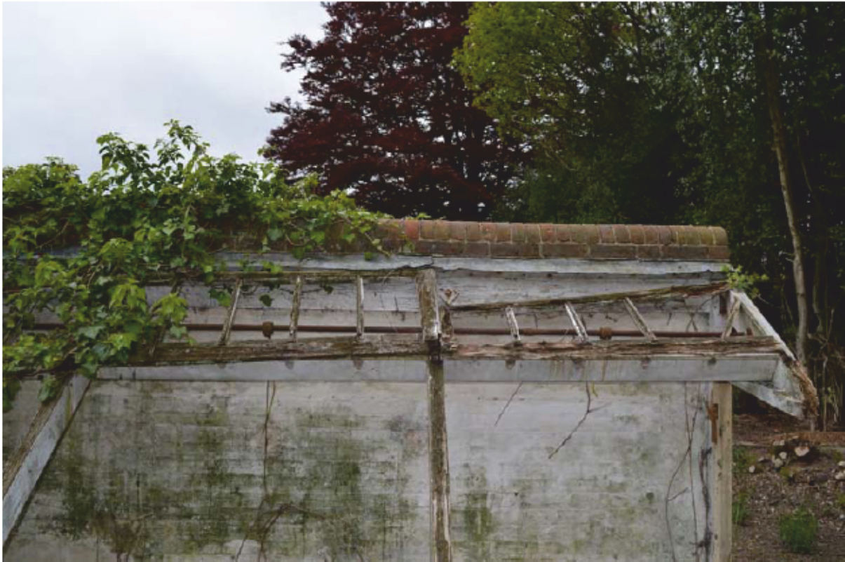
Plate 13: Northern lean-to, Building 1, Looking south (Photo #48)
