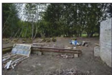
7494-0007 Combers Glasshouses - Building 2 - Bay 1. Facing west
