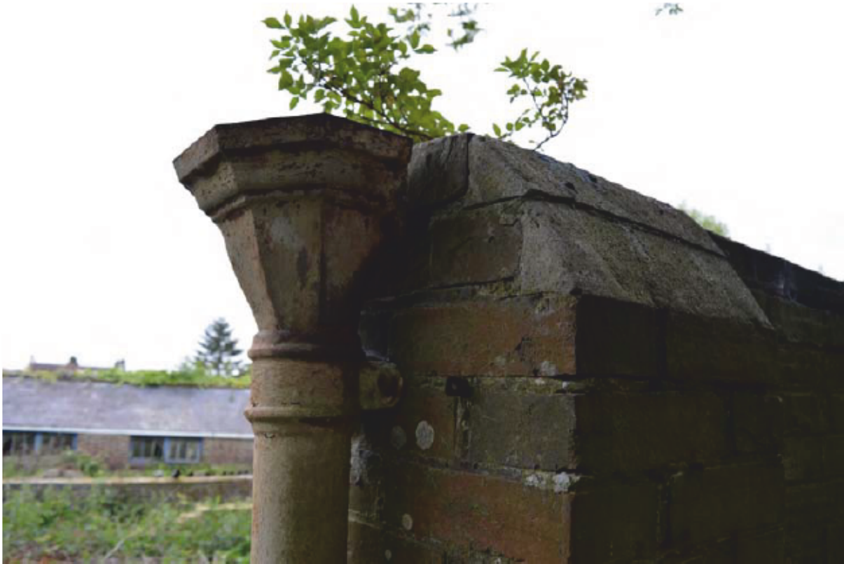
Plate 25: Building 2, downpipe and hopper head, looking south (Photo #102)
