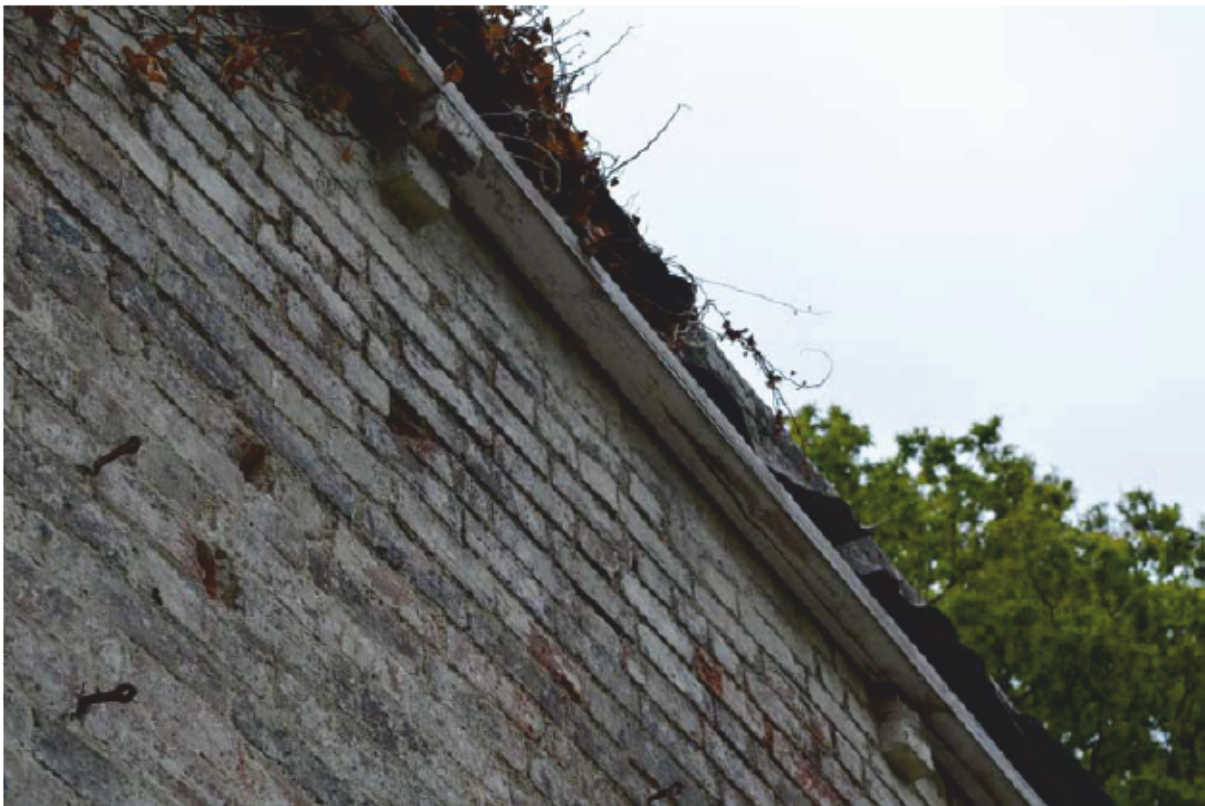
Plate 26: Building 2, ridge board on brick brackets, looking north-east (Photo #20)
