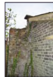
7494-0087 Combers Glasshouses - Building 5 - straight joint abutting kitchen garden wall. Facing east
