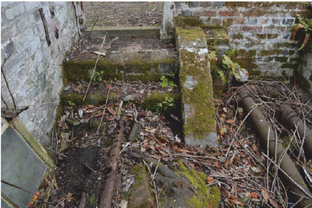
Plate 12: Northern lean-to, Building 1, doorway and steps down, looking west (Photo #58)
