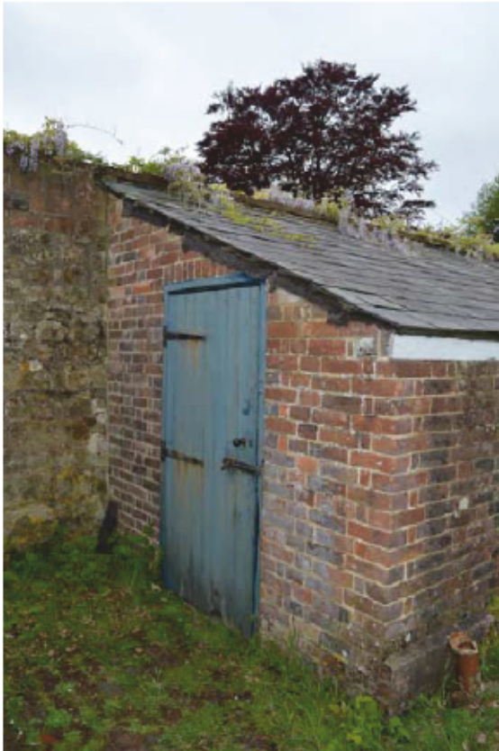
Plate 33: Building 4, east entrance, looking south-west (Photo #34)
