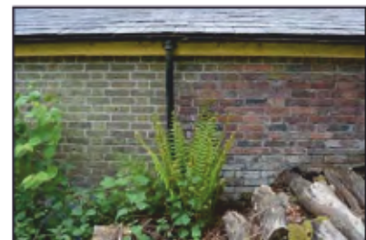
7494-0084 Combers Glasshouses - Building 5 - intersection of structures in west elevation. Facing east
