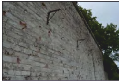
7494-0017 Combers Glasshouses - Building 2 - Bays 2 and 3, iron pegs and wires. Facing north-east
