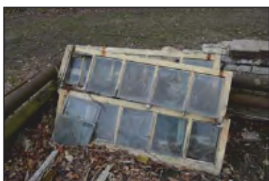
7494-0008 Combers Glasshouses - Building 2 - Bay 1. Facing west
