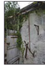
7494-0066 Combers Glasshouses - Building 1 - lever tackle and window opening device. Facing north-west
