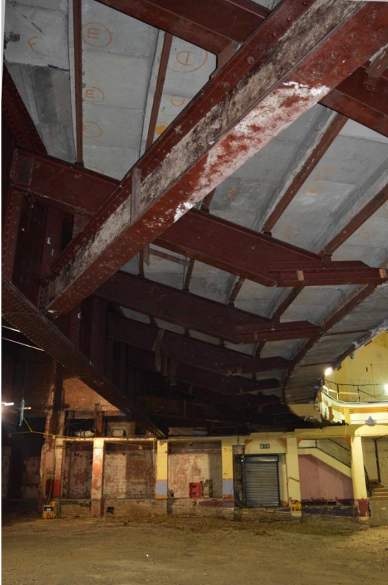
Plate 19: Ground floor, auditorium, detail of balcony construction, facing west (7533_0035)
