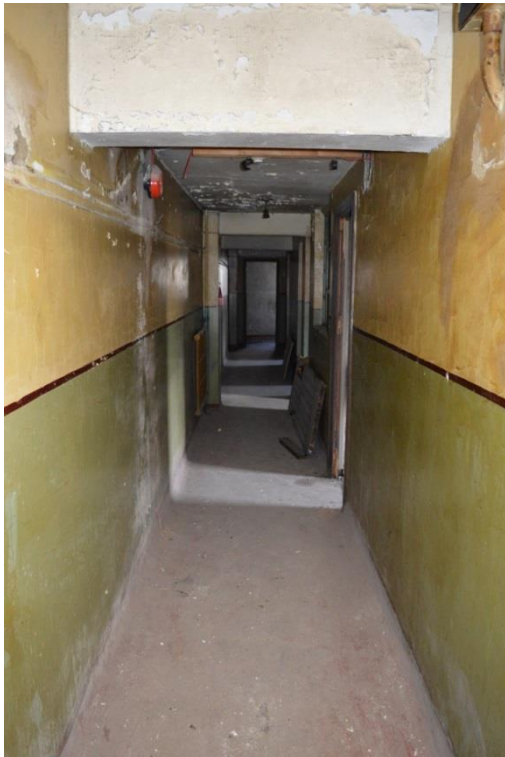
Plate 44: First floor, east wing, view of access corridor, facing north (7533_0104)
