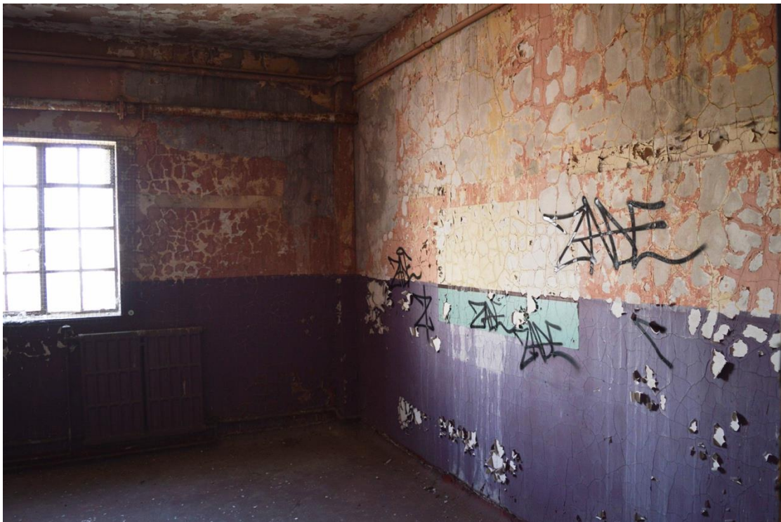
Plate 46: First floor, east wing, view of dressing room, facing south-east (7533_0114)
