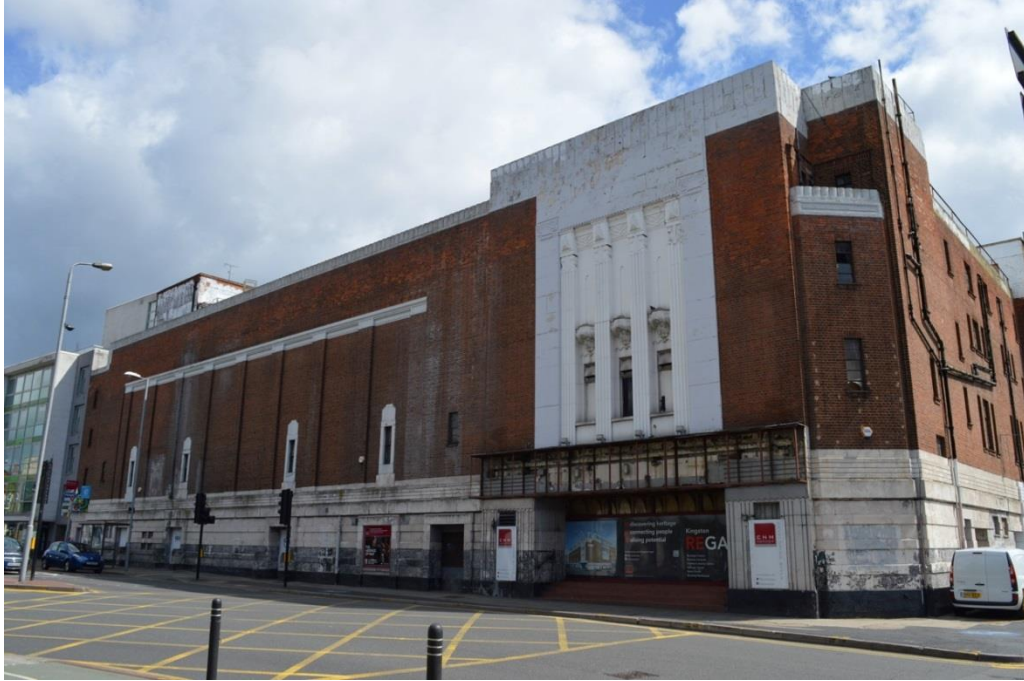
Plate 1: Exterior view of west elevation, facing north-east (7533_0001)
