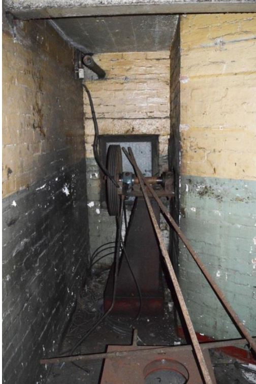
Plate 49: Third floor, east wing, intake room containing original projection equipment, facing north (7533_0108)
