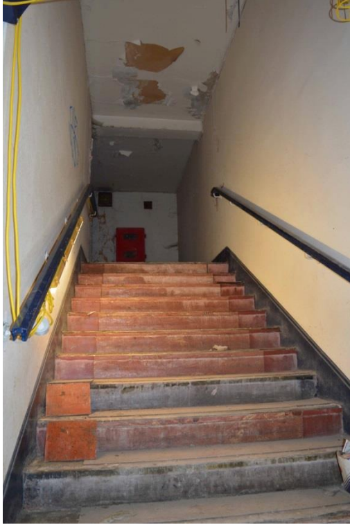
Plate 55: Ground floor, southern wing, western access stair, facing west (7533_0051)
