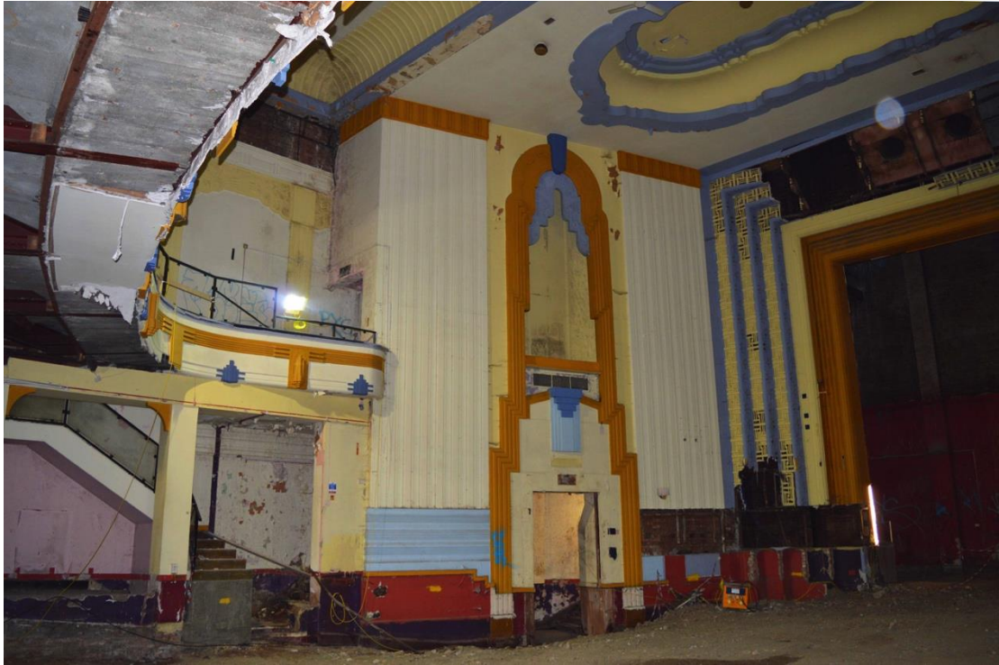
Plate 29: Ground floor, view of western side of auditorium, facing north-west (7533_0037)
