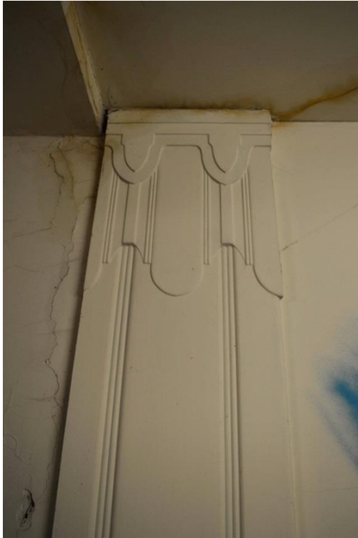
Plate 59: First floor, southern wing, plaster moulding to balcony support pillars, facing east (7533_0054)
