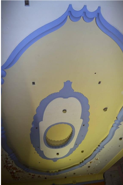
Plate 41: Third floor, balcony, oval moulded plasterwork ceiling, facing east (7533_0060)
