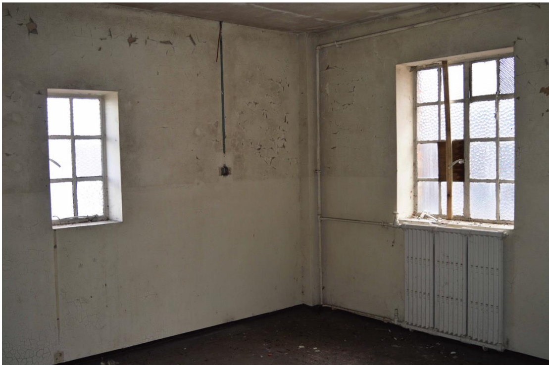
Plate 28: First floor, staff room and WC, facing south-east (7533_0097)
