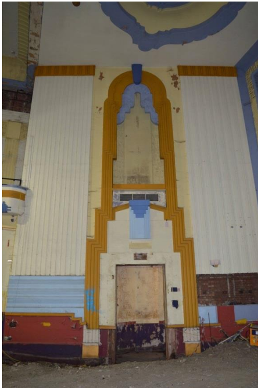
Plate 24: Ground floor, auditorium, Art Deco niche detailing, facing west (7533_0039)
