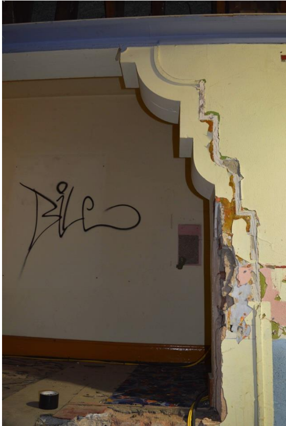
Plate 17: Ground floor, entrance hall, eastern balcony stair, facing east (7533_0030)
