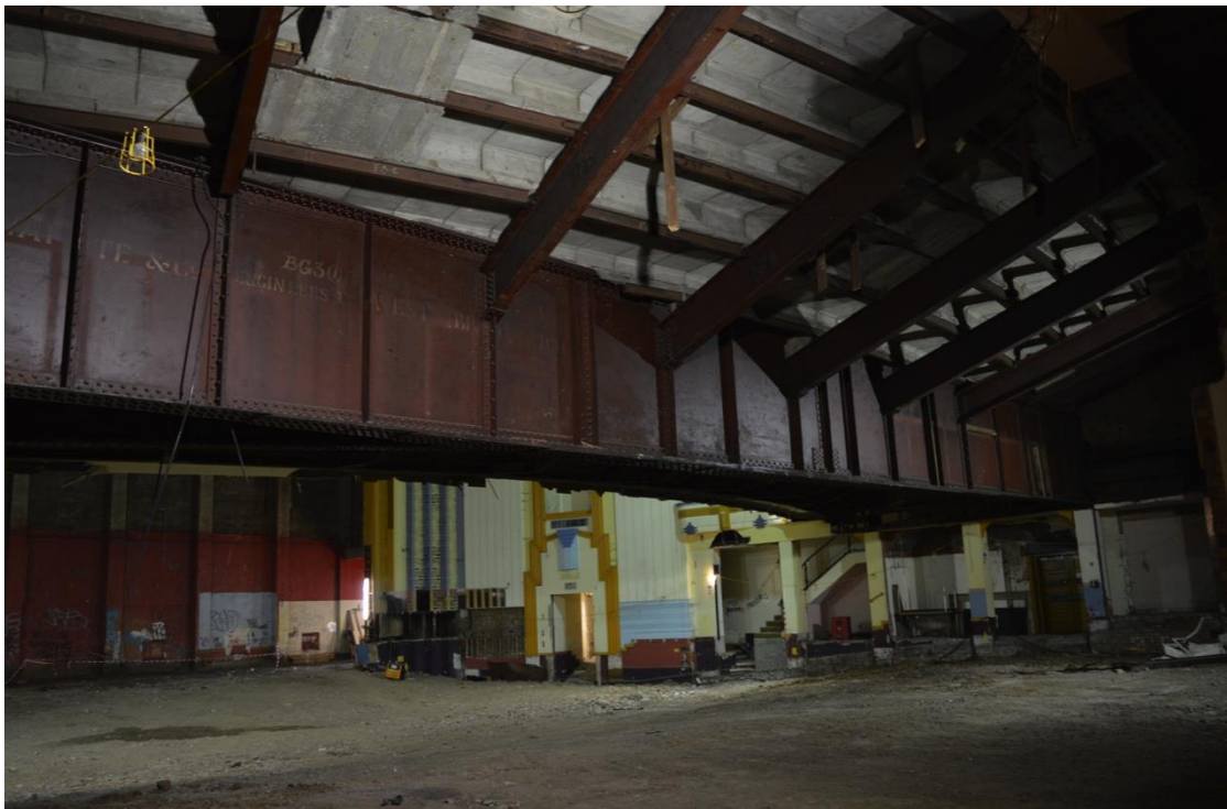
Plate 18: Ground floor, auditorium, detail of balcony construction, facing north-east (7533_0033)
