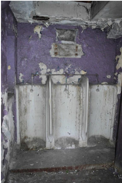
Plate 68: Third floor, southern wing, male WC with original fittings, facing west (7533_0084)
