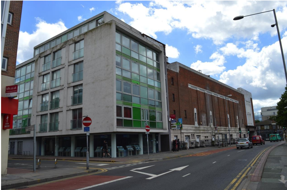
Plate 8: Exterior, general view of obscured north elevation, facing south-east (7533_0013)
