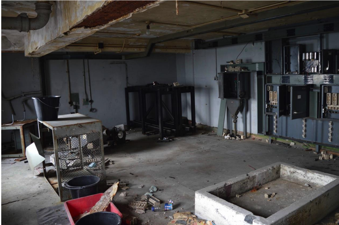
Plate 73: Third floor, southern wing, projector generator room, facing north-west (7533_0080)
