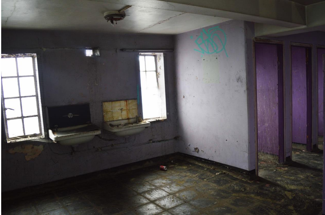
Plate 69: Third floor, southern wing, female WC with original fittings, facing south-west (7533_0083)
