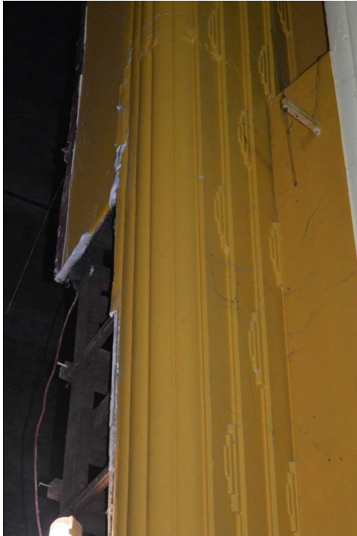
Plate 23: Ground floor, auditorium, proscenium arch stepped plaster detailing, facing north-east (7533_0043)
