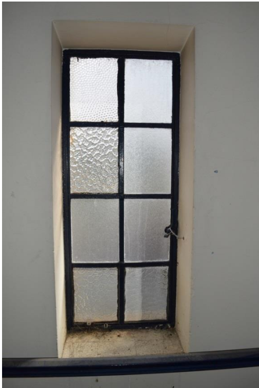
Plate 58: First floor, southern wing, western corridor window arrangement, facing west (7533_0092)
