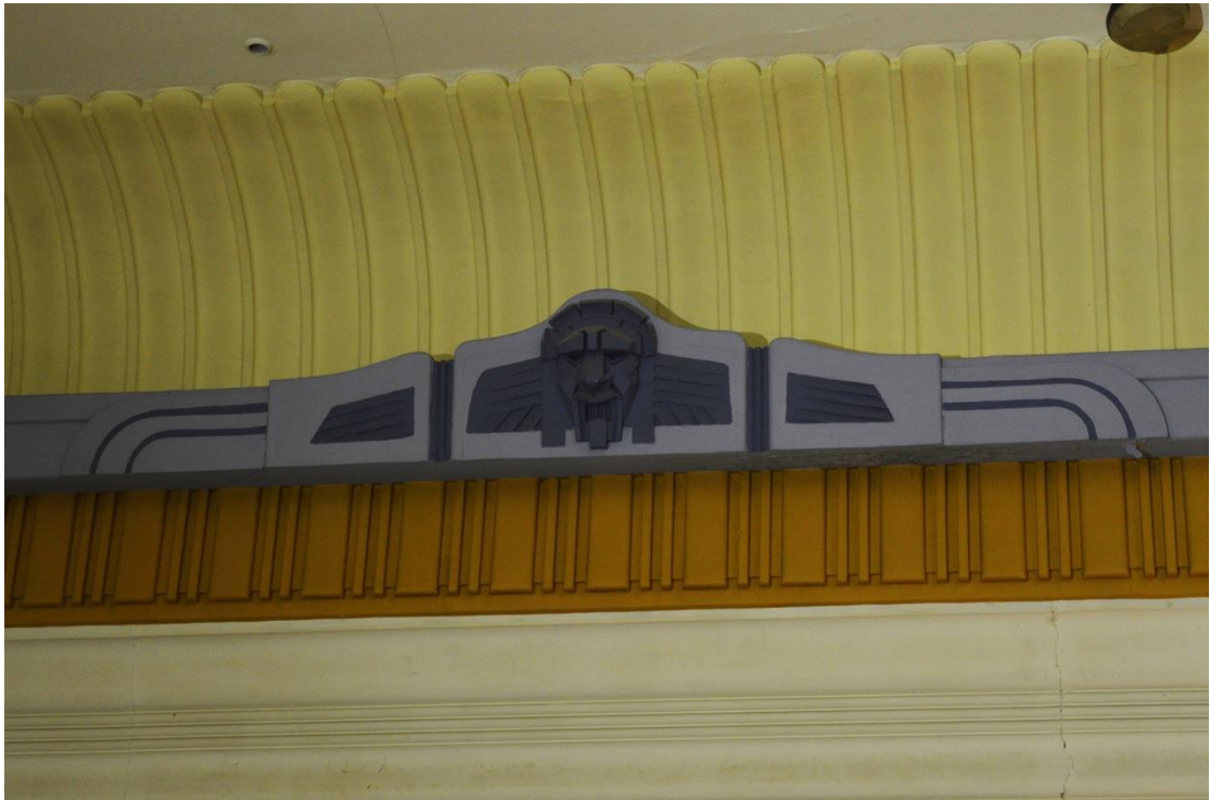
Plate 26: Ground floor, auditorium, lion's head plaster mould detail, facing north (7533_0063)
