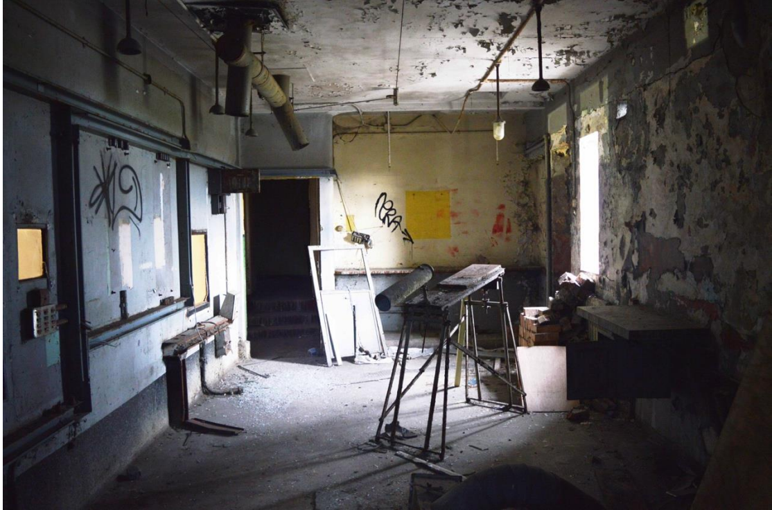
Plate 75: Fourth floor, southern wing, projection chamber, facing east (7533_0077)
