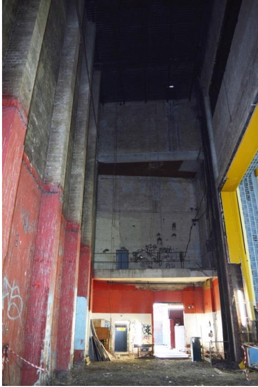
Plate 43: Ground floor, facing east wing; note electrician's gallery, facing east (7533_0046)
