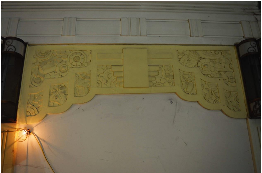
Plate 38: Third floor, balcony, moulded plasterwork detailing, facing east (7533_0058)
