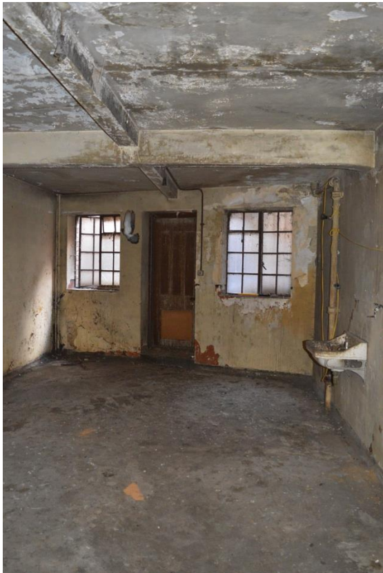
Plate 54: Second floor, west wing, former band room, facing south (7533_0101)
