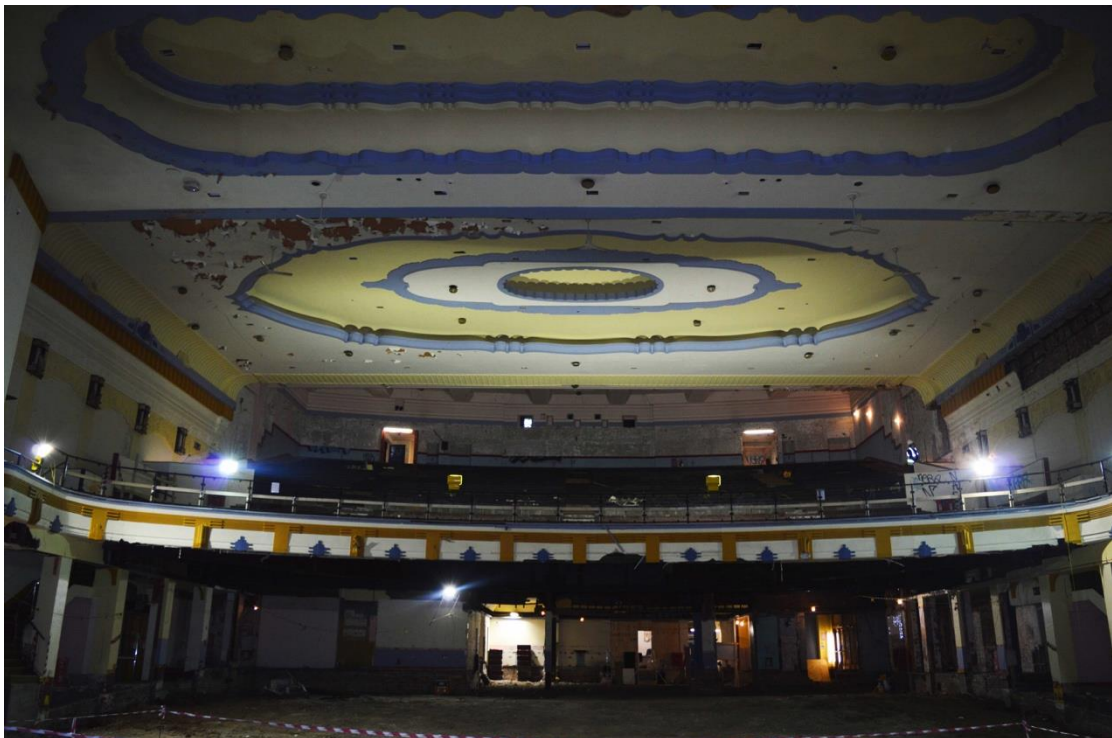
Plate 20: Ground floor, view of auditorium and balcony, facing south (7533_0045)
