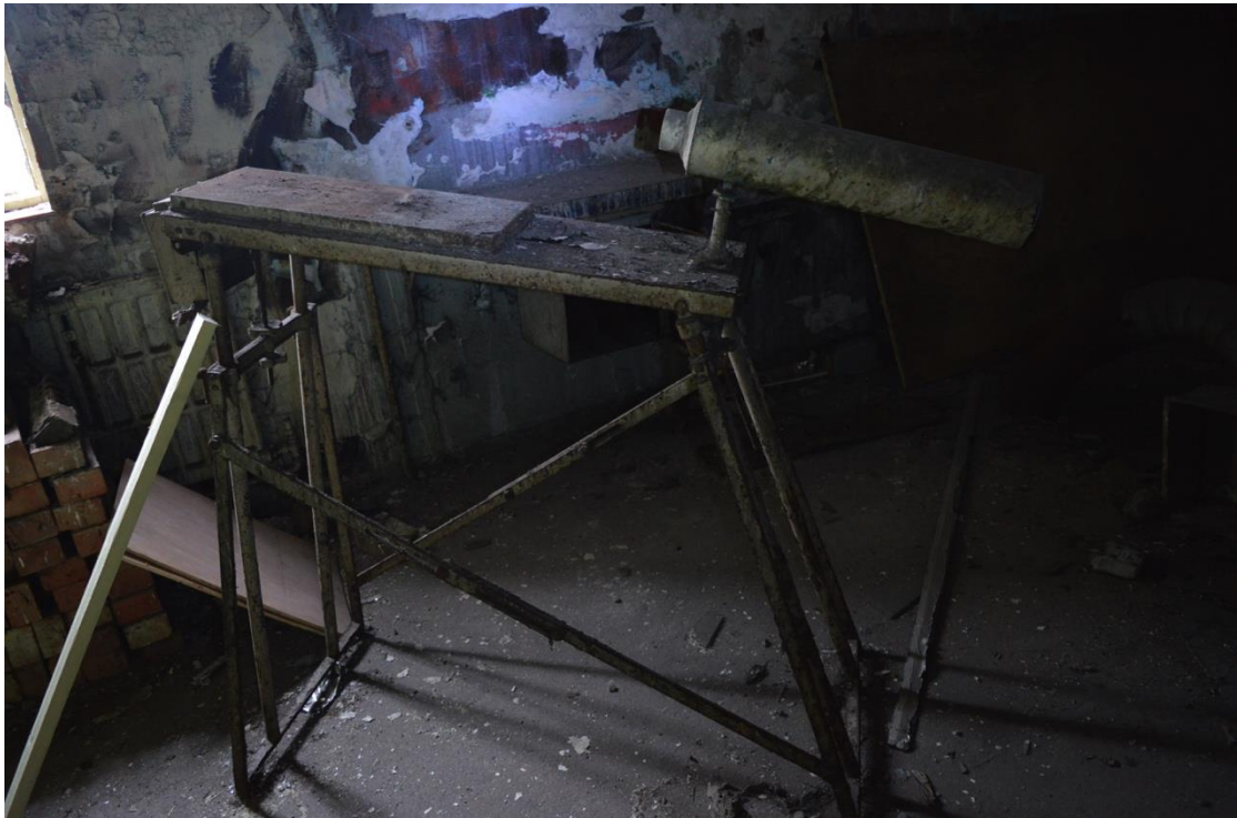
Plate 76: Fourth floor, southern wing, projection chamber, detail of original projection equipment, facing south-west (7533_0075)
