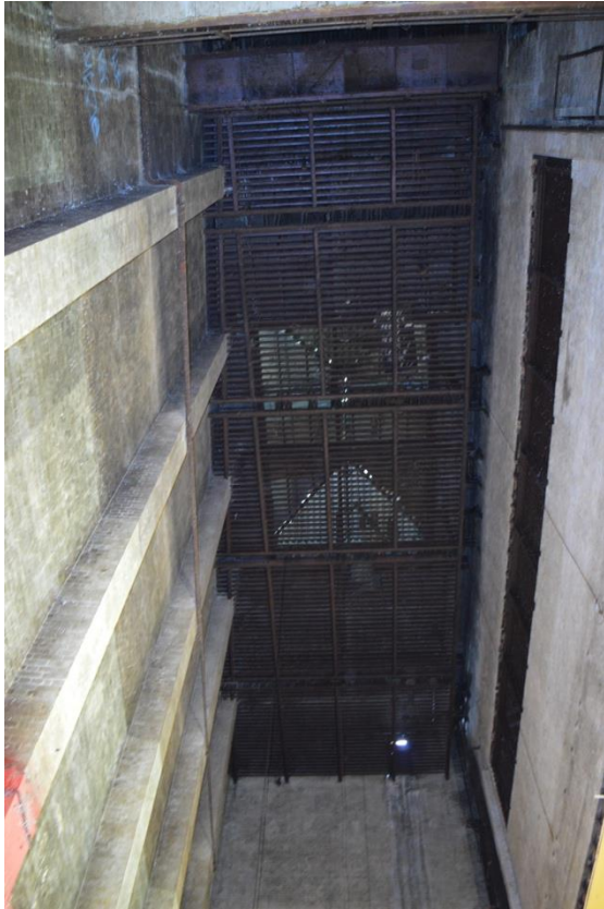
Plate 31: Ground floor, former stage roof and skylight, facing east (7533_0047)
