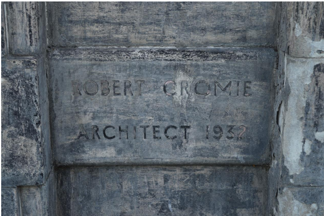
Plate 4: Exterior, west elevation, foundation stone detailing, facing east (7533-0006)
