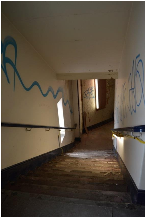
Plate 62: Second floor, southern wing, eastern access stair, facing east (7533_0091)
