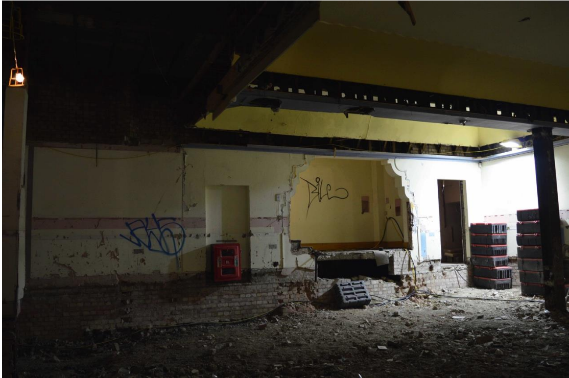
Plate 15: Ground floor, eastern end to entrance hall and stairs to balcony (former balcony pay box – now redundant), facing east (7533_0028)
