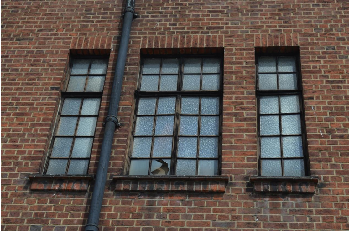
Plate 7: Exterior, detail of Crittall-style window arrangement, facing north (7533_0009)
