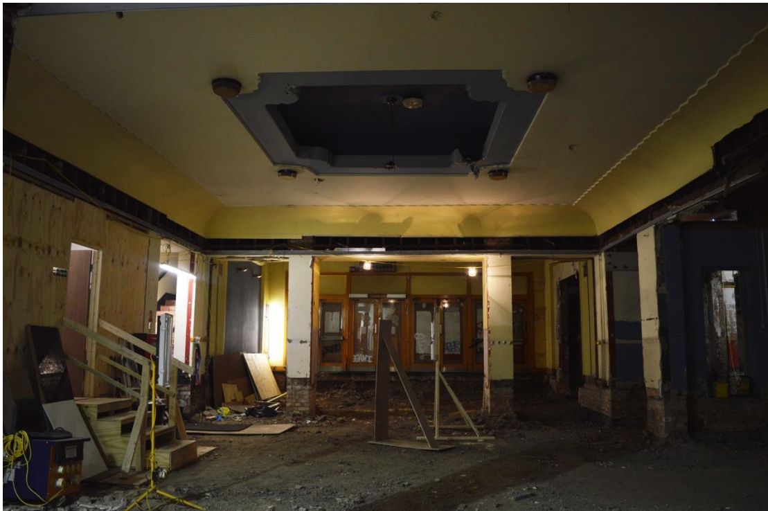
Plate 14: Ground floor, entrance hall and lobby, facing west (7533_0024)
