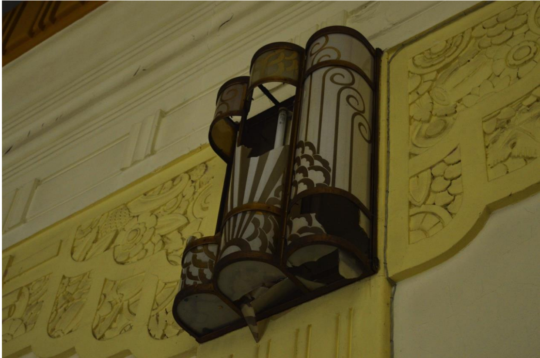
Plate 37: Third floor, balcony, original light fitting, facing north-east (7533_0062)
