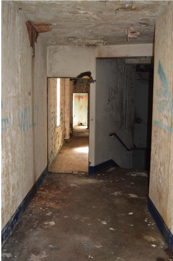
Plate 33: First floor, western access corridor and W/C, facing north (7533_0099)
