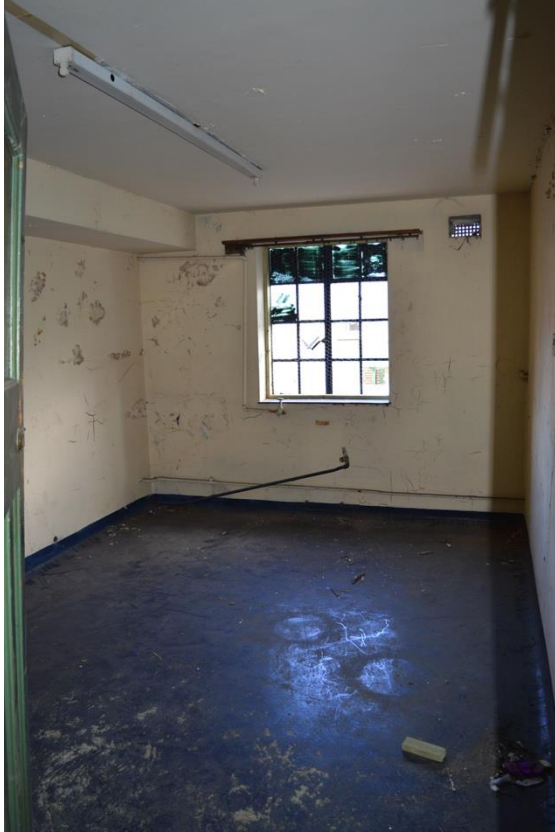
Plate 53: Fourth floor, east wing dressing room detail, facing east, (7533_0105)
