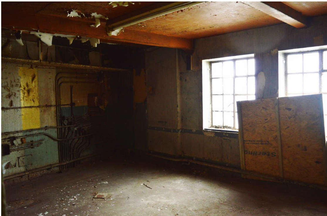
Plate 78: Fourth floor, southern wing, extract fan chamber, facing south-east (7533_0072)
