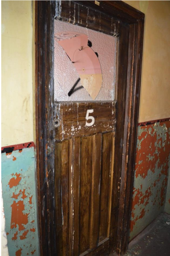
Plate 45: Third floor, east wing, dressing room door detailing, facing south-east (7533_0110)
