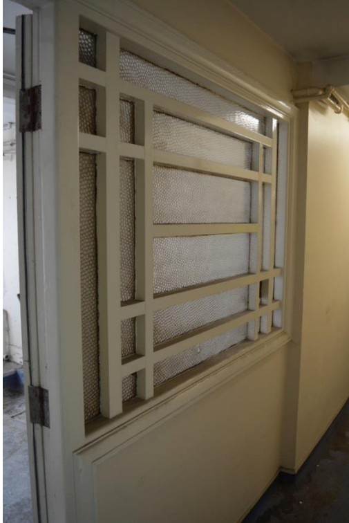
Plate 67: Second floor, southern wing, glazed panelling to corridor, facing south-east (7533_0088)
