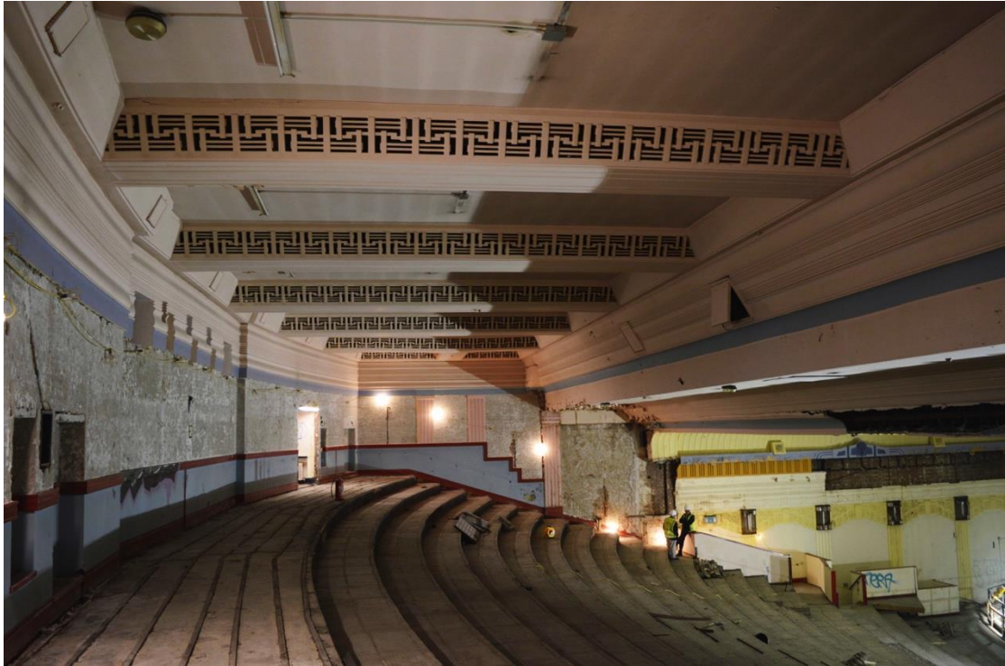
Plate 39: Third floor, rear of balcony with Greek key design downstand patterning and attendant seat alcoves, facing west (7533_0065)
