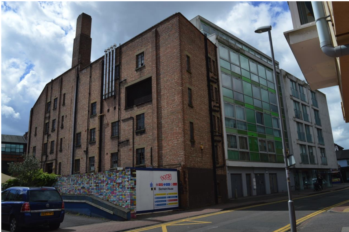
Plate 10: Exterior, view of northern end of east elevation (eastern wing), facing south-west (7533_0012)
