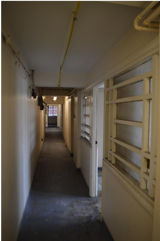
Plate 66: Second floor, southern wing, access corridor, facing east (7533_0087)
