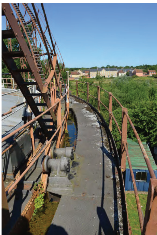
Plate 26: Detail of tank platform and guard rail, facing north (TYB15-0027)
