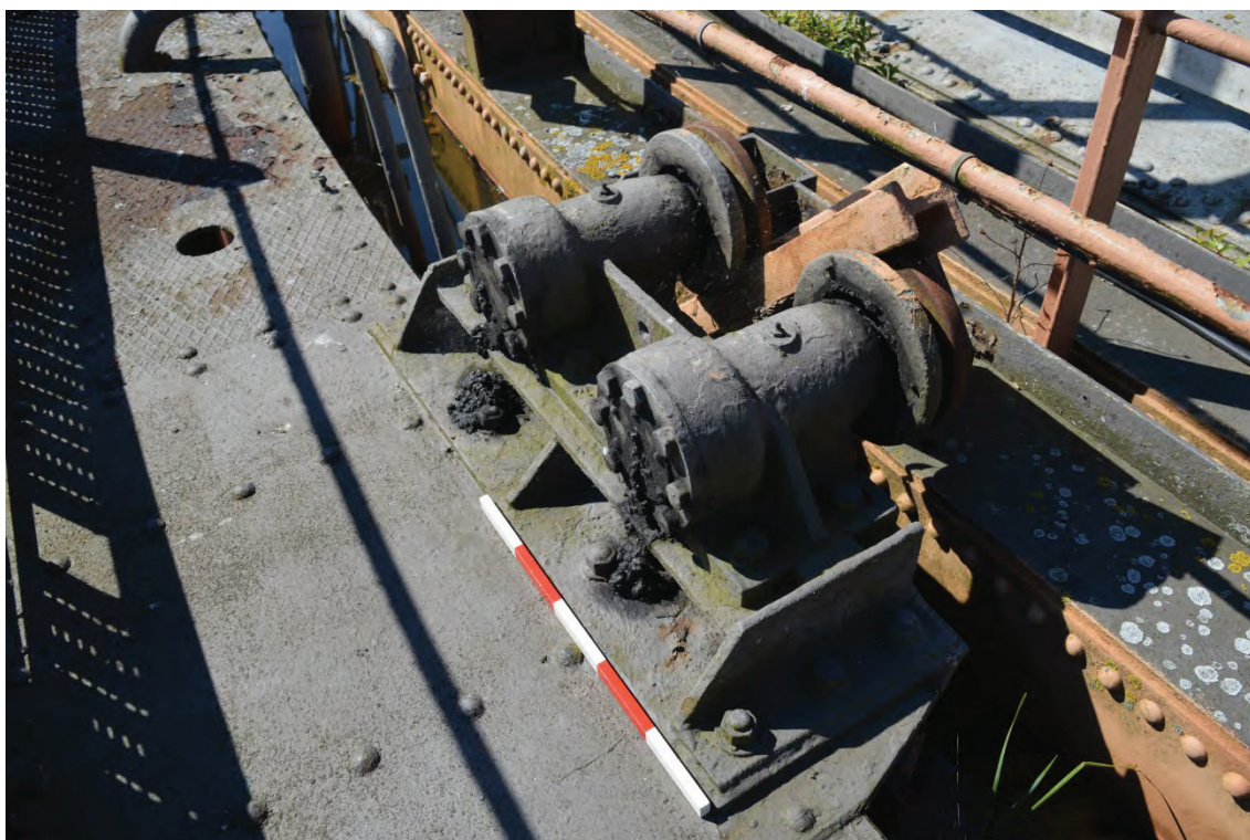
Plate 12: Detail of carriage wheel construction located on the inner edge of the tank platform, facing south (TYB15-0029)
