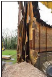
TYB15-0115 Section through lifts and tank wall. Facing north-west
