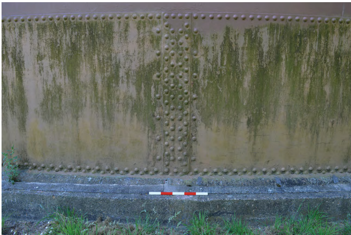
Plate 21: Detail of riveted steel plate tank construction, facing south (TYB15-0014)
