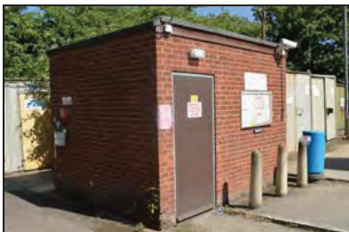
TYB15-0058 Communication room. Facing north
