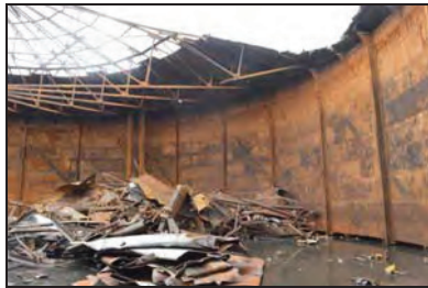
TYB15-0113 Interior of the gasholder. Facing north-west
