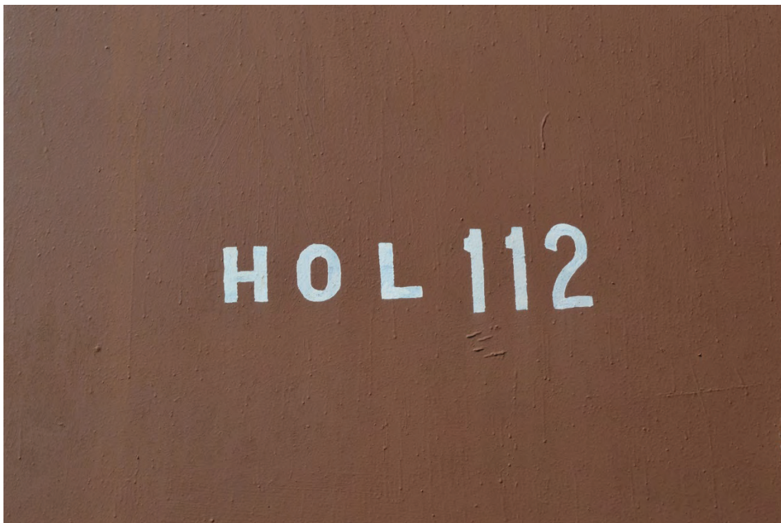
Plate 27: Detail of the gasholder identification marking and acrylic paint covering, facing west (TYB15-0003)
