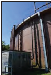
TYB15-0055 Concrete housing and tank elevation. Facing south
