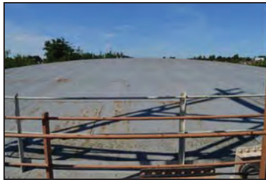
TYB15-0023 Crown. Facing south-west
