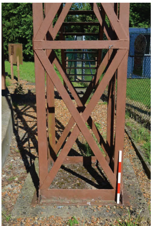
Plate 24: Detail of staircase base and support standard arrangement, facing north (TYB15-0018)
