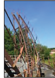
TYB15-0051 Lift stairs. Facing west
