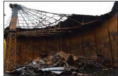
TYB15-0114 Interior of the gasholder. Facing north-west
