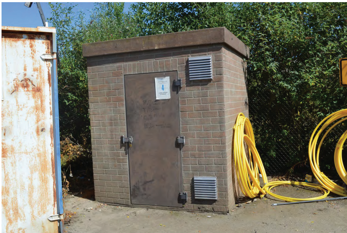
Plate 37: View of the Lorry Driver Store located to the site's eastern boundary, facing east (TYB15-0059)
