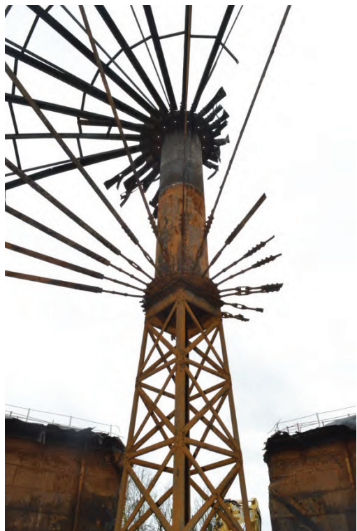
Plate 5: Detail of the central stanchion and pedestal rest, facing south-west (TYB15-0094)
