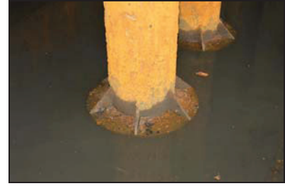
TYB15-0108 Base of pipes. Facing east
