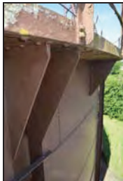
TYB15-0052 Brackets supporting the tank platform. Facing west
