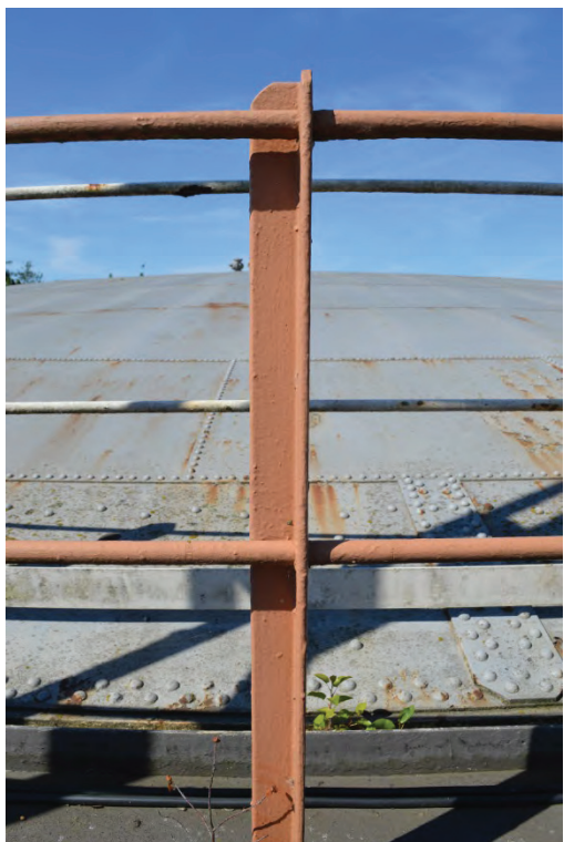
Plate 15: Detail of outer lift guard rail arrangement, facing west (TYB15-0044)
