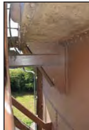
TYB15-0053 Brackets supporting the tank platform. Facing south
