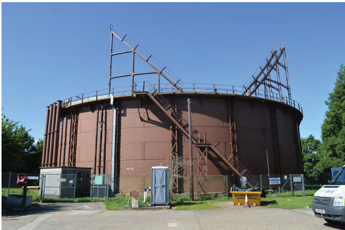
Plate 1: General view of the gasholder, facing west (TYB15-0001)
