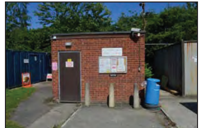
TYB15-0057 Communication room. Facing north-west
