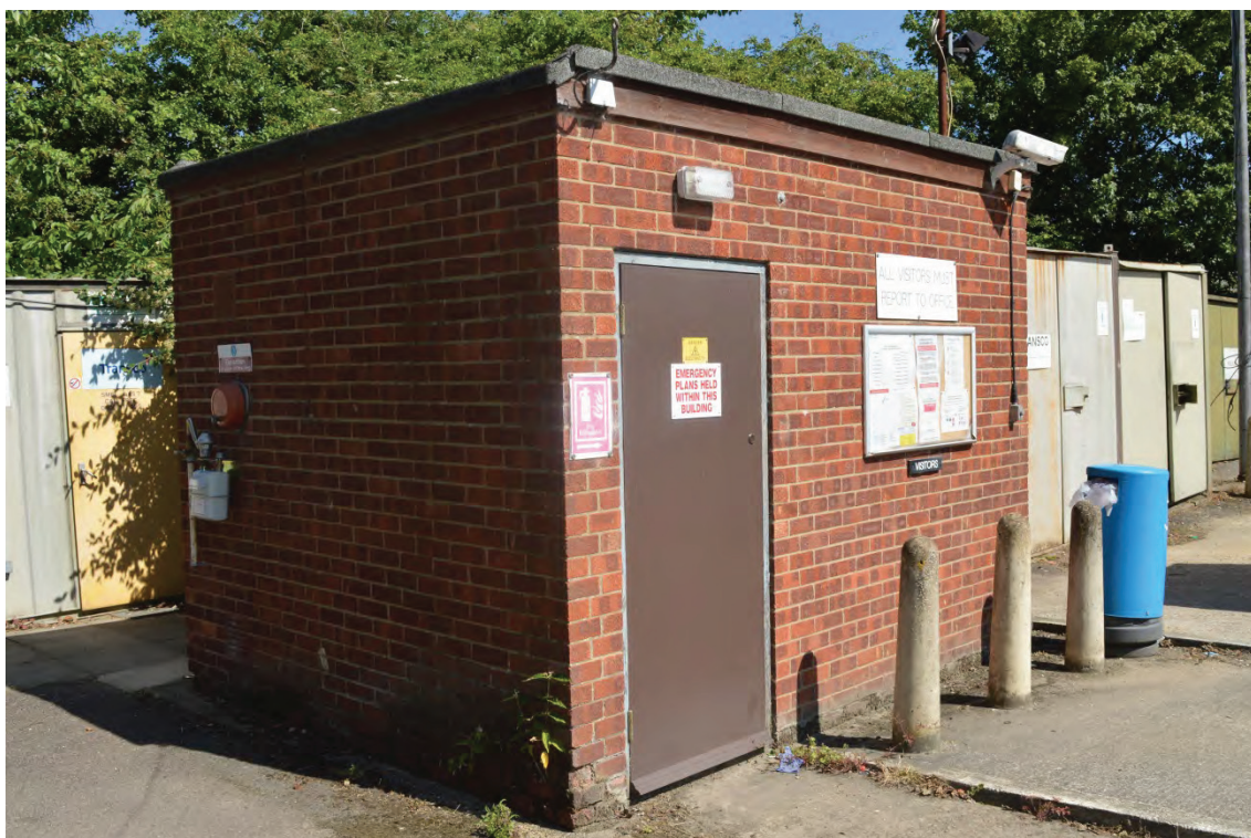
Plate 36: View of the brick built Communication Room, facing north-east (TYB15-0058)
