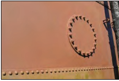
TYB15-0016 Access hatch. Facing west
