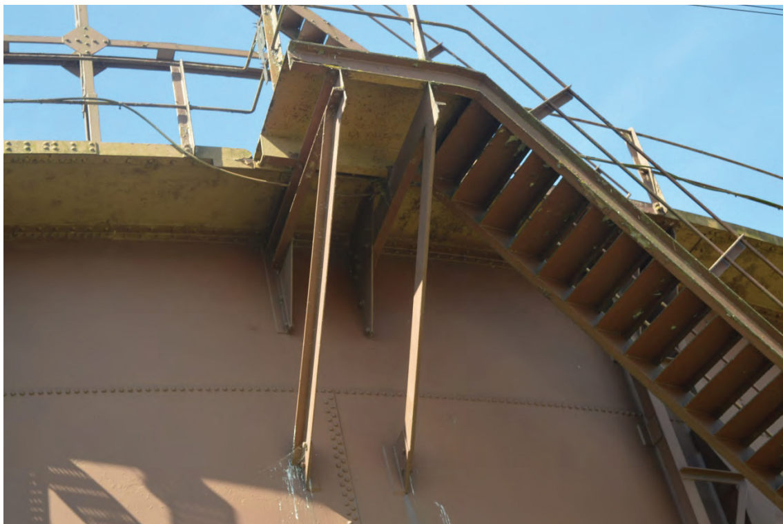
Plate 25: Detail of staircase landing and tank platform supports, facing west (TYB15-0064)
