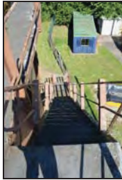
TYB15-0049 Stairs down from tank platform. Facing west
