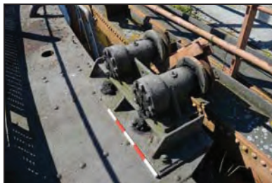
TYB15-0029 Carriage detail. Facing south
