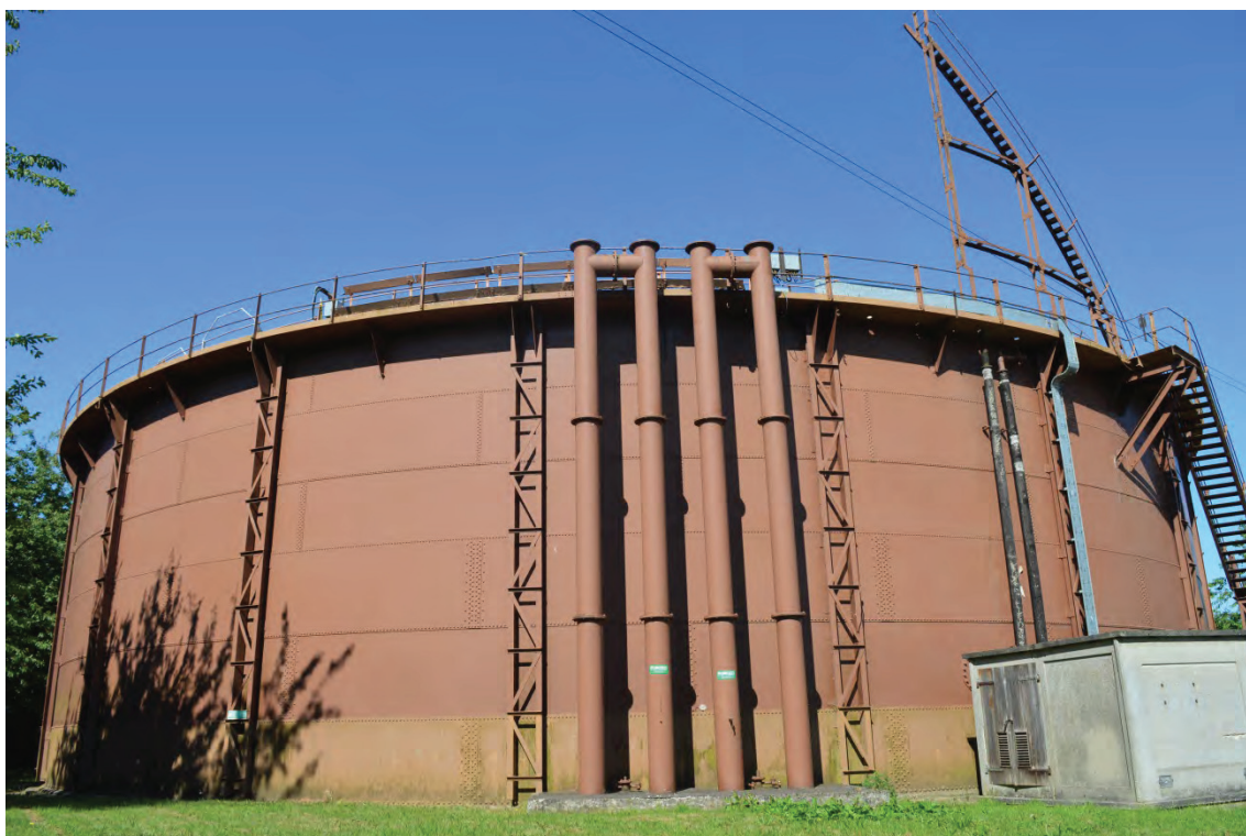
Plate 20: General view of gasholder tank construction, facing north-west (TYB15-0004)
