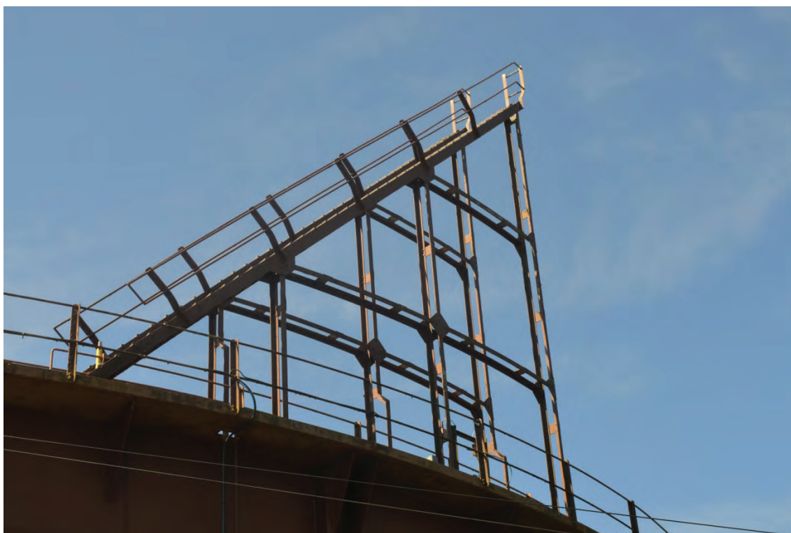
Plate 16: Detail of lift staircase construction, facing north-west (TYB15-0061)
