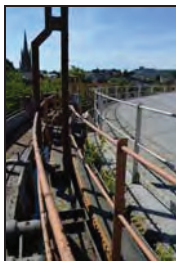
TYB15-0028 Three lift arrangement. Facing south
