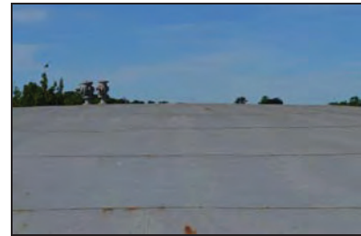
TYB15-0024 Crown. Facing south-west
