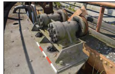
TYB15-0030 Carriage detail. Facing south
