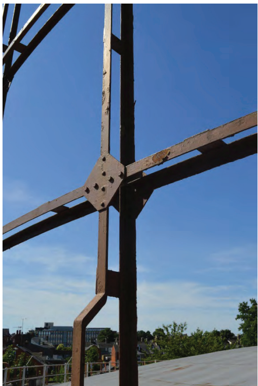
Plate 17: Detail of middle access stair construction, facing south-west (TYB15-0041)
