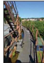
TYB15-0027 Tank platform. Facing west
