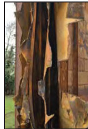
TYB15-0116 Section through lifts and tank wall. Facing north-west
