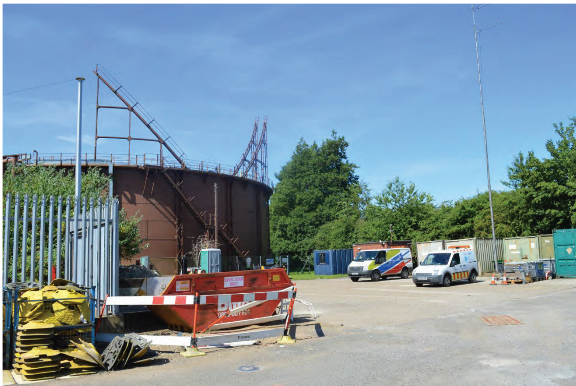
Plate 33: General view of the site compound containing ancillary brick buildings, cargo storage units and vehicle access areas to the east of the gasholder, facing north-west (TYB15-0062)
