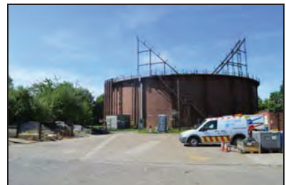
TYB15-0060 View to the gasholder. Facing south
