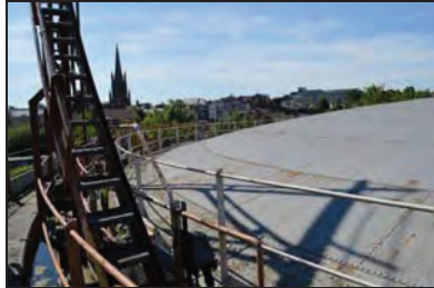
TYB15-0050 Crown, lift stairs. Facing south-east
