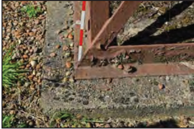
TYB15-0019 Stair support base. Facing south-west
