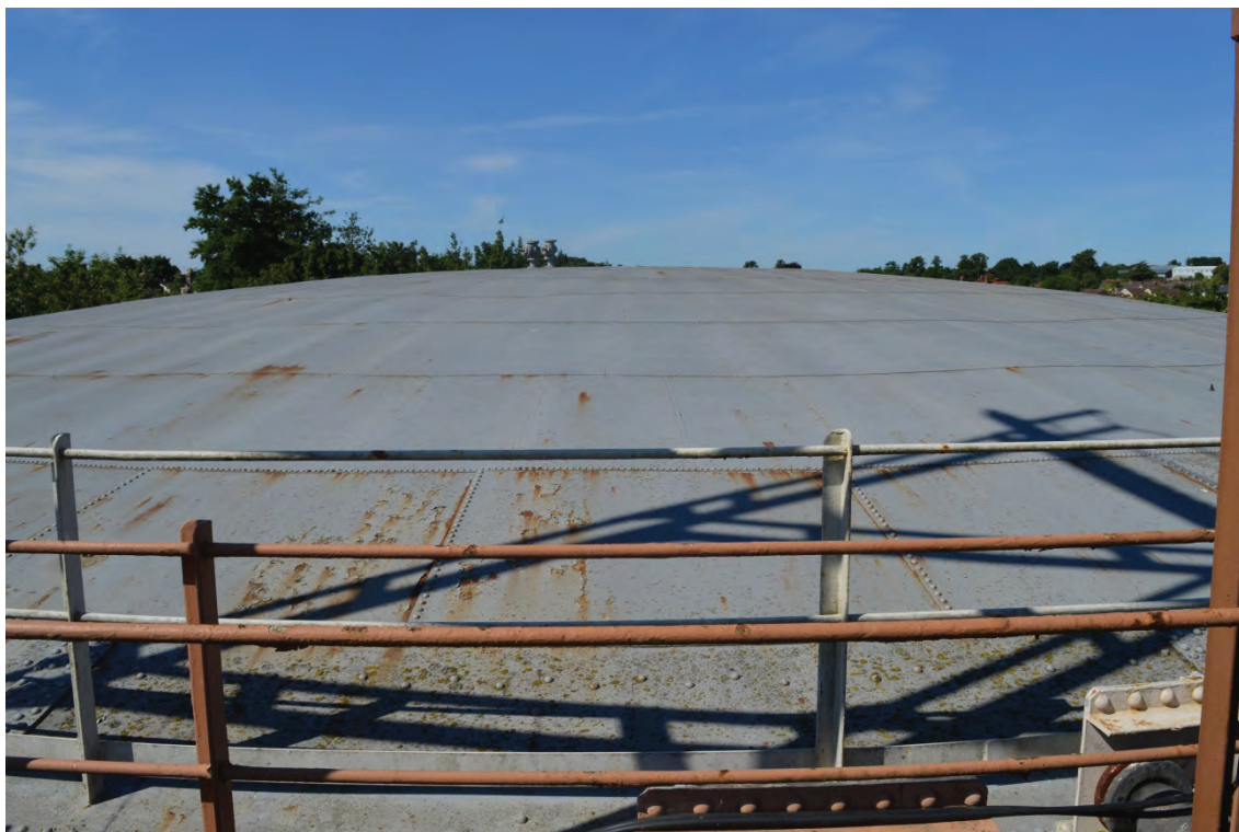
Plate 3: Detail of the gasholder bell crown construction, facing west (TYB15-0023)
