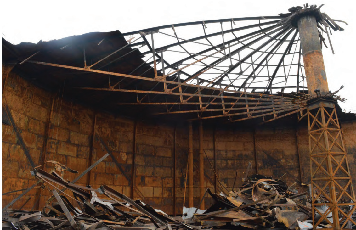
Plate 4: View of the truss construction supporting the bell, facing east (TYB15-0108)
