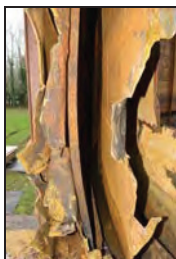
TYB15-0118 Section through lifts and tank wall. Facing north-west
