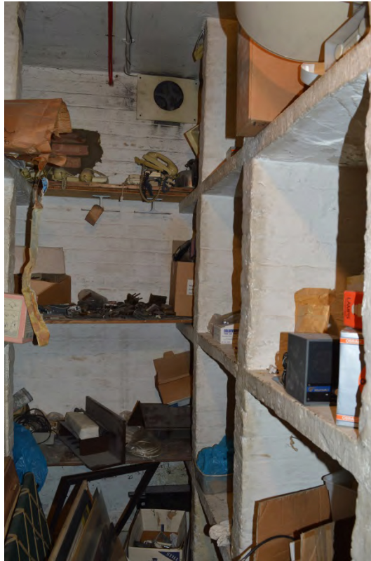
Plate 15: Wine racks in a store within the basement, 154 Bayswater Road (Photo 184).
