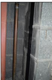
7330-0043 7330_Room 119. Facing north
