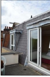
7330-0226 7330_Principal Elevation. Facing north-west
