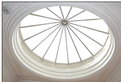
7330-0278 7330_Second Floor Landing. Facing west
