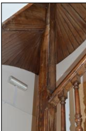
7330-0277 7330_Servant's Staircase. Facing north-east
