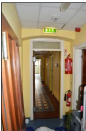
7330-0187 7330_Corridor in Basement. Facing south
