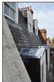
7330-0026 7330_Roof of 6 Bayswater Road. Facing west
