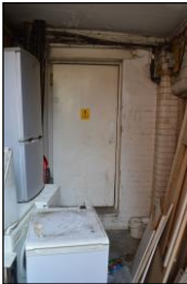
7330-0382 7330_Lower Ground Floor Front. Facing east
