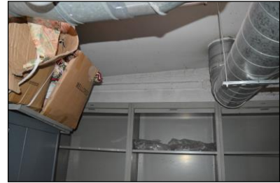
7330-0363 7330_Store. Facing north
