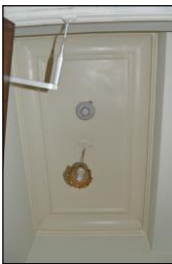
7330-0262 7330_Lobby to Room 148. Facing south
