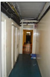
7330-0175 7330_Corridor in Basement. Facing north
