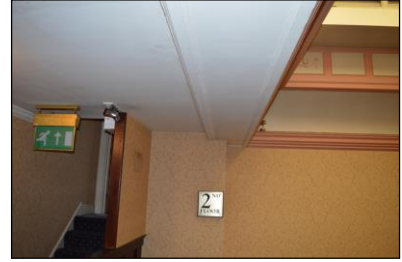
7330-0063 7330_Second Floor Landing. Facing west
