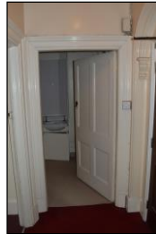
7330-0290 7330_Room 145. Facing east
