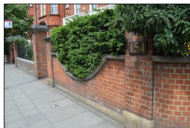
7330-0131 7330_Front Wall. Facing north-west
