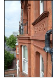
7330-0051 7330_Facade of 6 Palace Court. Facing west
