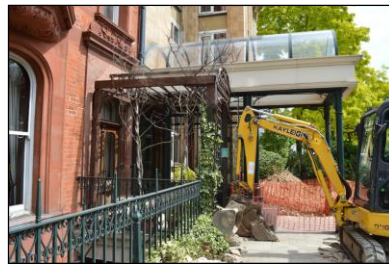
7330-0128 7330_Principal elevation. Facing east
