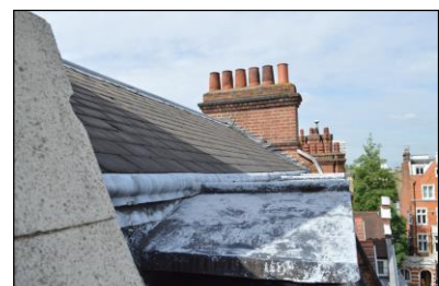
7330-0030 7330_Roof of 6 Palace Court. Facing south-west
