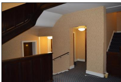
7330-0085 7330_Main Staircase. Facing north-east
