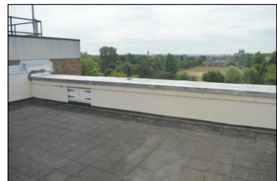
7330-0390 7330_Sixth Floor Roof. Facing south
