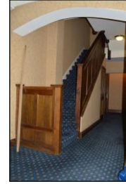
7330-0153 7330_Servant's Staircase. Facing east
