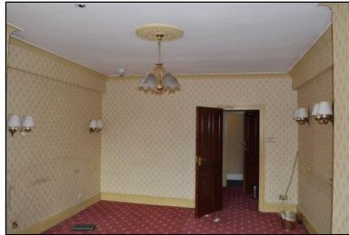
7330-0080 7330_Room 114. Facing north
