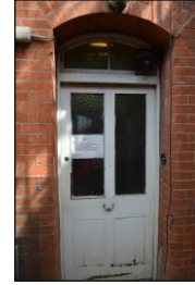
7330-0378 7330_Lower Ground Floor Entrance. Facing north
