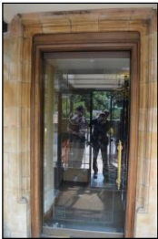
7330-0142 7330_Front Door to 154 bayswater Road. Facing north
