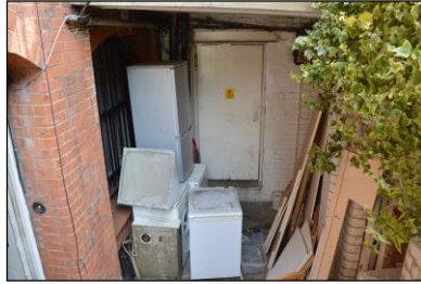
7330-0380 7330_Lower Ground Floor Front. Facing east
