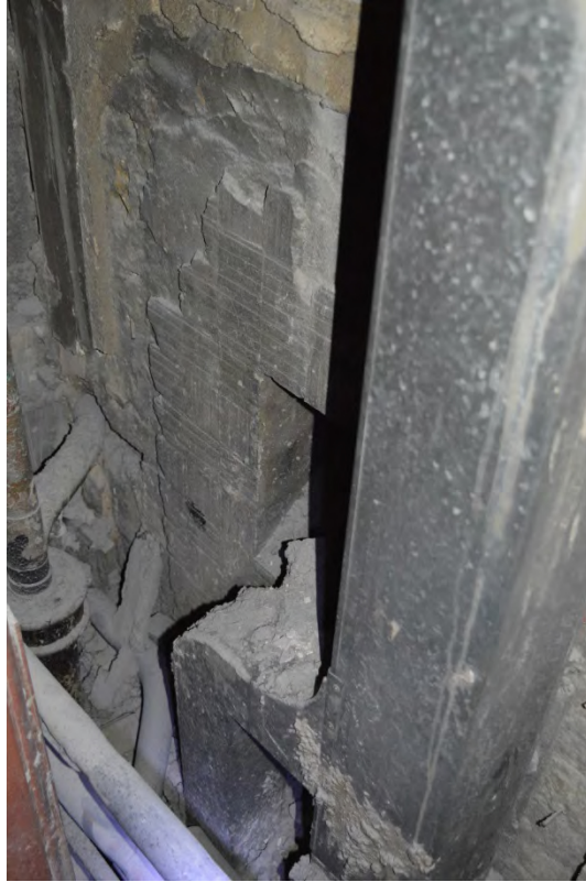
Plate 41: Former fireplace within a void in room 119, 154 Bayswater Road (Photo 42).
