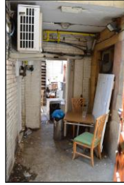
7330-0212 7330_Lower Ground Floor Front. Facing west
