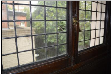
7330-0094 7330_Room 105. Facing north-east
