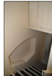
7330-0342 7330_Lower Ground Floor Staircase. Facing east
