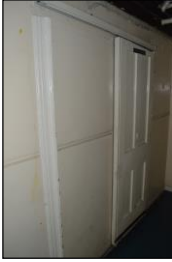
7330-0181 7330_Corridor in Basement. Facing north-west
