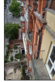
7330-0228 7330_Principal Elevation. Facing west
