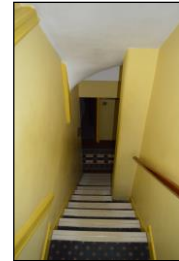
7330-0171 7330_Stairs to Basement. Facing west
