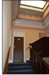
7330-0065 7330_Main Staircase. Facing east
