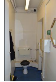
7330-0201 7330_Toilet in Corridor. Facing east
