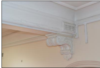
7330-0275 7330_Second Floor Landing. Facing west
