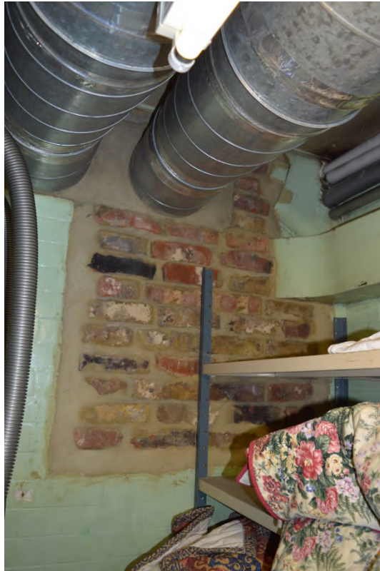
Plate 58: Blocked arch in basement store room, 6 Palace Court (Photo 368).
