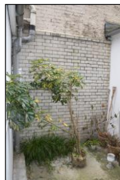
7330-0356 7330_Yard. Facing north
