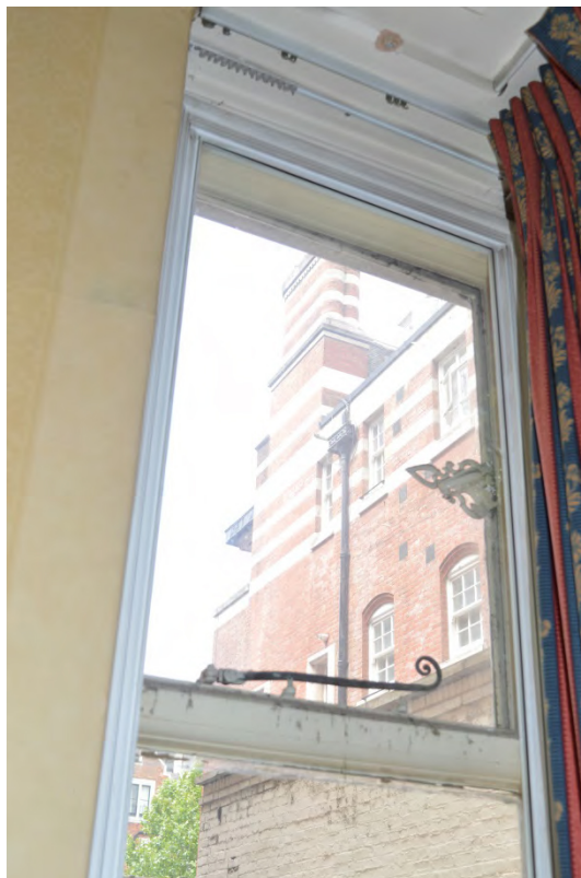
Plate 32: Room 102, Bay window detailing, 154 Bayswater Road (Photo 169).
