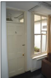
7330-0352 7330_Flat 136. Facing north
