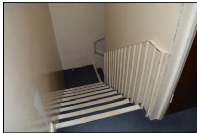
7330-0341 7330_Lower Ground Floor Staircase. Facing north
