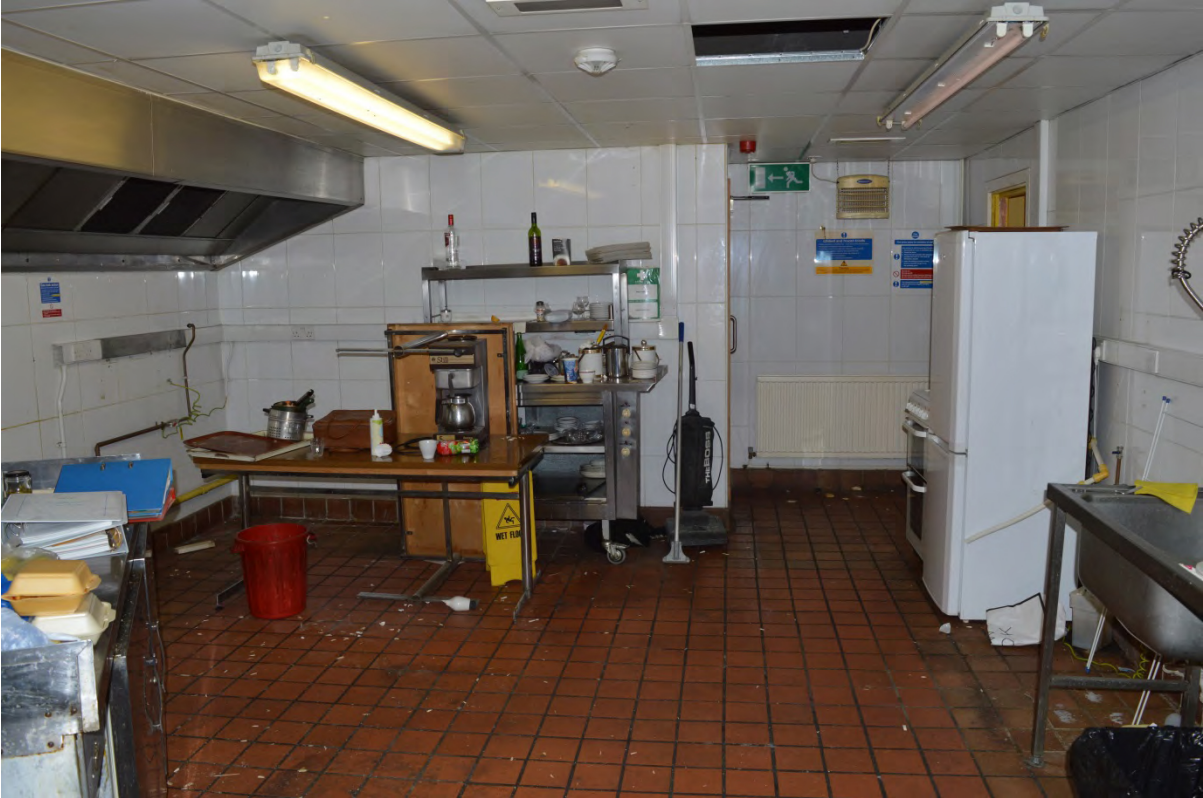
Plate 13: Kithcen in the basement of 154 Bayswater Road (Photo 198).
