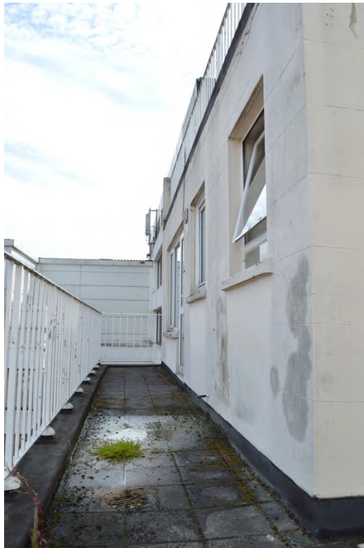
Plate 8: Fifth floor balcony, 154 Bayswater Road (Photo 29).
