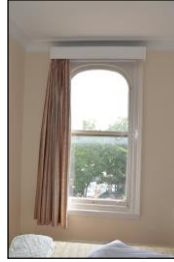
7330-0272 7330_Room 147. Facing south
