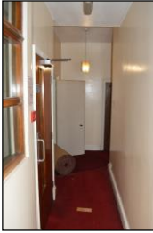
7330-0229 7330_Fourth Floor Corridor. Facing south
