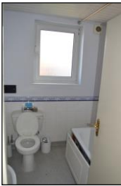
7330-0010 7330_Room 129. Facing north
