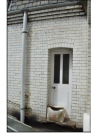
7330-0258 7330_Roof around skylight. Facing north
