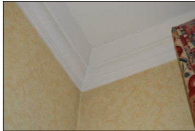
7330-0068 7330_Room 110. Facing north-west
