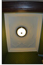
7330-0092 7330_Lobby to Room 105. Facing west
