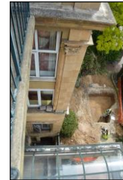
7330-0054 7330_Room 121 Balcony and façade of 154 Baswater Road. Facing south-east
