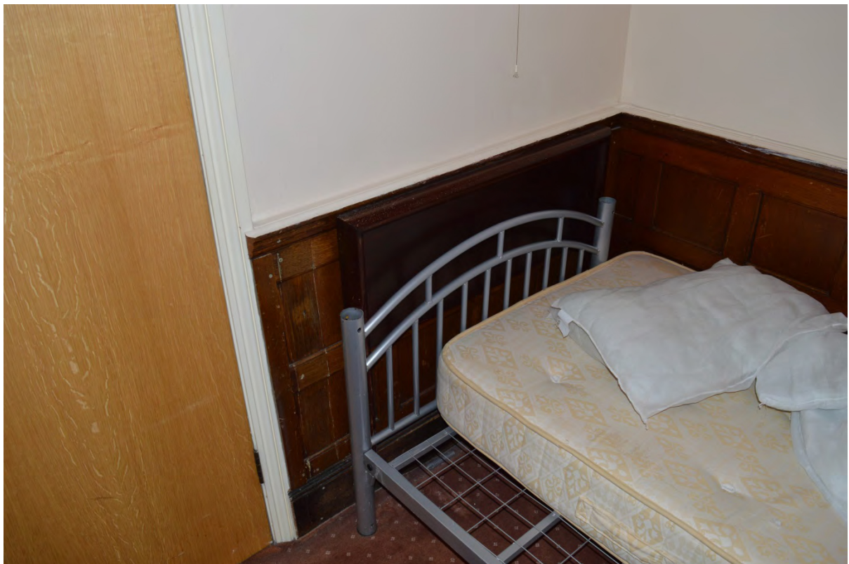
Plate 80: Flat 142 dado and chair rail, refitted to an inserted wall, 6 Palace Court (Photo 311).
