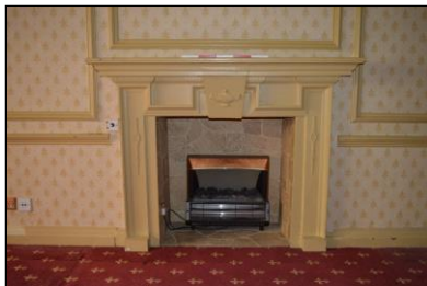
7330-0097 7330_Room 106. Facing east
