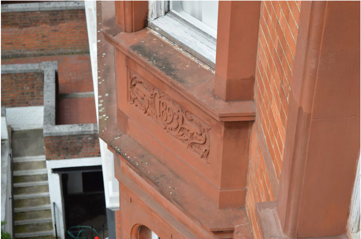
Plate 44: Date plaque on façade of 6 Palace Court (Photo 52).
