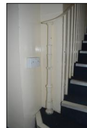
7330-0345 7330_Lower Ground Floor Staircase. Facing west
