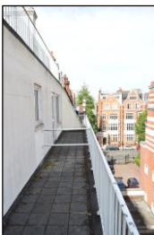
7330-0025 7330_Fourth Floor Balcony. Facing west
