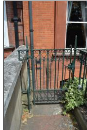
7330-0125 7330_Gate above lower ground floor. Facing north
