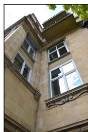
7330-0224 7330_Principal Elevation. Facing north- west
