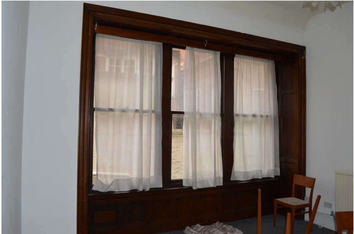
Plate 77: Bay window, flat 138, 6 palace court (Photo 338).
