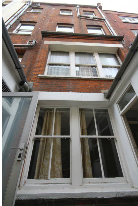
Plate 46: Rear elevation of 6 Palace Court (Photo 360).
