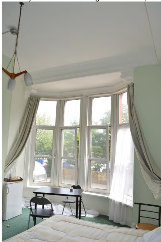
Plate 53: Console brackets within the orial bay, room 139, 6 Palace Court (Photo 318).
