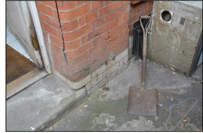
7330-0381 7330_Lower Ground Floor Front. Facing north-east
