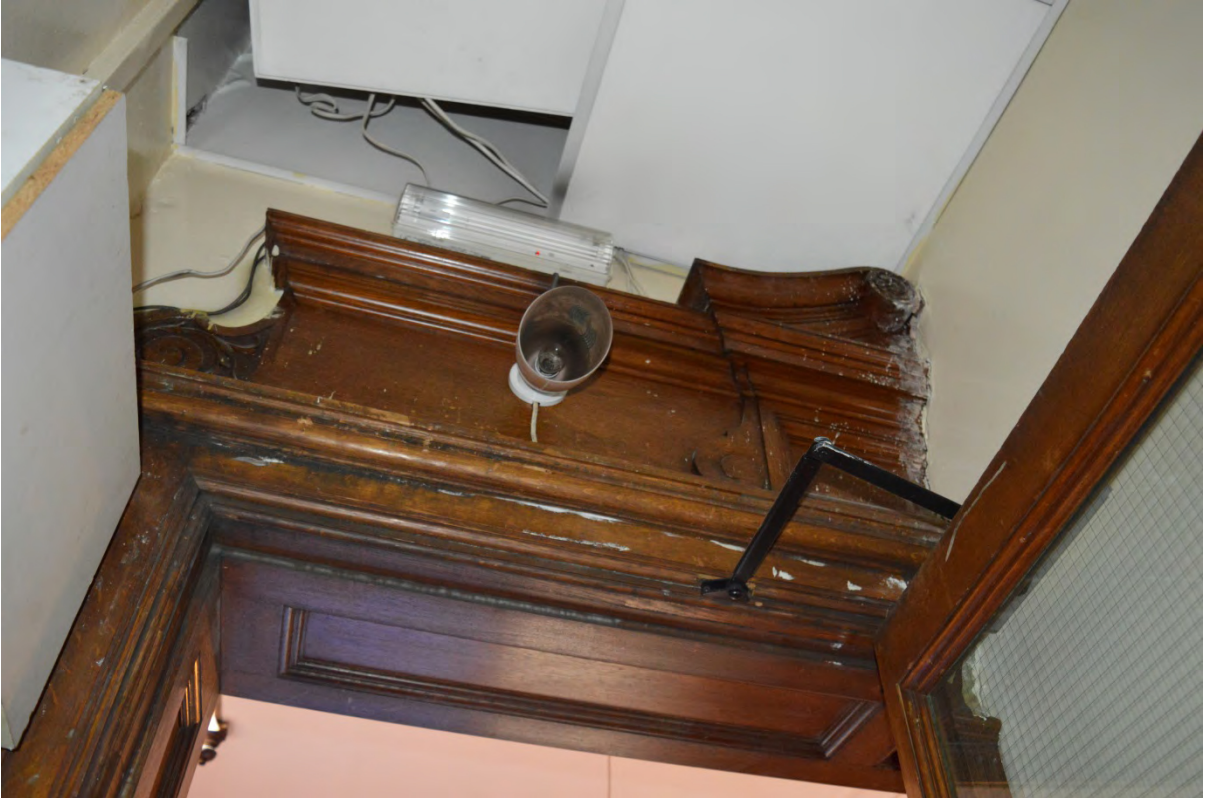
Plate 48: Wall inserted for the bathroom to room 140, 6 Palace Court (Photo 312).
