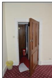
7330-0269 7330_Room 148 Doorway. Facing east
