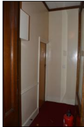
7330-0305 7330_Lobby to Room 141 and 142. Facing north
