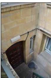
7330-0223 7330_Principal Elevation Entrance to Former Restaurant. Facing north-west
