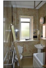
7330-0069 7330_Room 110. Facing north
