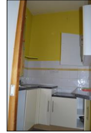
7330-0288 7330_Room 146. Facing east
