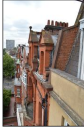
7330-0227 7330_Principal Elevation. Facing west
