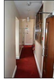
7330-0231 7330_Fourth Floor Corridor. Facing north
