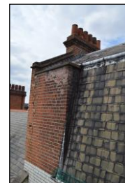
7330-0237 7330_Fourth Floor Mansard Roof above skylight. Facing north-west
