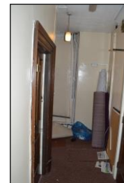
7330-0252 7330_Third Floor Corridor. Facing east
