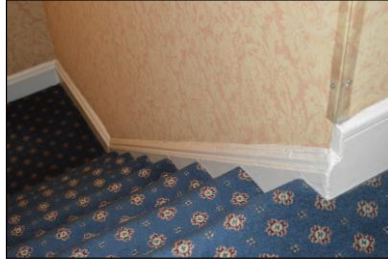
7330-0062 7330_Servant's Staircase. Facing east
