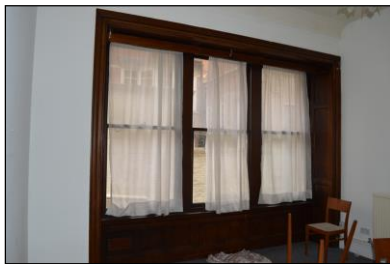
7330-0337 7330_Flat 138. Facing north
