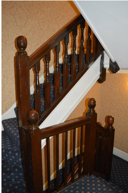
Plate 29: Original section of servant's staircase, 154 Bayswater Road (Photo 83).
