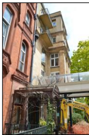
7330-0127 7330_Principal elevation. Facing north-east
