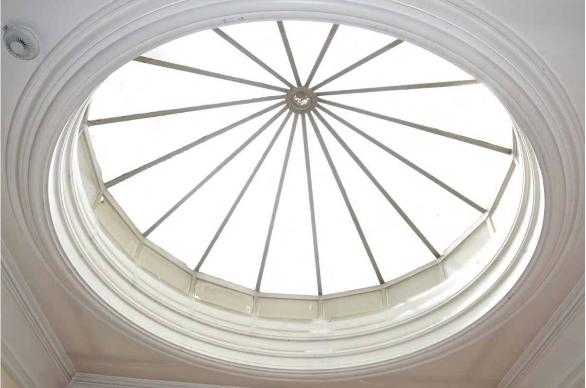
Plate 75: Skylight above main staircase, second floor landing, 6 Palace Court (Photo 279).
