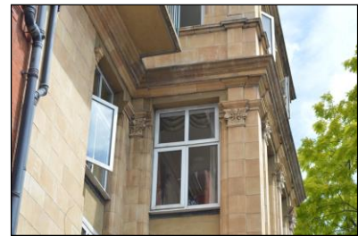
7330-0129 7330_Principal elevation. Facing east
