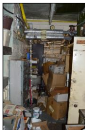
7330-0179 7330_Store in Basement. Facing north
