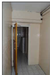
7330-0371 7330_Lower Ground Floor Corridor. Facing north
