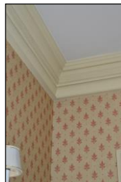
7330-0158 7330_Room 103. Facing north-west
