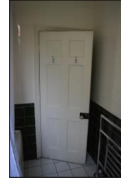
7330-0093 7330_Room 105. Facing south-west
