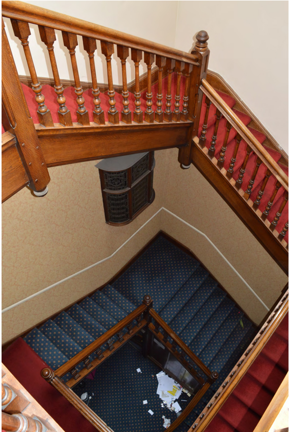
Plate 68: Main staircase, 6 Palace Court (Photo 280).
