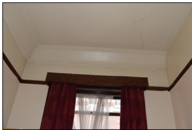
7330-0307 7330_Room 142. Facing north
