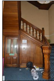
7330-0320 7330_Main Staircase Hallway. Facing west
