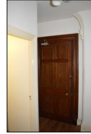
7330-0333 7330_Lobby to Flat 138. Facing south
