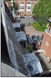
7330-0031 7330_Roof of 6 Palace Court. Facing south-west
