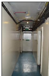
7330-0176 7330_Corridor in Basement. Facing south
