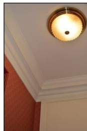
7330-0071 7330_Lobby to Room 111. Facing east
