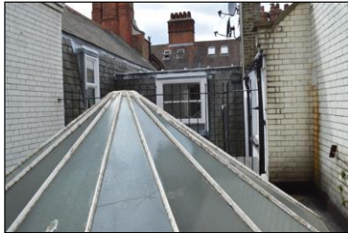
7330-0259 7330_Roof around skylight. Facing west
