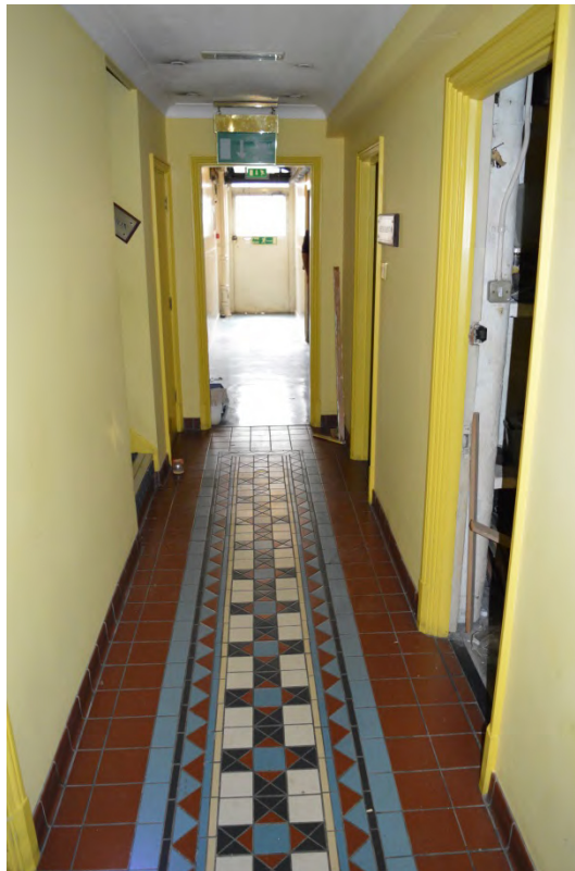
Plate 12: Tiled flooring in the basement, 154 Bayswater Road (Photo 174).
