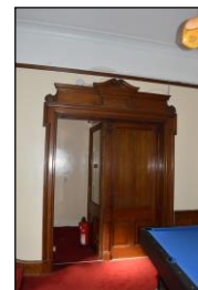
7330-0300 7330_First Floor Landing. Facing north
