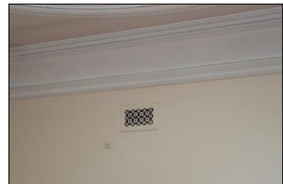
7330-0282 7330_Second Floor Landing. Facing north
