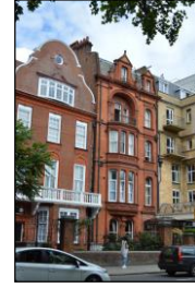
7330-0138 7330_Principal elevation. Facing north-east
