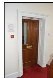
7330-0285 7330_Second Floor Landing. Facing south
