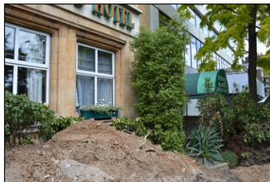
7330-0218 7330_Principal Elevation. Facing north- east
