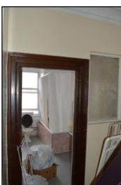
7330-0253 7330_Flat 149. Facing north
