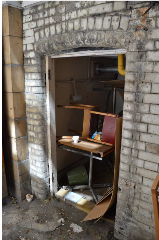
Plate 19: West vault, 154 Bayswater Road (Photo 215).
