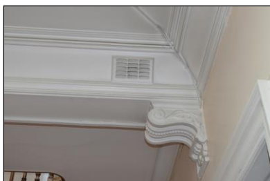
7330-0283 7330_Second Floor Landing. Facing east
