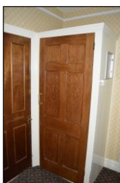
7330-0103 7330_Lobby to Room 107. Facing south-west
