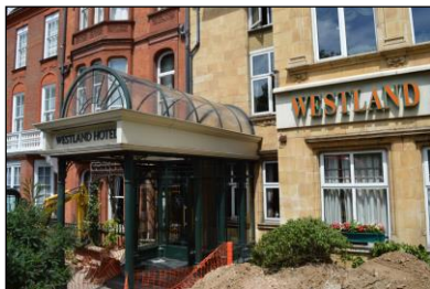
7330-0115 7330_Principal elevation. Facing north-west
