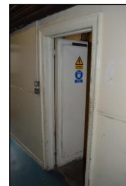
7330-0177 7330_Corridor in Basement. Facing south-west
