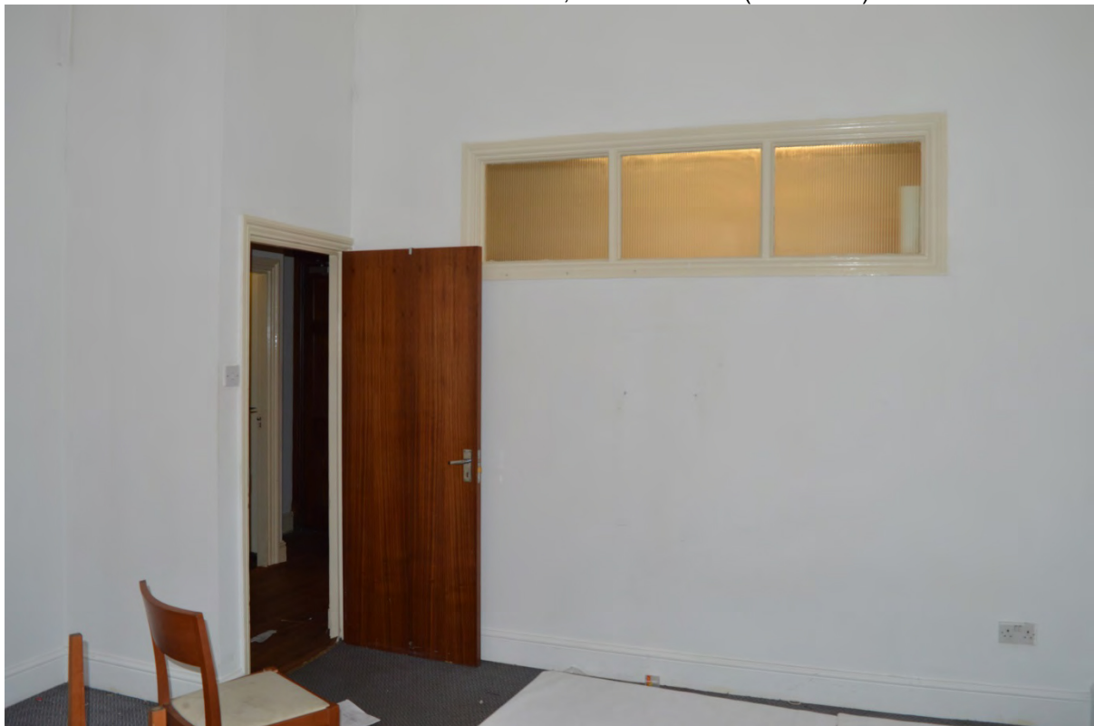
Plate 51: Wall inserted in the 1960s/70s in room 138, 6 Palace Court (Photo 339).
