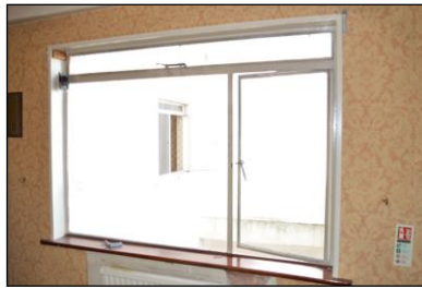
7330-0008 7330_Metal Frame Window Fifth Floor. Facing west
