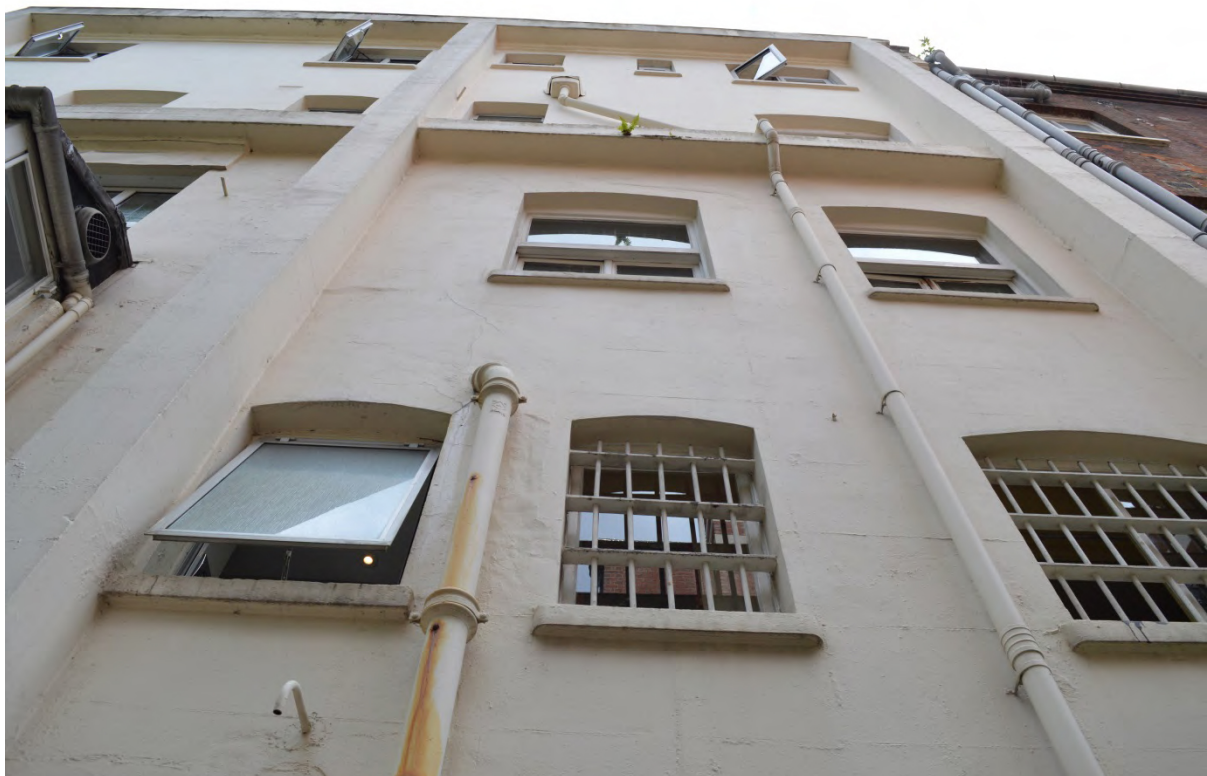
Plate 6: Rear elevation of 154 Bayswater Road (Photo 194).
