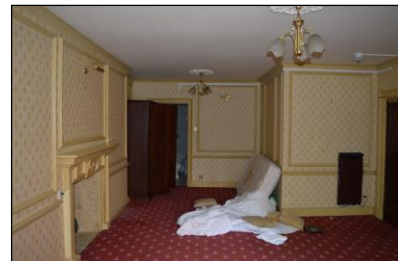
7330-0099 7330_Room 106. Facing south
