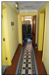
7330-0173 7330_Tiled Corridor in Basement. Facing north
