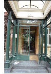
7330-0141 7330_Front Porch. Facing north
