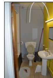
7330-0372 7330_Lower Ground Floor Bathroom. Facing east
