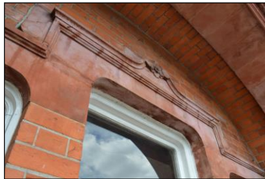
7330-0266 7330_Room 148 Balcony. Facing north
