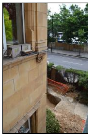
7330-0112 7330_Terracotta Mouldings. Facing south-east
