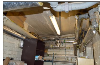
7330-0180 7330_Store in Basement. Facing north
