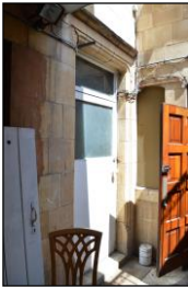
7330-0214 7330_Lower Ground Floor Front. Facing east
