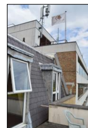
7330-0225 7330_Principal Elevation. Facing north- east
