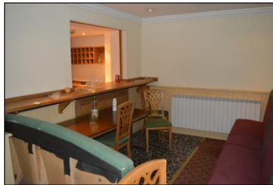
7330-0206 7330_Former Restaurant Dining Room. Facing east
