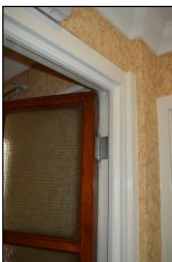
7330-0040 7330_Room 116. Facing south-west
