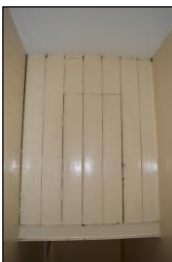
7330-0343 7330_Lower Ground Floor Staircase. Facing east
