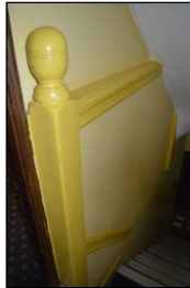
7330-0170 7330_Stairs to Basement. Facing west
