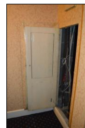
7330-0102 7330_Cupboard on First Floor Landing. Facing south-west
