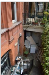
7330-0388 7330_Lower Ground Floor Front. Facing east
