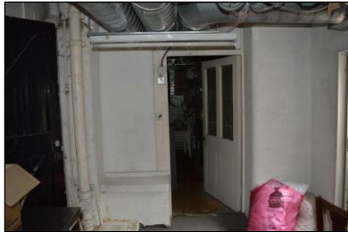
7330-0364 7330_Store. Facing south
