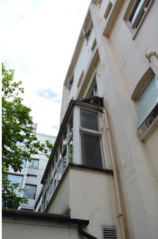
Plate 9: Remodeled bay window to rear of 154 Bayswater Road (Photo 195).
