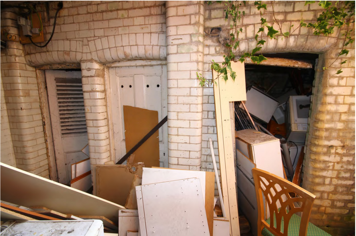
Plate 61: Glazed brick facing to vault, 6 Palace Court (Photo 385).
