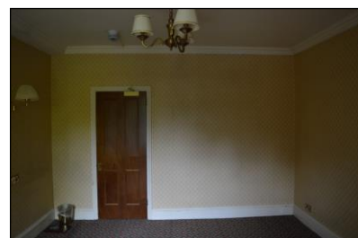
7330-0105 7330_Room 107. Facing north
