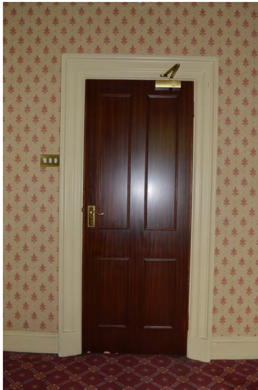
Plate 34: Room 103, 1930s architrave and skirting (Photo 157).
