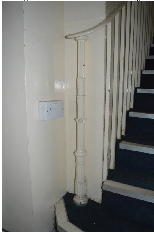
Plate 55: Newel post to staircase to basement, 6 Palace Court (Photo 346).
