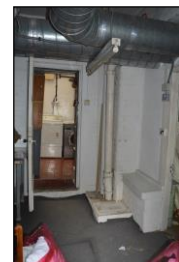
7330-0360 7330_Store. Facing east
