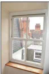
7330-0235 7330_Fourth Floor Corridor. Facing west
