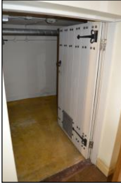
7330-0211 7330_Vault north of Former Restaurant Dining Room. Facing south
