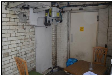
7330-0217 7330_Lower Ground Floor Front. Facing west
