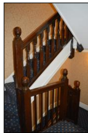
7330-0083 7330_Servant's Staircase. Facing north-east
