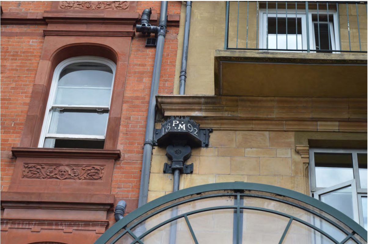
Plate 4: Initialed and dated hopper heads, 154 Bayswater Road (Photo 113).
