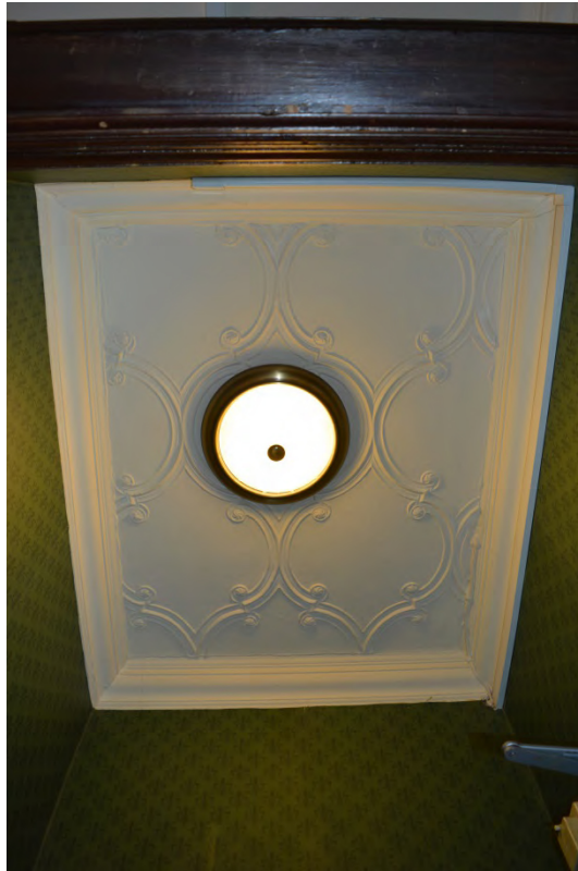
Plate 39: Room 105 intact decorative moulding on ceiling, 154 Bayswater Road (Photo 92).
