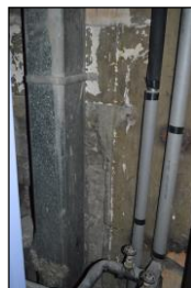
7330-0044 7330_Room 119. Facing north-east
