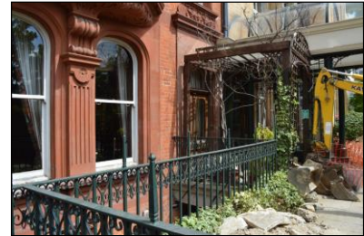
7330-0126 7330_Principal elevation. Facing north-east
