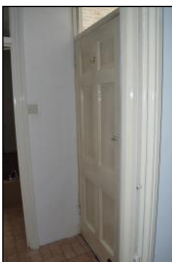
7330-0355 7330_Flat 136. Facing north
