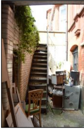
7330-0379 7330_Lower Ground Floor Front Staircase. Facing west
