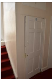
7330-0238 7330_Fourth Floor Corridor. Facing east
