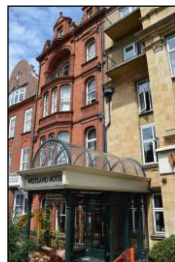
7330-0116 7330_Principal elevation. Facing north-west
