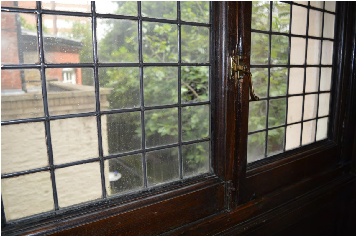
Plate 37: Room 105 leaded windows, 154 Bayswater Road (Photo 88).
