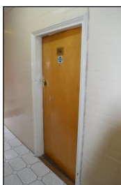
7330-0373 7330_Lower Ground Floor Corridor. Facing south
