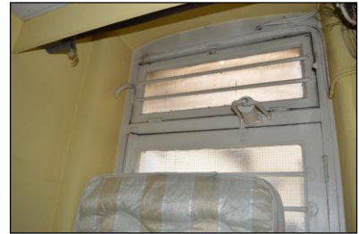
7330-0186 7330_Corridor in Basement. Facing north
