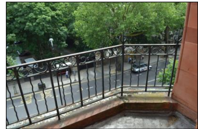
7330-0267 7330_Room 148 Balcony. Facing south-west
