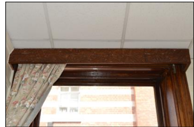
7330-0402 7330_Room 141. Facing north
