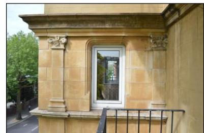
7330-0045 7330_Room 119 Balcony. Facing west
