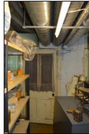
7330-0365 7330_Store. Facing north
