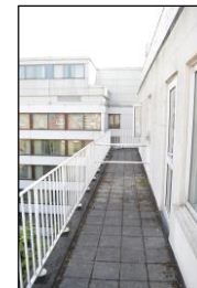
7330-0024 7330_Fourth Floor Balcony. Facing east
