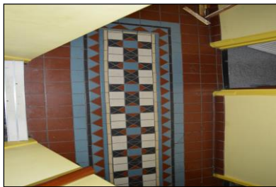
7330-0172 7330_Tiled Corridor in Basement. Facing west
