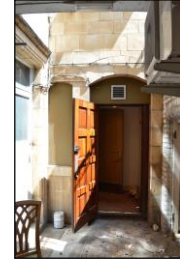
7330-0213 7330_Lower Ground Floor Front. Facing east
