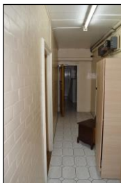
7330-0370 7330_Lower Ground Floor Corridor. Facing north
