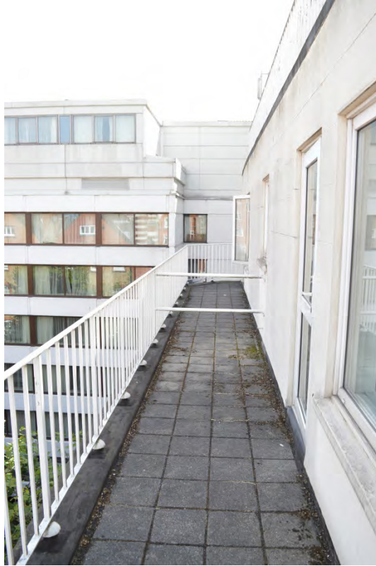
Plate 7: Fourth floor balcony, 154 Bayswater Road (Photo 24).
