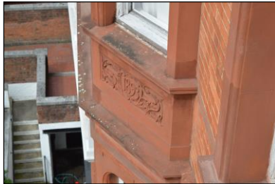
7330-0052 7330_Facade of 6 Palace Court. Facing west
