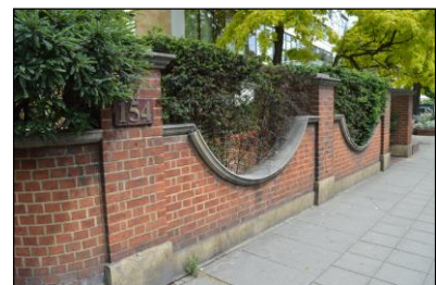
7330-0132 7330_Front Wall. Facing north-east
