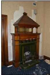
7330-0319 7330_Main Staircase Hallway. Facing north-east
