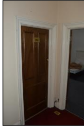
7330-0230 7330_Fourth Floor Corridor. Facing south-west
