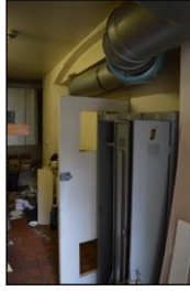
7330-0197 7330_Store. Facing east
