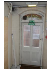
7330-0369 7330_Lower Ground Floor Corridor. Facing south
