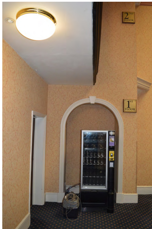
Plate 26: Blind arch on the first floor, 154 Bayswater Road (Photo 86).
