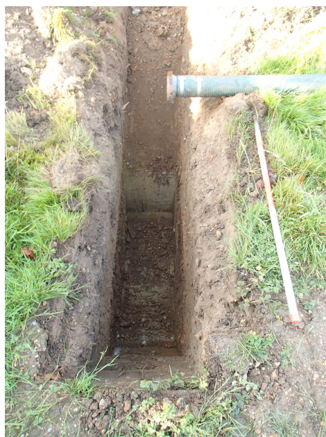
Trial pit 5 looking south-west
