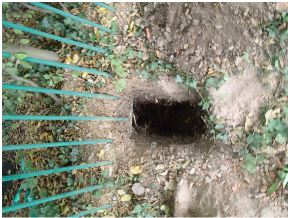
Trial pit 3 looking south
