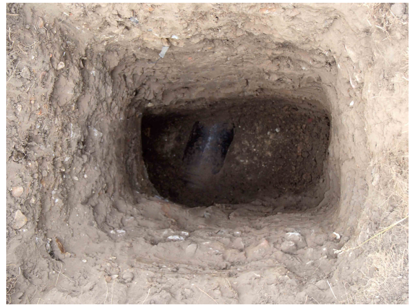
Trial pit 4 looking south
