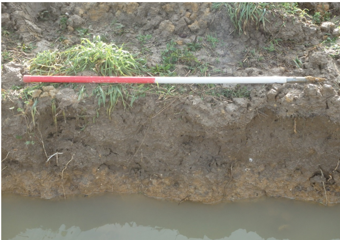
Figure 3: Typical cable trench section showing topsoil overlying subsoil and illustrating ground conditions.
