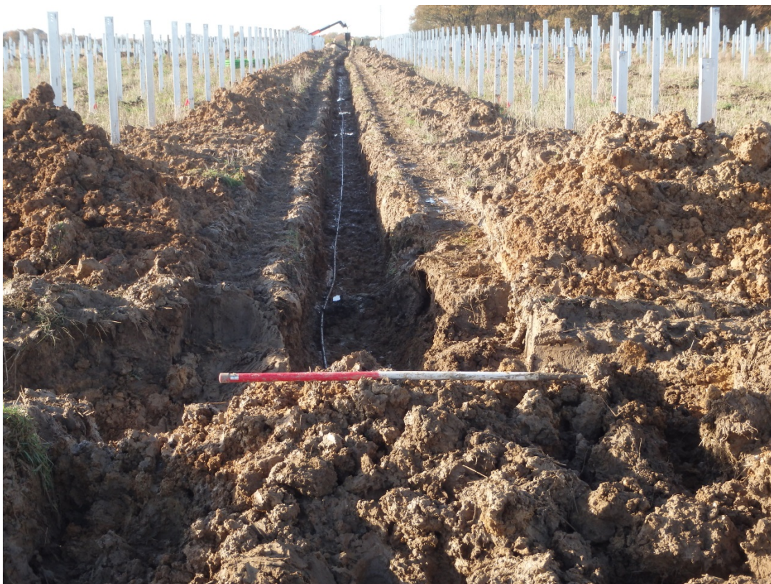
Figure 6: General view of pipe trench under excavation – November 2014.
