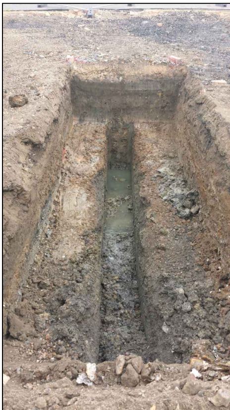
Trench 1 under excavation
