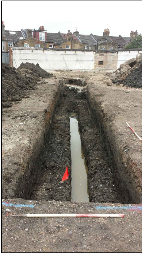
Trench 2 looking north-west
