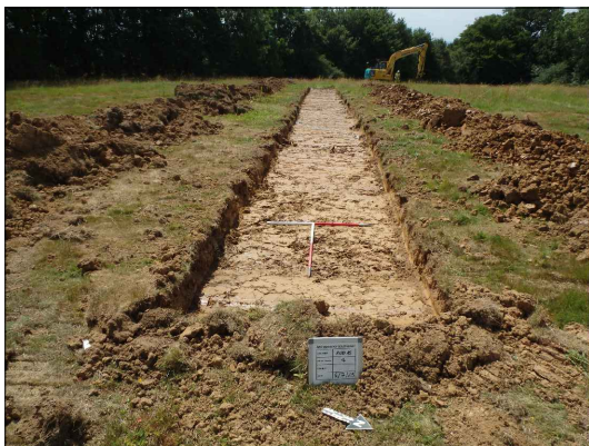
Trench 7 looking south-west
