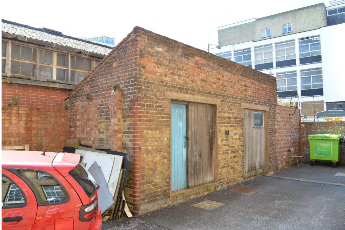
Plate 7: Girl's WC and Store within the former girl's playground, facing south-east (6176_008)
