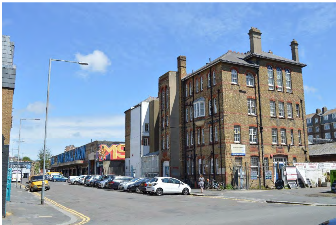
Plate 1: External view of the west elevation, looking north-east (6176_061)
