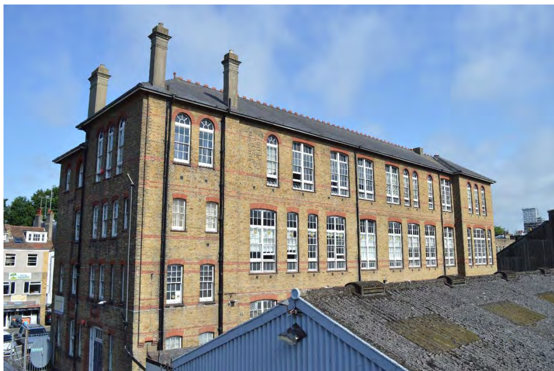
Plate 2: External view of the east elevation, looking north-west (6176_002)
