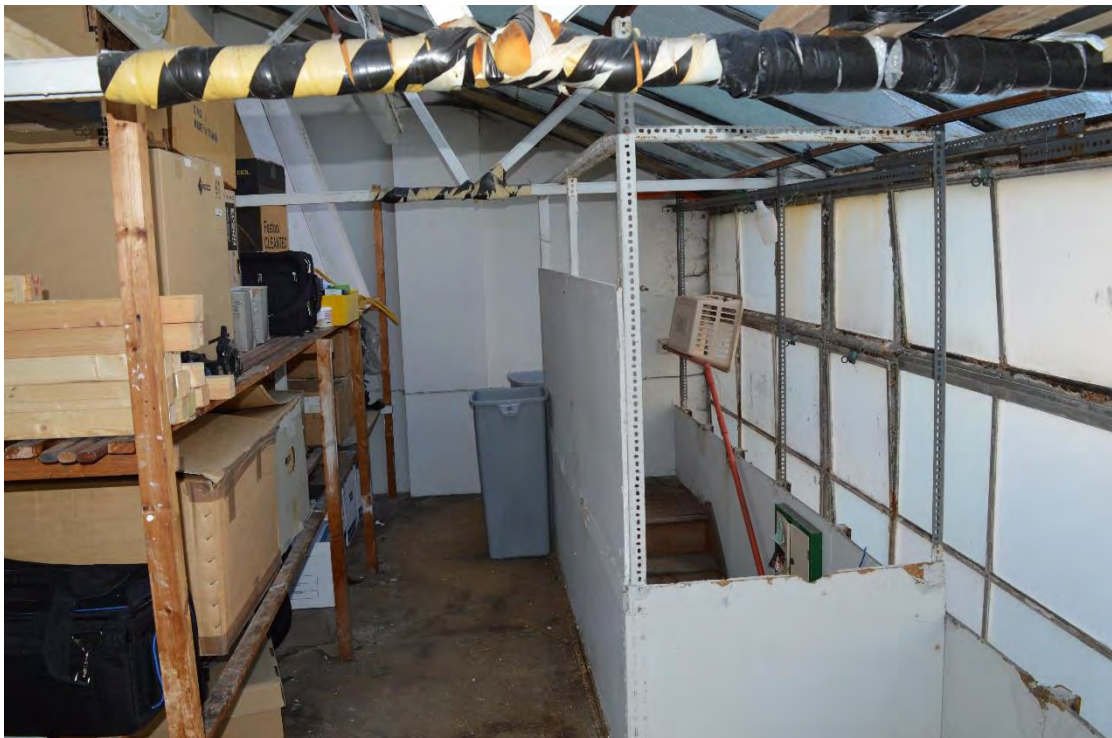
Plate 10: Ground floor, general view of the western lean-to structure, facing south (6176_033)
