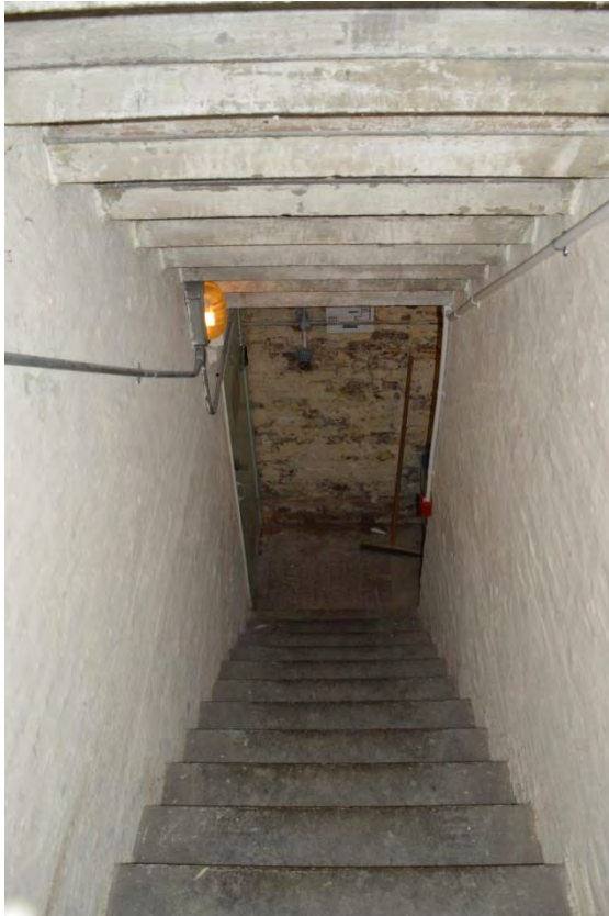
Plate 13: Basement, view of access corridor, facing south (6176_032)
