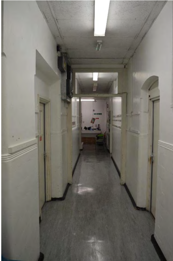
Plate 9: Ground floor, general view of corridor, facing south (6176_022)
