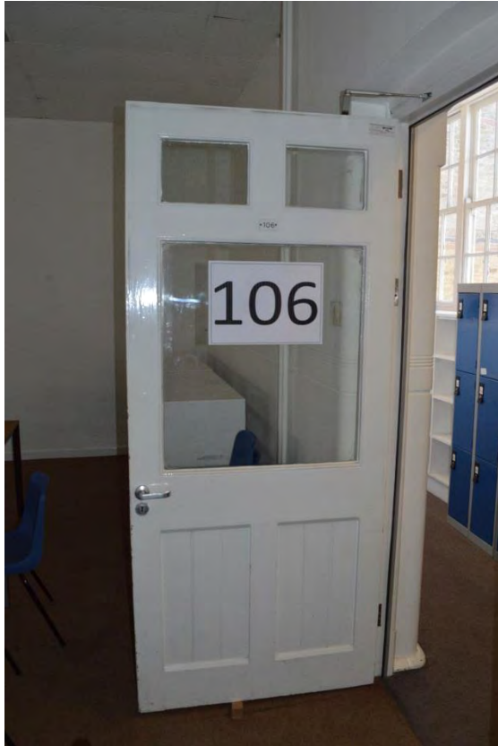
Plate 15: First floor, detail of an early timber door, facing south (6176_064)
