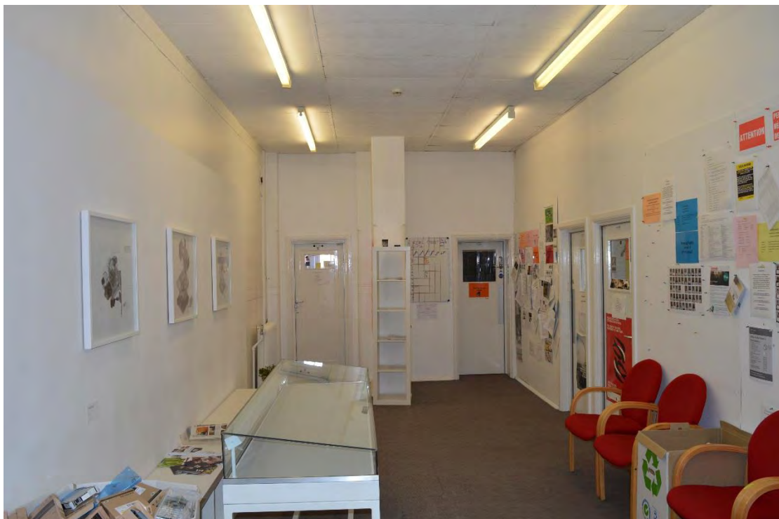
Plate 16: First floor, general view of access corridor and extended lobby within the northern range, facing north (6176_036)
