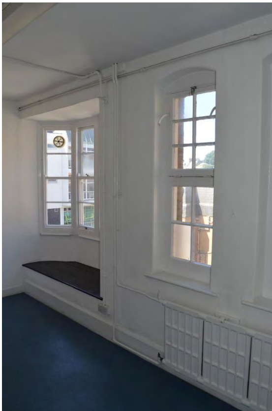
Plate 20: Mezzanine level, view of entrance lobby, facing south-west (6176_047)
