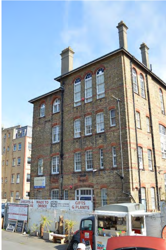
Plate 3: External view of the south elevation, looking north-west (6176_001)
