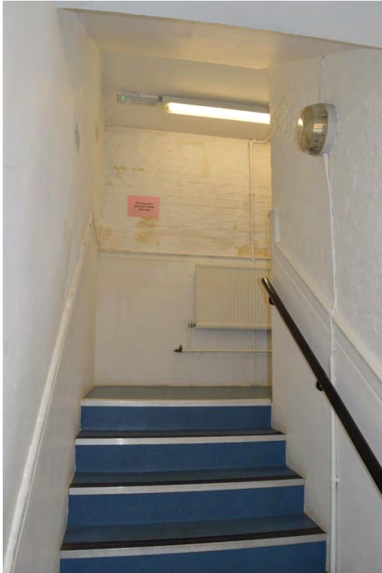
Plate 11: Ground floor, general view of the western service tower, facing south (6176_034)
