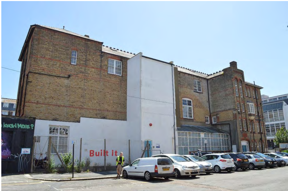
Plate 5: External view of the west elevation, facing south-east (6176_053)
