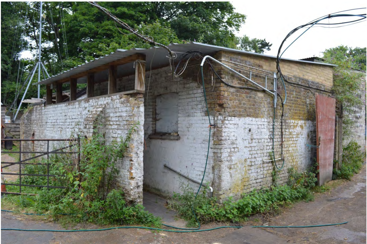
Plate 10: The western storage/tack building (Photo #39).
