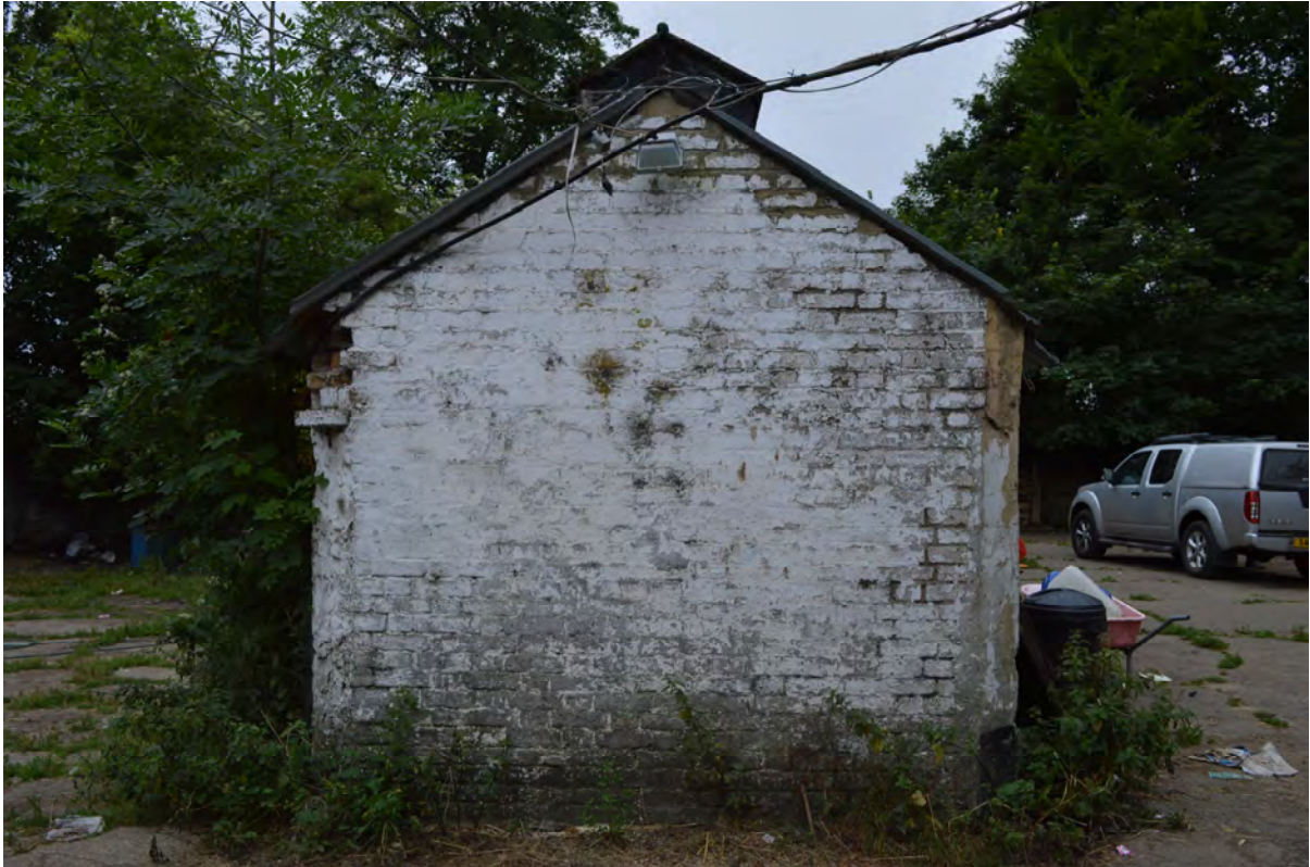
Plate 27: North elevation of the central building (Photo #20).
