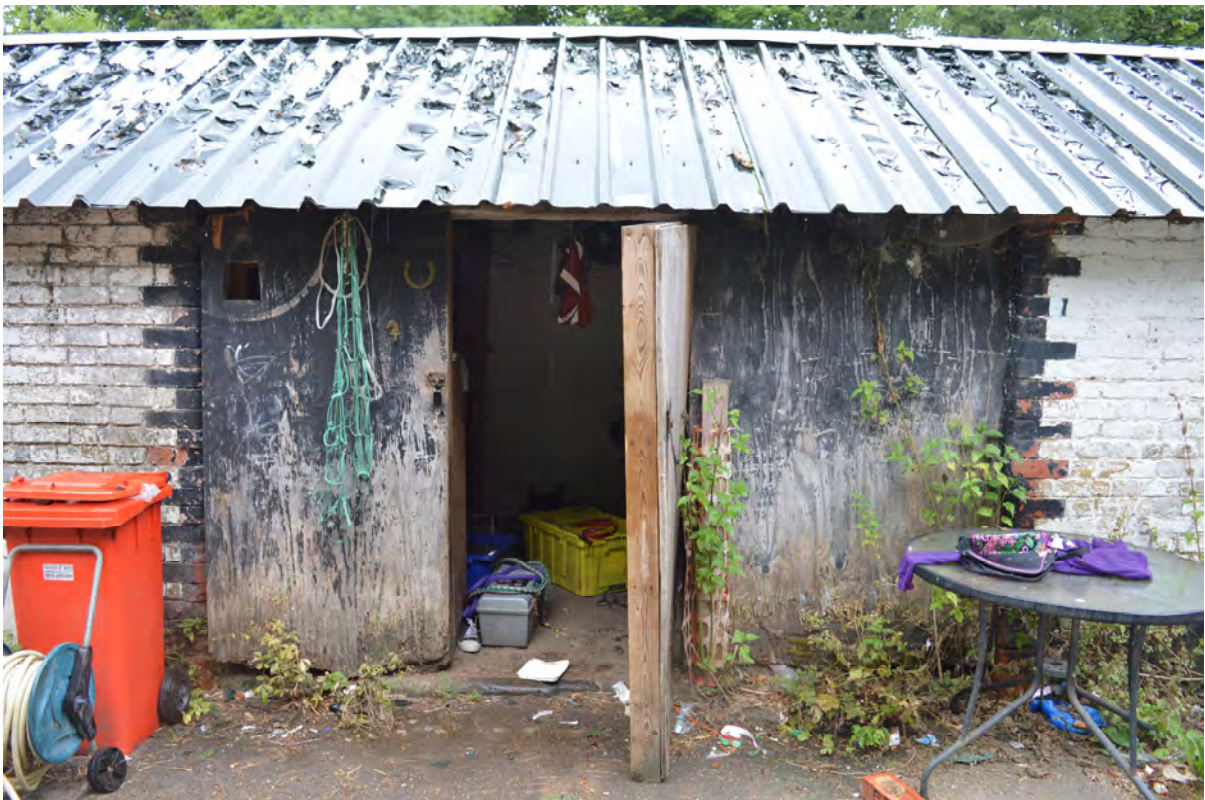
Plate 24: Doorway to the north side of the central building (Photo #72).
