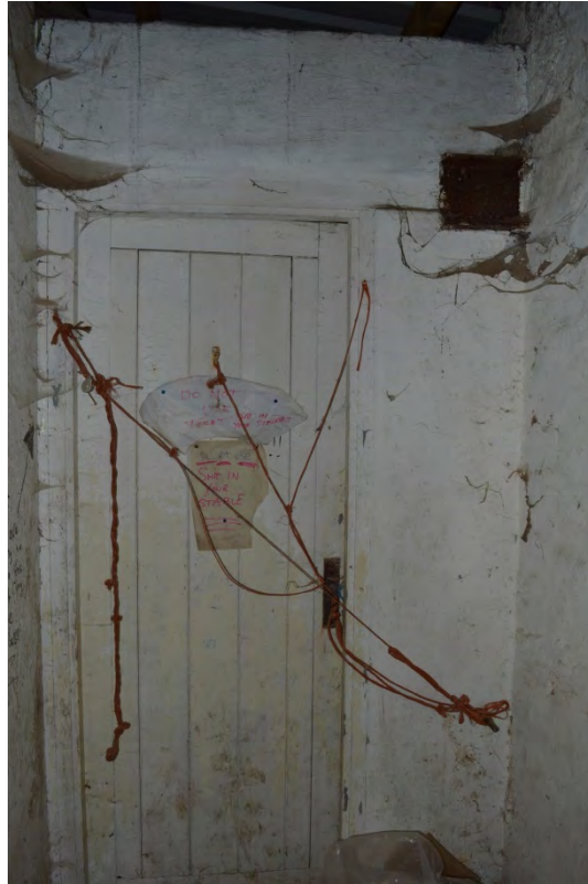
Plate 13: Toilet in the western storage/tack building (Photo #42).
