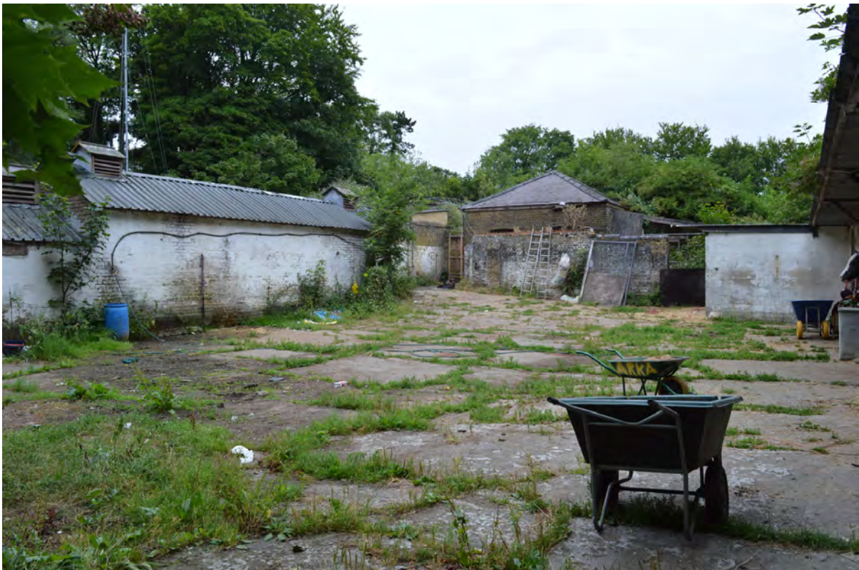
Plate 34: Eastern yard (Photo #5).
