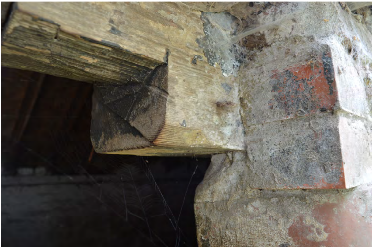
Plate 32: Detail of stop chamfer (Photo #16).
