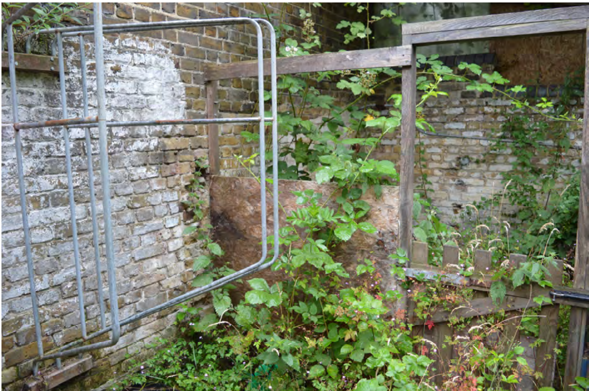
Plate 42: Remains of timber structure (Photo #36).
