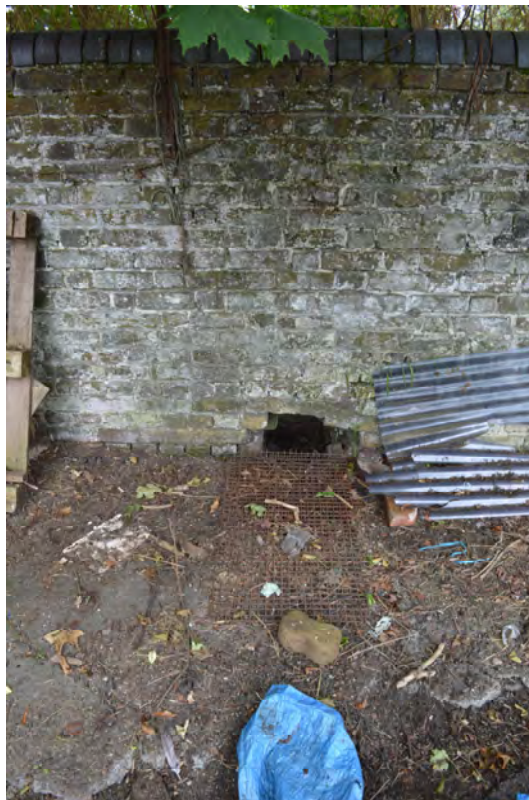
Plate 36: Drain in the south of the eastern yard (Photo #18).
