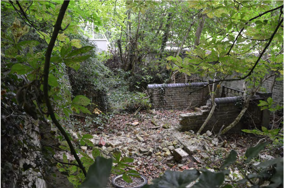
Plate 15: Pigsties in the west of the piggery (Photo #109).
