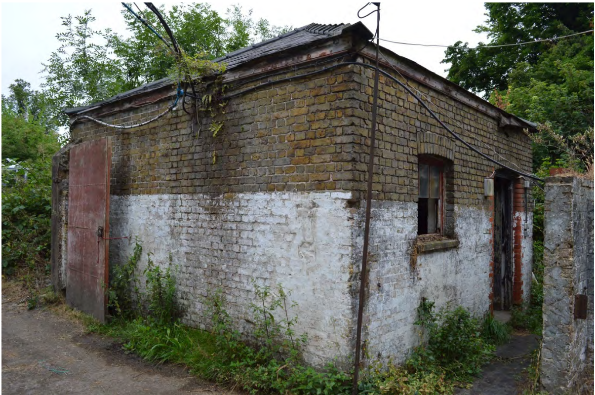
Plate 6: Eastern storage/tack building (Photo #25).
