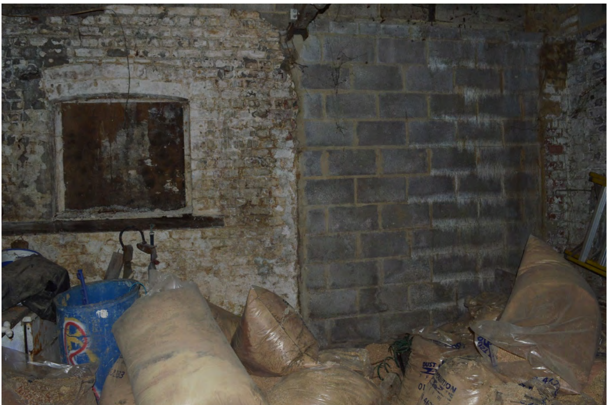
Plate 12: Interior of the western storage/tack building – note blocked openings (Photo #44).
