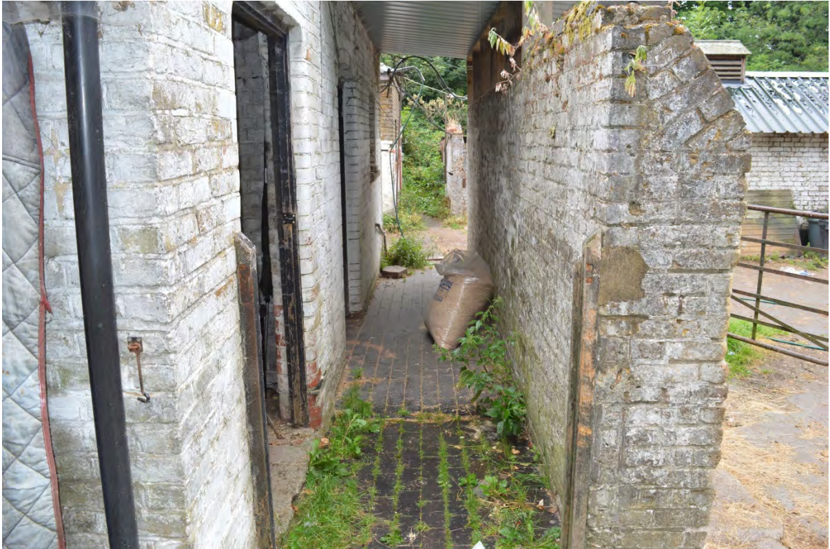
Plate 5: Feeding passage across the front of the storage/tack buildings (Photo #51).
