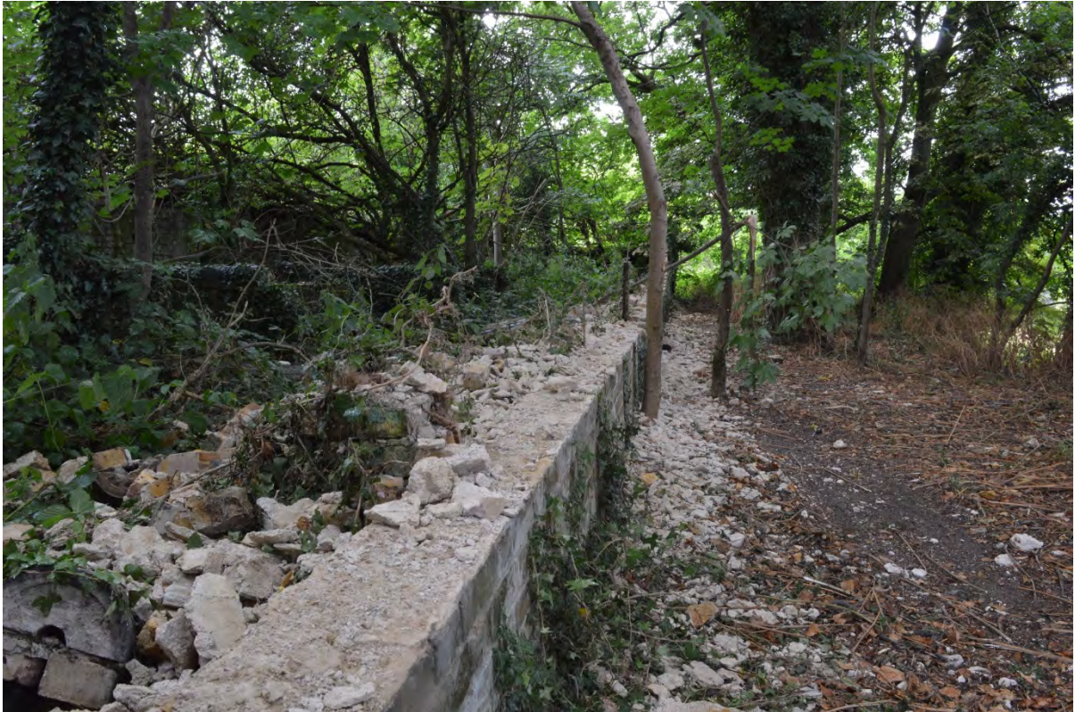
Plate 3: East wall of the piggery (Photo #113).
