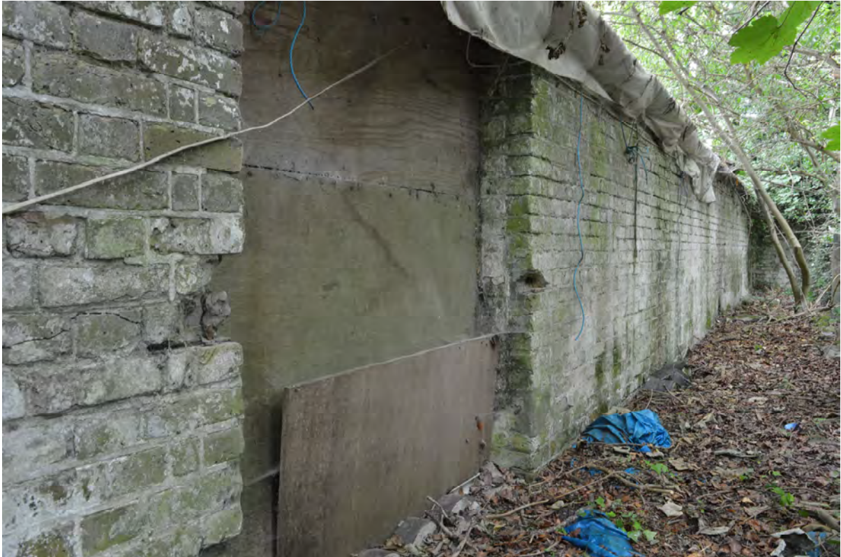
Plate 21: Blocked doorway from feeding passage to yard (Photo #93).
