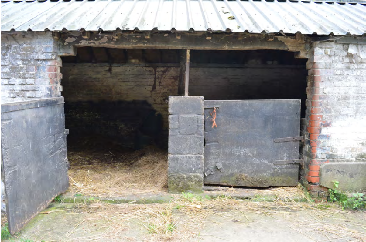
Plate 25: Doorway to south side of the central building (Photo #8).
