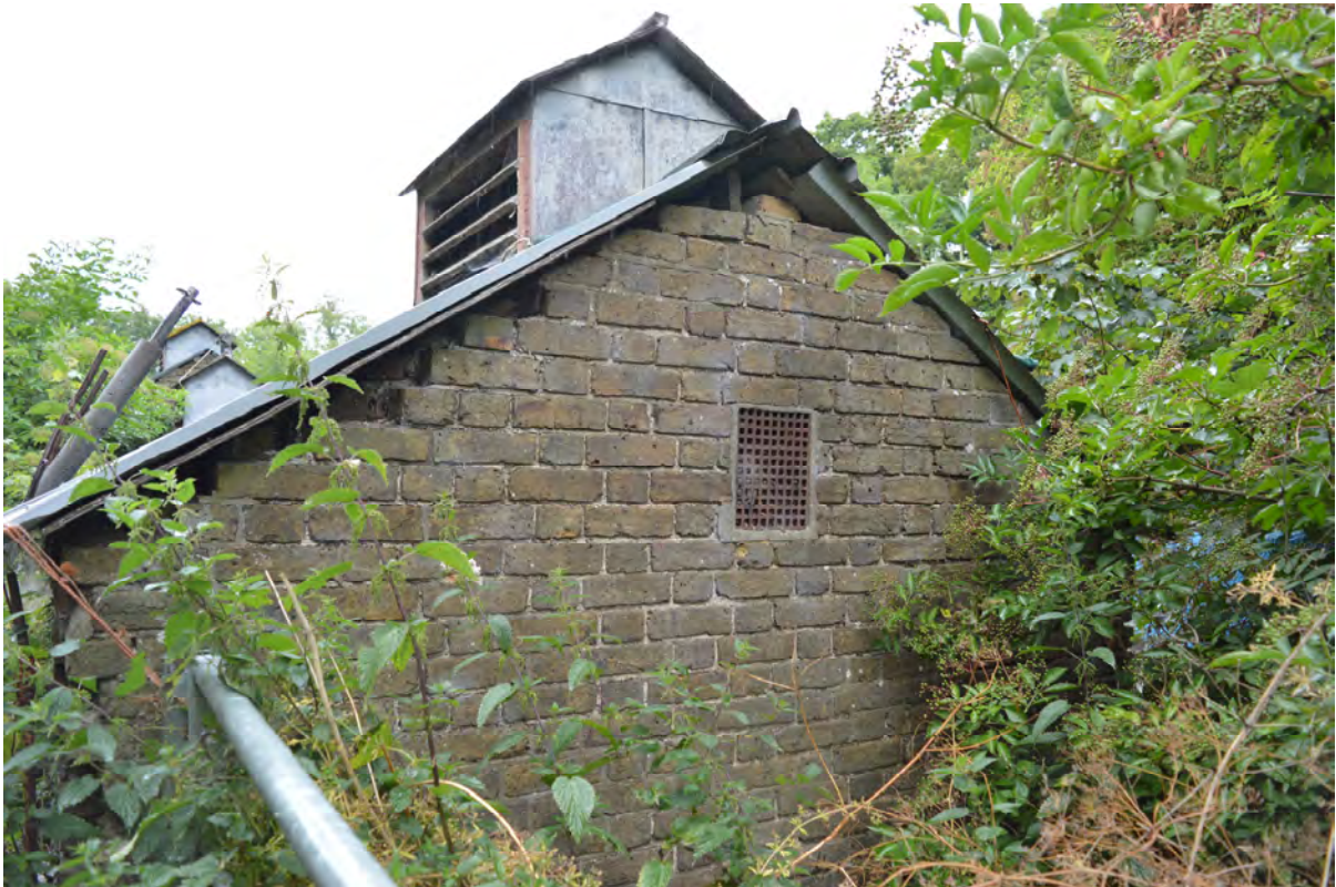
Plate 23: South elevation of the central building (Photo #70).
