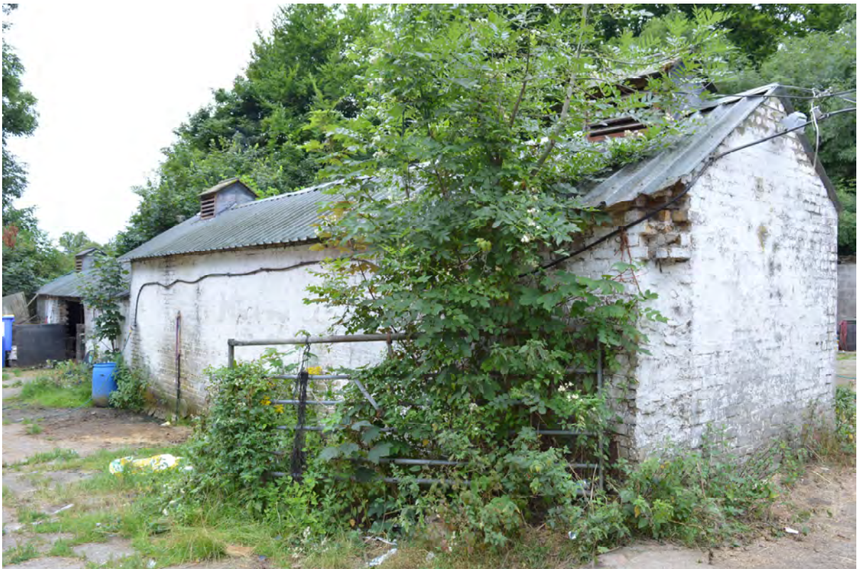
Plate 22: Central building, east side (Photo #2).
