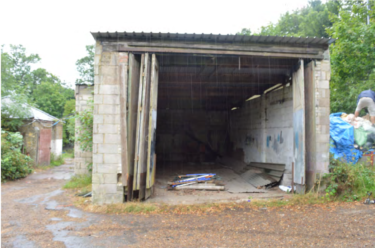
Plate 43: Breezeblock structure to north of the piggery (Photo #128).
