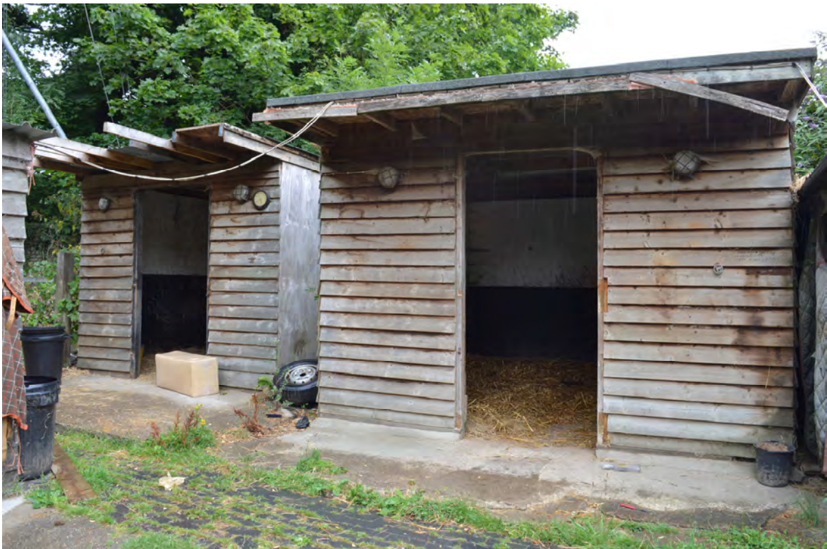
Plate 40: Timber stables in the northwest of the site (Photo #57).
