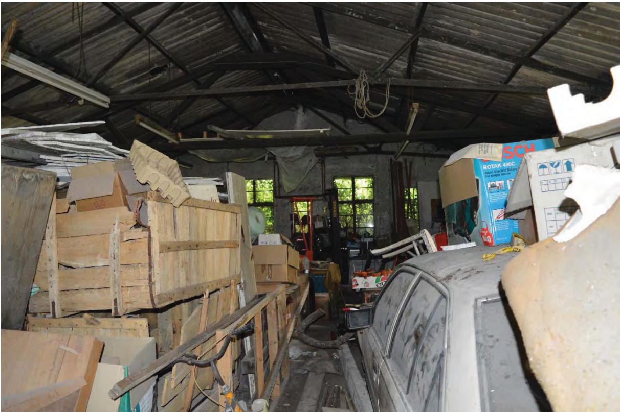
Plate 32 Building 3, Room 3, looking south-east (84)
