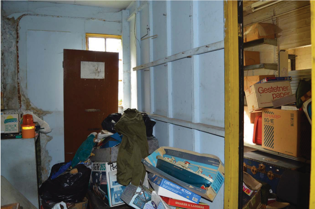
Plate 31 Building 3, Room 2, showing lightweight timber stud partition dividing the room (83).
