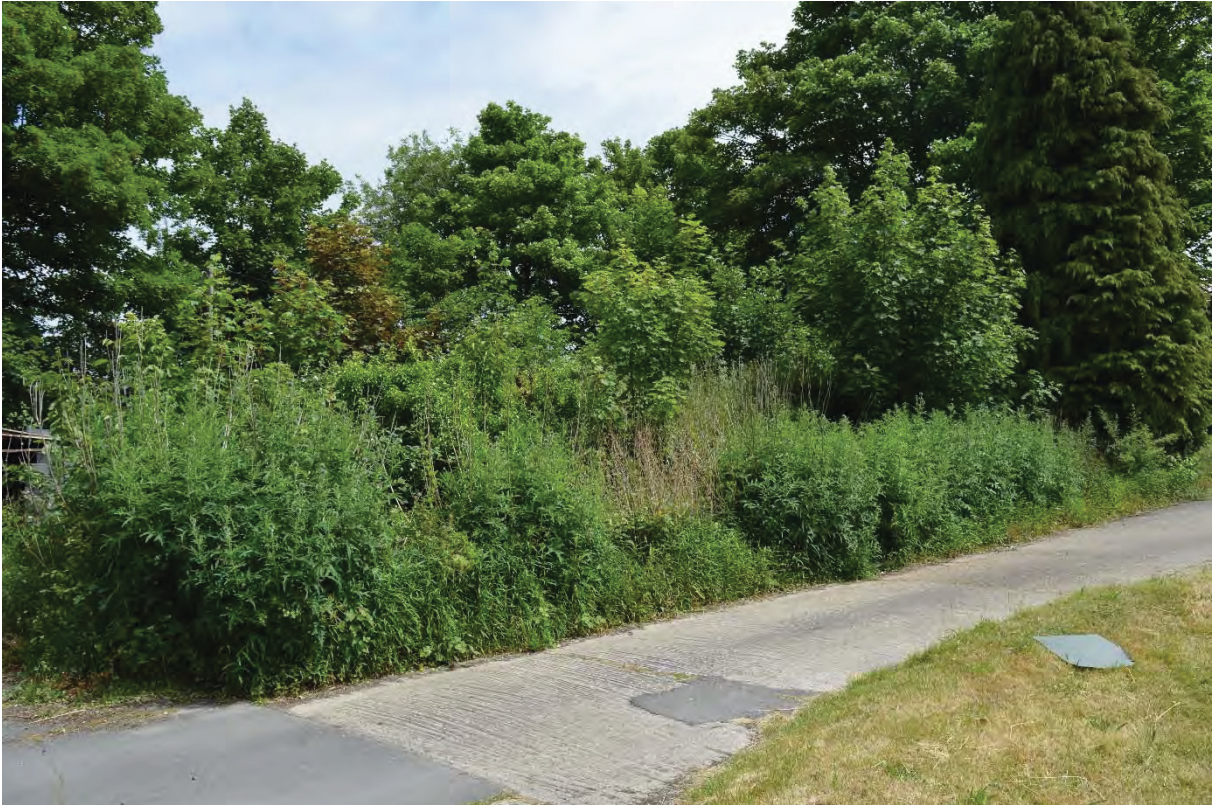
Plate 53 Air-raid shelter 2, looking east (119)
