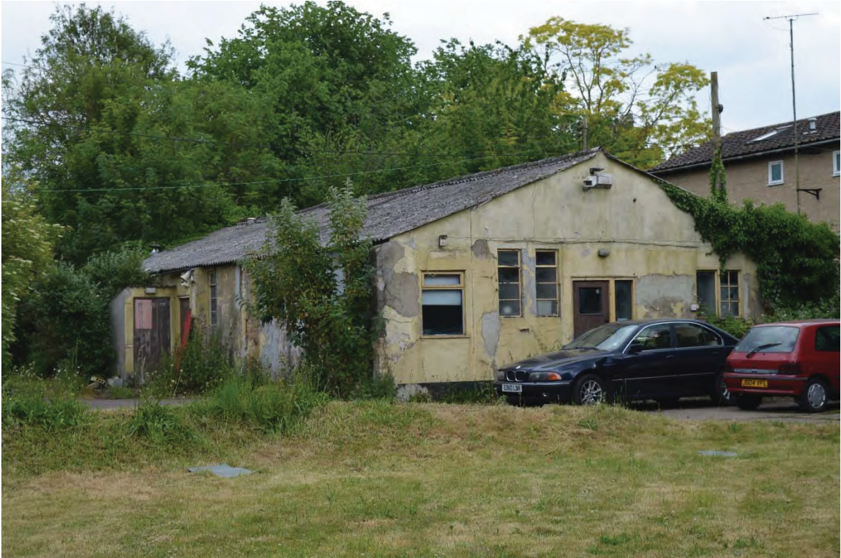
Plate 27 Building 3, looking south (78)
