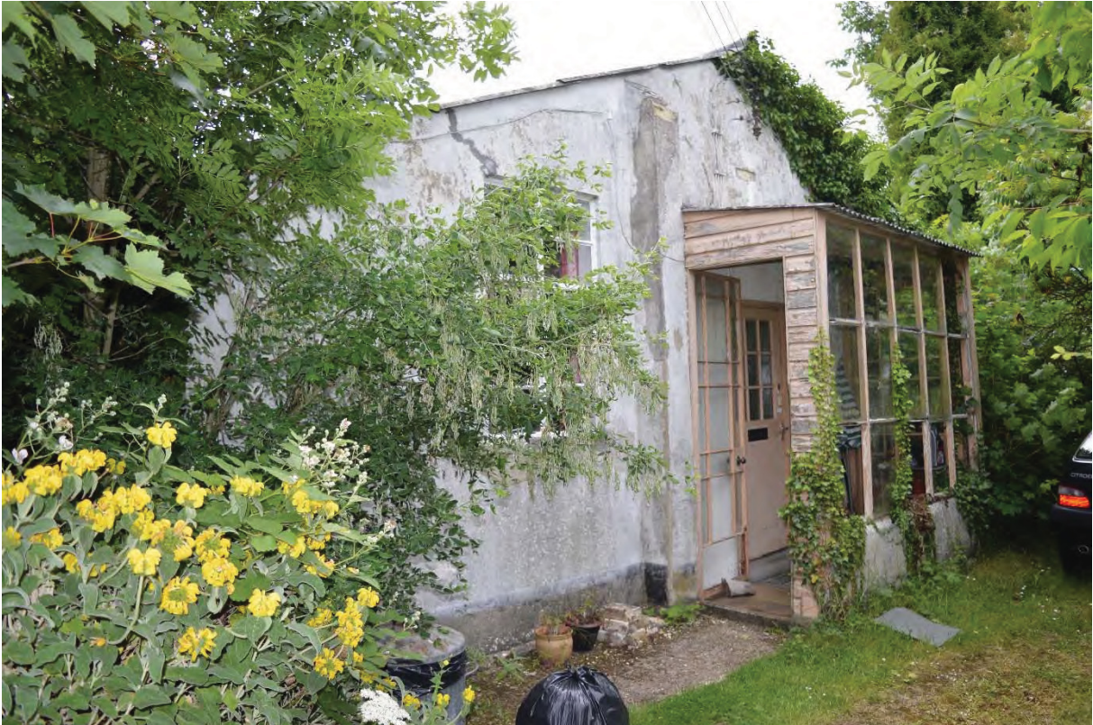
Plate 37 Principal elevation of south-east range Building 4, showing later porch (94)
