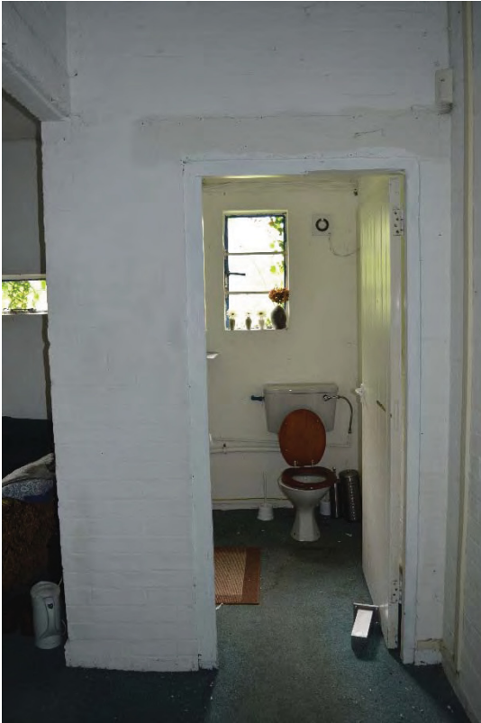
Plate 21 WC in north-west range, Building 2 (66)
