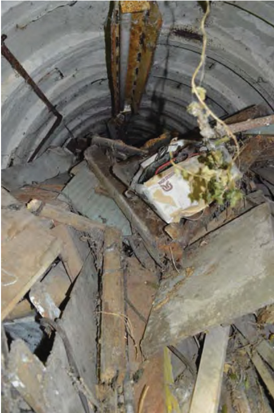
Plate 55 Interior of air-raid shelter 2 (118)
