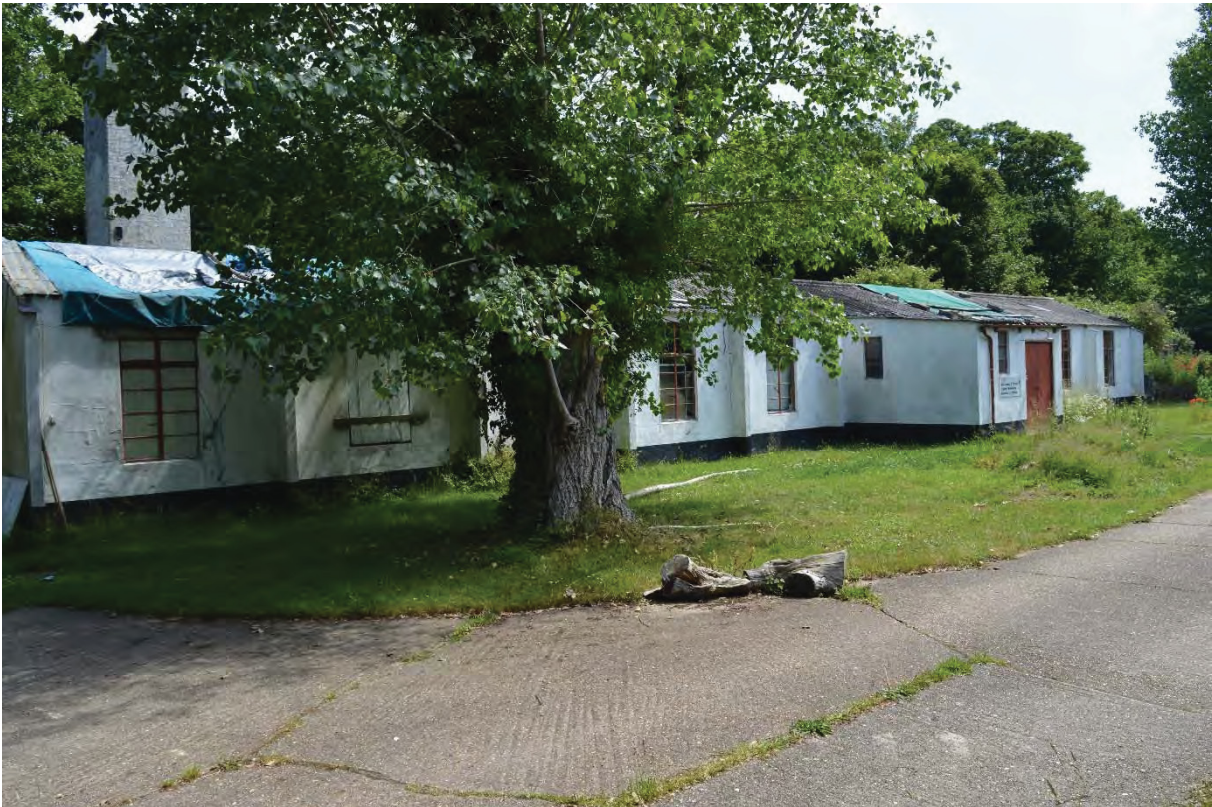
Plate 2 Building 1, principal elevation, showing projecting entrance (1)
