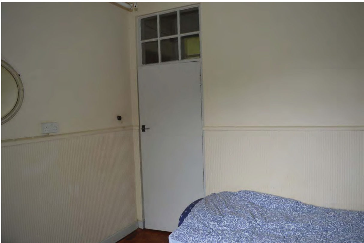
Plate 42 Doorway with glazed overhead, Building 4 (112)
