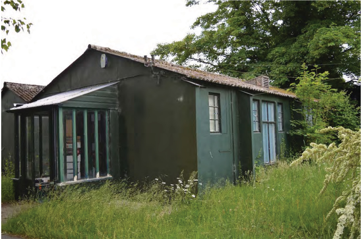
Plate 15 Building 2, looking south-east (56)
