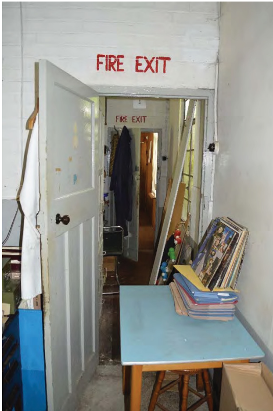
Plate 5 Typical doorway, Building 1 (28)
