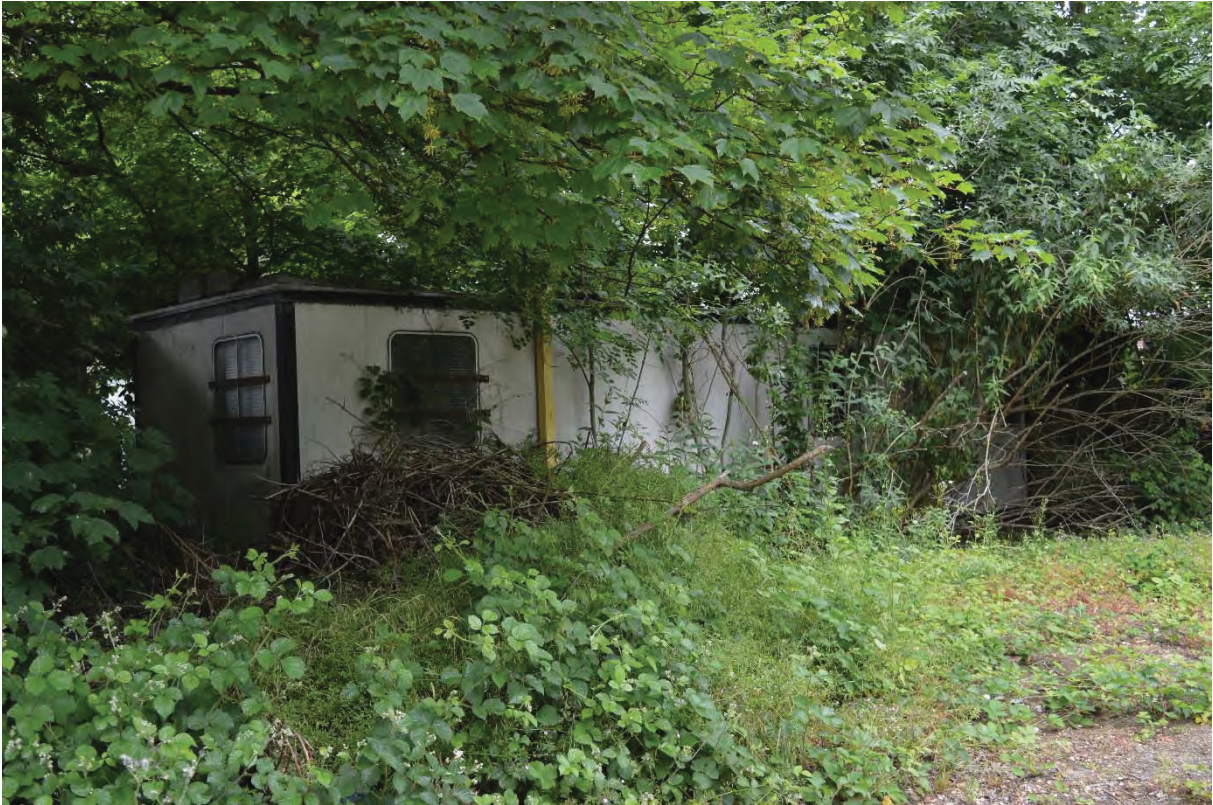
Plate 51 Portacabin east of Building 5 (48)
