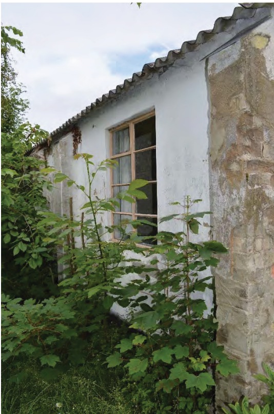
Plate 36 Typical window to Building 4 (93)
