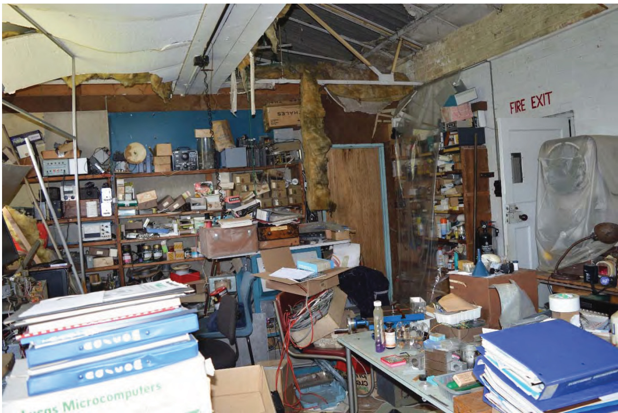
Plate 6 Building 1, with metal roof truss visible (21)
