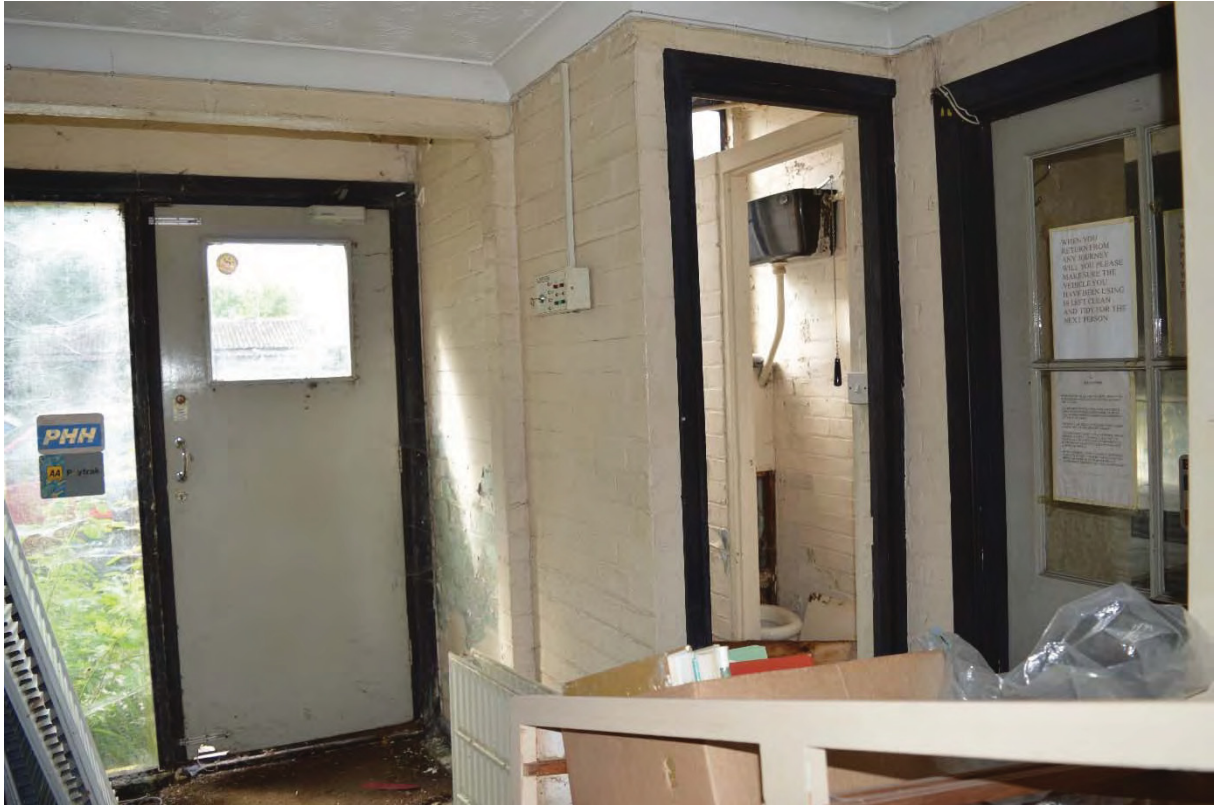
Plate 29 Lobby to Building 3, looking north-west (82)
