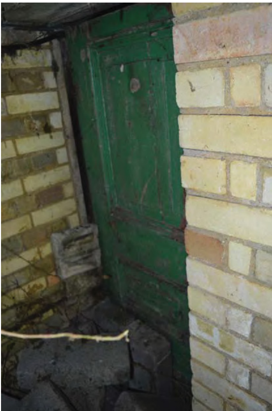
Plate 56 The surviving entrance door to air-raid shelter 1 (77)
