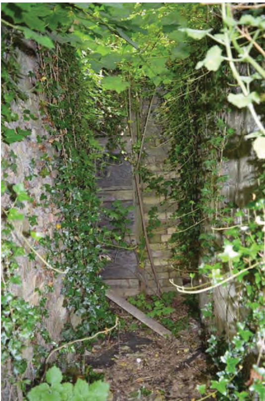
Plate 54 Entrance passage to air-raid shelter 2 (117)
