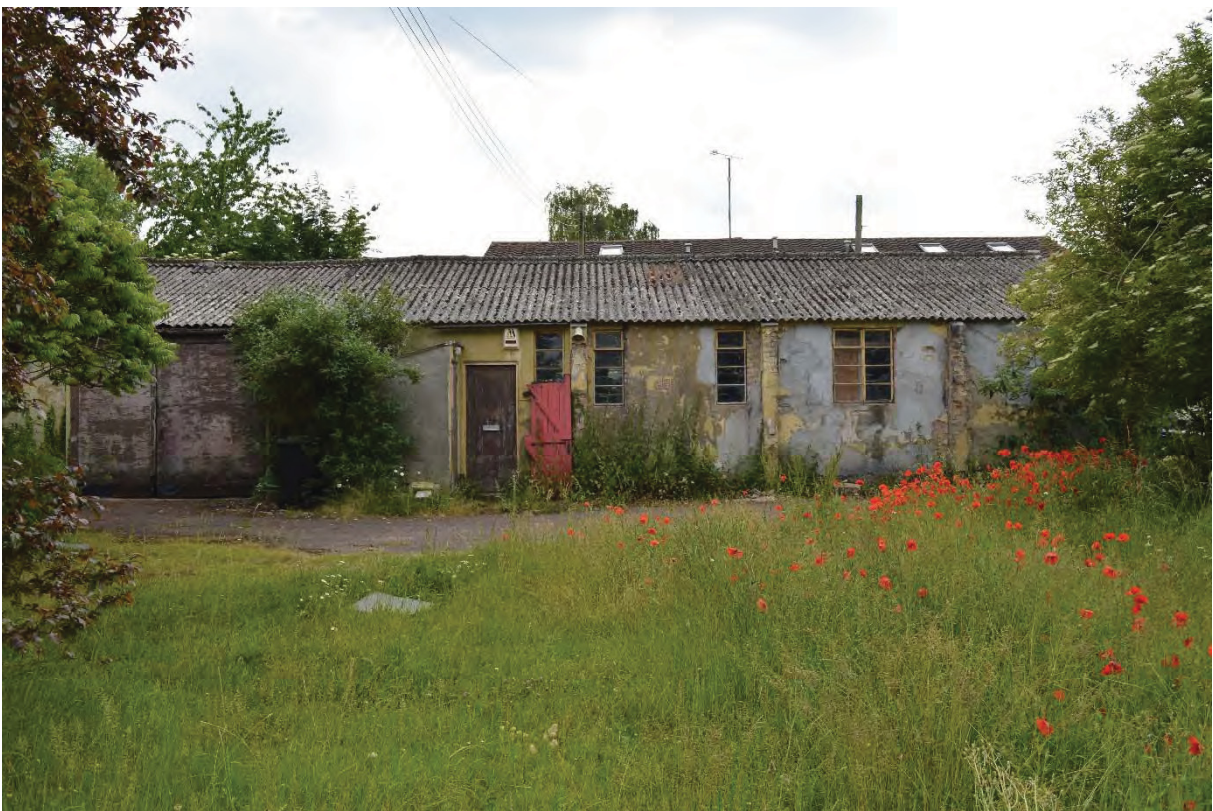
Plate 28 Building 3, north-east elevation (79)
