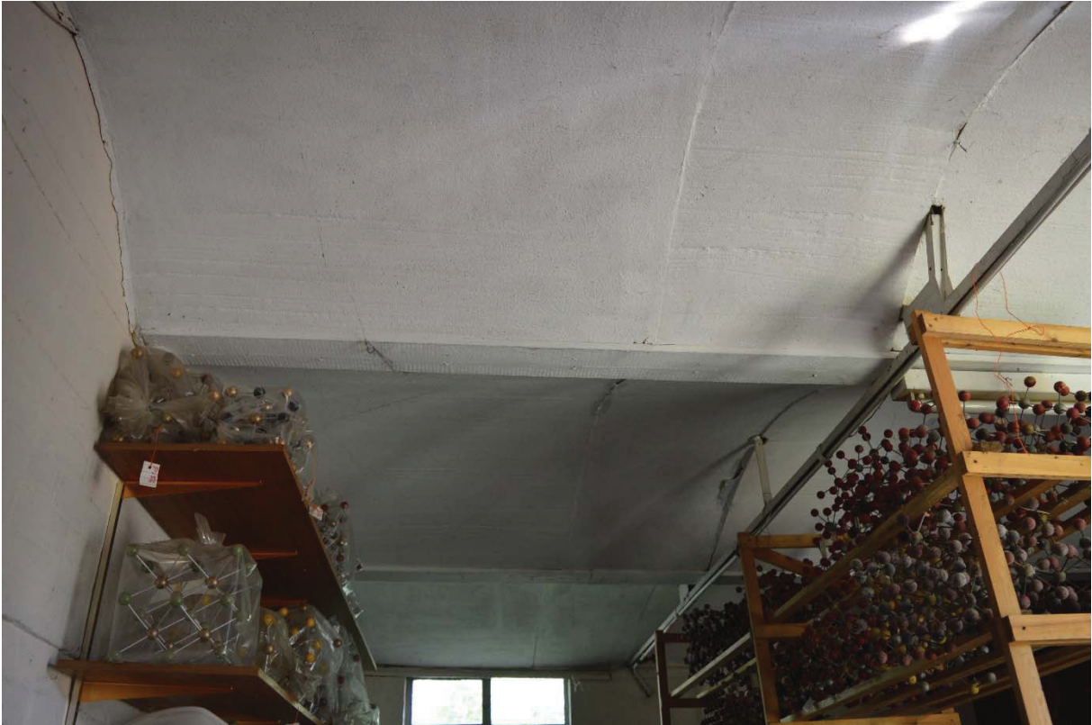
Plate 7 Example of vaulted polystyrene ceiling cladding in Building 1 (18)
