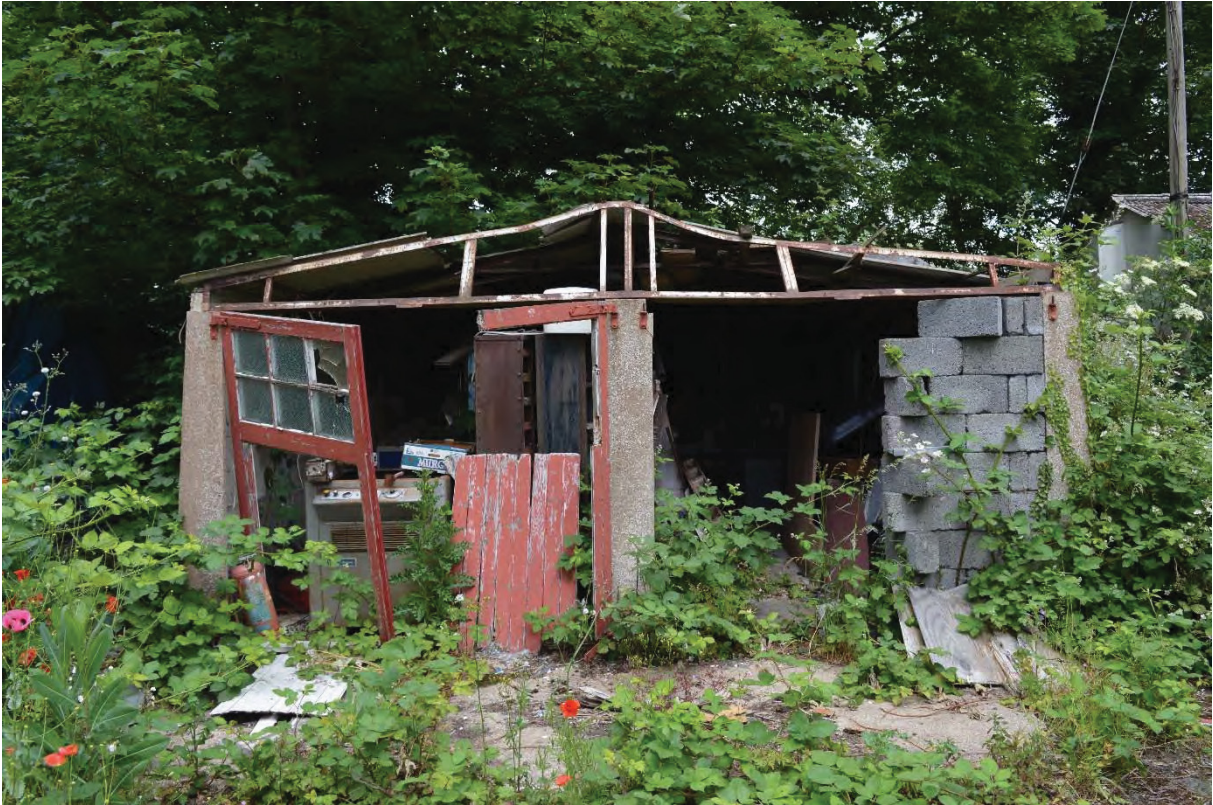
Plate 57 Garage north-west of Building 6 (46)
