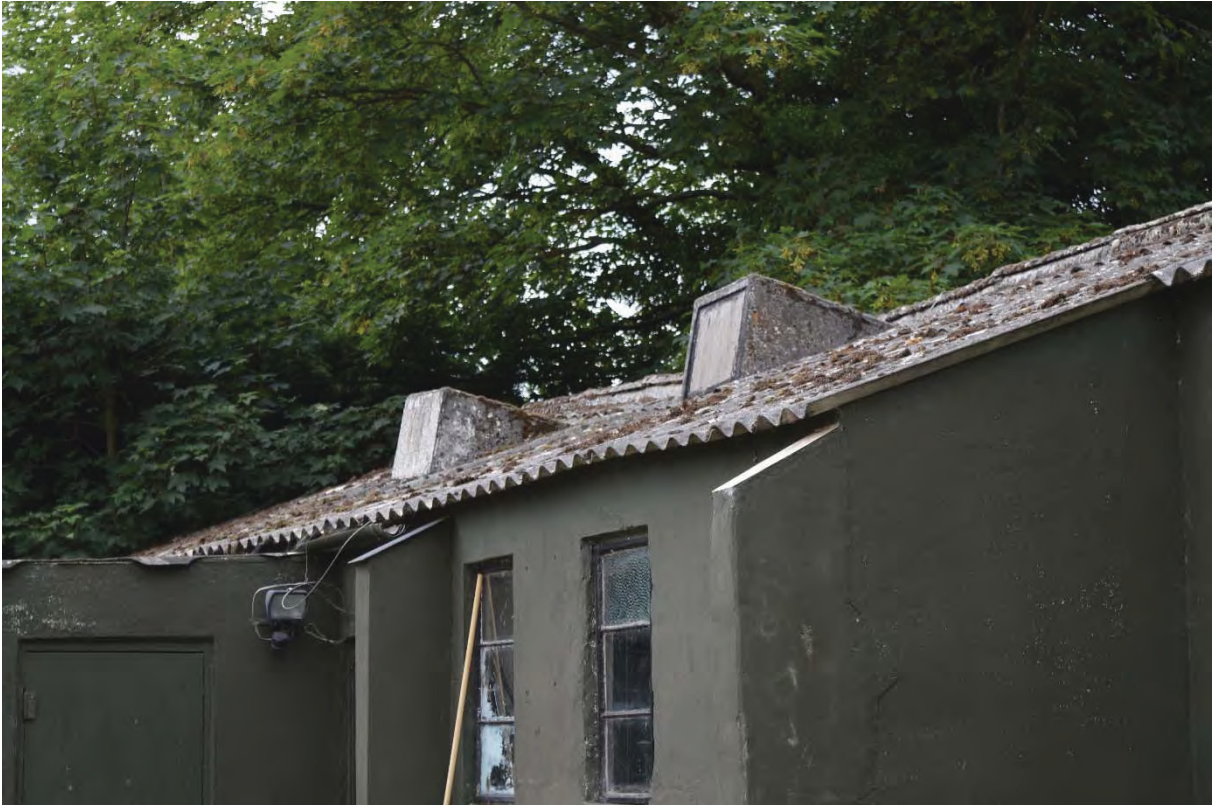
Plate 17 Roof vents to Building 2 (54)
