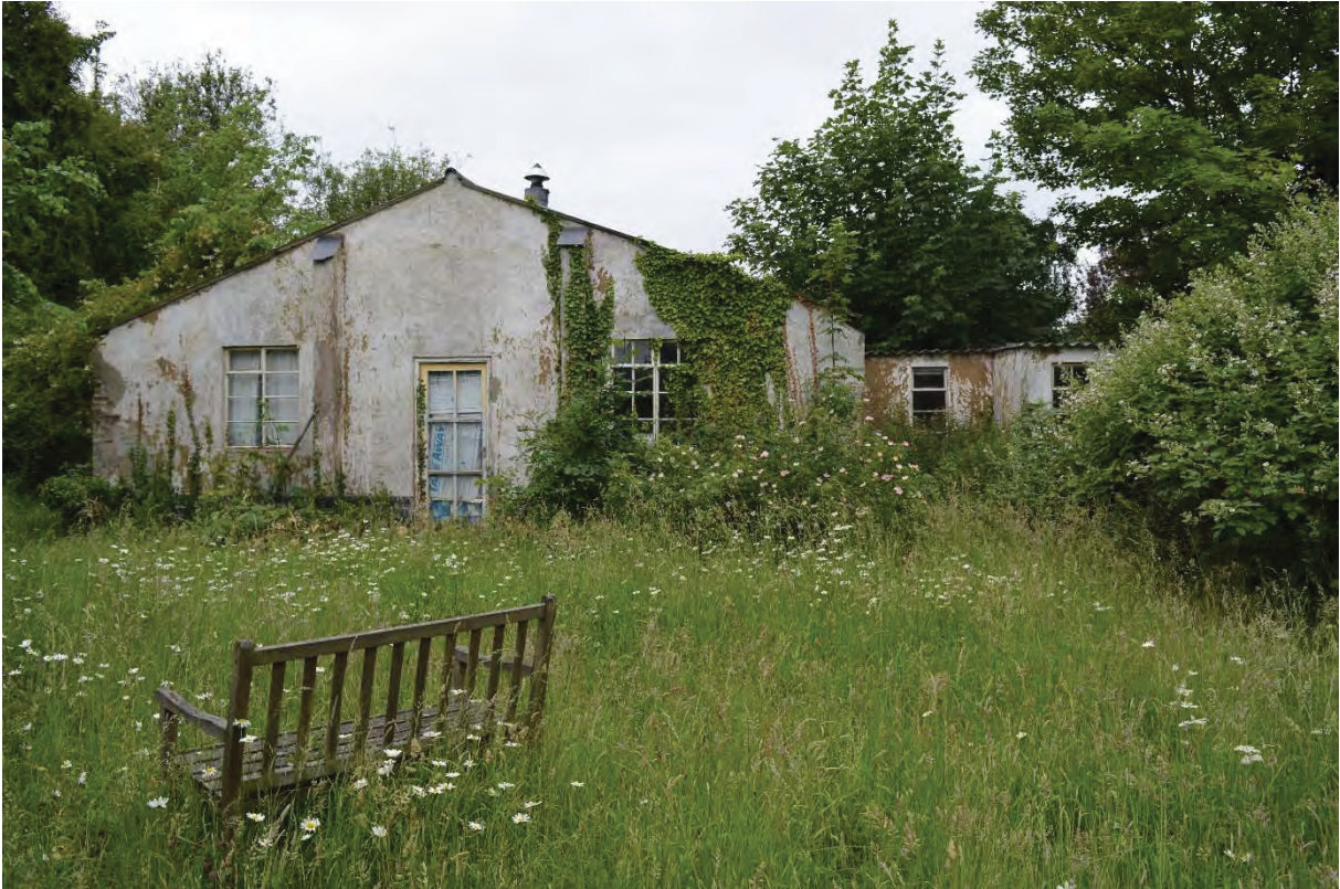
Plate 35 Building 4, looking south-west (92)
