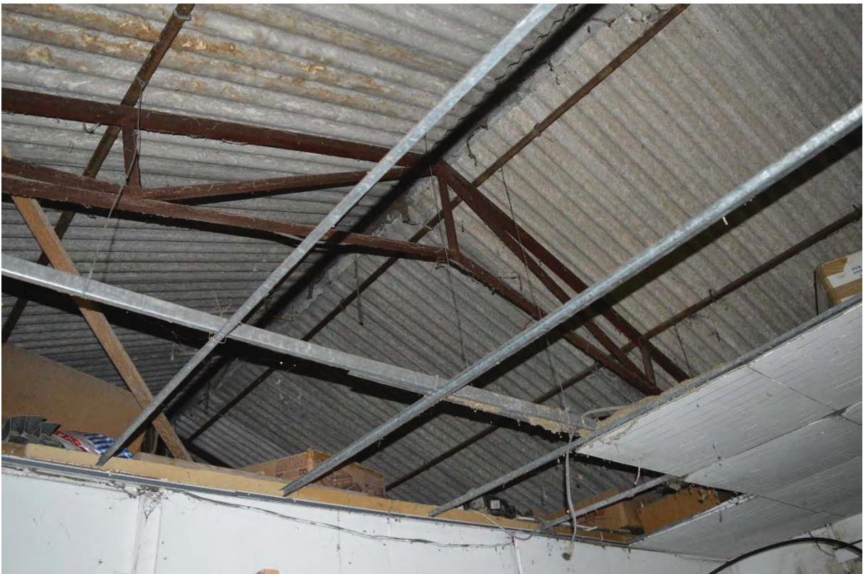
Plate 50 Roof to Building 5 (51)
