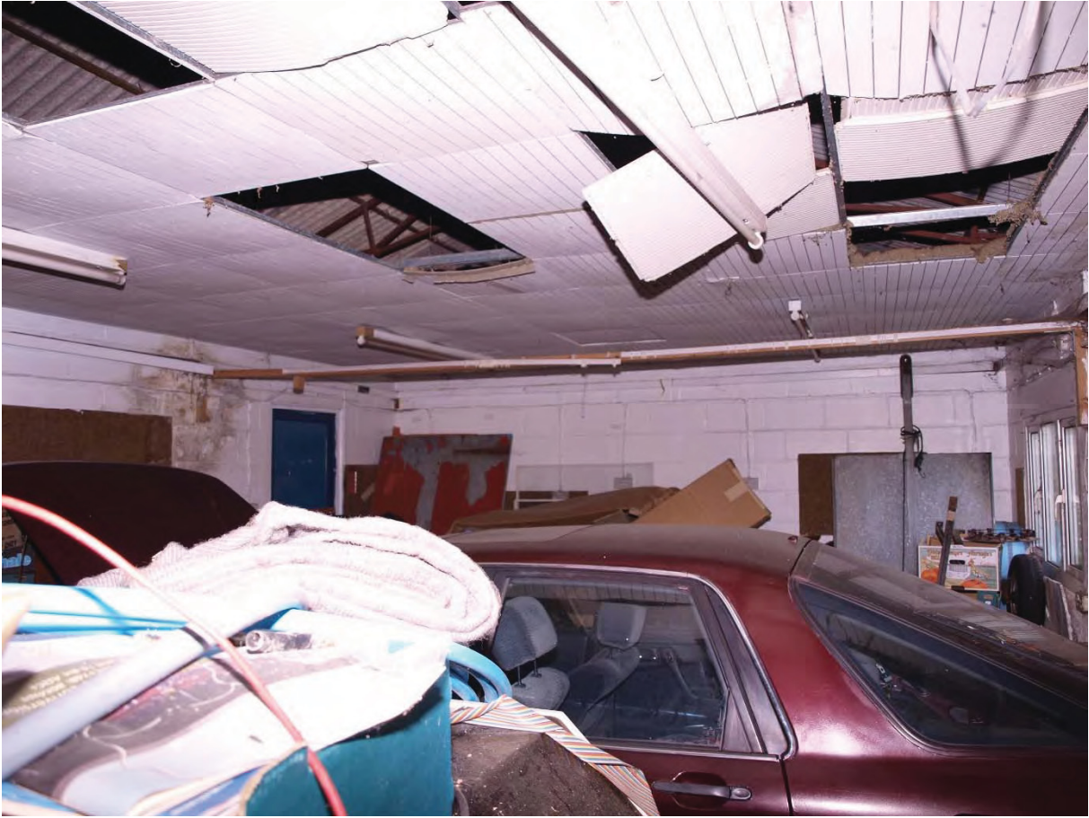
Plate 49 Interior of Building 5 (50)
