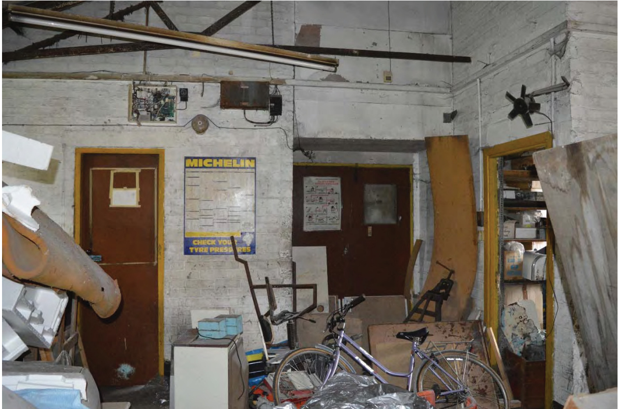
Plate 33 Building 3, Room 3, looking north-west (86)
