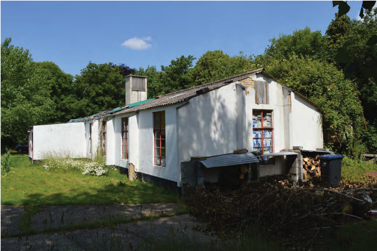
Plate 1 Building 1, looking north-west (10)
