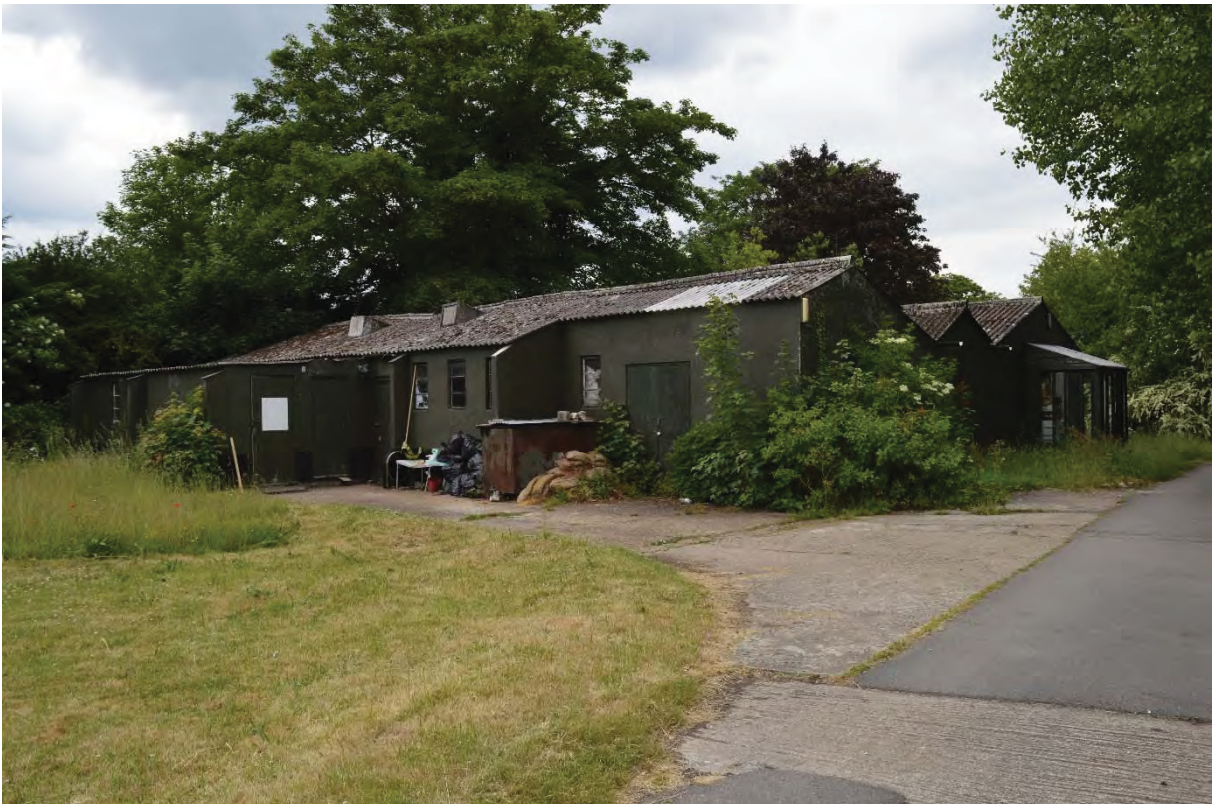
Plate 14 Building 2, looking south-west (53)
