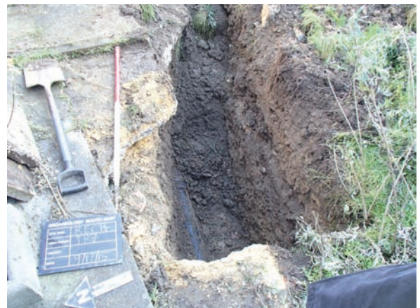
Trial pit 13 looking east
