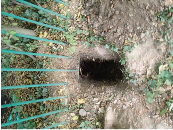
Trial pit 9 looking south
