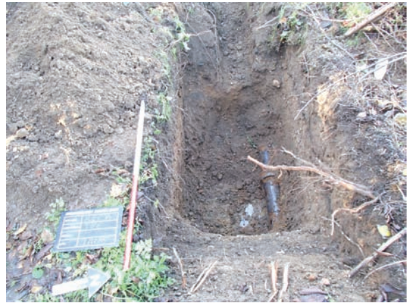
Trial pit 12 looking west
